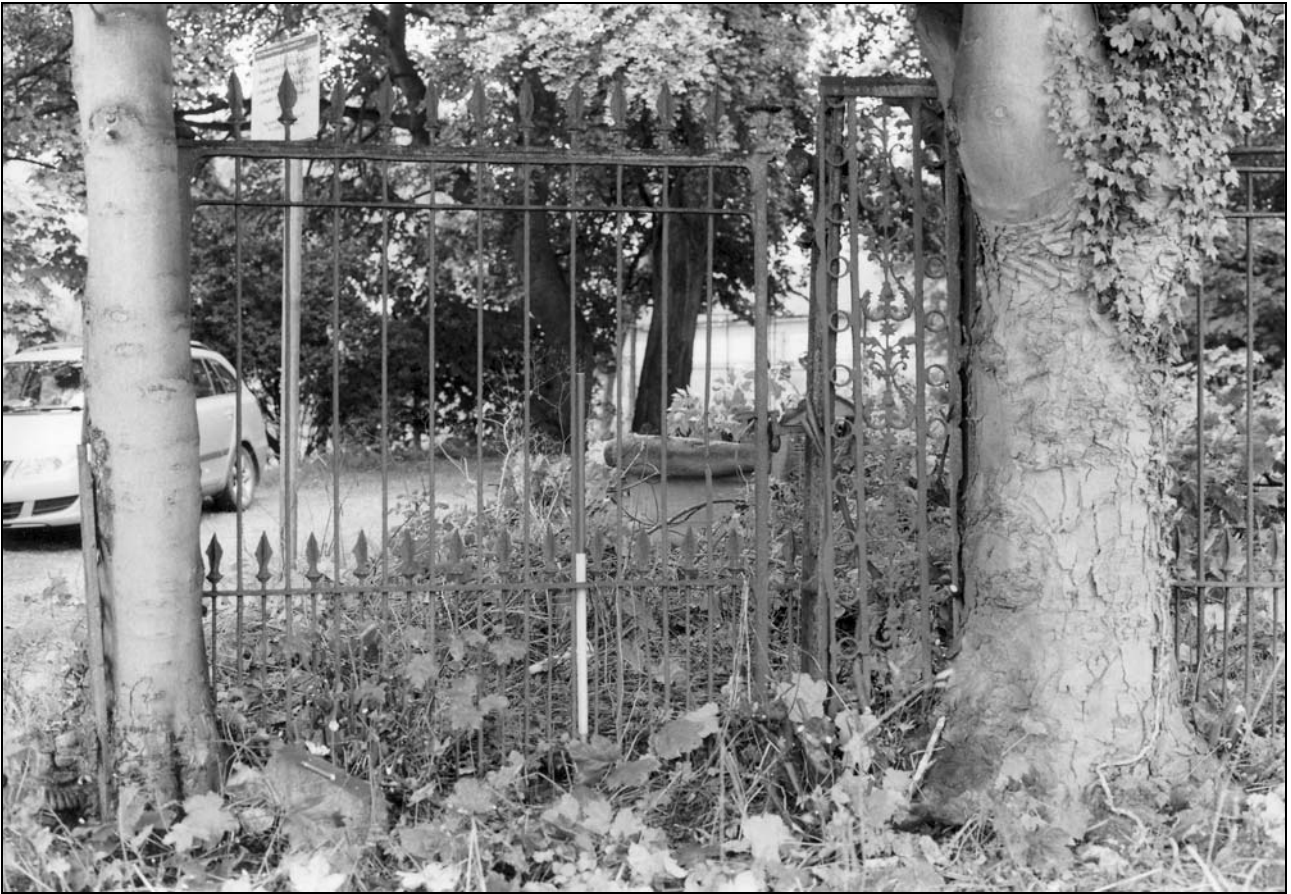
Photo 20: Pedestrian gate, looking west (film 1, frame 5)
