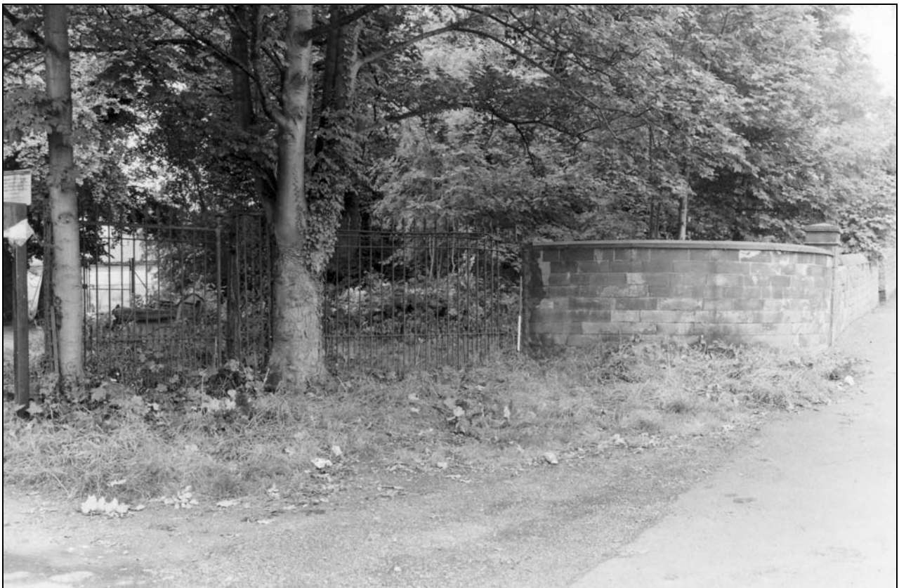
Photo 6: Surviving structures in north side of gateway, looking north-west (film 1, frame 1)
