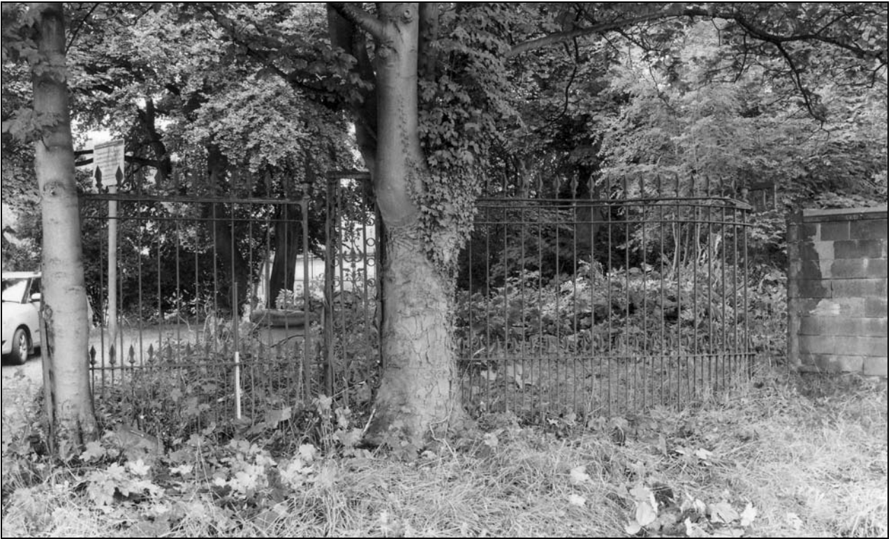
Photo 11: Surviving railings (right) and pedestrian gate (left), looking west (film 1, frame 6)
