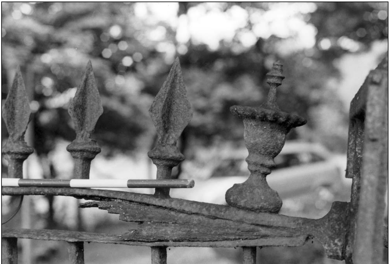
Photo 25: Detail of spearhead and urn finials on gate, looking west (film 2, frame 11)
