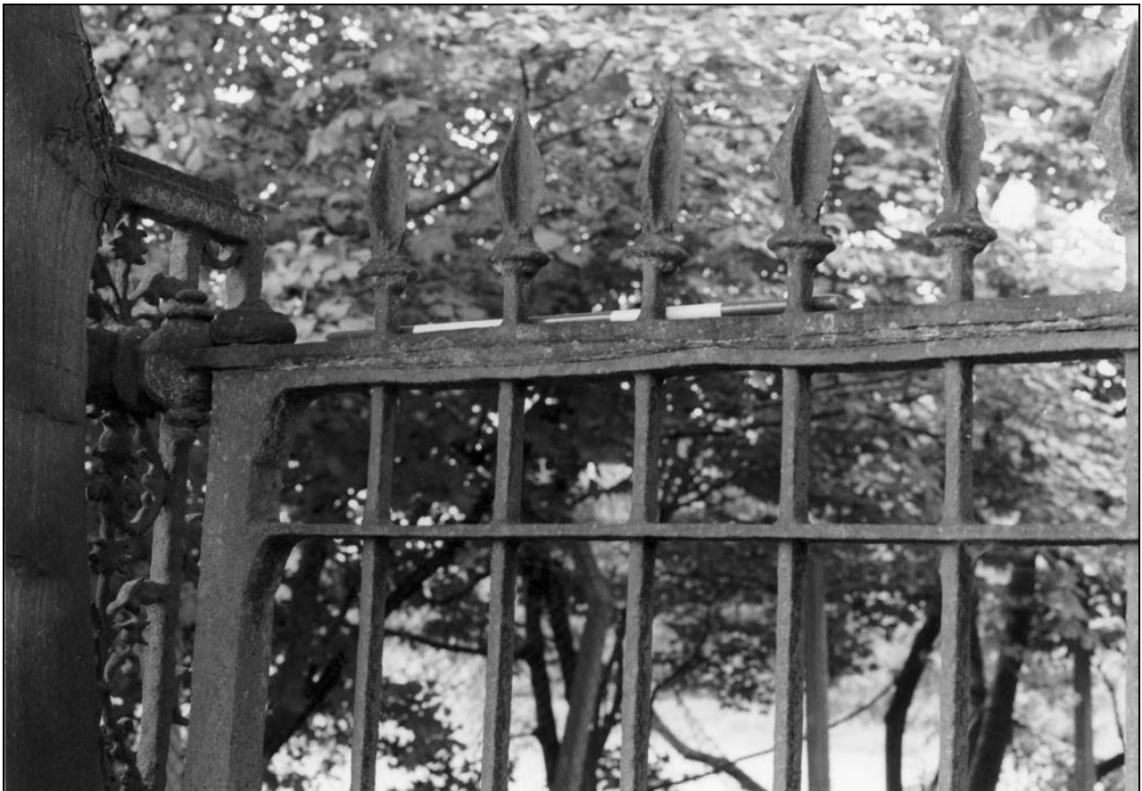
Photo 21: Detail of finials and hinge on gate, looking west (film 2, frame 7)
