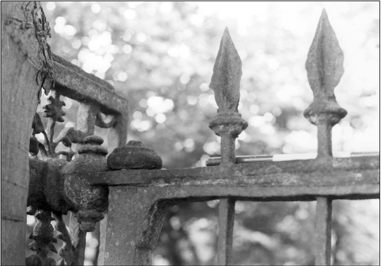
Photo 22: Detail of hinge on gate, looking west (film 2, frame 13)
