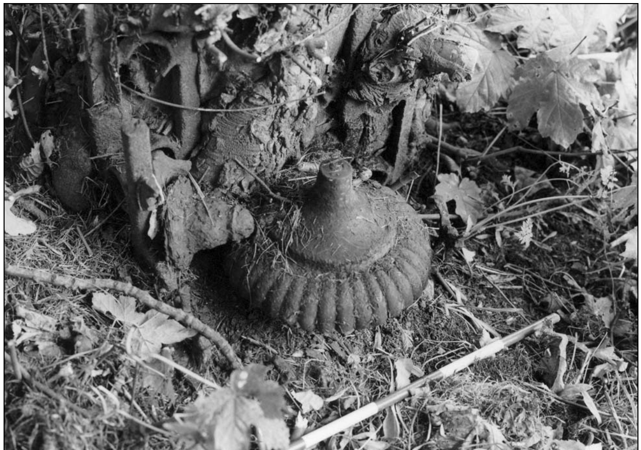
Photo 29: Cast iron fixture at foot of cross panel, perhaps hinge to former carriage gate (film 2, frame 5)
