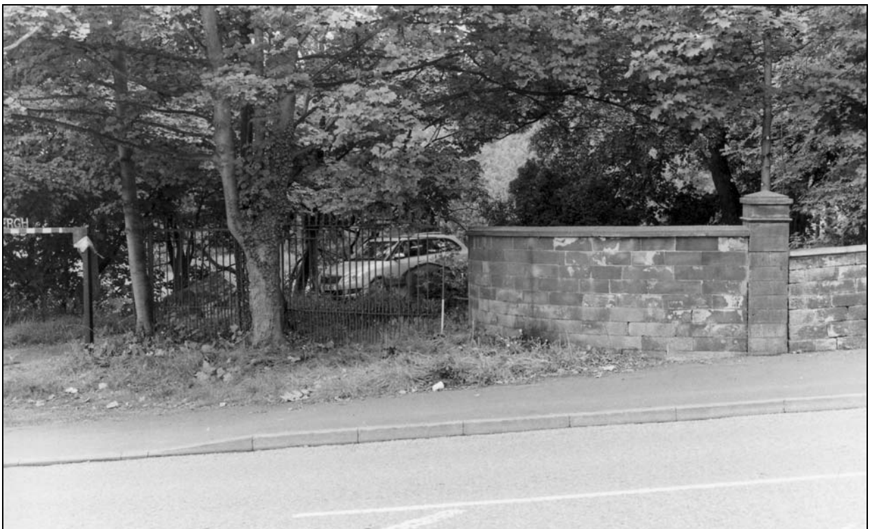
Photo 2: Surviving structures in north side of gateway, looking west (film 1, frame 4)
