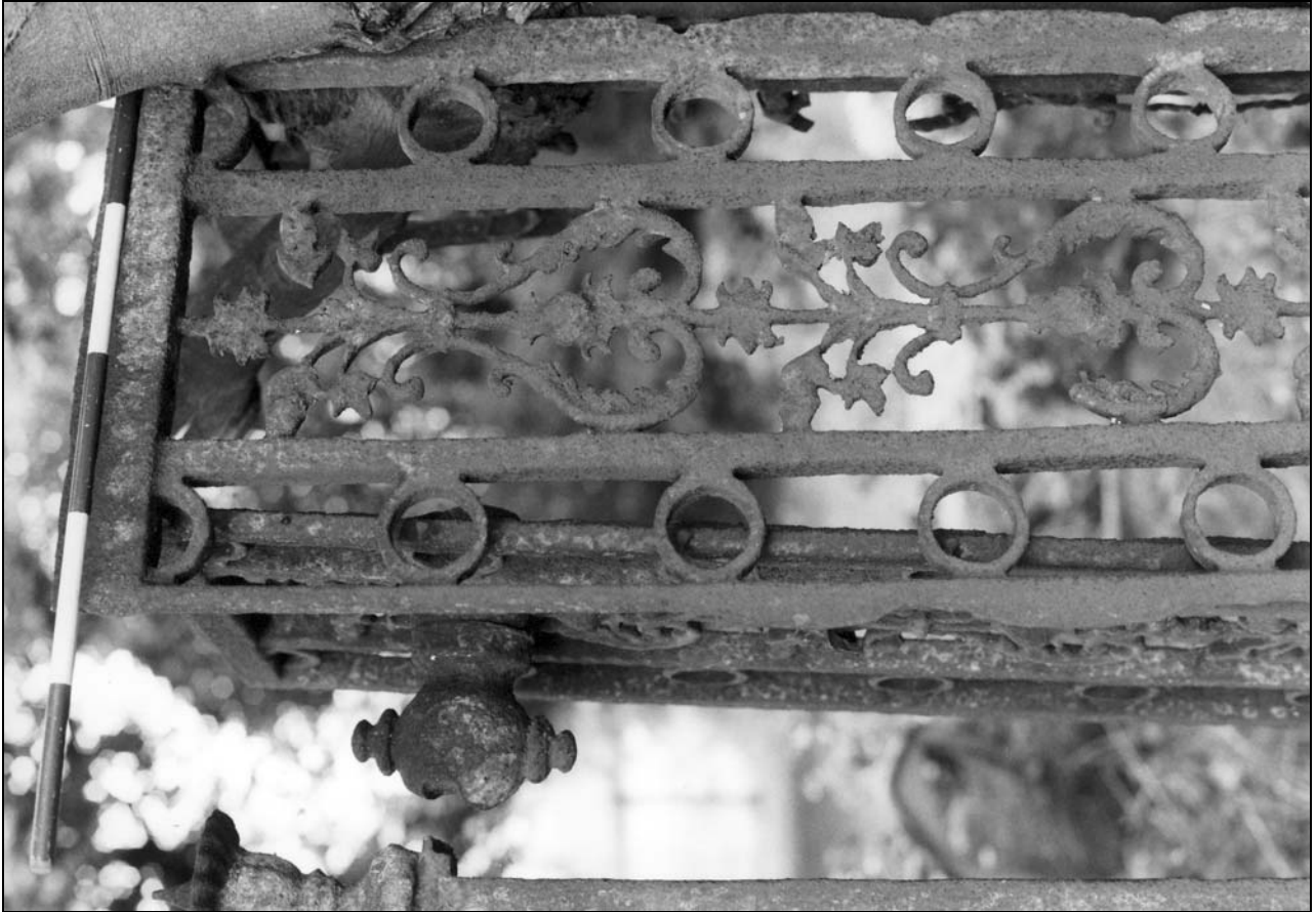
Photo 17: Detail of square pier between railings and pedestrian gate, looking north-west (film 2, frame 16)
