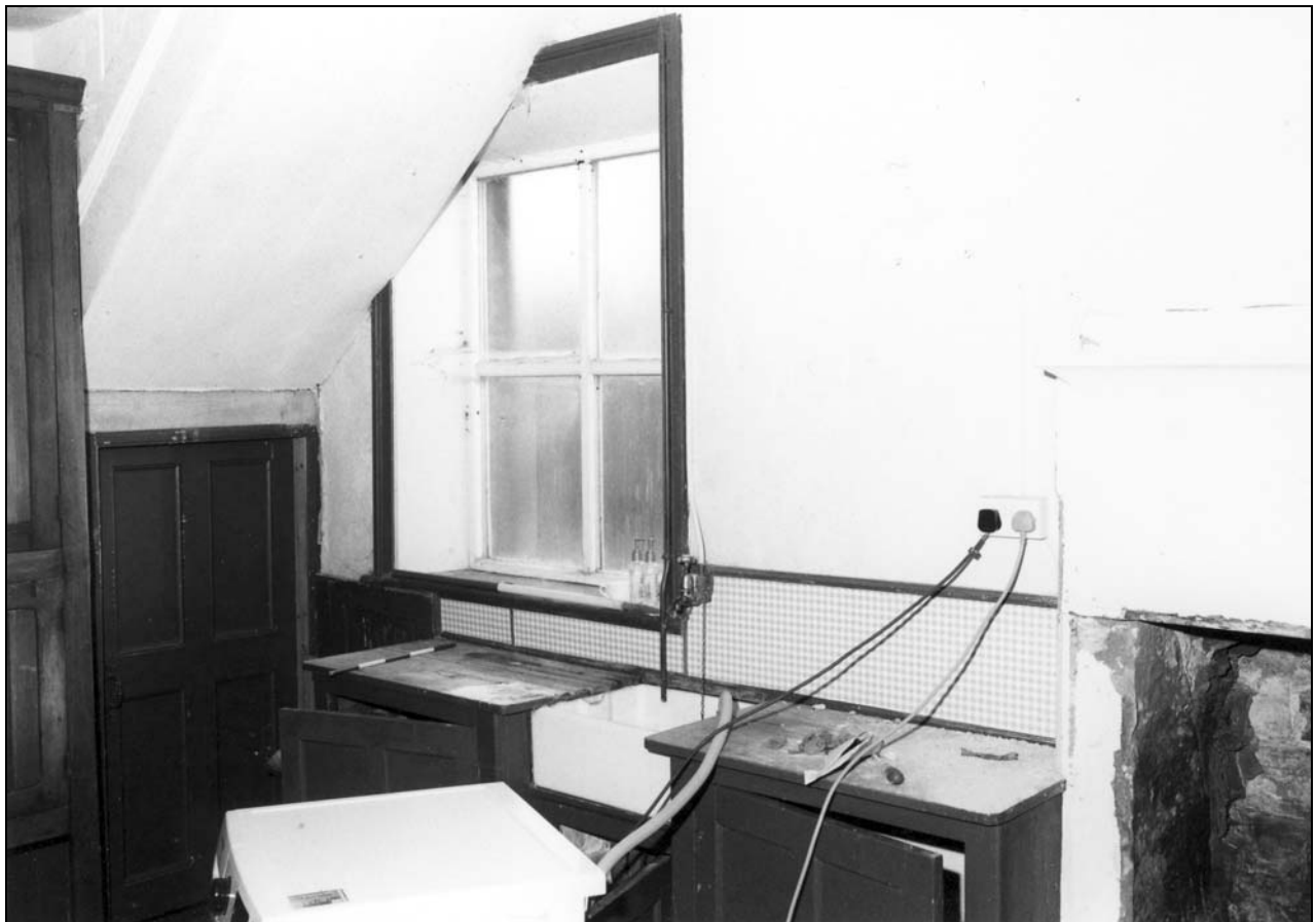
Photo 35: Present kitchen, looking south-west (film 4, frame 5)
