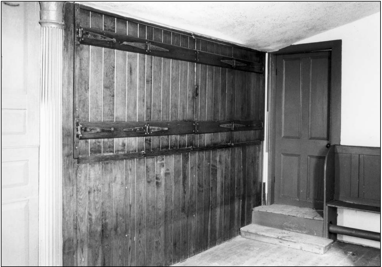
Photo 44: Main east room, looking north-west (film 1, frame 2)
