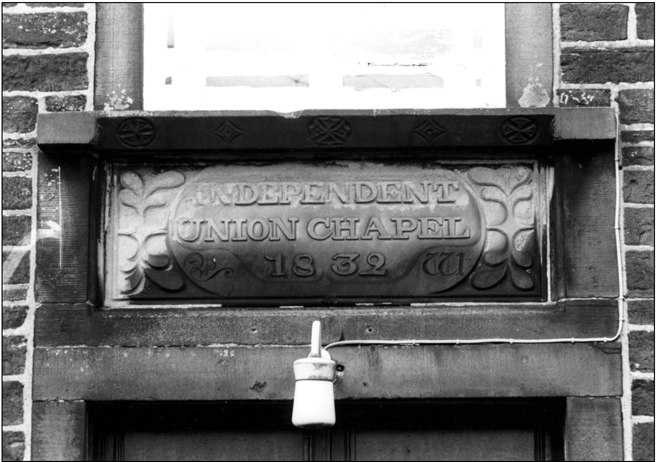
Photo 3: Detail of foundation stone over front doorway (film 4, frame 17)
