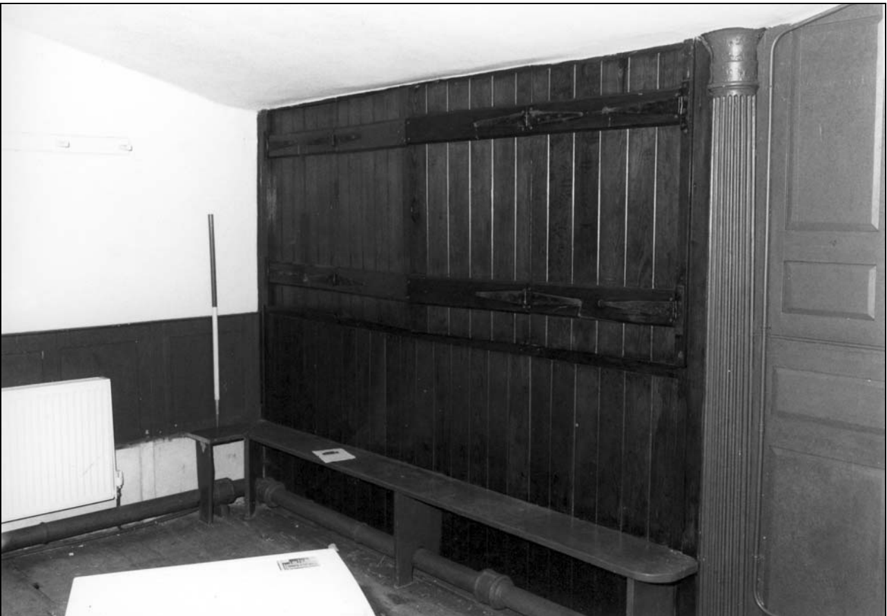
Photo 37: Present kitchen, looking north-east (film 4, frame 2)
