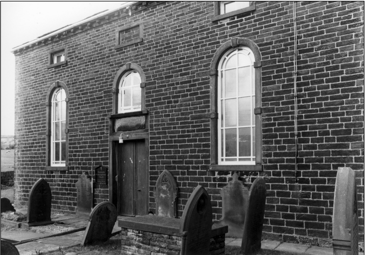
Photo 6: Front elevation, from the south-east (film 4, frame 11)
