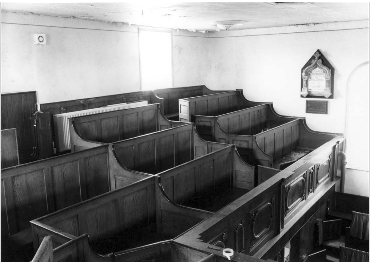
Photo 56: West side of gallery, looking north-west (film 3, frame 5)
