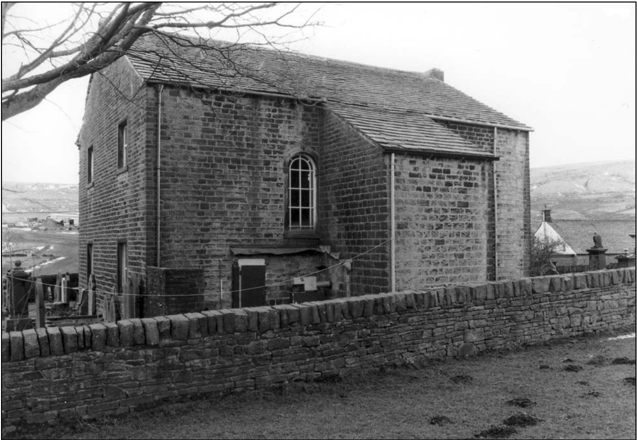
Photo 12: General view, from the north-east (film 5, frame 5)
