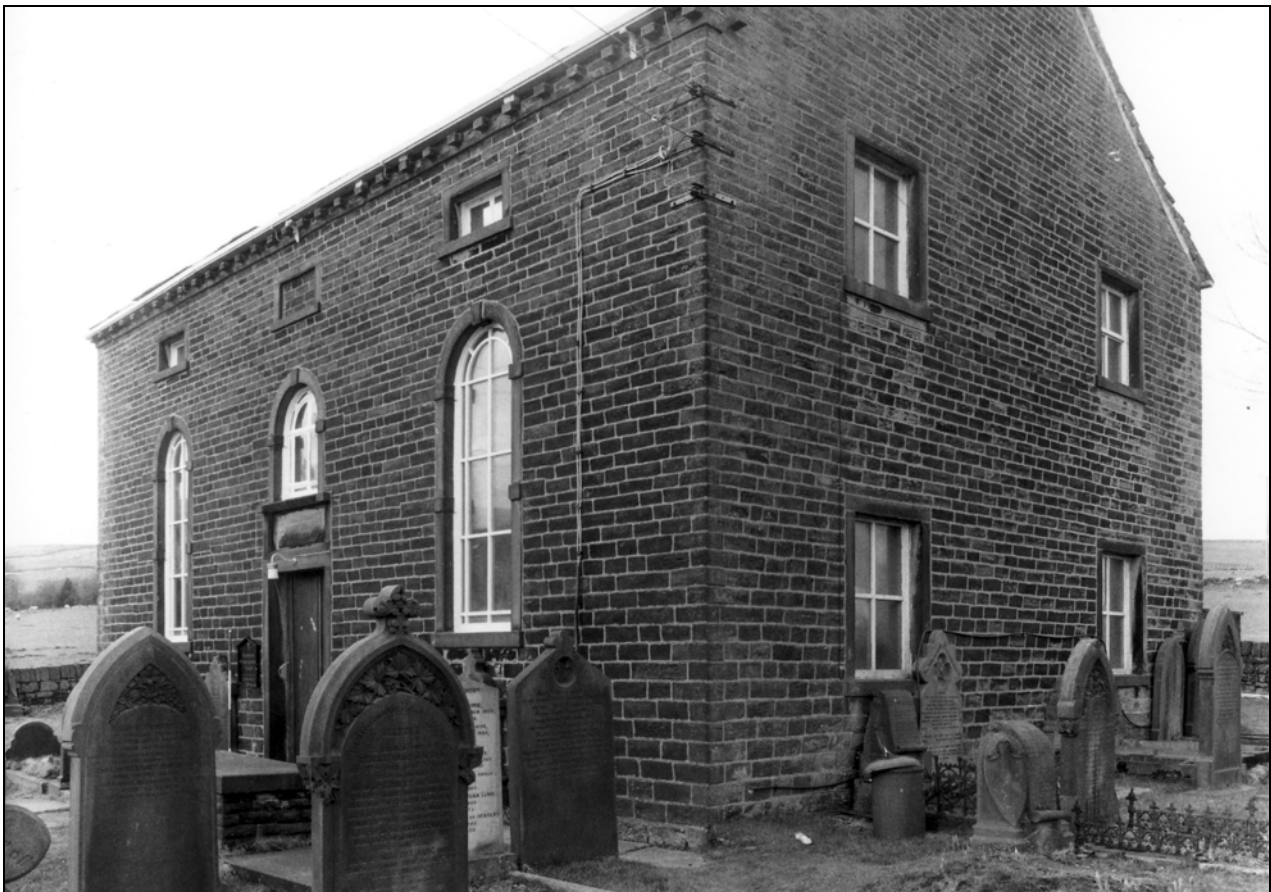
Photo 9: General view, from the south-east (film 4, frame 9)
