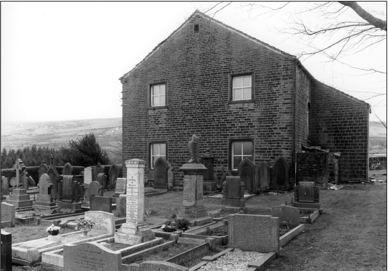
Photo 10: General view, from the north-east (film 5, frame 7)
