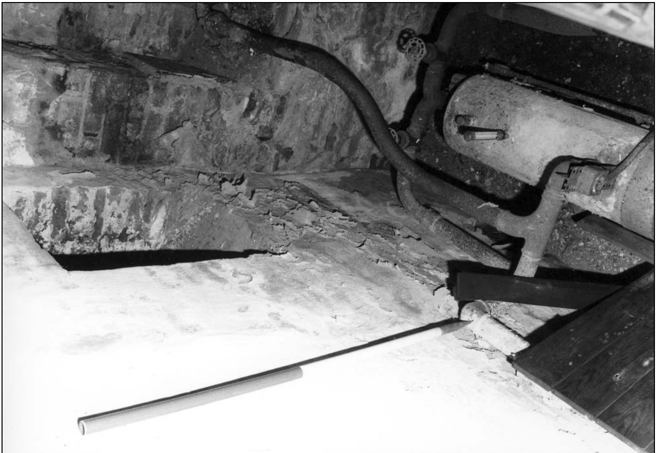
Photo 49: Boiler room with coal hole, looking east (film 1, frame 8)
