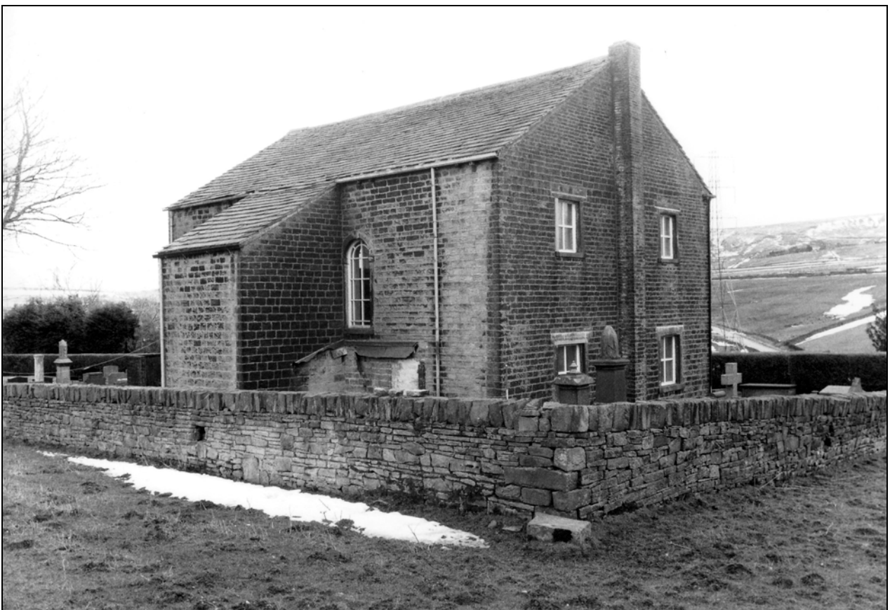
Photo 11: General view, from the north-west (film 5, frame 2)
