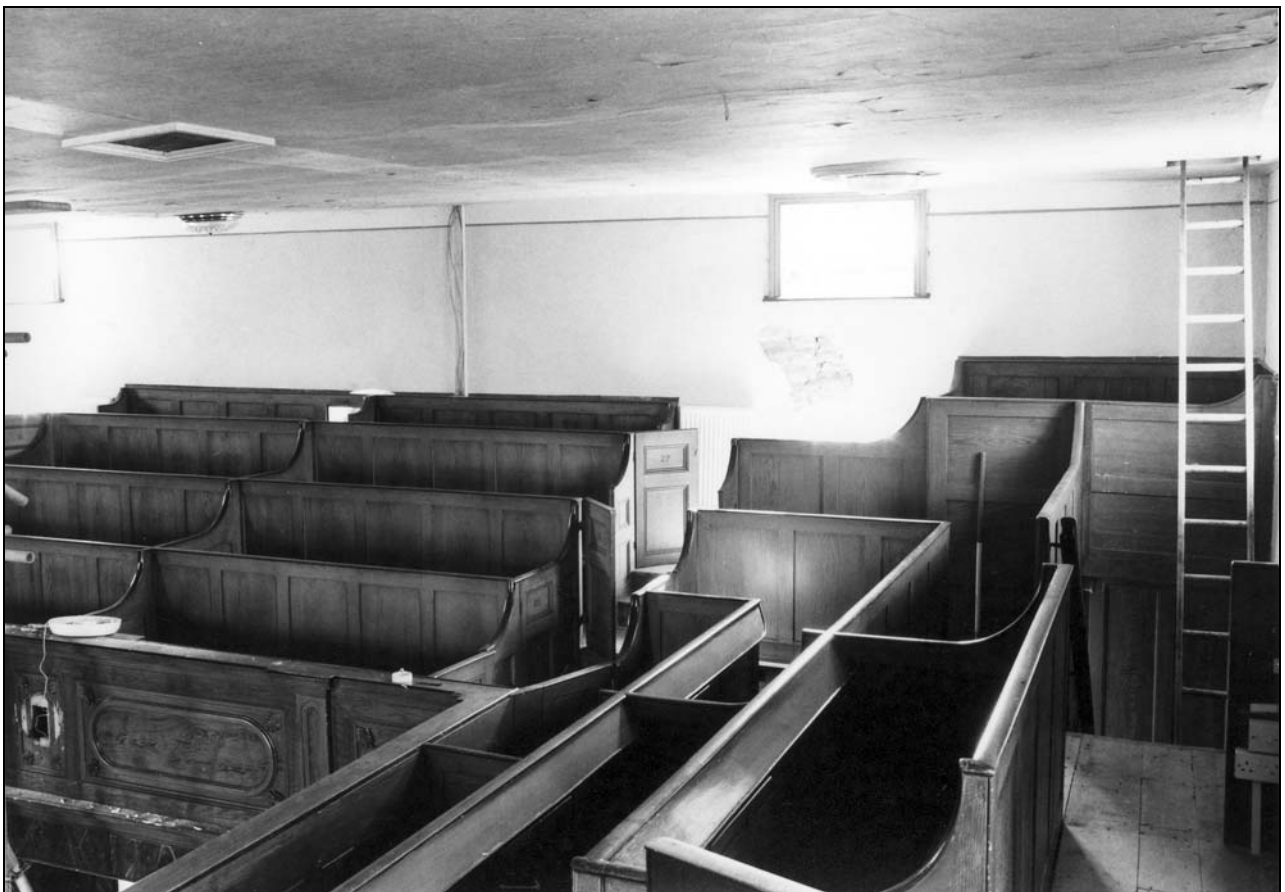
Photo 54: South side of gallery, looking south-east (film 3, frame 8)
