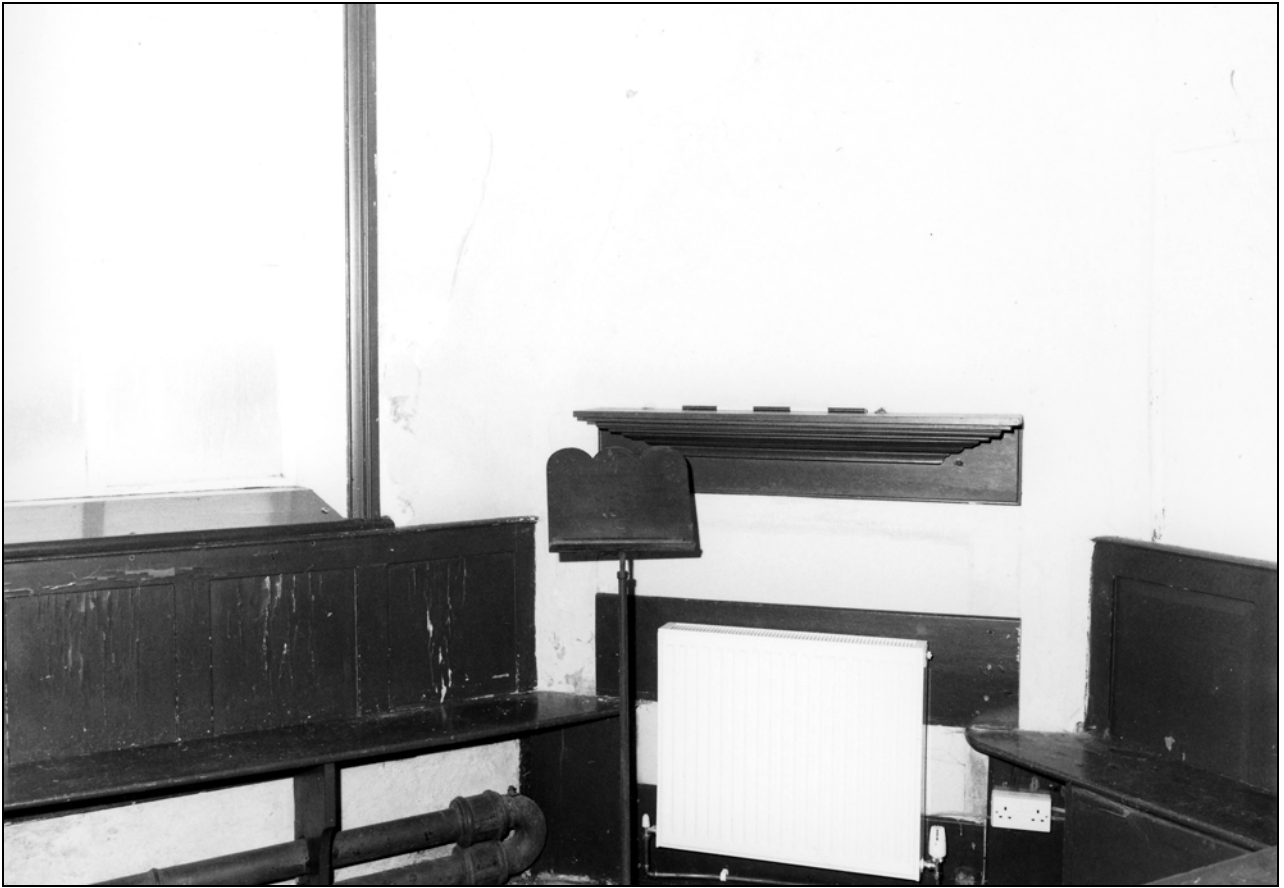
Photo 42: North-west room, looking north-west (film 1, frame 9)
