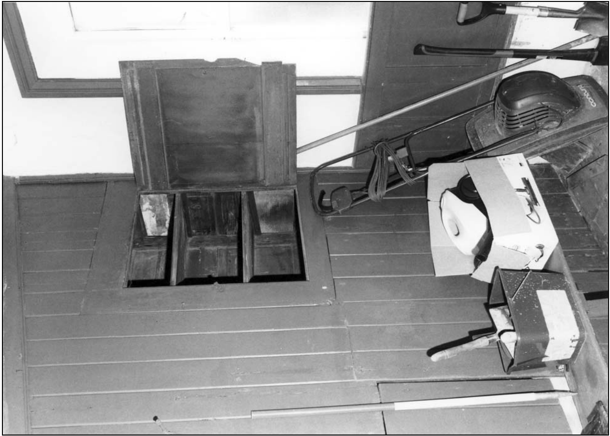
Photo 48: Small north-east room, looking north-east (film 1, frame 7)
