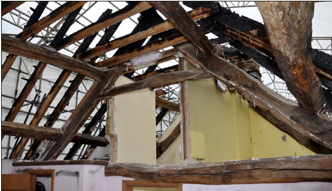
Photo 1: West face (upper face) of west truss
