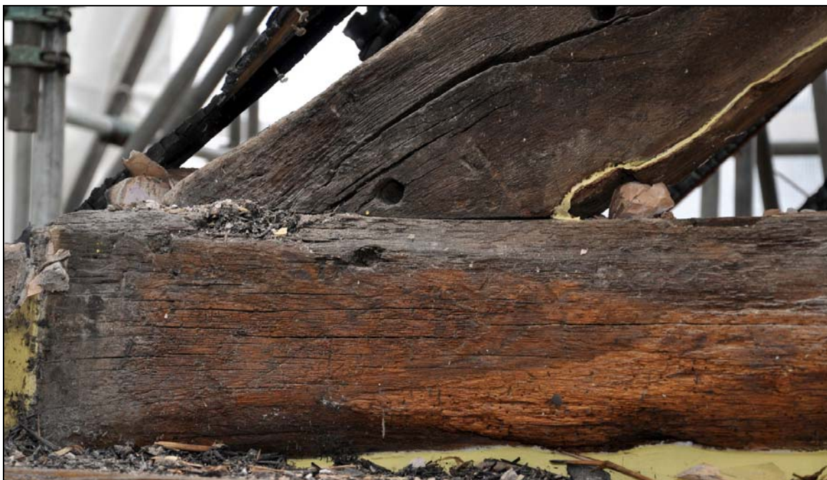
Photo 2: Detail of pegs and numbering on west truss
