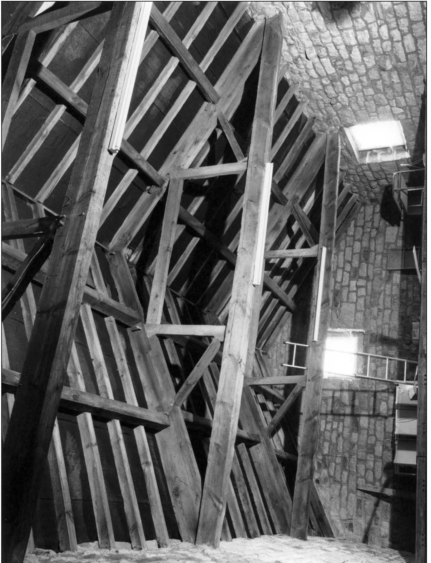
Photo 20: Barn interior: roof trusses, looking north (film 1, frame 7)
