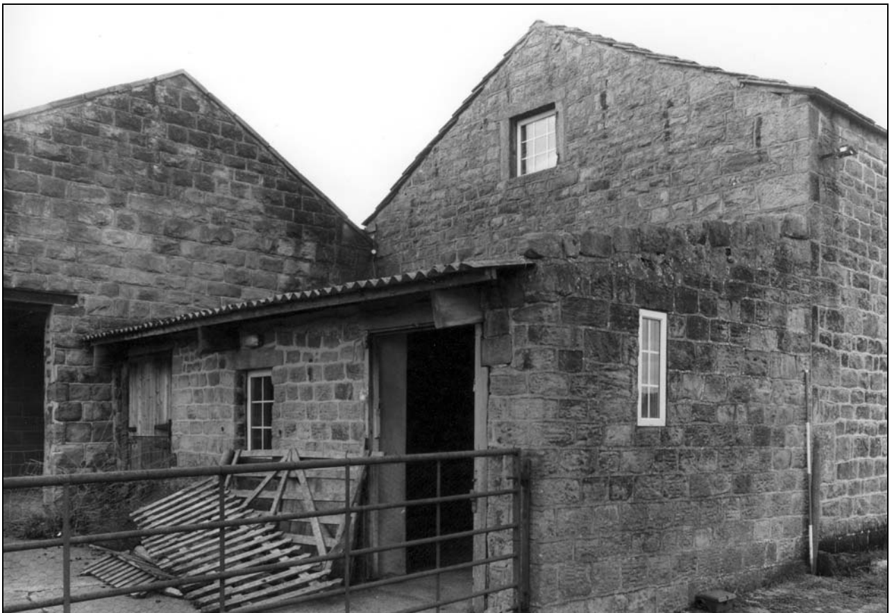
Photo 9: Modern lean-to at south-east gable of barn, looking west (film 2, frame 5)
