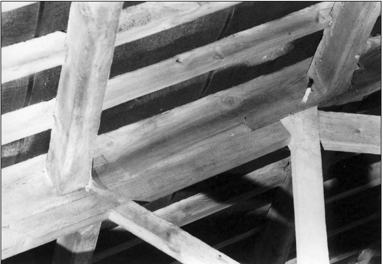
Photo 19: Barn interior: detail of roof truss (film 1, frame 8)
