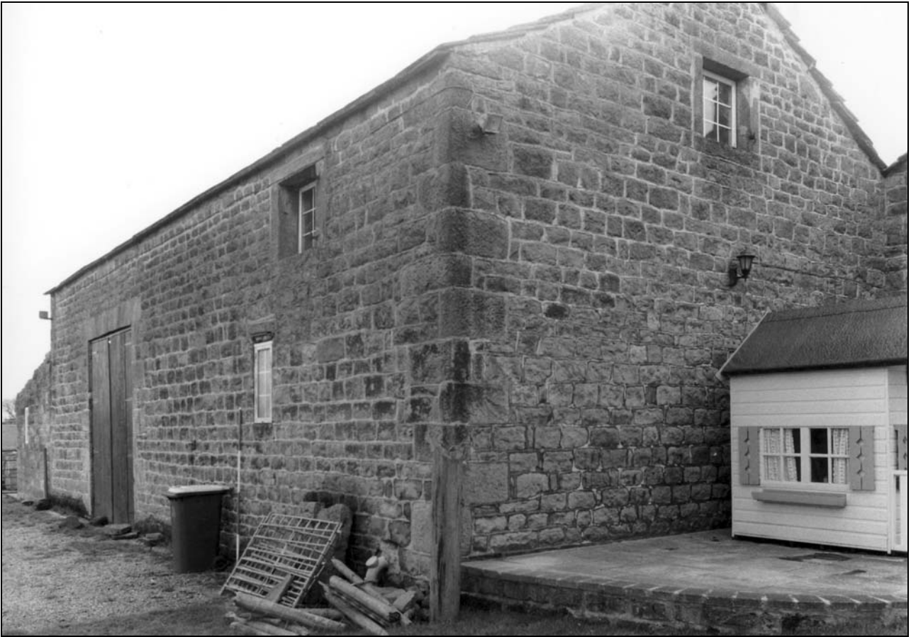
Photo 8: View of the rear of the barn, looking south (film 2, frame 1)
