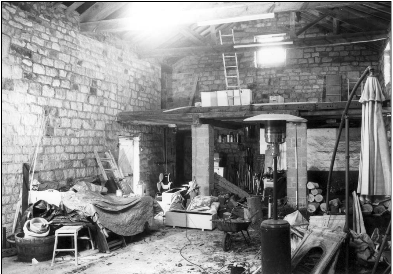
Photo 15: Barn interior: west corner (film 1, frame 2)
