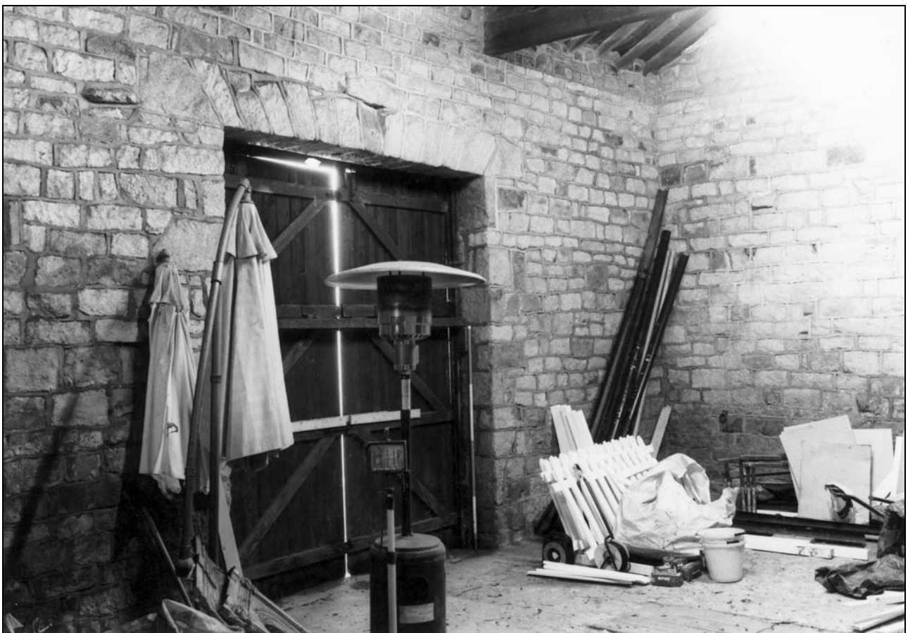
Photo 13: Barn interior: east corner (film 1, frame 5)
