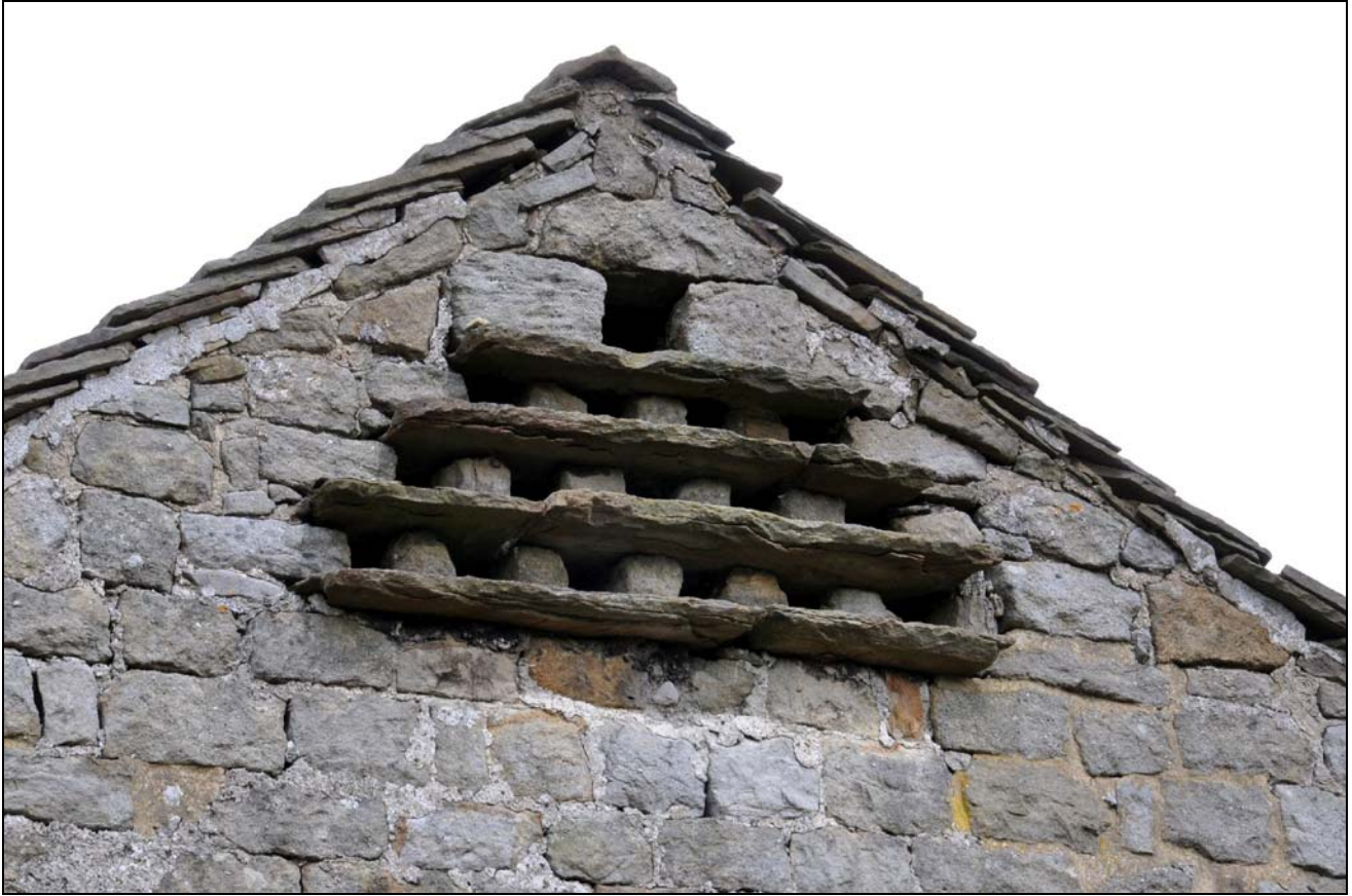
Photo 18: Detail of pigeon loft in south gable
