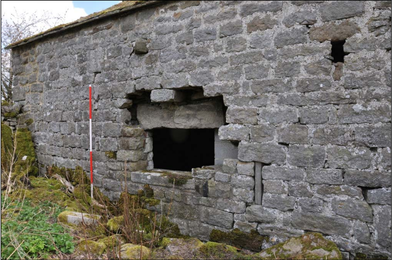
Photo 13: Present window (former doorway) in west elevation, with adjacent breathers
