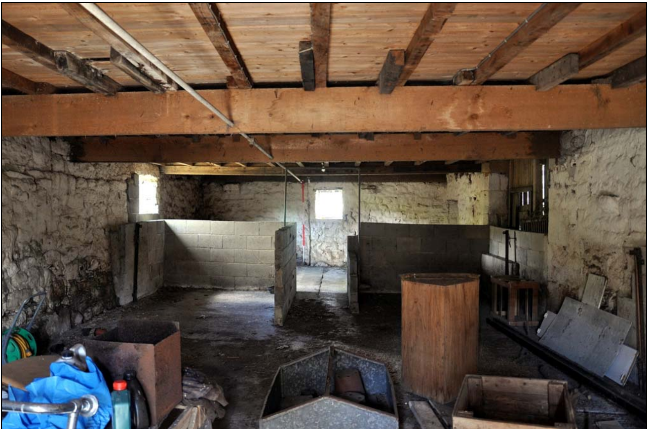
Photo 19: Interior: ground floor, from the south
