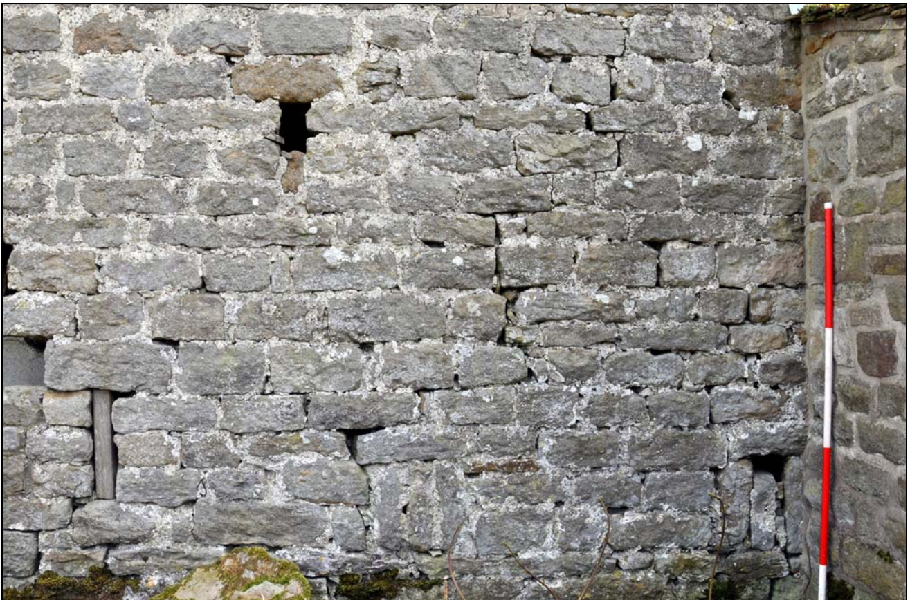
Photo 14: Detail of breathers in west elevation (two types)
