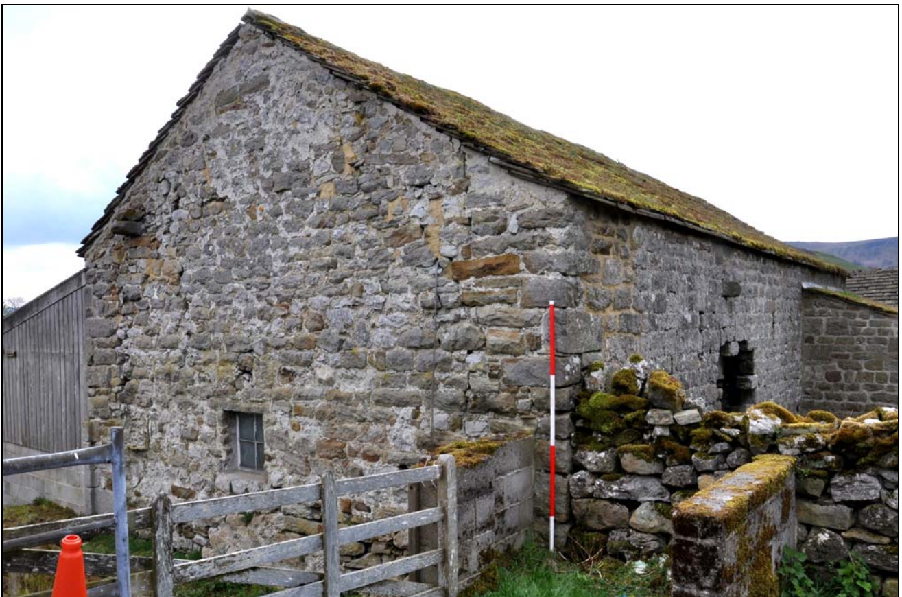
Photo 11: North gable (former internal wall), from the north-west
