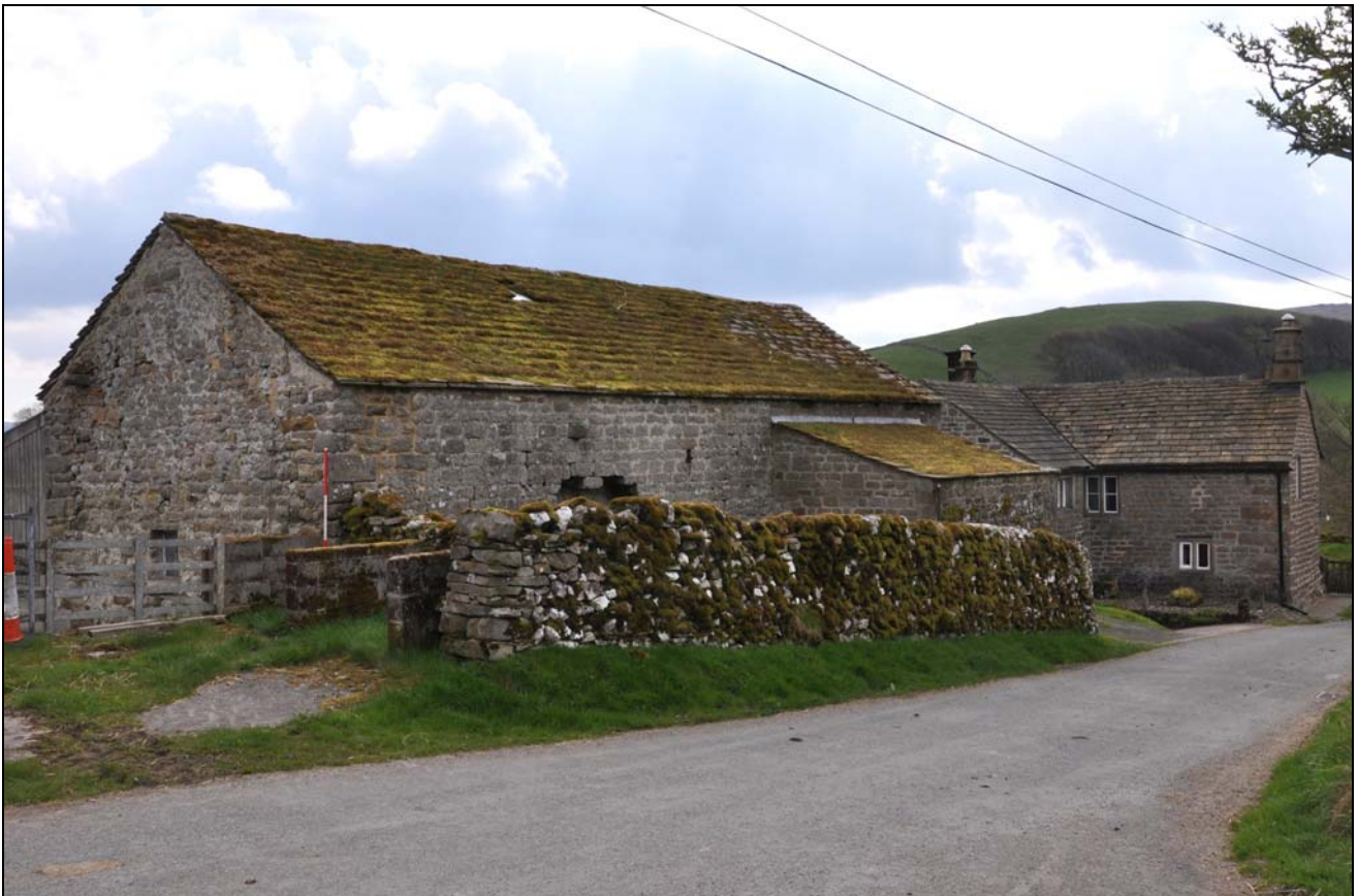
Photo 2: General view of the barn, from the north-west
