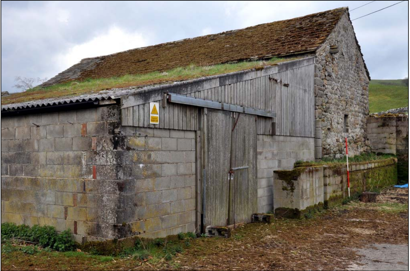
Photo 1: General view of the barn, from the north-east
