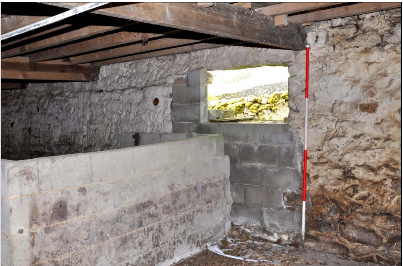
Photo 25: Interior: former doorway in west wall
