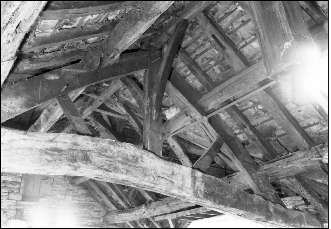
Photo 41: South truss, looking south-west (film 3, frame 18)
