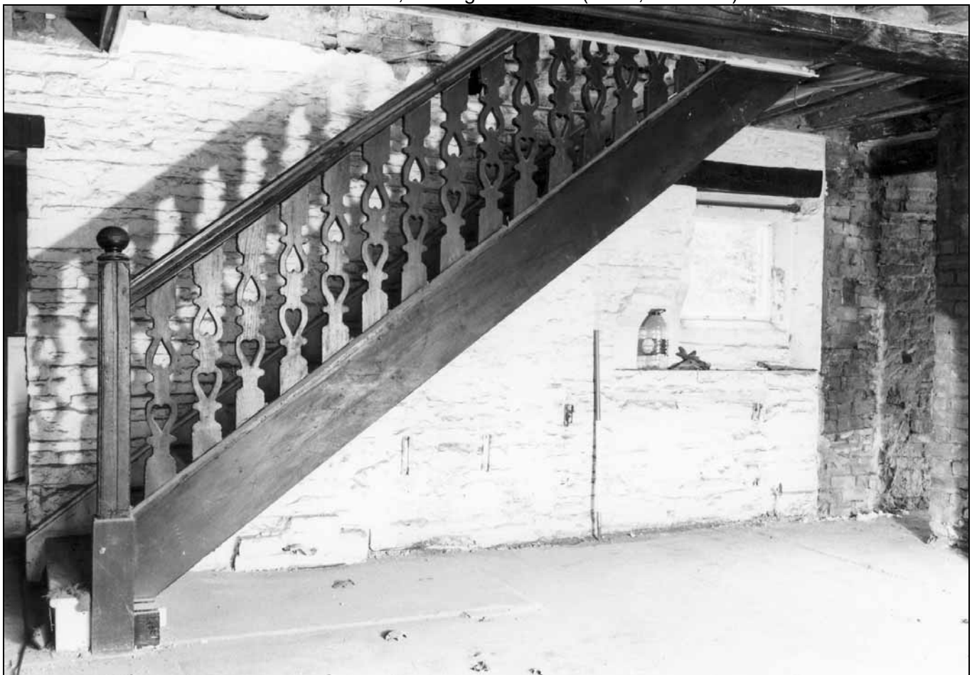
Photo 24: Kitchen, looking north-west, with re-sited/rebuilt stair, and fire window below (film 1, frame 12)
