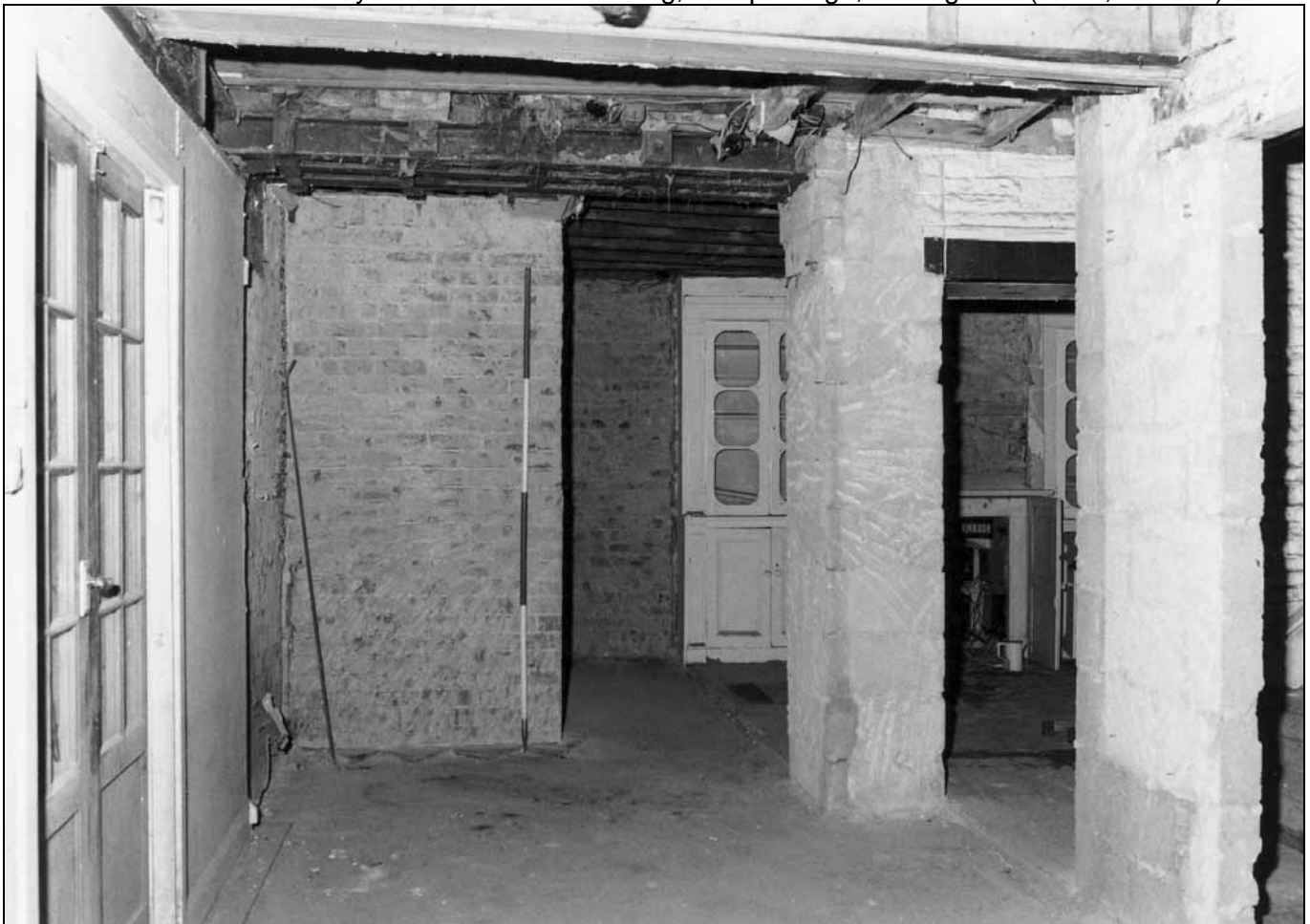
Photo 15: Passage in east wing, looking west (film 1, frame 10)
