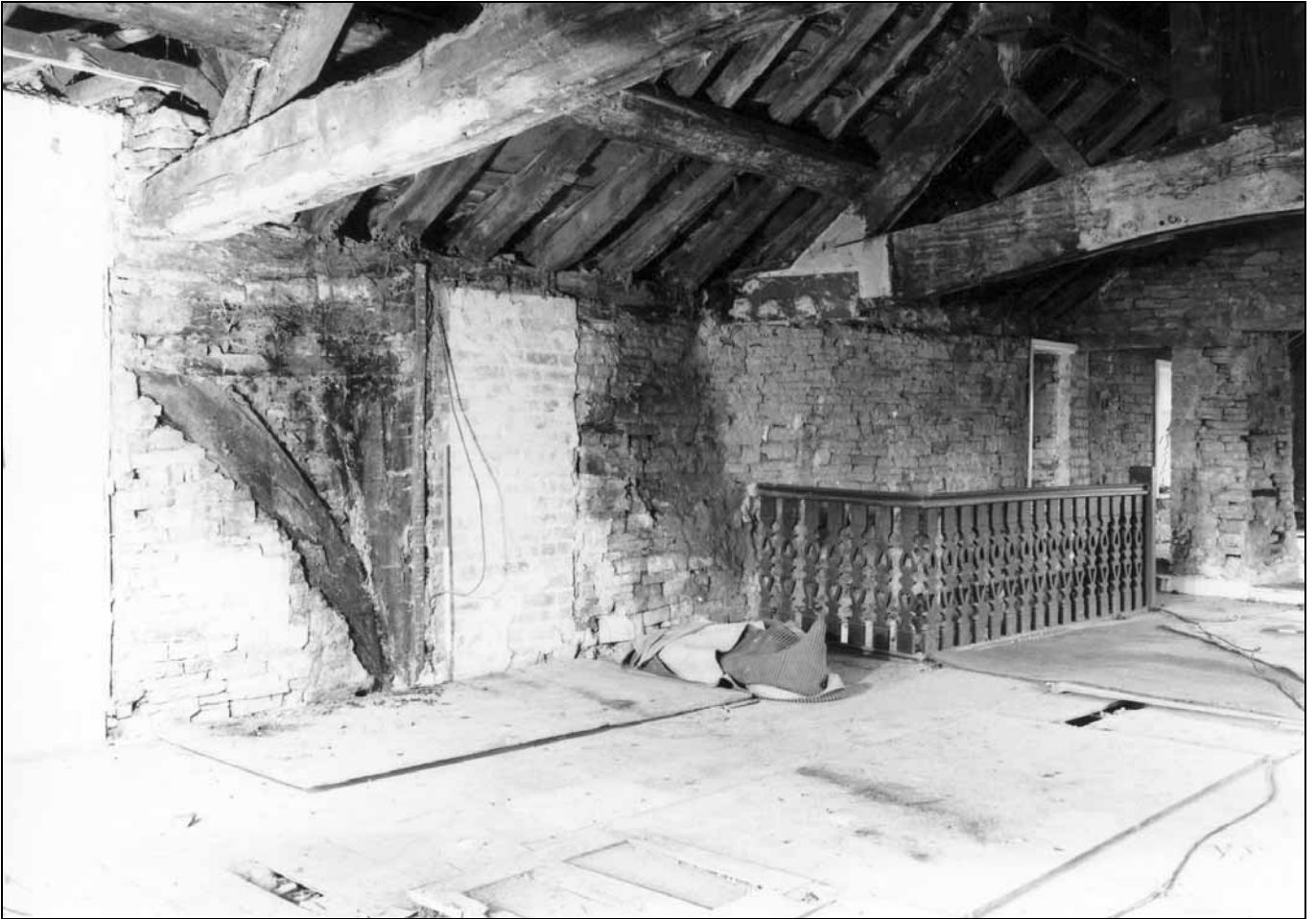
Photo 31: First floor, looking north-west, with arcade post and arch brace visible (film 3, frame 12)
