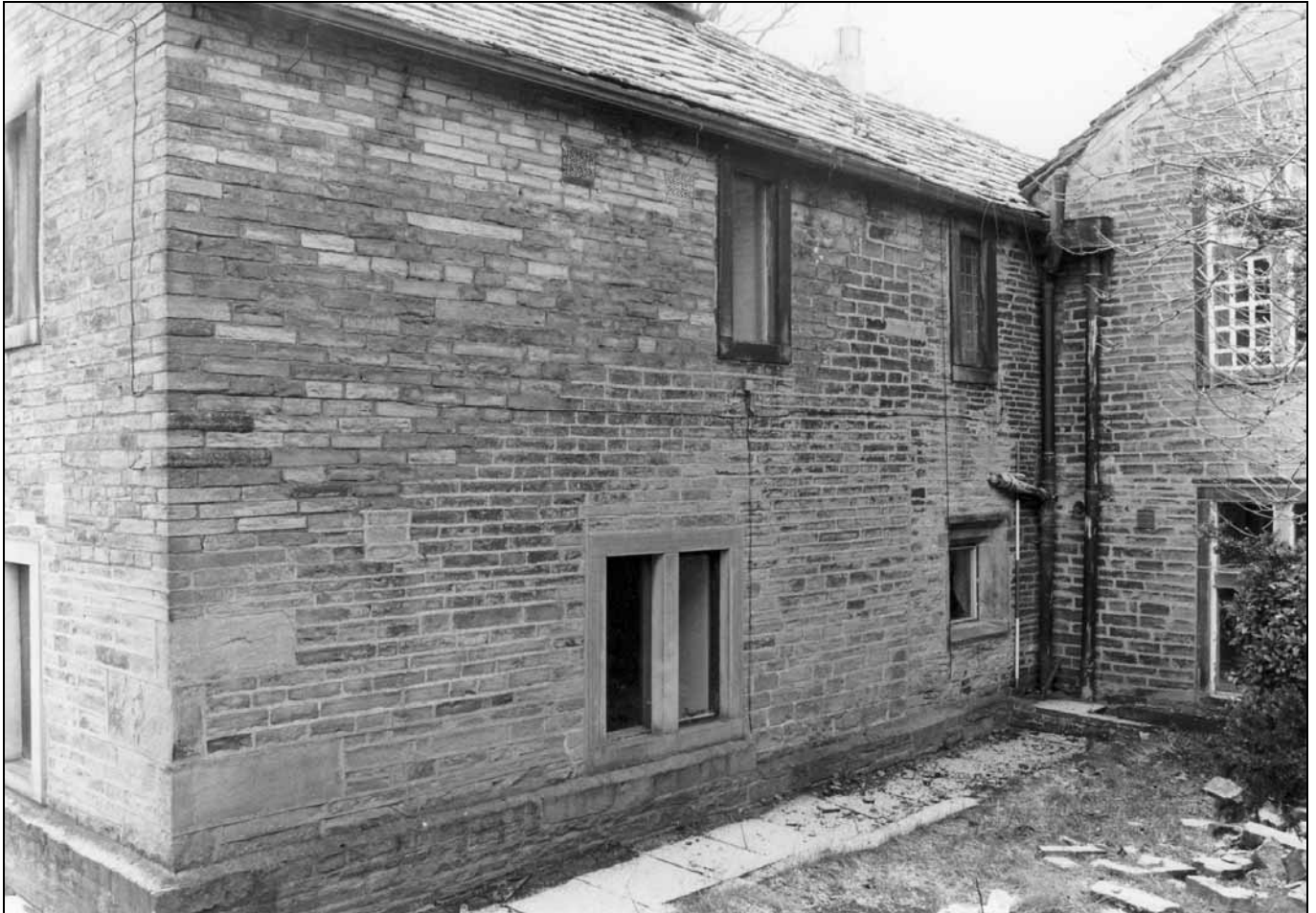
Photo 8: East wing, looking south-east, with 18th/19th century extension in foreground (earlier fire window at lower right) (film 2, frame 11)
