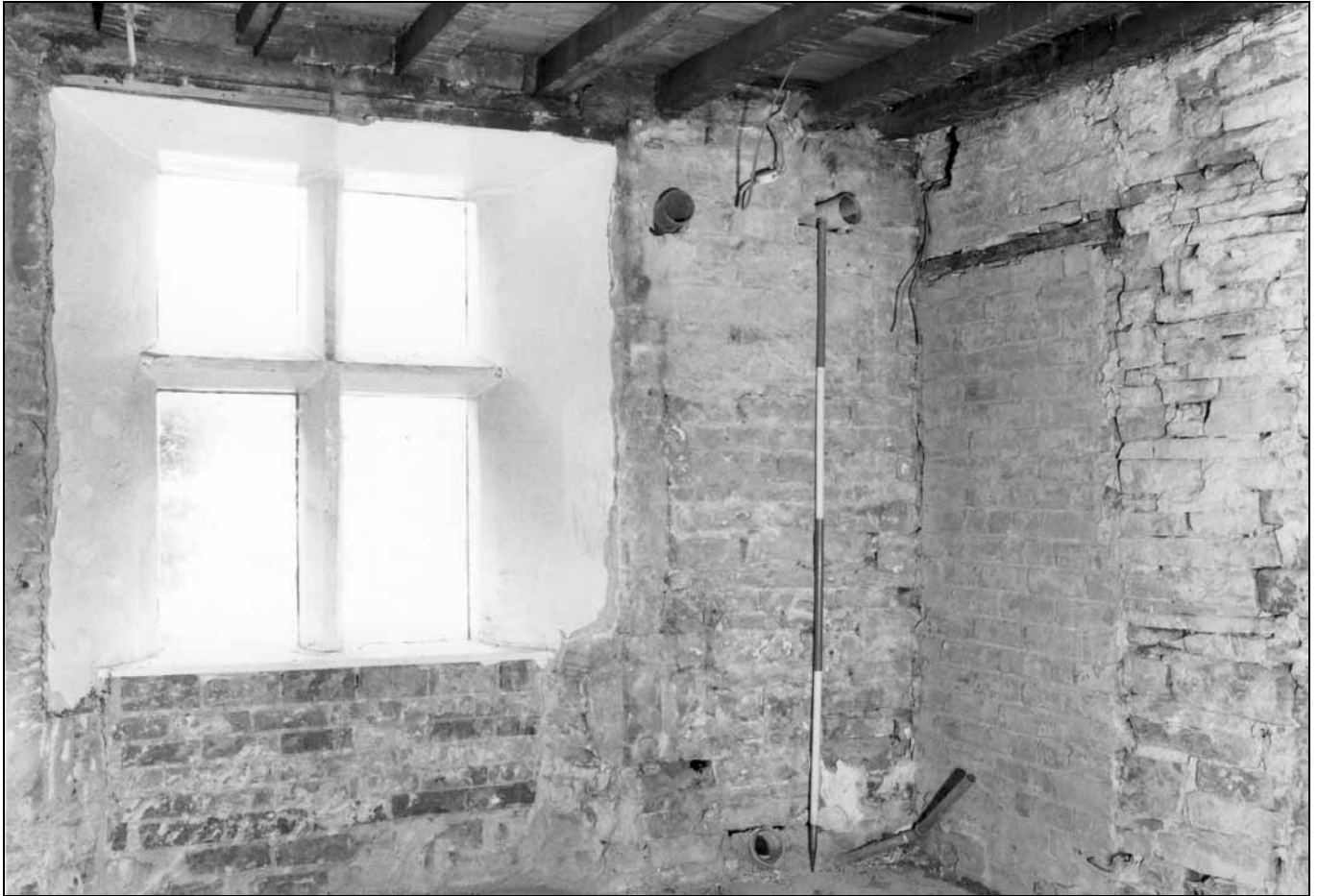
Photo 27: Ground floor room to rear of housebody, looking north-east (film 2, frame 17)
