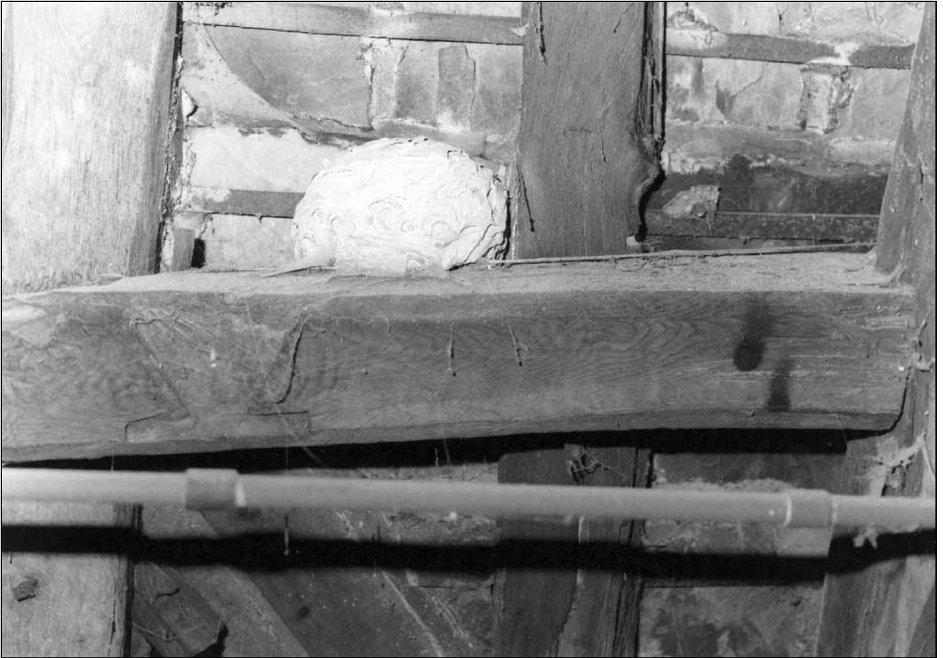
Photo 48: Candle soot marks on purlin, next to south truss, looking west (film 4, frame 8)
