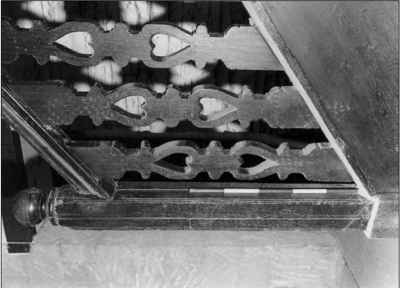
Photo 25: Detail of historic newel and handrail, and later balusters (film 4, frame 5)
