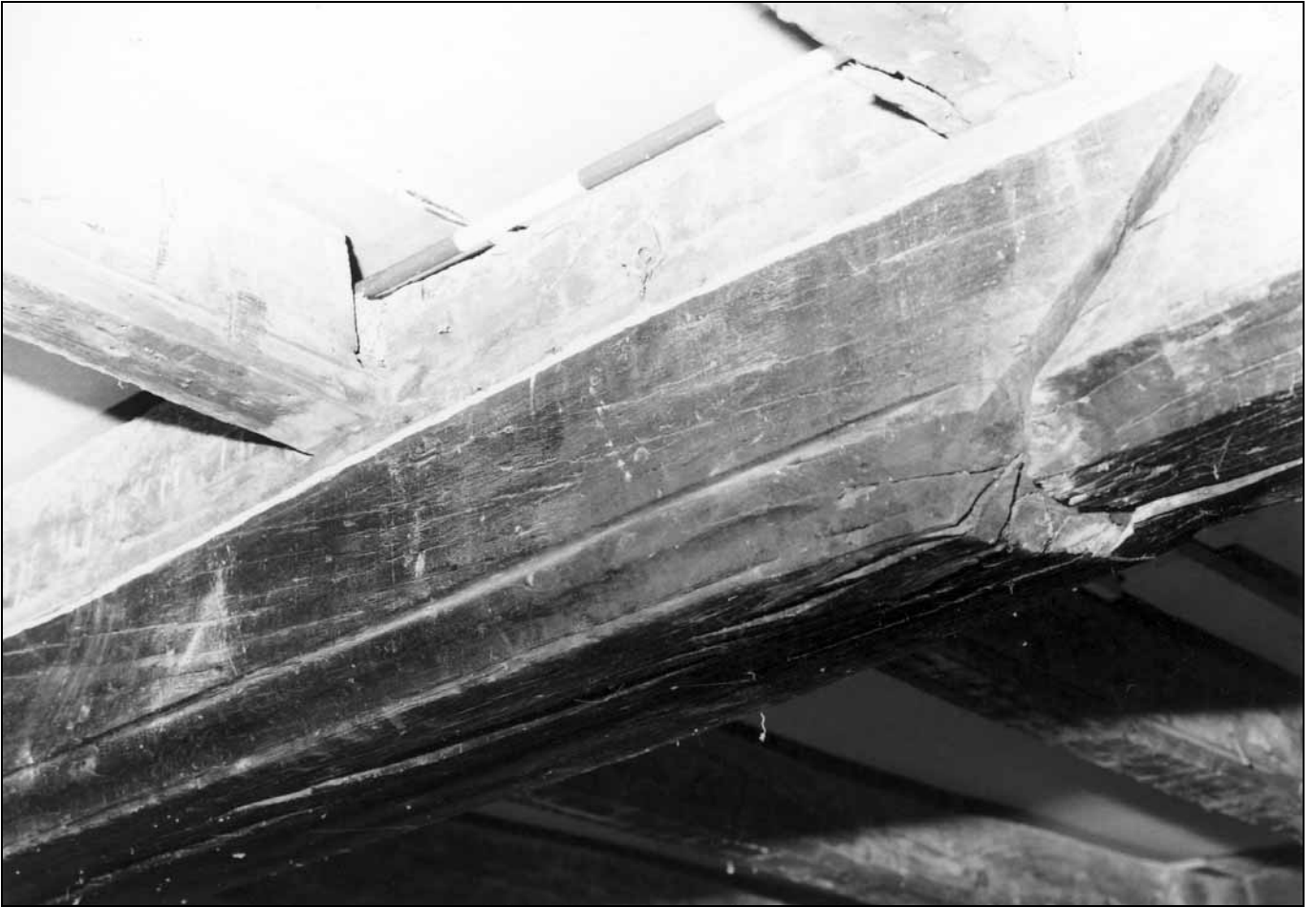
Photo 21: East ceiling beam in kitchen, with cyma moulding (film 1, frame 15)
