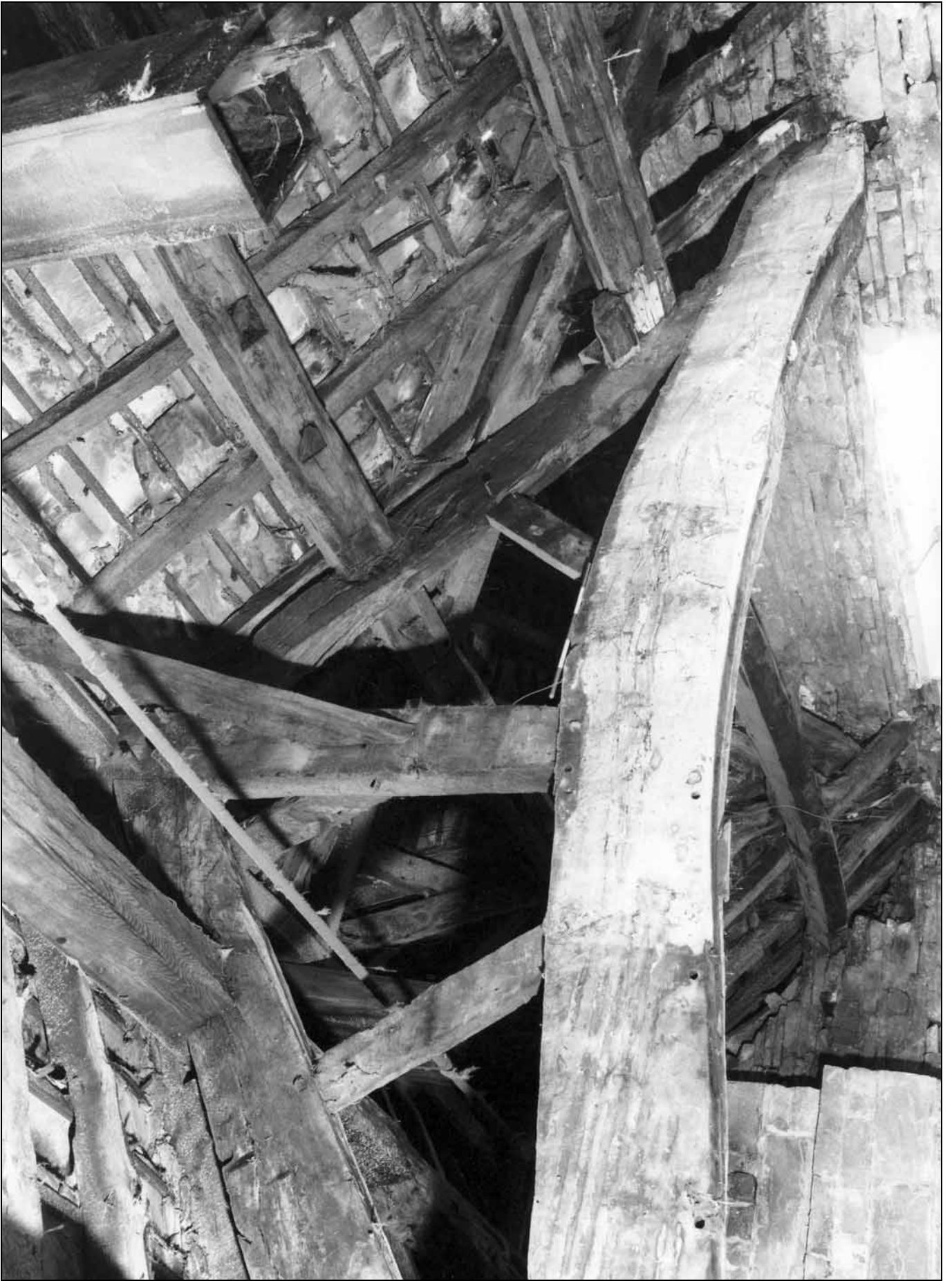
Photo 42: North truss, looking north-east (film 3, frame 17)
