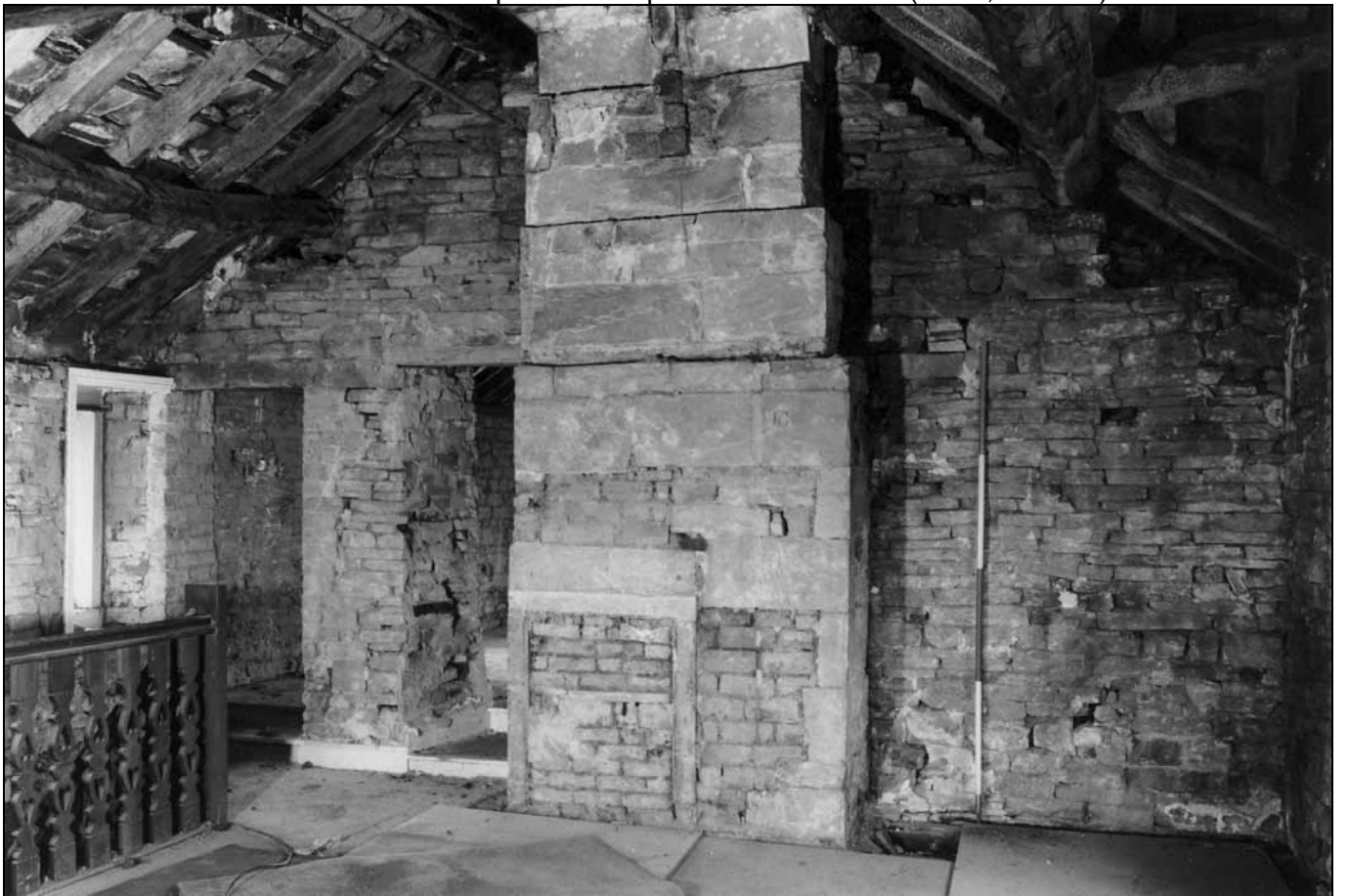
Photo 34: First floor, looking north towards inserted 1726 chimney with blocked fireplace (film 3, frame 4)
