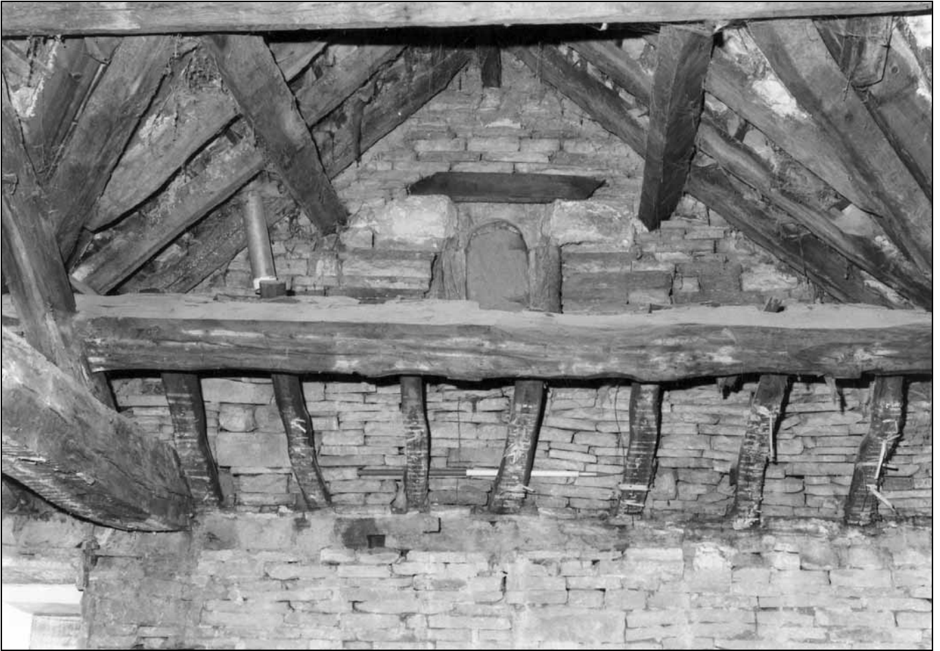
Photo 35: Interior of south gable in east side of wing, with blocked attic window, and purlin with rafters (film 4, frame 11)
