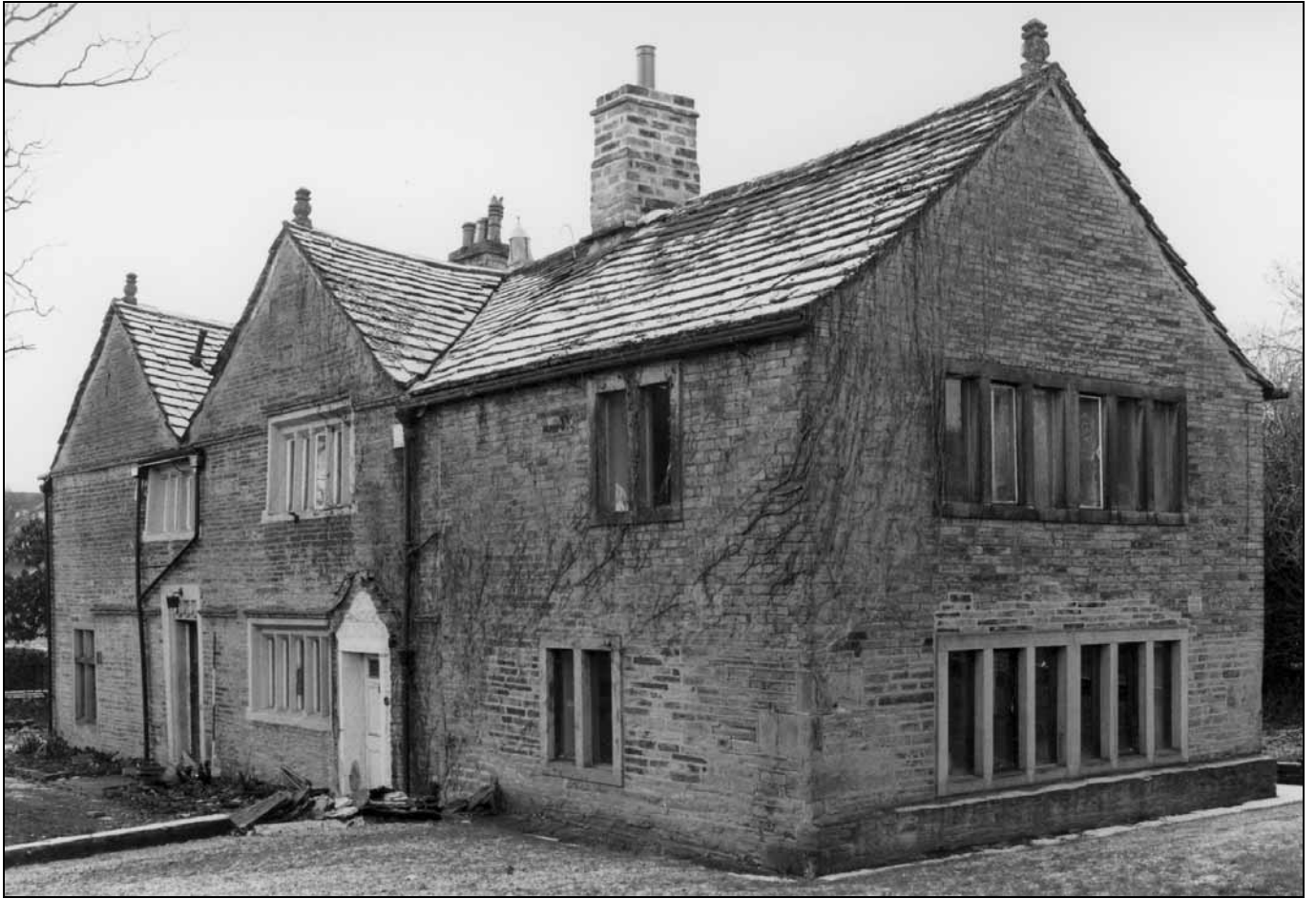
Photo 6: East wing, looking south-west, with 18th/19th century extension in foreground (film 2, frame 7)
