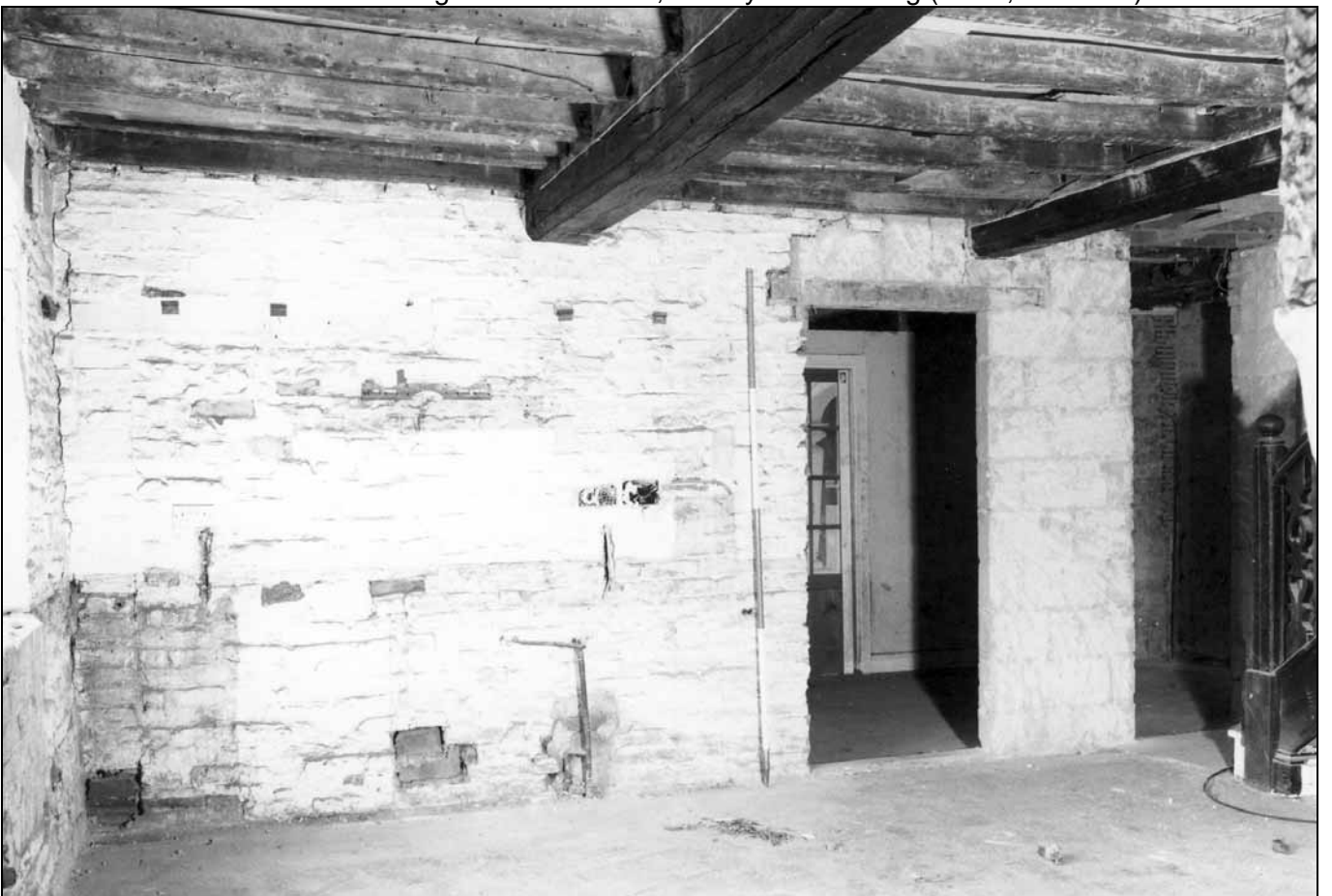
Photo 22: Kitchen, looking south-west (film 1, frame 18)
