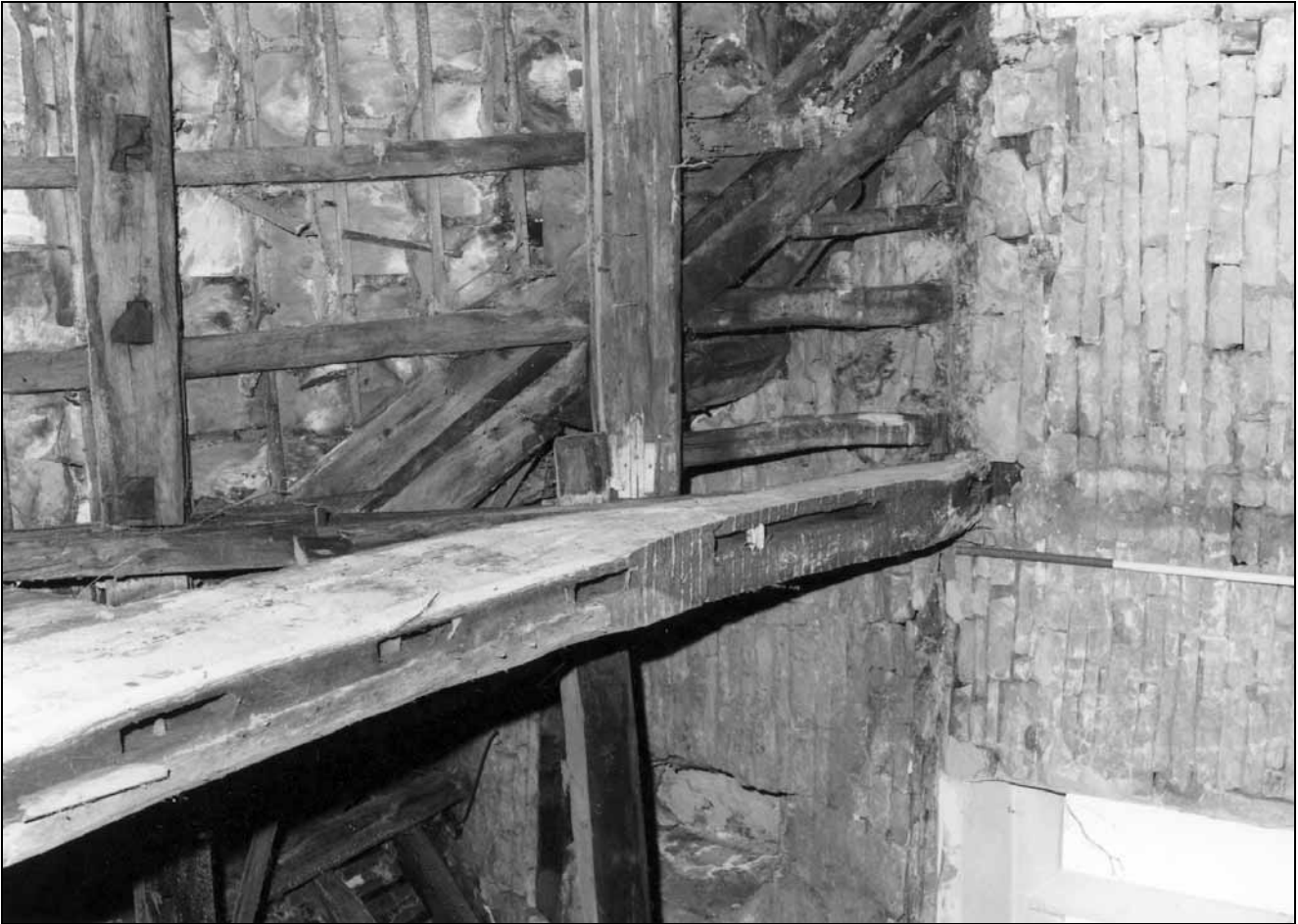
Photo 44: Underside of tie beam to north truss, looking east (film 4, frame 7)
