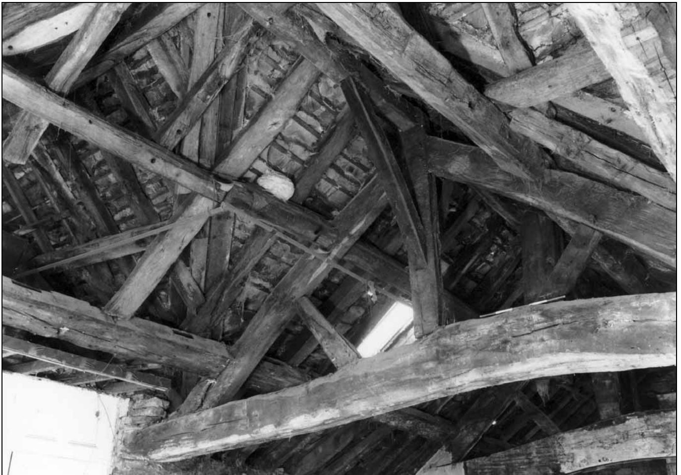
Photo 40: South truss, looking north-west (film 4, frame 1)
