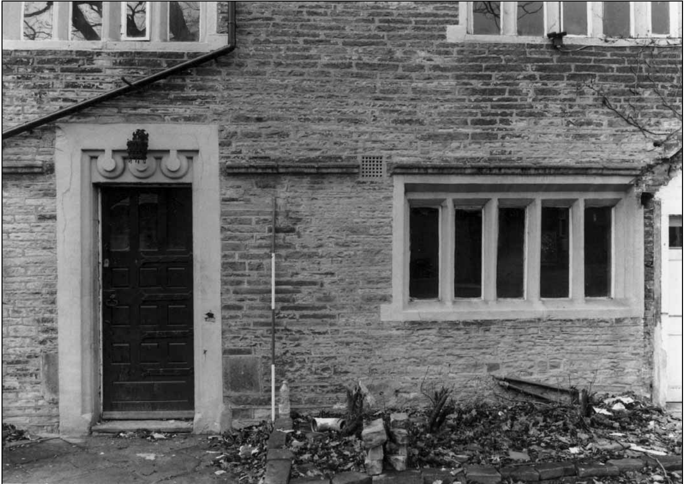
Photo 4: East wing, east elevation: original window and later doorway (film 2, frame 6)
