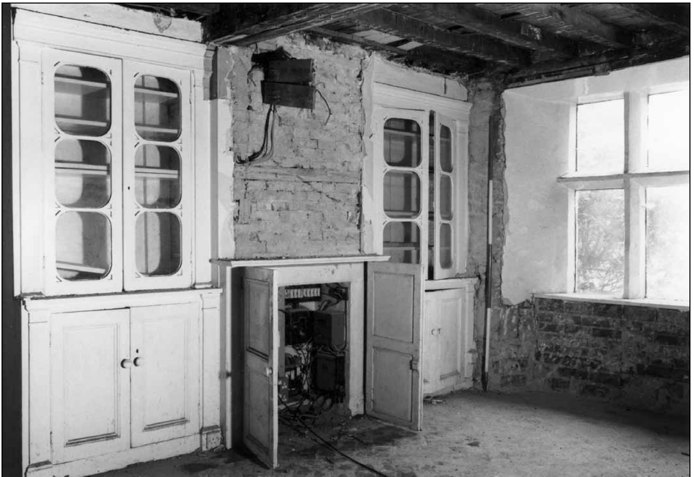
Photo 26: Ground floor room to rear of housebody, looking north-west (film 2, frame 15)
