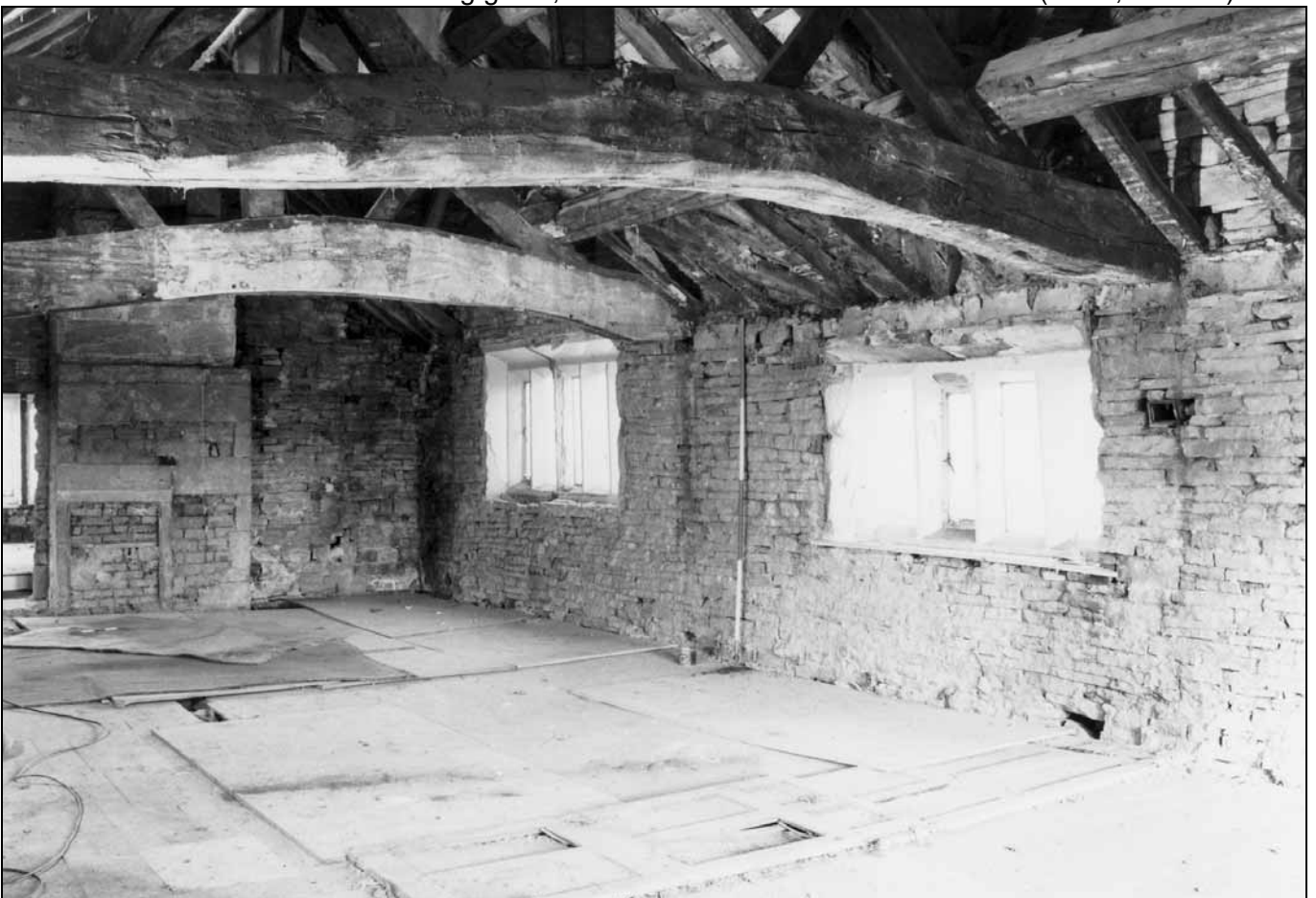
Photo 38: First floor, looking north-east (film 3, frame 16)
