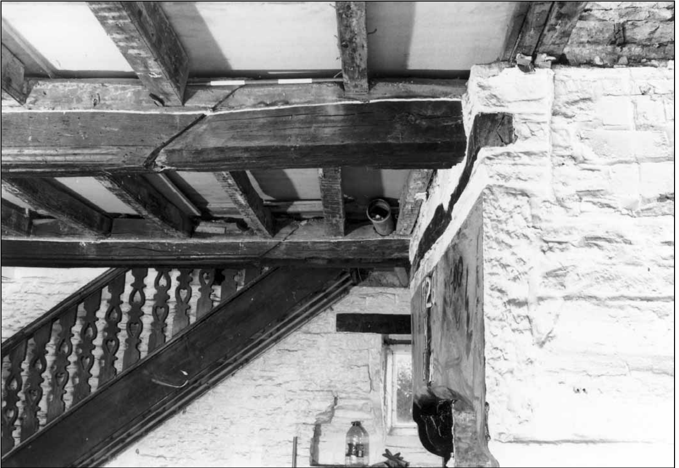
Photo 19: Ceiling beams above 1726 fireplace, with scarf joints (film 1, frame 14)
