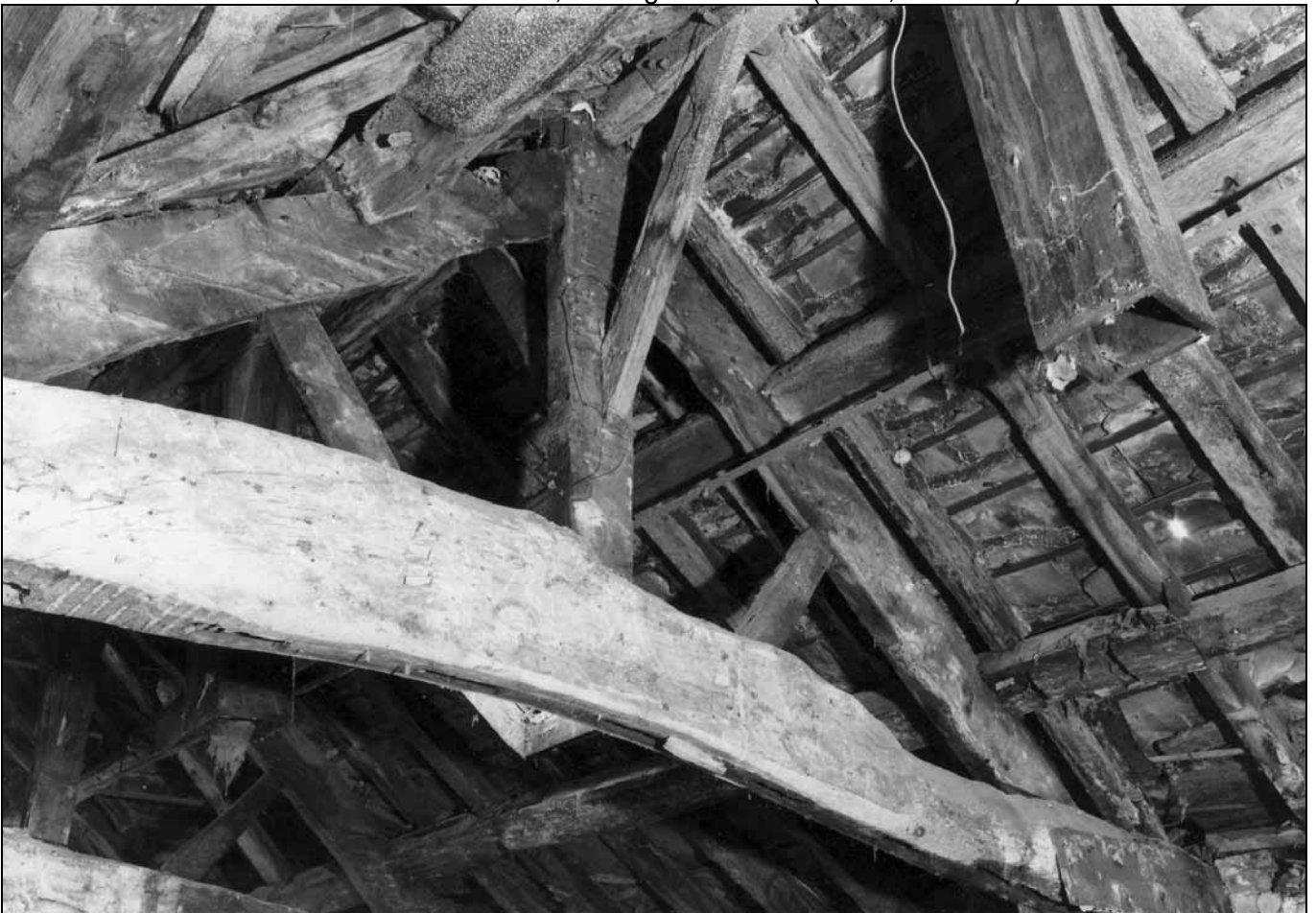
Photo 43: North truss, looking south-west (film 3, frame 7)
