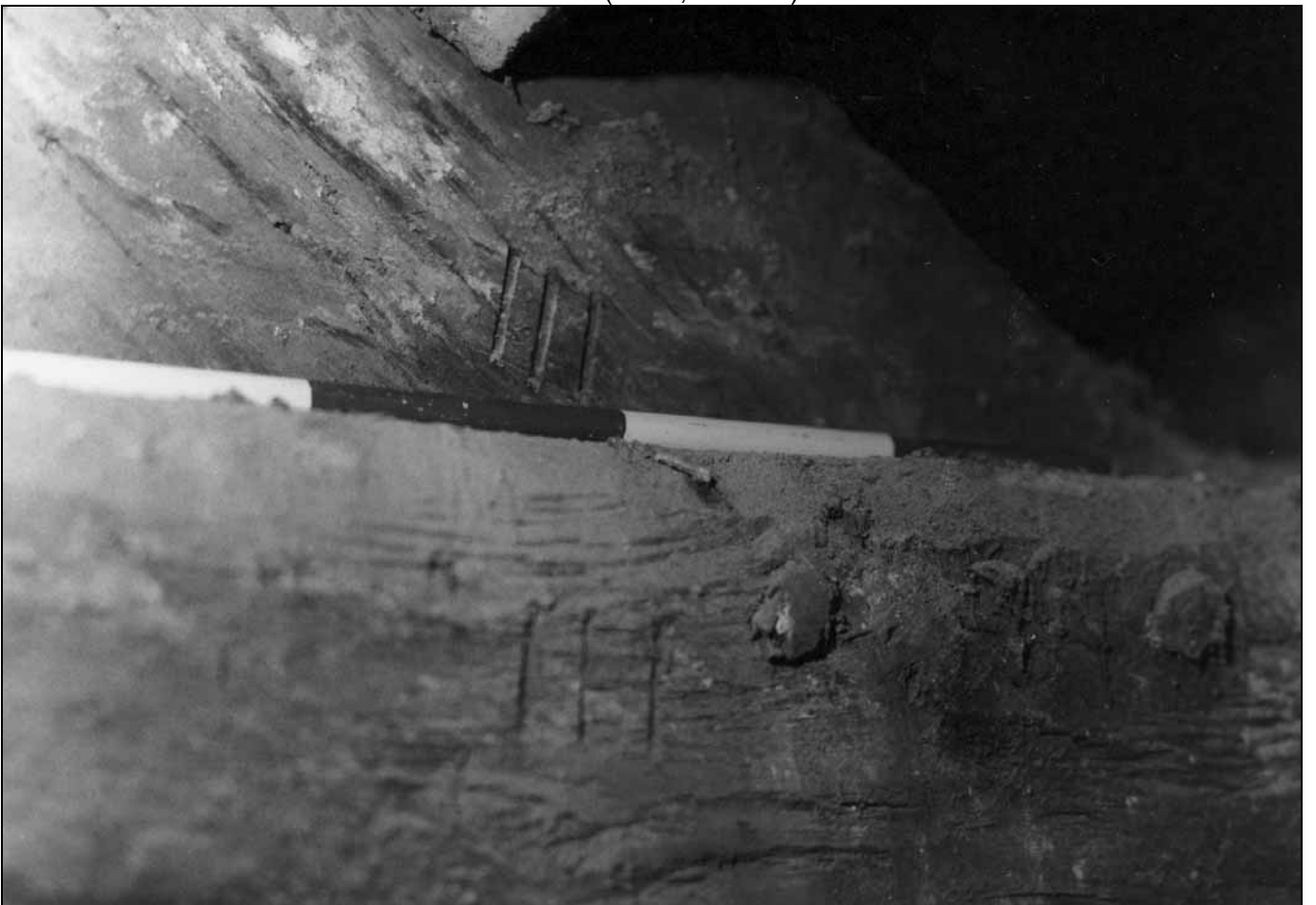
Photo 47: Detail of typical carpenter's numerals on south truss (film 4, frame 10)
