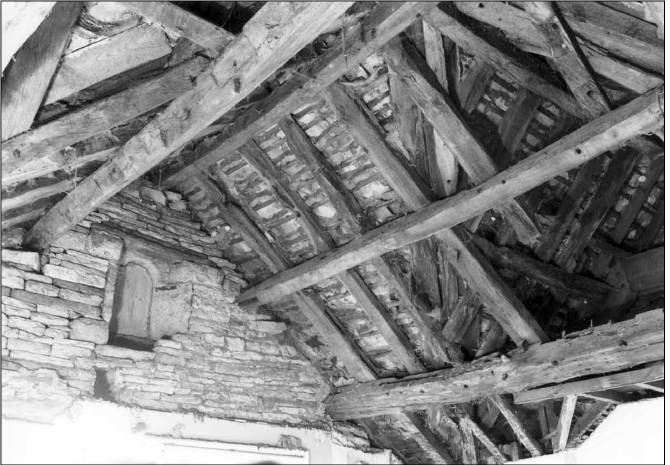
Photo 37: Roof and south-facing gable, with numerous reused timbers visible (film 4, frame 2)
