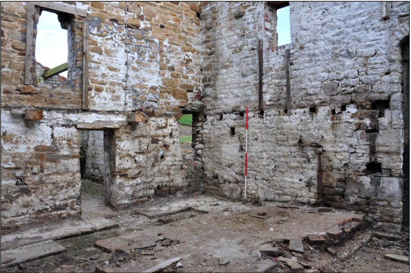
Photo 55: Barn interior, looking south-east (site of shippon)
