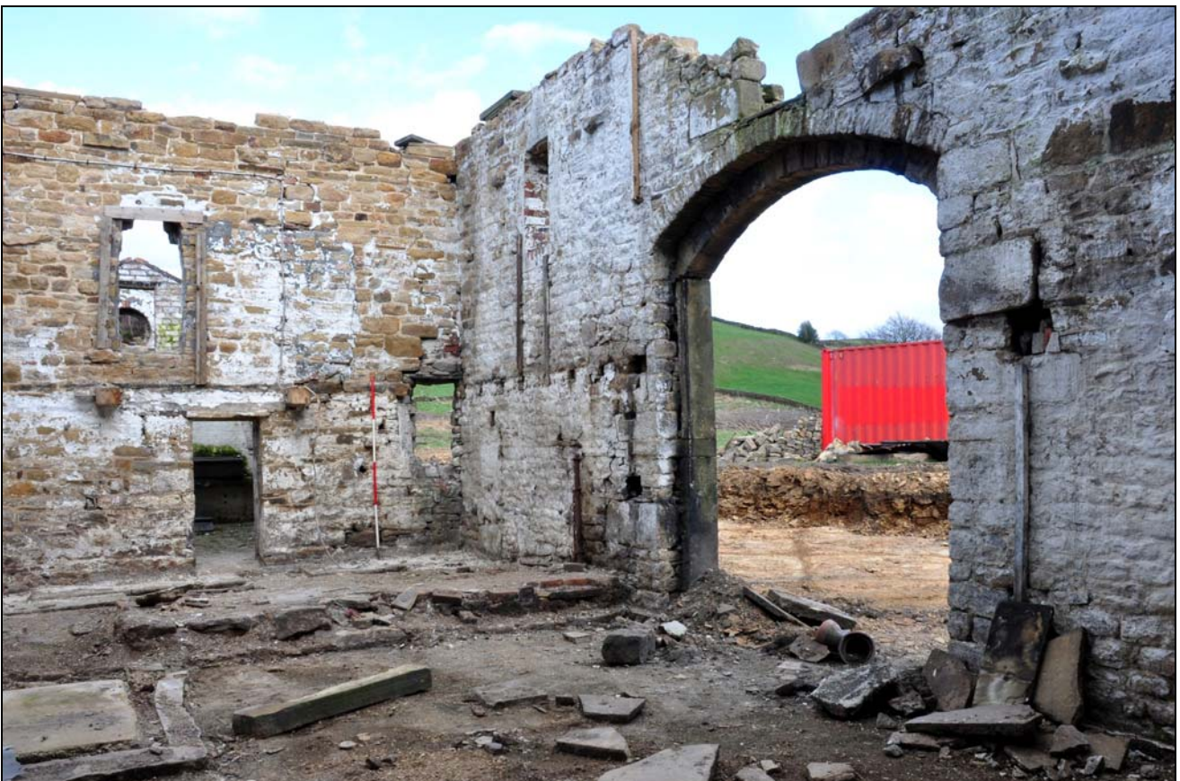
Photo 54: Barn interior, looking south-east
