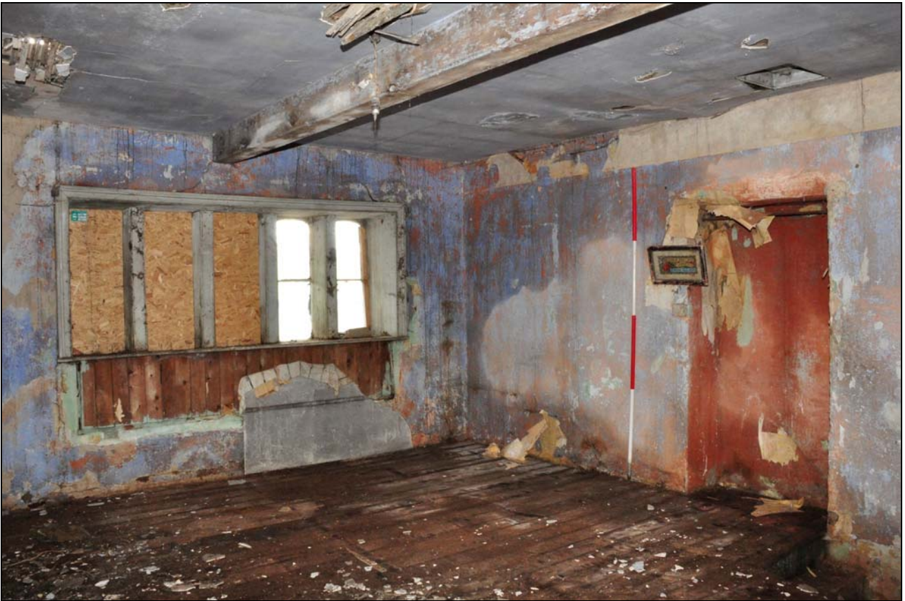
Photo 41: First floor, east room, looking south-west
