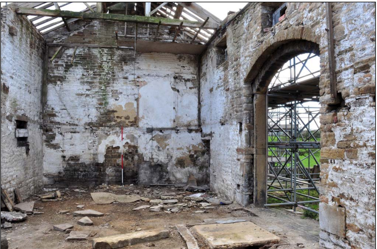
Photo 56: Barn interior, looking north-west
