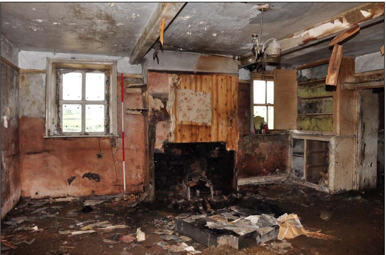
Photo 26: Ground floor, west room, looking north-west
