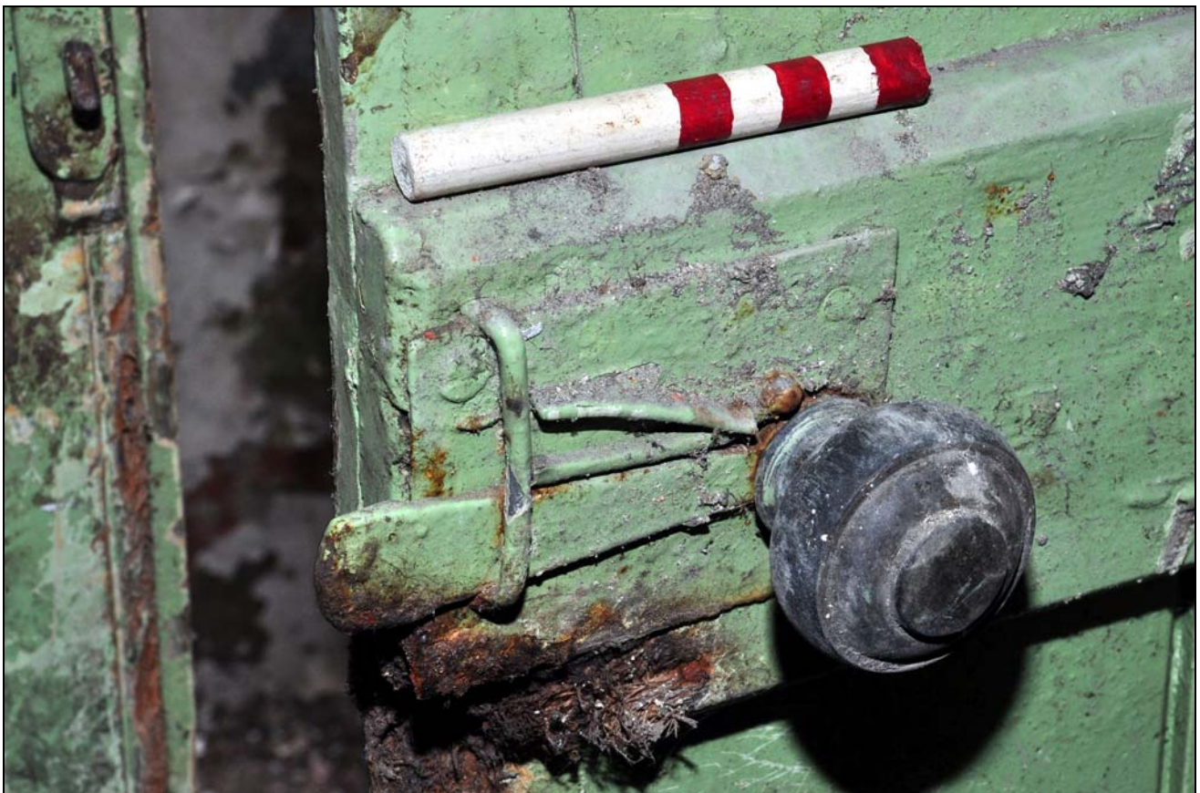
Photo 48: First floor, north room: detail of sprung latch to door
