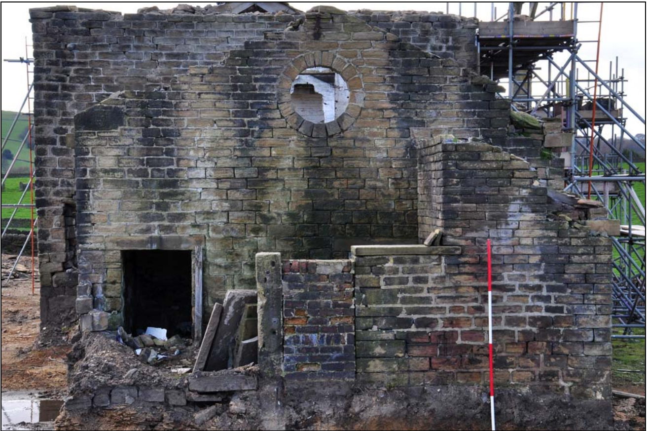
Photo 63: Stable, pigsty and coal stores, looking west
