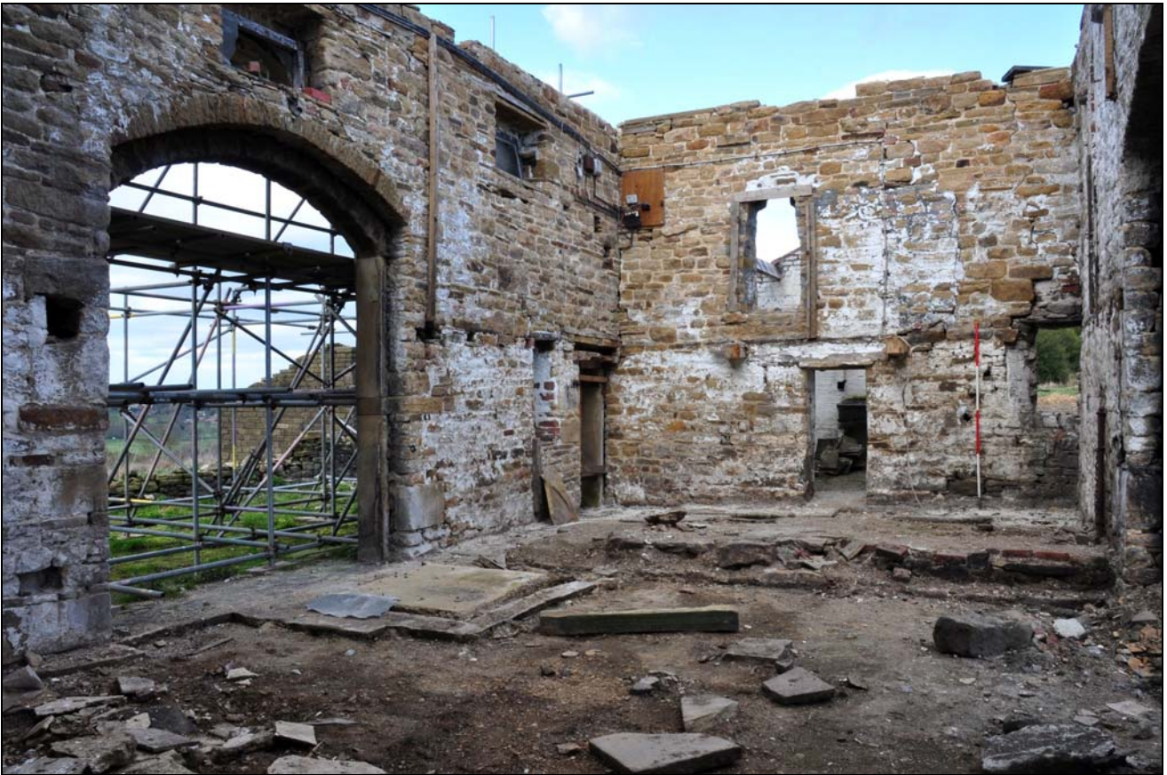
Photo 53: Barn interior, looking north-east
