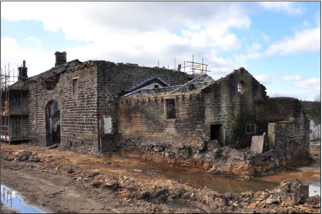
Photo 51: Barn, stable and pigsty, looking north-west
