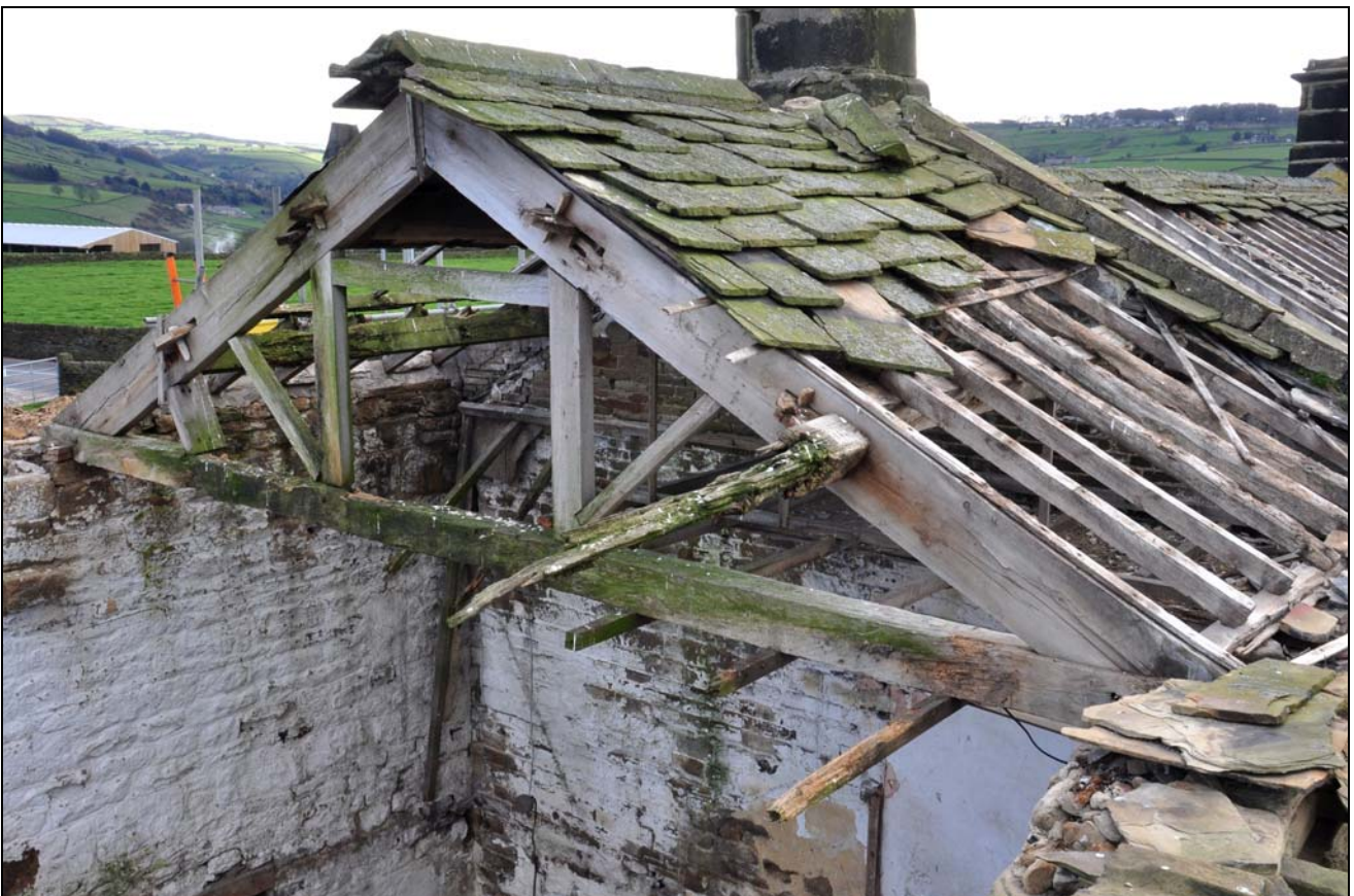
Photo 58: Barn: west roof truss
