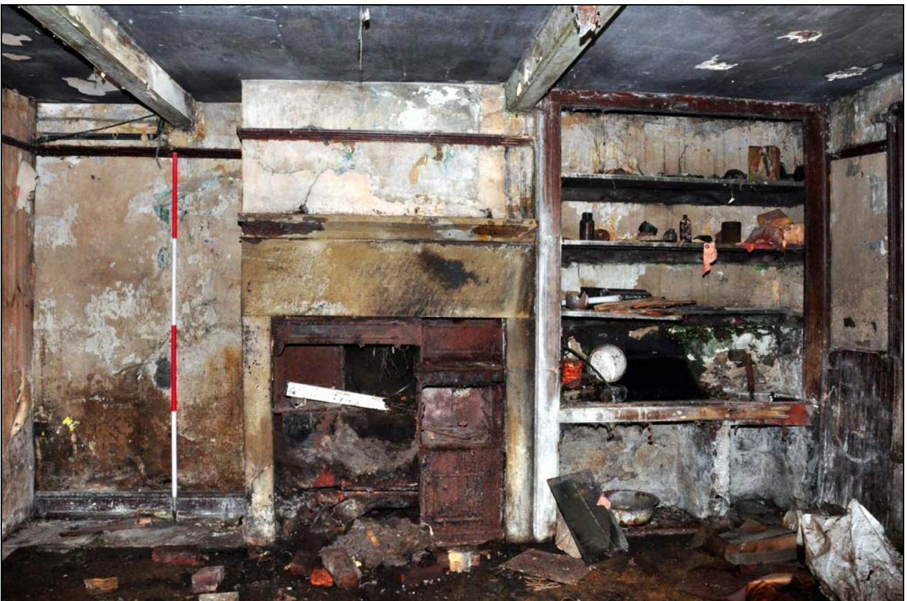
Photo 32: Ground floor, east room, looking east
