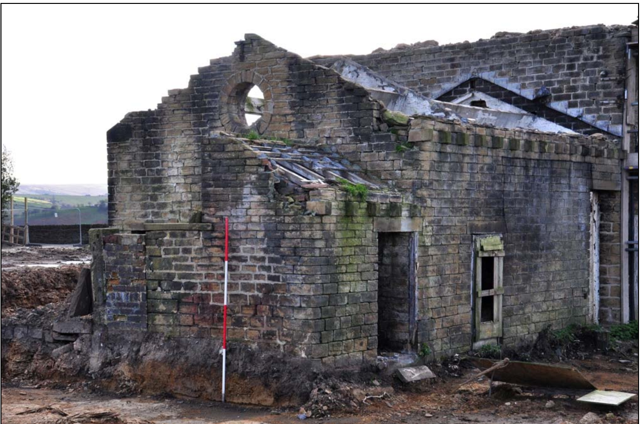
Photo 60: Stable and coal stores, looking south-west
