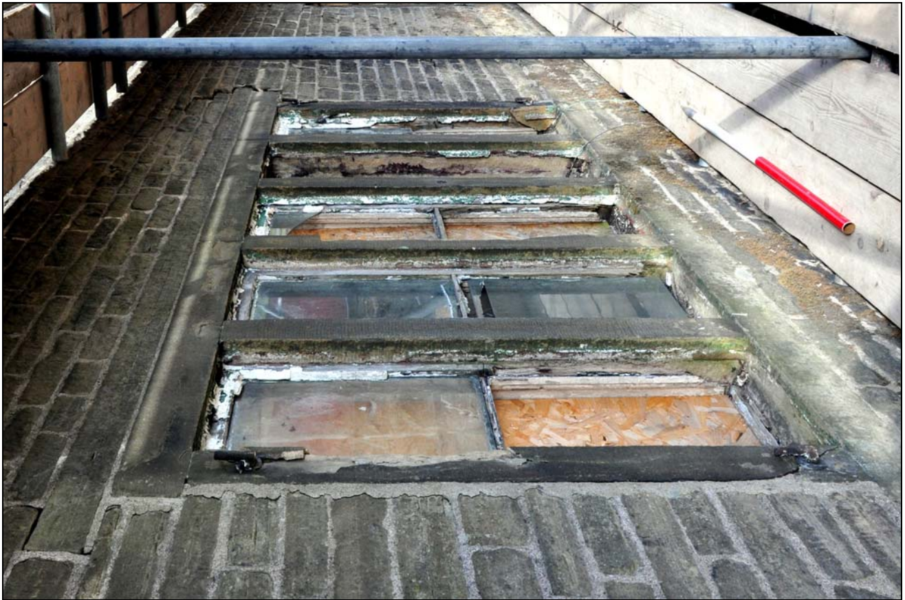
Photo 13: Detail of west, ground floor window to south elevation of house
