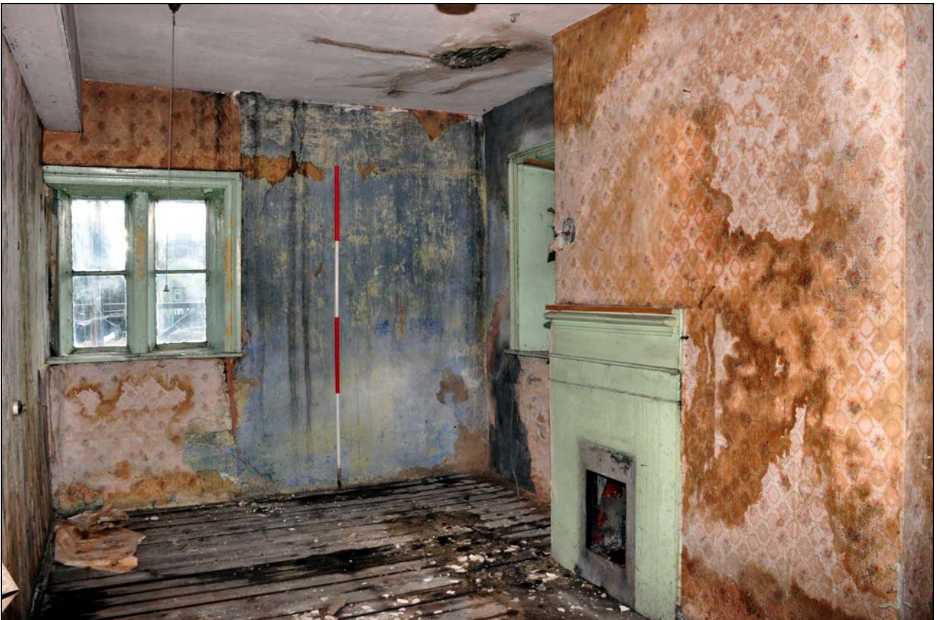
Photo 38: First floor, west room, west half, looking south
