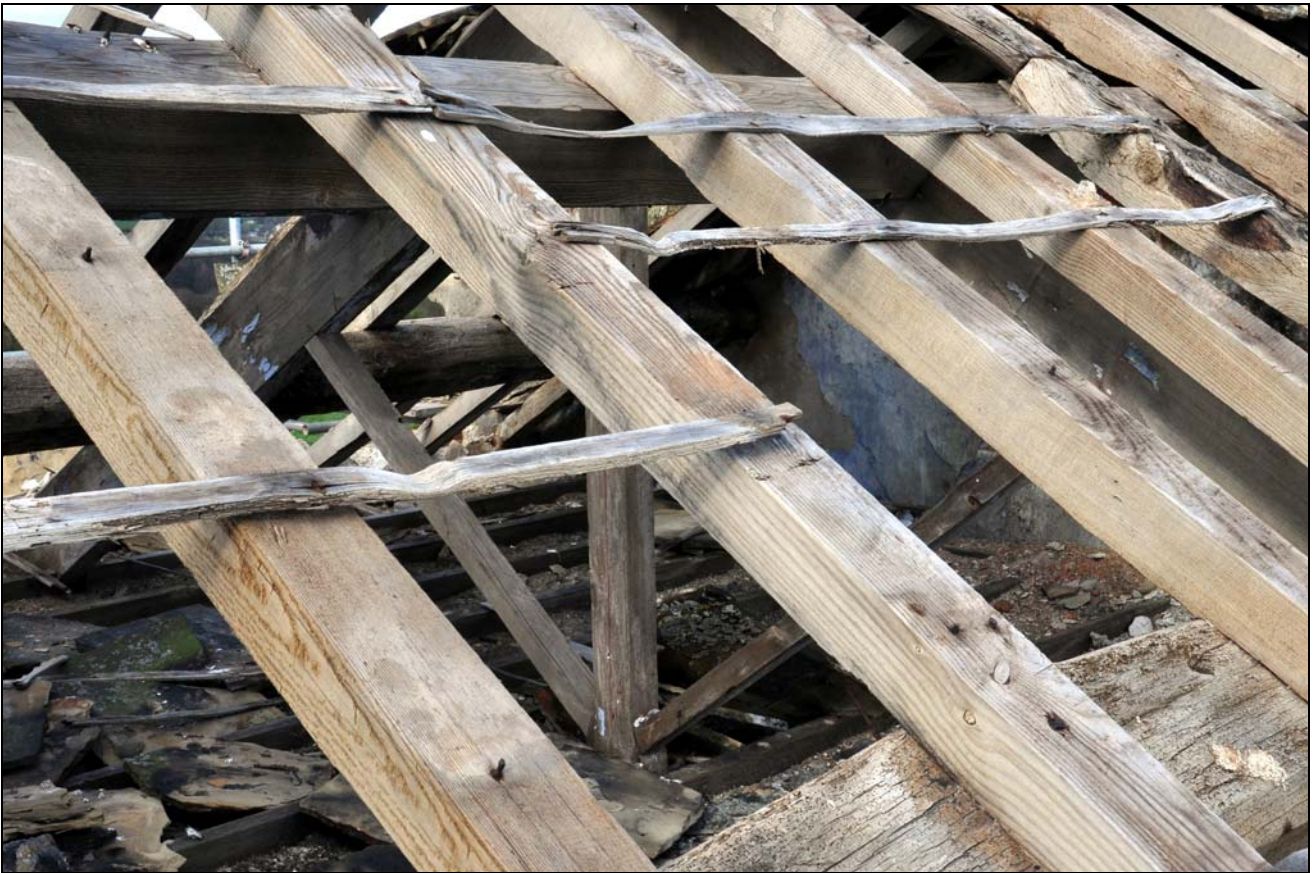
Photo 11: Roof structure over east end of house, looking north-east
