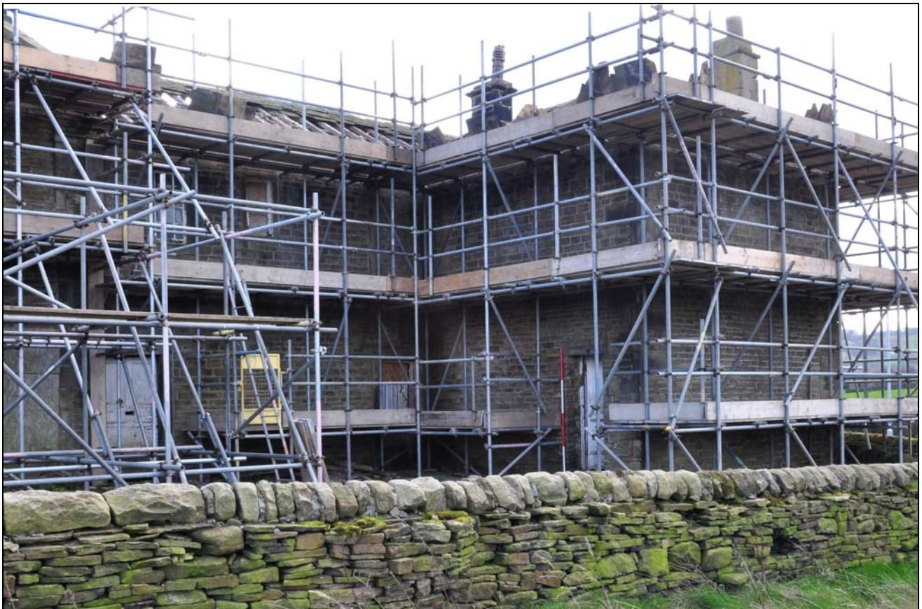
Photo 16: Rear of the house
