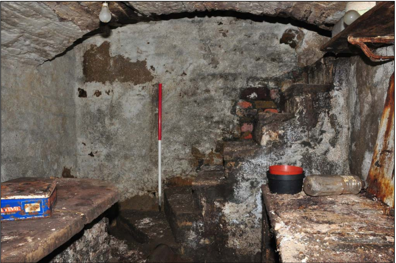
Photo 31: Cellar, looking east
