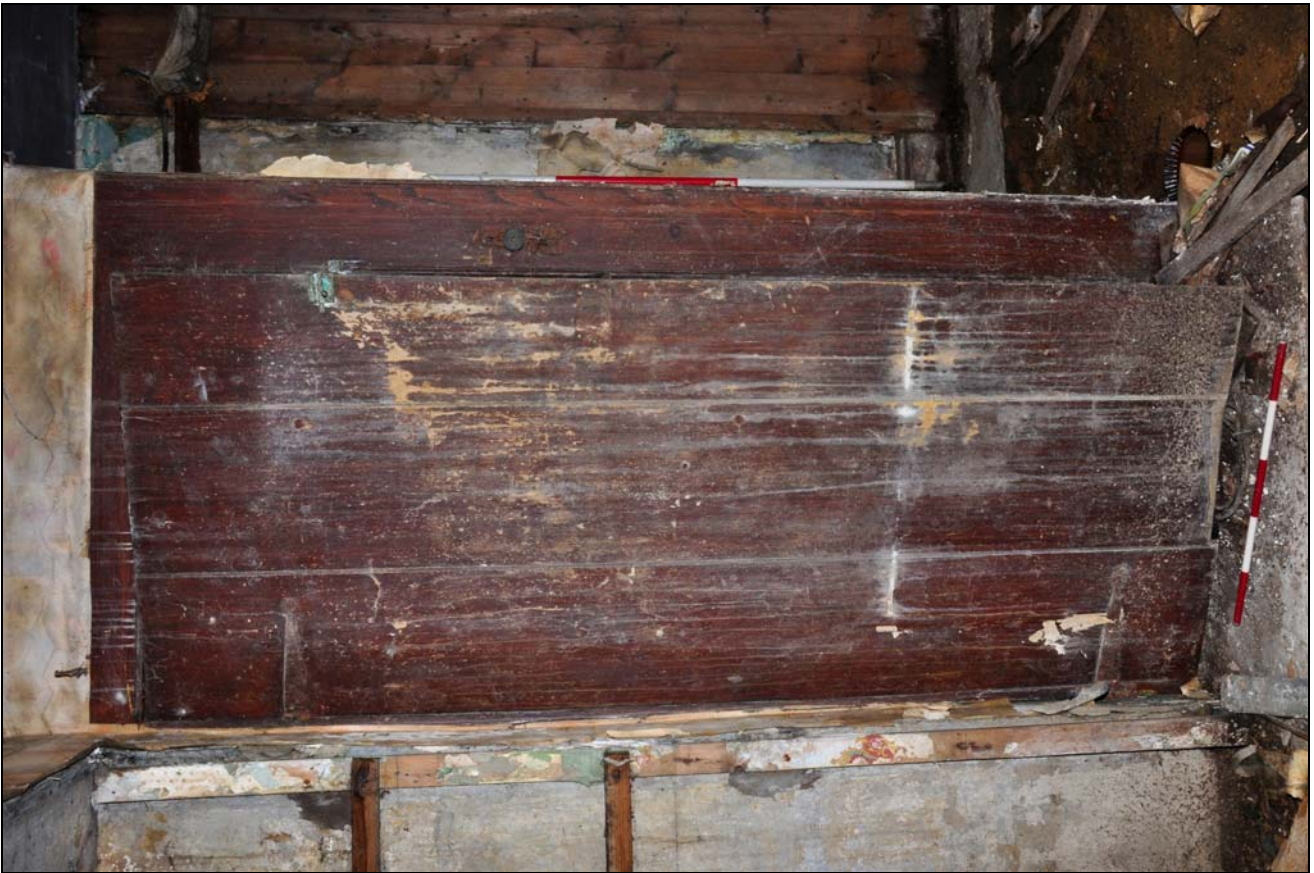
Photo 37: Ground floor, east room: door to cupboard beneath stairs
