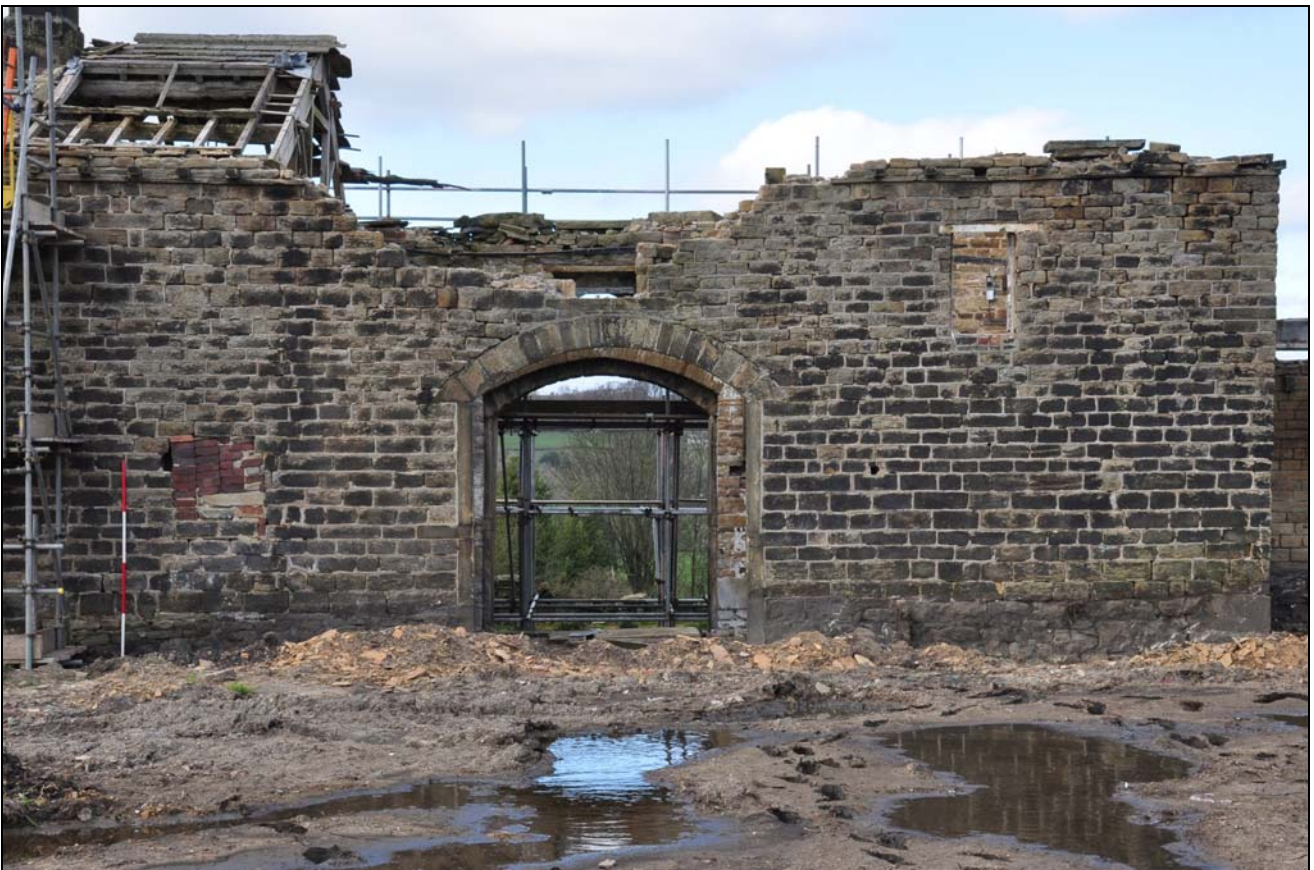
Photo 52: South (rear) elevation of the barn
