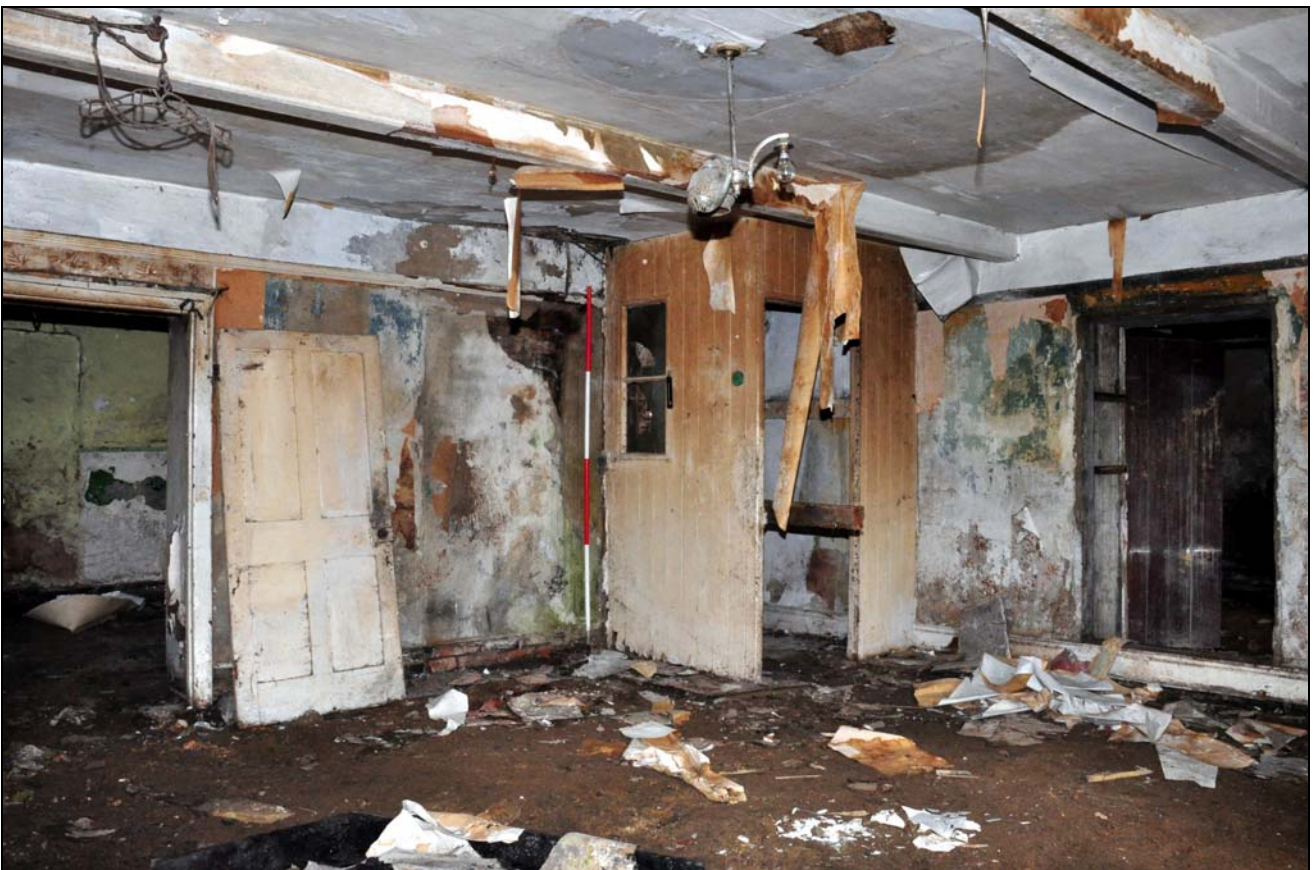
Photo 24: Ground floor, west room, looking north-east
