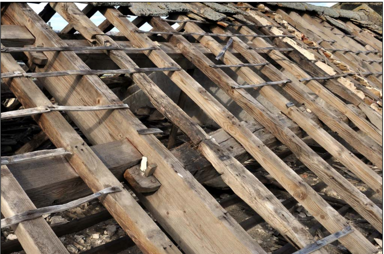
Photo 12: Roof structure over west end of house, looking north-east
