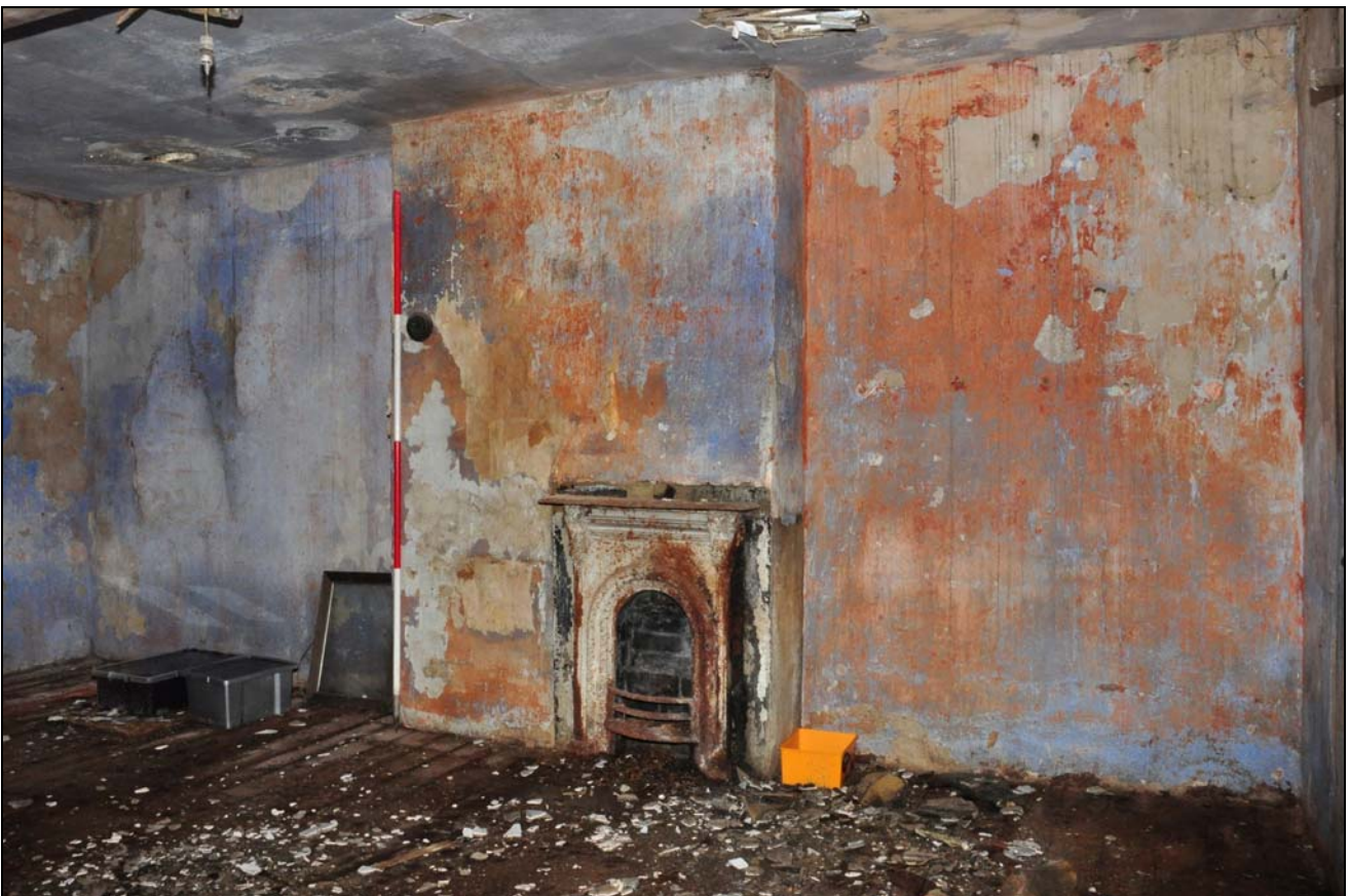
Photo 40: First floor, east room, looking north-east
