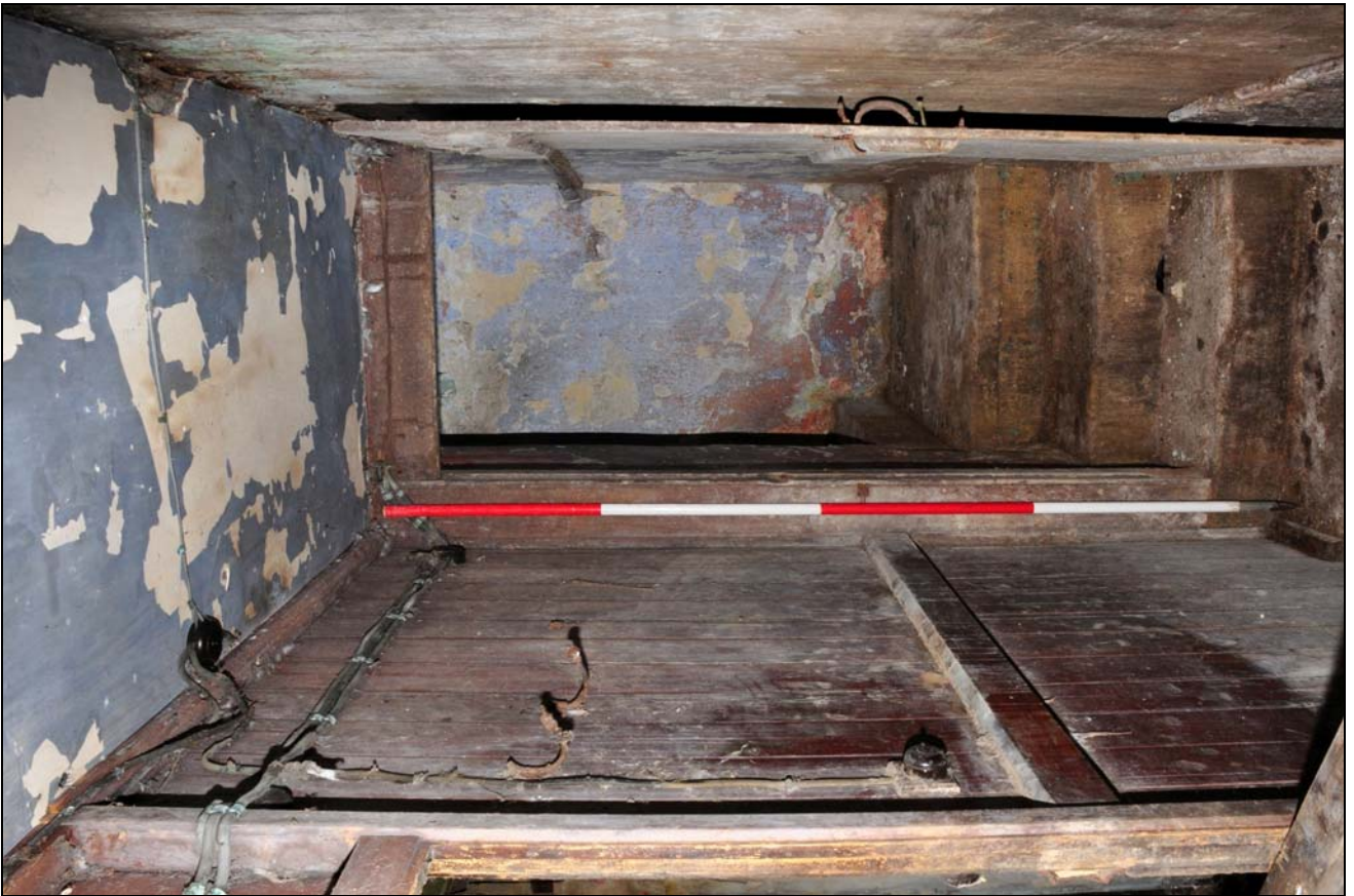
Photo 35: Ground floor, east room: foot of stairs to first floor
