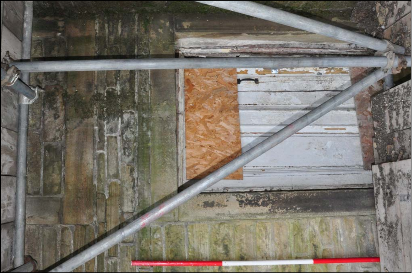
Photo 19: Ground floor, west rear doorway (D2)
