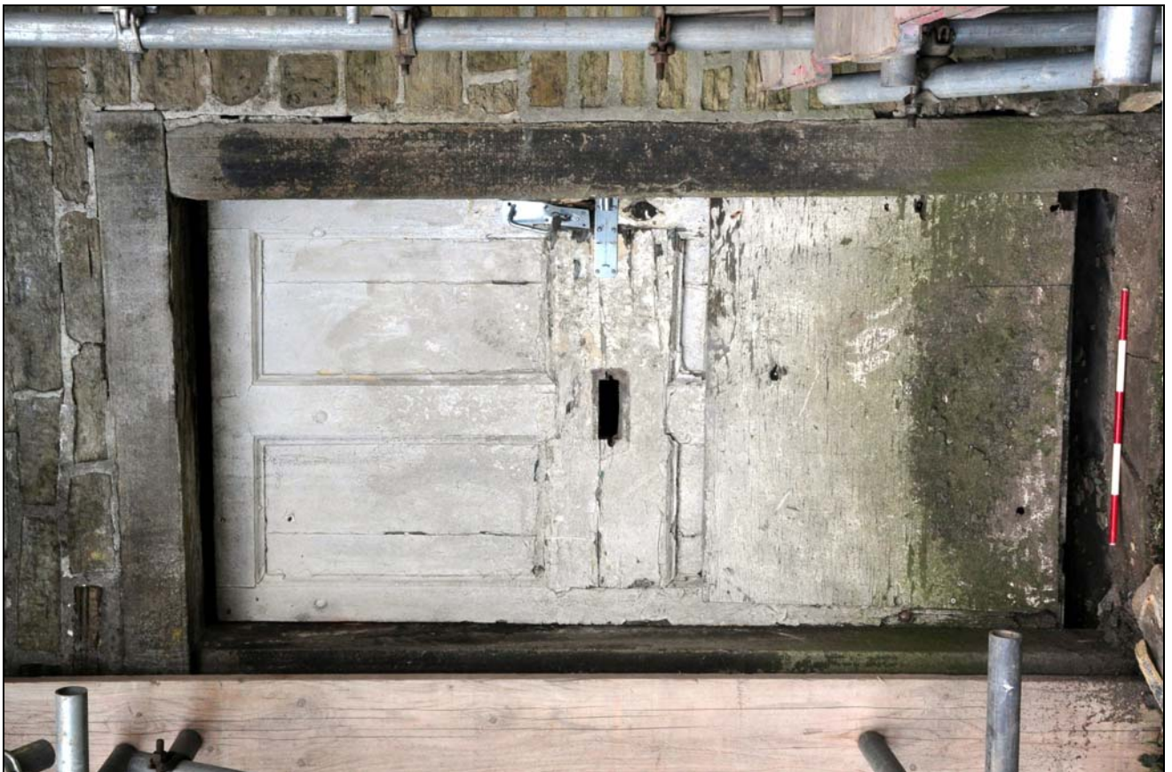
Photo 18: Ground floor, east rear doorway (D1)
