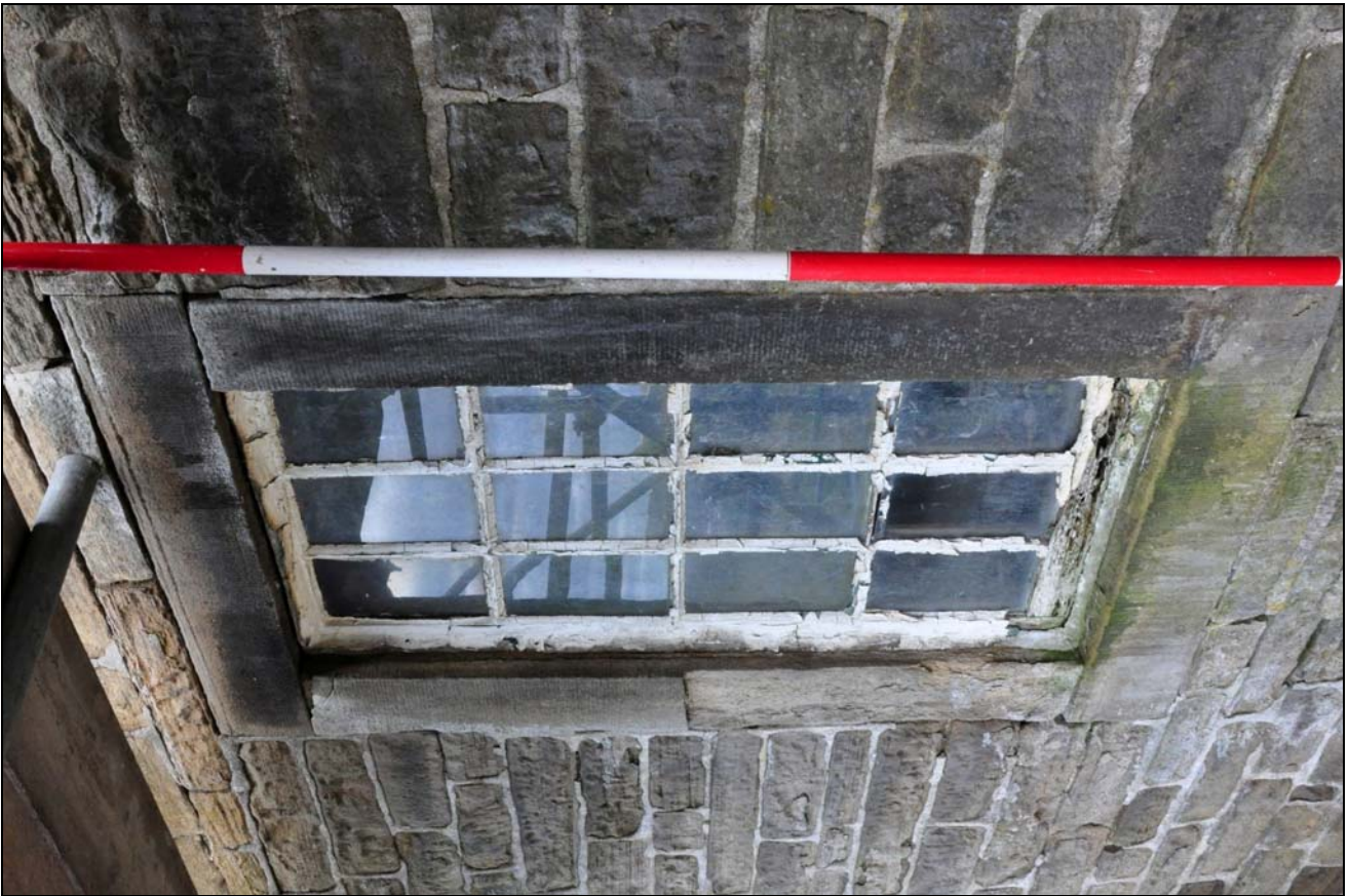
Photo 23: First floor rear window
