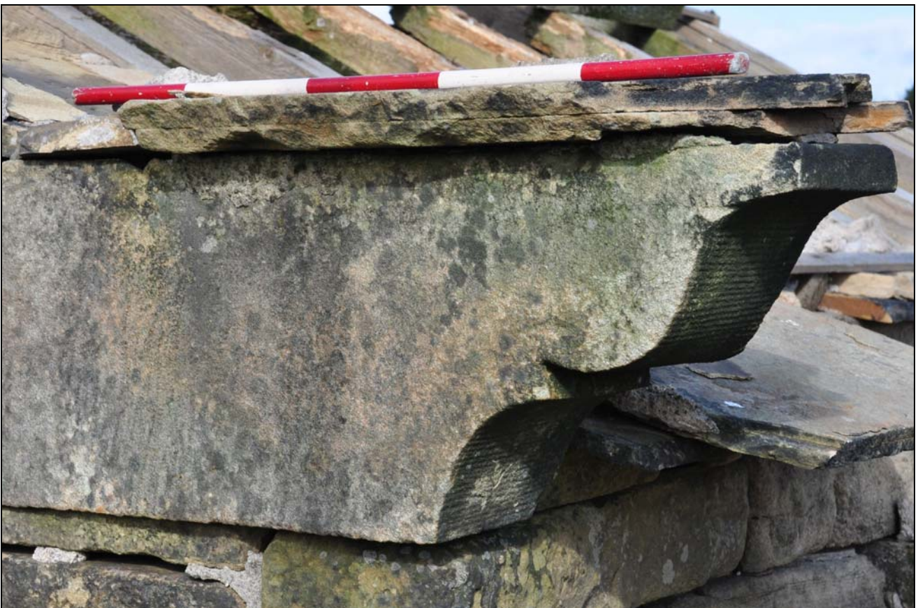
Photo 8: Detail of kneeler, south-west corner of barn
