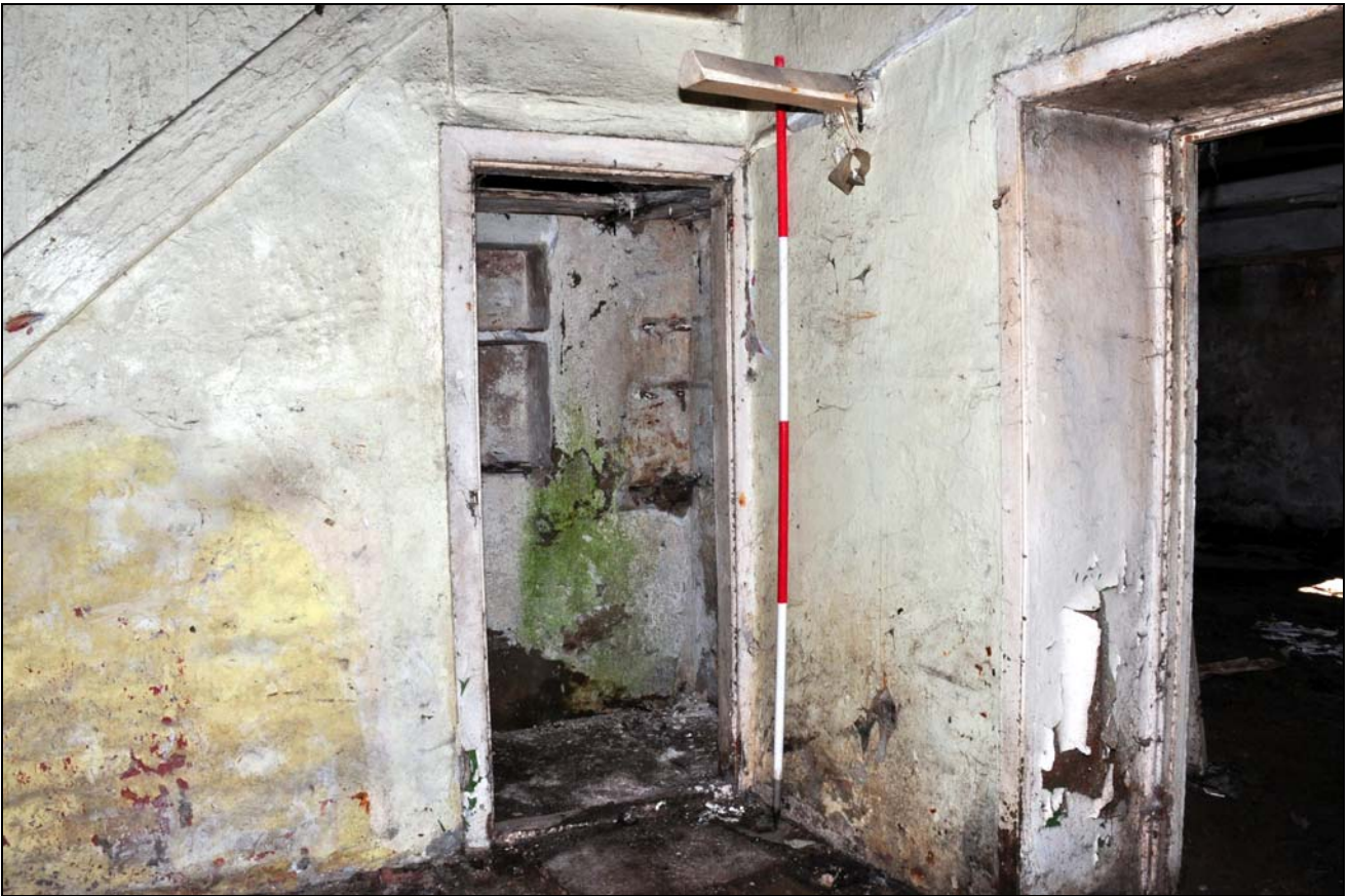
Photo 29: Ground floor, west room, looking south-east (head of cellar stairs)
