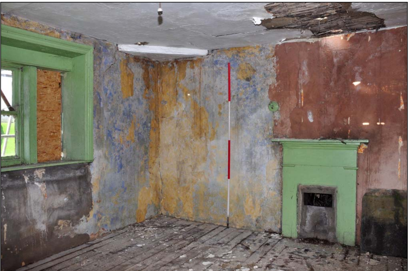
Photo 46: First floor, north room, looking north-west
