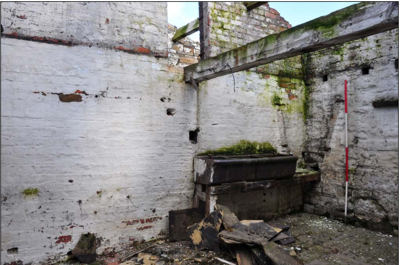
Photo 62: Interior of stable, looking south-east
