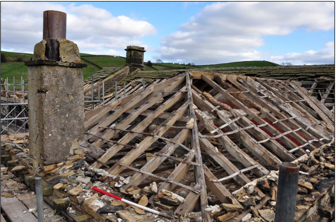
Photo 10: Hipped roof to rear wing, with plain north chimney
