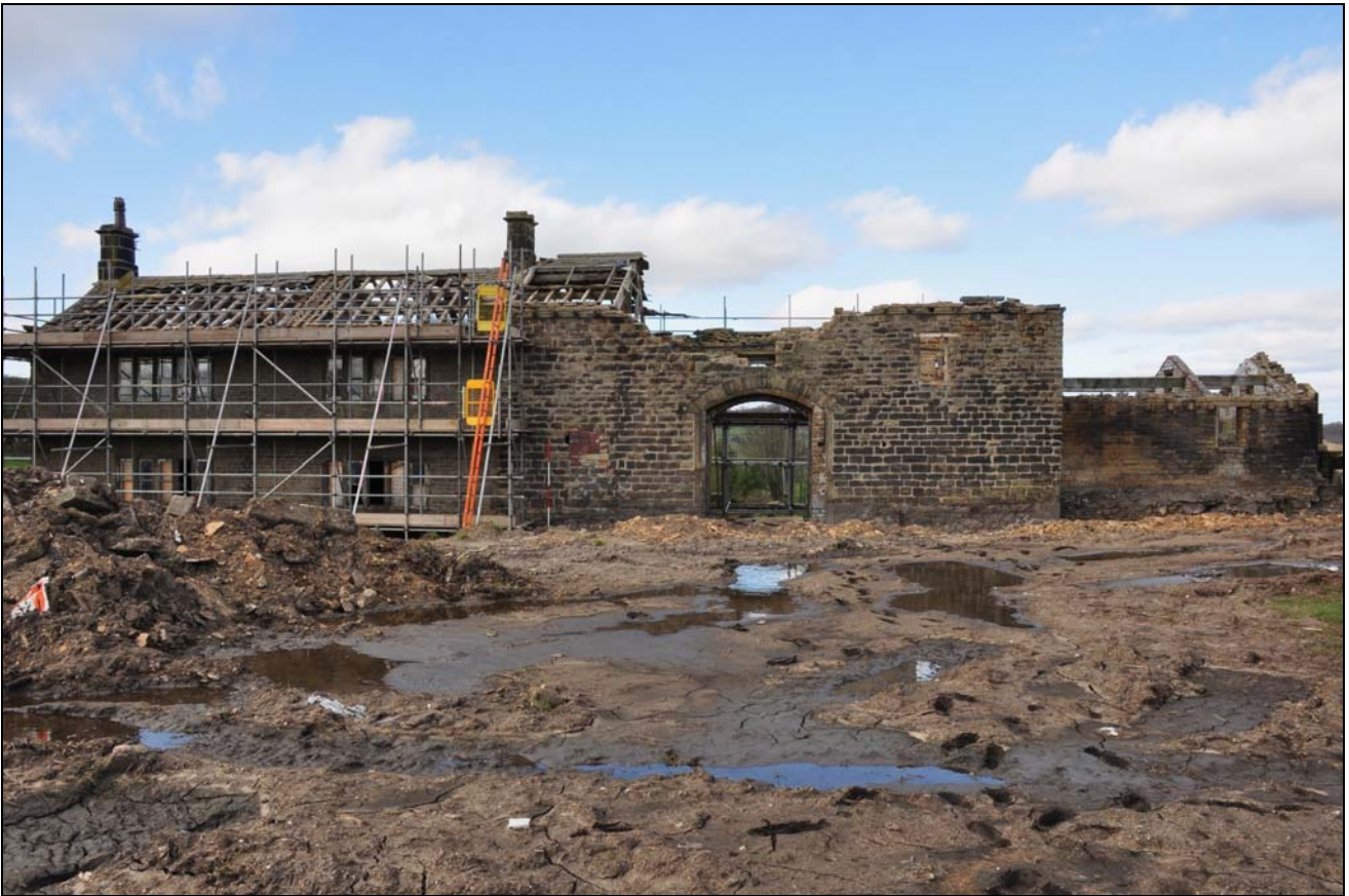
Photo 3: House and barn, from the south
