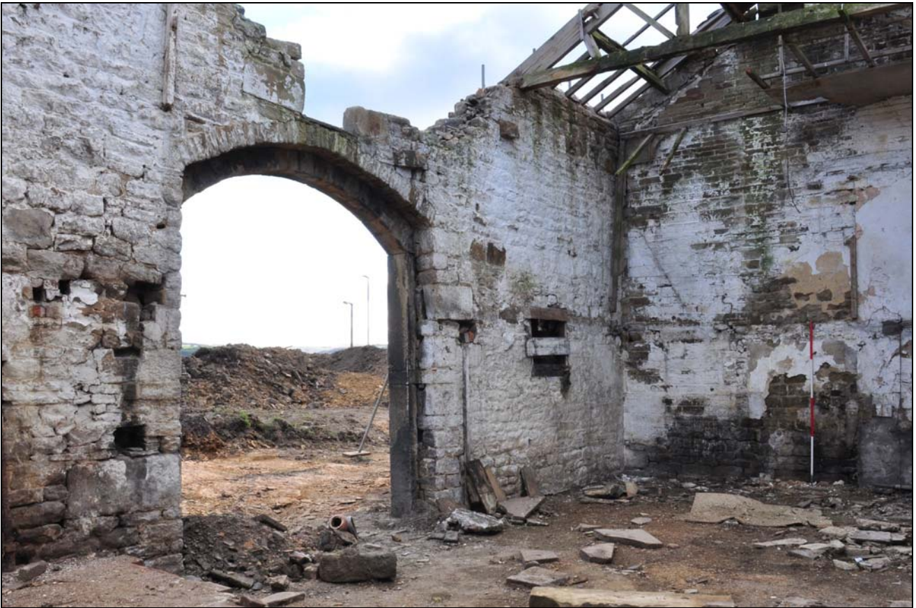
Photo 57: Barn interior, looking south-west
