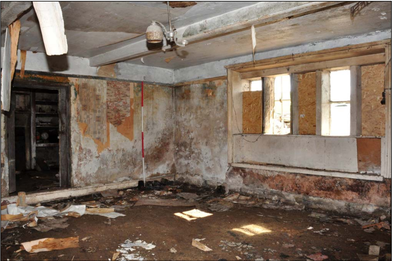
Photo 25: Ground floor, west room, looking south-east
