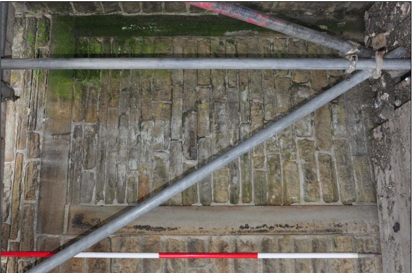
Photo 20: Blocked, first floor "piece" doorway, in rear
