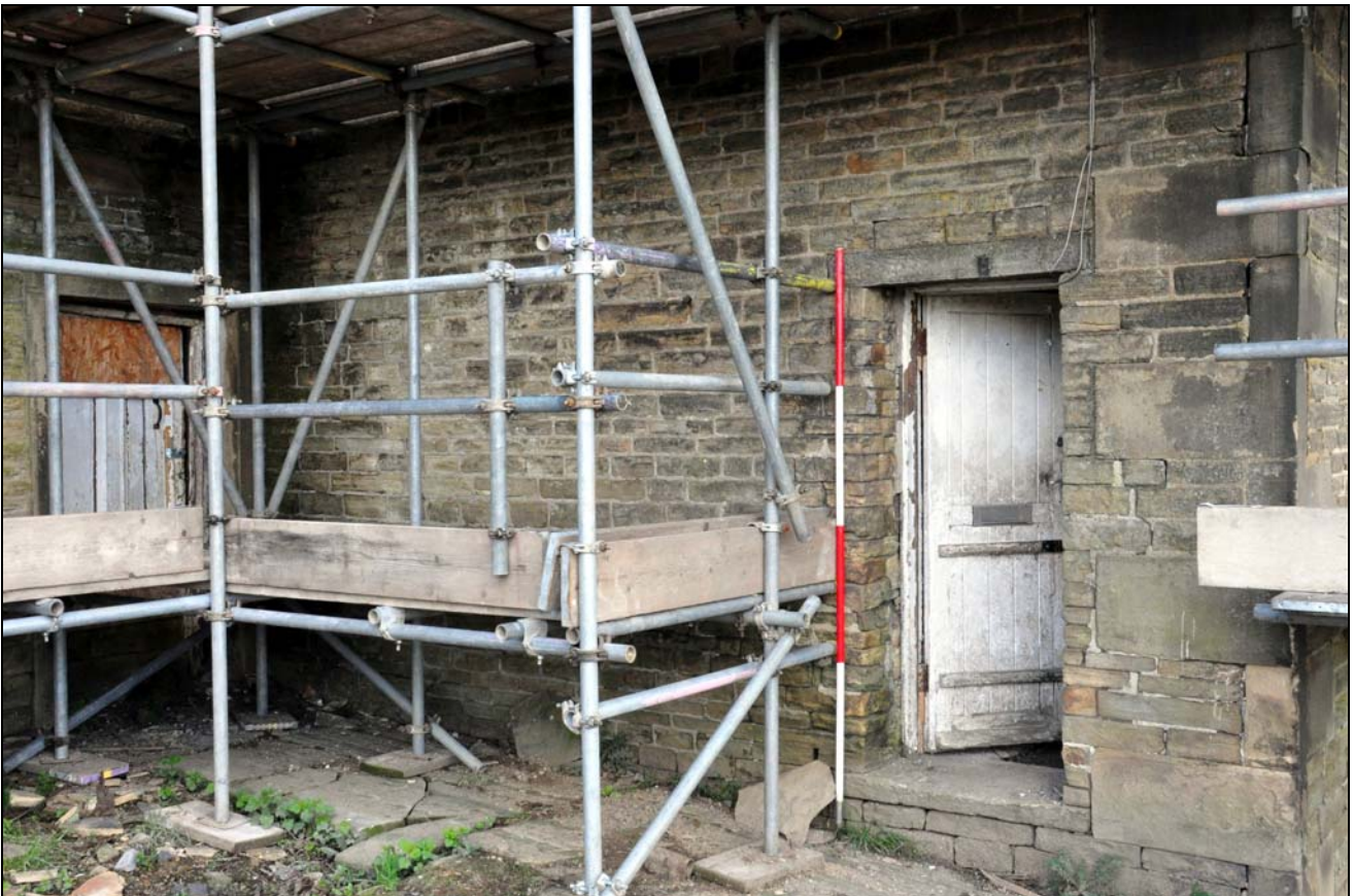
Photo 22: East side of rear wing, with inserted doorway
