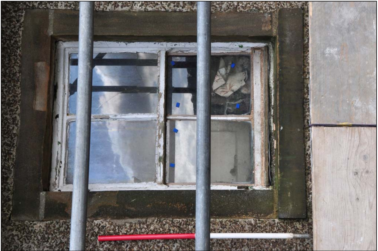
Photo 15: Detail of 19th/20th century ground floor window, west side of house
