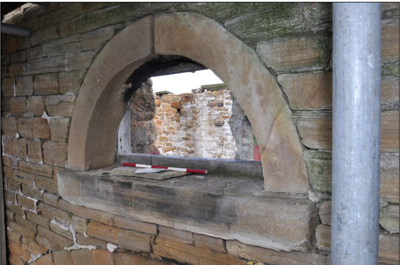
Photo 50: Window over central doorway, north side of barn
