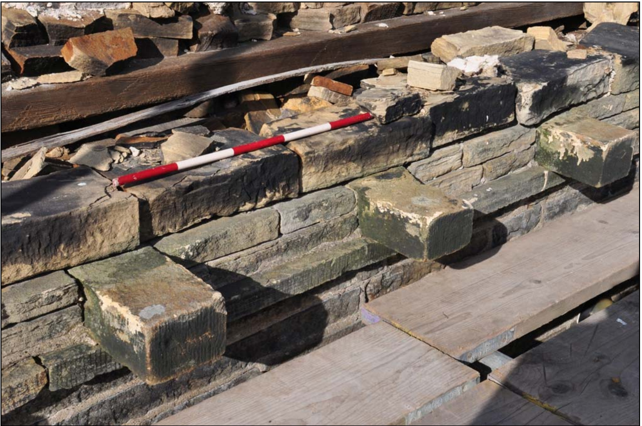
Photo 7: Detail of eaves corbels, south elevation
