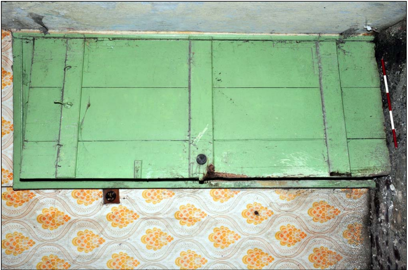
Photo 47: First floor, north room: detail of plank and batten door
