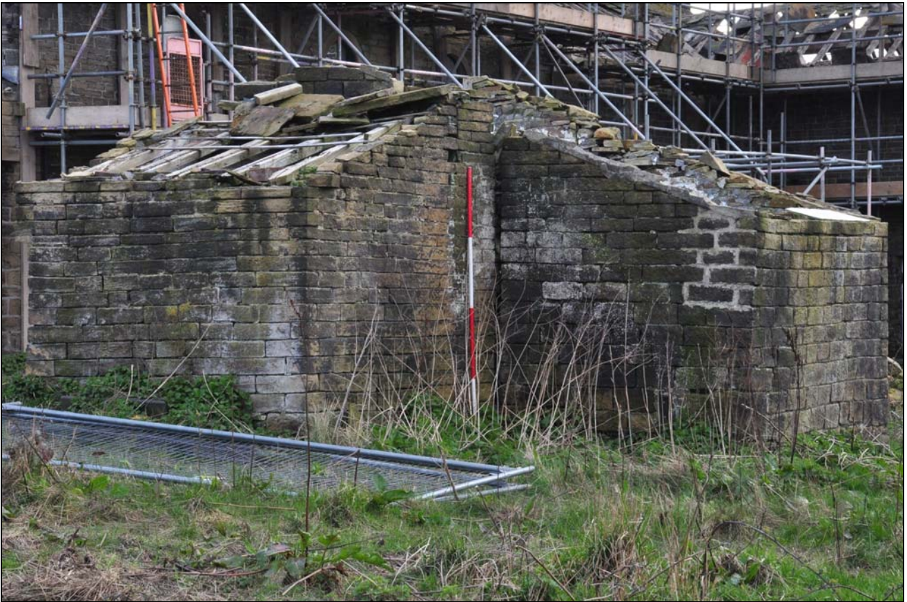
Photo 65: Trap-house and earth closet, looking south-west
