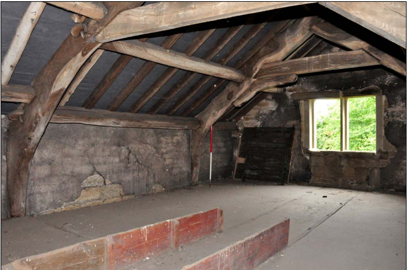
Photo 30: First floor, looking west
