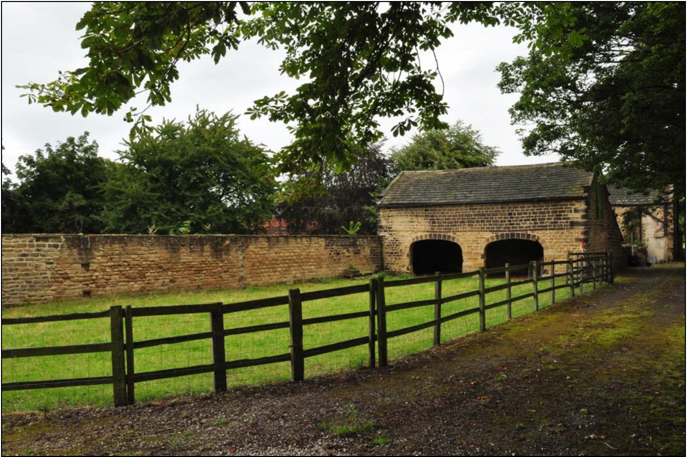
Photo 1: General view of the building, looking north-east
