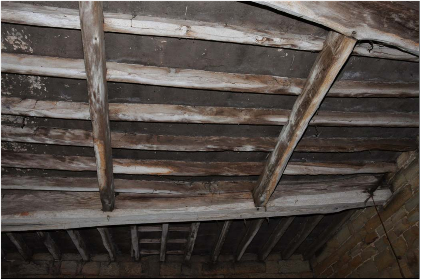
Photo 23: Underside of first floor, looking north-west
