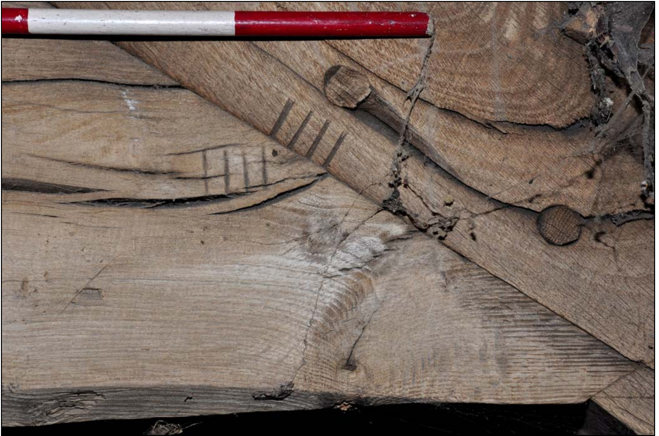
Photo 47: Detail of joint numbering on collar at joint with cruck, south-east truss
