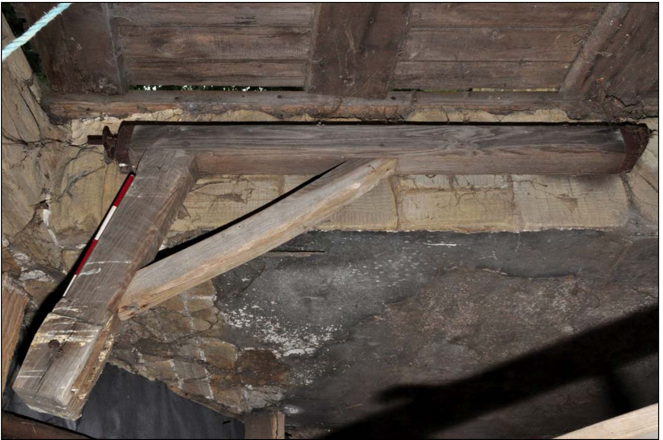
Photo 35: Crane in south-east loading doorway
