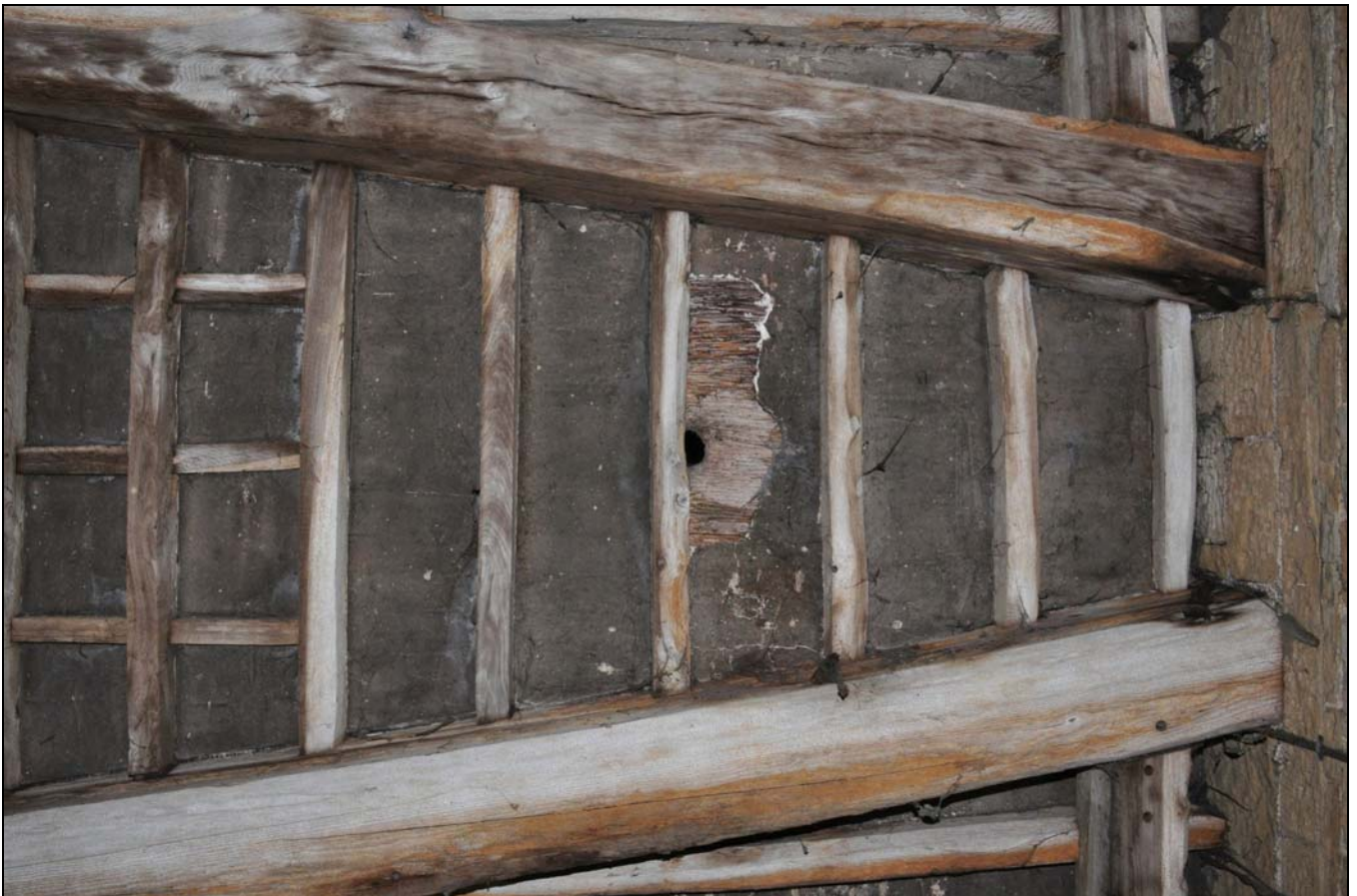
Photo 24: Underside of first floor in centre of building, looking south-west
