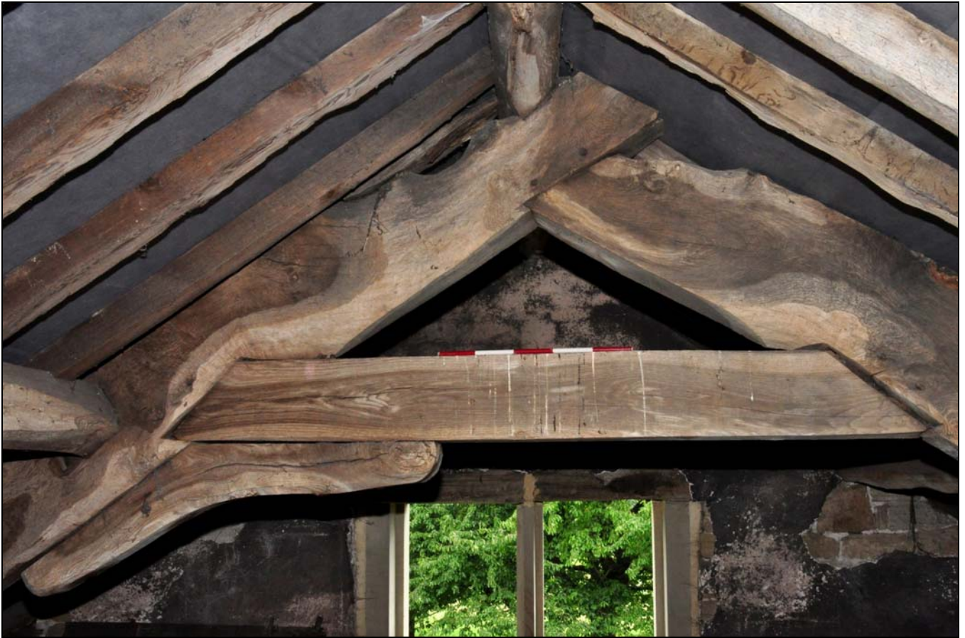
Photo 45: Detail of collar in north-west truss, looking north-west
