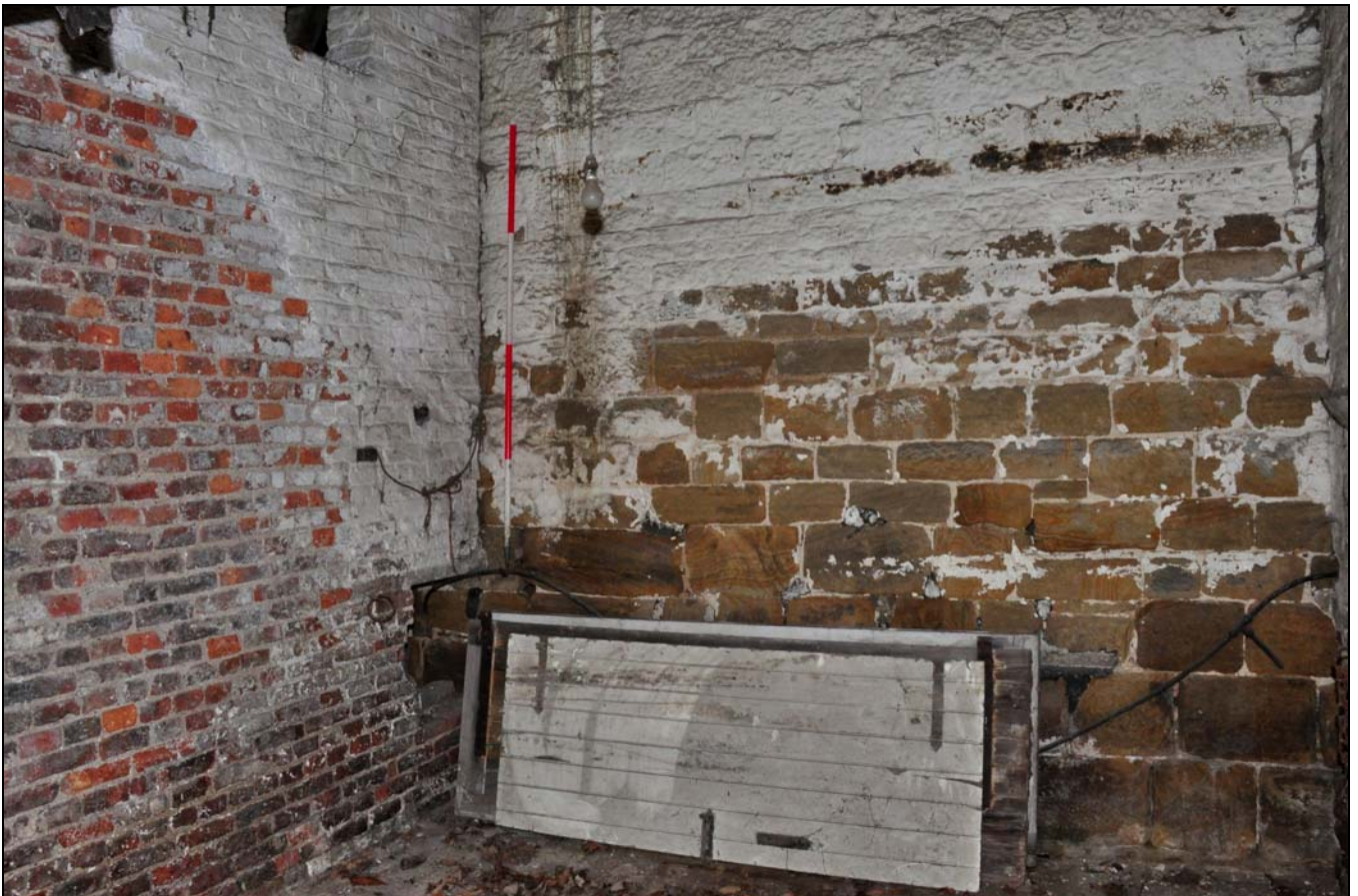
Photo 56: Central bay of rear lean-to, looking south
