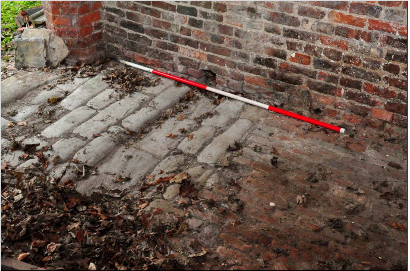
Photo 57: Floor surfaces in central bay of rear lean-to, looking east
