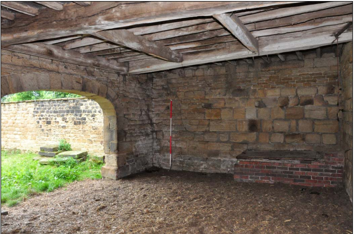
Photo 16: Ground floor of cart-shed, looking into west corner
