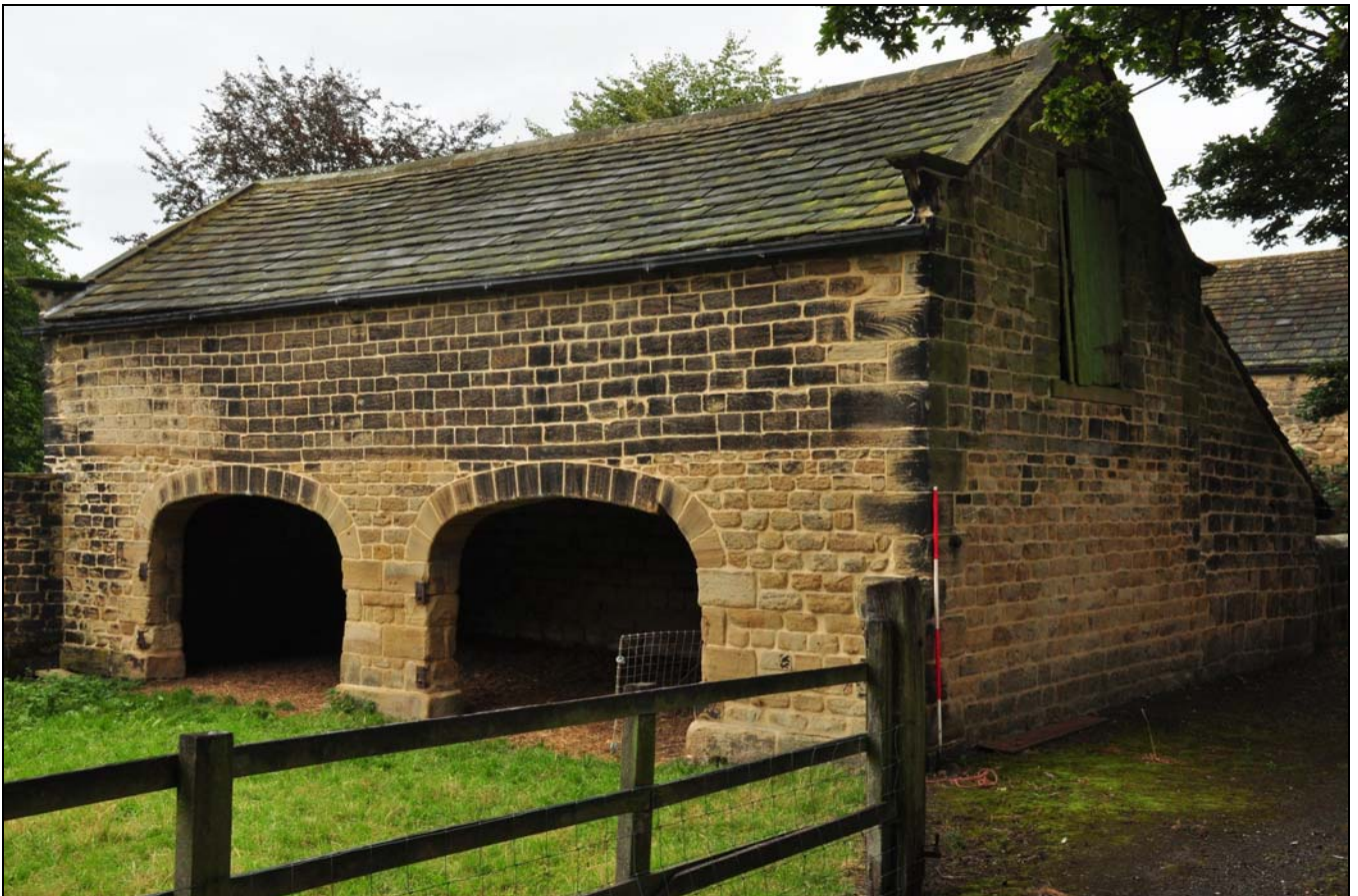
Photo 6: General view of the building, looking north
