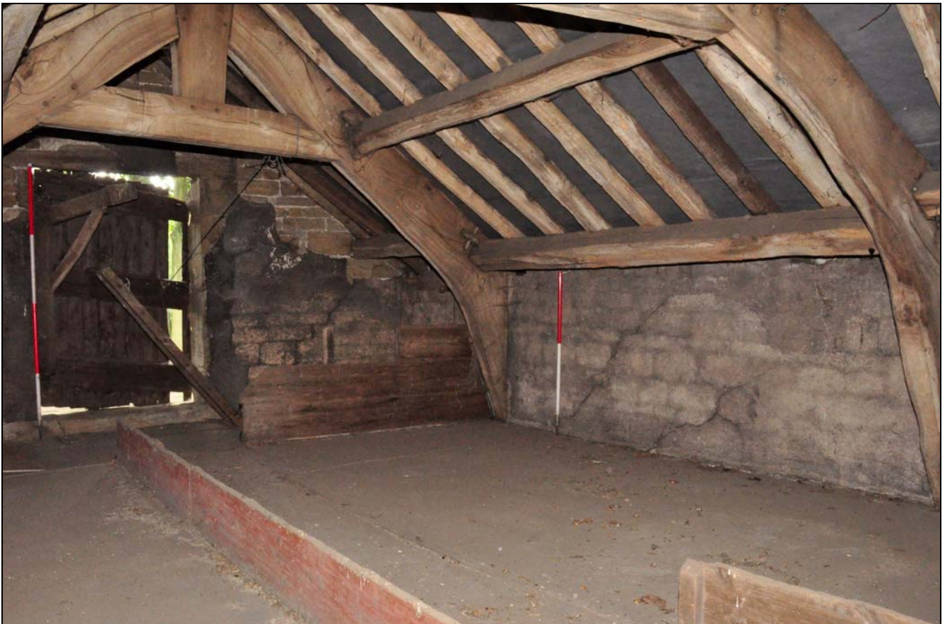
Photo 28: First floor, looking south
