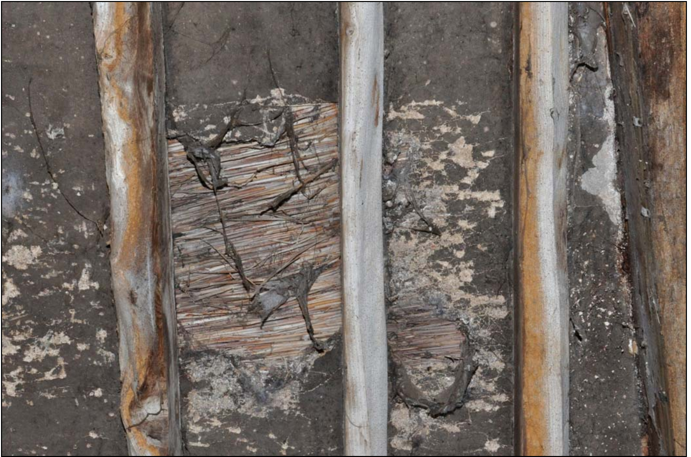
Photo 31: Underside of first floor, showing exposed reeds below lime-ash floor
