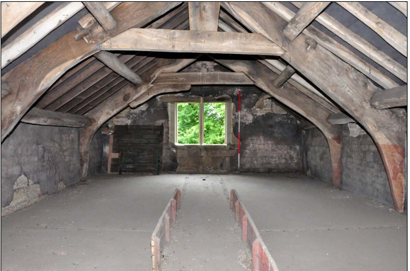
Photo 38: First floor, looking north-west
