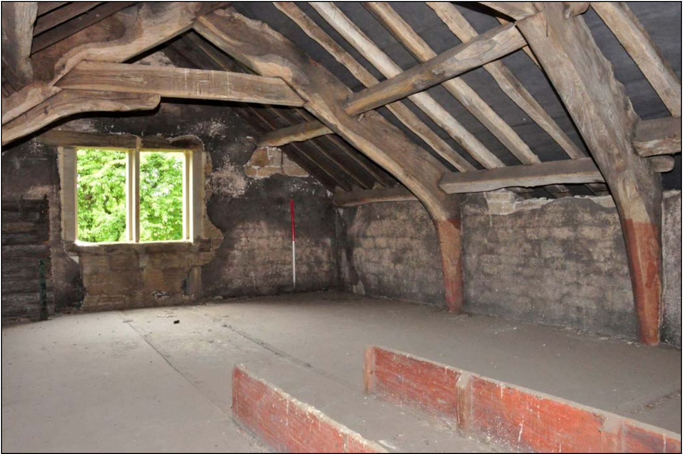
Photo 29: First floor, looking north
