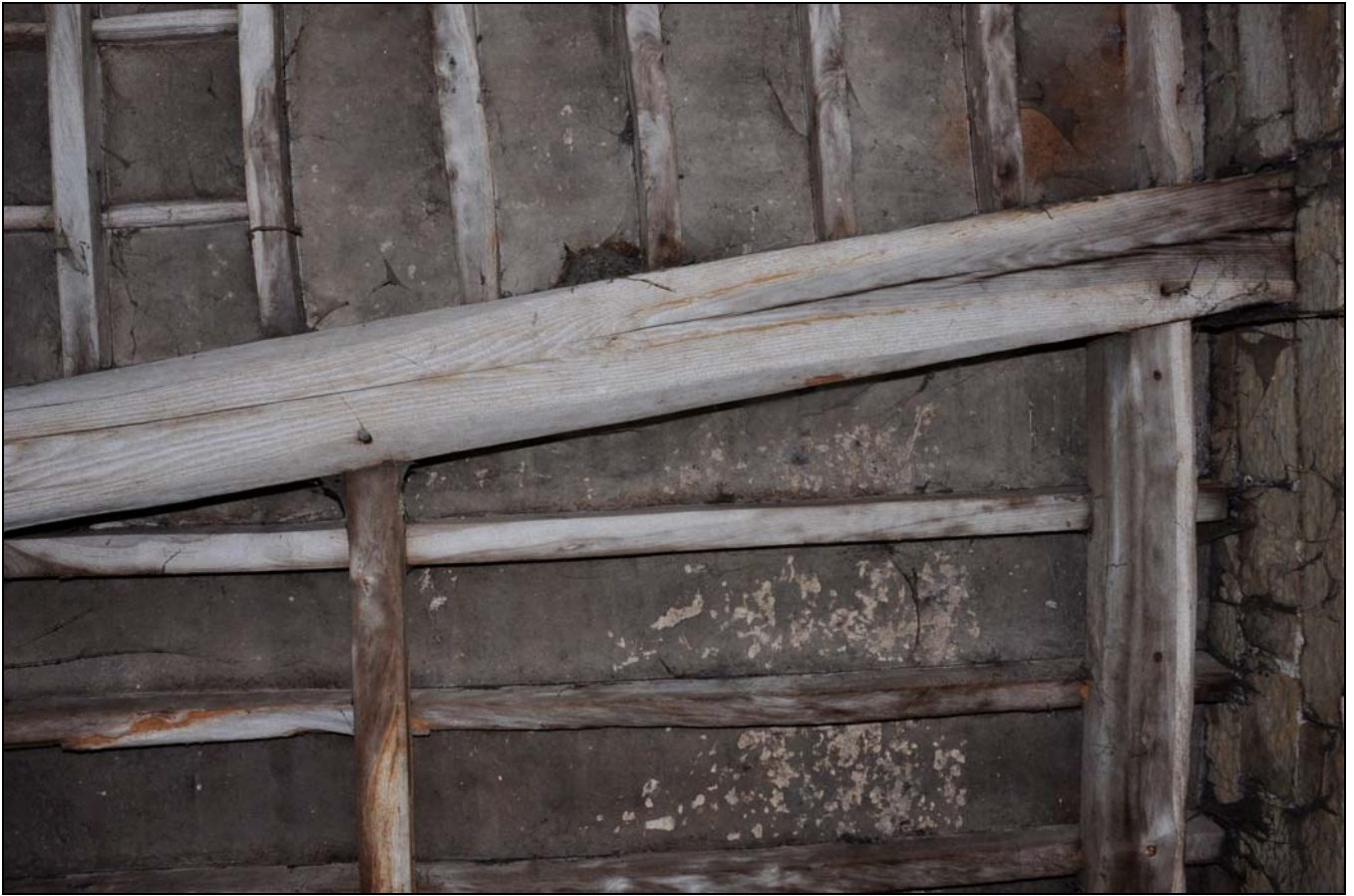
Photo 27: Underside of first floor by front arch, with pegs/peg-holes in beam
