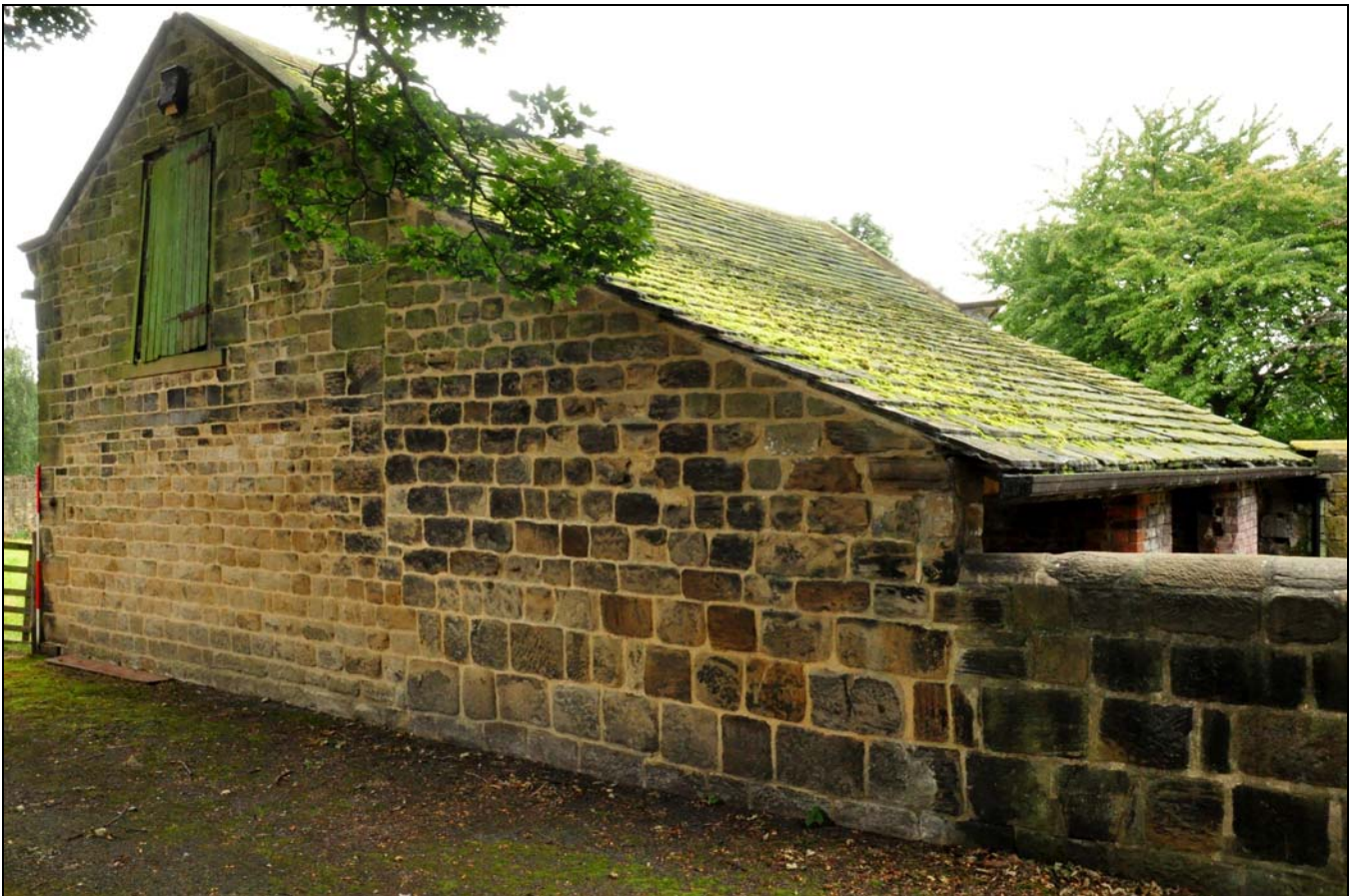
Photo 12: General view of the building, looking west
