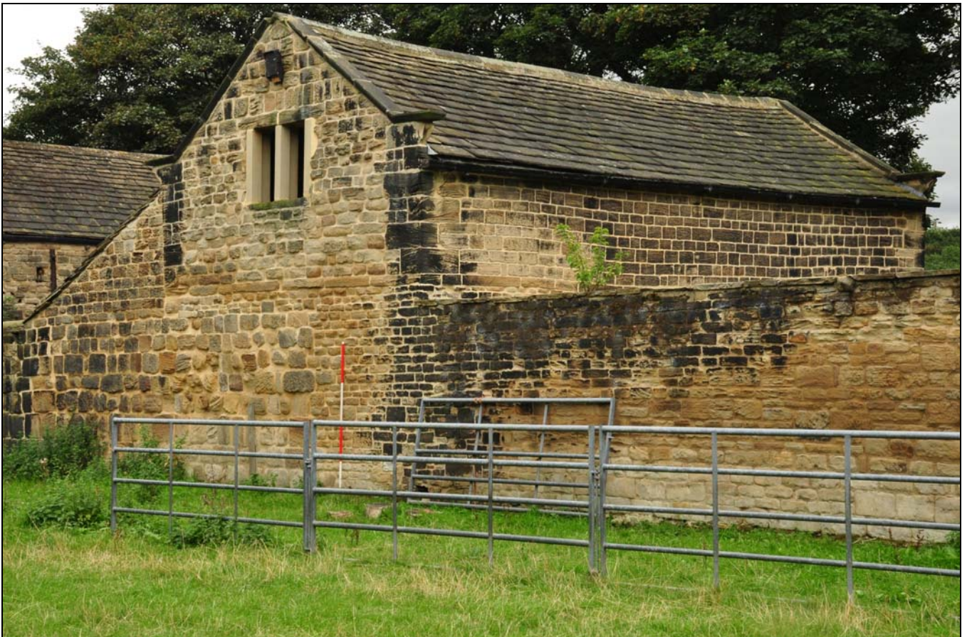
Photo 8: General view of the building, looking east
