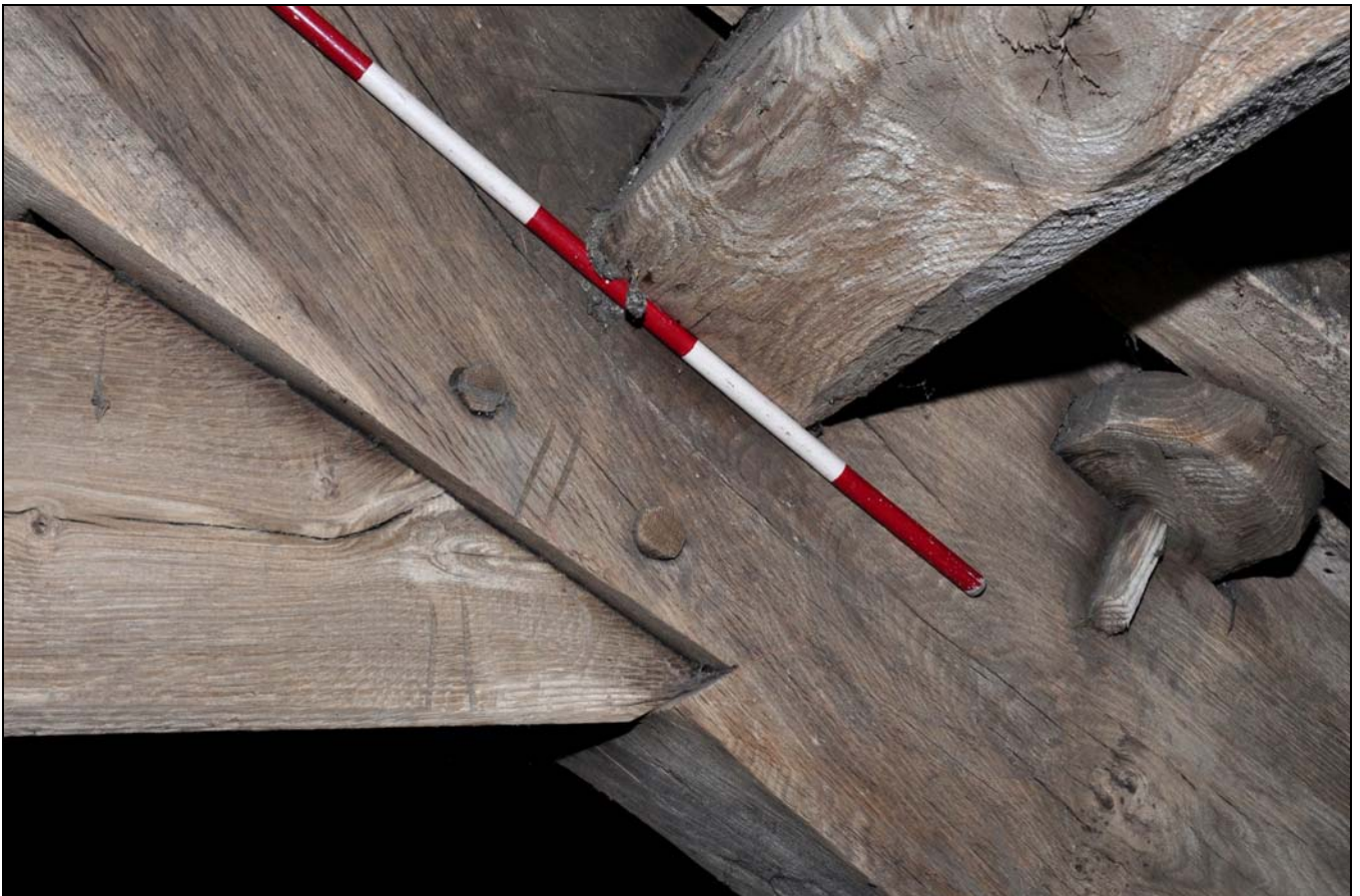
Photo 50: Detail of joint numbering and purlin tenon, north-east side of roof
