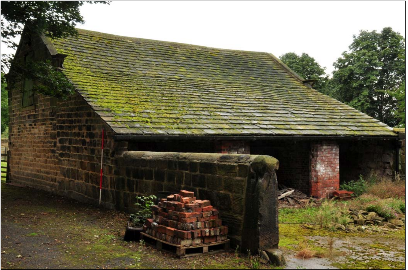
Photo 51: General view of the rear lean-to, looking west
