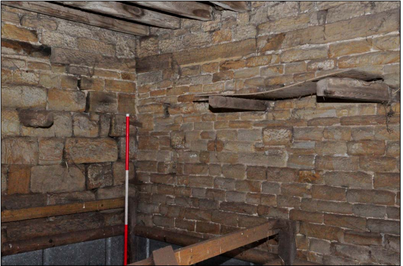
Photo 21: Ground floor of cart-shed, looking towards east corner, with oak brackets in wall
