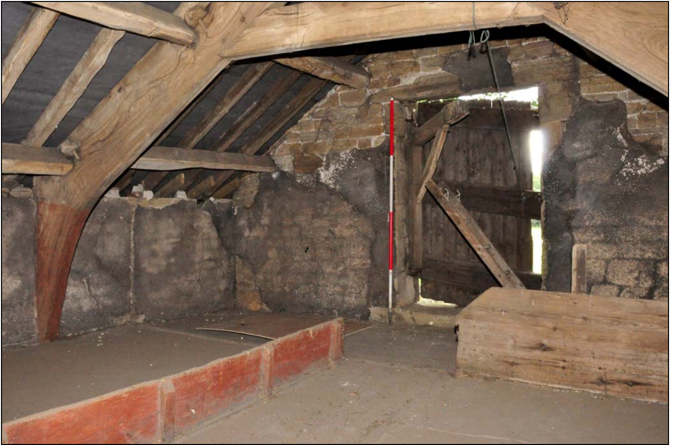
Photo 41: View towards east corner of first floor
