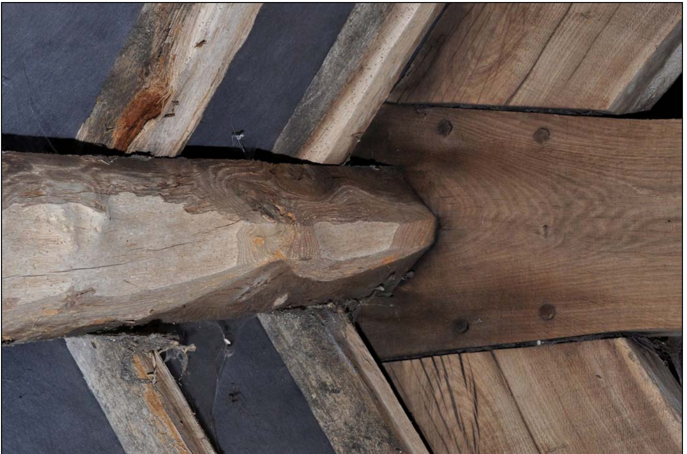
Photo 47: Detail of joint numbering on collar at joint with cruck, south-east truss
