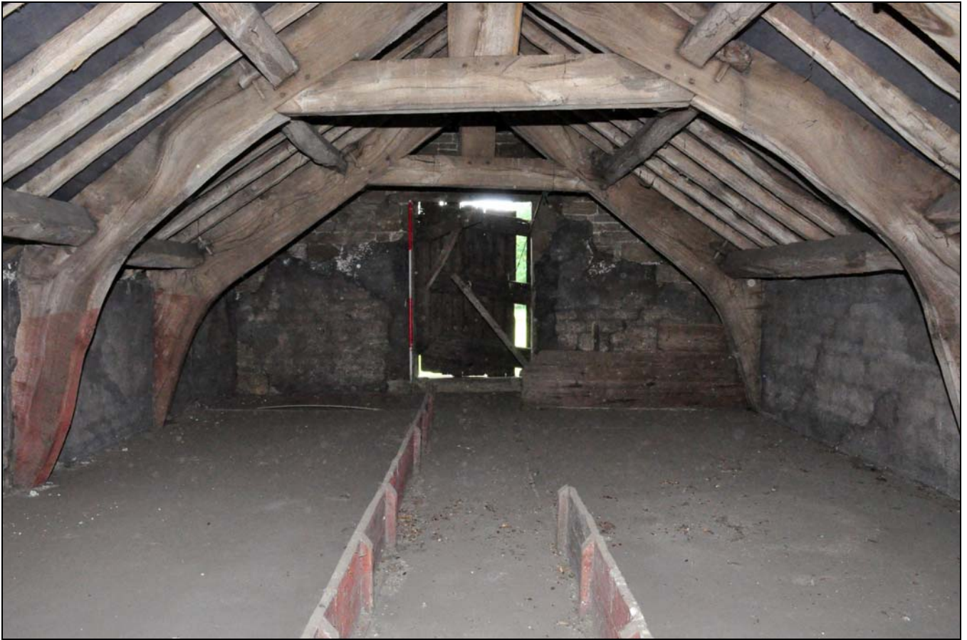
Photo 37: First floor, looking south-east
