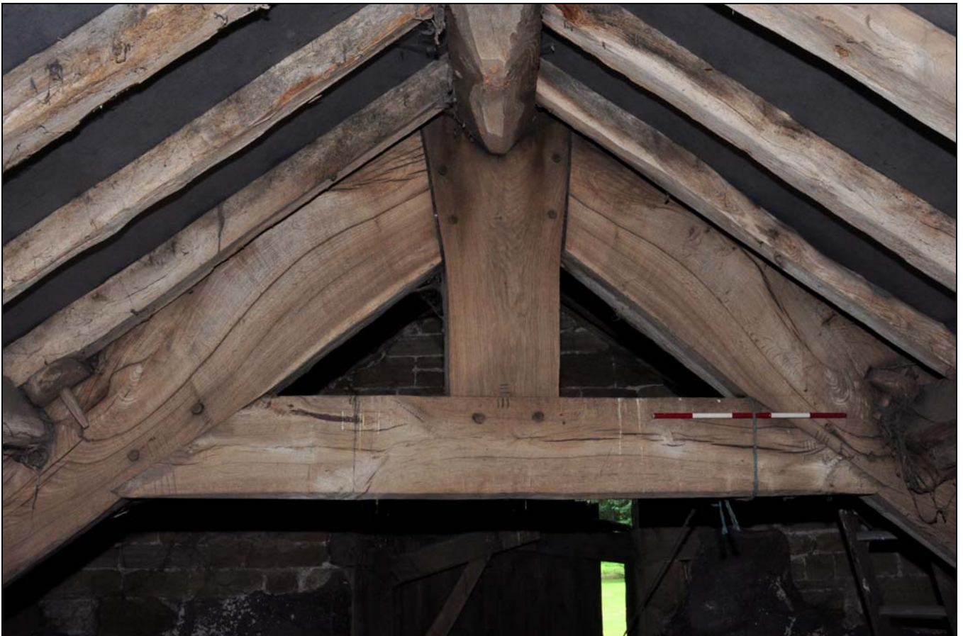
Photo 44: Detail of collar and king-post in south-east truss, looking south-east
