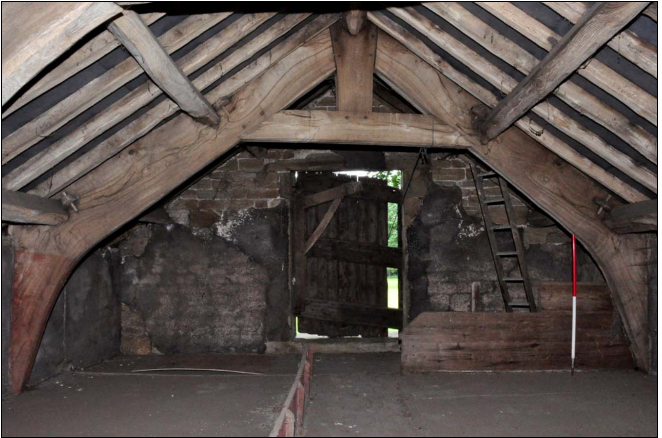
Photo 43: South-east truss, looking south-east
