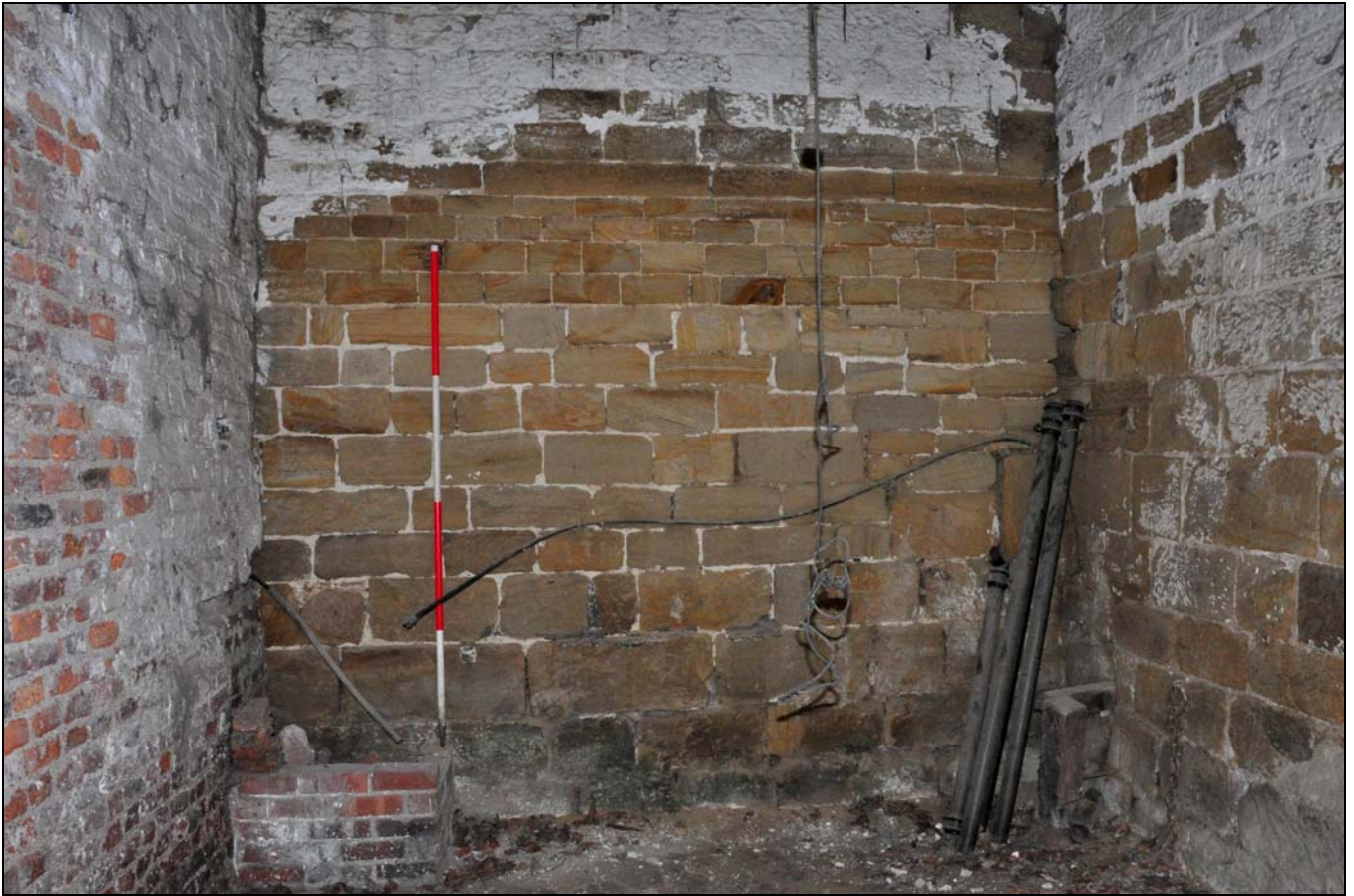
Photo 13: Rear of cart-shed within lean-to, looking south-west
