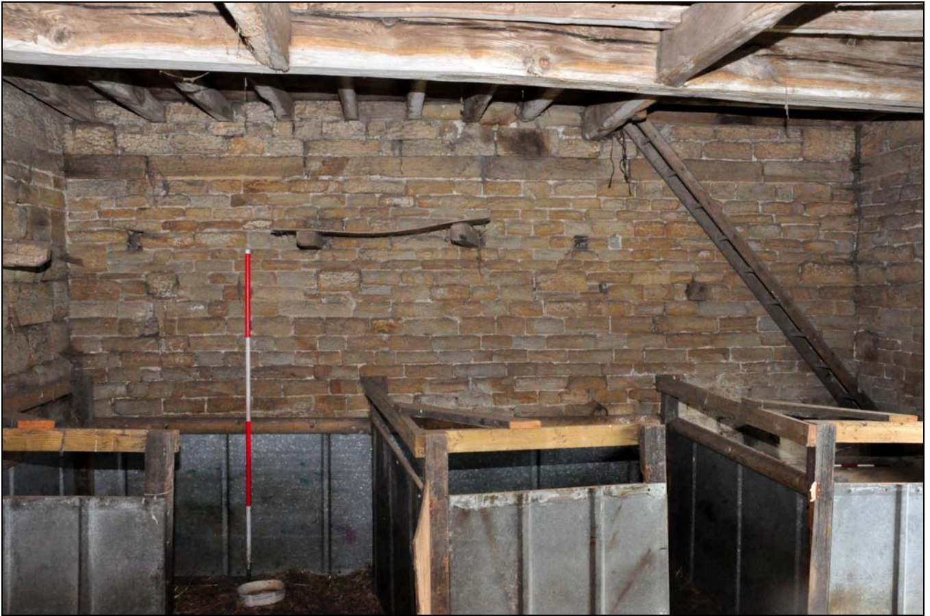
Photo 19: Ground floor of cart-shed, looking towards south-east wall
