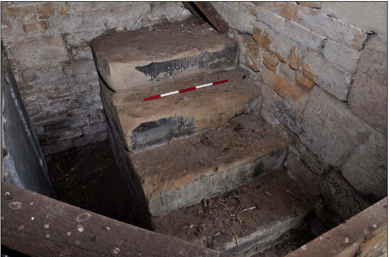
Photo 18: Detail of stone steps in south corner of ground floor
