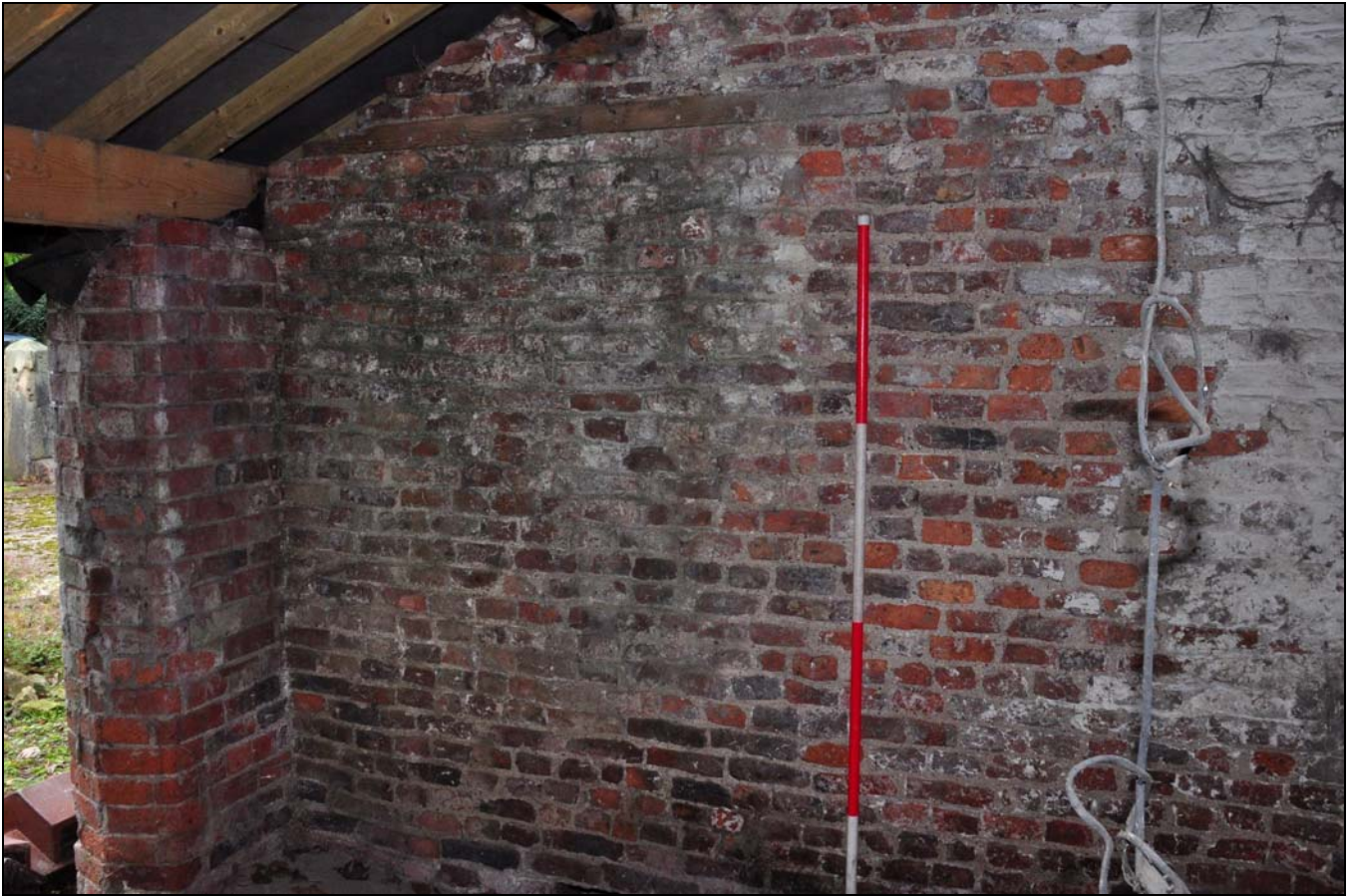
Photo 55: Cross-wall between bays 2 and 3 of rear lean-to, looking south-east
