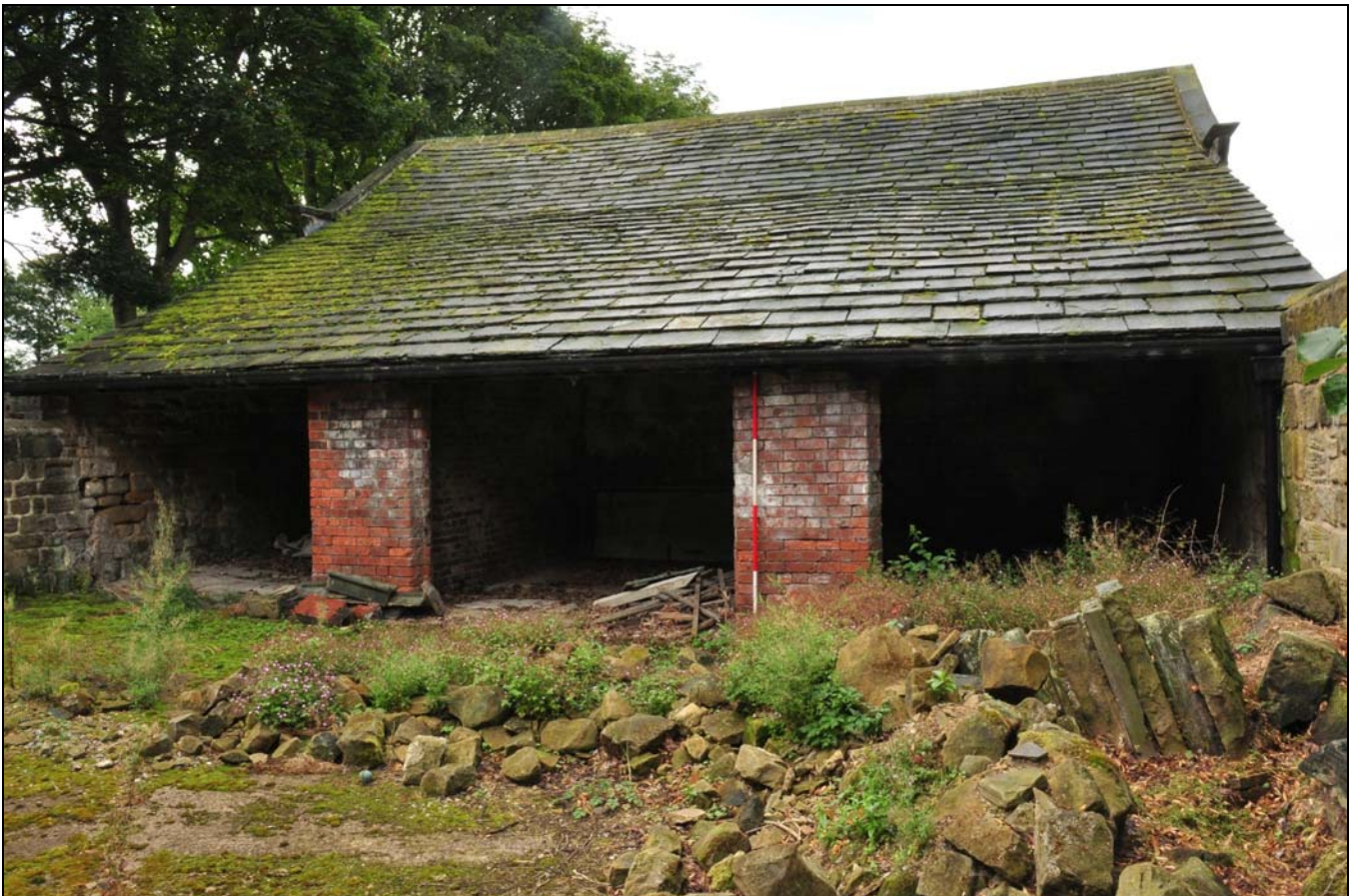
Photo 52: General view of the rear lean-to, looking south
