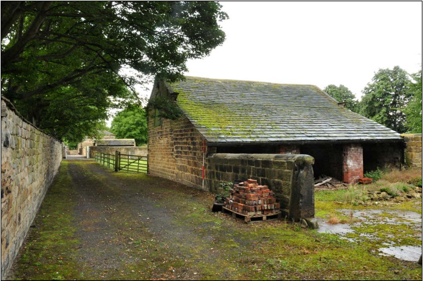
Photo 3: General view of the building, looking south-west
