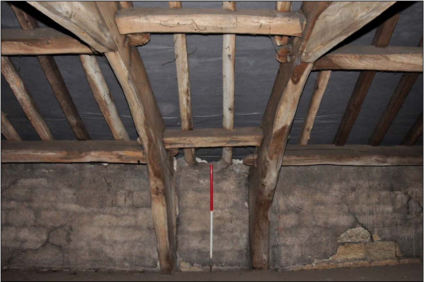
Photo 49: South-west side of first floor, showing closely spaced upper cruck trusses and short purlins
