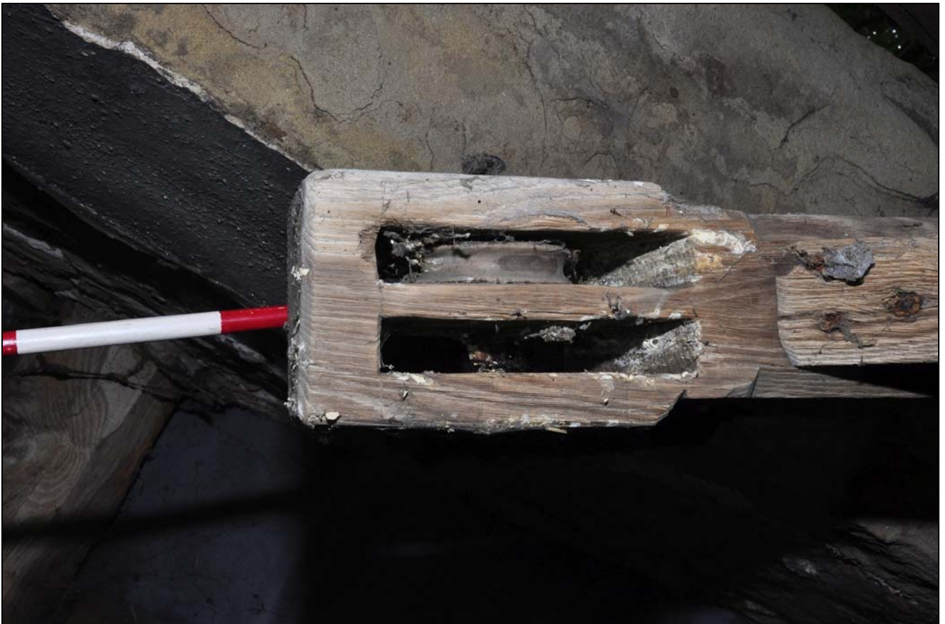
Photo 36: Detail of underside of crane jib, with wooden pulley
