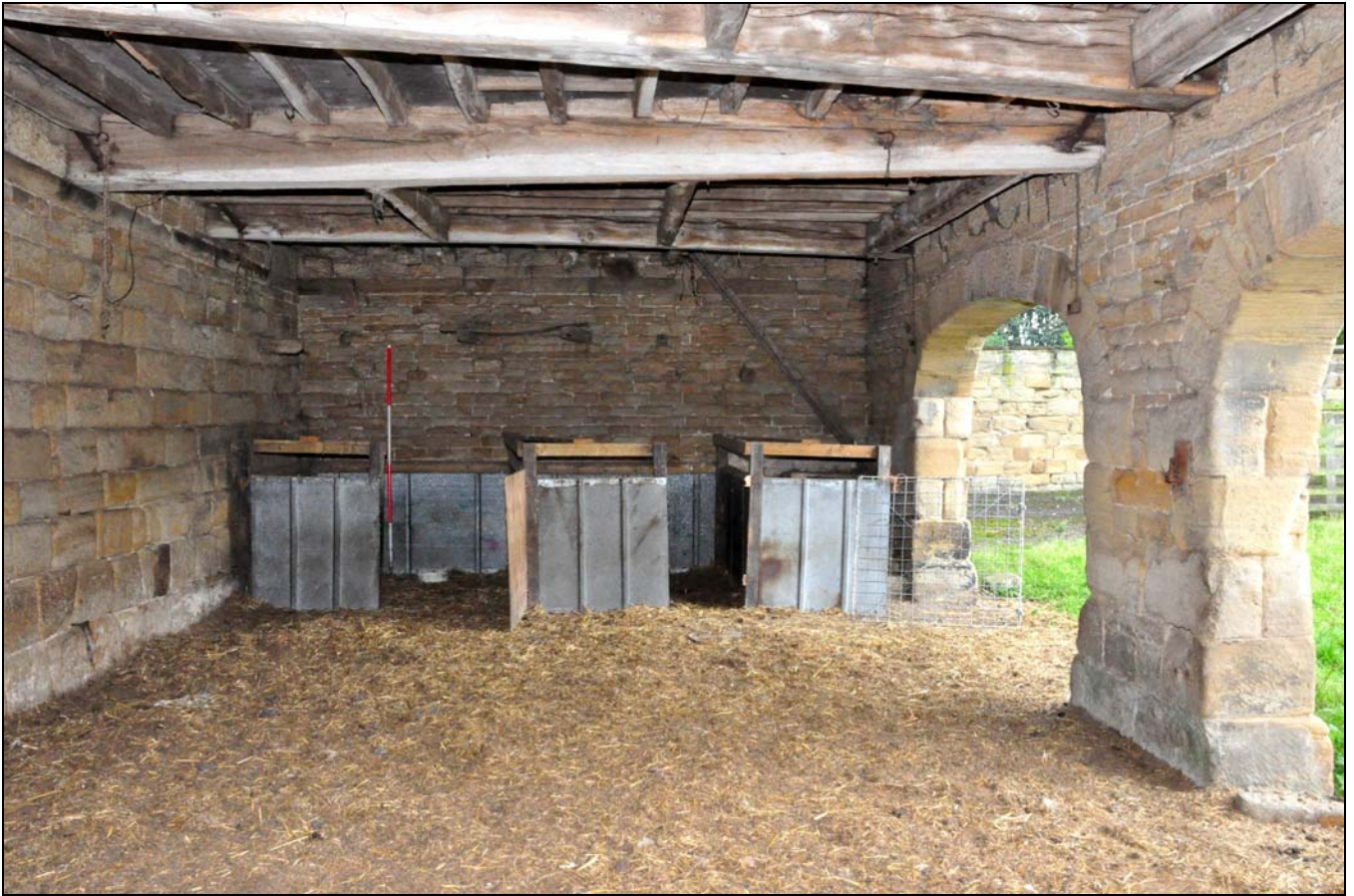
Photo 15: Ground floor of cart-shed, looking south-east
