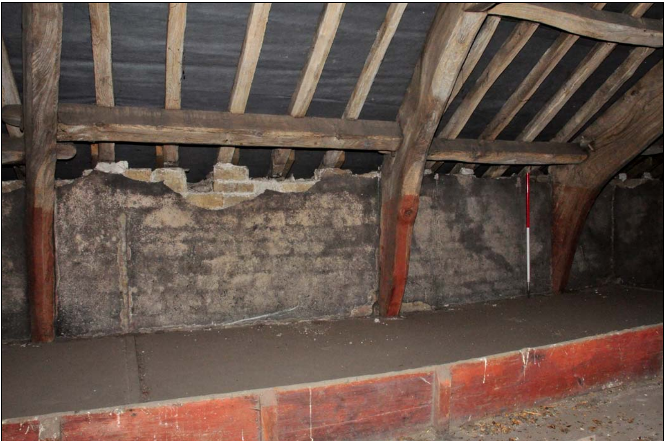
Photo 42: North-east side of first floor, with traces of removed partition
