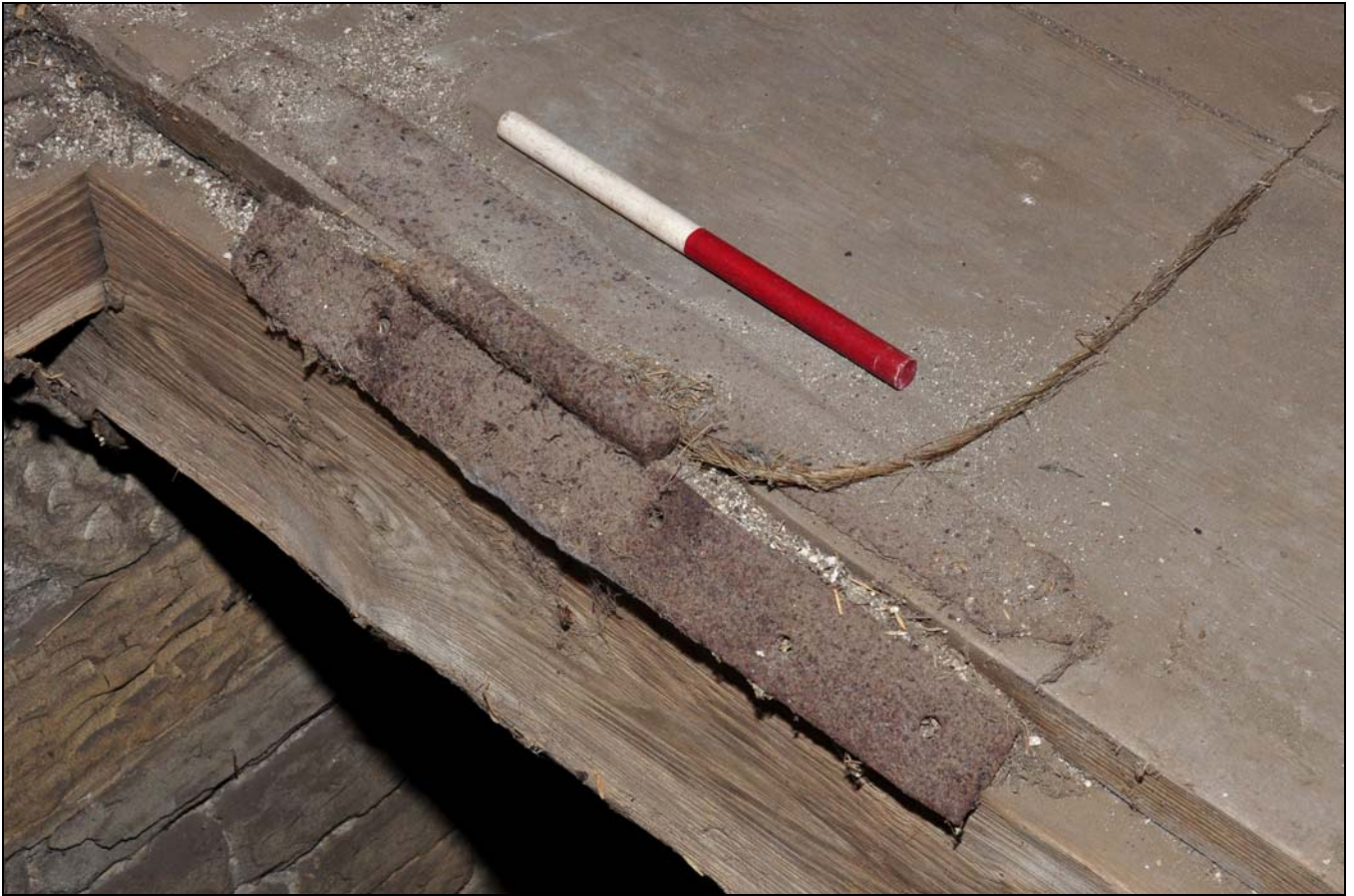
Photo 33: Detail of hinge from trap-door in first floor, looking west
