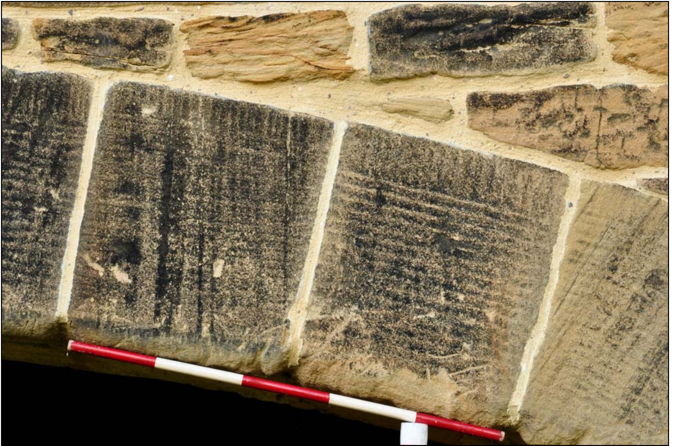
Photo 5: Detail of voussoirs to left-hand arch, front elevation
