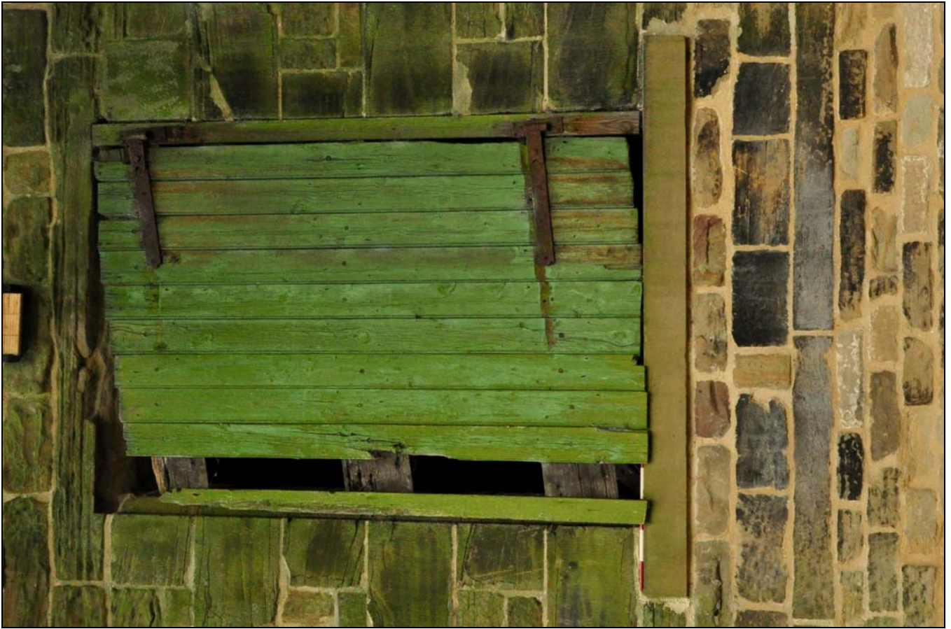
Photo 11: Loading door in south-east gable
