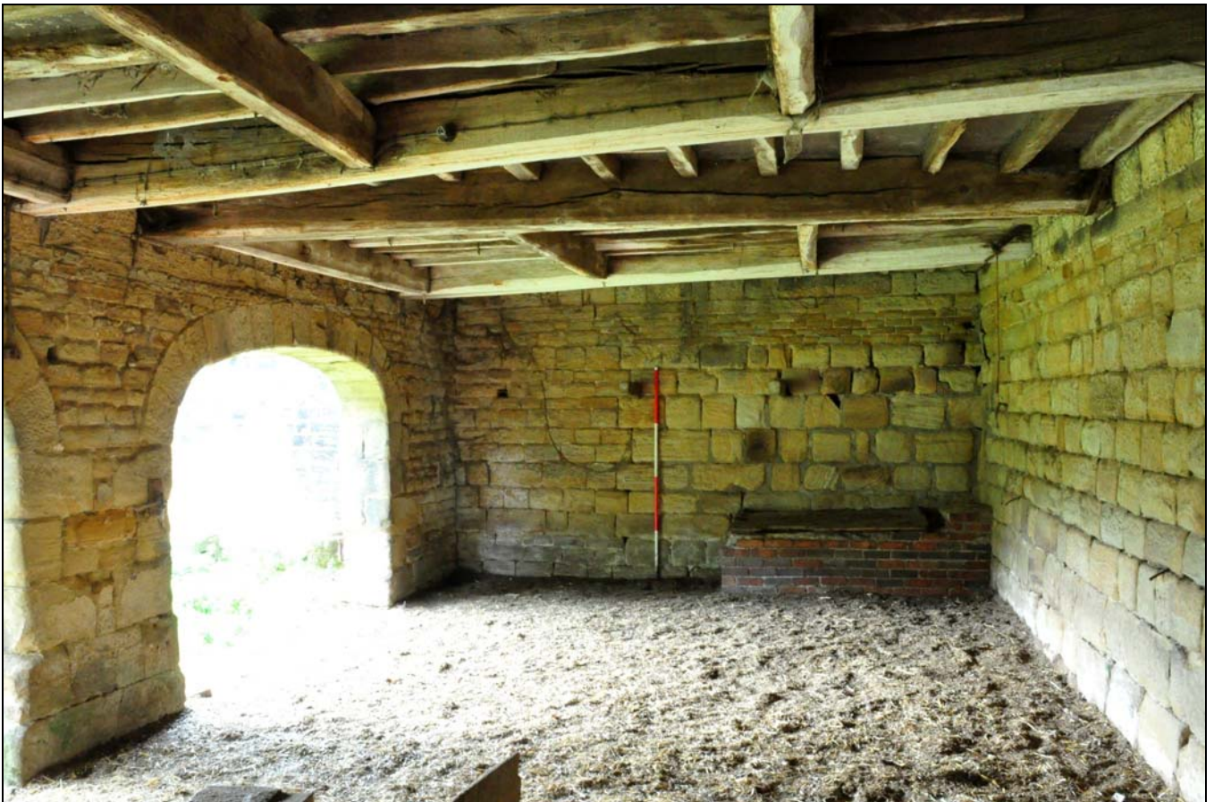
Photo 14: Ground floor of cart-shed, looking north-west
