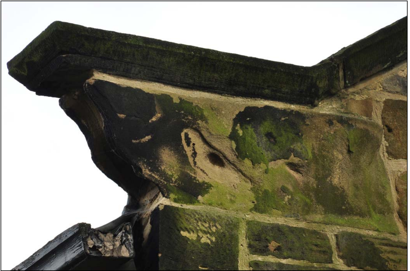
Photo 7: Detail of kneeler at south corner
