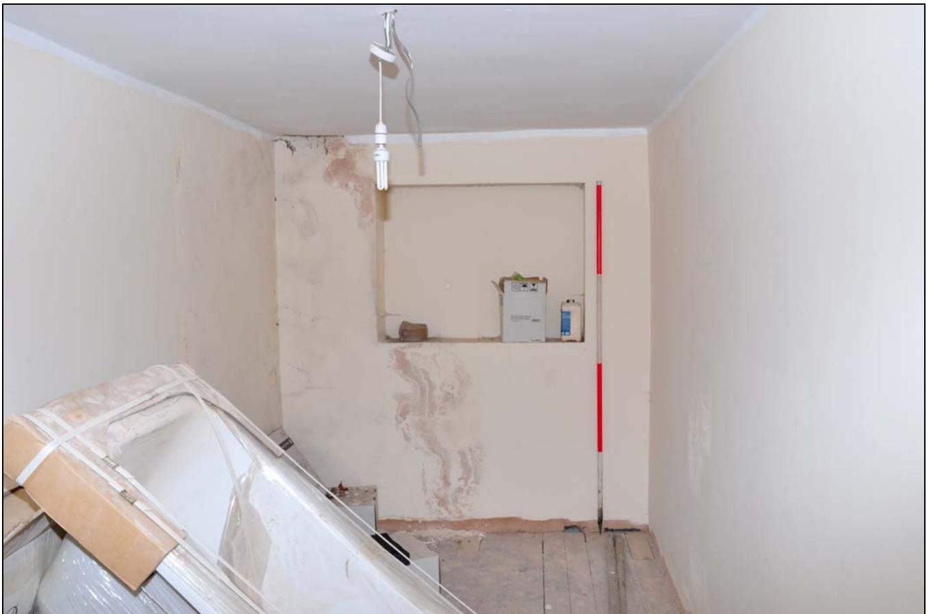
Photo 94: First floor: R28, looking west, to blocked window
