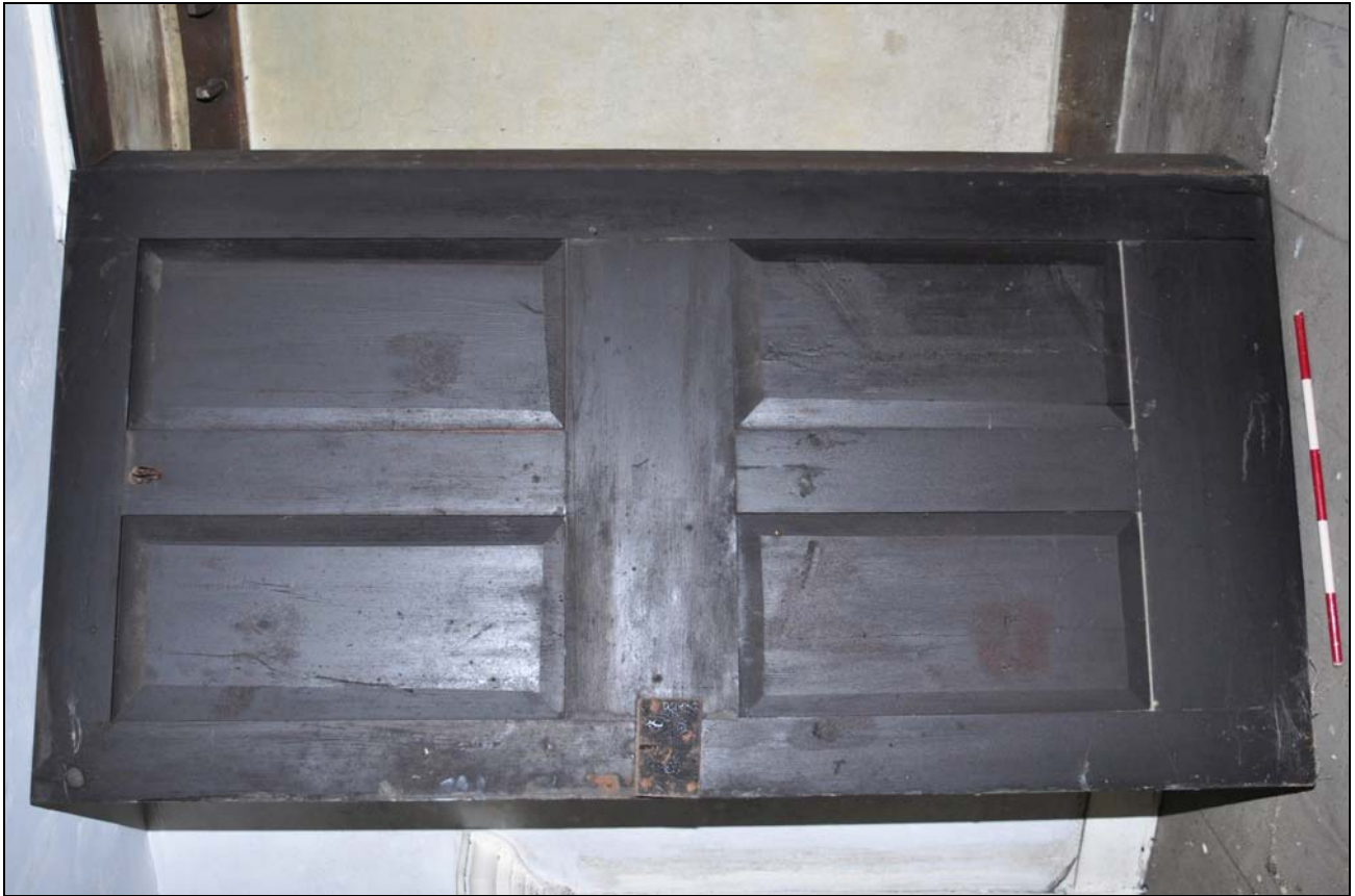
Photo 127: Second floor: R44, detail of door to cupboard (inner face)
