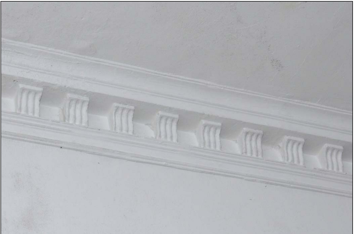
Photo 74: First floor: R20 (main landing), detail of ceiling cornice
