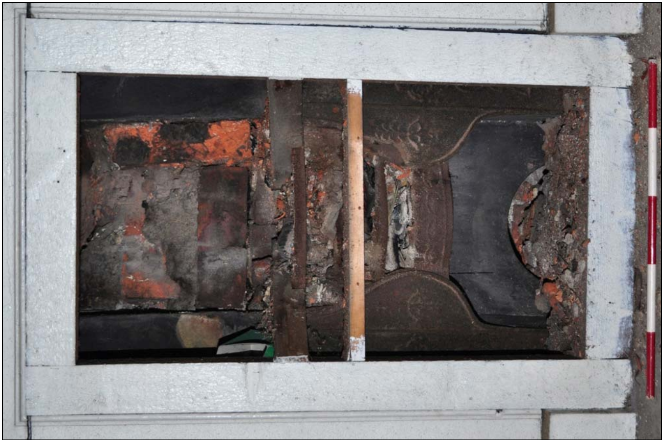
Photo 119: Second floor: R38 (C19 addition), detail of fireplace
