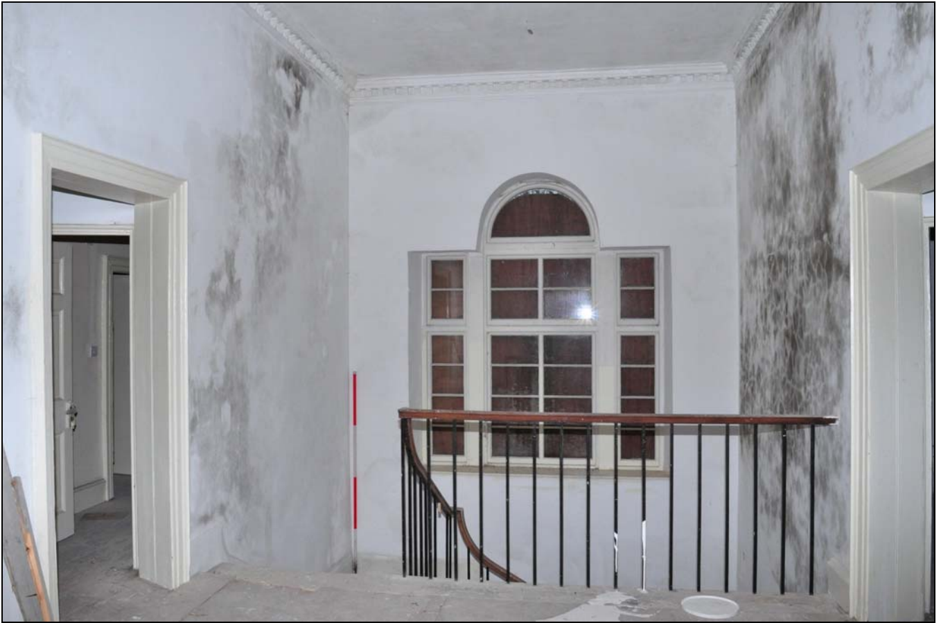
Photo 73: First floor: R20 (main landing), looking north
