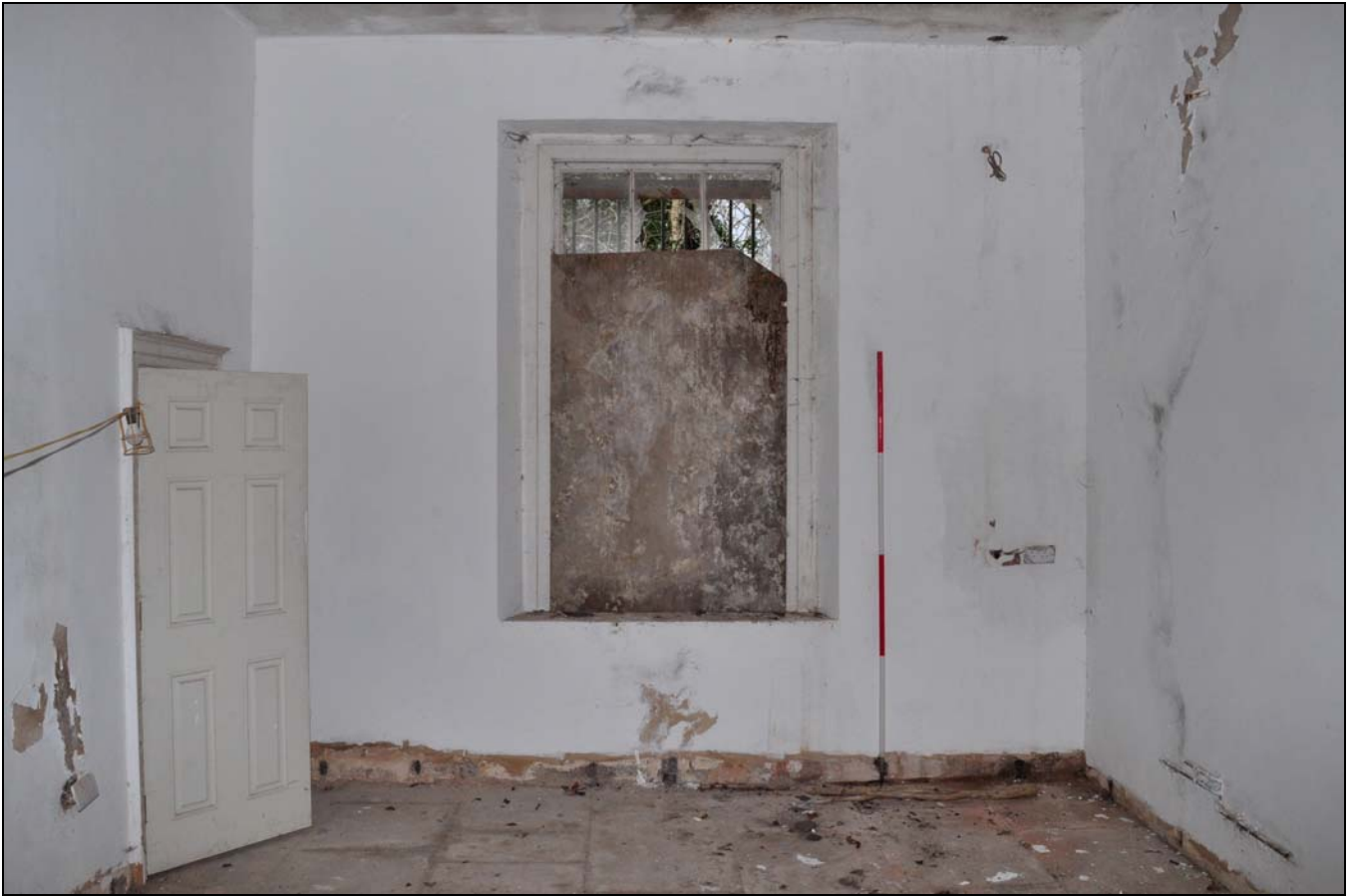
Photo 53: Ground floor: R5, looking west
