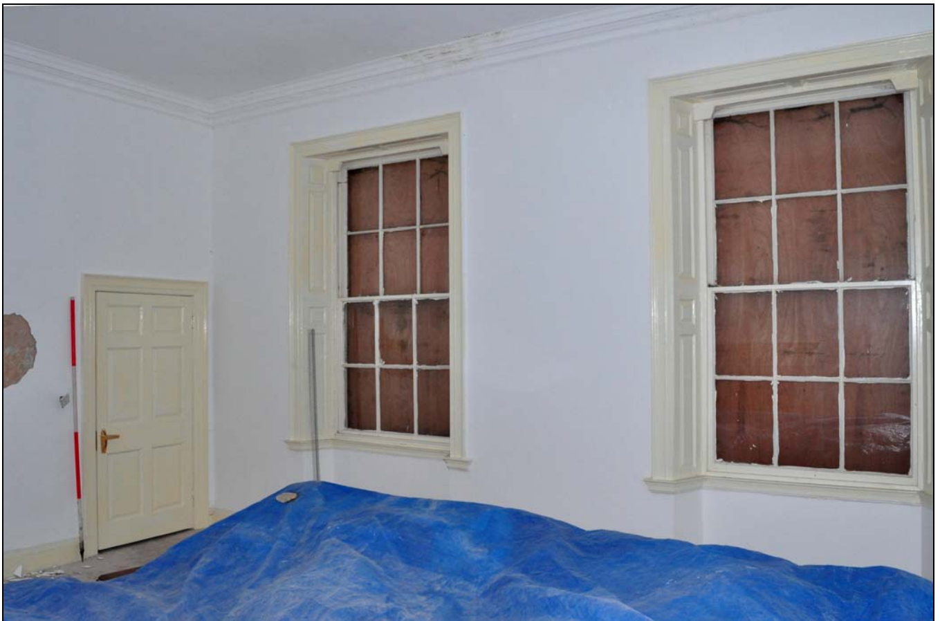
Photo 78: First floor: R22, looking south-east
