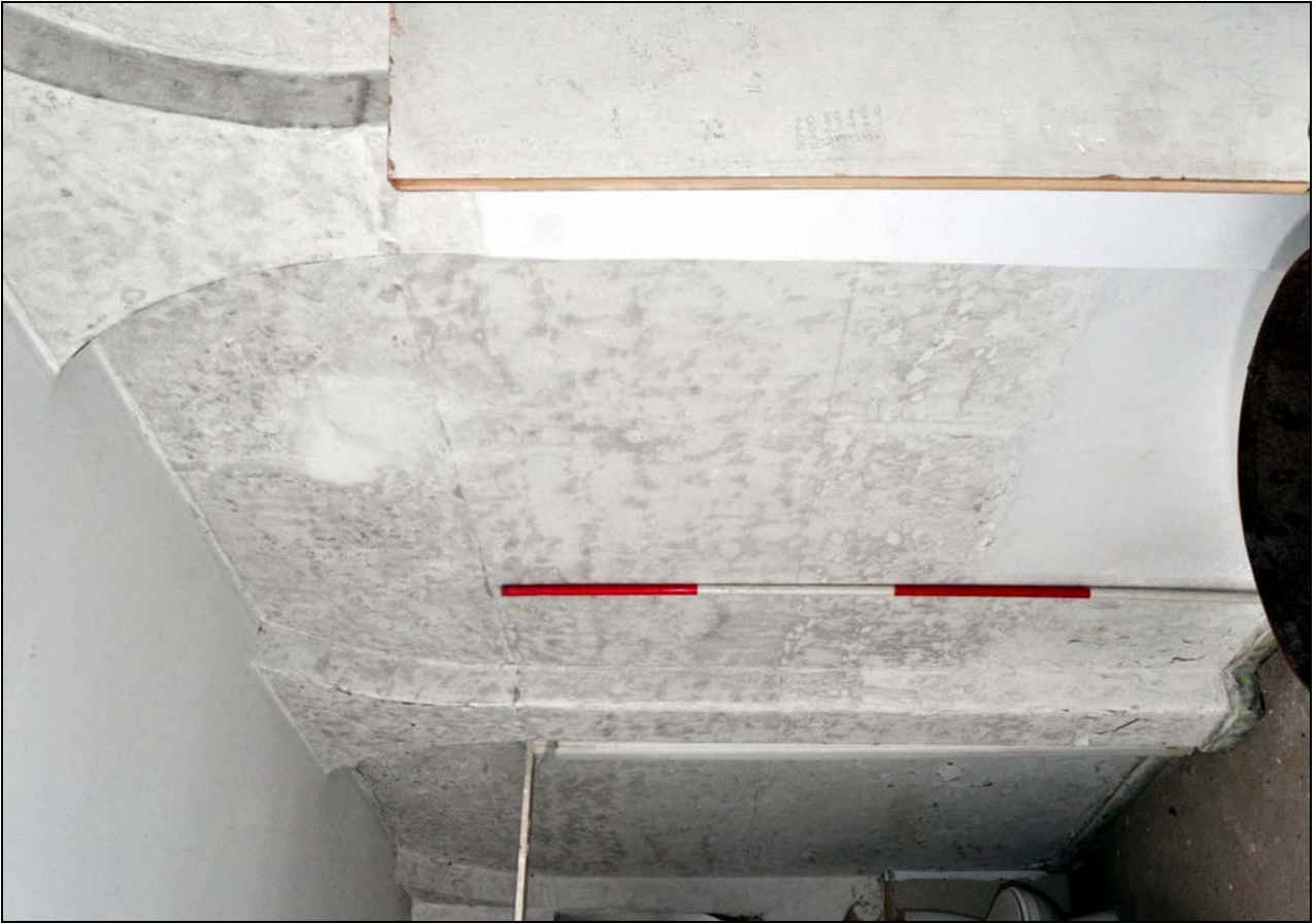
Photo 61: Ground floor: R11, looking south-east towards blind arcade
