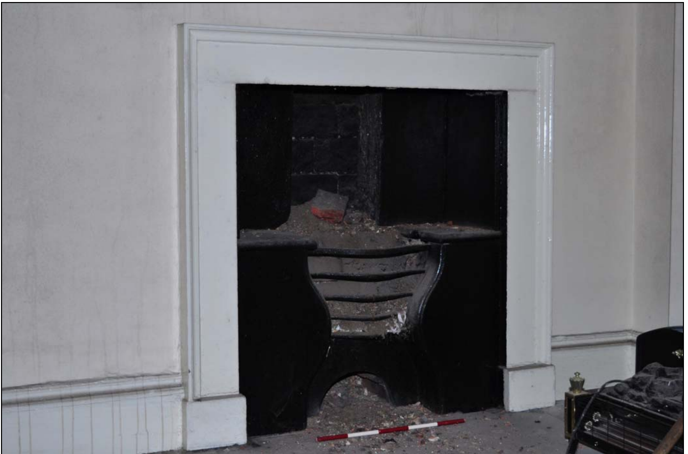
Photo 108: First floor: R36, detail of fireplace
