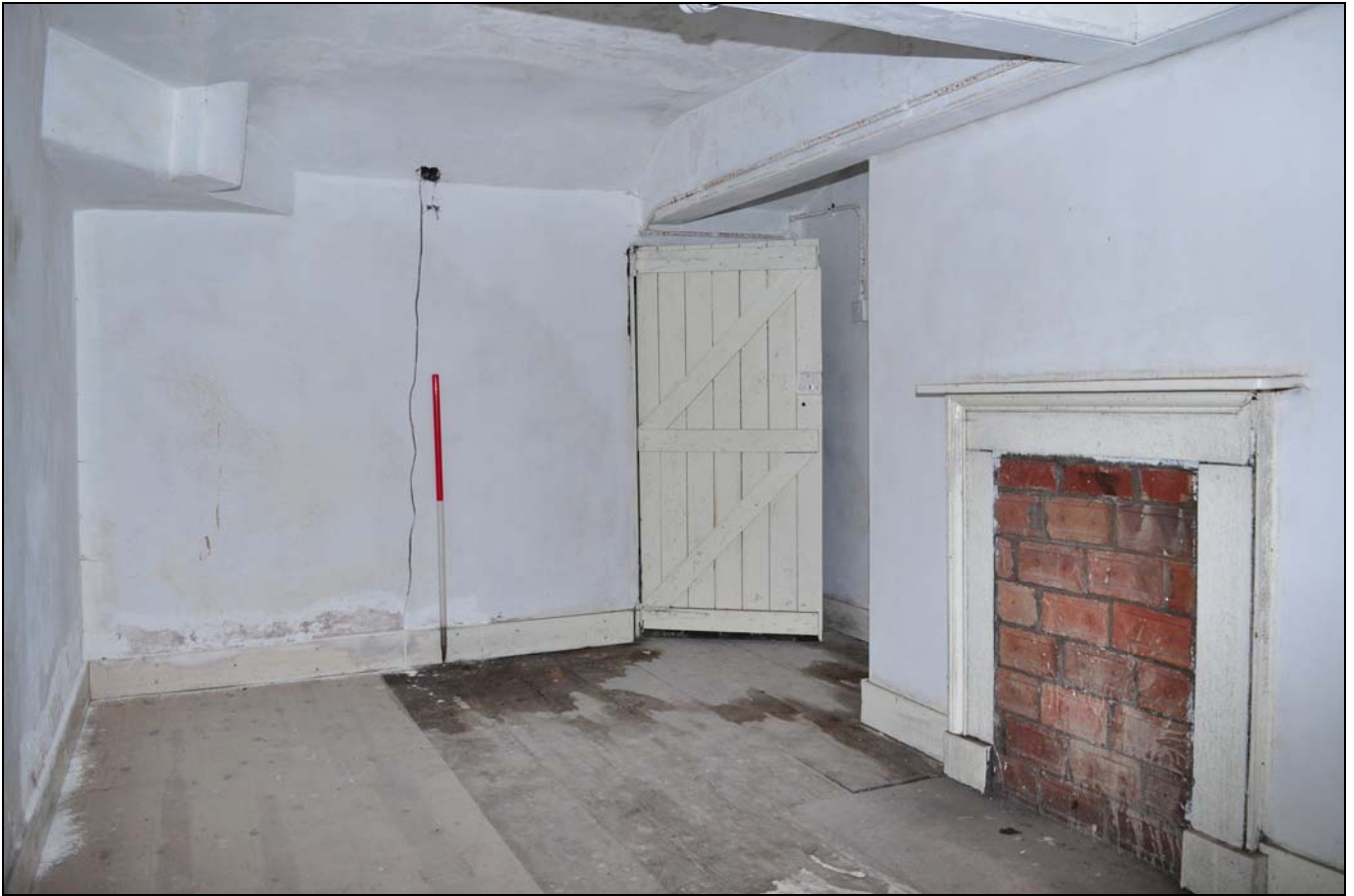
Photo 121: Second floor: R42 (C19 addition), looking south-east
