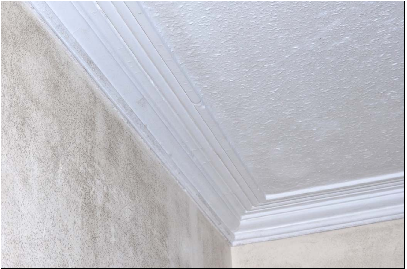
Photo 101: First floor: R33, detail of ceiling cornice, looking north-west
