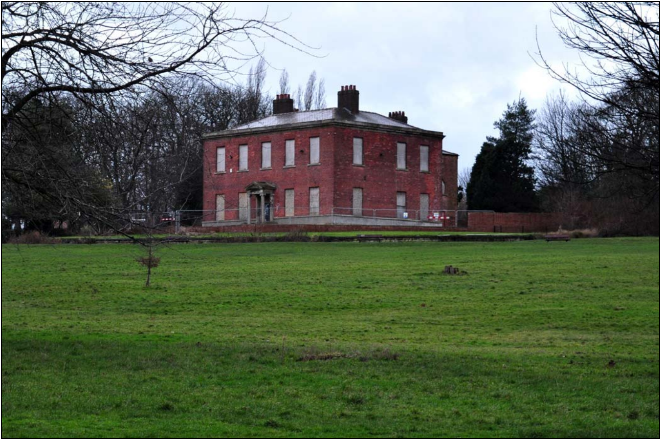
Photo 1: Distant view of Carr Lodge, from the south-east
