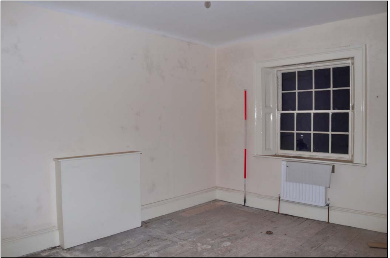
Photo 99: First floor: R32, looking south-west
