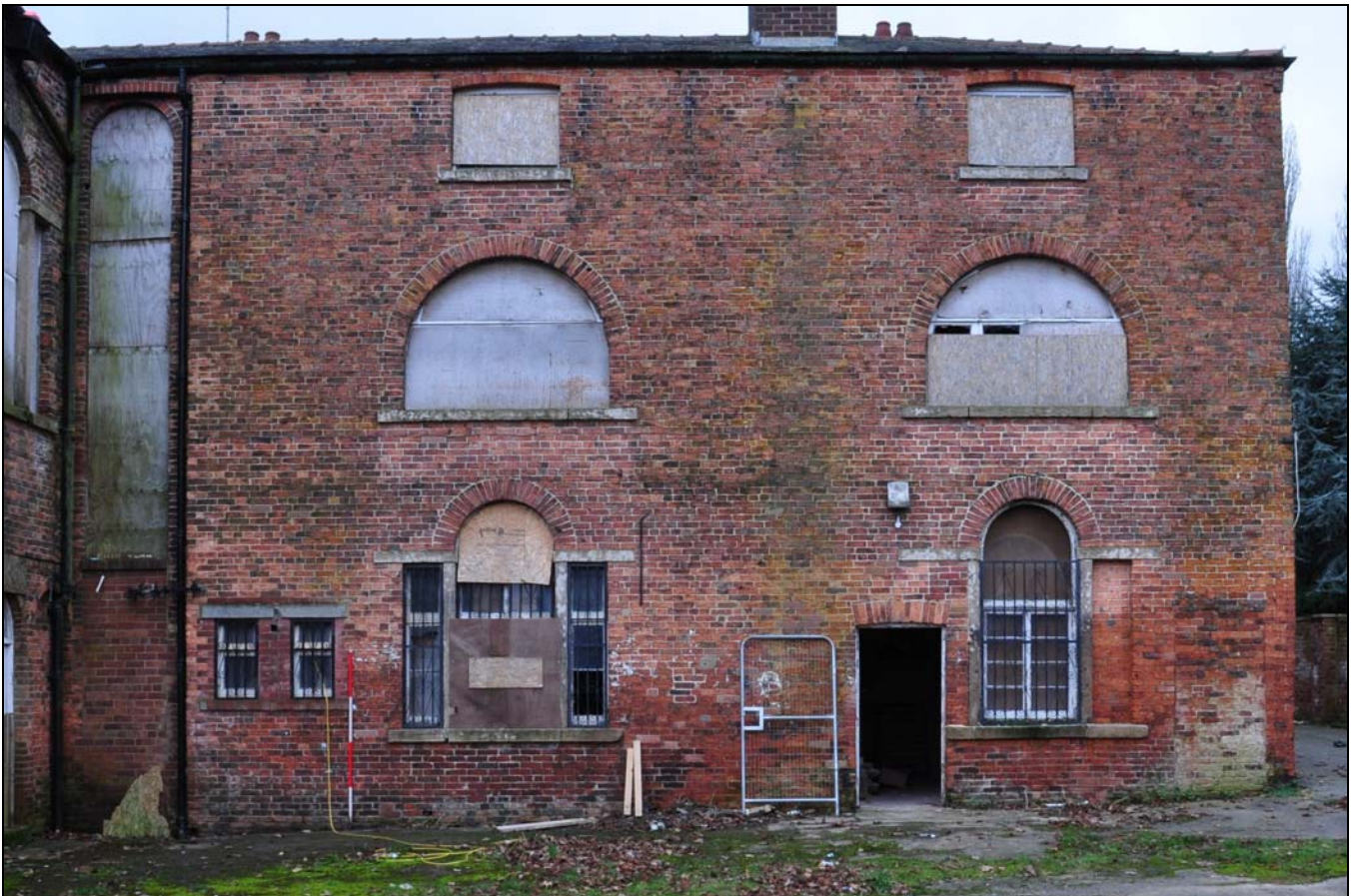
Photo 26: East elevation of rear range
