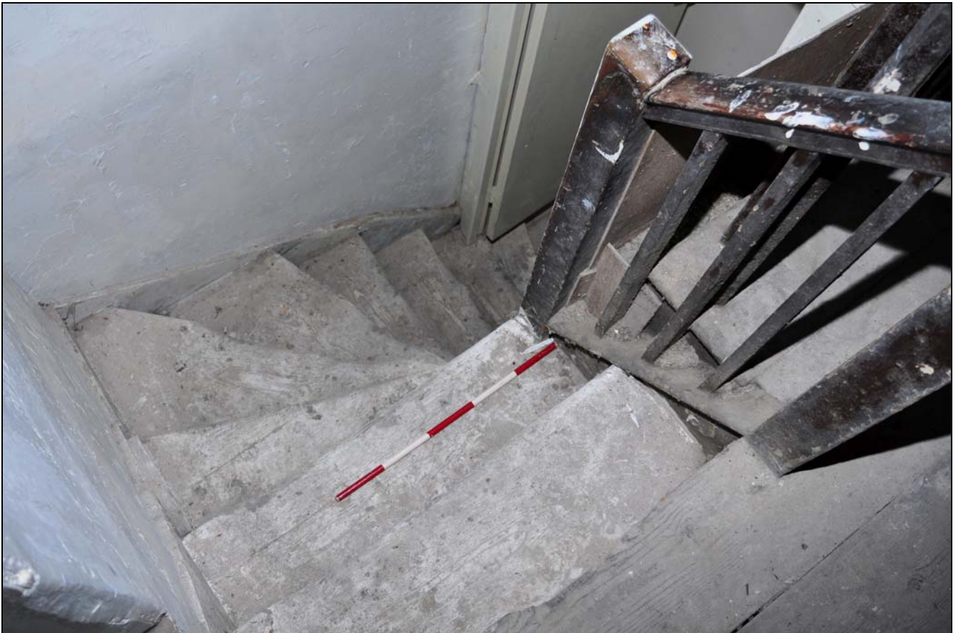
Photo 110: Second floor: R37, looking down stairs towards first floor
