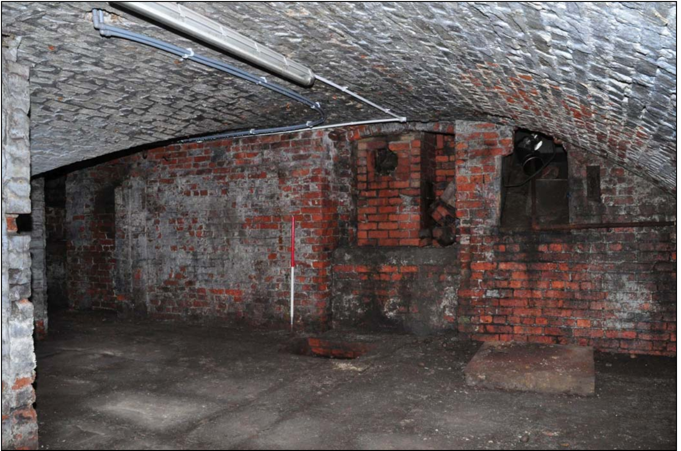
Photo 71: Cellar: R19 (east barrel vault), looking north-west
