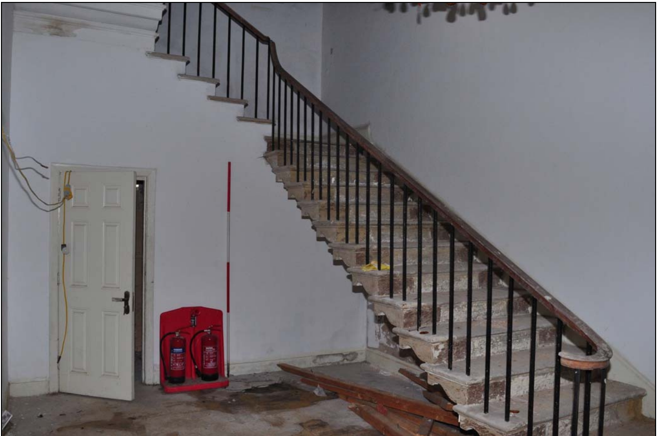
Photo 54: Ground floor: R6 (stair hall), looking north-east
