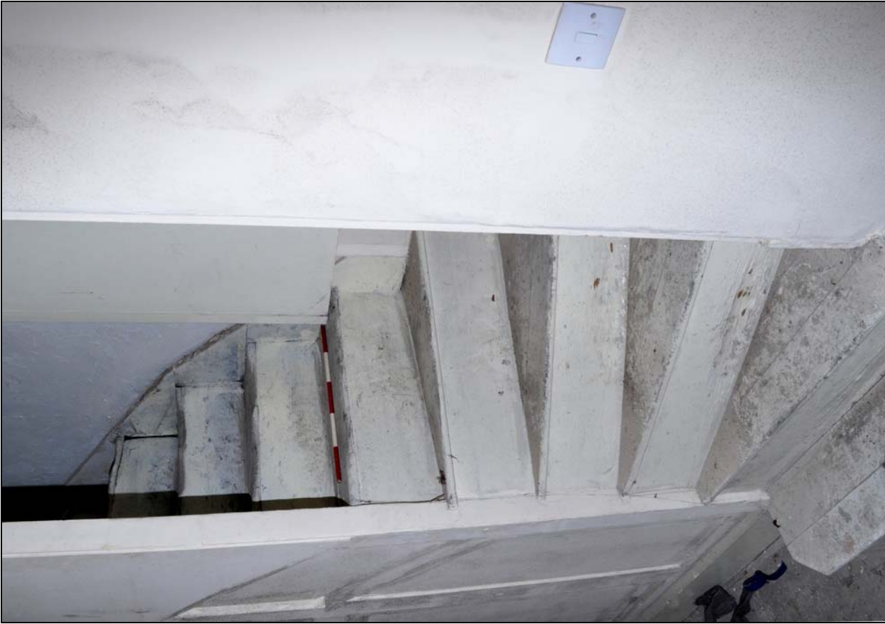
Photo 109: First floor: R30, detail of stairs to second floor, looking north-east
