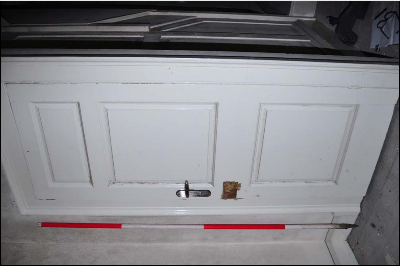
Photo 111: First floor: R30, detail of door to understairs cupboard
