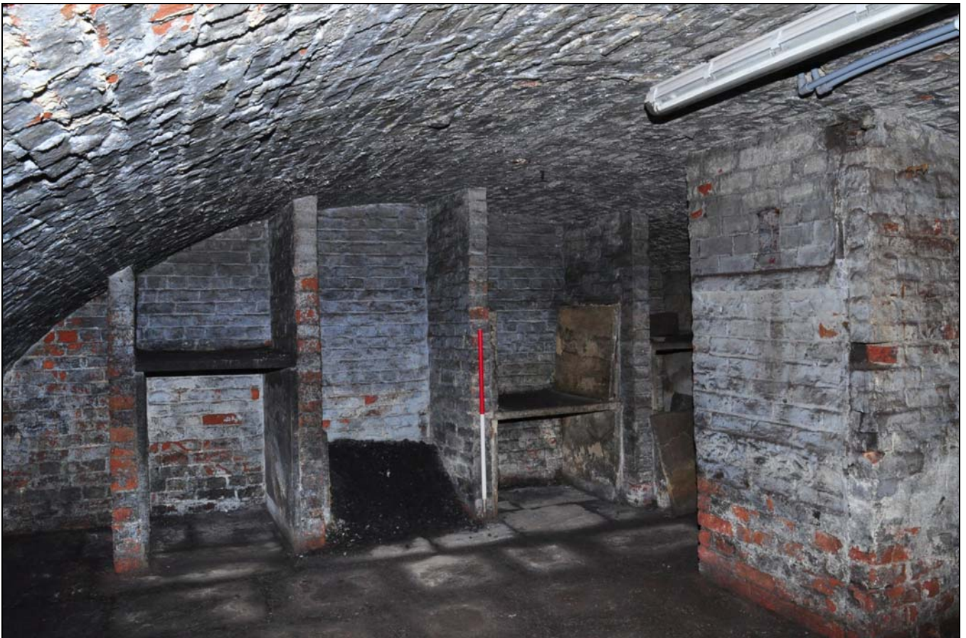
Photo 72: Cellar: R19 (east barrel vault), looking south
