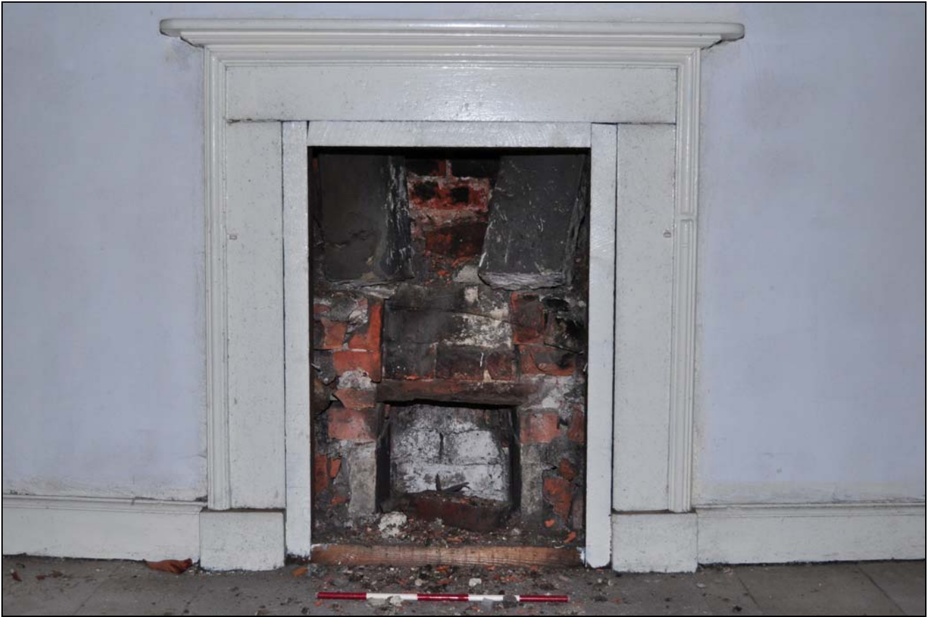
Photo 117: Second floor: R41, detail of fireplace
