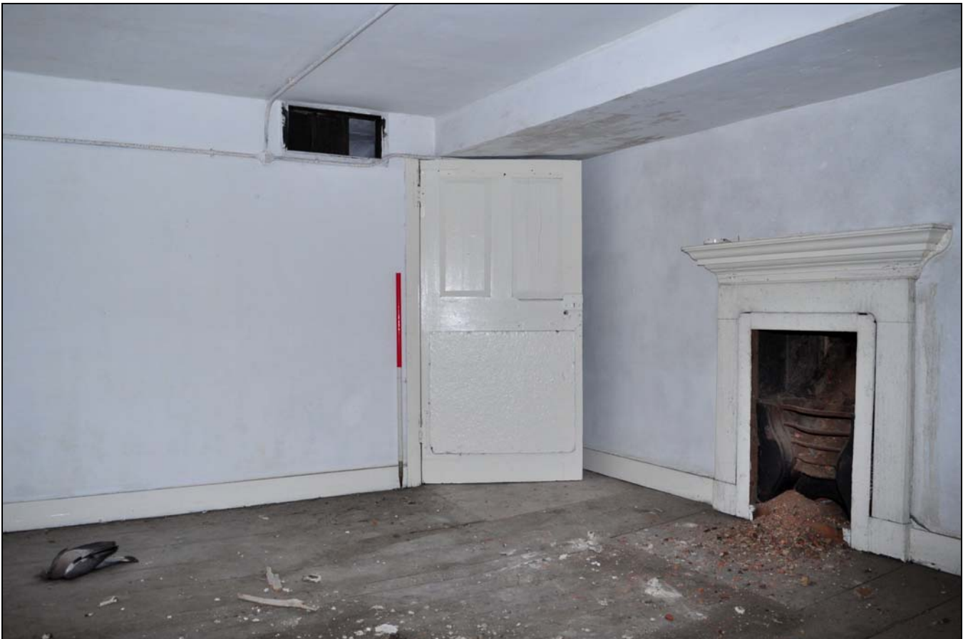
Photo 124: Second floor: R44, looking north-west
