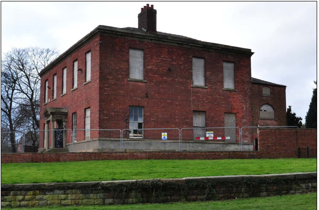
Photo 10: The east elevation of the front range
