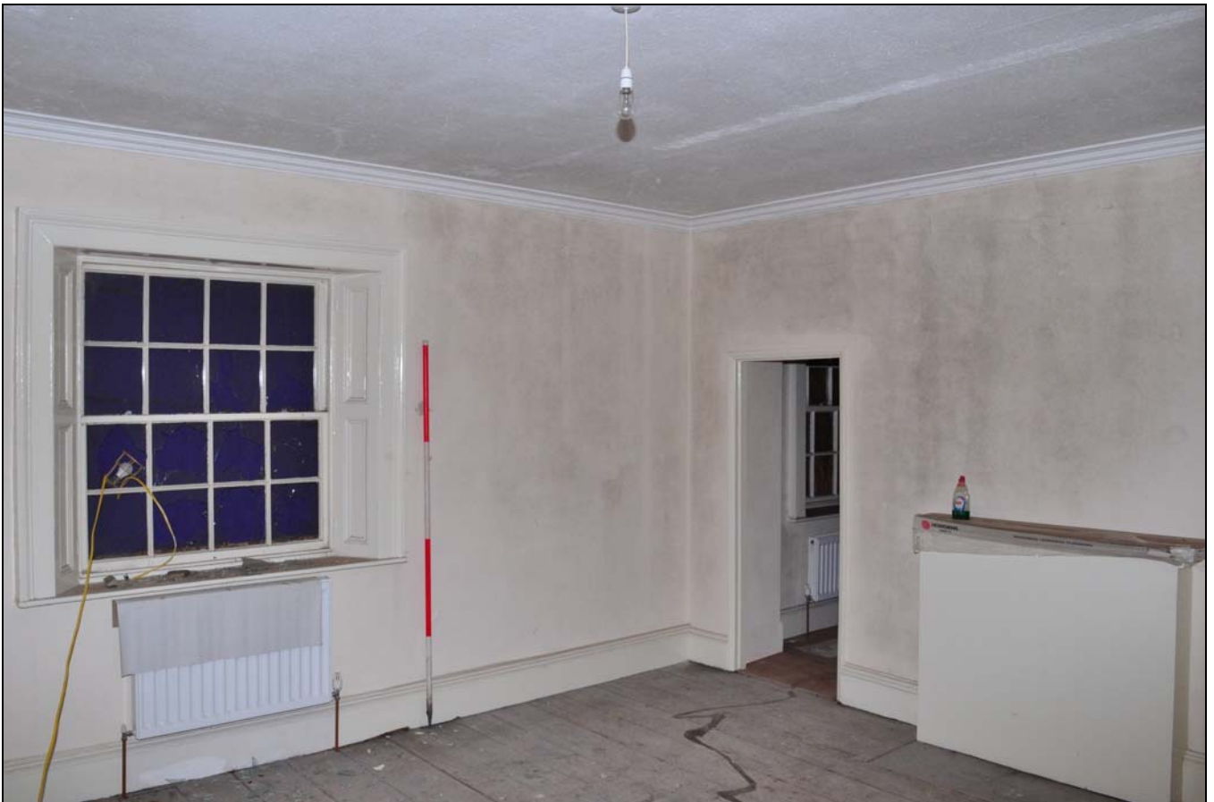
Photo 100: First floor: R33, looking north-west
