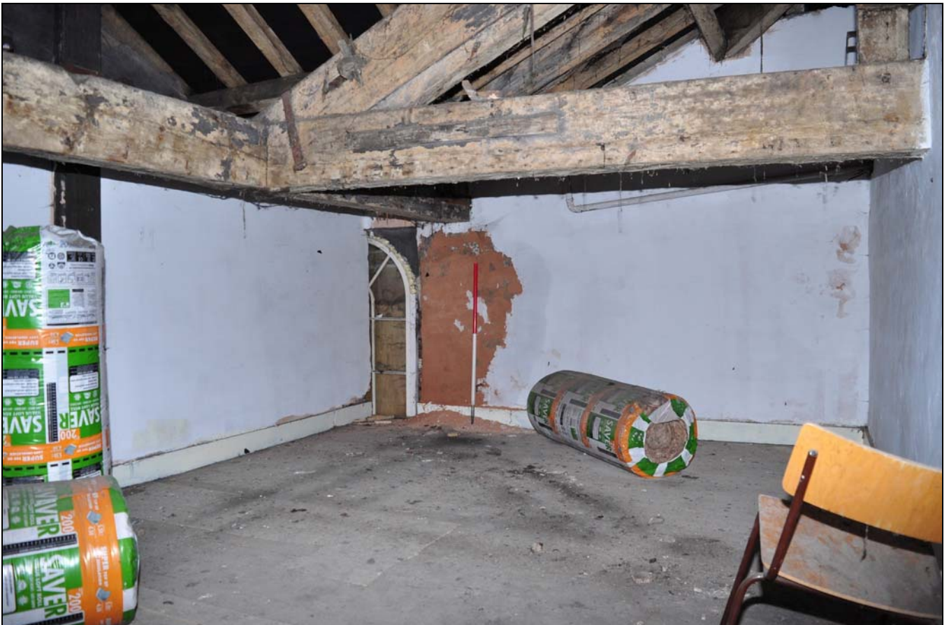
Photo 130: Second floor: R46, looking north-east
