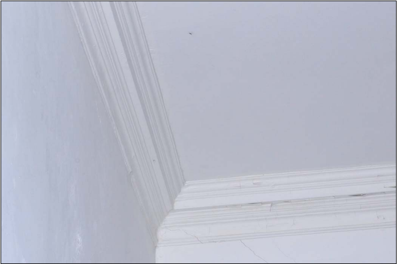
Photo 37: Ground floor: ceiling cornice in R2, looking north-west
