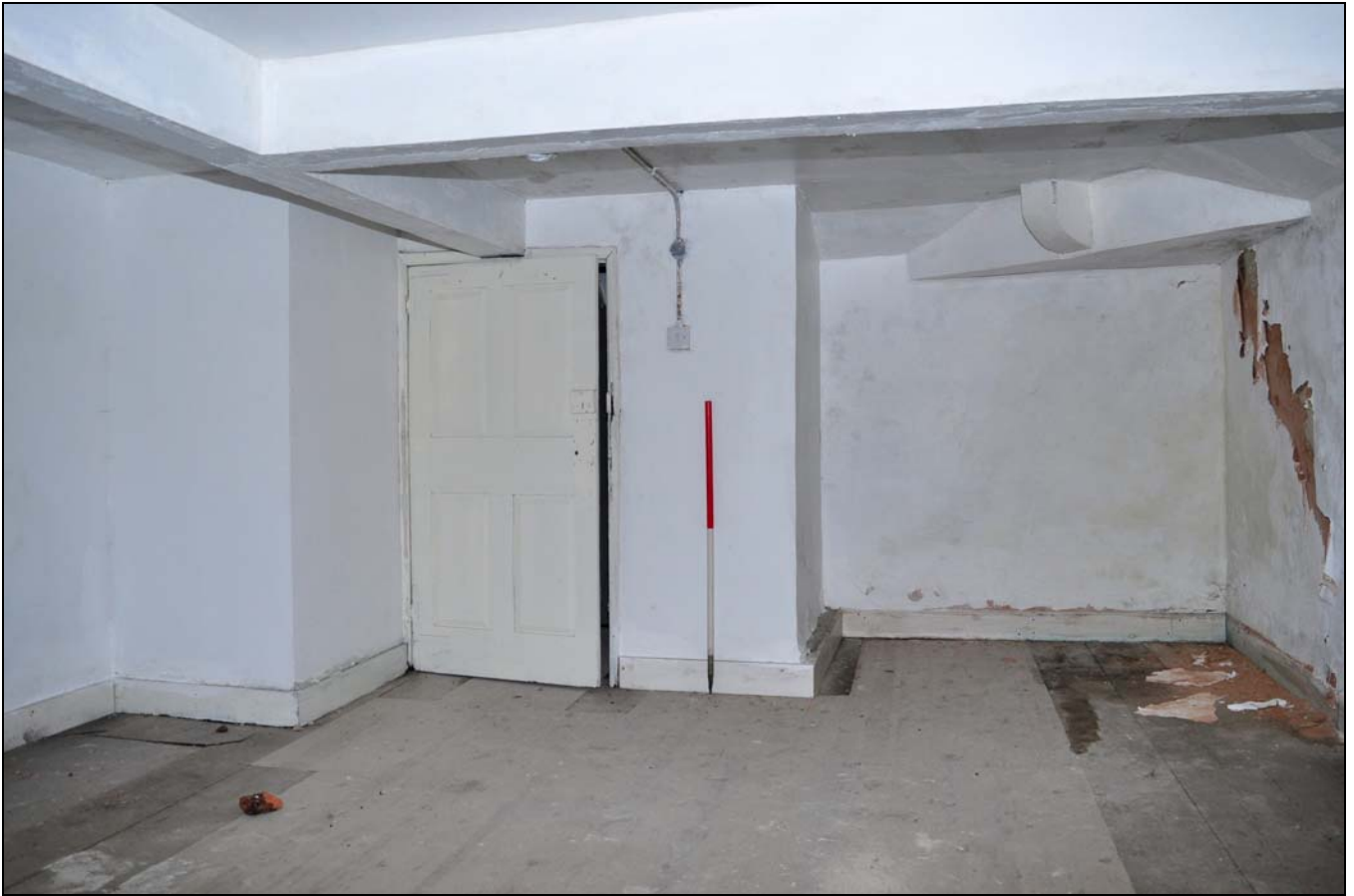
Photo 129: Second floor: R45, looking west
