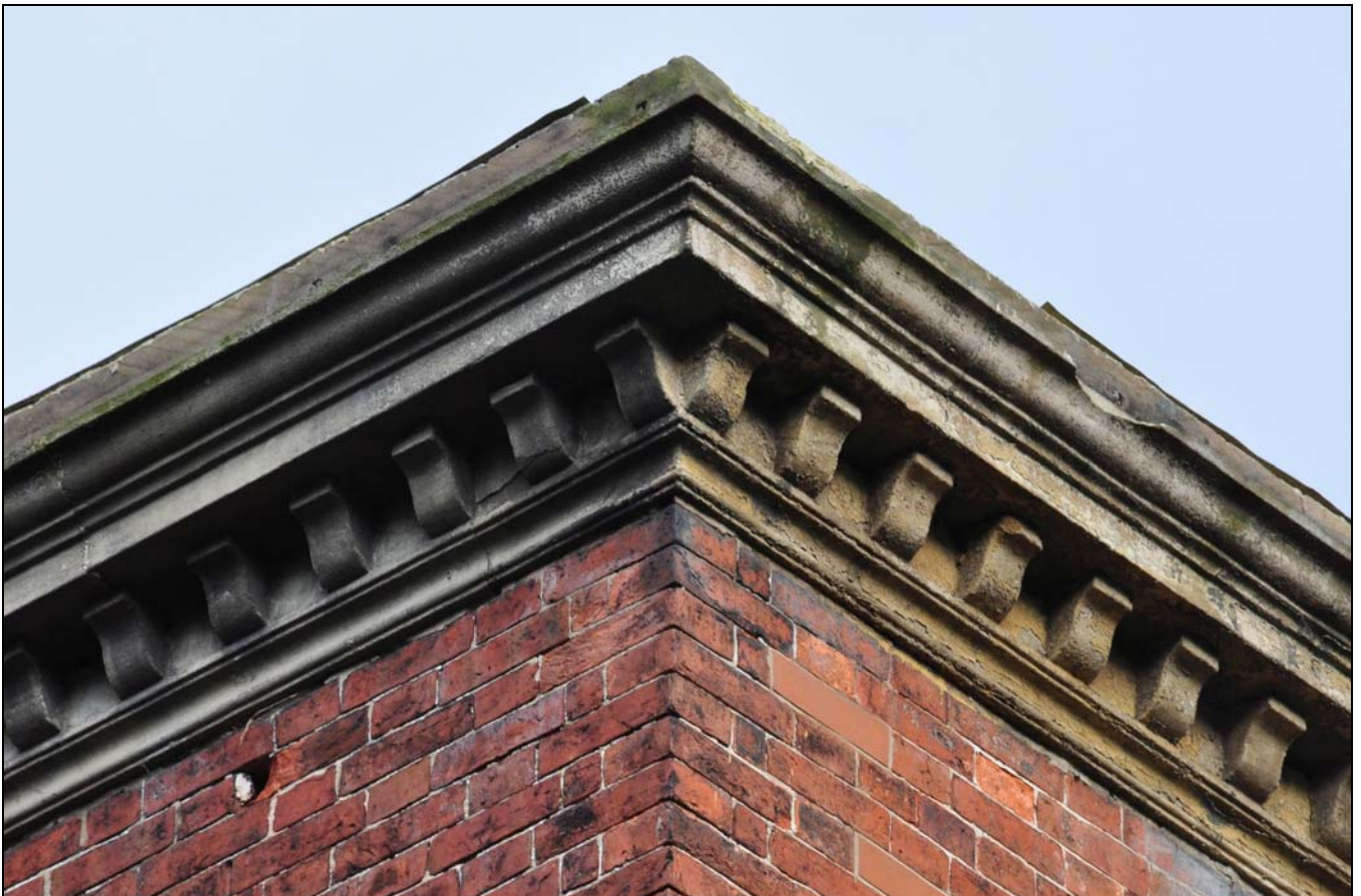
Photo 4: Detail of eaves cornice at south-west corner, front range
