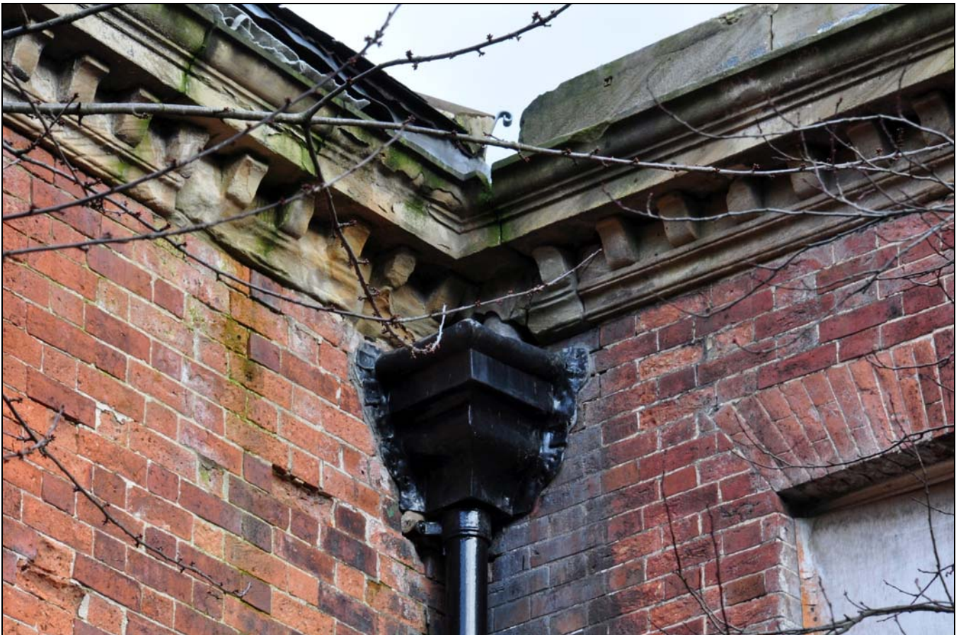
Photo 24: Detail of rainwater hopper, at corner between front and rear ranges, looking north-east
