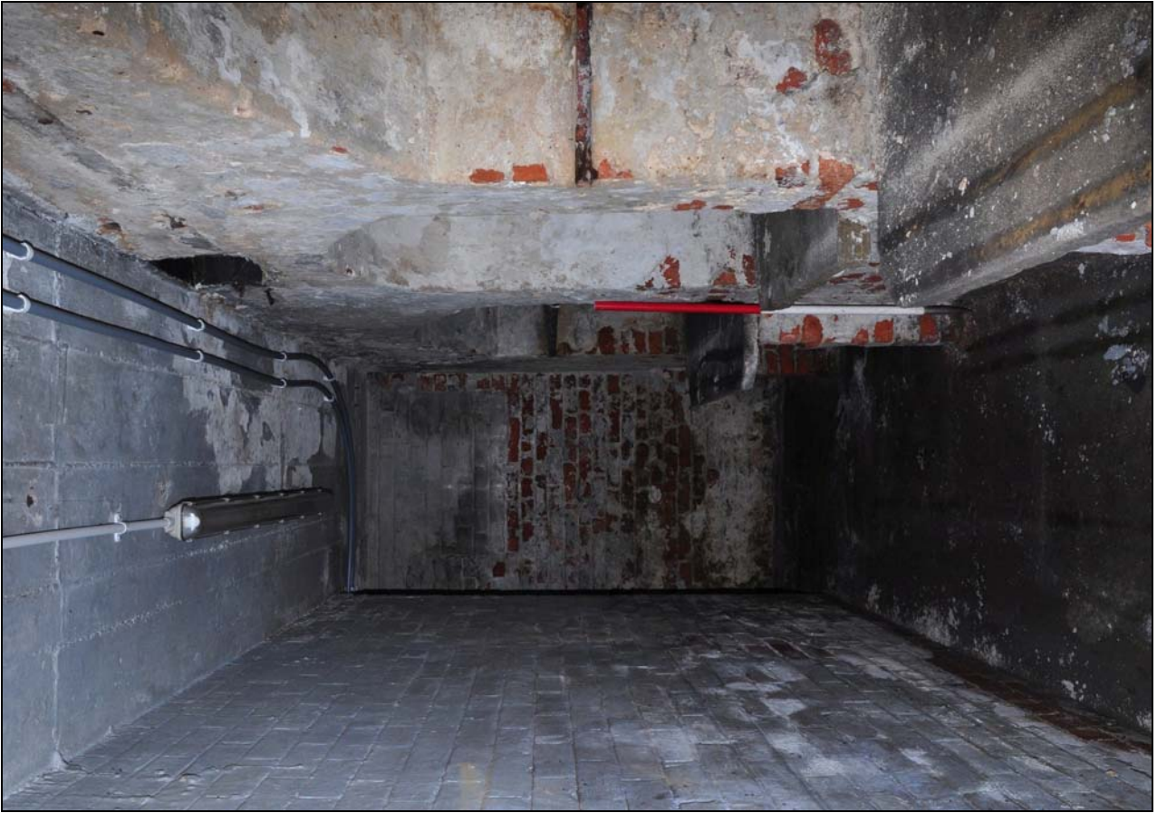
Photo 67: Cellar: blind passage R17, looking west
