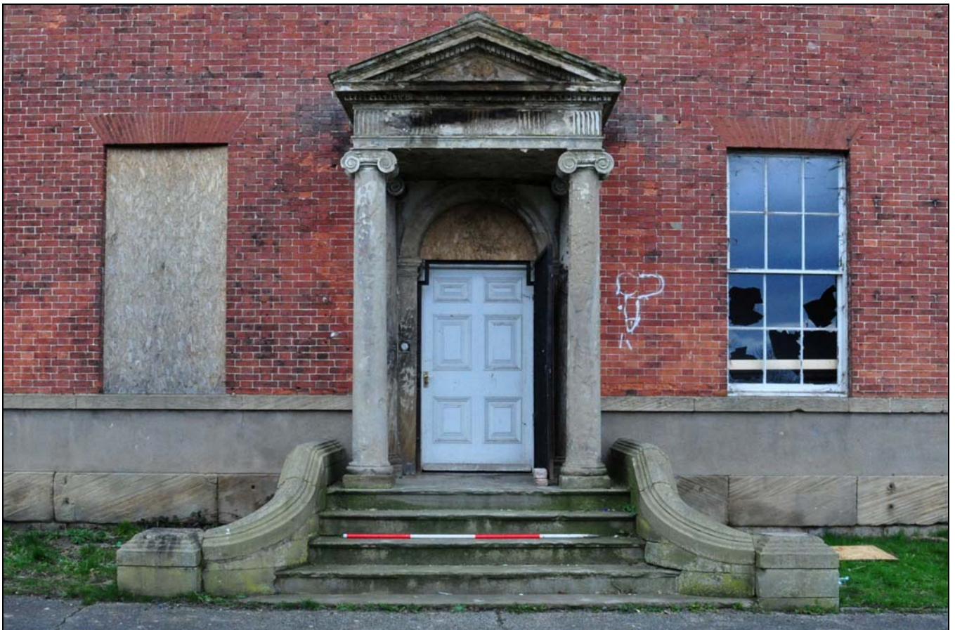
Photo 6: Front entrance, with portico and steps
