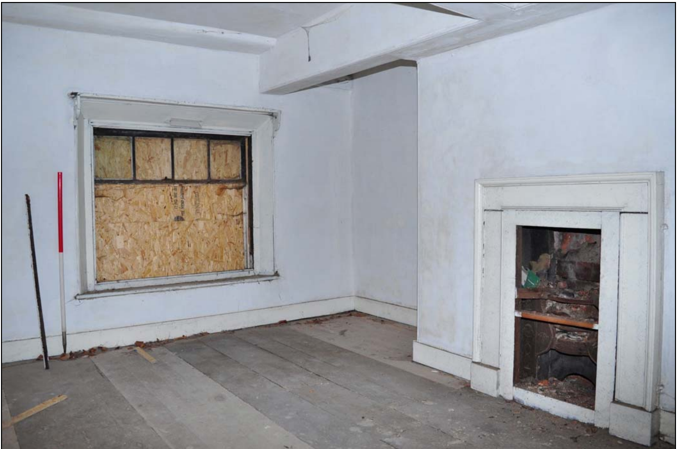
Photo 118: Second floor: R38 (C19 addition), looking north-west
