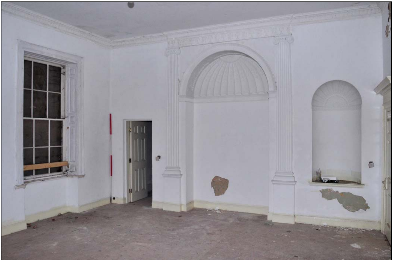
Photo 44: Ground floor: R4 (dining room), looking south-east
