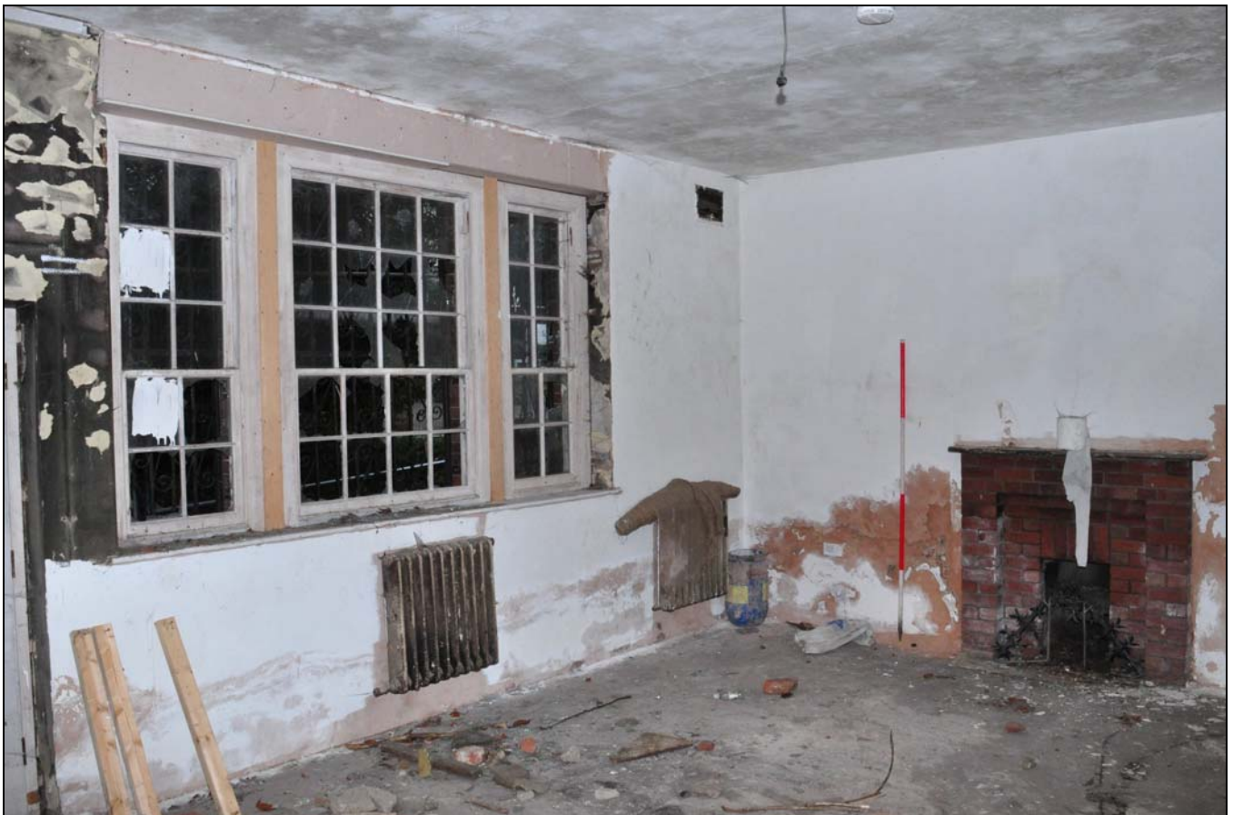
Photo 64: Ground floor: R14, looking north-west
