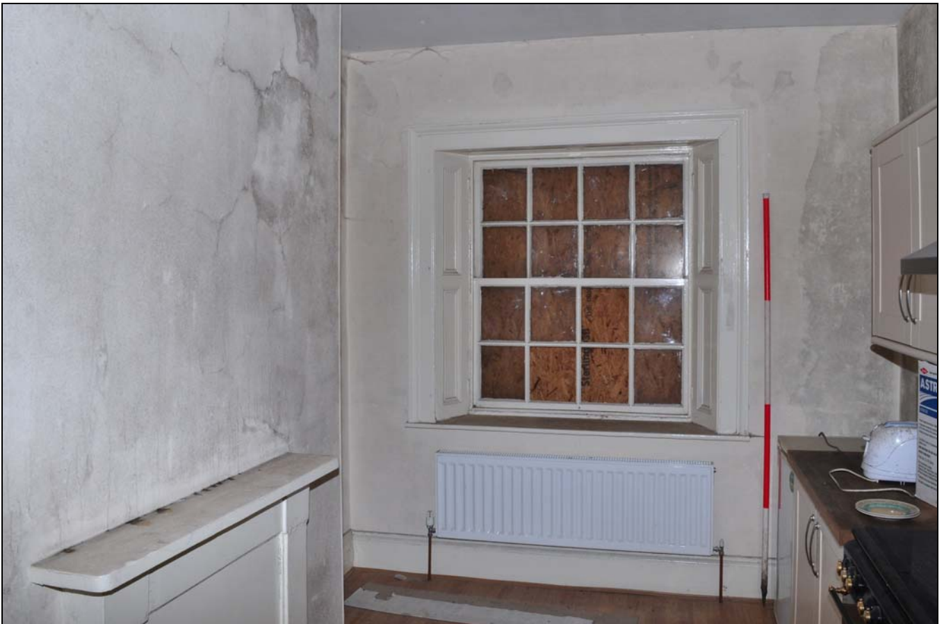
Photo 102: First floor: R34 (C19 addition), looking south-west
