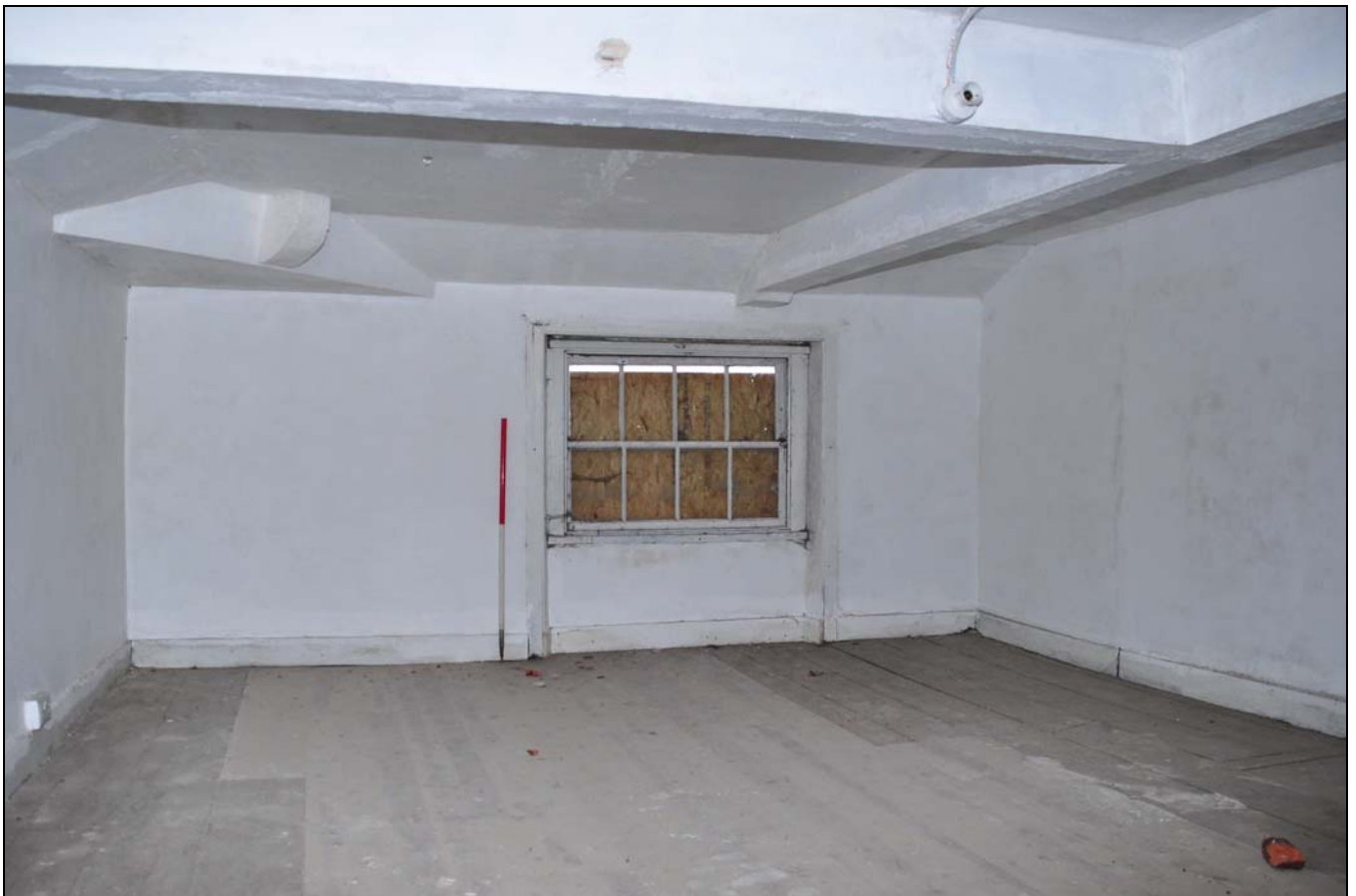
Photo 128: Second floor: R45, looking south-east
