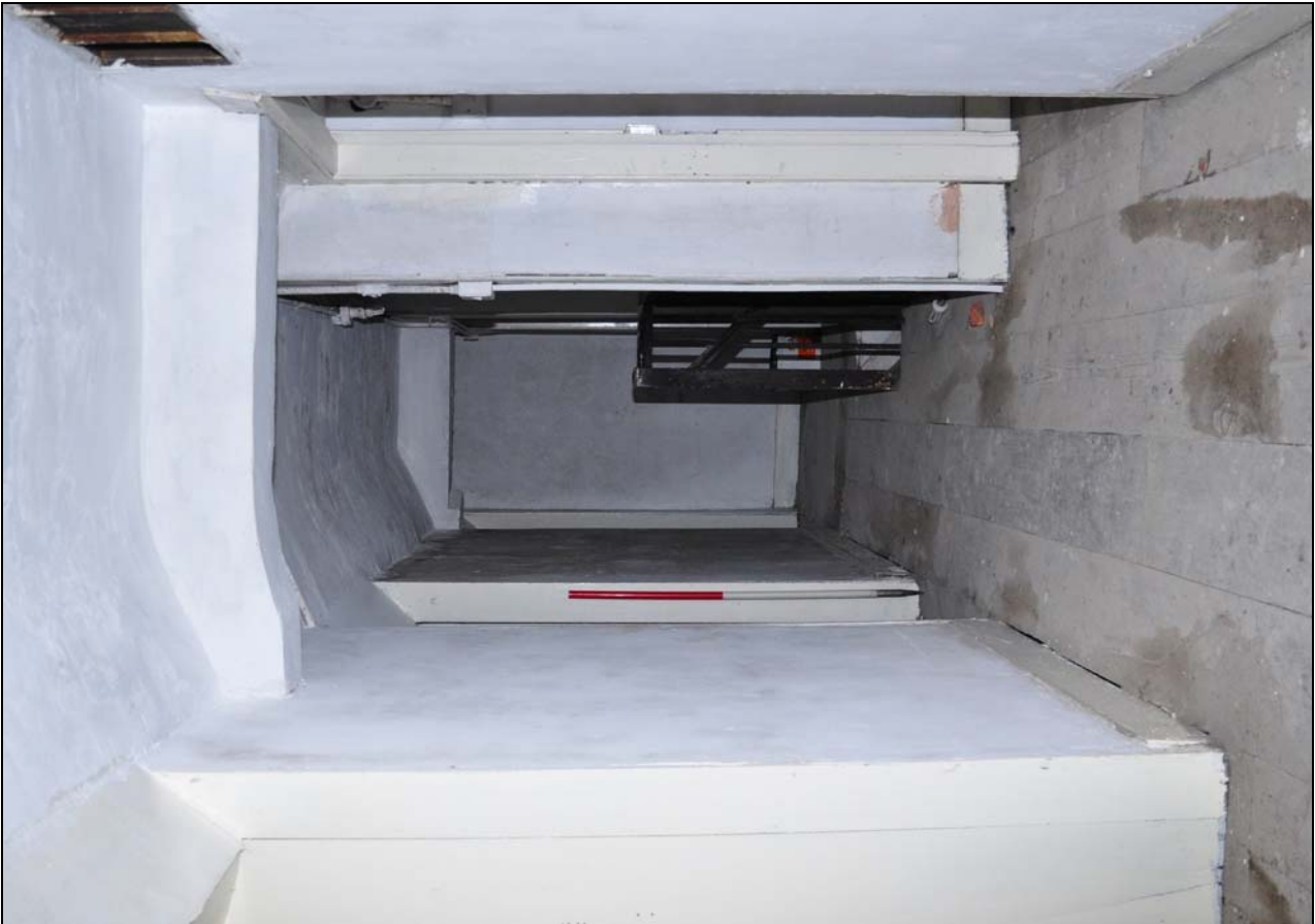
Photo 112: Second floor: R37 (corridor), looking north
