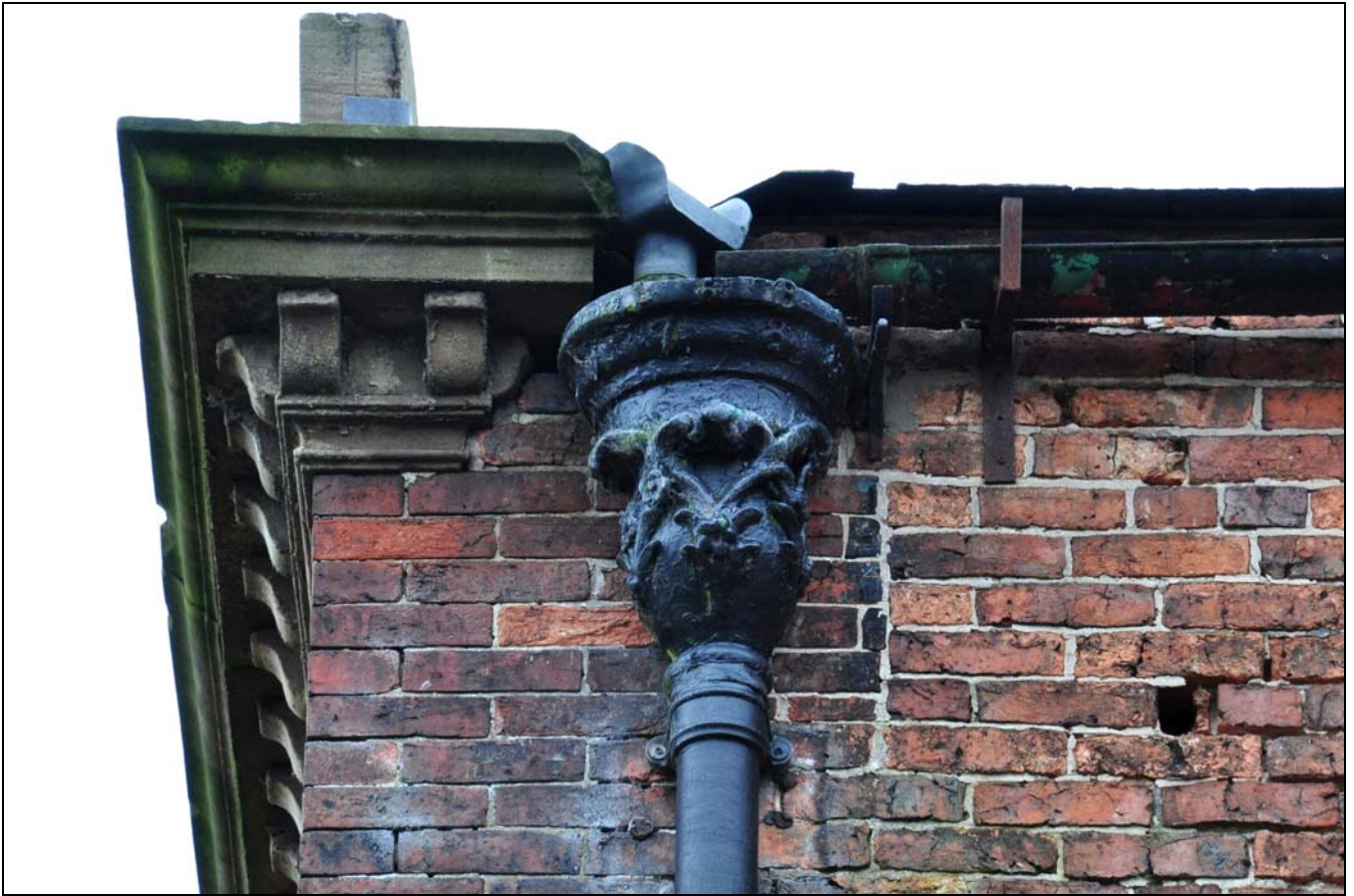
Photo 19: Detail of rainwater hopper on rear of front range, embossed "1788"
