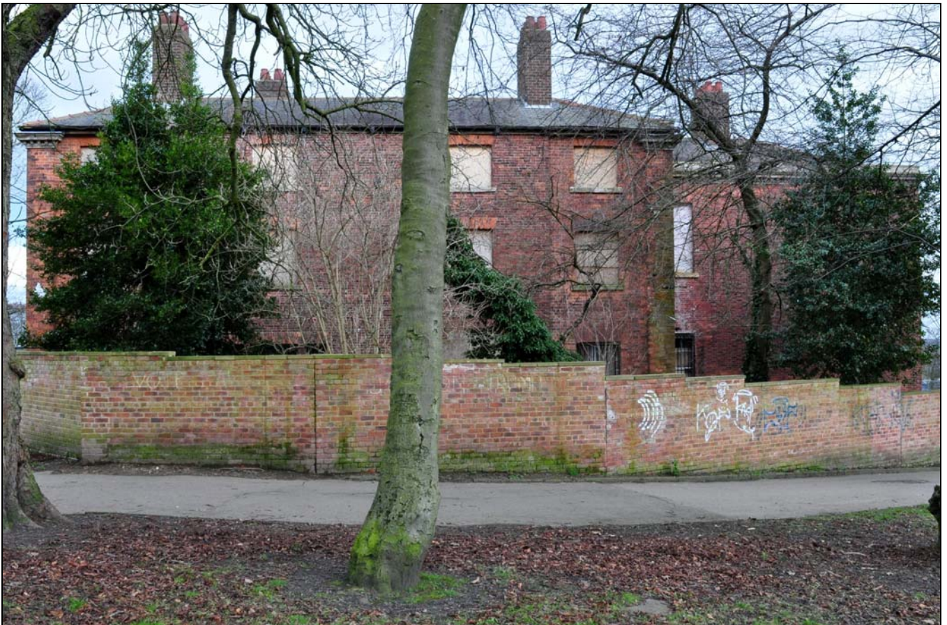
Photo 20: The west elevations of front and rear ranges
