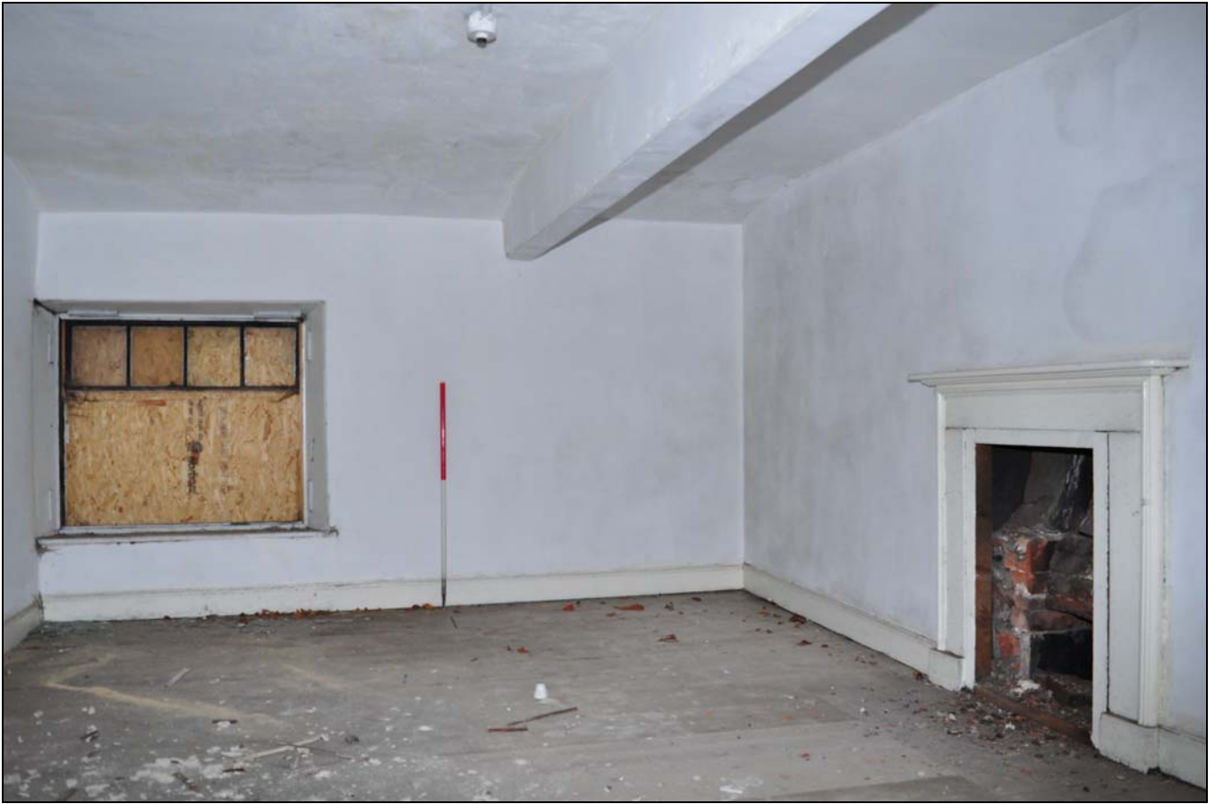
Photo 115: Second floor: R41, looking north-west
