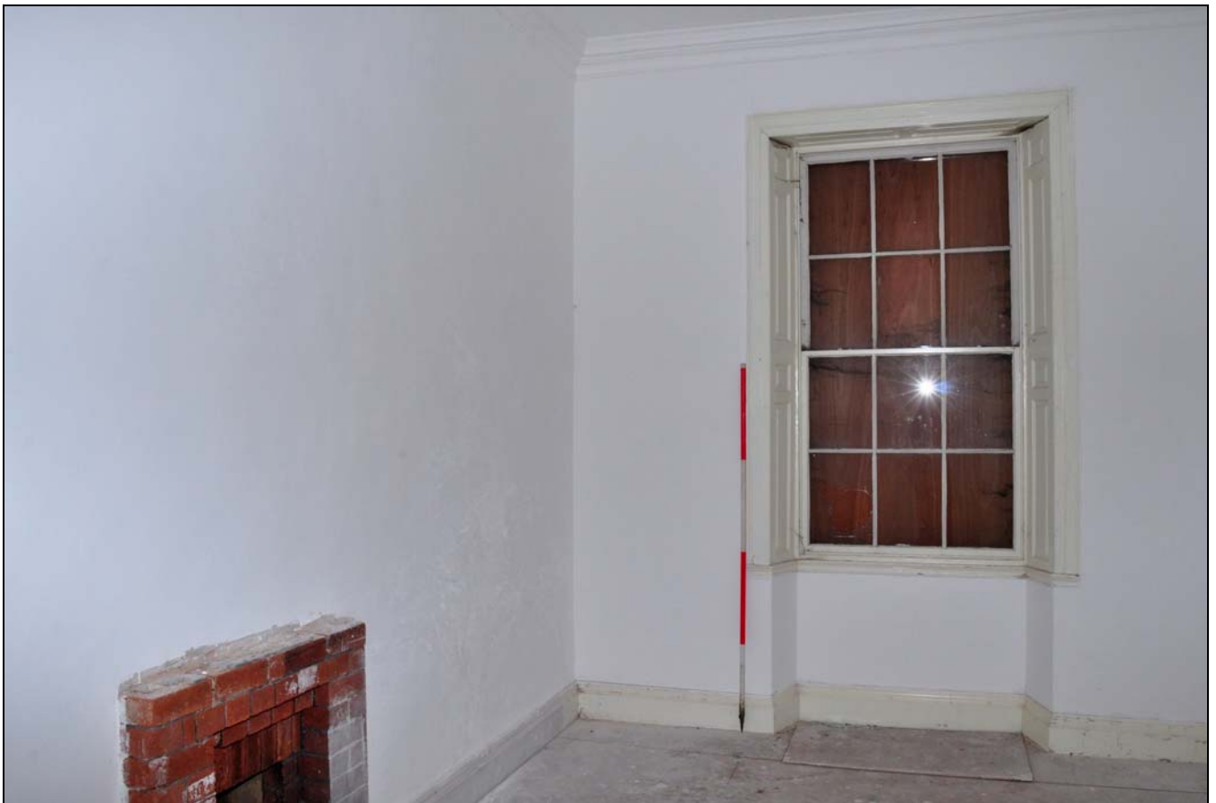
Photo 92: First floor: R27, looking north-east
