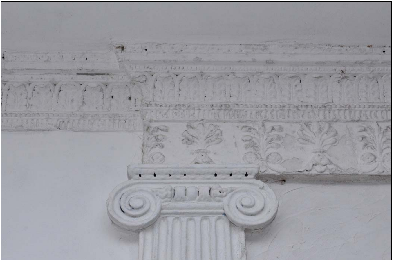
Photo 48: Ground floor: R4 (dining room), detail of cornice and pilaster capitals to sideboard recess
