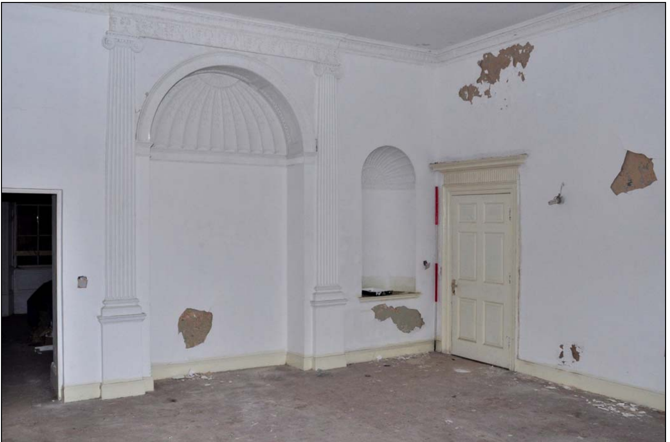
Photo 42: Ground floor: R4 (dining room), looking south-west
