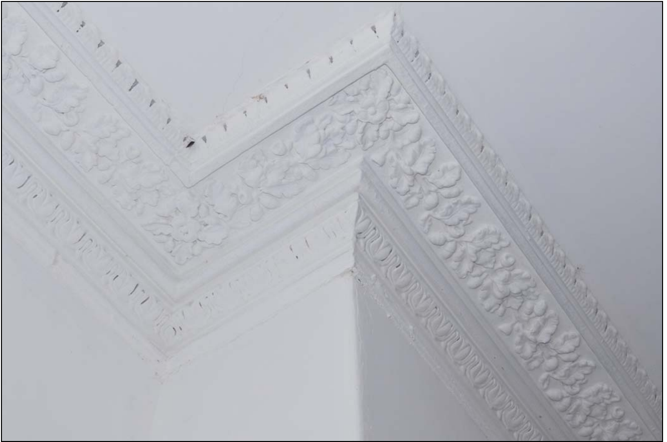
Photo 41: Ground floor: R3, detail of ceiling cornice
