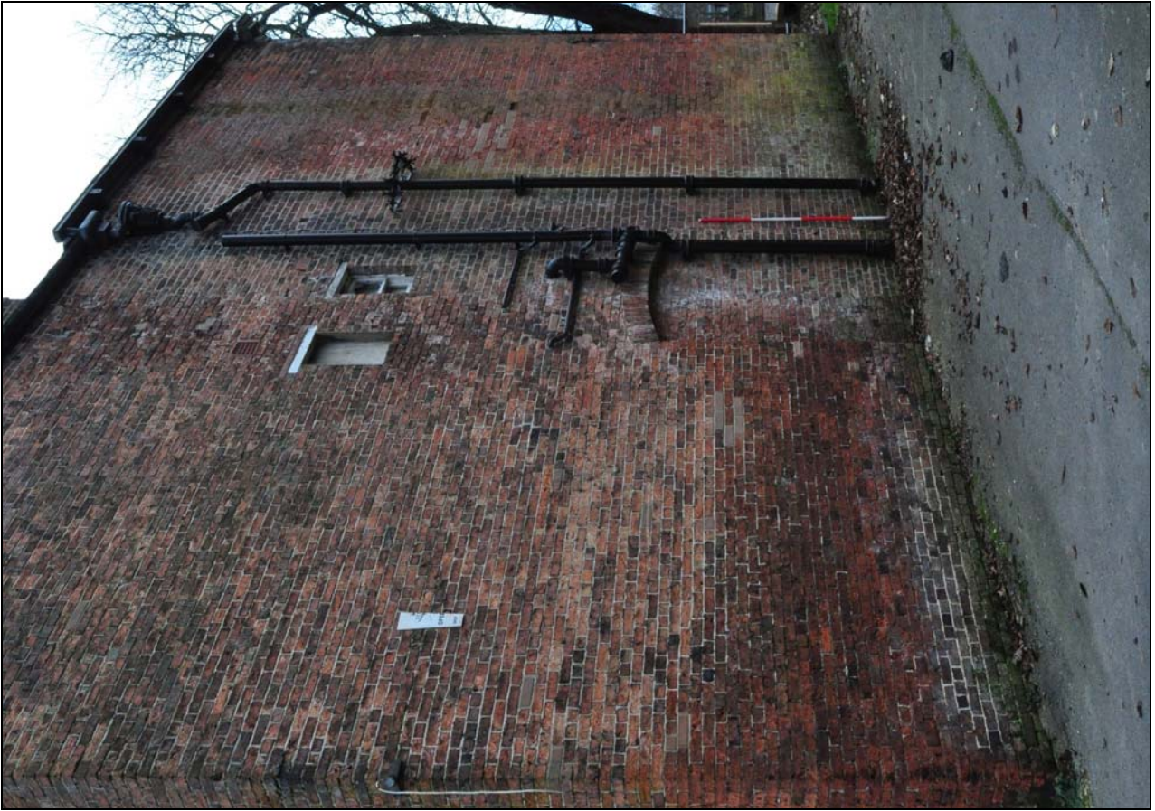
Photo 29: North end of rear range, looking south-west
