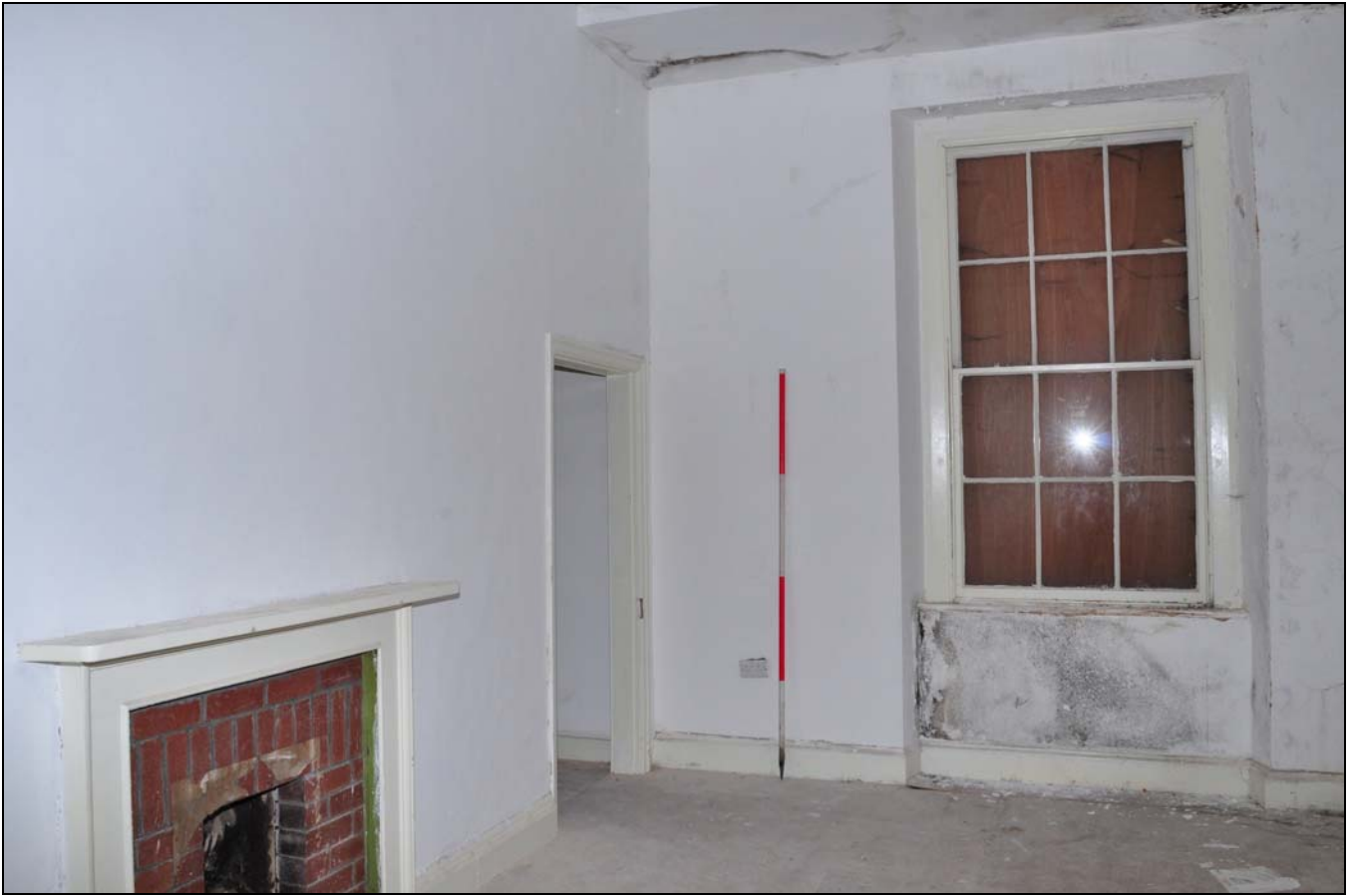
Photo 85: First floor: R25, looking south-west
