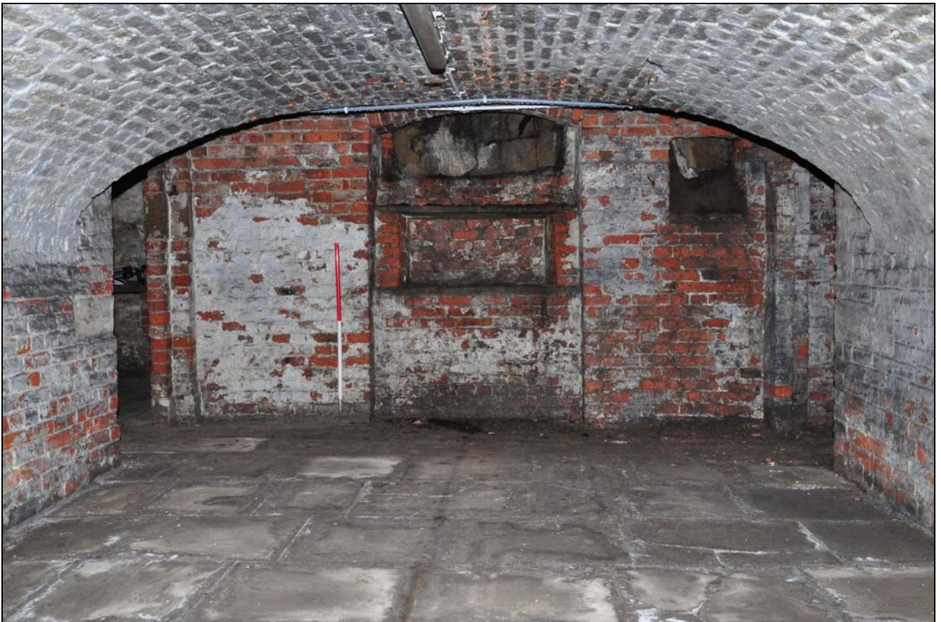
Photo 70: Cellar: R18 (west barrel vault), looking north
