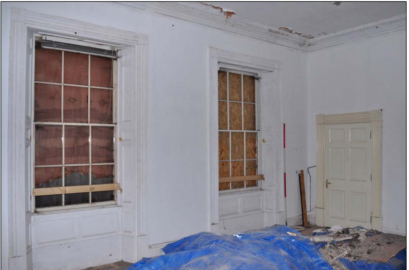
Photo 38: Ground floor: R3, looking south-west
