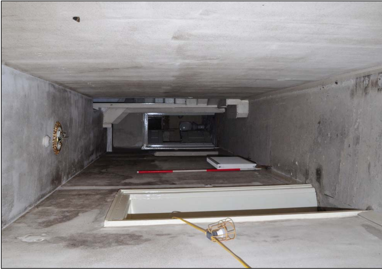
Photo 97: First floor: R30 (corridor), looking north
