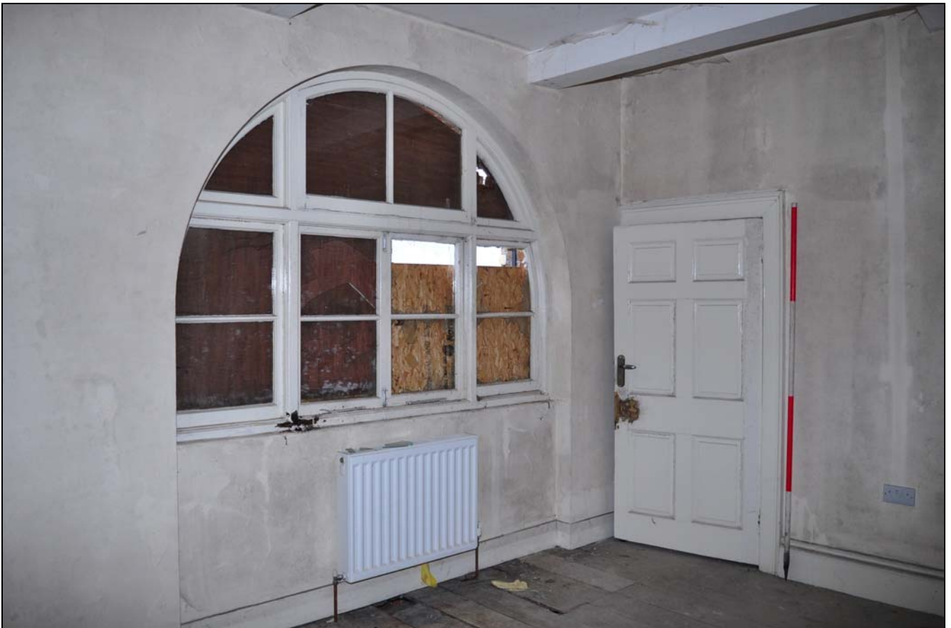
Photo 106: First floor: R36, looking south-east
