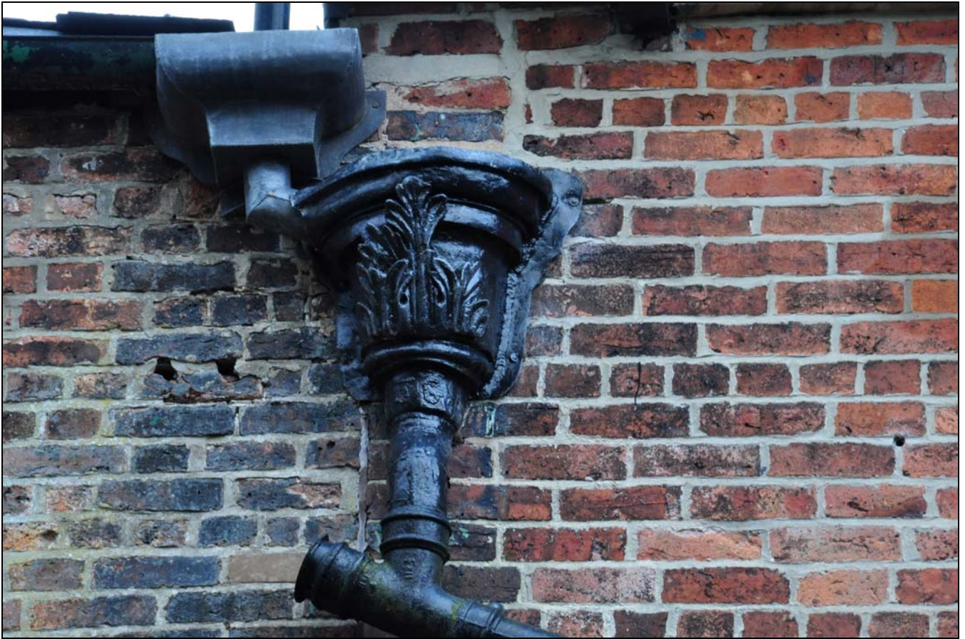
Photo 31: Rainwater hopper on north end of rear range, embossed "JG" below decoration
