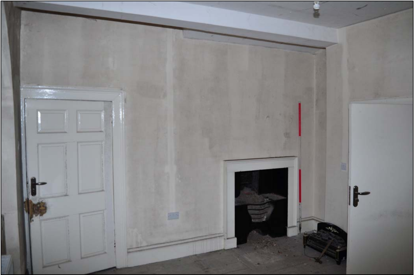
Photo 107: First floor: R36, looking south-west
