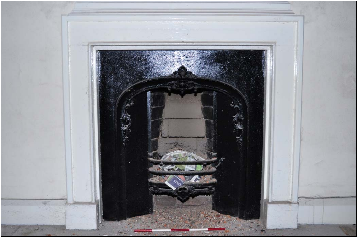
Photo 105: First floor: R35, detail of fireplace
