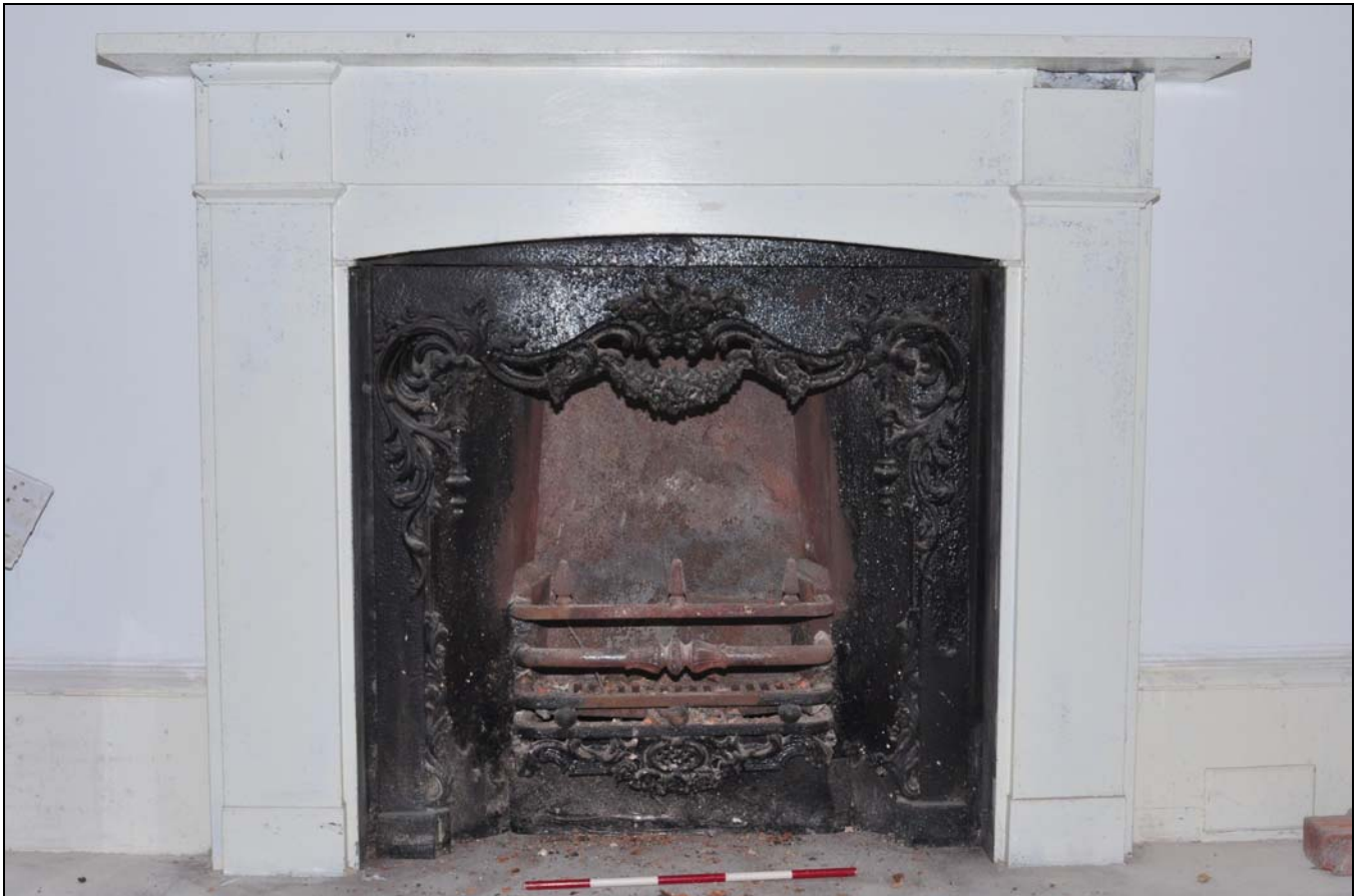
Photo 90: First floor: R26, detail of fireplace
