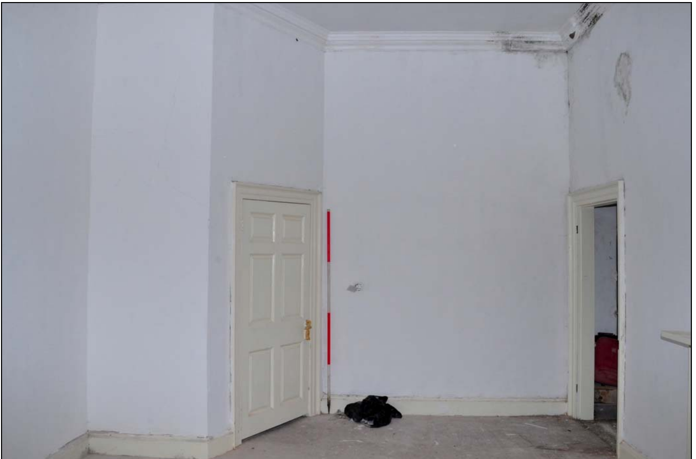
Photo 86: First floor: R25, looking east
