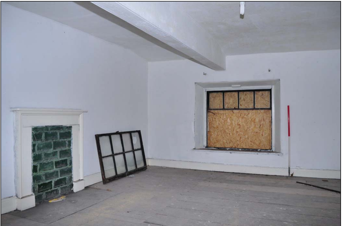
Photo 114: Second floor: R39, looking south-west
