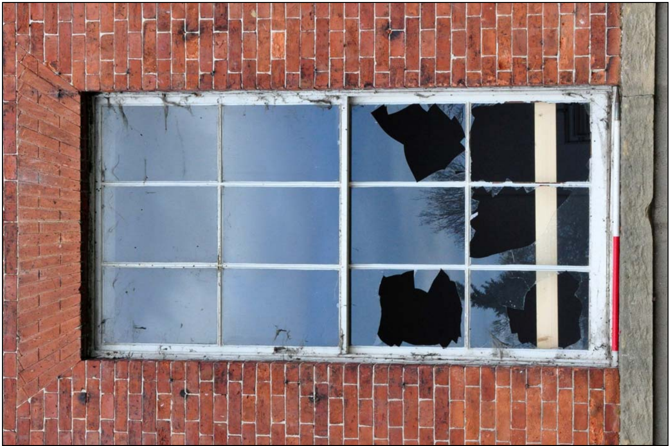
Photo 9: Detail of ground floor window detail, front elevation
