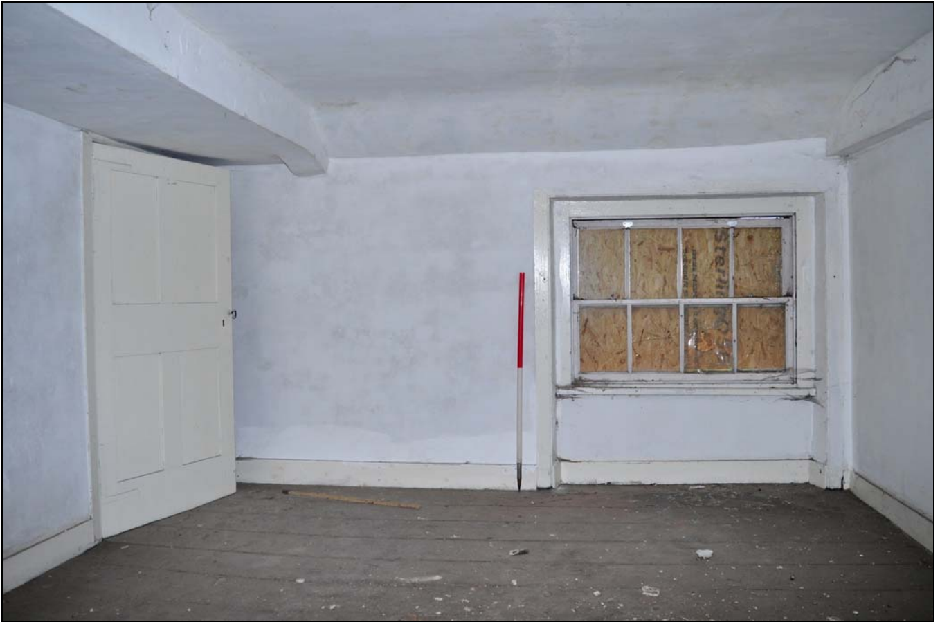
Photo 123: Second floor: R44, looking east
