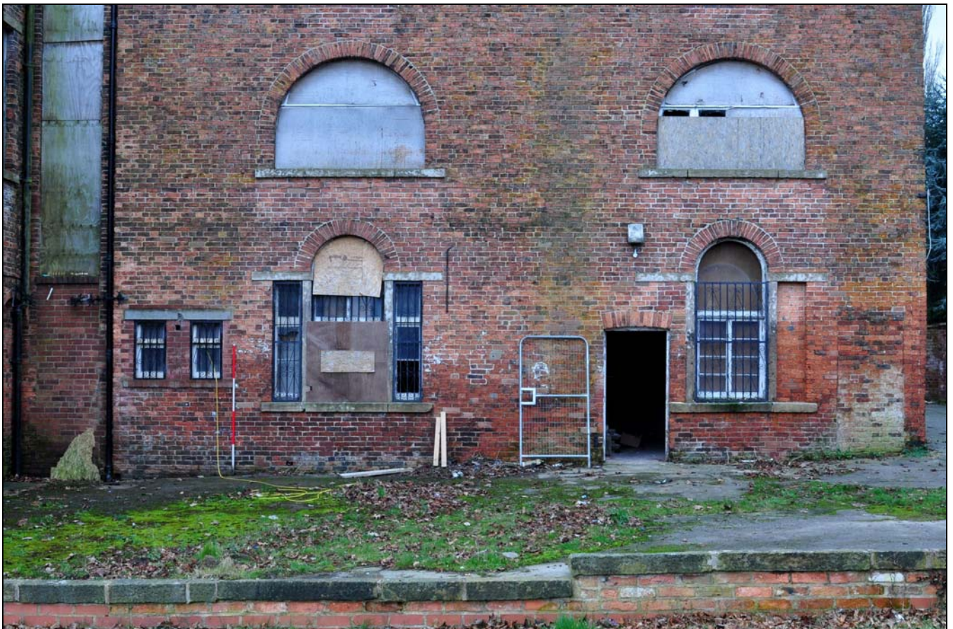
Photo 28: East elevation of rear range (ground and first floors)
