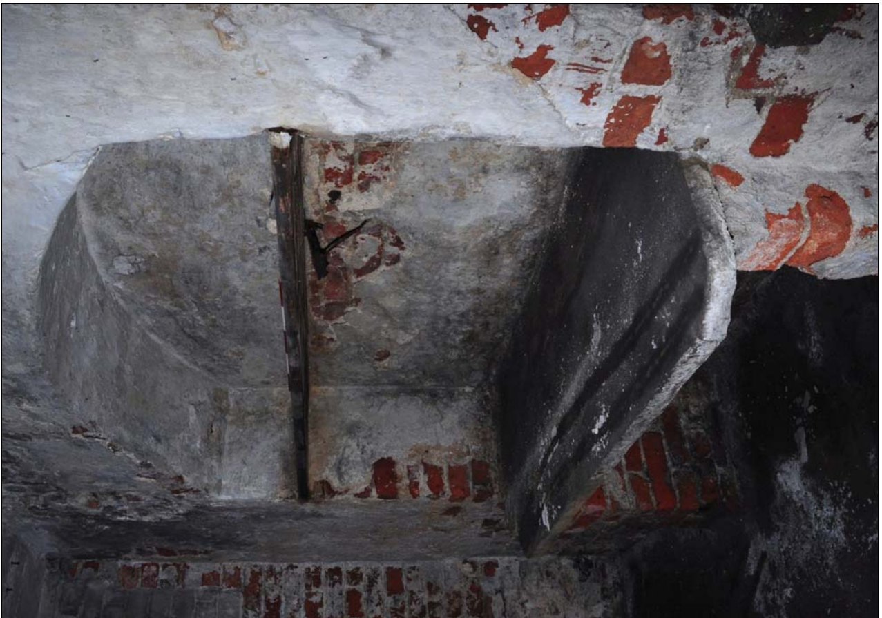
Photo 68: Cellar: storage recess in blind passage R17, looking north-west
