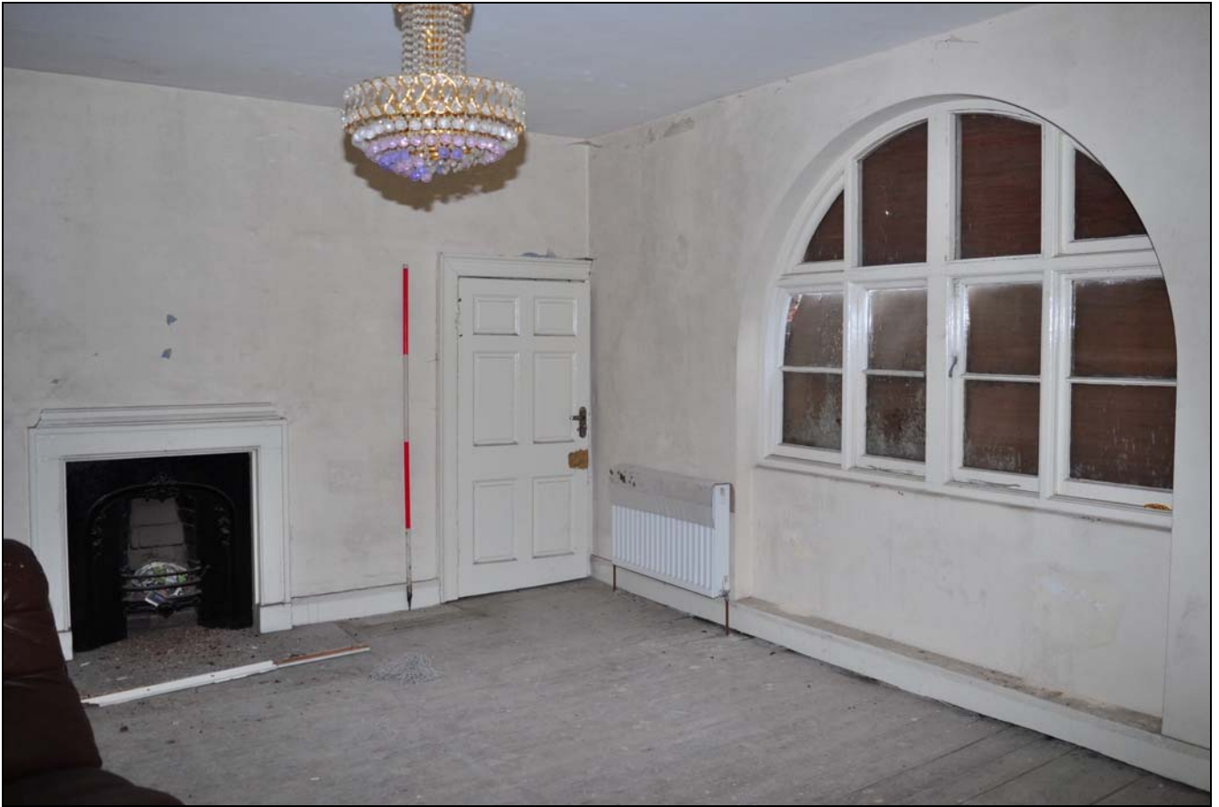
Photo 103: First floor: R35, looking north-east
