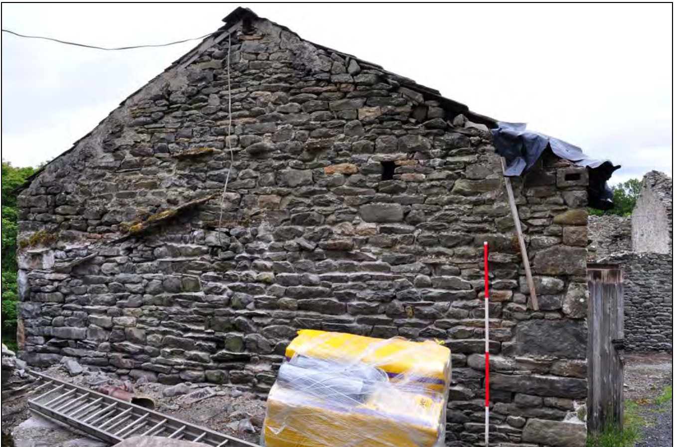
Photo 8: North gable of main range (added bay)
