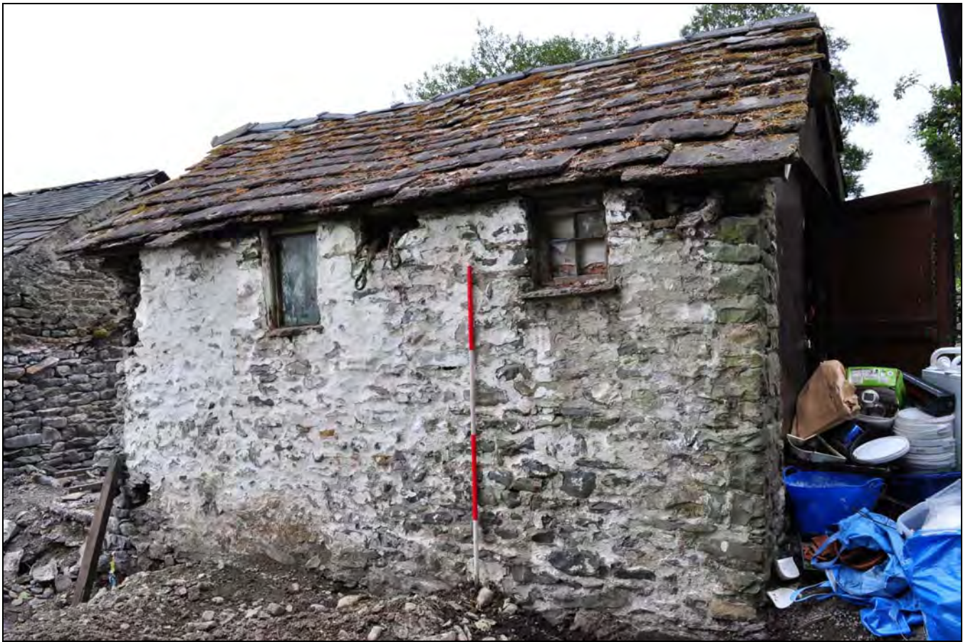
Photo 63: Garage, from the east
