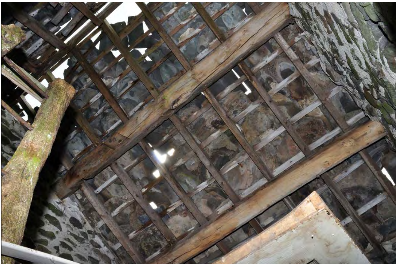
Photo 54: Underside of roof over former stable
