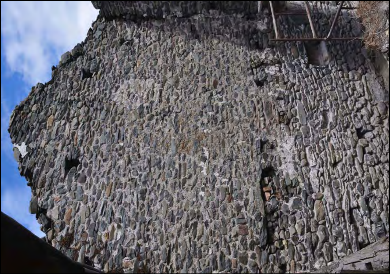
Photo 39: East gable of south wing, from the north-west
