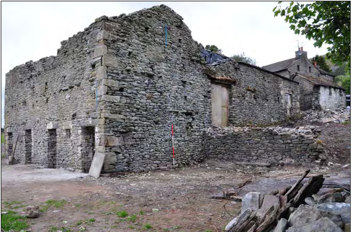
Photo 24: General view of the barn, from the south-east
