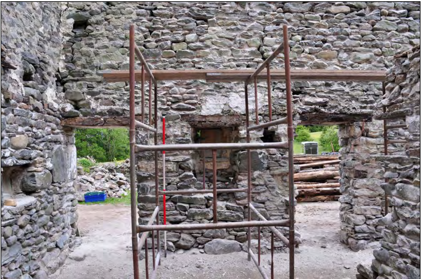
Photo 42: South-east corner of south wing, from the north
