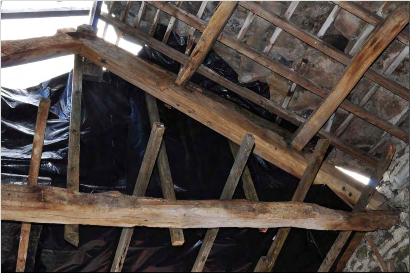
Photo 33: Roof truss over threshing bay, from the north
