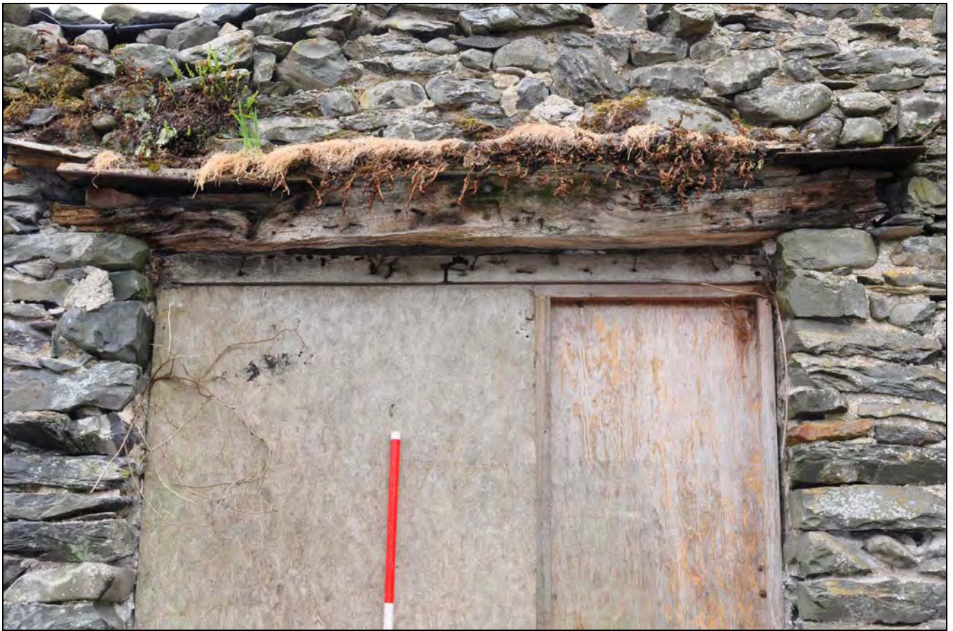
Photo 11: Detail of lintel, east doorway to threshing bay
