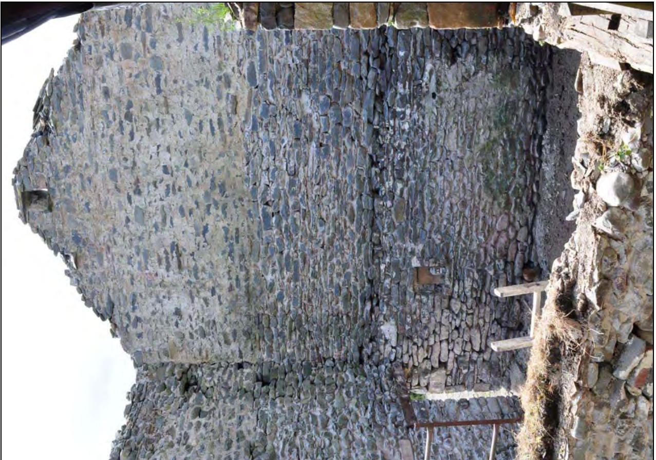
Photo 40: West gable of south wing, from the north-east
