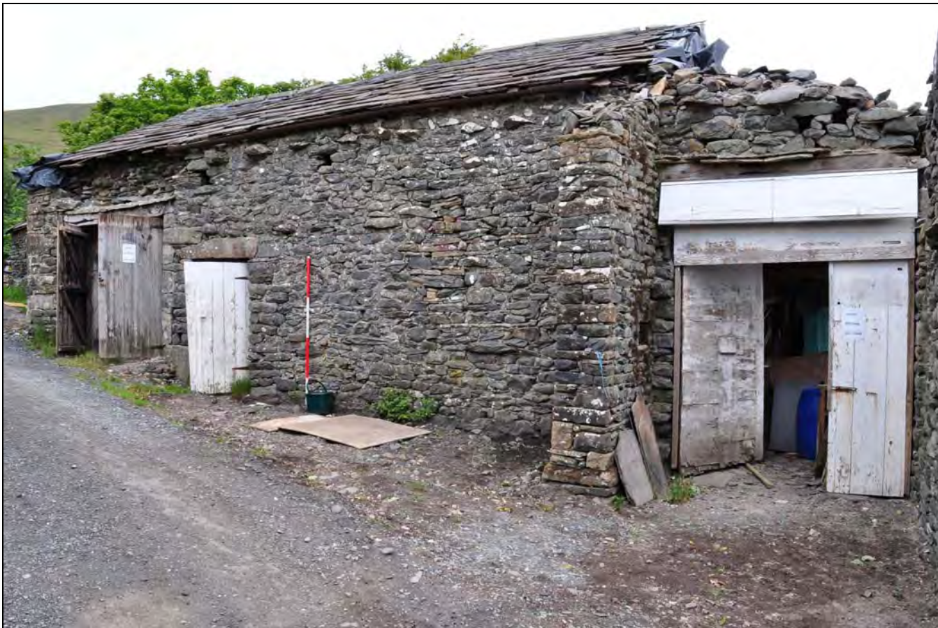
Photo 3: Front of main range, from the south-west
