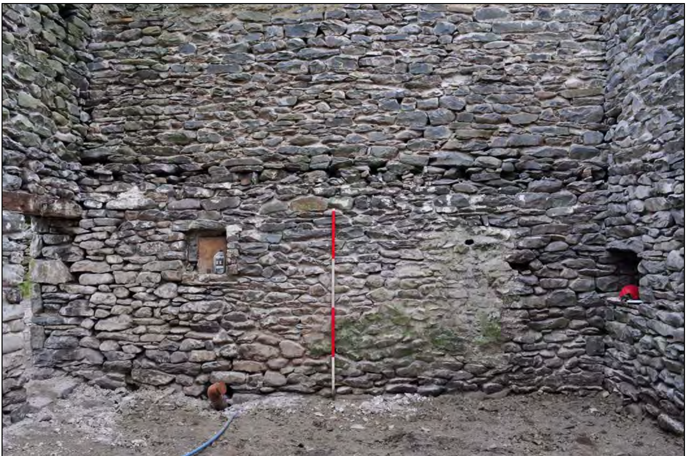
Photo 44: West gable of south wing, from the north-east
