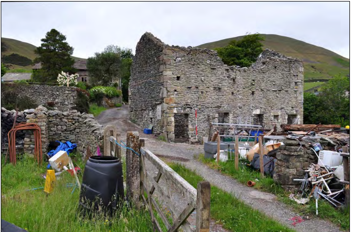
Photo 2: The south wing and forecourt, from the south-west
