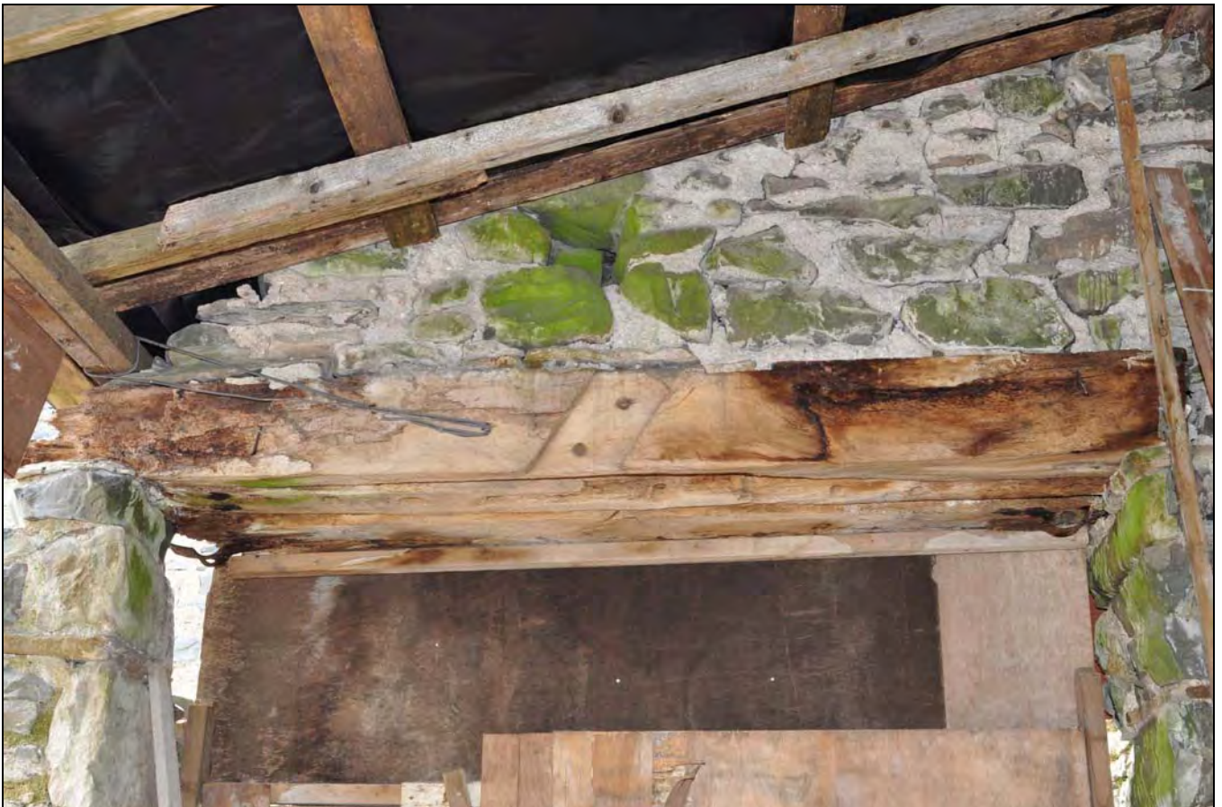
Photo 30: Detail of lintel, west doorway to threshing bay
