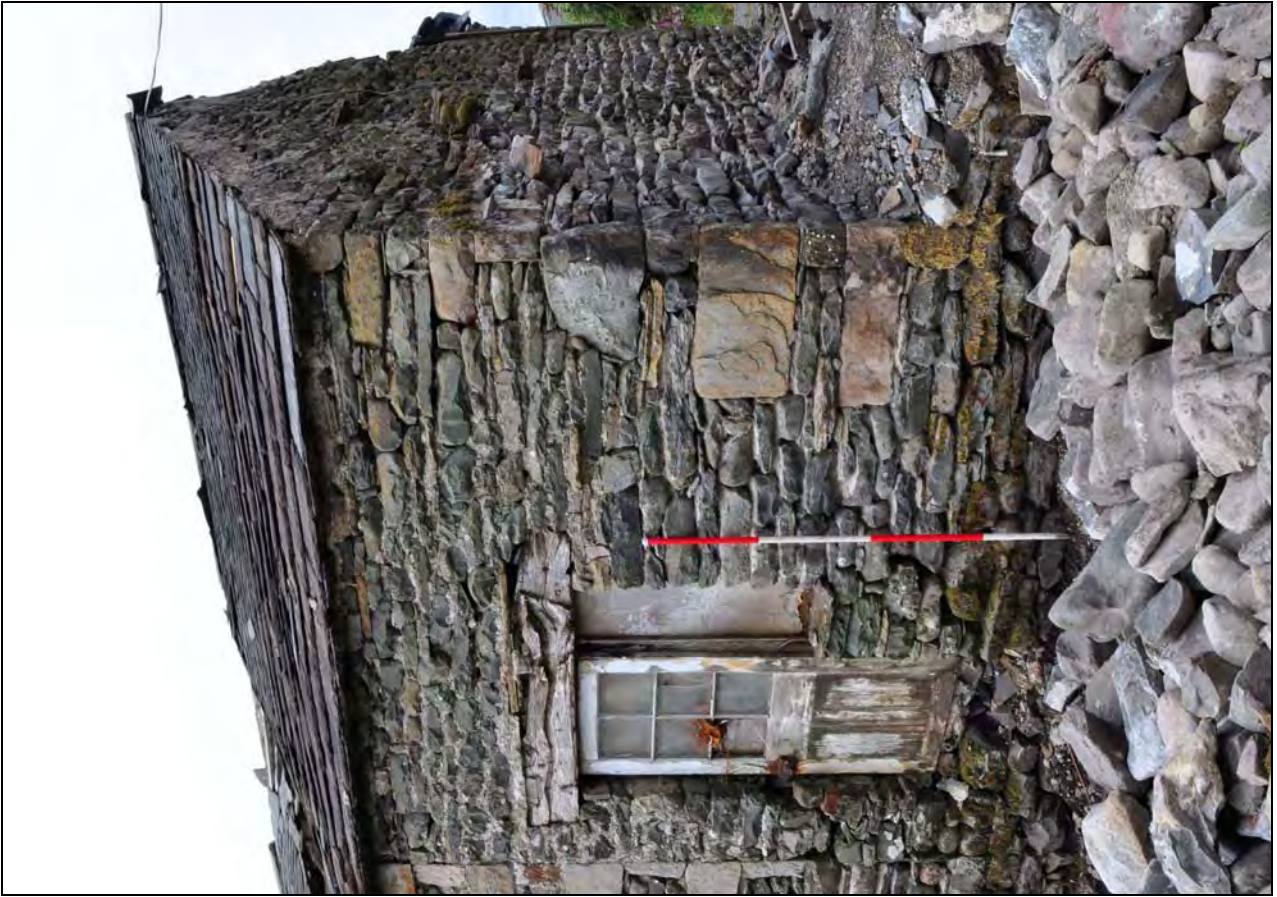
Photo 17: East side of added bay at north end of main range
