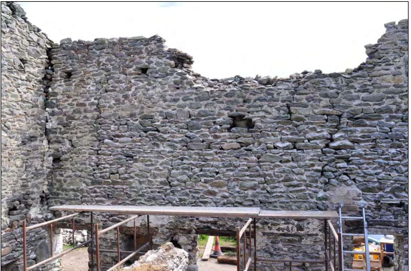
Photo 38: South-east corner of south wing, from the north-west
