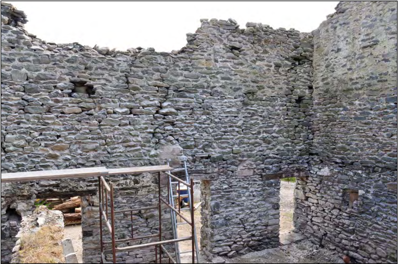
Photo 37: South-west corner of south wing, from the north-east
