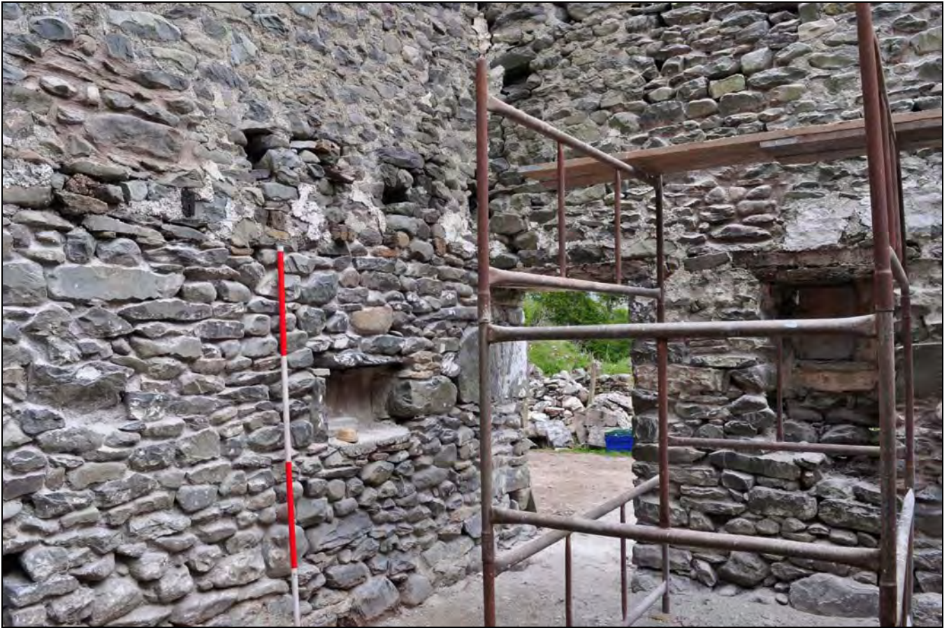
Photo 41: South-east corner of south wing, from the north-west
