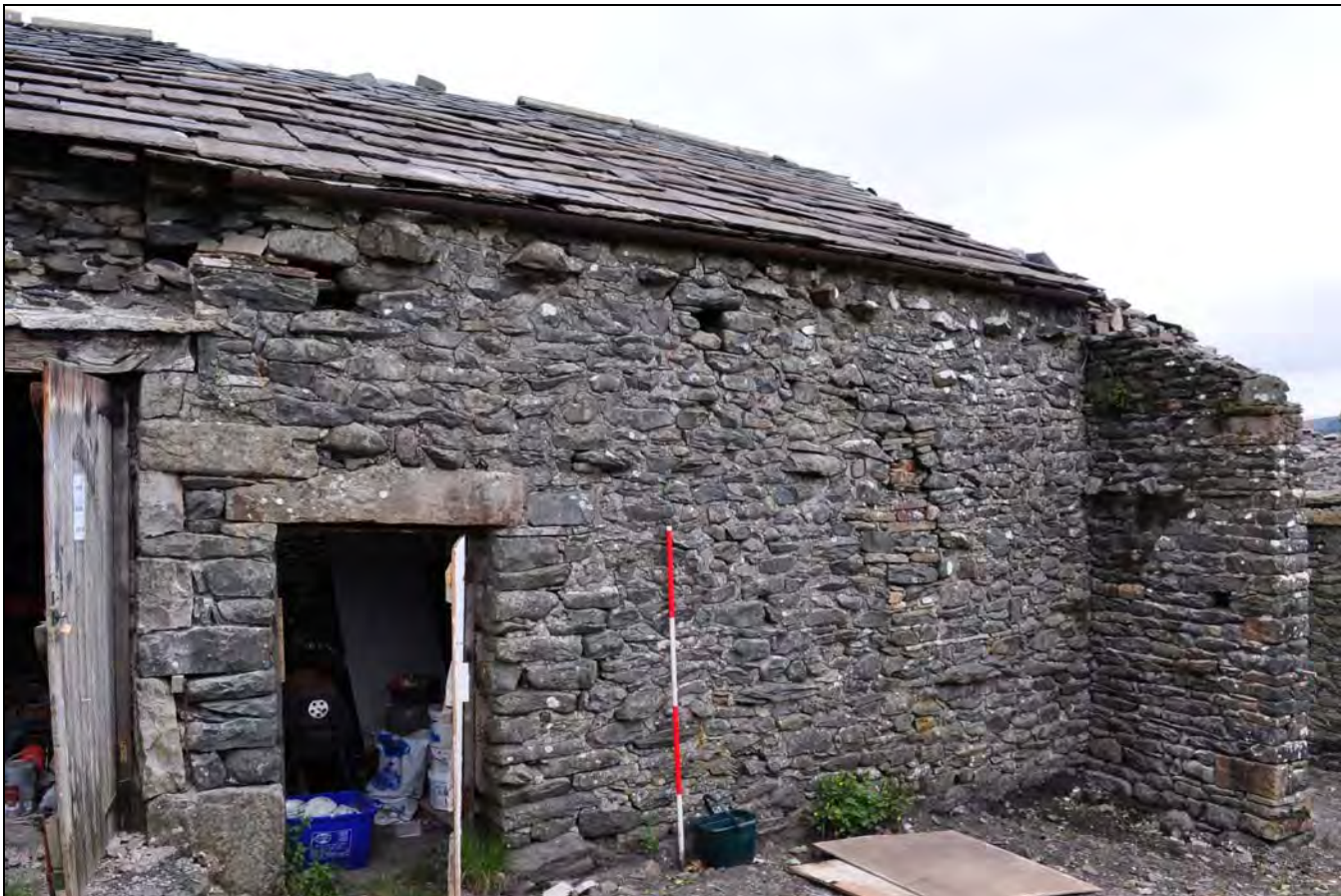
Photo 4: Front of main range, from the north-west
