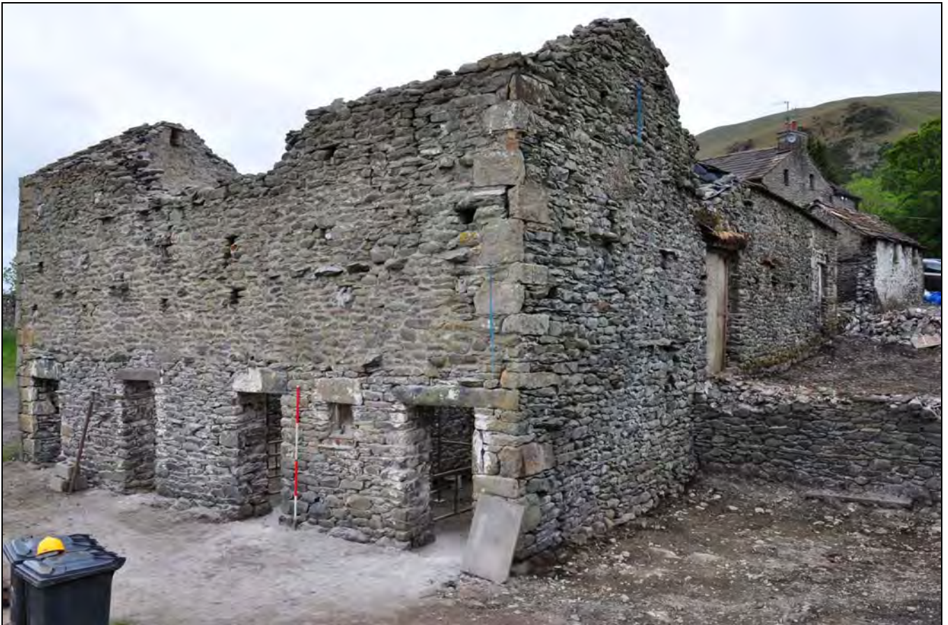
Photo 22: South wing, with main range to right, from the south-east
