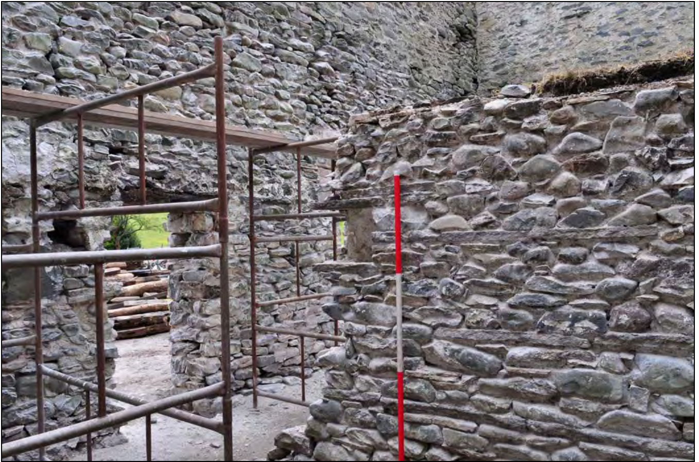
Photo 47: Secondary cross-wall in south wing, from the north-east
