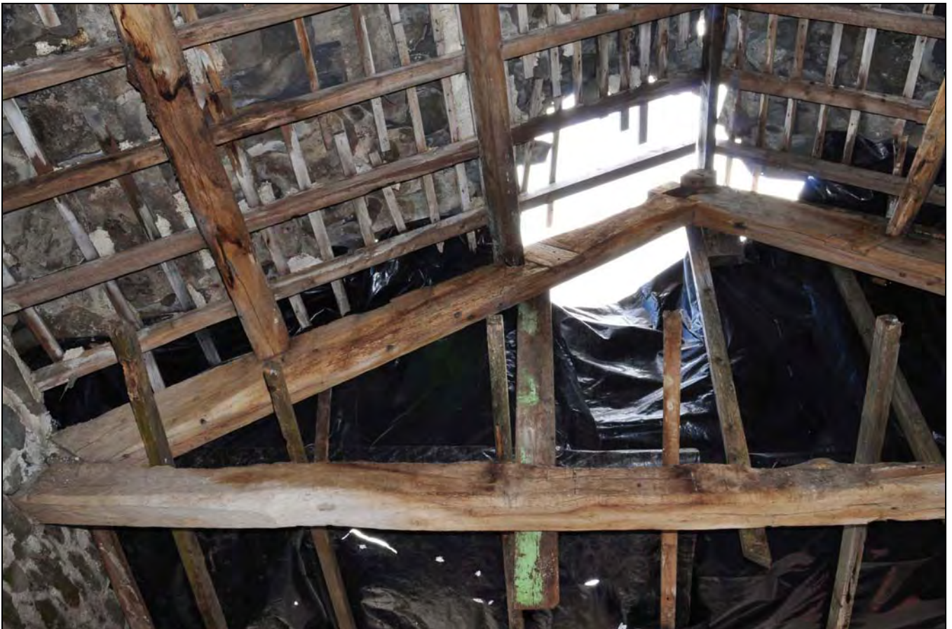
Photo 32: Roof truss over threshing bay, from the north
