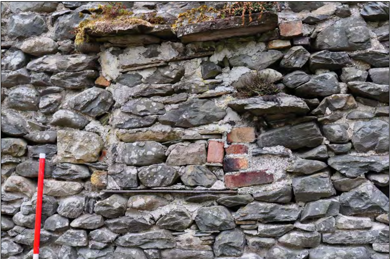
Photo 14: Detail of blocked window, east side of main range
