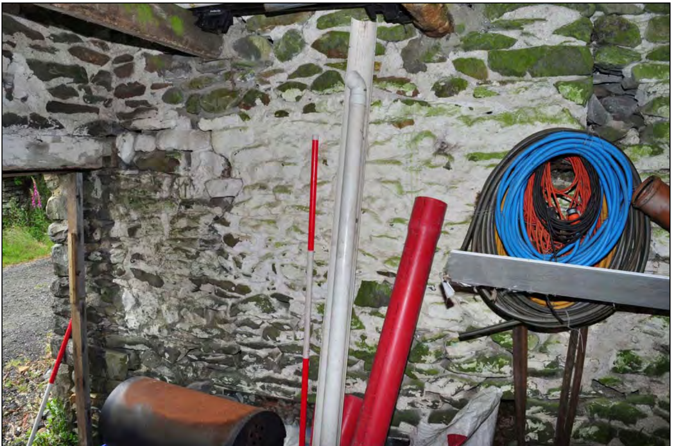
Photo 52: North side of former stable (proposed for new opening)
