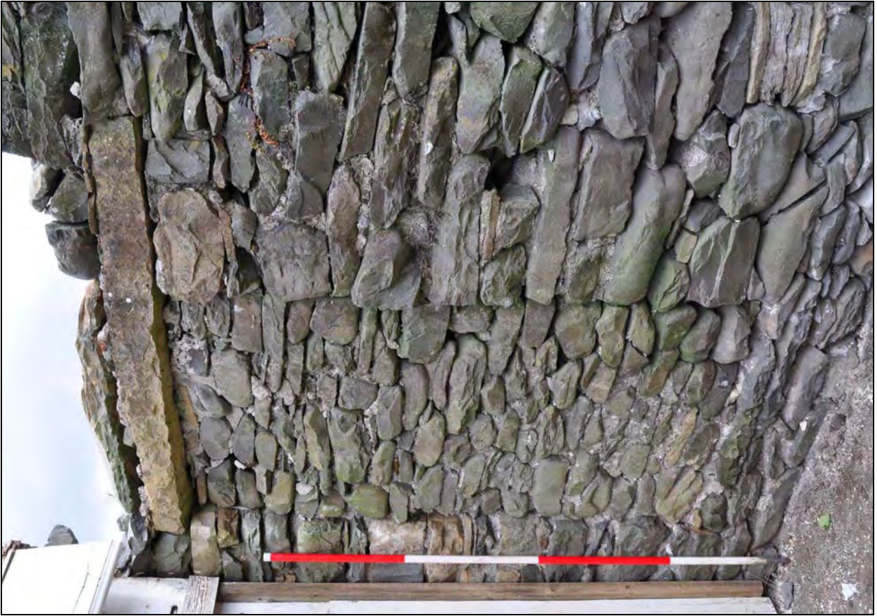
Photo 27: Blocked doorway in north side of south wing, formerly within porch
