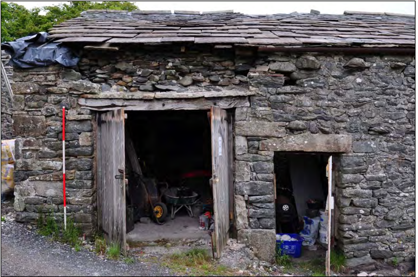
Photo 7: Added bay at north end of main range, from the west
