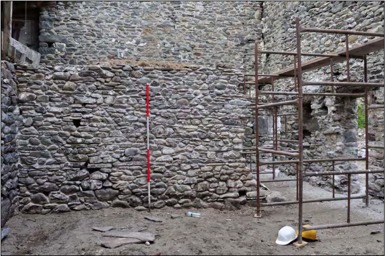
Photo 45: Secondary cross-wall in south wing, from the west
