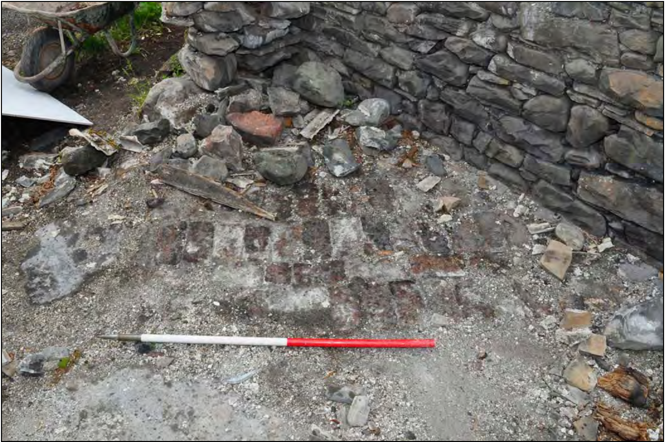
Photo 65: Brick floor within link building, between garage and main range
