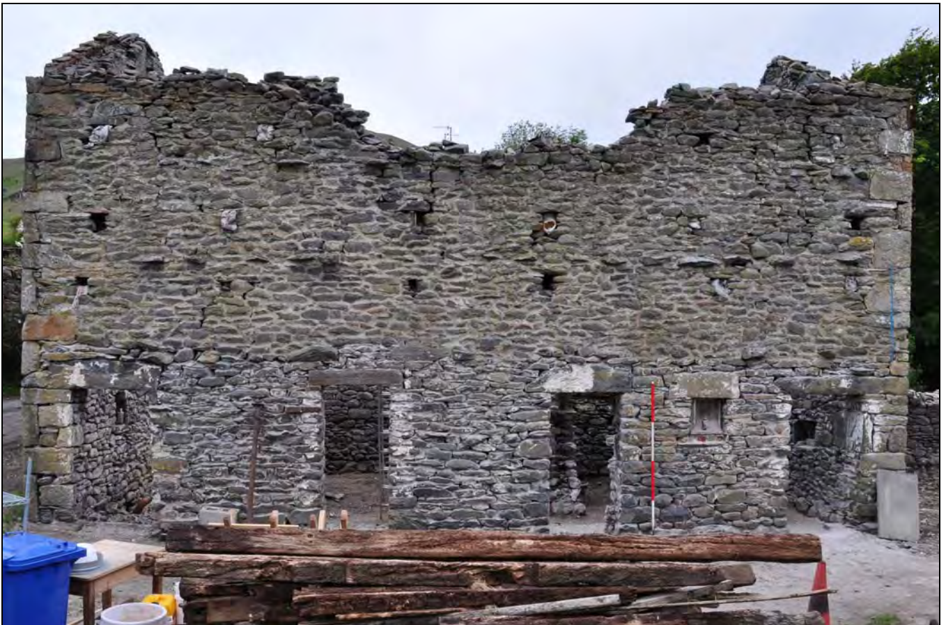
Photo 20: South side of south wing
