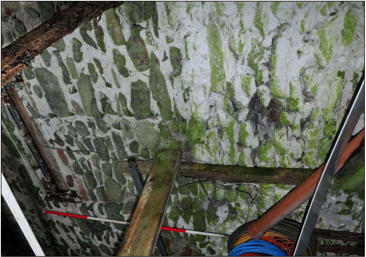
Photo 51: Blocked doorway at upper level, north side of former stable
