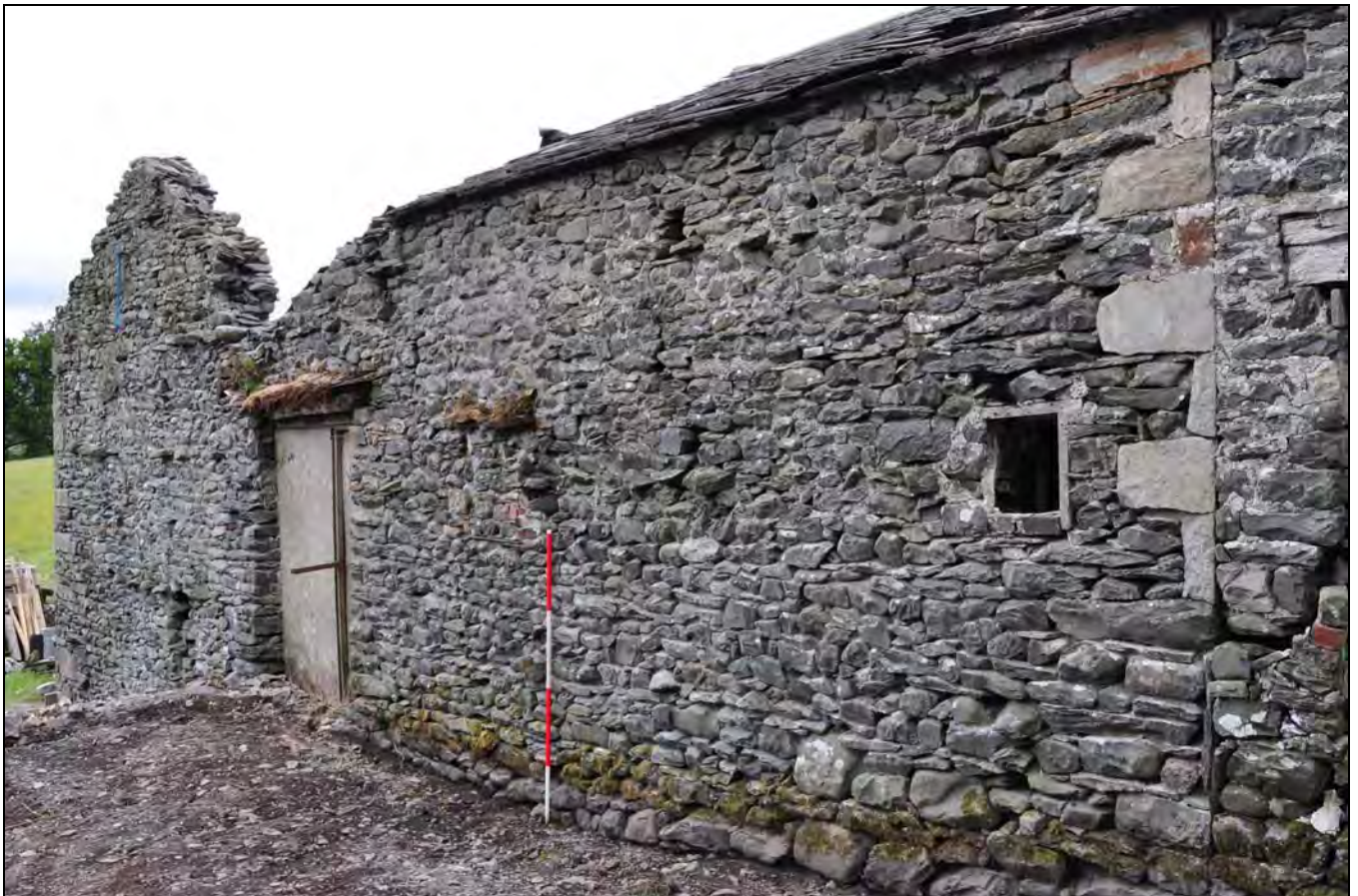
Photo 12: East side of main range and south wing, from the north-east
