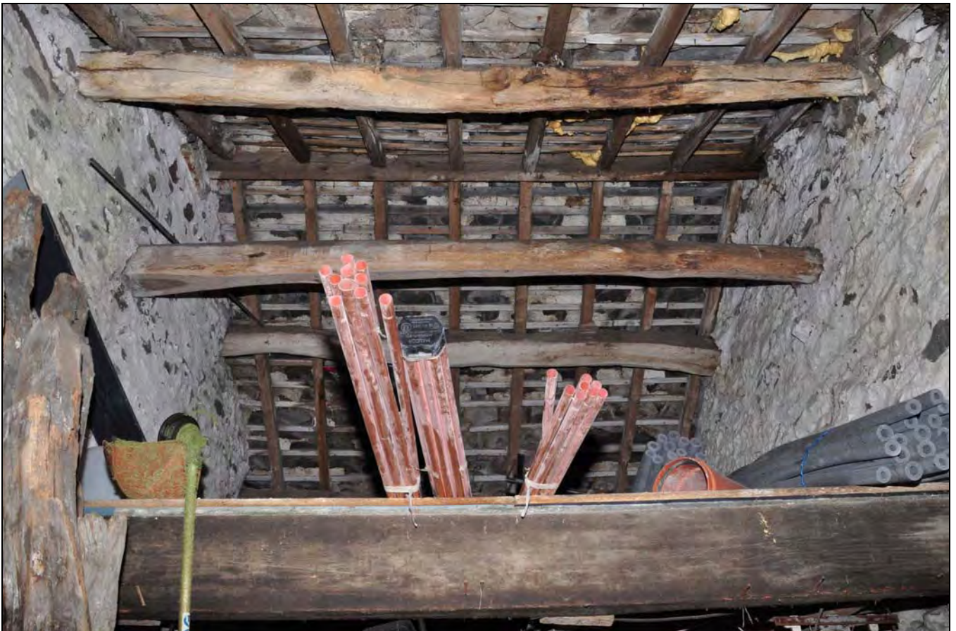
Photo 58: Underside of roof over added north bay
