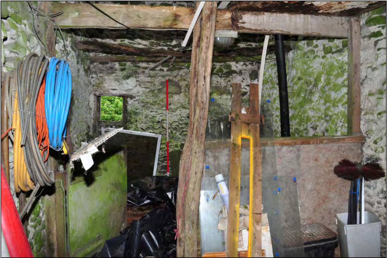
Photo 49: Former stable, from the west
