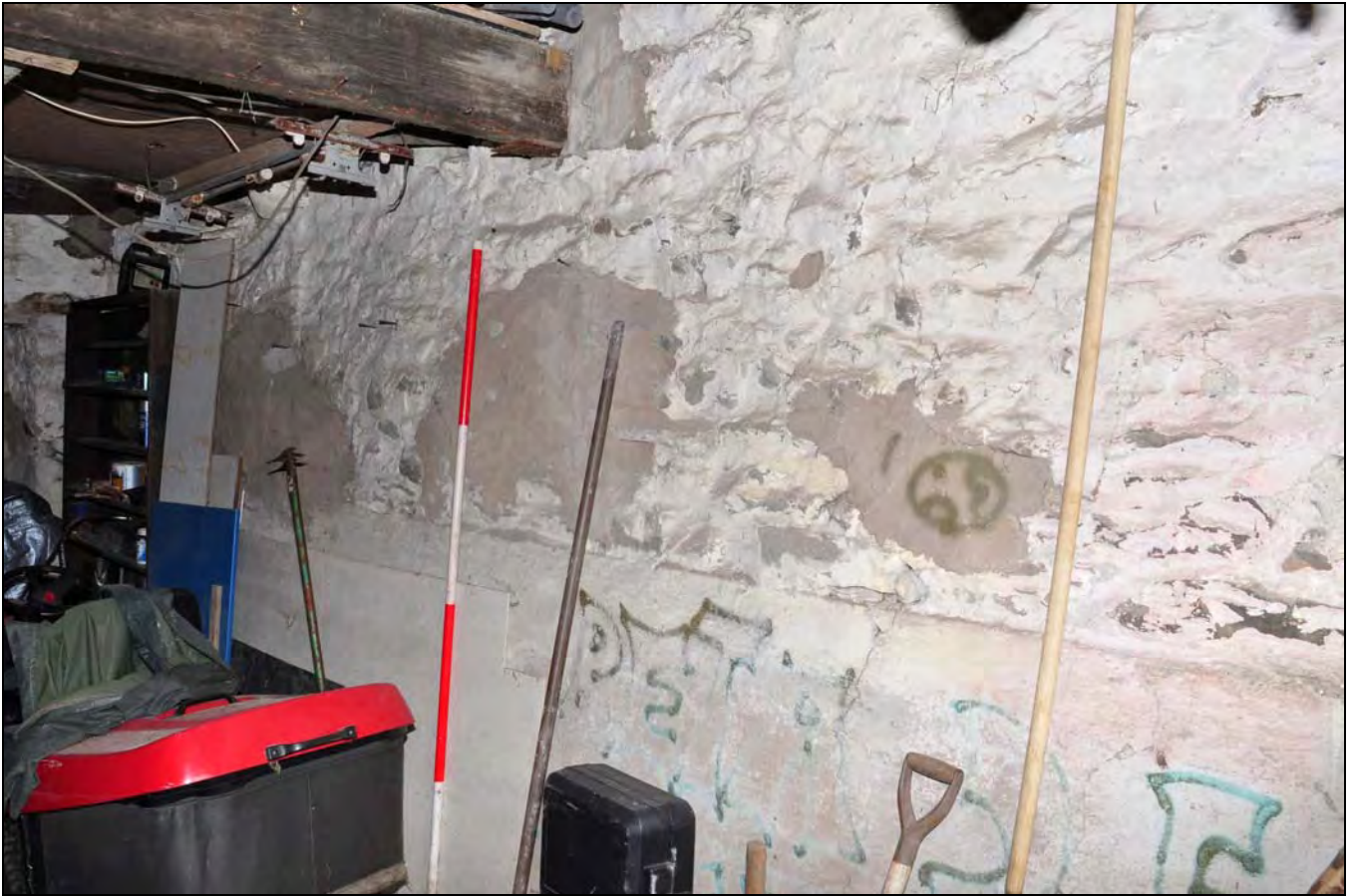
Photo 57: South side of added north bay (proposed for new opening)
