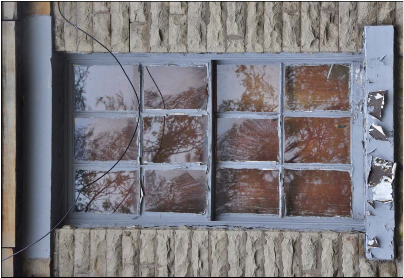
Photo 16: Twelve-pane sash (probably original), top floor, Holme Street elevation
