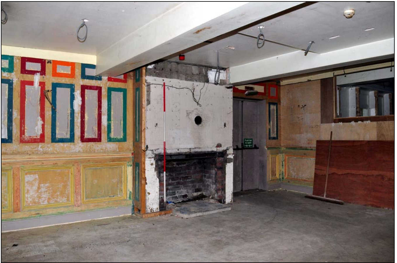
Photo 37: Basement: present bar area within former stables, looking east
