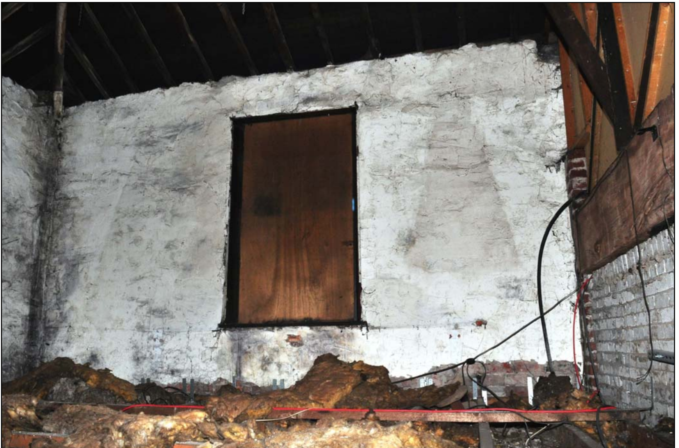
Photo 50: First floor: top floor of Dutton Street dwelling, looking south
