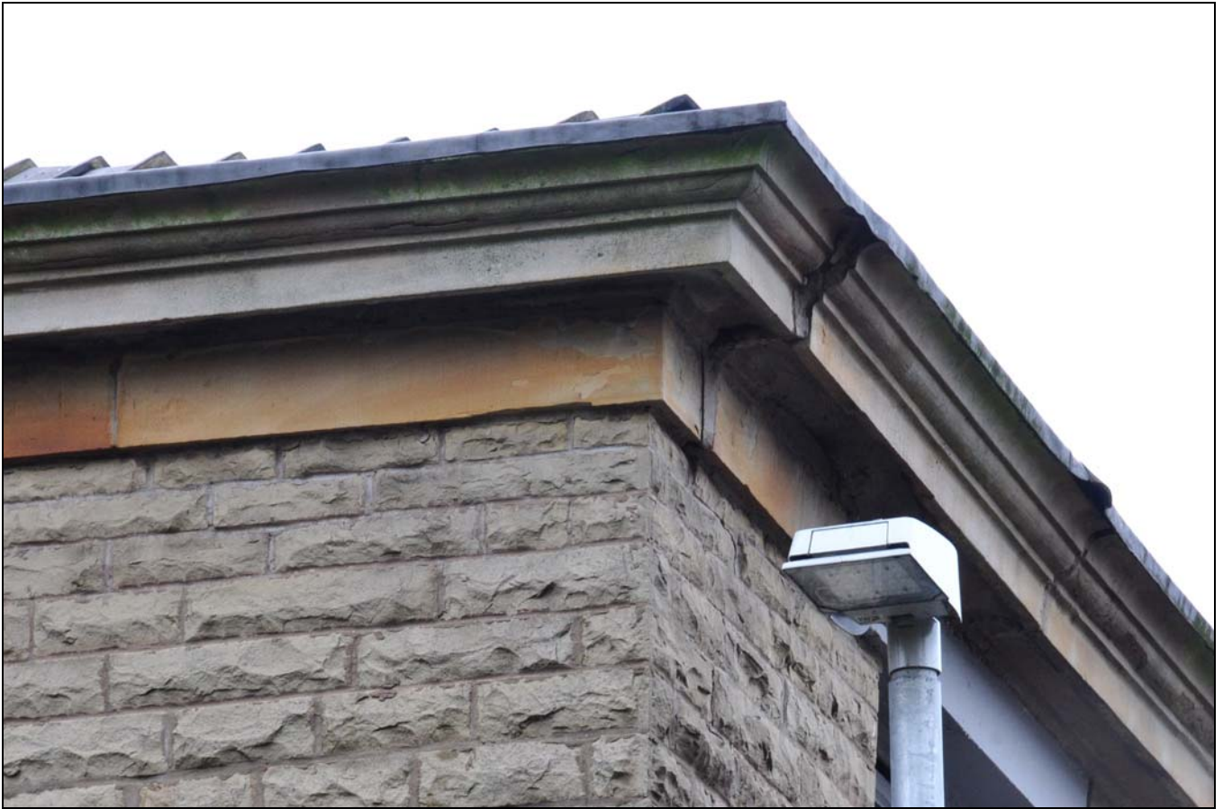
Photo 7: Detail of stone cornice (rainwater trough)
