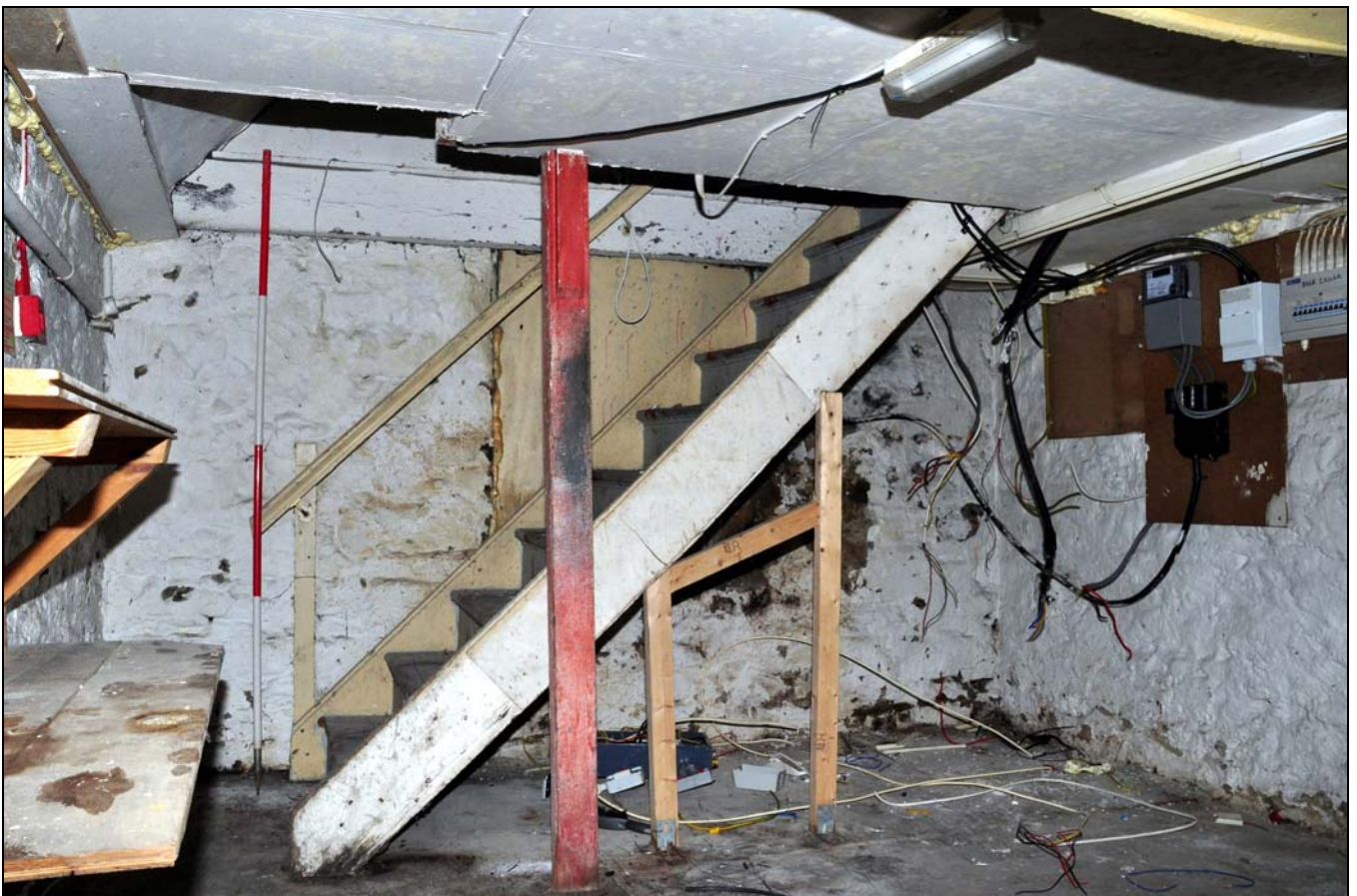
Photo 34: Basement: modern staircase in west cellar, looking north-west
