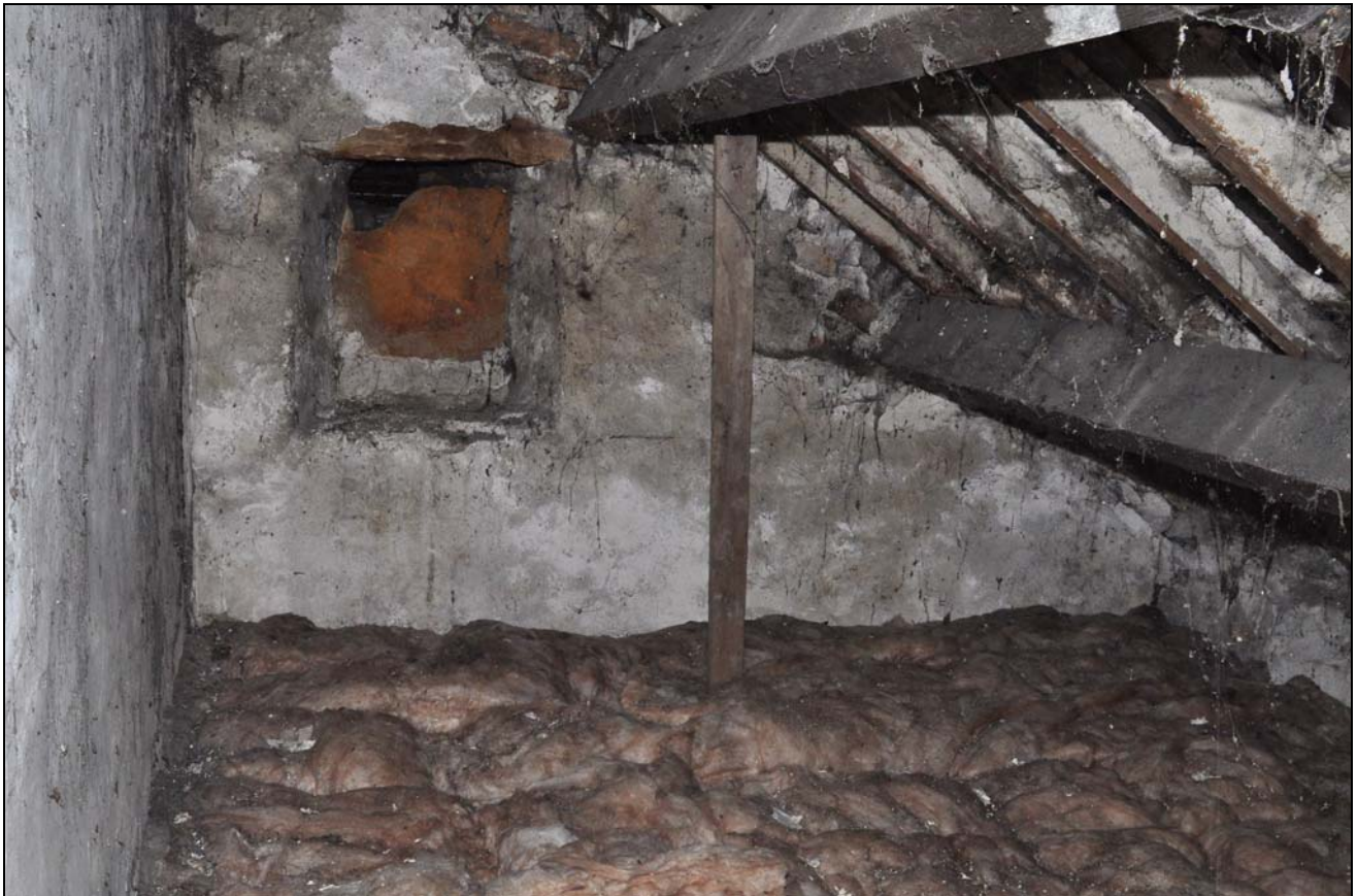
Photo 46: House interior: attic, north-west room
