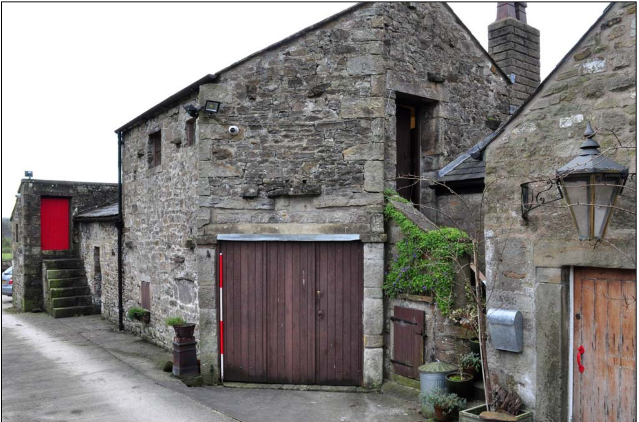
Photo 53: Trap-house, looking south-east
