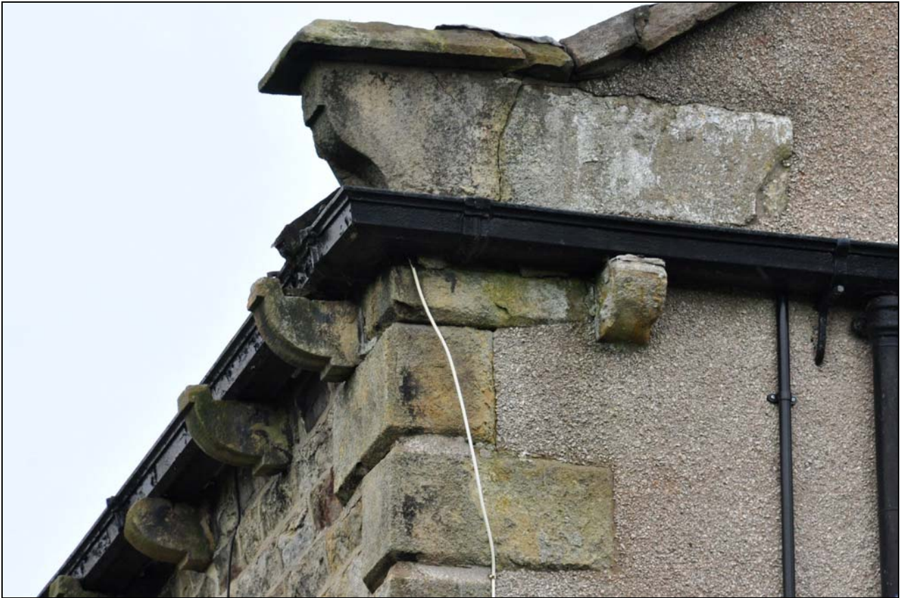
Photo 13: House: detail of quoins, kneeler and corbels at south-east corner
