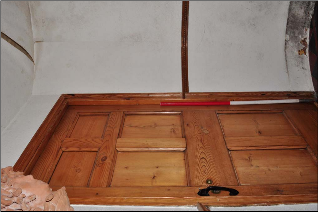
Photo 20: House interior: front lobby, with door to parlour
