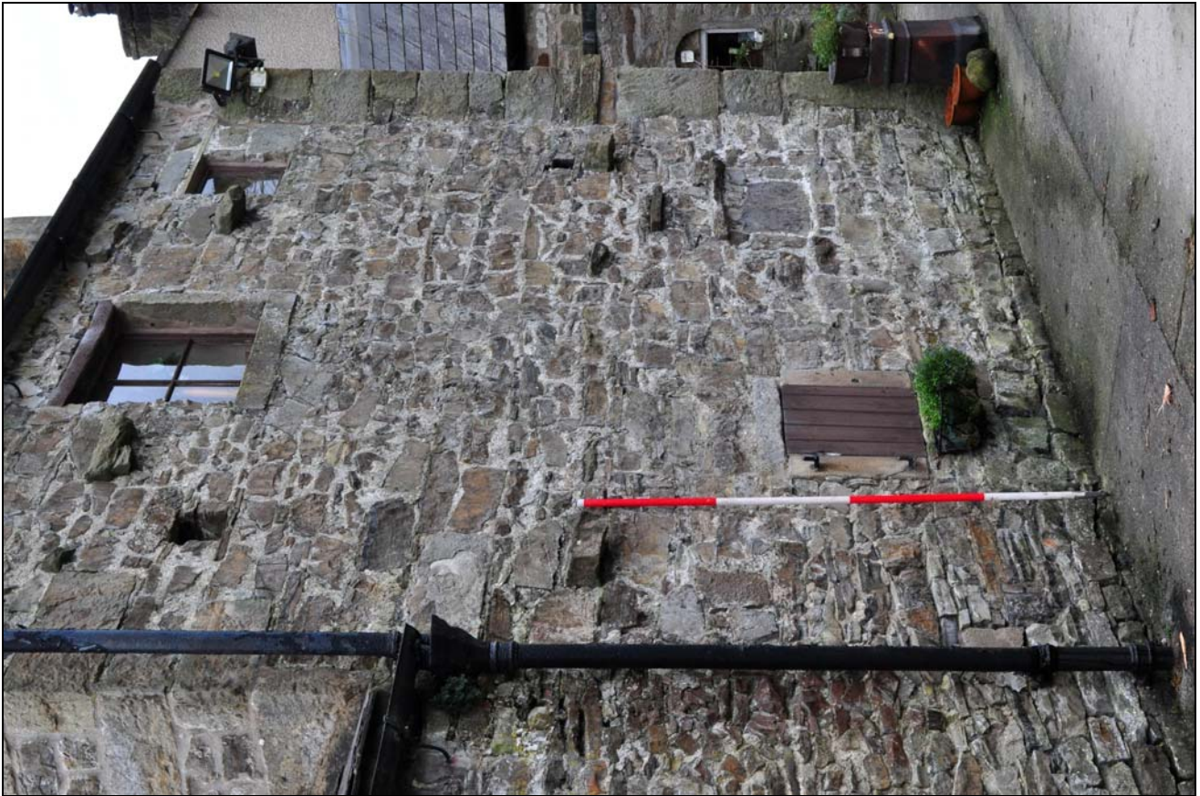
Photo 55: Trap-house, north side, looking south-east
