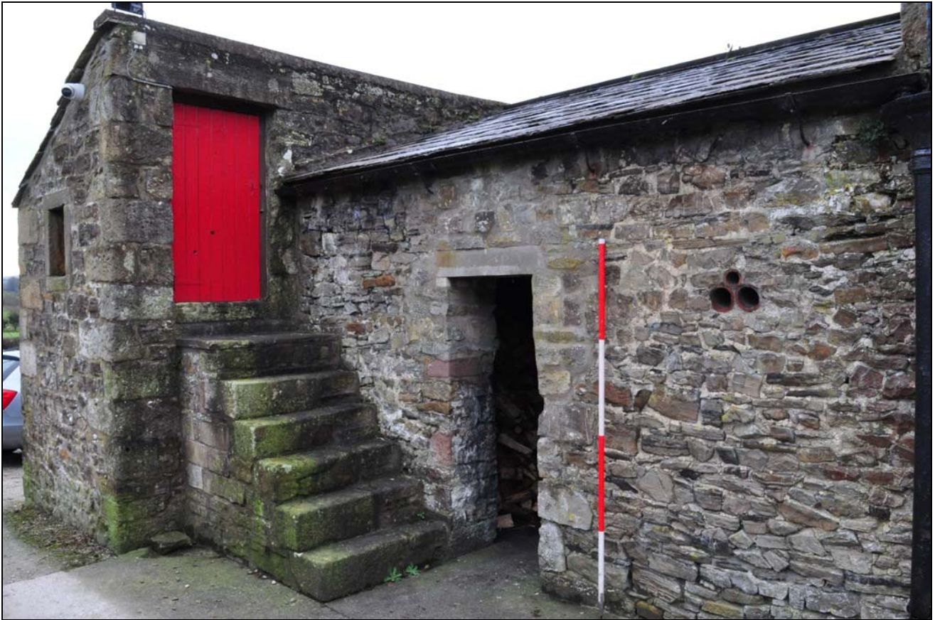
Photo 61: Outbuildings at east end, looking south-east
