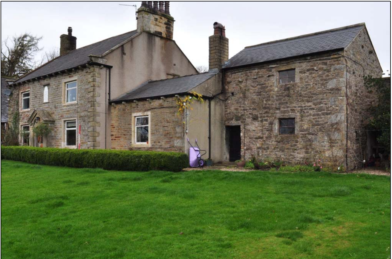
Photo 5: House and trap-house, from the south-east
