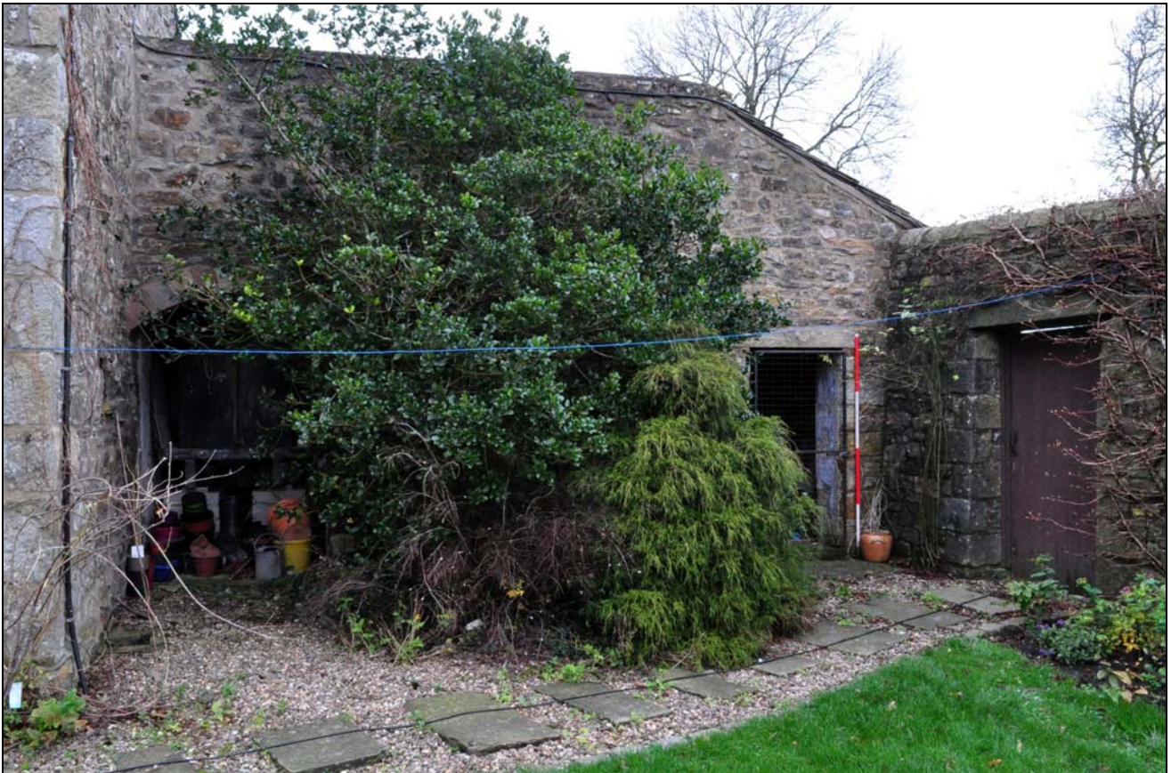
Photo 63: Outbuildings at east end, looking north
