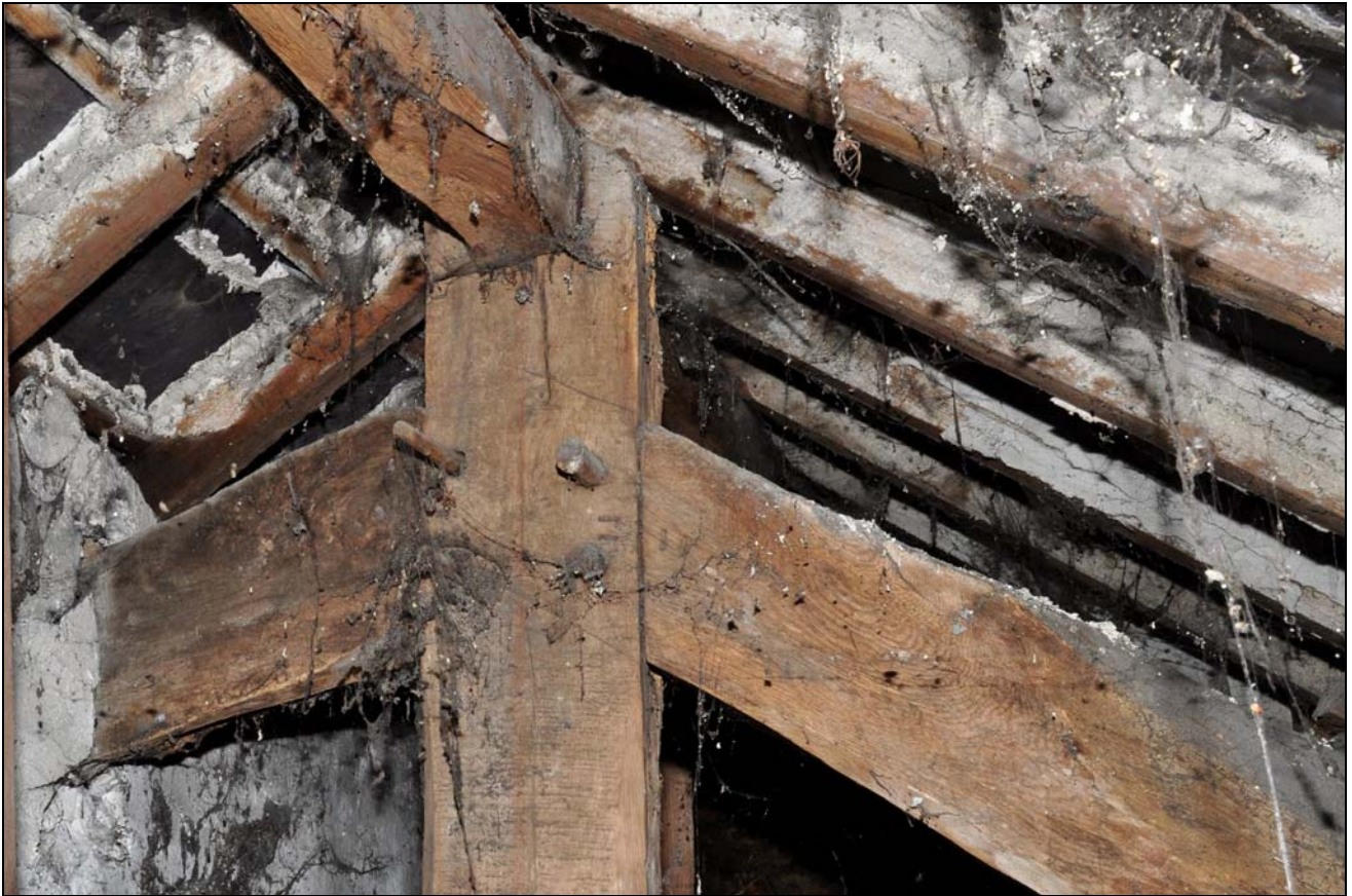
Photo 51: House interior: head of east roof truss
