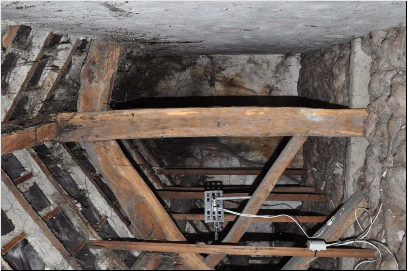
Photo 47: House interior: west roof truss, looking west
