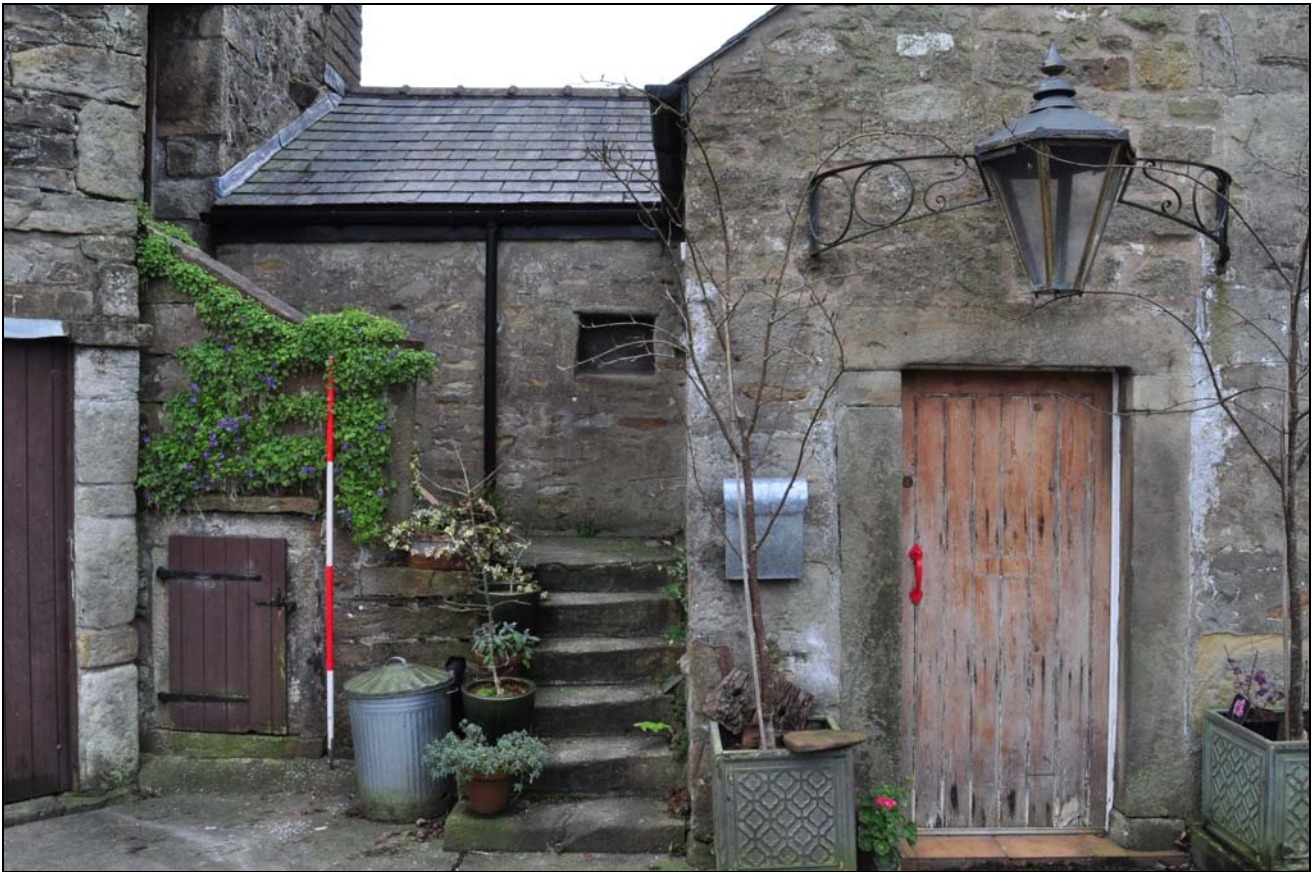
Photo 57: Rear porch to house, and link to trap-house, from the north
