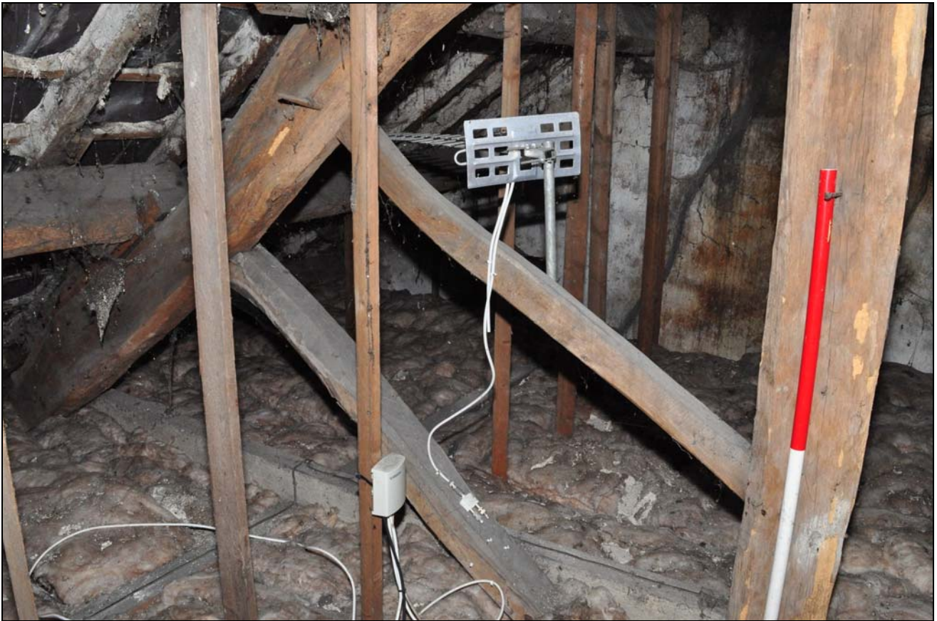
Photo 48: House interior: west roof truss, looking south-west
