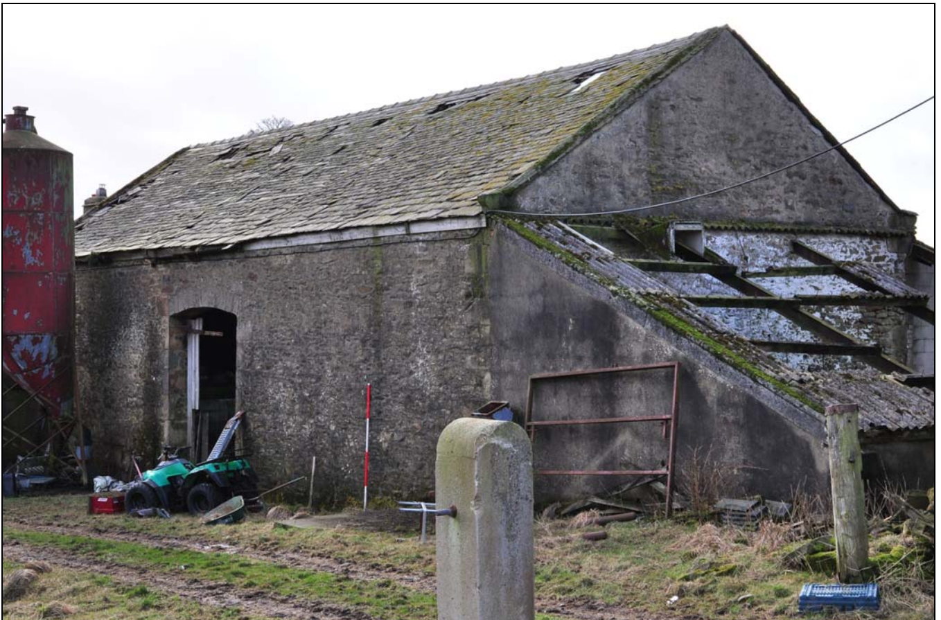
Photo 3: Barn 1: general view, looking south-west
