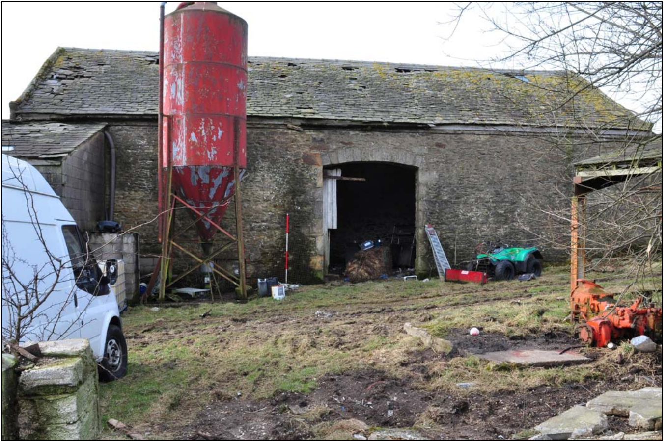
Photo 1: Barn 1: general view, looking west
