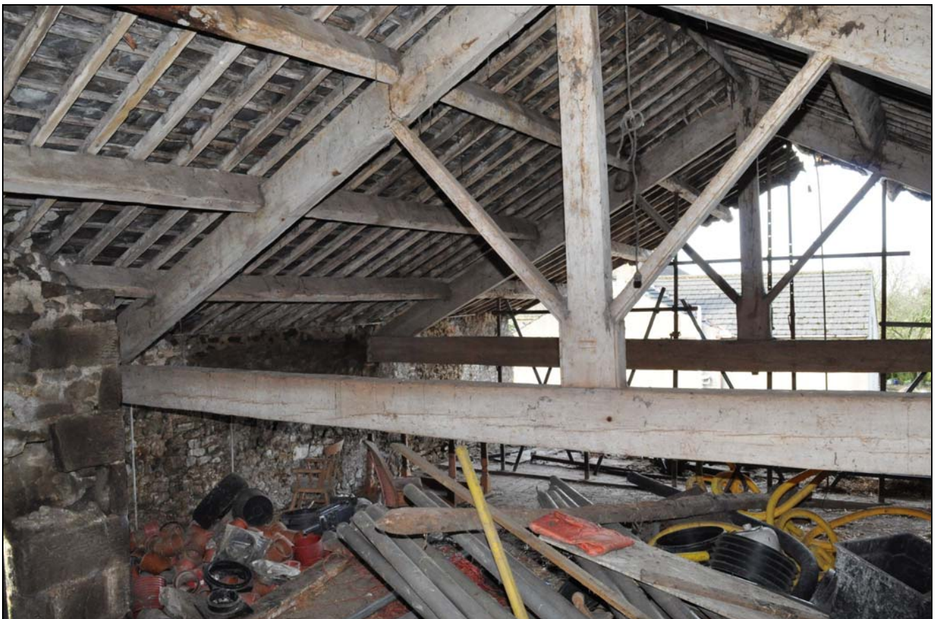
Photo 32: Barn 2: roof trusses and hayloft, looking south-west
