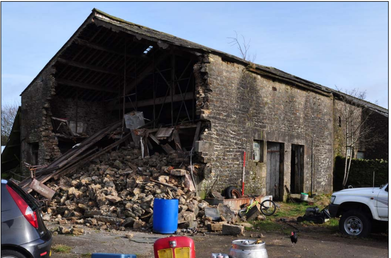
Photo 22: Barn 2, looking north-east
