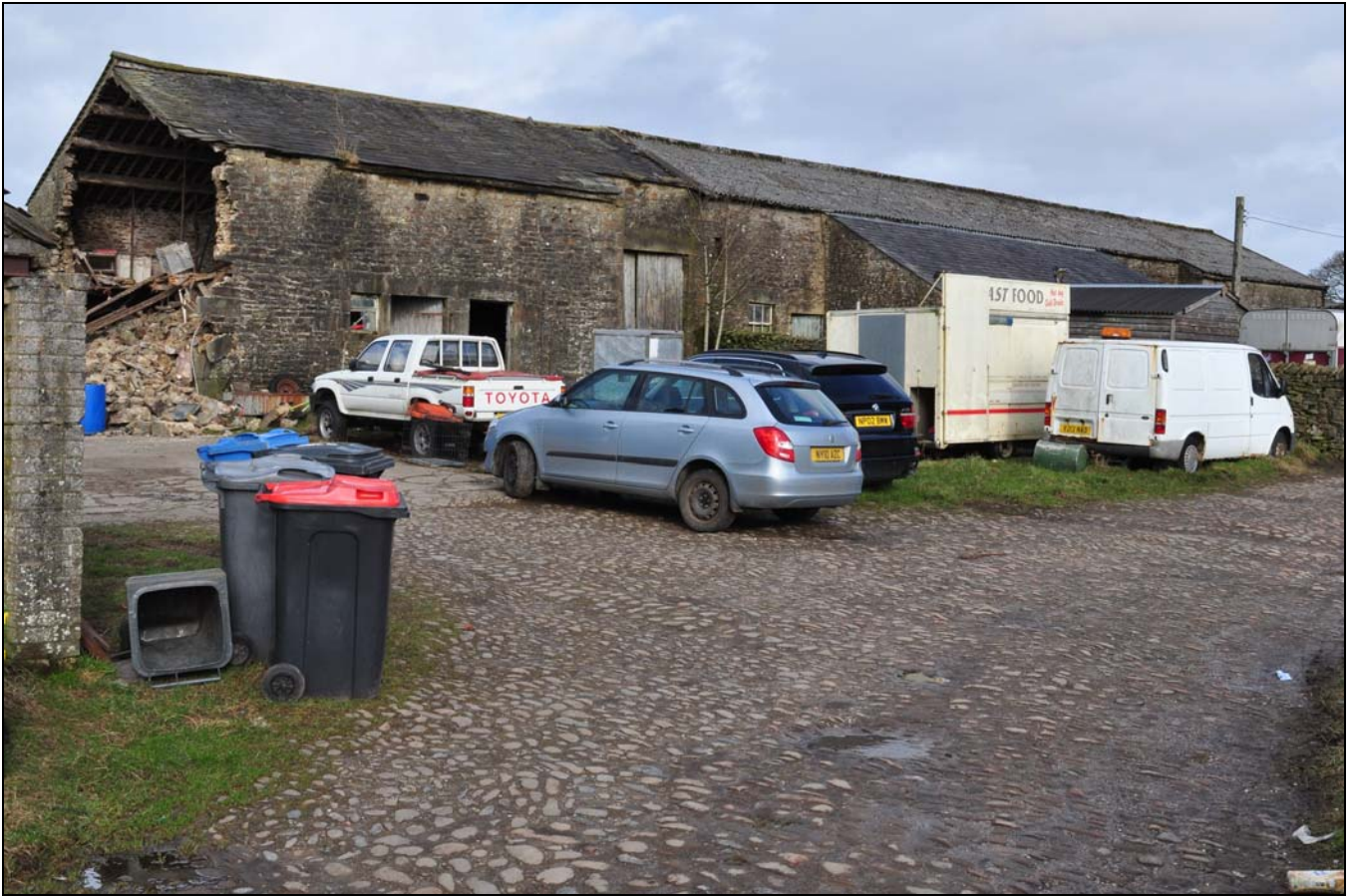
Photo 21: Barn 2 and adjoining range (part of adjacent property), looking north-east
