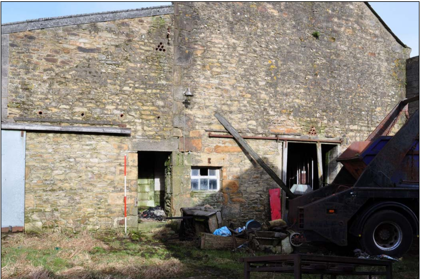
Photo 10: Barn 1: south gable, with remnant of added outhshut at left
