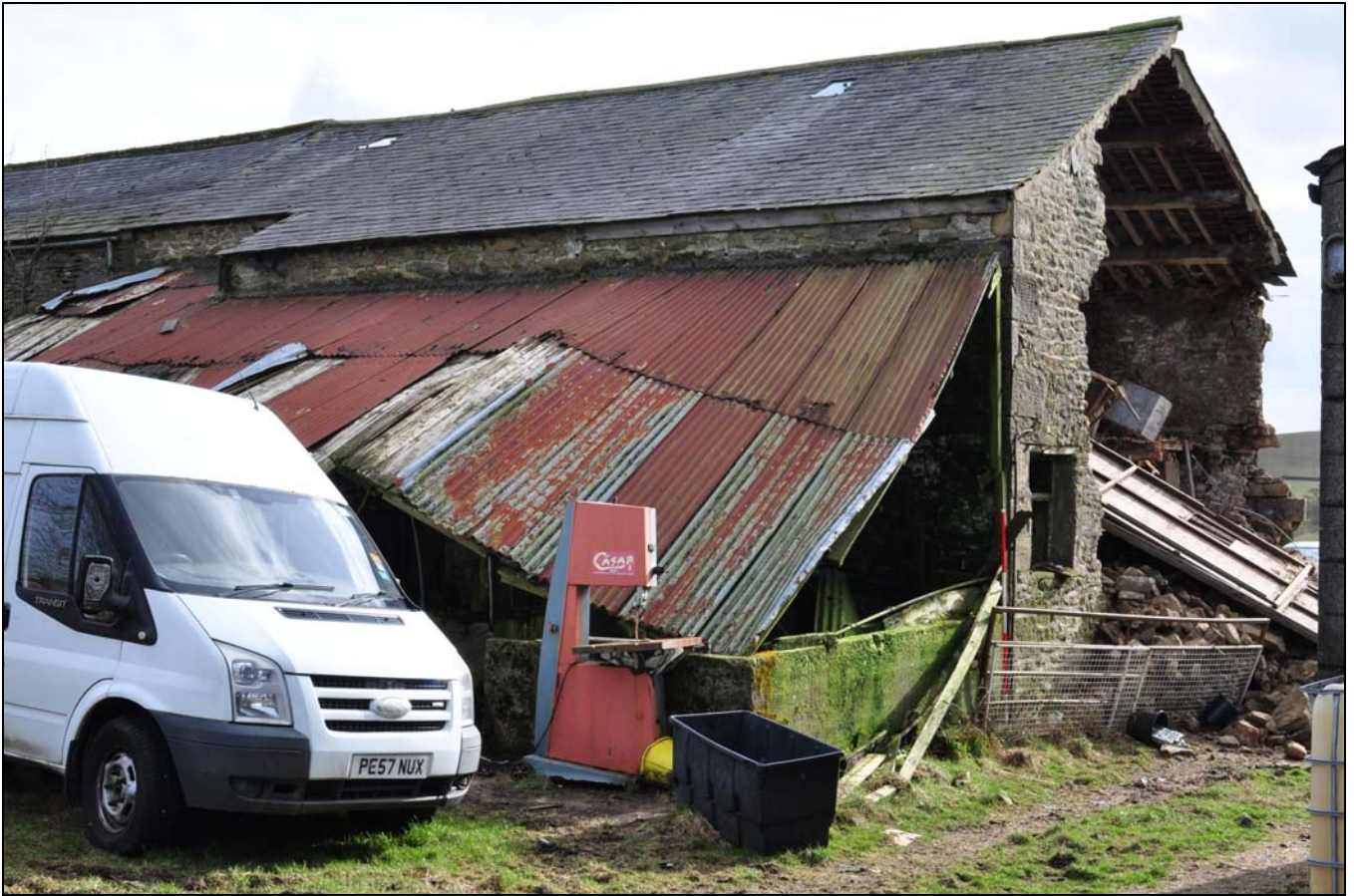
Photo 26: Barn 2, looking south-east
