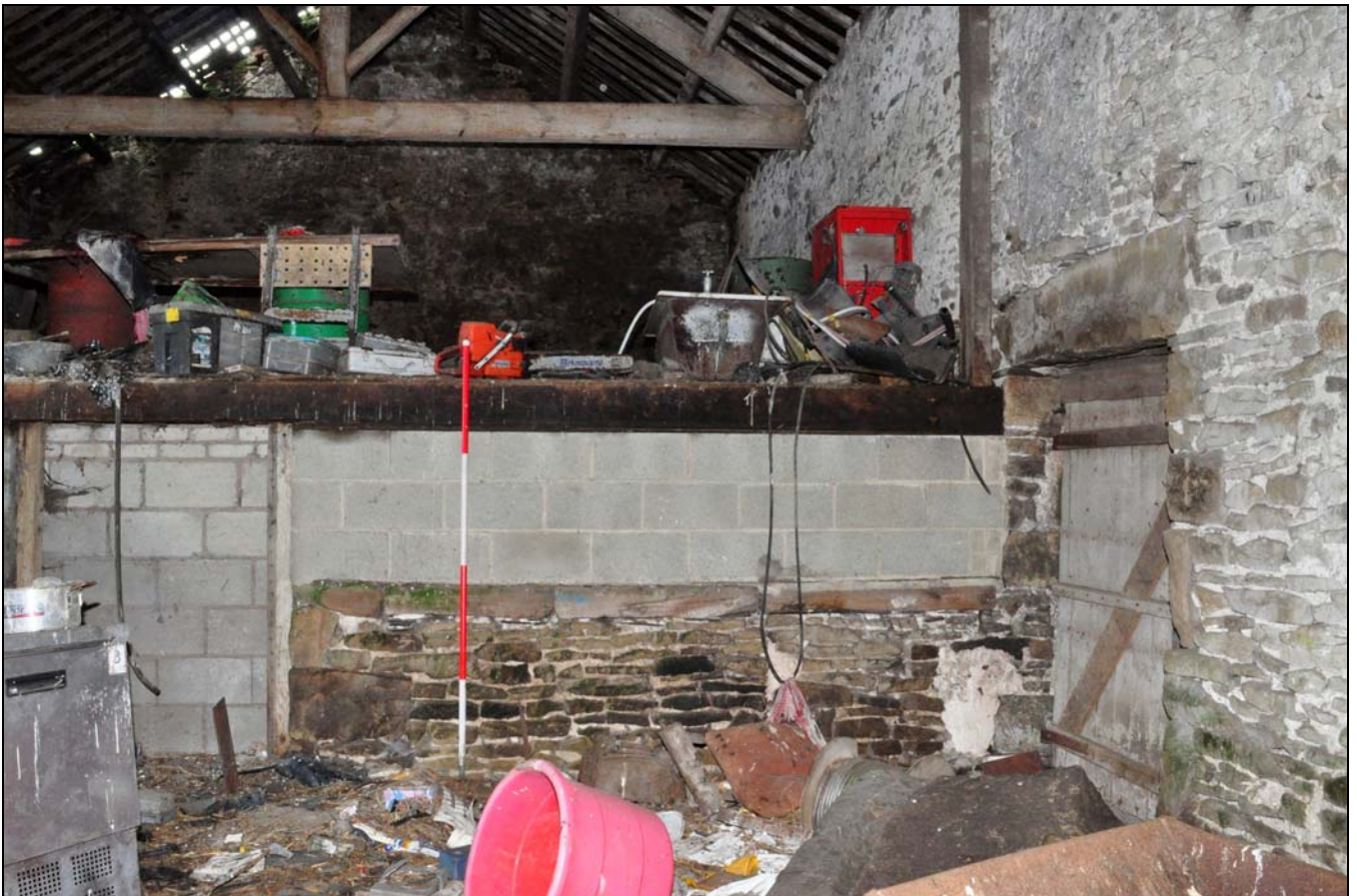
Photo 16: Barn 1: stone cross-wall enclosing former shippon in south end
