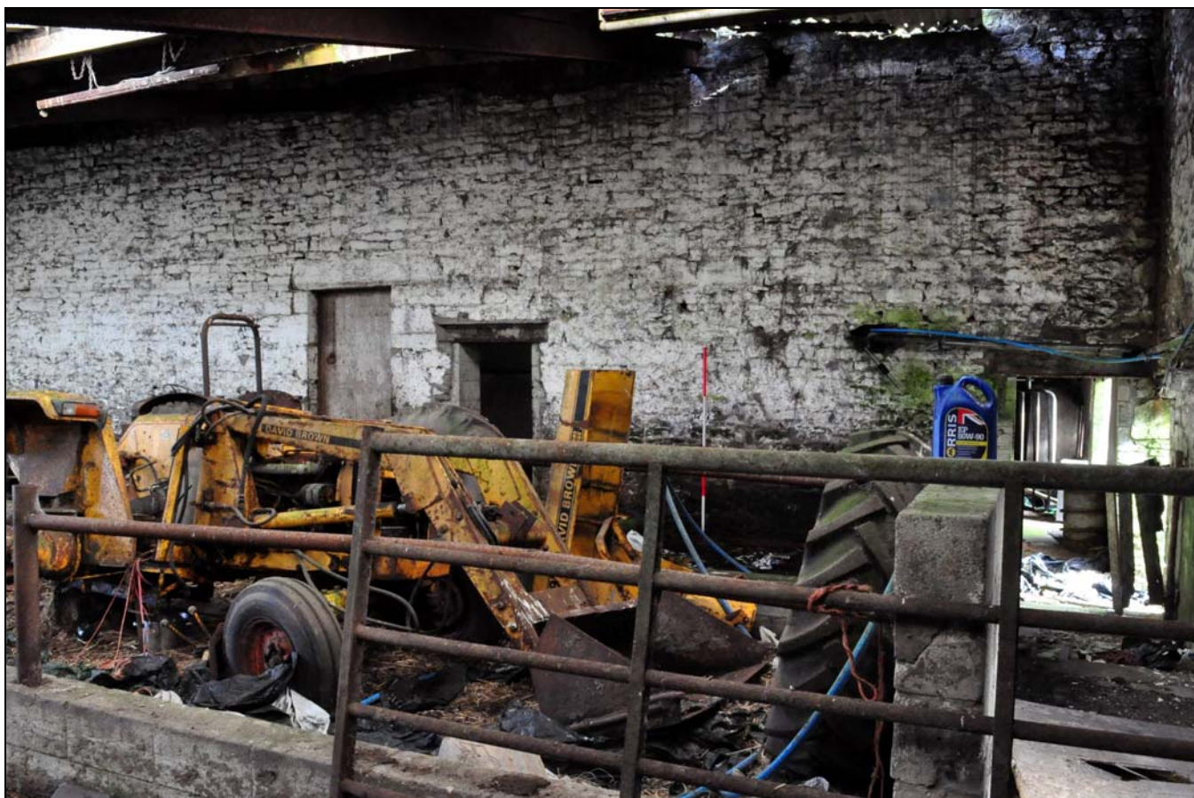
Photo 6: Barn 1: west elevation, looking north-east
