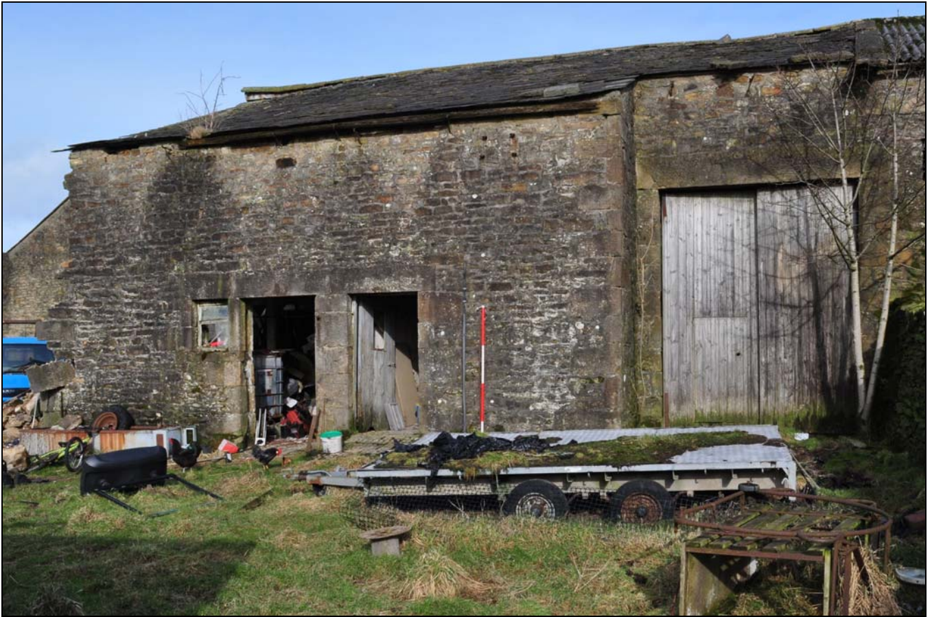
Photo 23: Barn 2: south elevation
