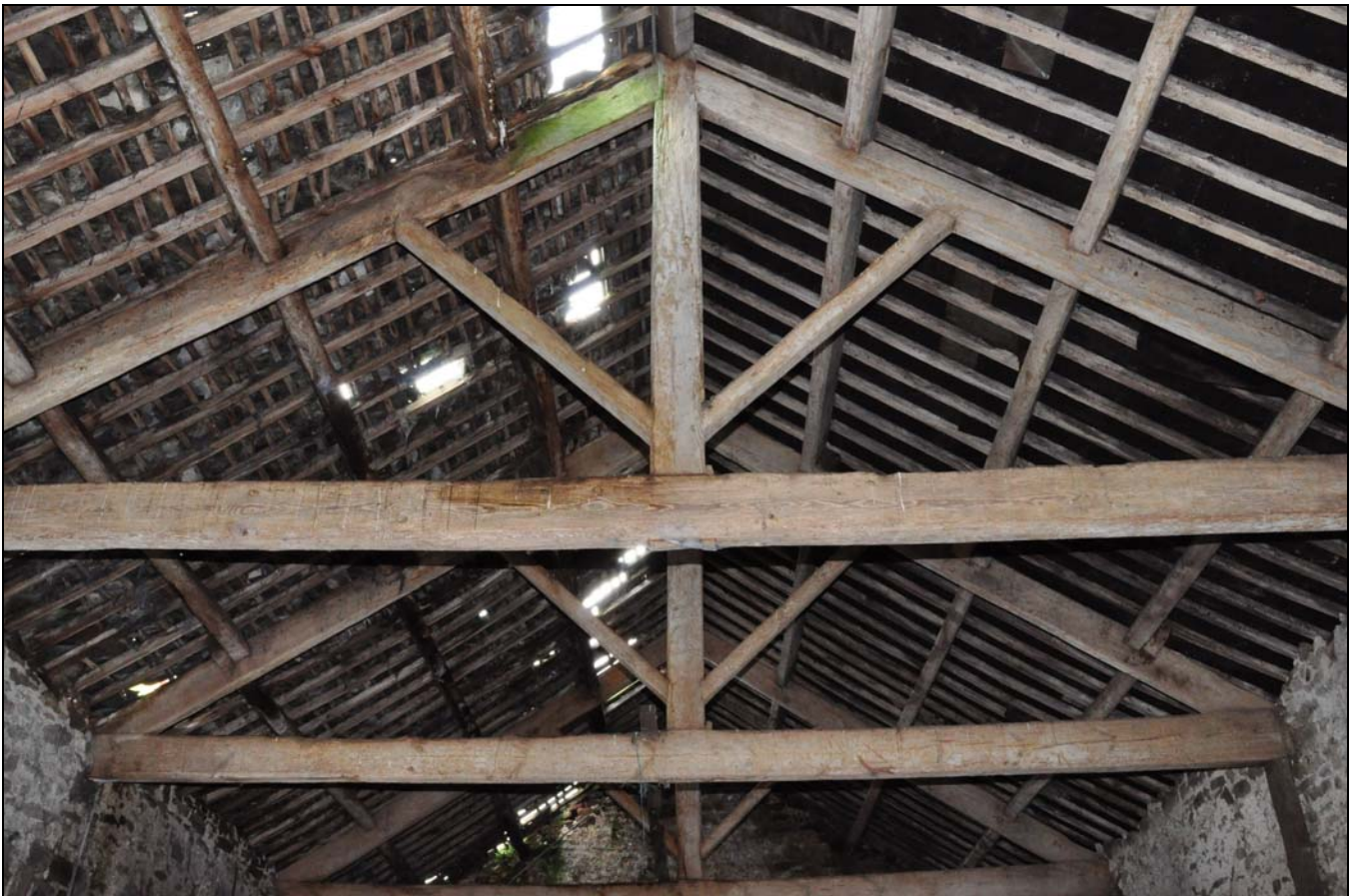
Photo 20: Barn 1: roof trusses, looking south
