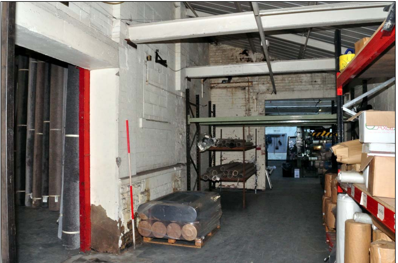
Photo 43: Detached weaving shed: interior of extension to warehouse (1917 engine house?)
