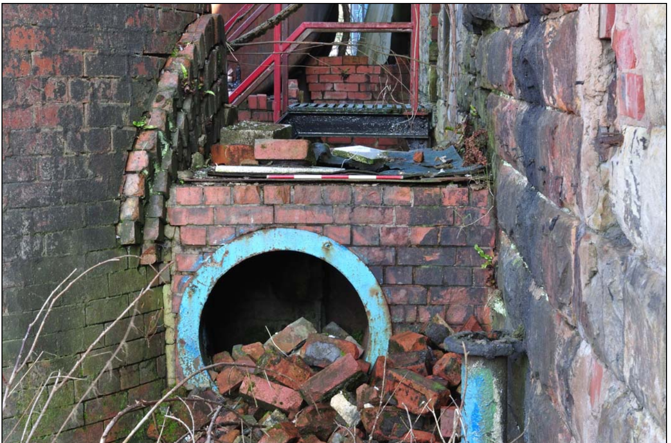
Photo 14: Pipe in west side of flue to chimney
