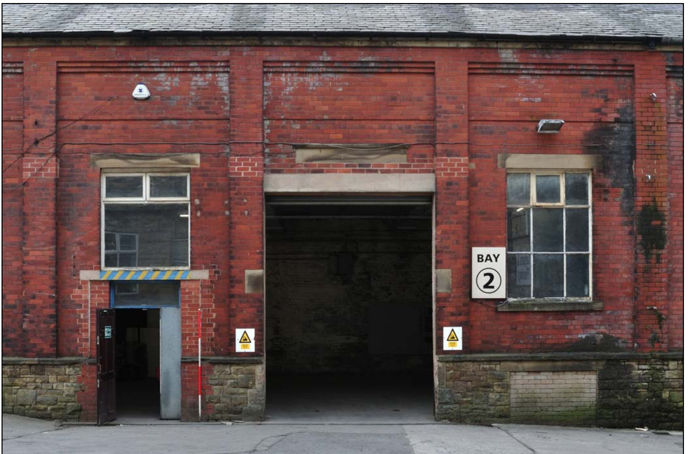
Photo 26: Detached weaving shed: enlarged loading entrance to warehouse
