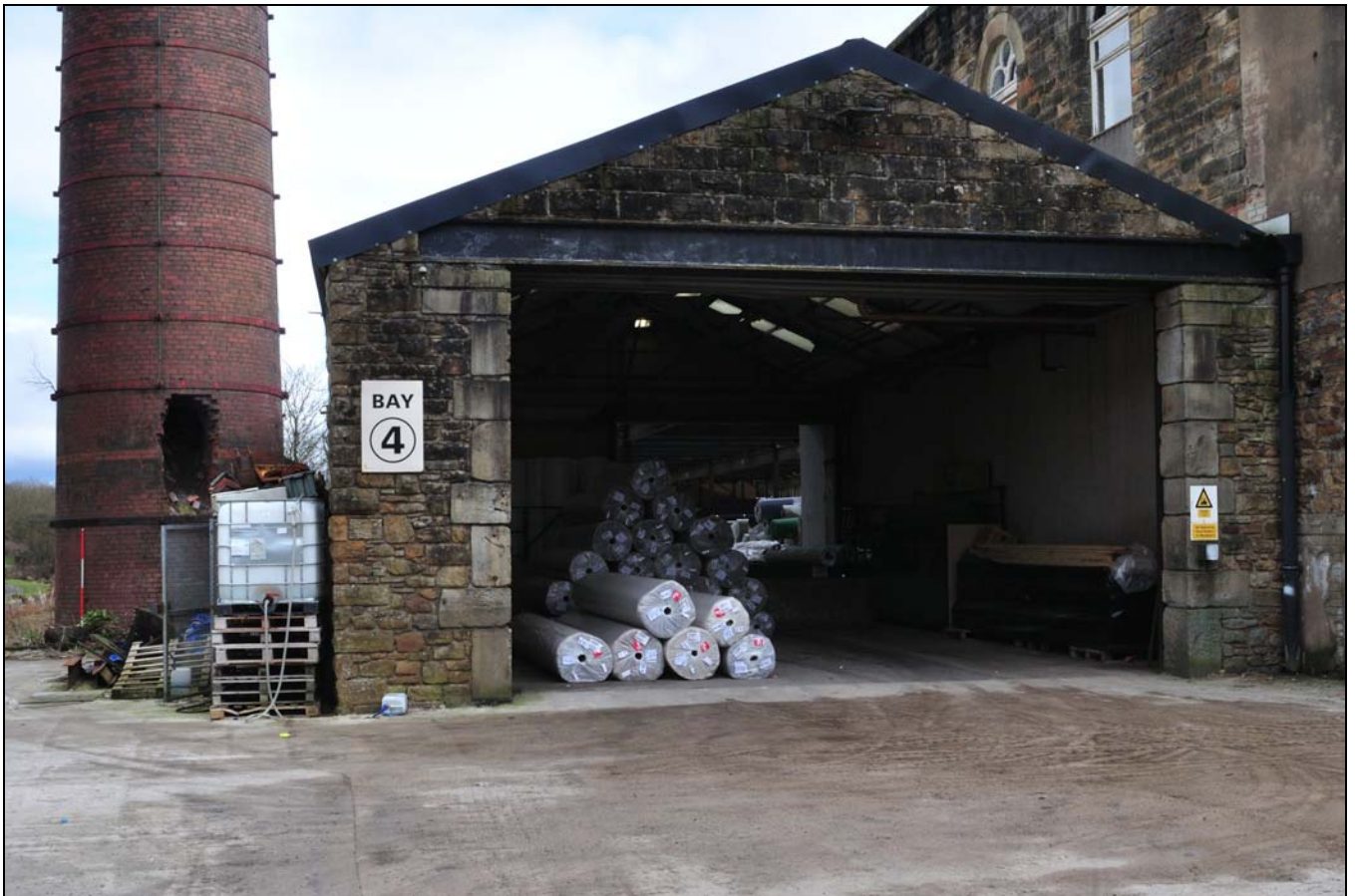
Photo 10: Chimney and boiler house, from the south-west
