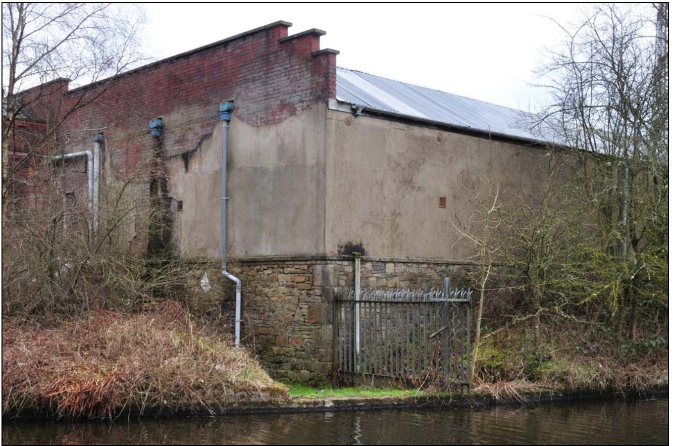
Photo 21: Detached weaving shed: west corner
