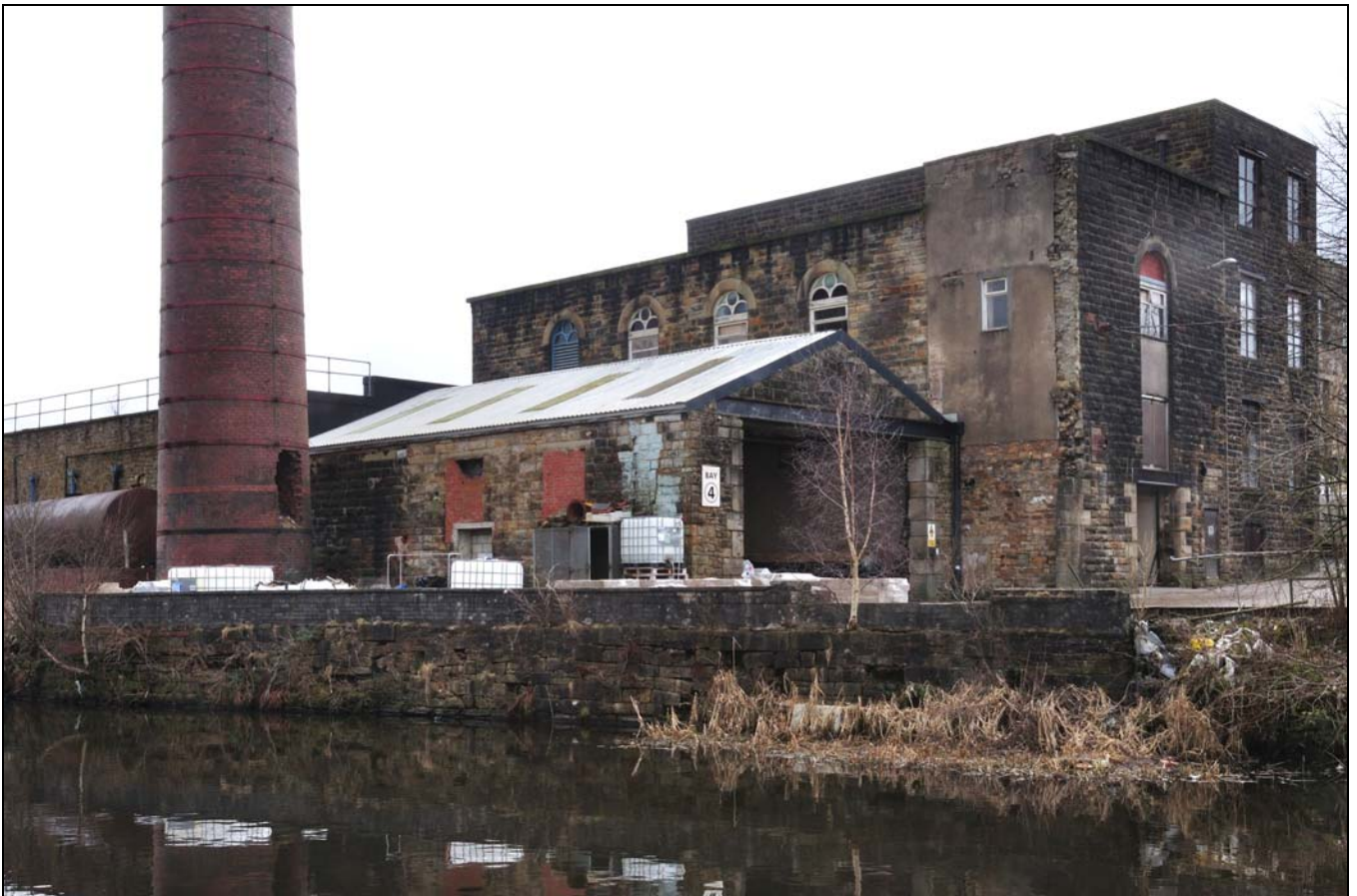
Photo 9: Chimney, boiler house, and engine house, from the north-west
