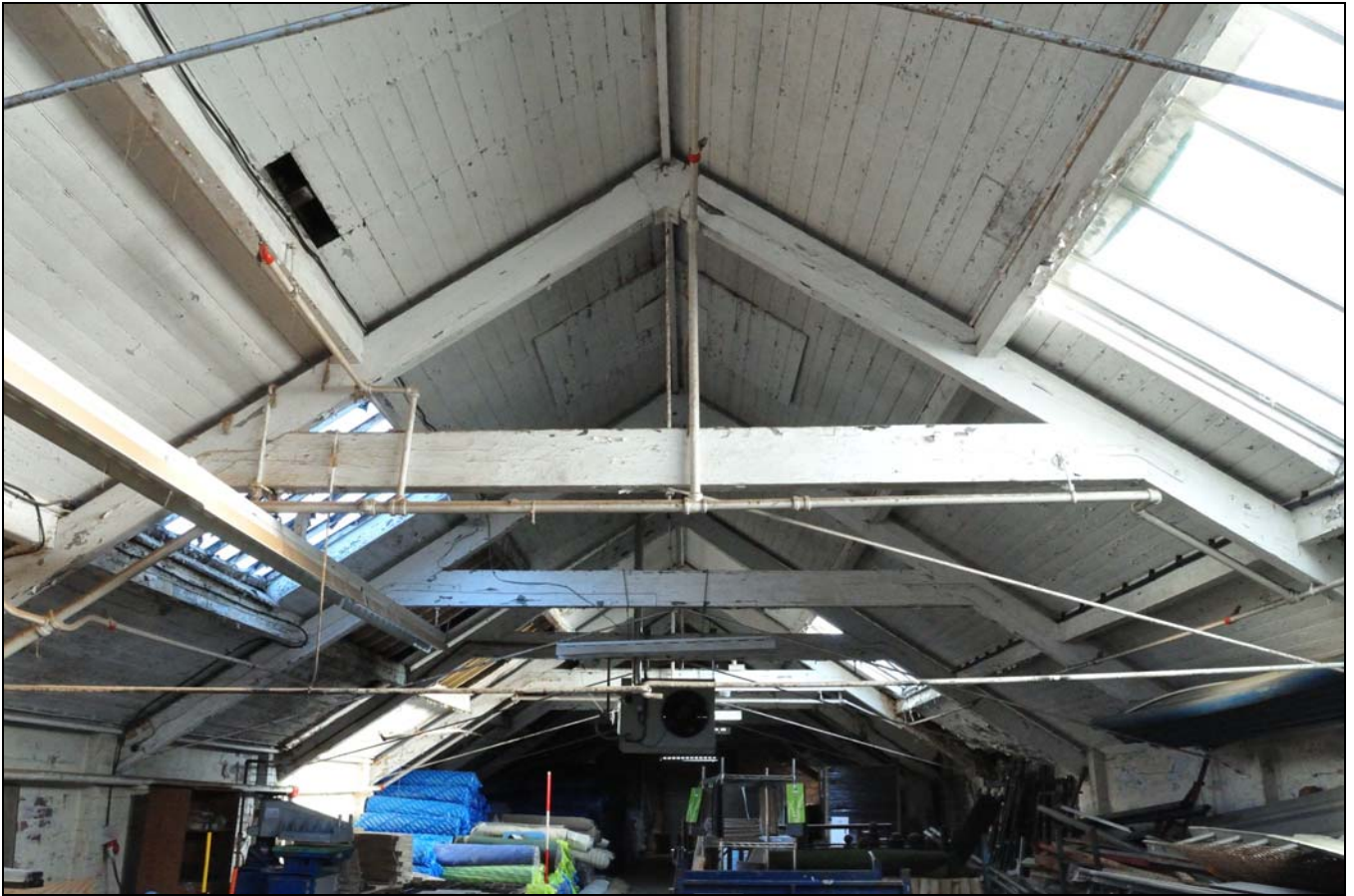
Photo 38: Detached weaving shed: roof structure to warehouse, looking south-east
