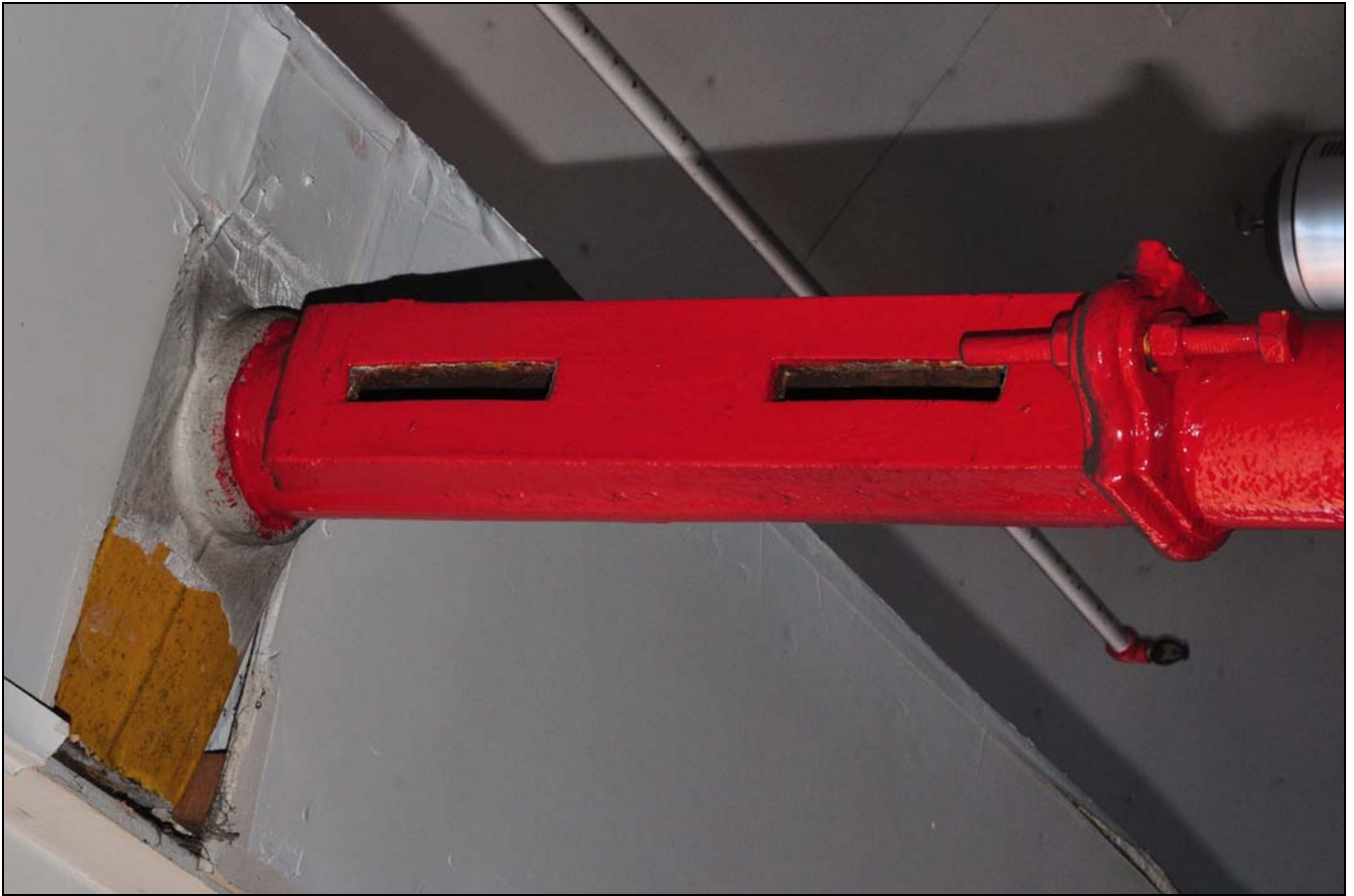
Photo 51: Detached weaving shed: detail of column head bolting face
