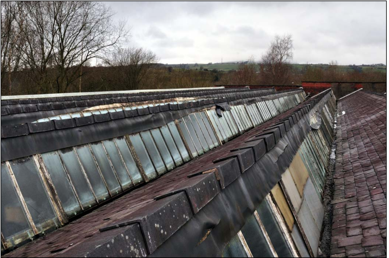
Photo 45: Detached weaving shed: saw-tooth roof, looking north-west
