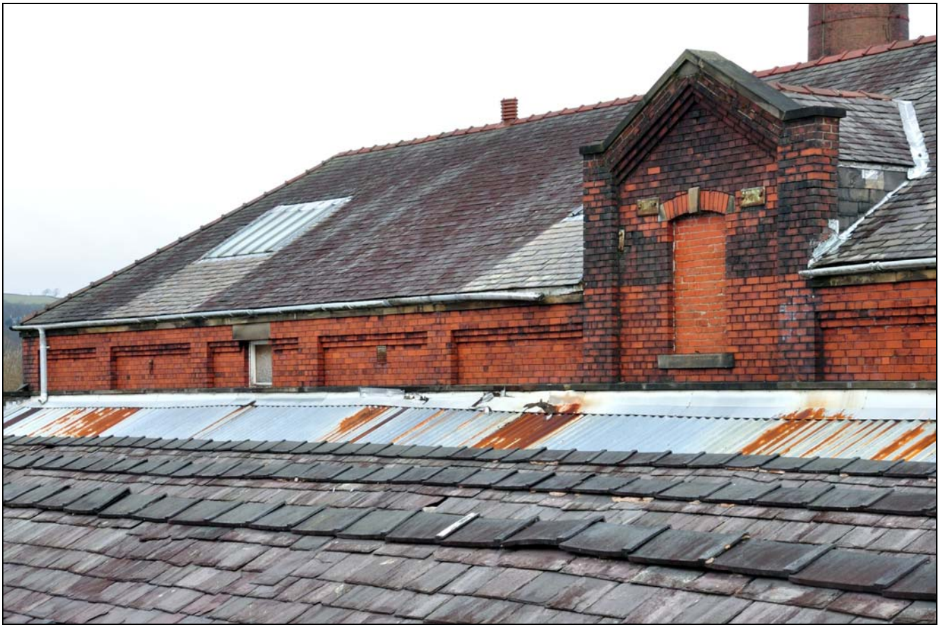
Photo 32: Detached weaving shed: south-west side of warehouse, north-east end
