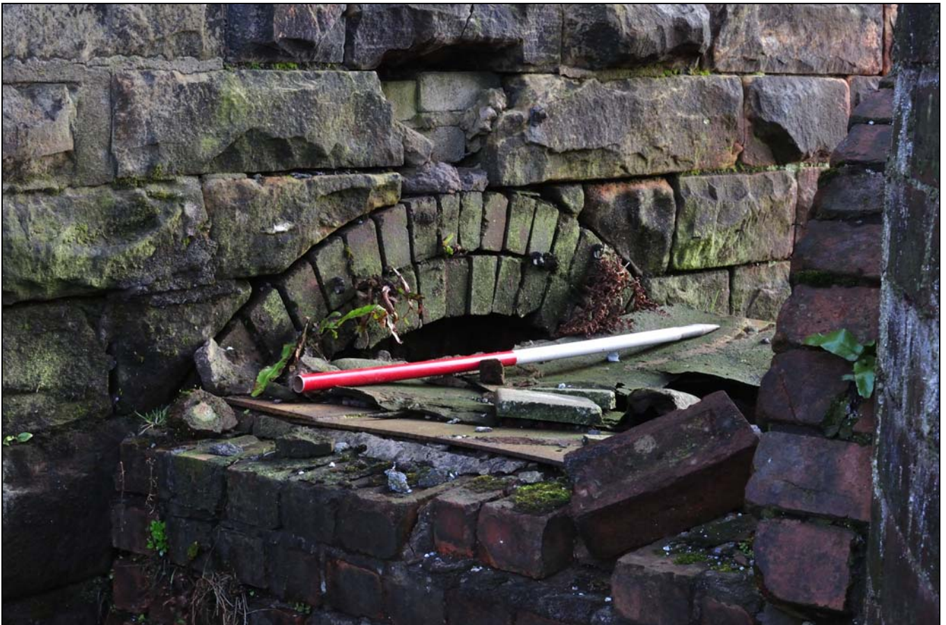
Photo 17: Detail of arched construction to flue, egress from boiler house
