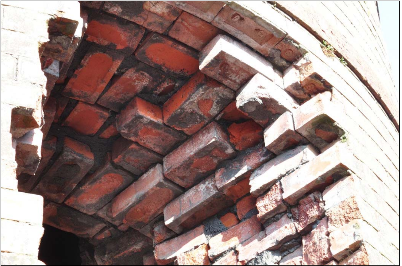
Photo 8: Detail of chimney construction, looking up into modern opening
