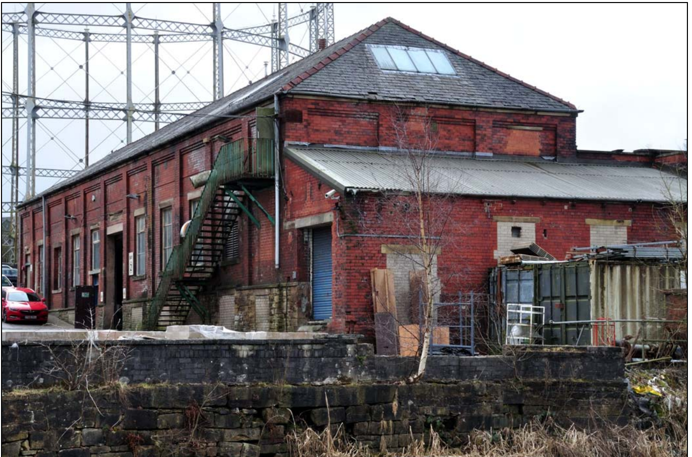
Photo 19: Detached weaving shed: warehouse, from the north
