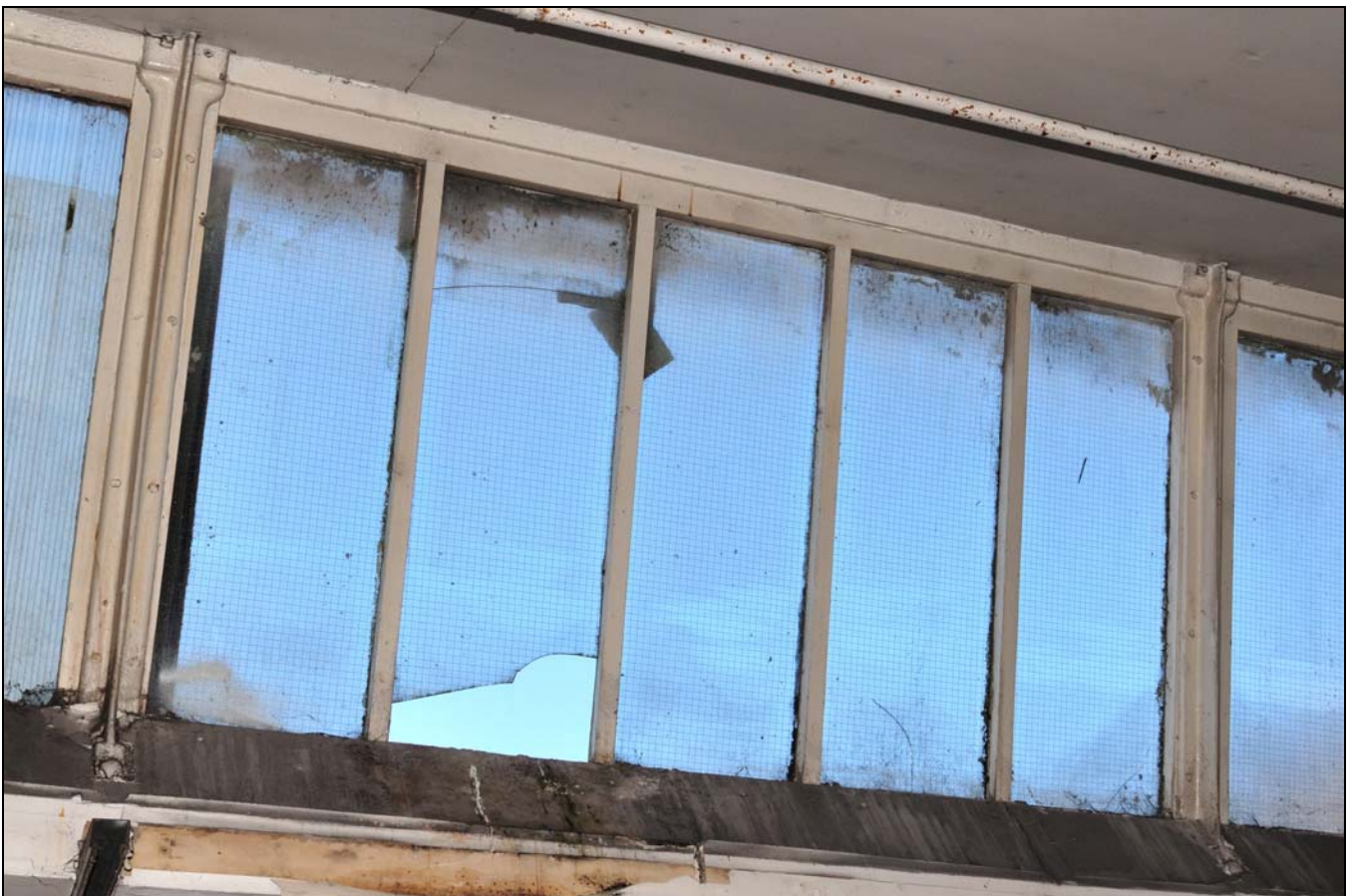
Photo 52: Detached weaving shed: detail of roof light
