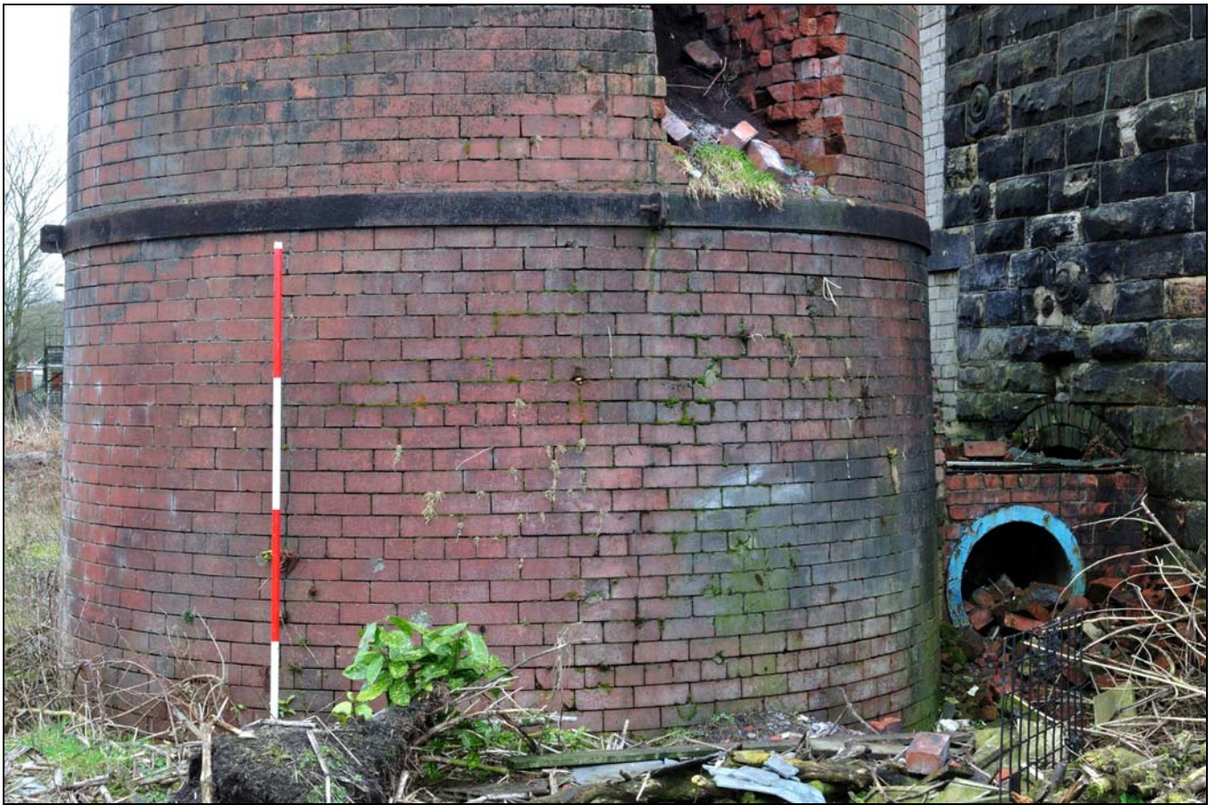
Photo 12: Base of chimney with flue from boiler house, from the west
