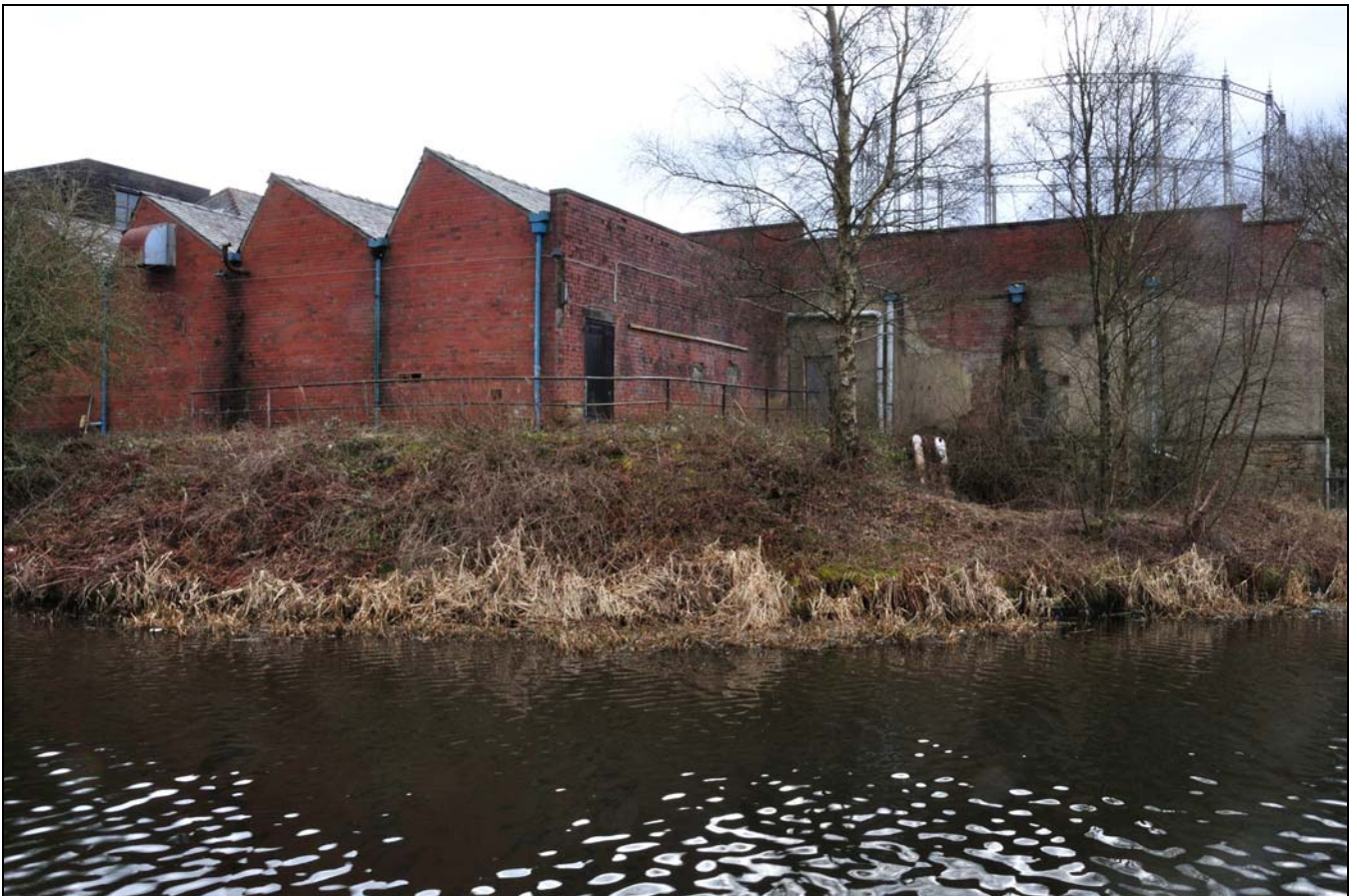
Photo 56: Detached weaving shed: north-west extension (1905-1910), looking south-east
