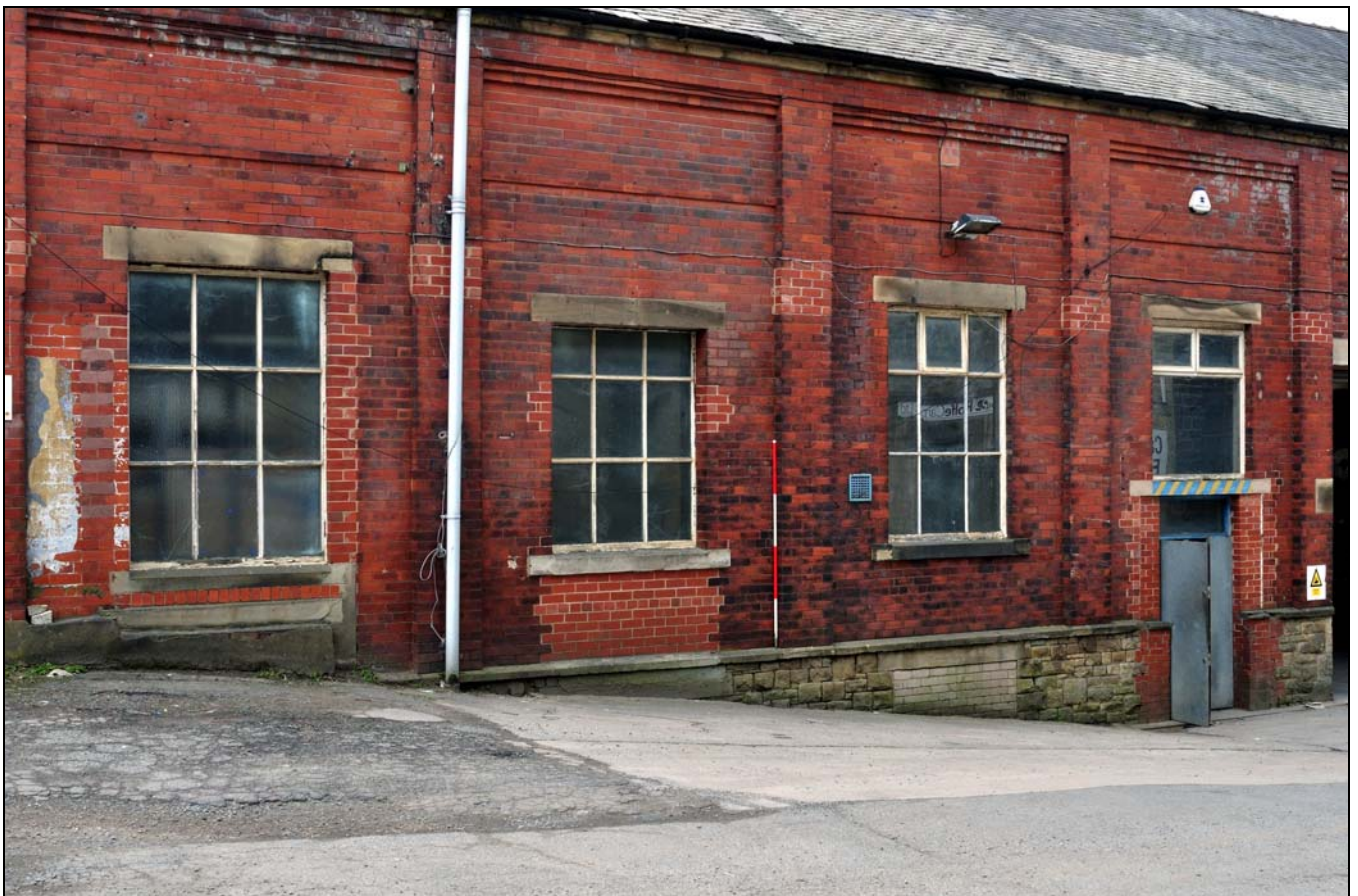
Photo 28: Detached weaving shed: north-east front of warehouse, upper end
