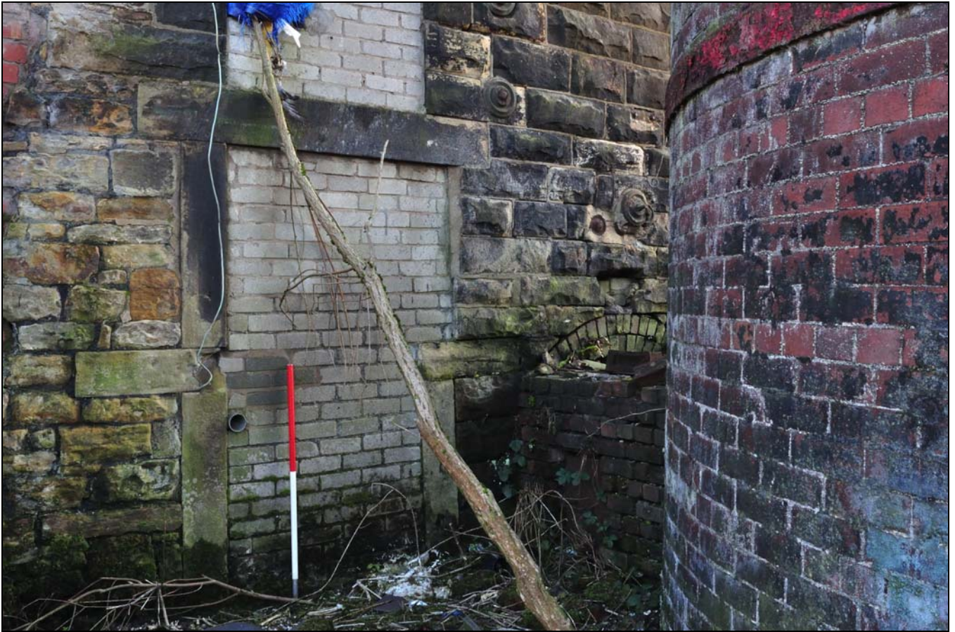
Photo 16: Flue and blocked doorway to boiler house, from the north-east
