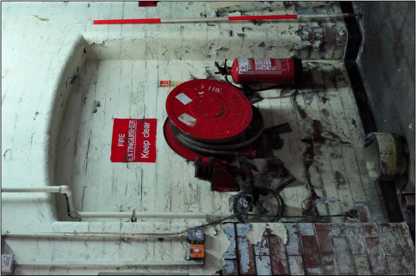
Photo 53: Detached weaving shed: arched recess in north-east side
