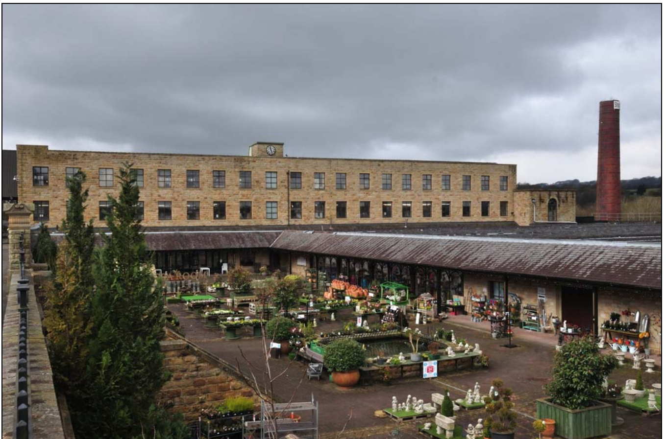
Photo 6: 1891 warehouse and weaving shed, with chimney beyond, from the east
