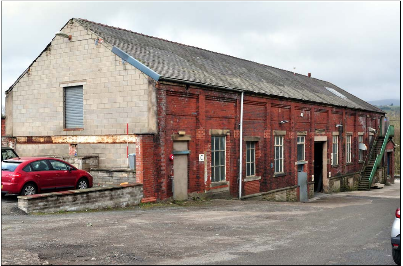
Photo 23: Detached weaving shed: warehouse, from the south-east (end rebuilt)
