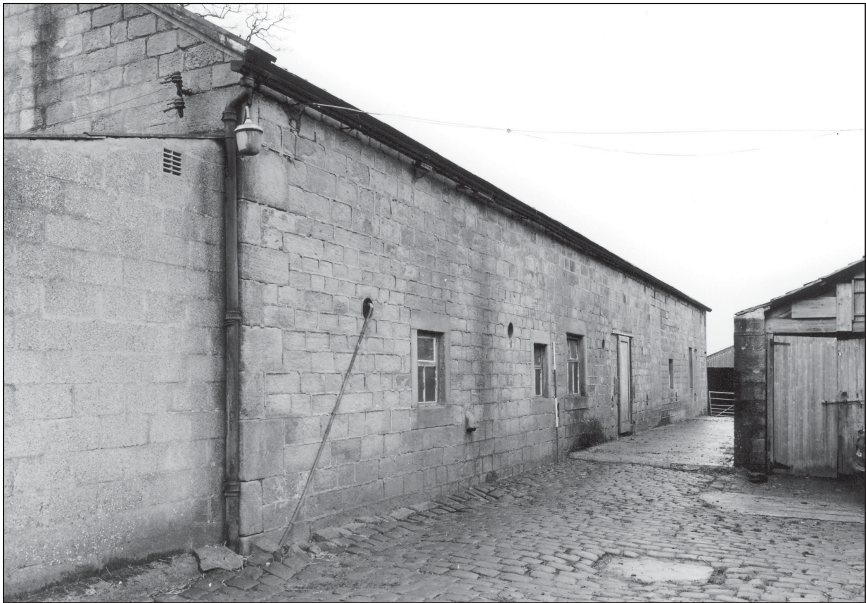
Photo 6: North side of building 1 (barn), from the north-west
