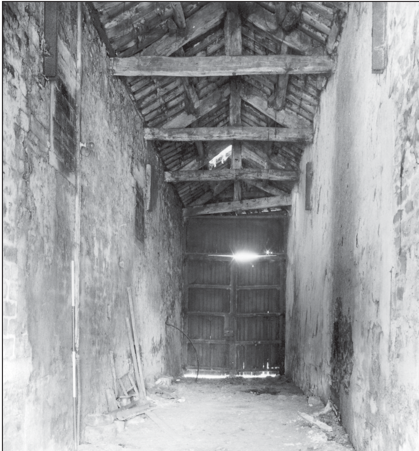
Photo 14: Interior of building 2 (cart-shed), from the west
