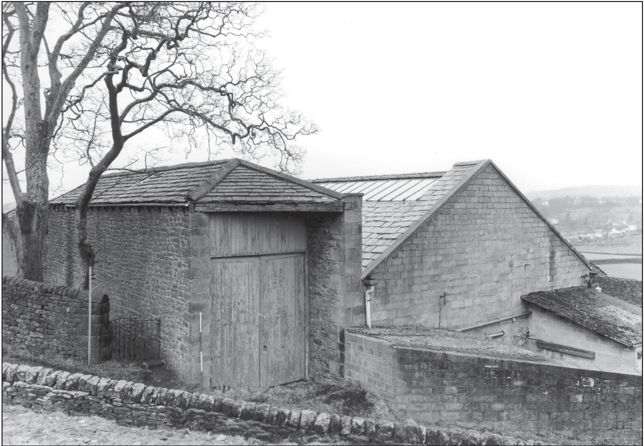
Photo 20: Buildings 1 & 2 (barn & cart-shed), from the south-east
