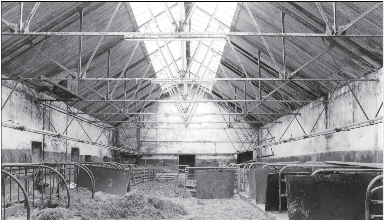
Photo 18: Interior of building 1 (barn), from the west
