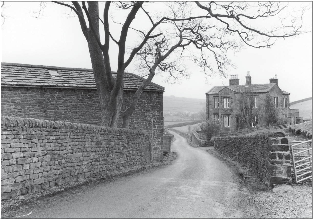
Photo 1: Building 2 (cart-shed) and farmhouse, from the south-west
