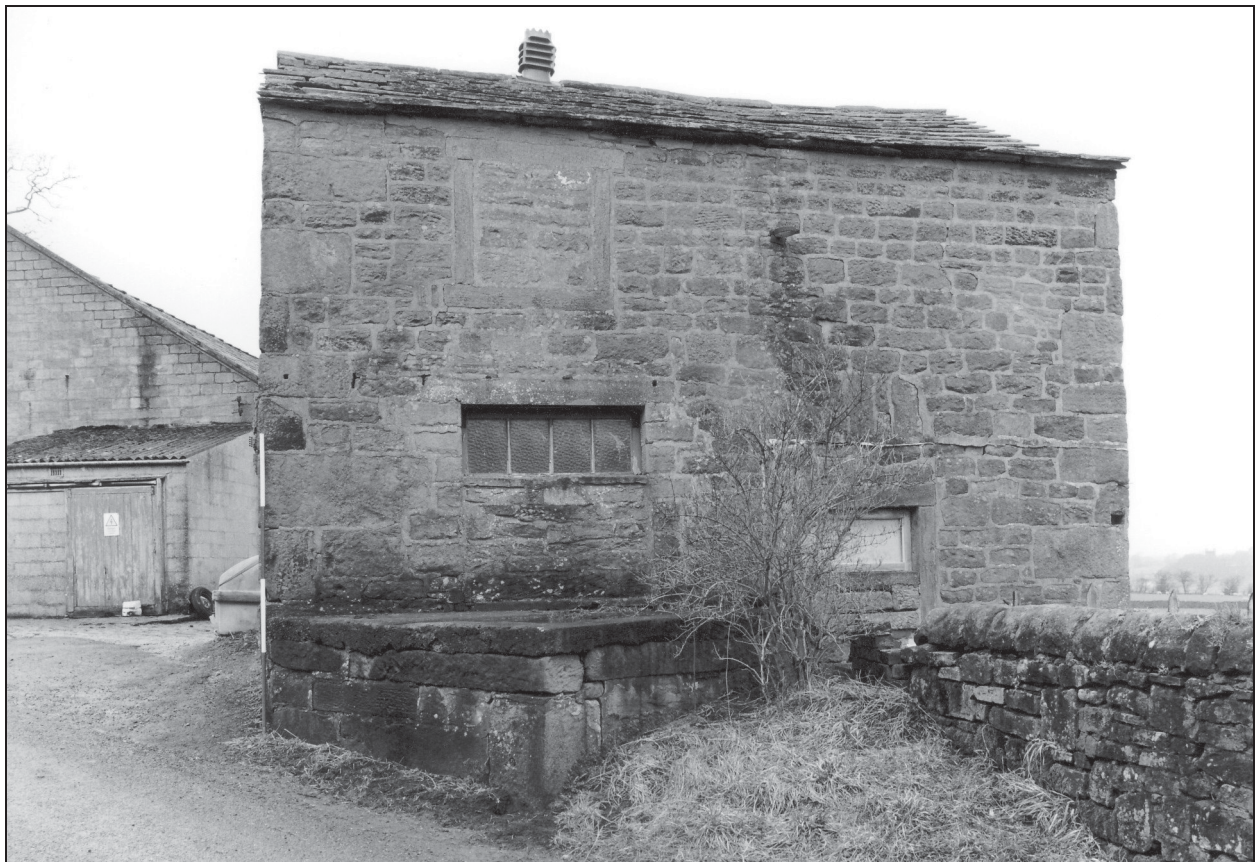
Photo 29: Building 3 (former cottage?) from the east
