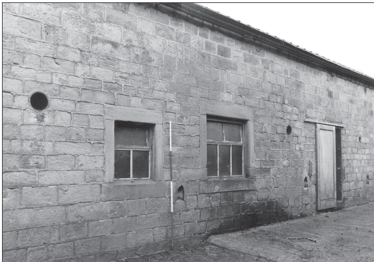
Photo 8: Different window openings in north side of building 1 (barn), from the north-west
