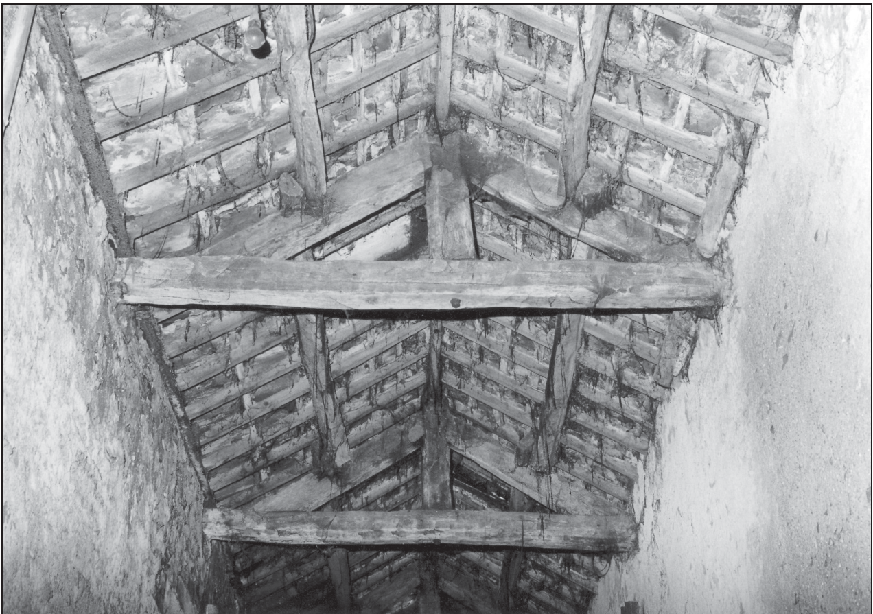
Photo 23: Detail of roof structure of building 2 (cart-shed), from the west
