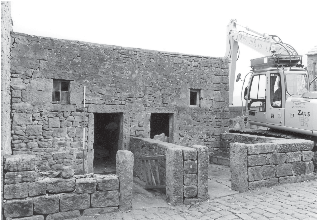
Photo 33: Building 4 (pig sties), from the south-west
