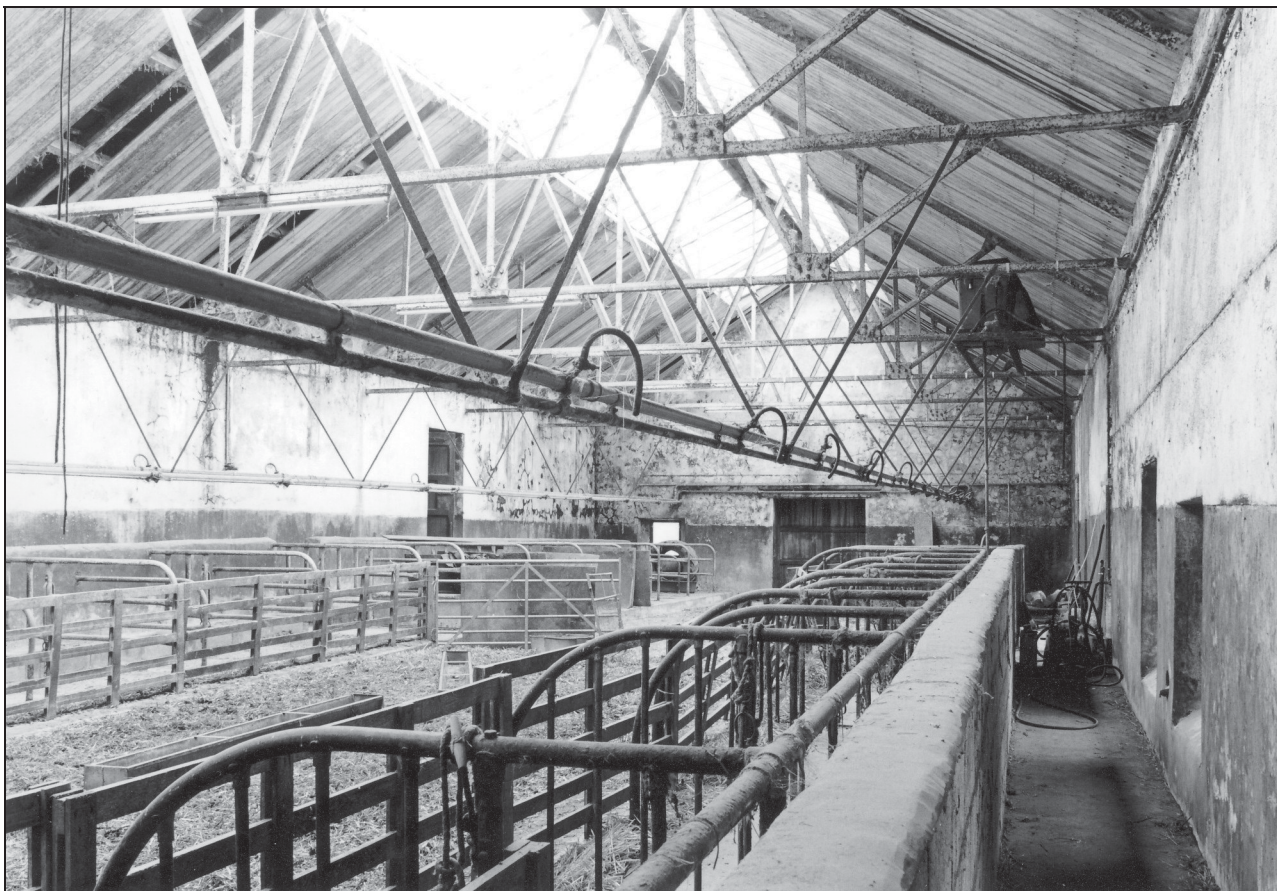
Photo 16: Interior of building 1 (barn), from the north-east
