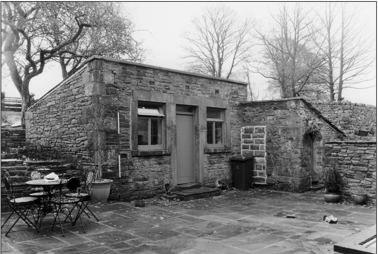
Photo 43: Former wash-house, from the west
