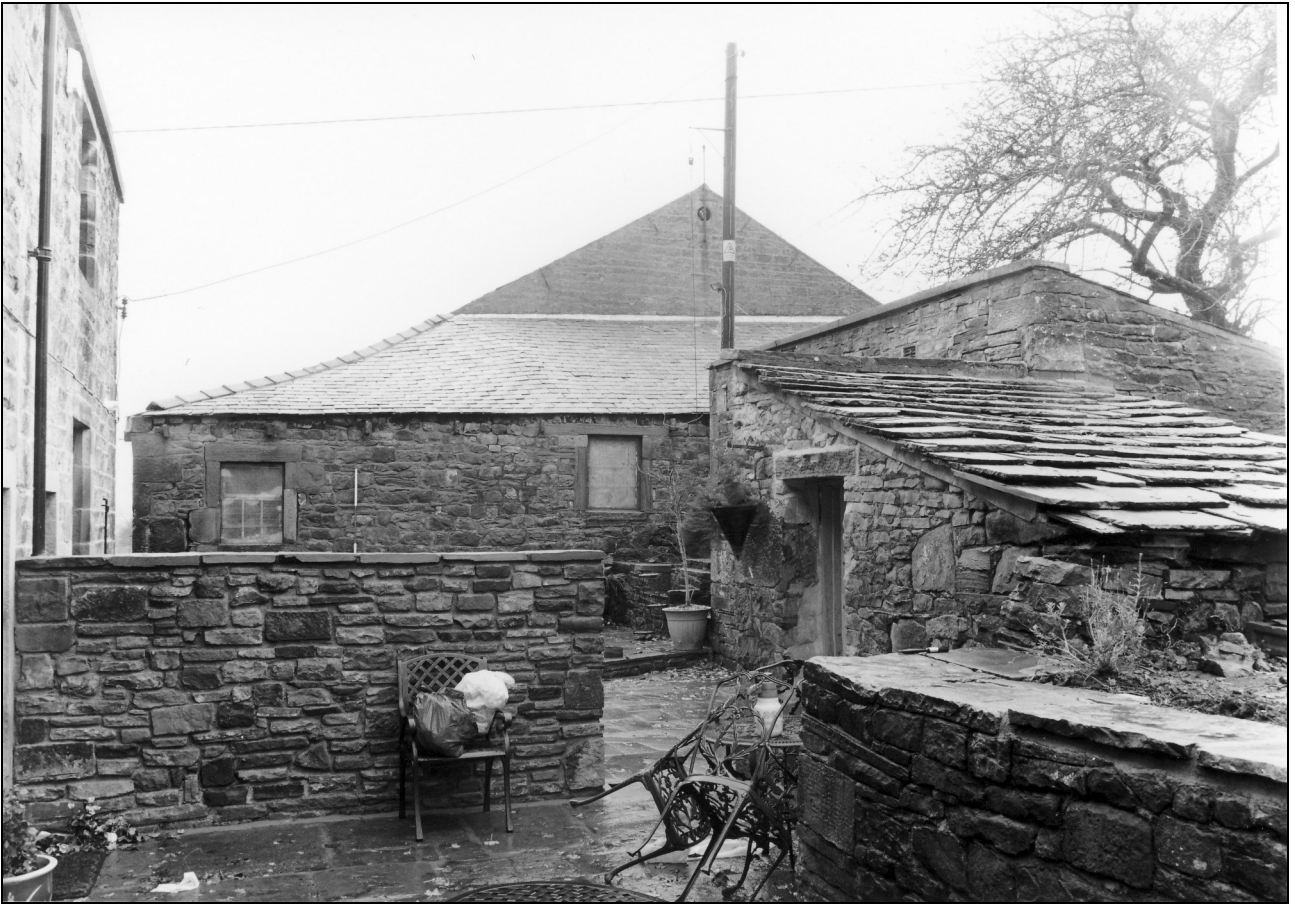
Photo 13: View of the barn and former wash-house, from the south-east
