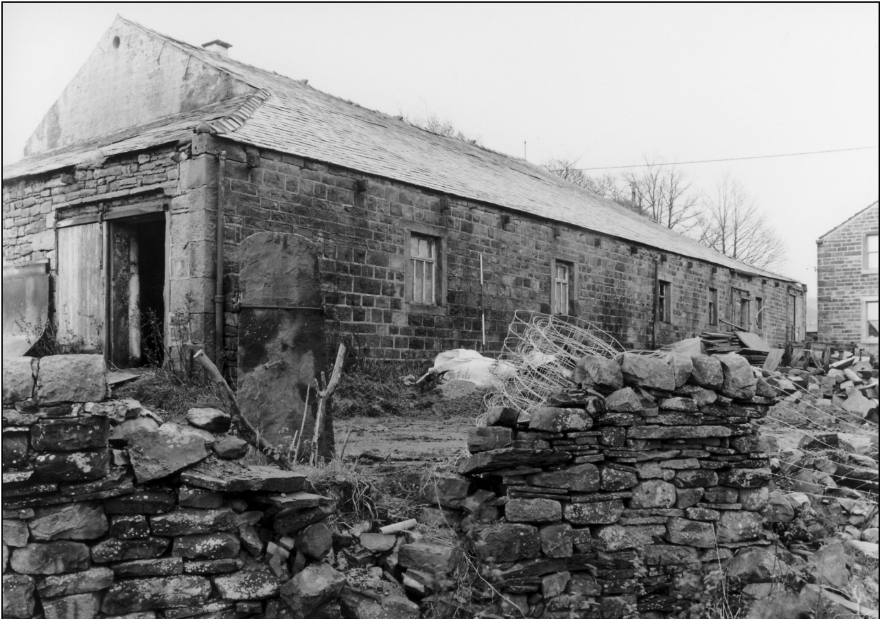
Photo 7: View of the barn, from the west
