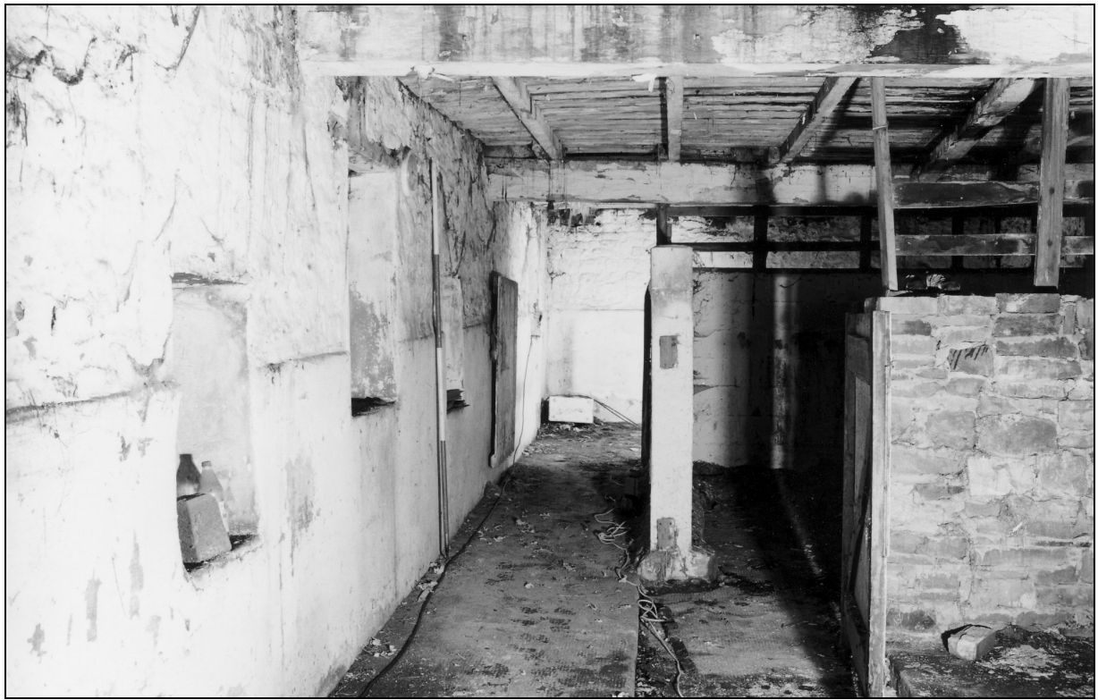
Photo 26: Interior of shippon, at north-west end of barn
