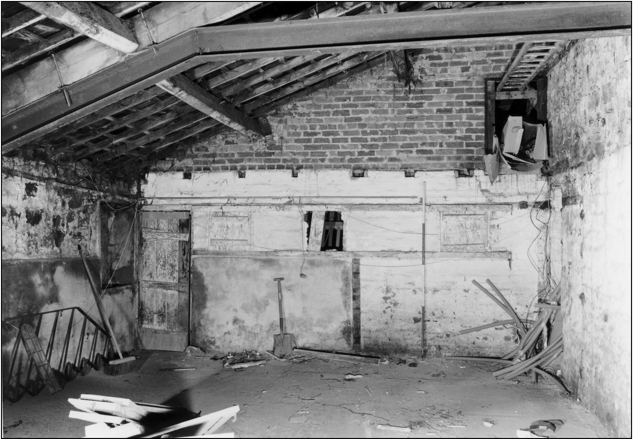
Photo 34: Interior of south-east end of barn (former shippon or stable)
