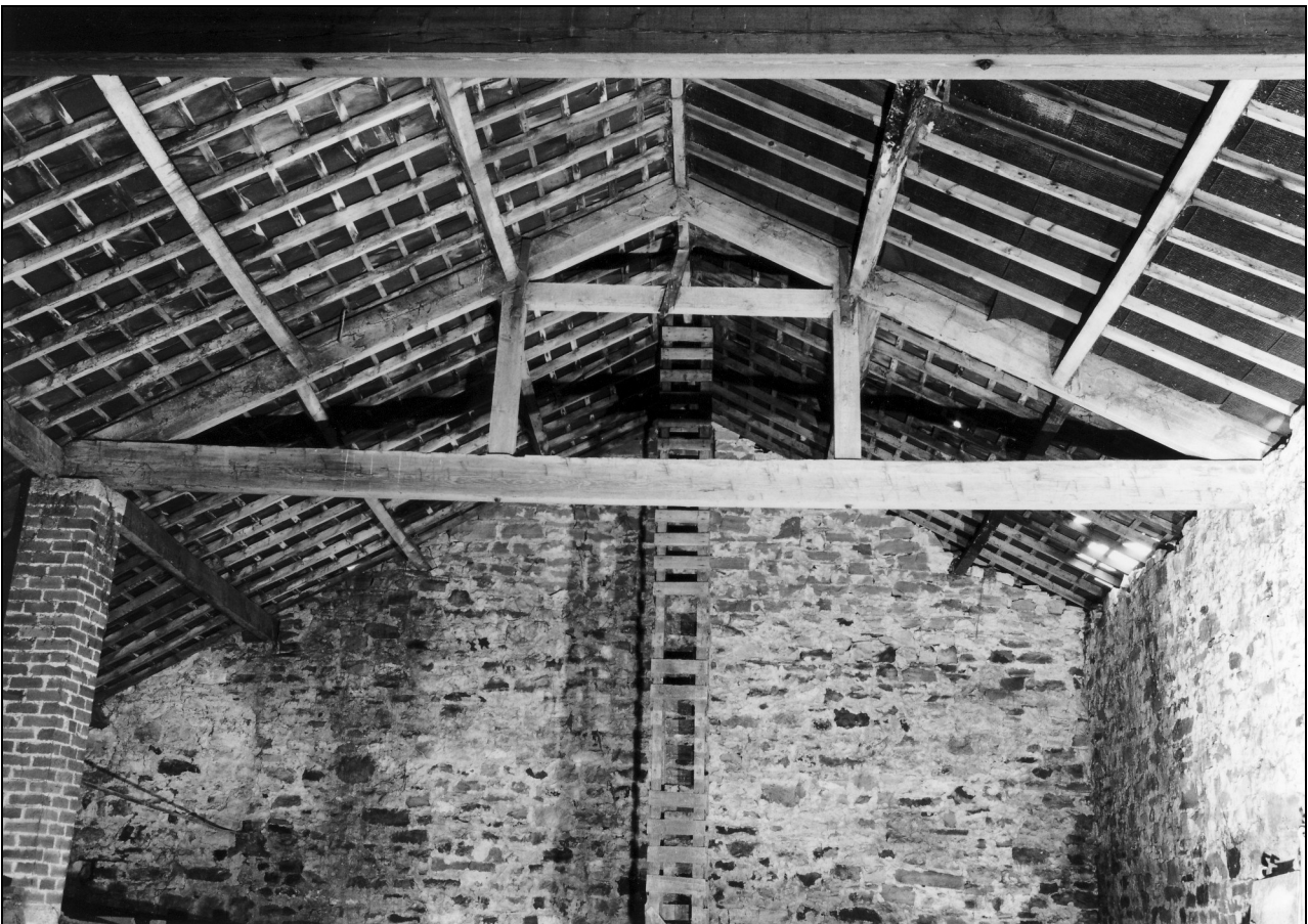
Photo 21: Roof structure over barn, from the south-east
