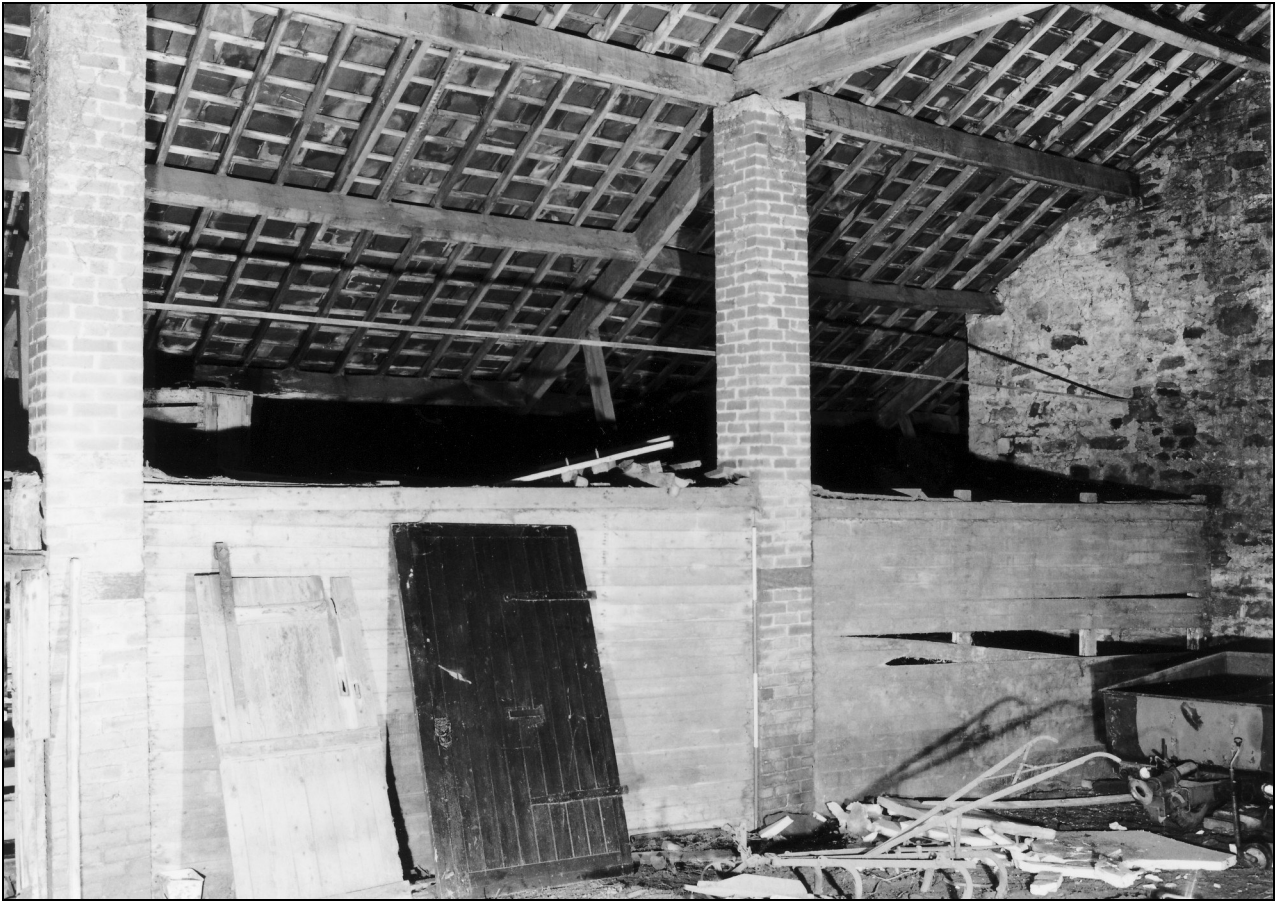
Photo 20: Interior of barn from the east, showing partition to shippon
