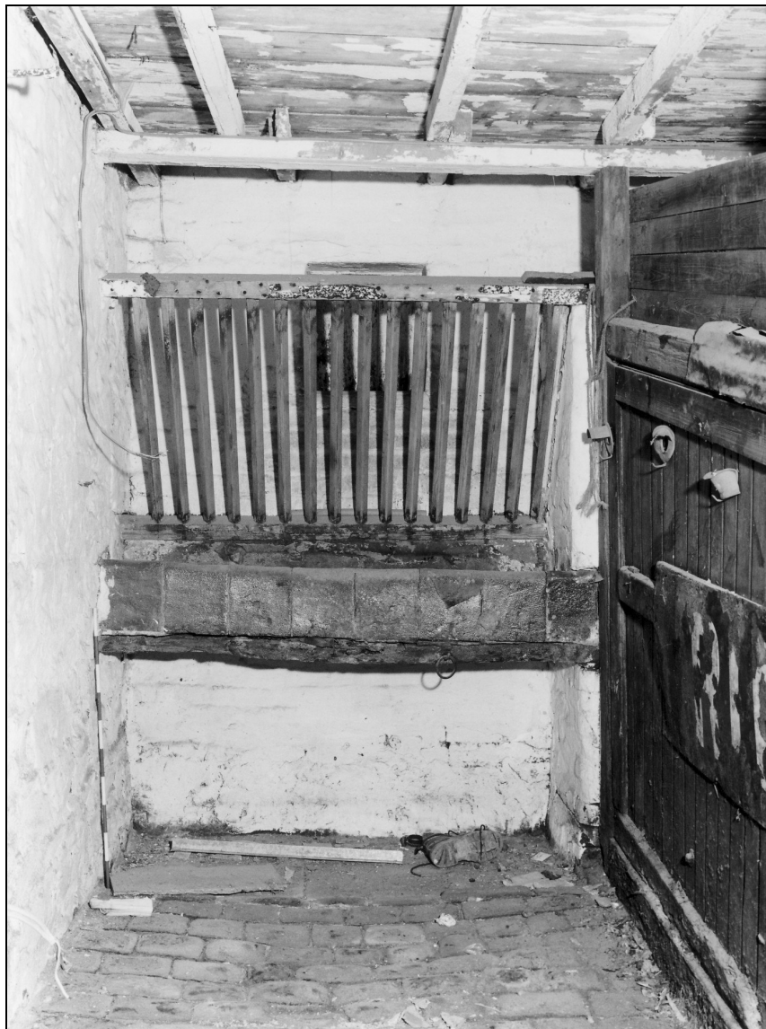
Photo 32: Stall with hay rack and manger in stable, south-east end of barn
