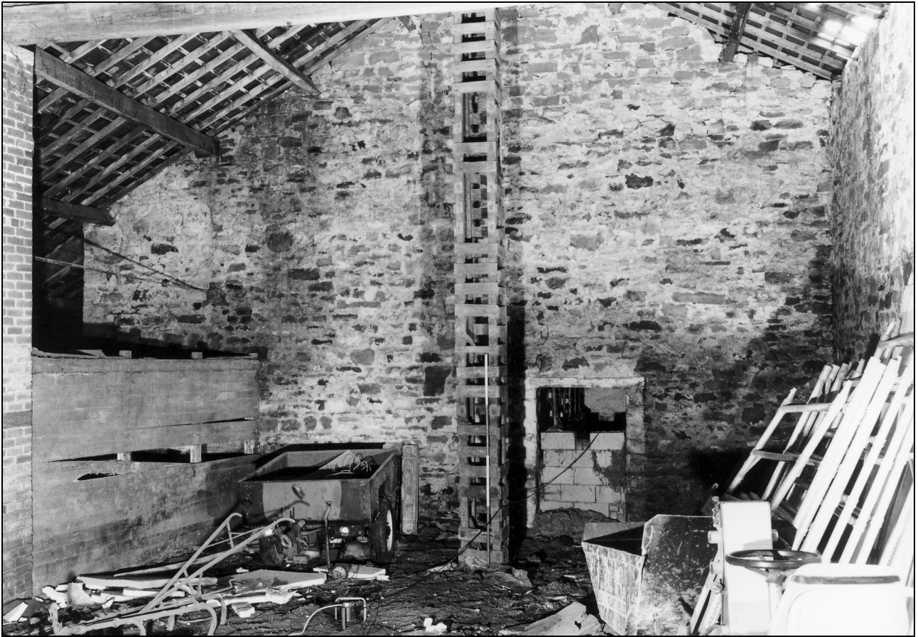
Photo 17: Interior of barn mewstead, from the south-east, showing ventilator
