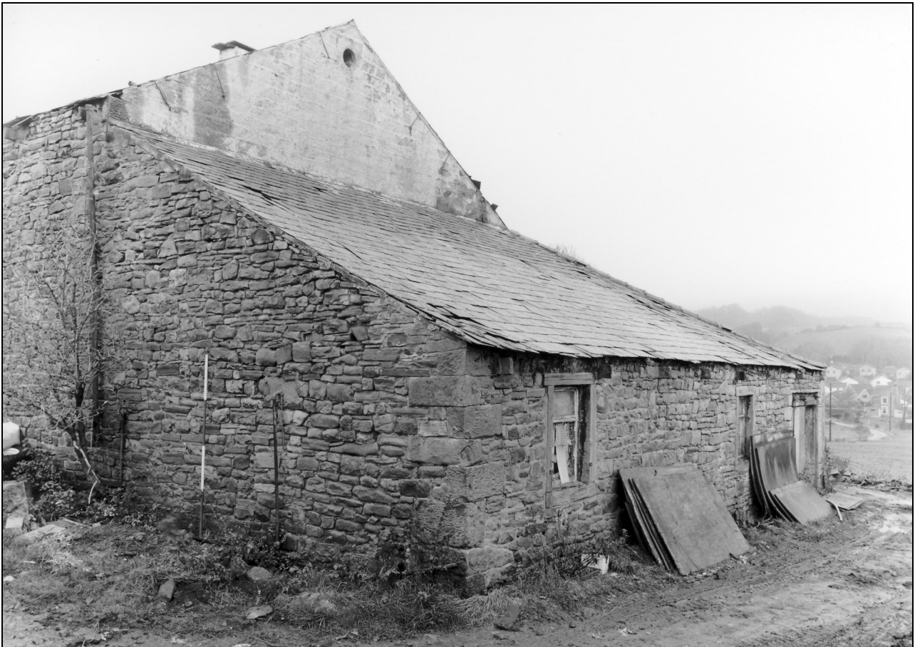
Photo 3: Exterior of shippon at north-west end of barn, from the north
