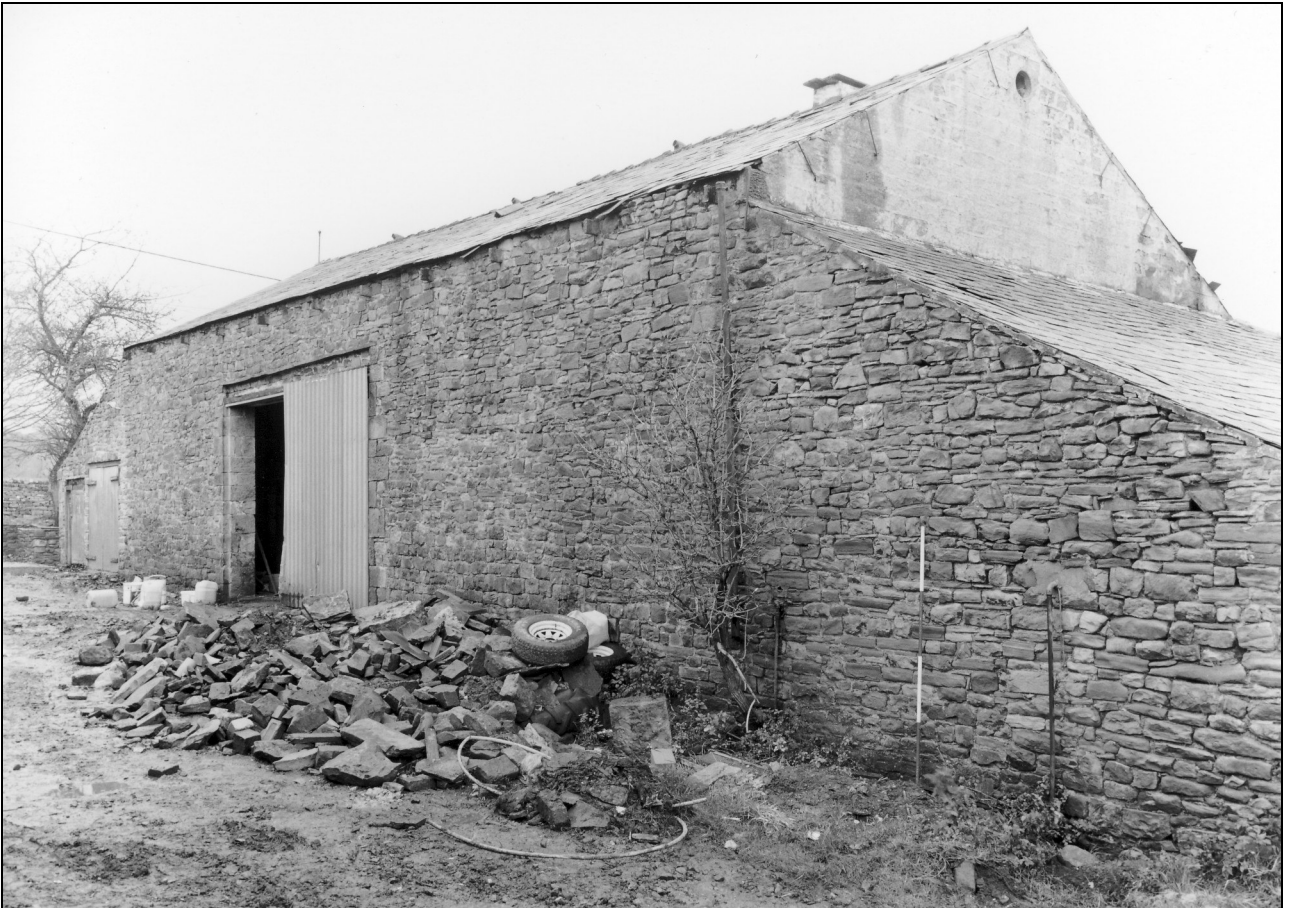
Photo 4: North-east elevation of barn, from the north
