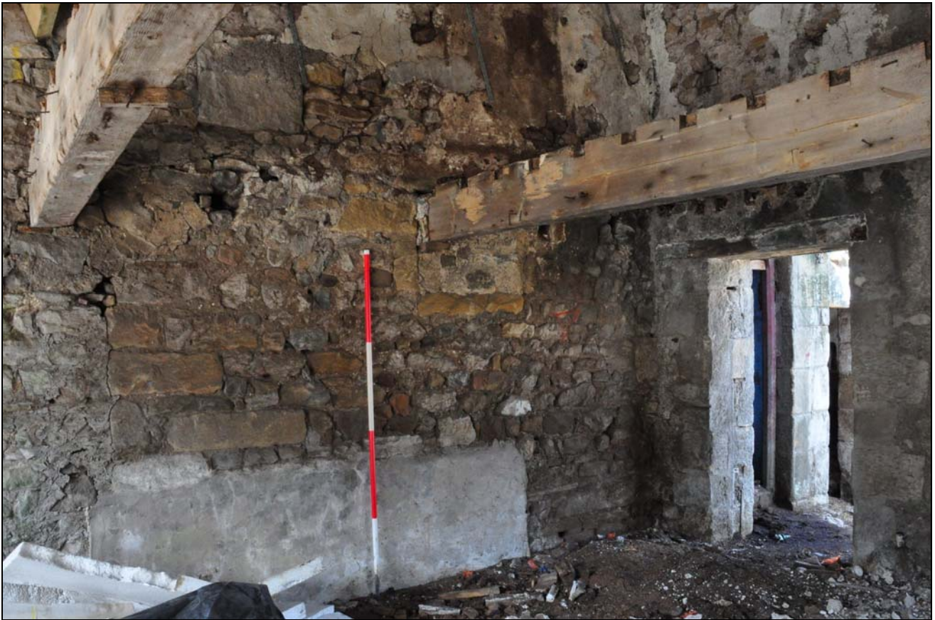
Photo 78: Building 10: interior, looking north
