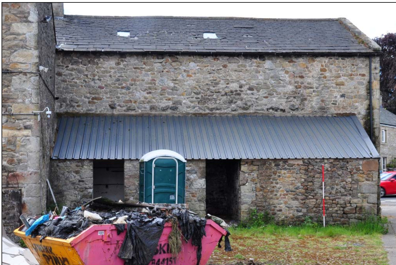
Photo 90: Building 7: rear elevation
