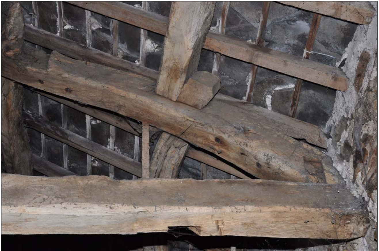
Photo 31: Building 1: detail of truss I at north-west end (with re-used crucks)
