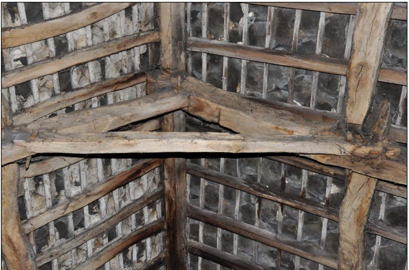
Photo 32: Building 1: detail of truss I at north-west end (with re-used crucks)
