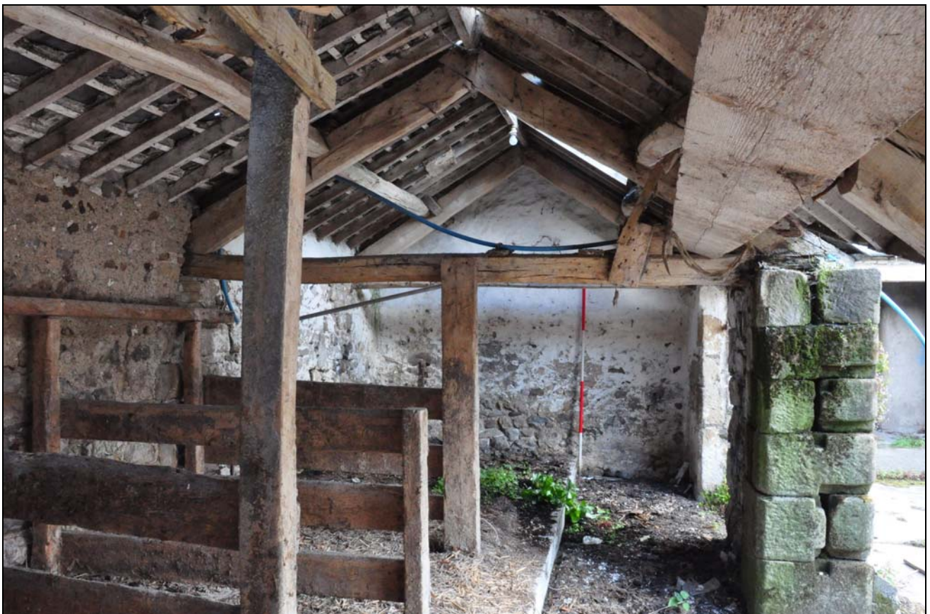
Photo 42: Building 2: interior, looking north-east
