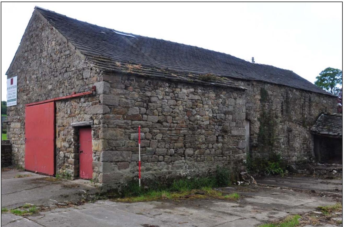
Photo 13: Building 1: general view, looking west
