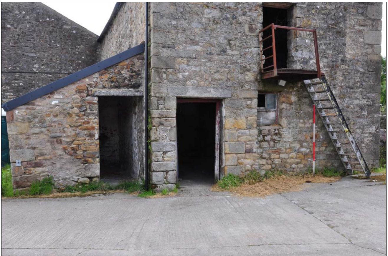
Photo 89: Building 7: stable doorway, west gable
