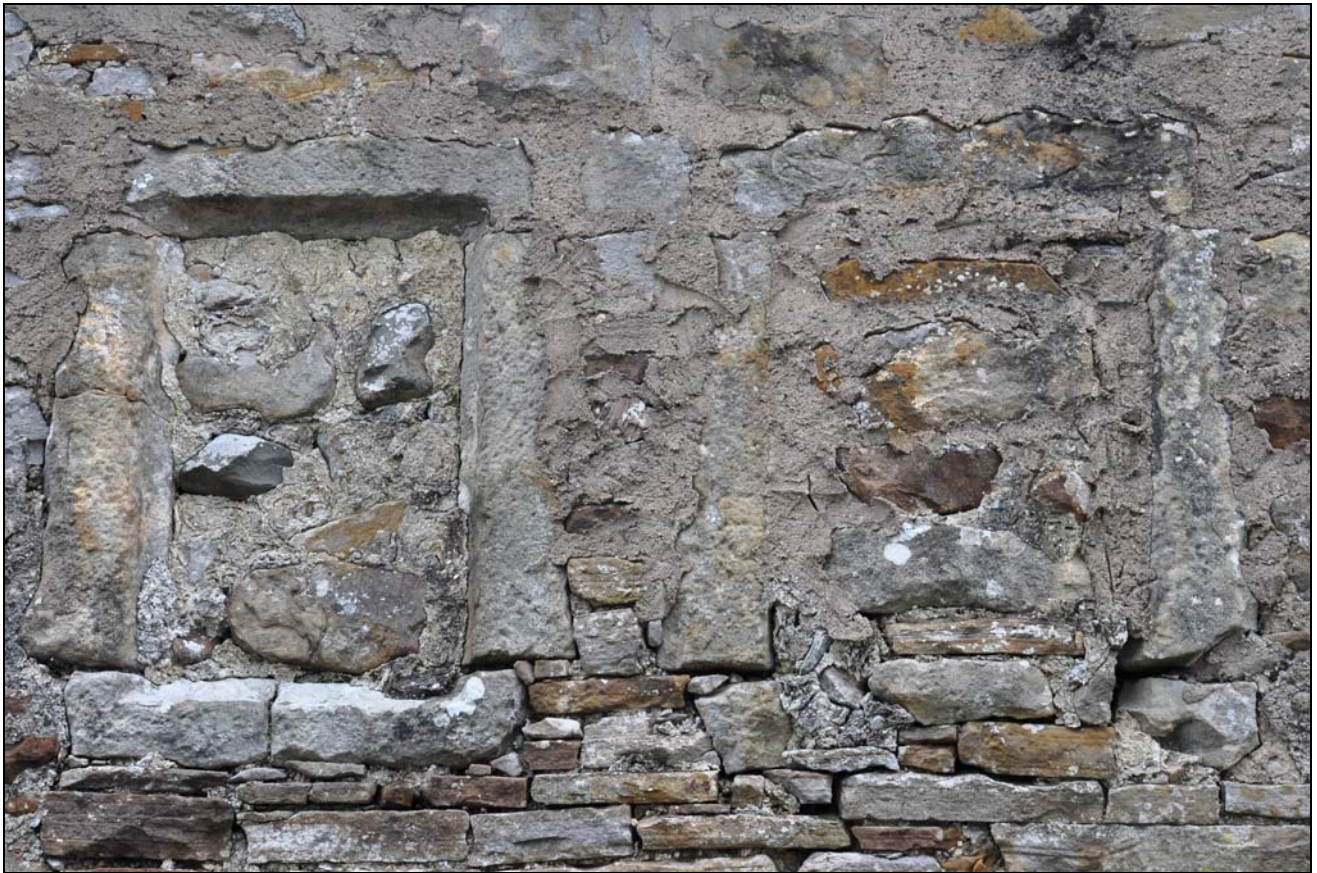
Photo 8: Building 1: detail of re-sited windows in front elevation
