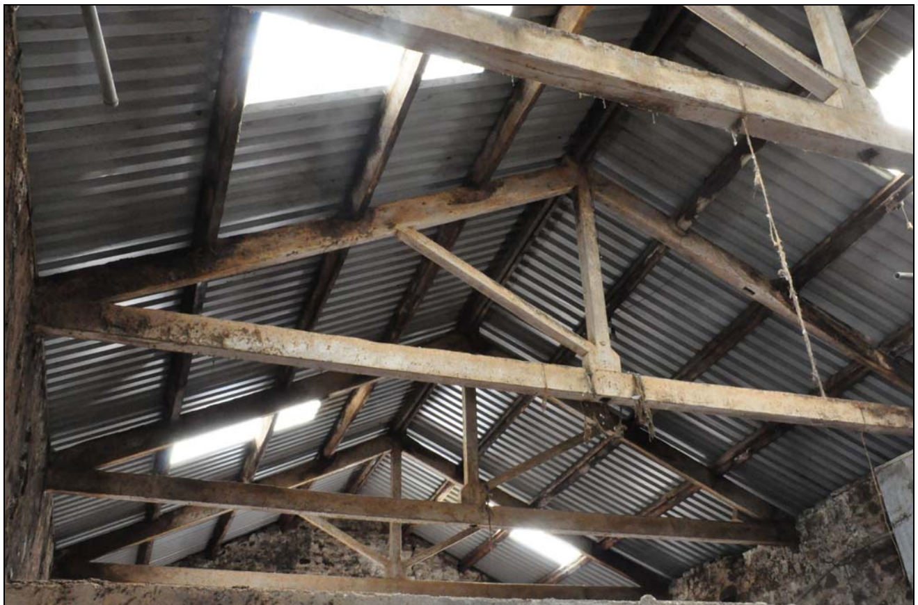
Photo 66: Building 4: roof trusses, looking south-east
