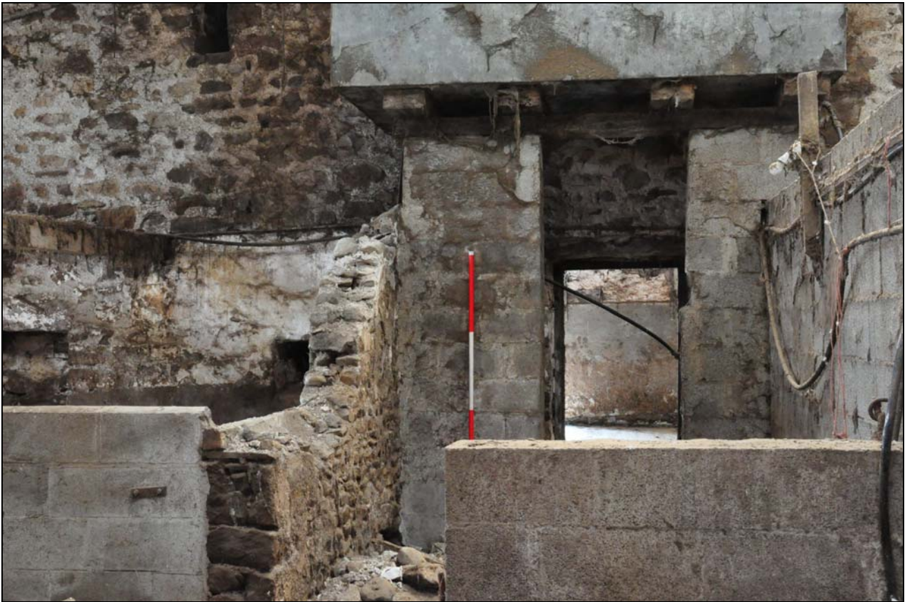
Photo 55: Building 4: threshing bay, looking south-west, with remains of cross-wall at left
