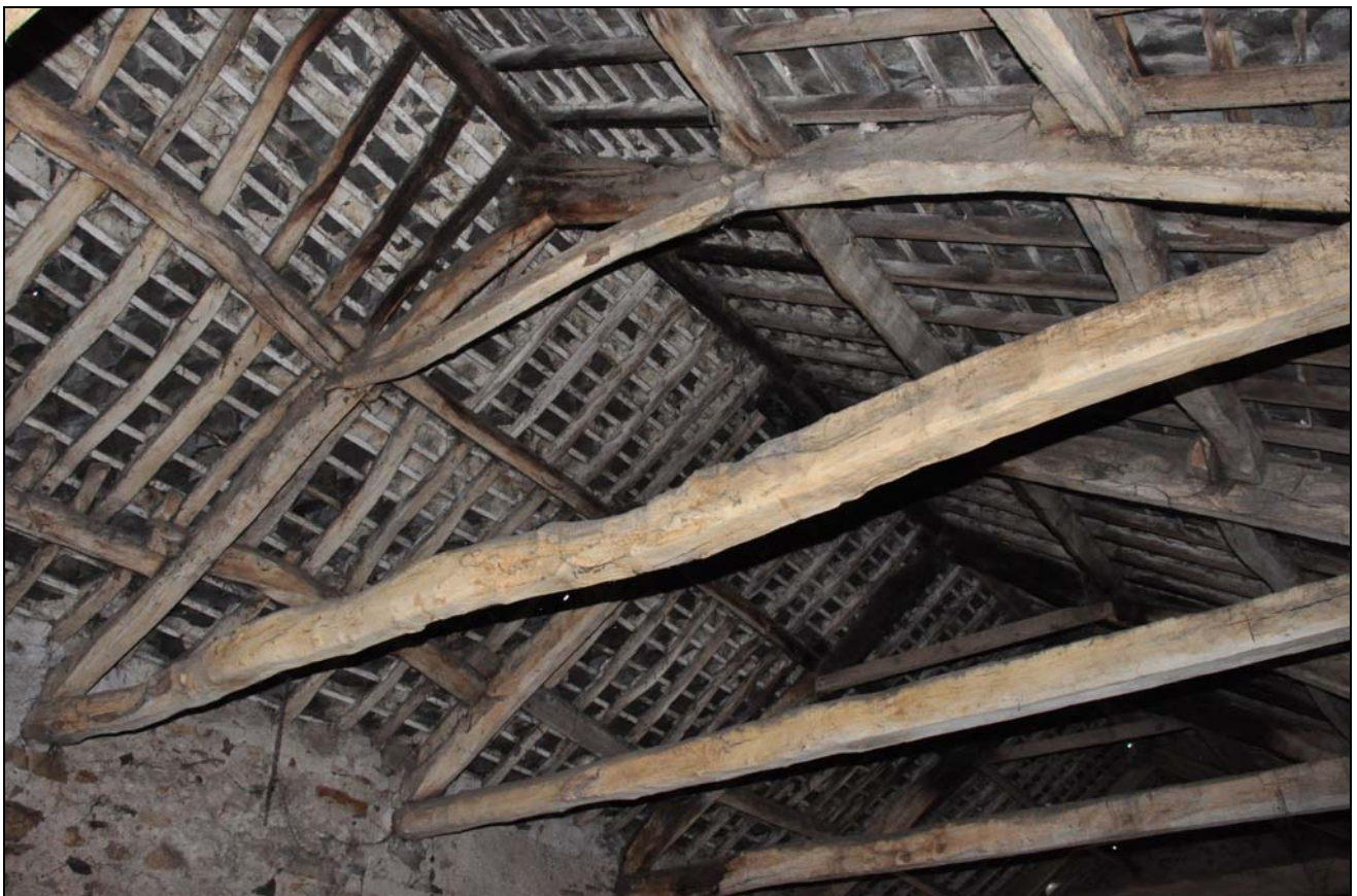
Photo 26: Building 1: roof trusses, looking east
