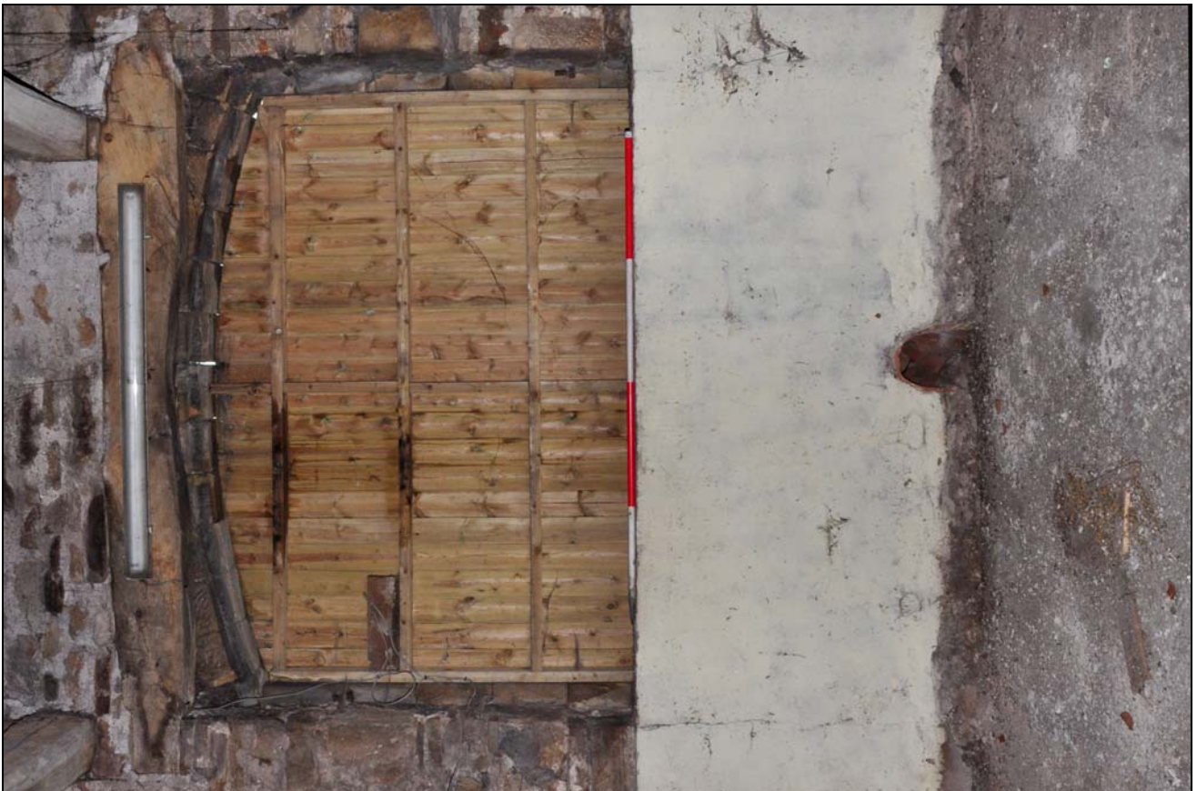
Photo 6: Building 1 : interior view of front cart entrance
