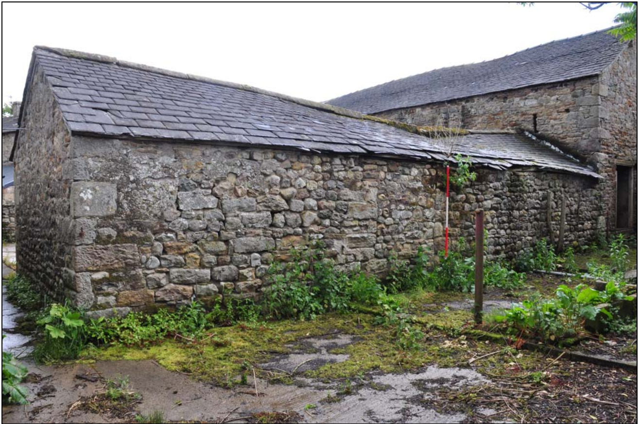
Photo 40: Building 2: rear elevation, looking south
