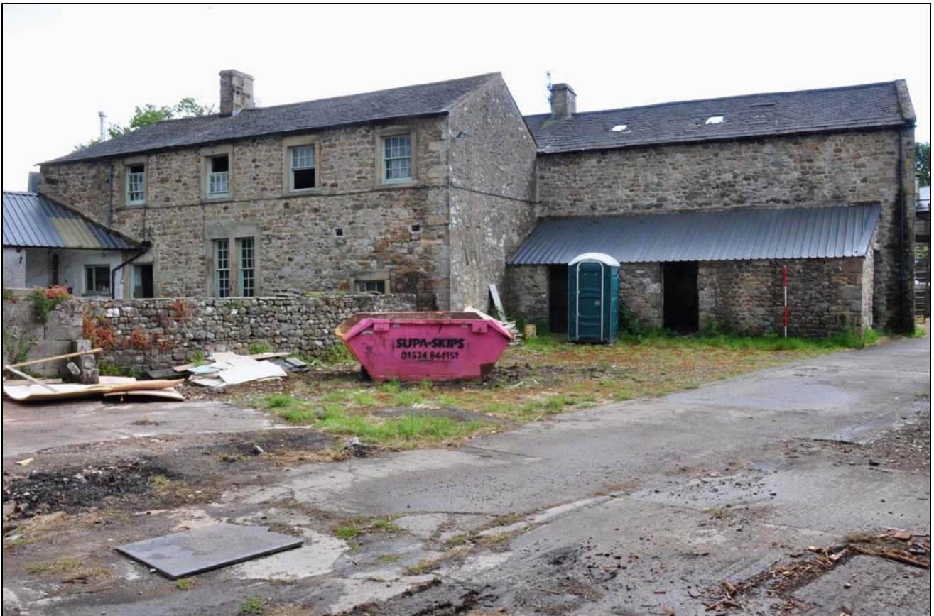
Photo 104: Building 7: rear elevation, with house at left
