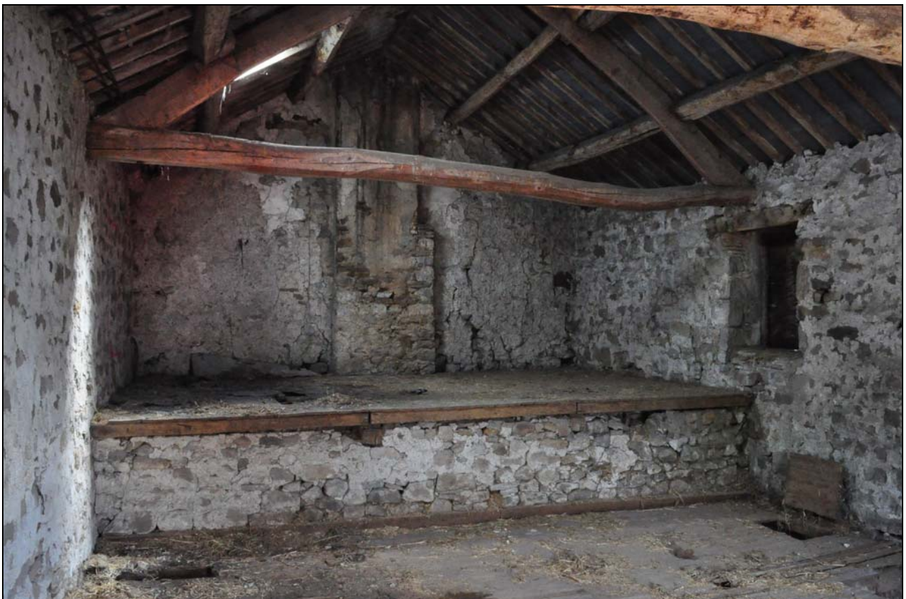
Photo 98: Building 7: hay loft, looking south-east
