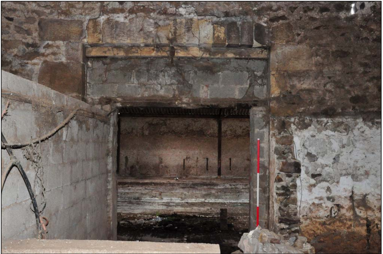
Photo 52: Building 4: internal view of north-east cart entrance
