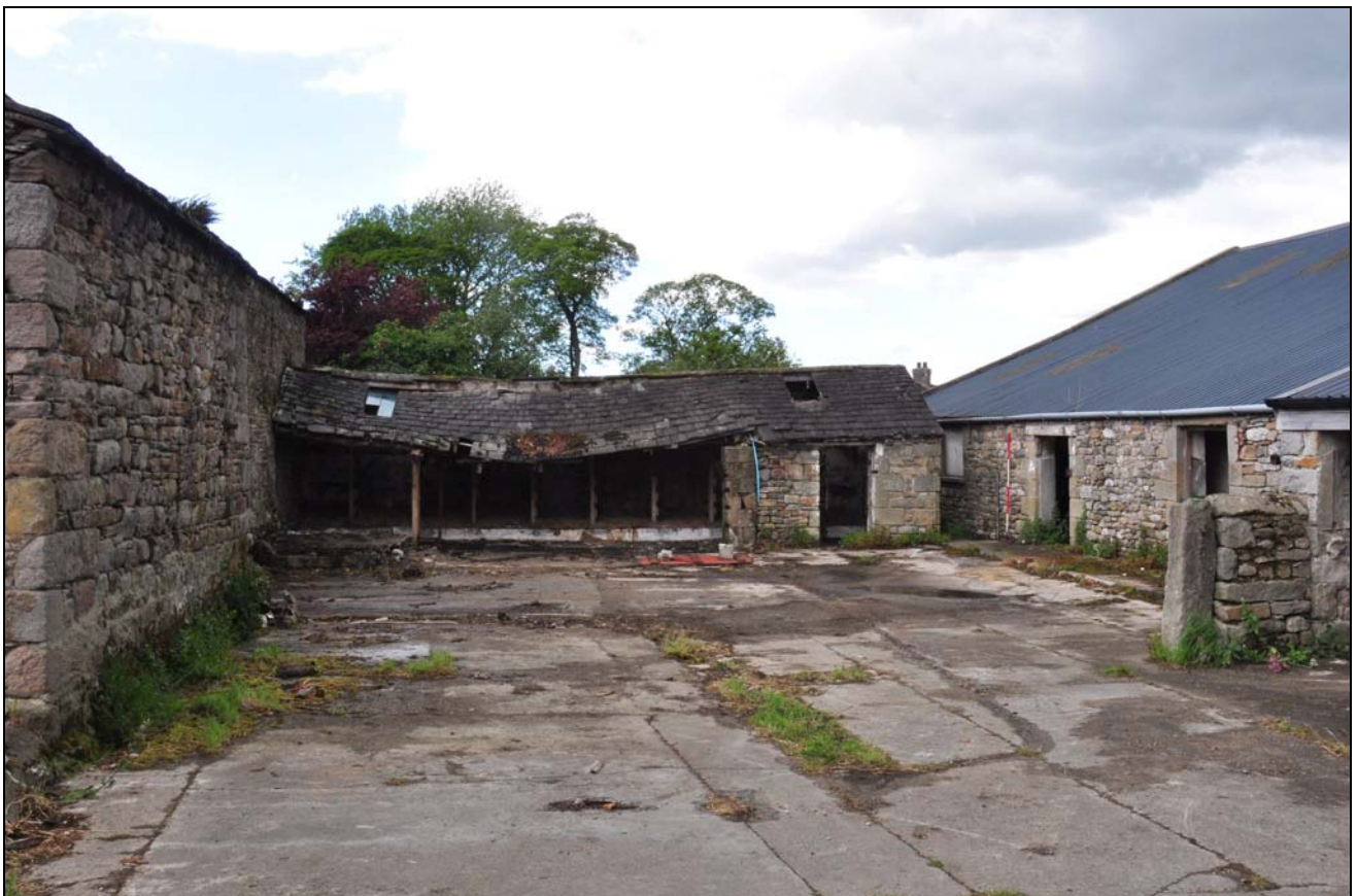
Photo 36: Former fold-yard to rear of Building 1, looking north-west
