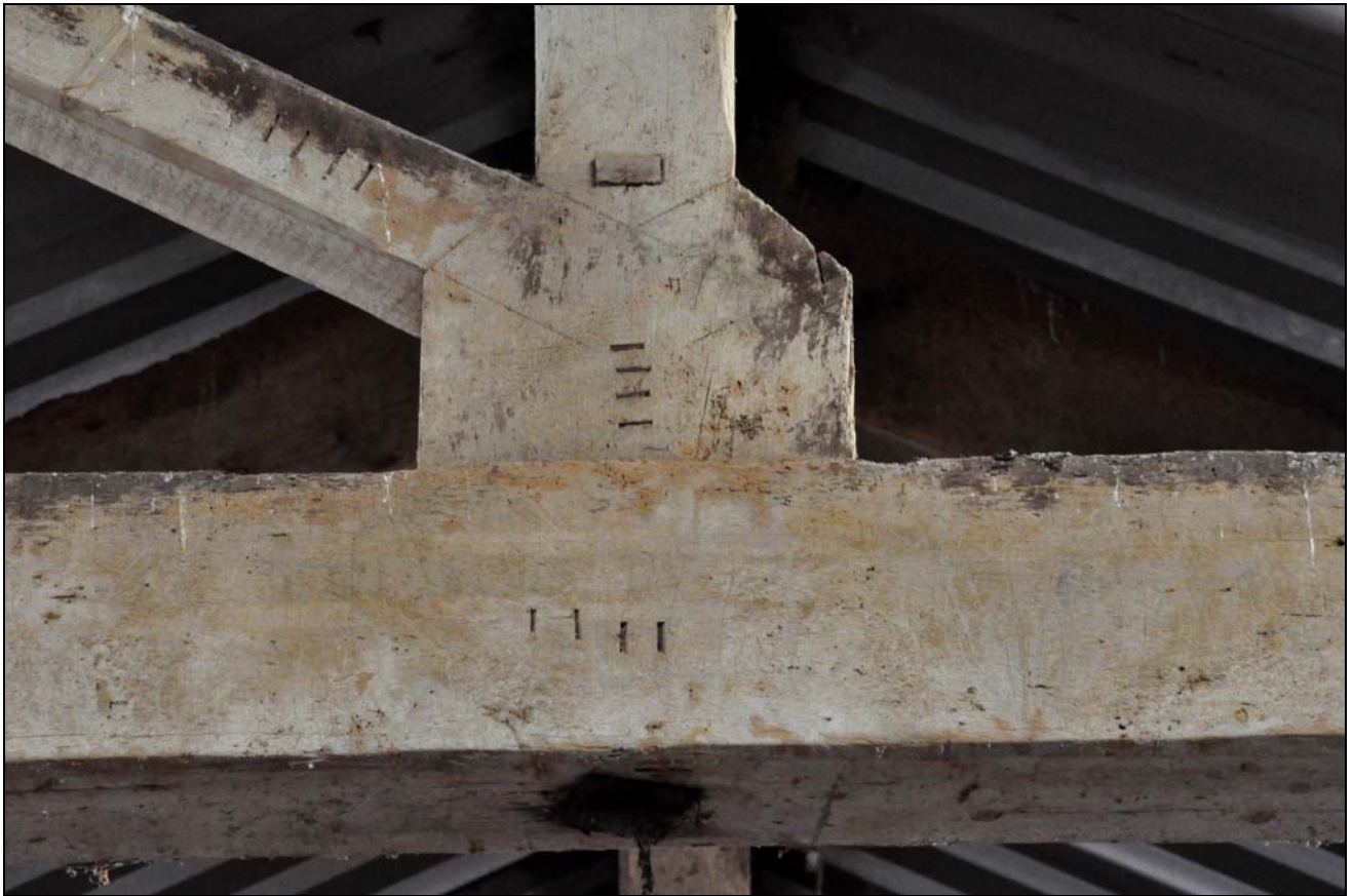
Photo 67: Building 4: detail of numbering on roof truss, looking south-east
