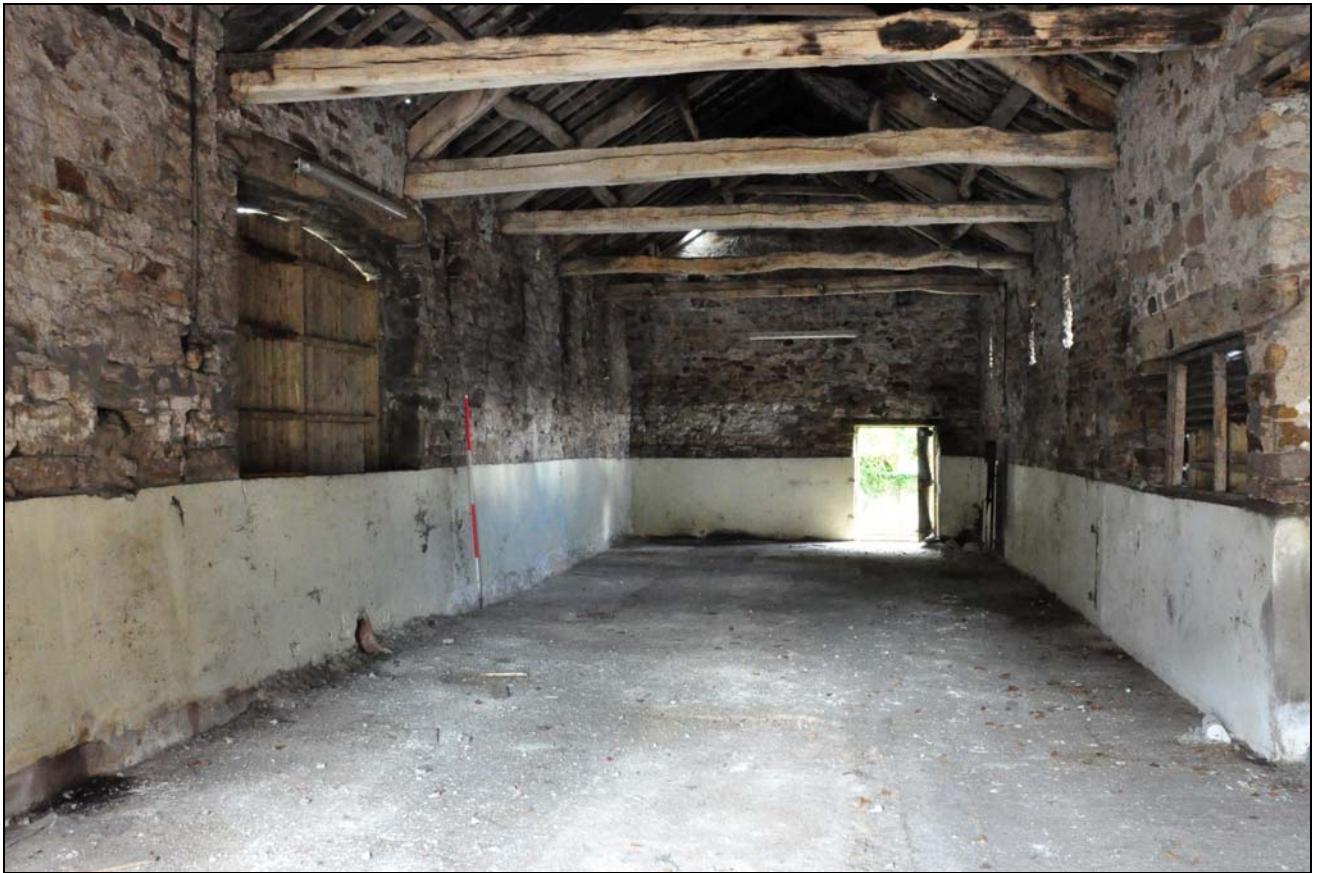
Photo 20: Building 1: interior, looking north-west
