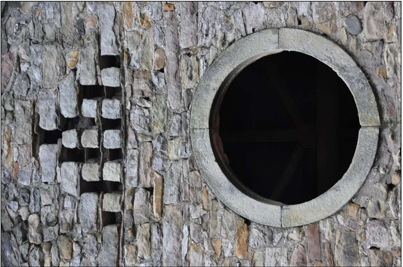
Photo 48: Building 4: detail of forking hole/pitching eye, and nesting boxes, south-east gable
