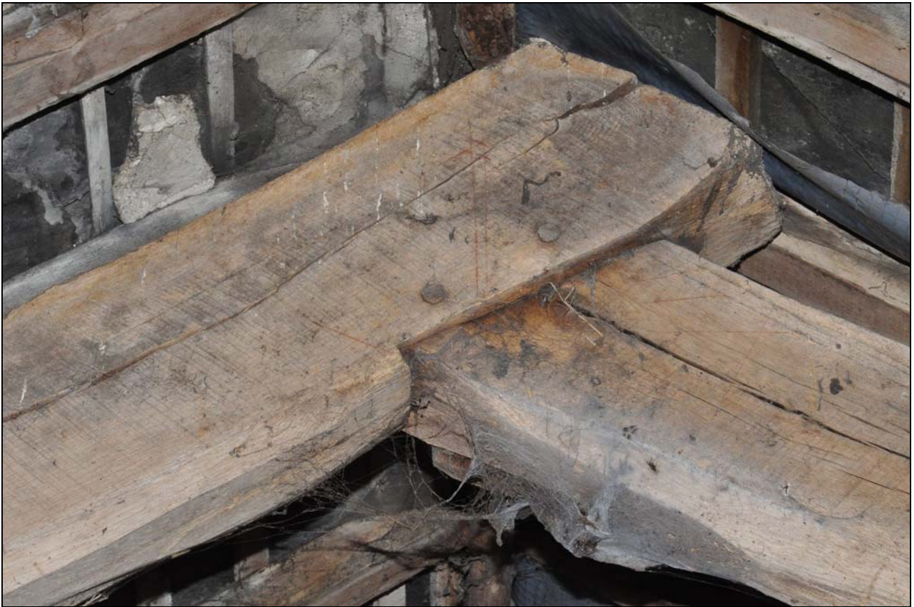
Photo 103: Building 7: detail of ridge to west roof truss, looking east
