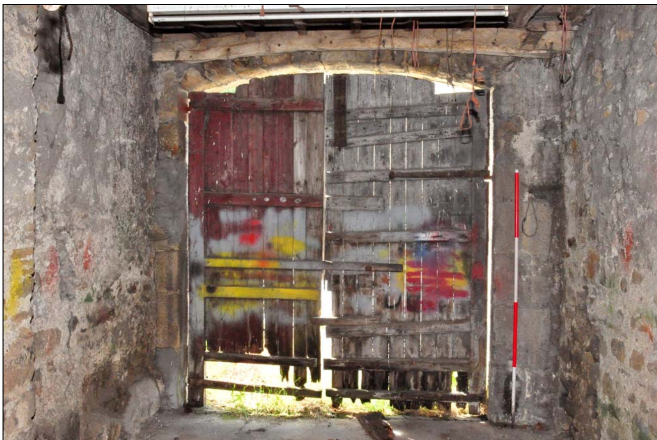
Photo 92: Building 7: trap house, looking south
