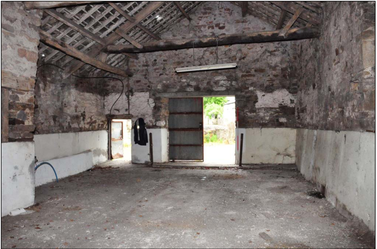
Photo 22: Building 1: interior, looking south-east
