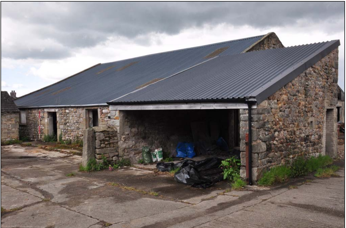
Photo 74: Building 10: general view, looking north
