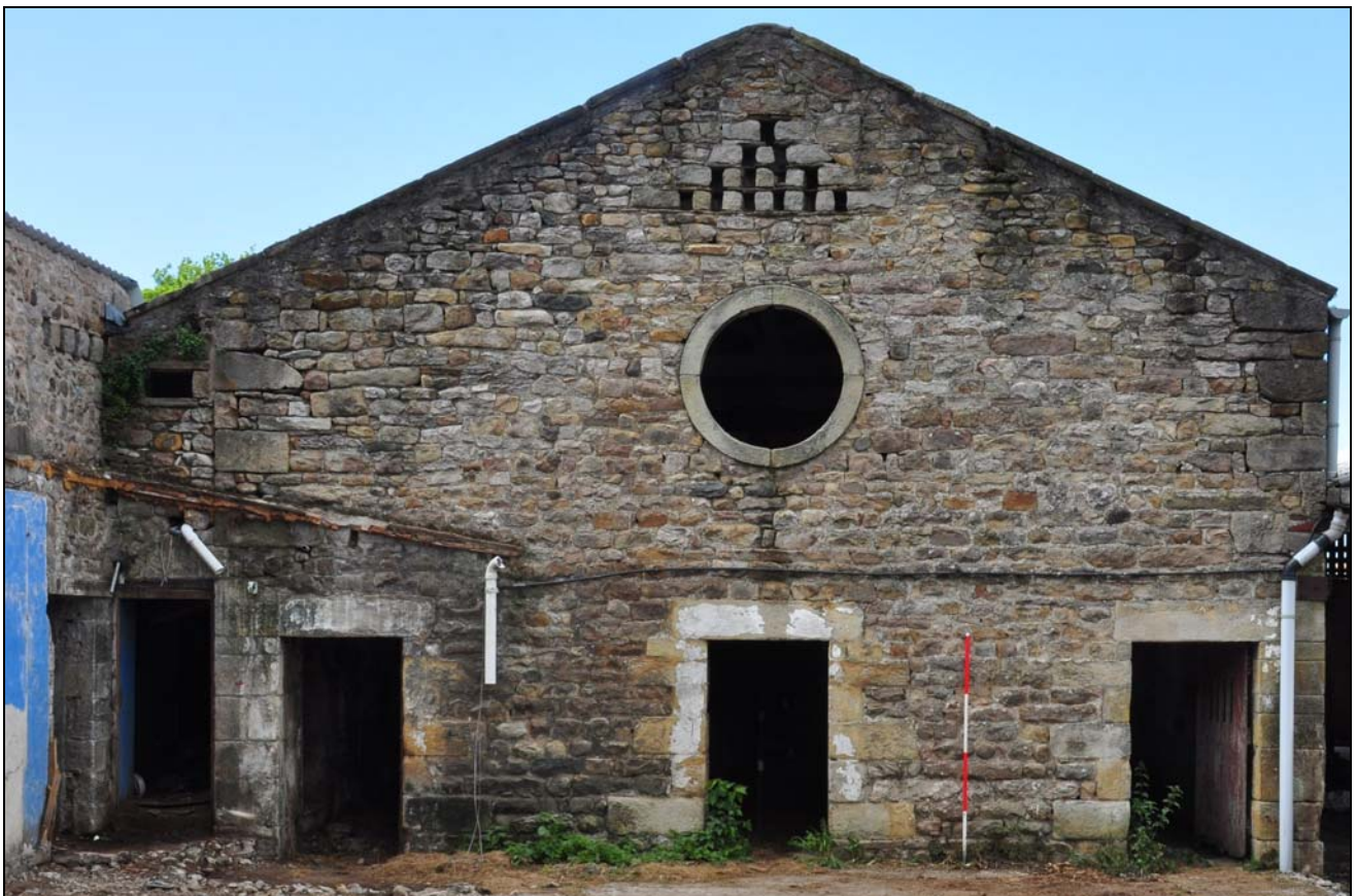
Photo 46: Building 4: south-east gable
