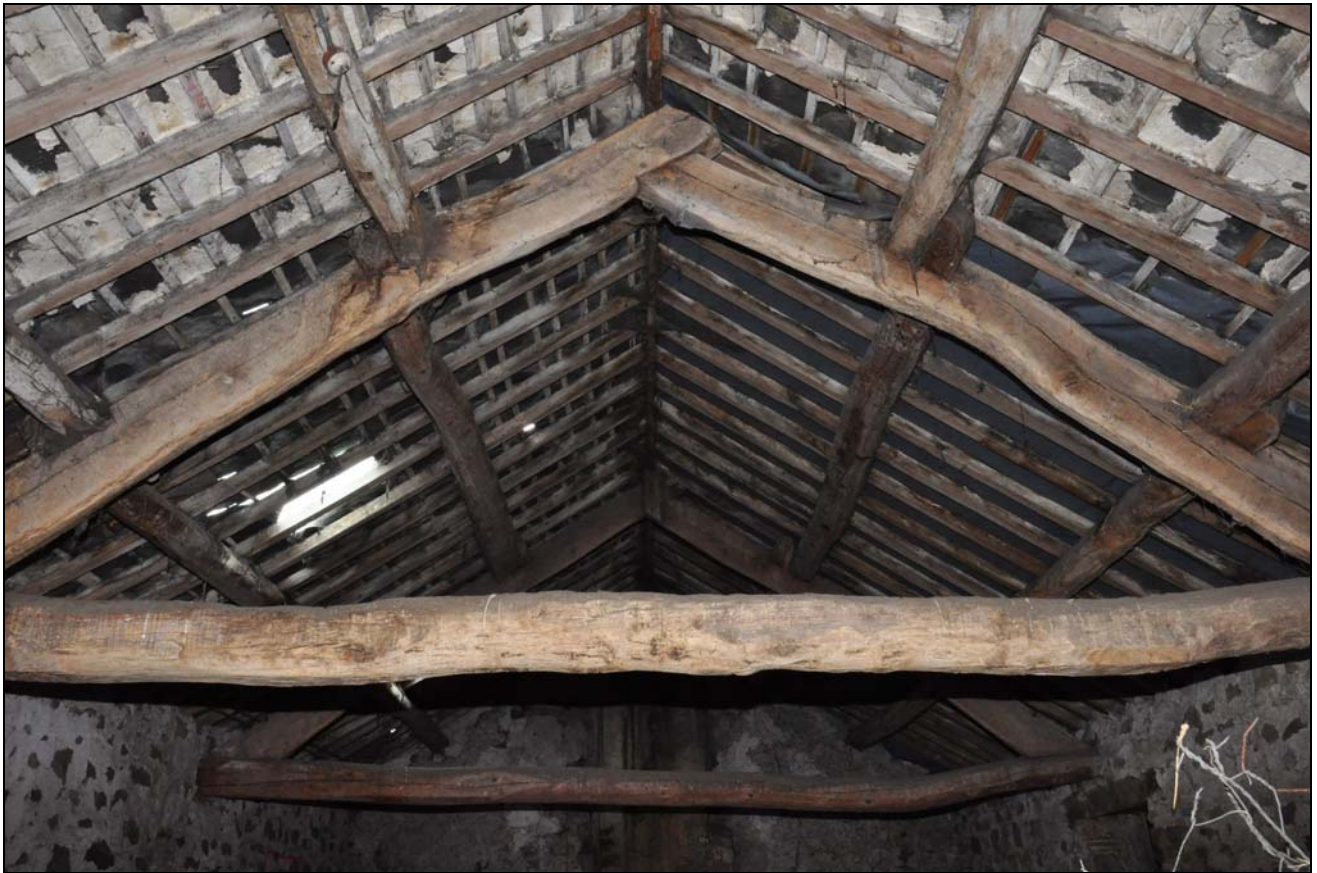
Photo 99: Building 7: west roof truss, looking east
