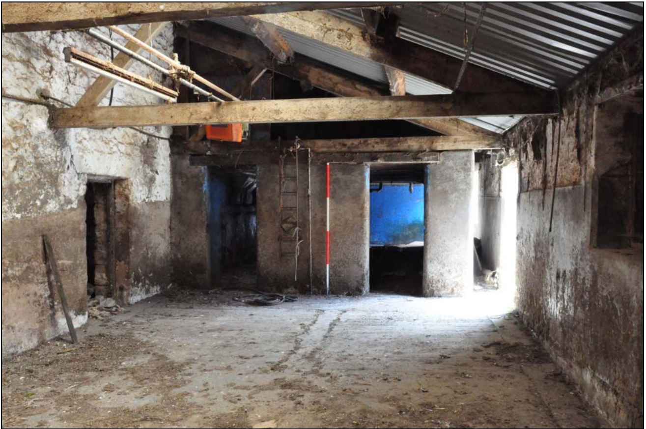
Photo 72: Building 3: interior, looking south-east towards 1960s milking parlour
