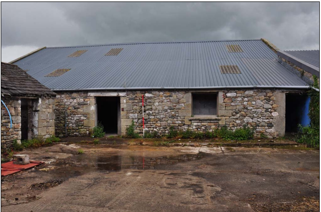
Photo 69: Building 3: south-west side
