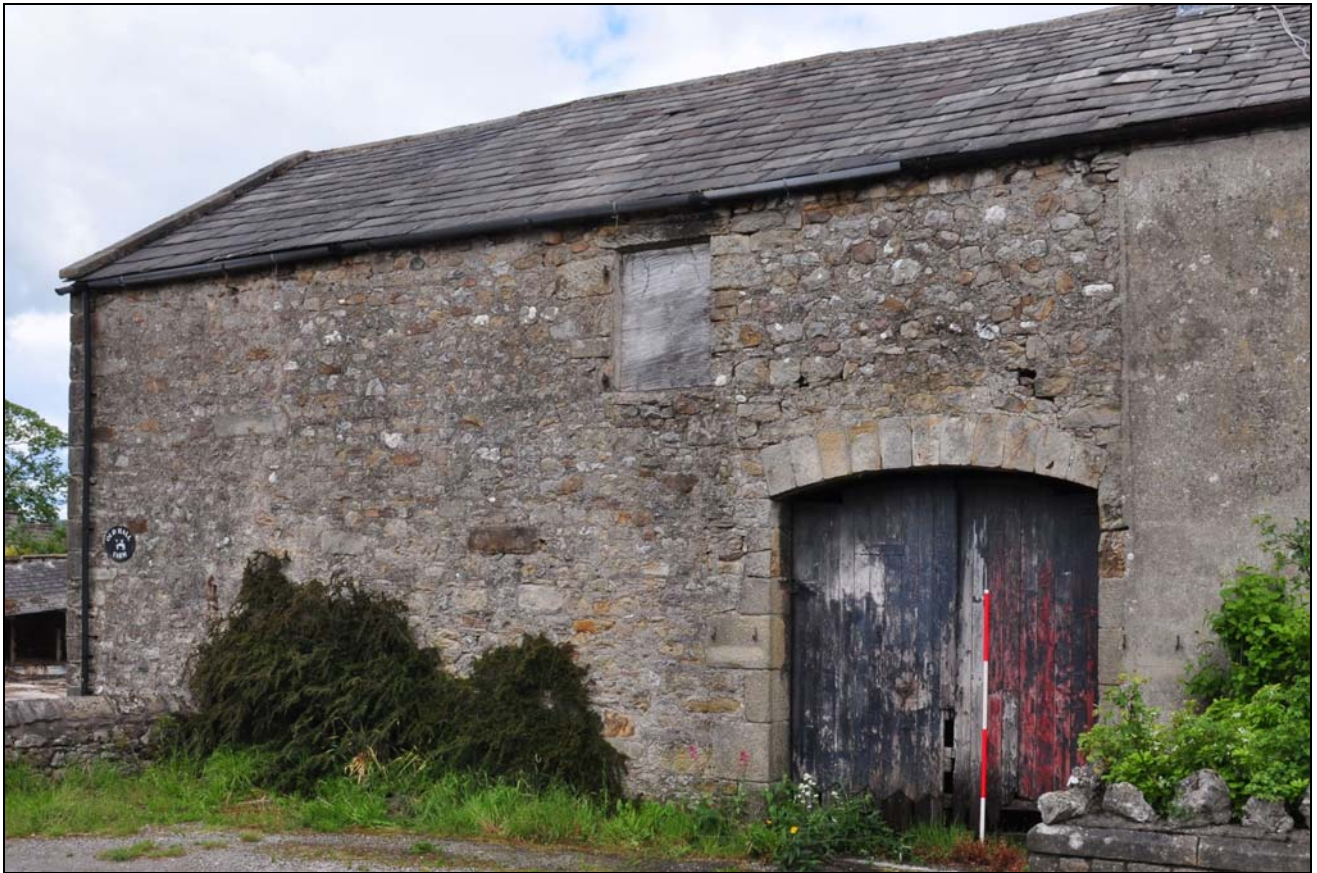
Photo 87: Building 7: front elevation
