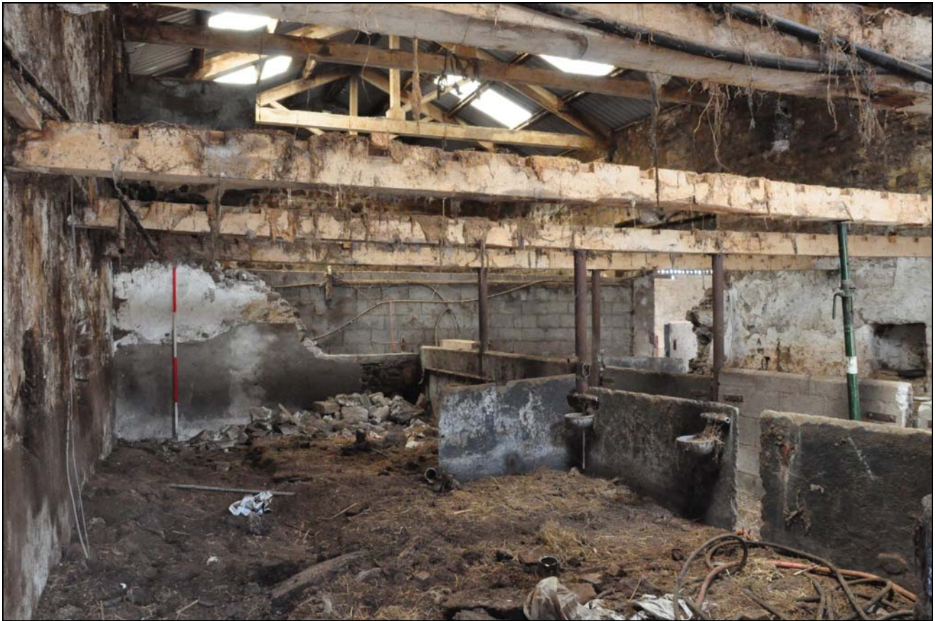
Photo 59: Building 4: view into shippon, looking north
