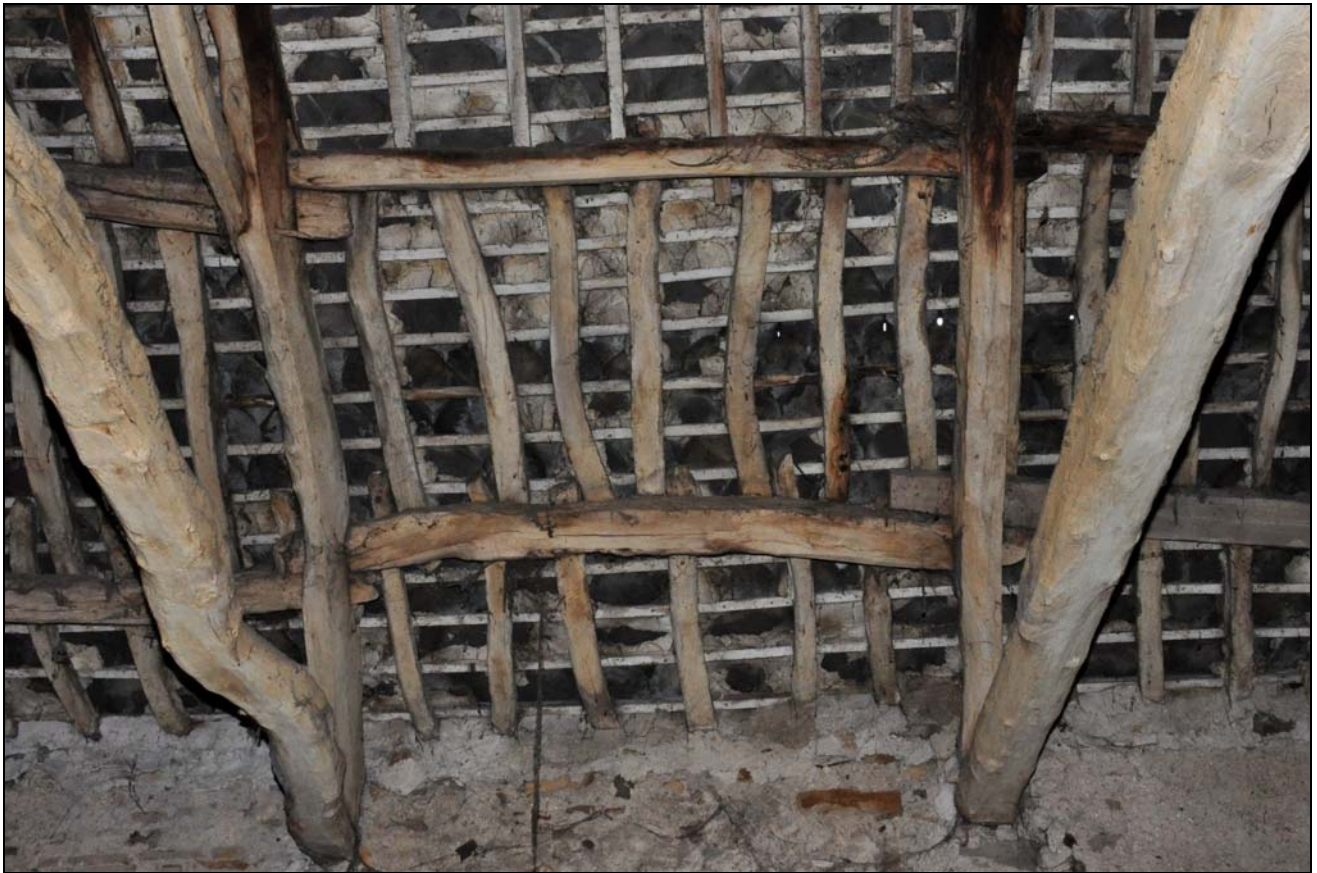
Photo 34: Building 1: underside of rear roof pitch, showing original rafters
