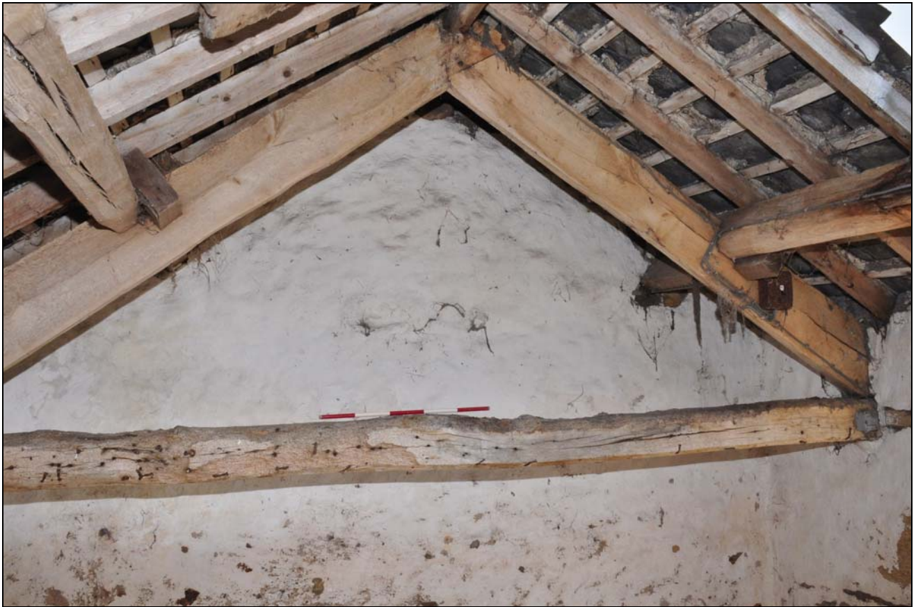
Photo 44: Building 2: end roof truss, looking north-east
