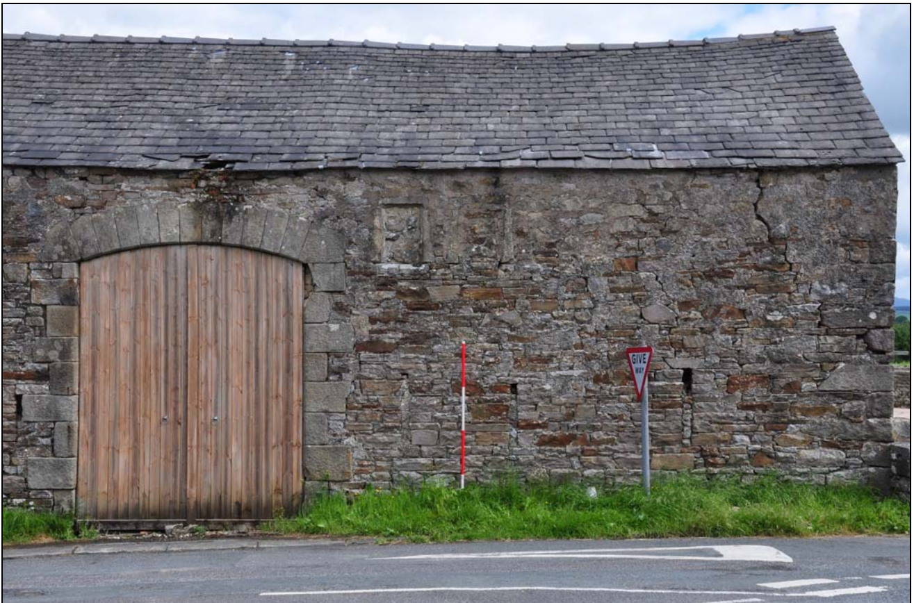
Photo 4: Building 1: right-hand part of front elevation
