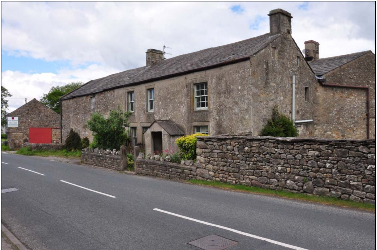
Photo 84: General view of Building 7, and house
