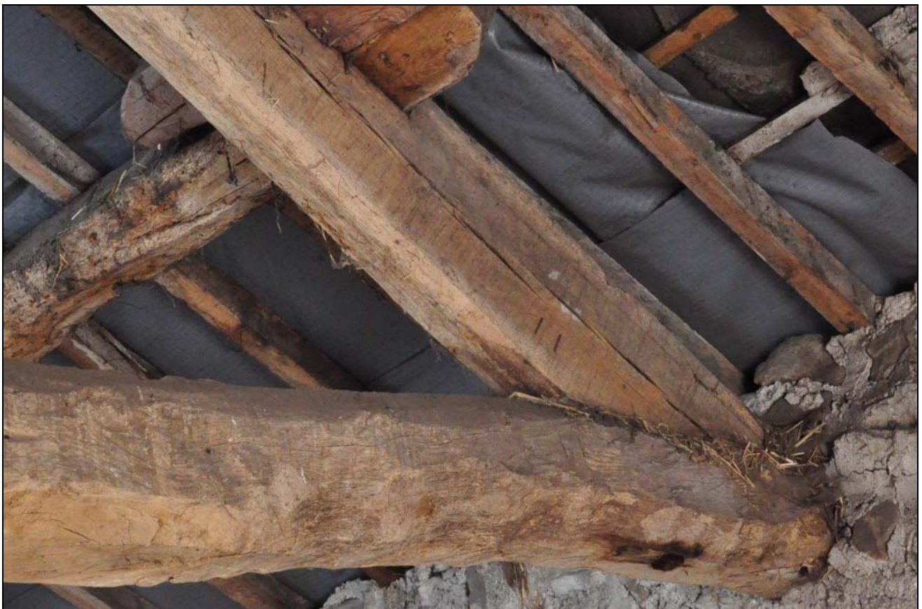
Photo 102: Building 7: numbering on west roof truss, looking east
