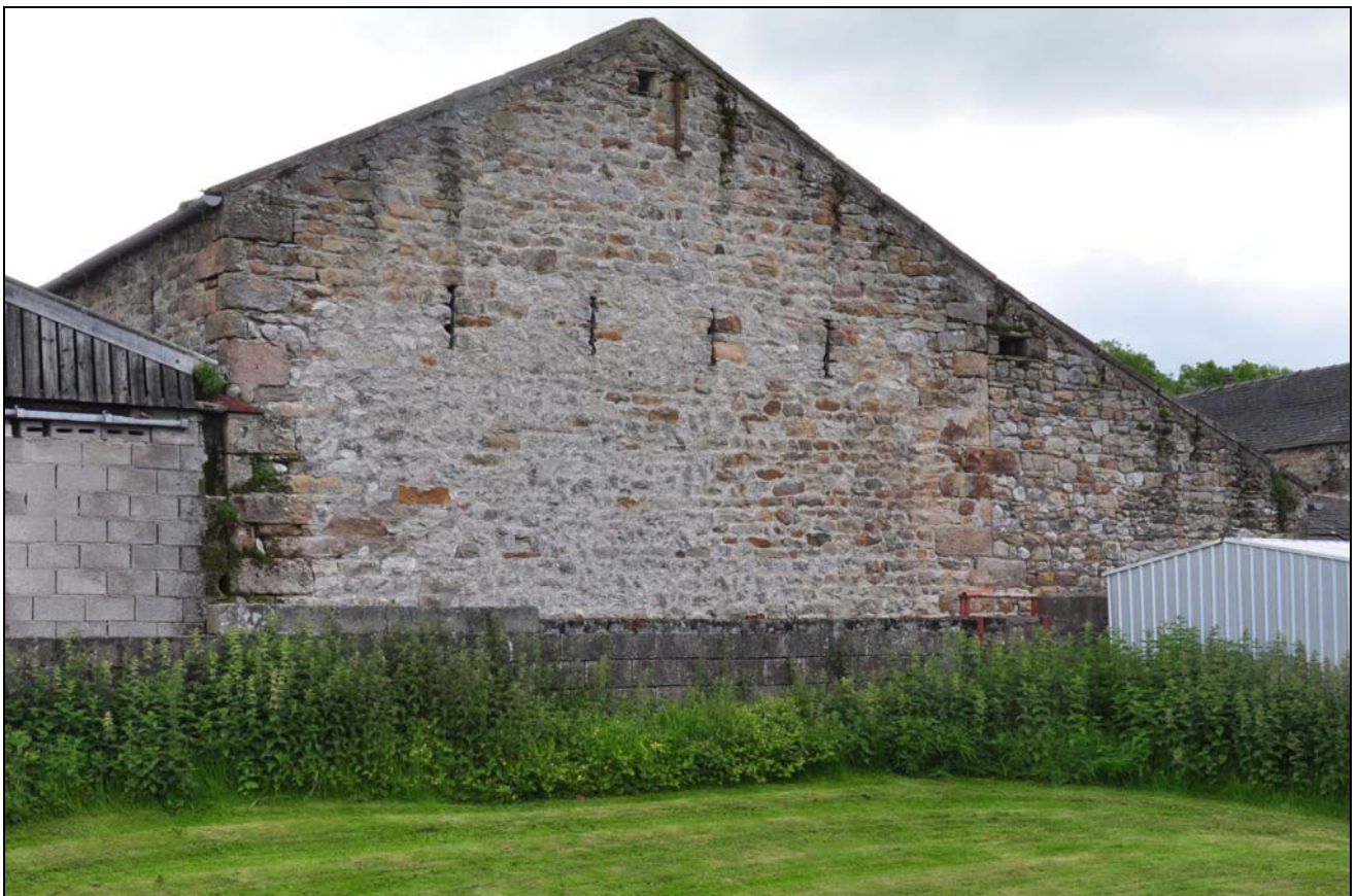
Photo 53: Building 4: north-west gable
