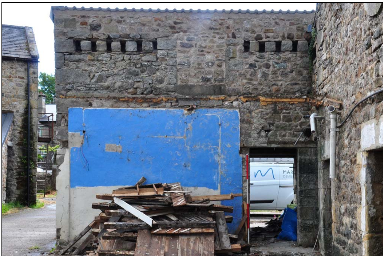
Photo 77: Building 10: north-east side
