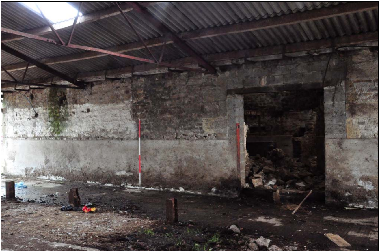
Photo 51: Building 4: cart entrance in north-east side, looking south
