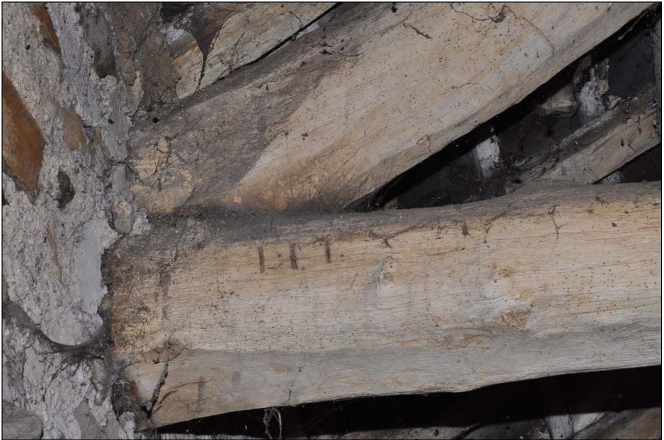
Photo 27: Building 1: detail of truss numbering
