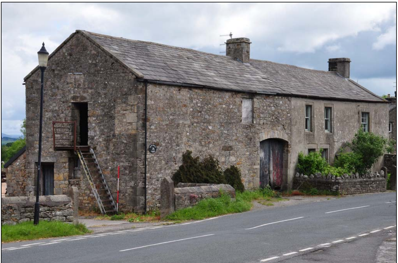
Photo 85: General view of Building 7, and house
