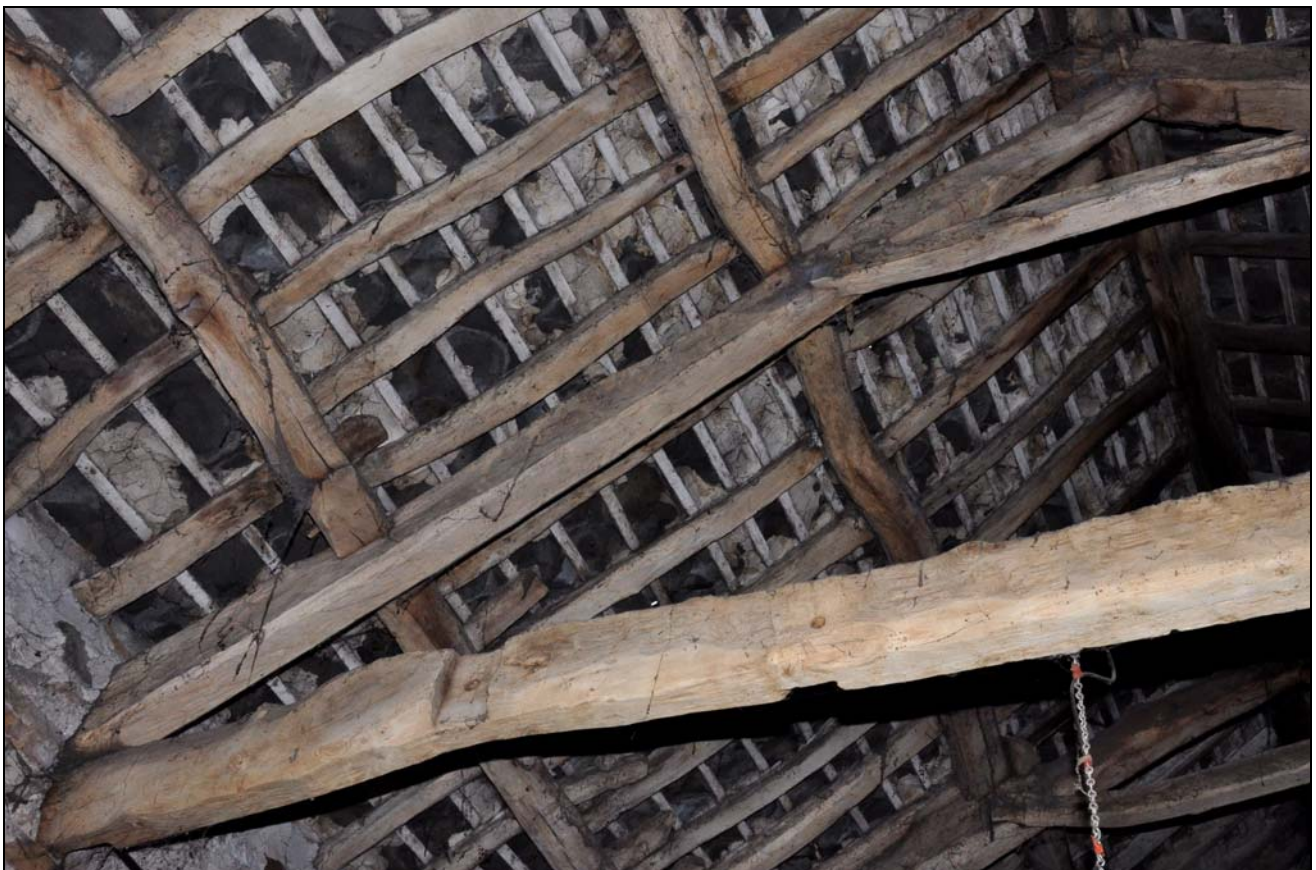
Photo 28: Building 1: detail of truss I at north-west end (with re-used crucks)
