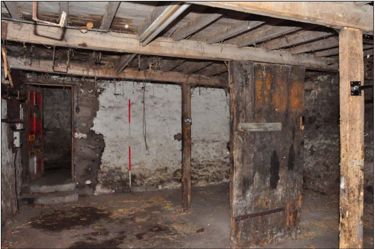
Photo 94: Building 7: stable, looking south-east
