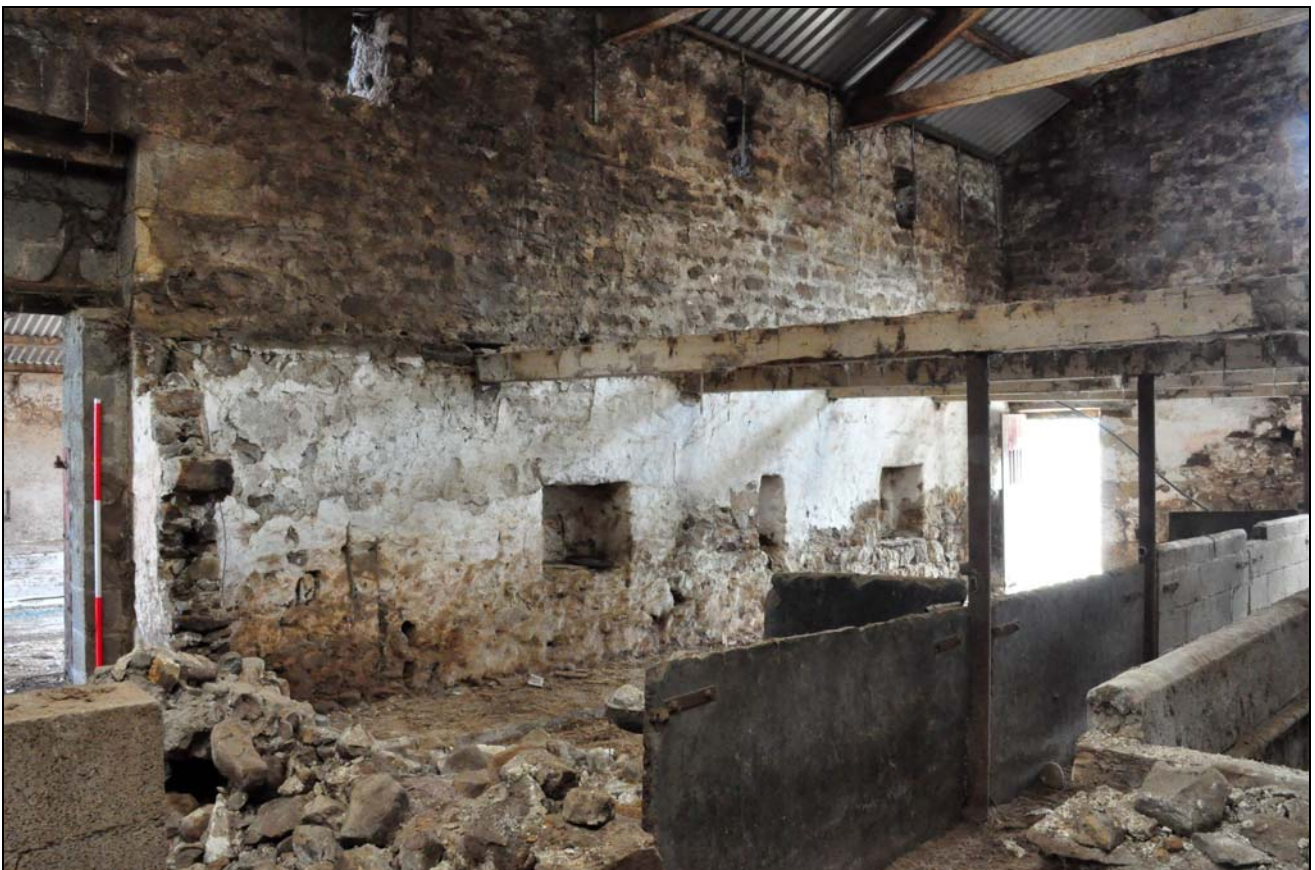
Photo 57: Building 4: view into shippon across former cross-wall, looking east
