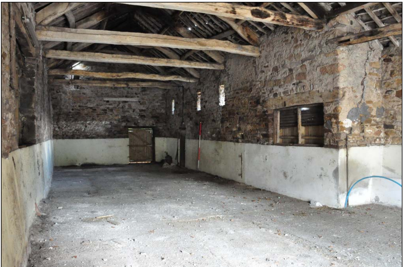
Photo 21: Building 1: interior, looking north
