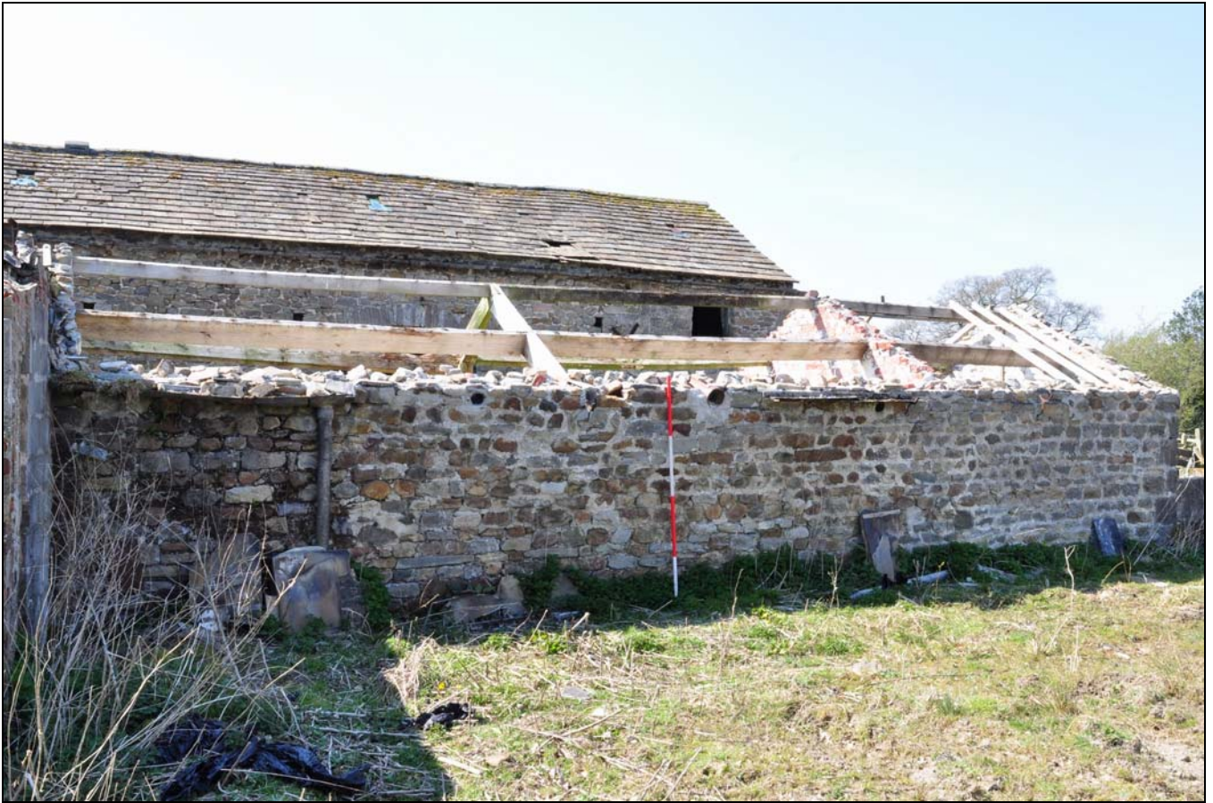
Photo 49: Detached outbuilding, looking north-west
