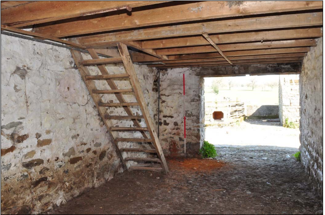
Photo 43: Cart-shed: ground floor, looking east
