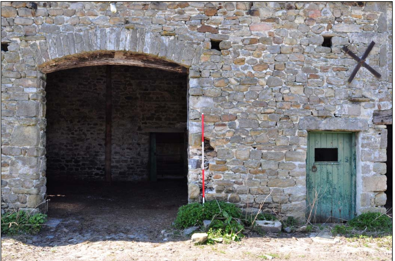
Photo 4: Cart entrance and shippon doorway, in front of original barn
