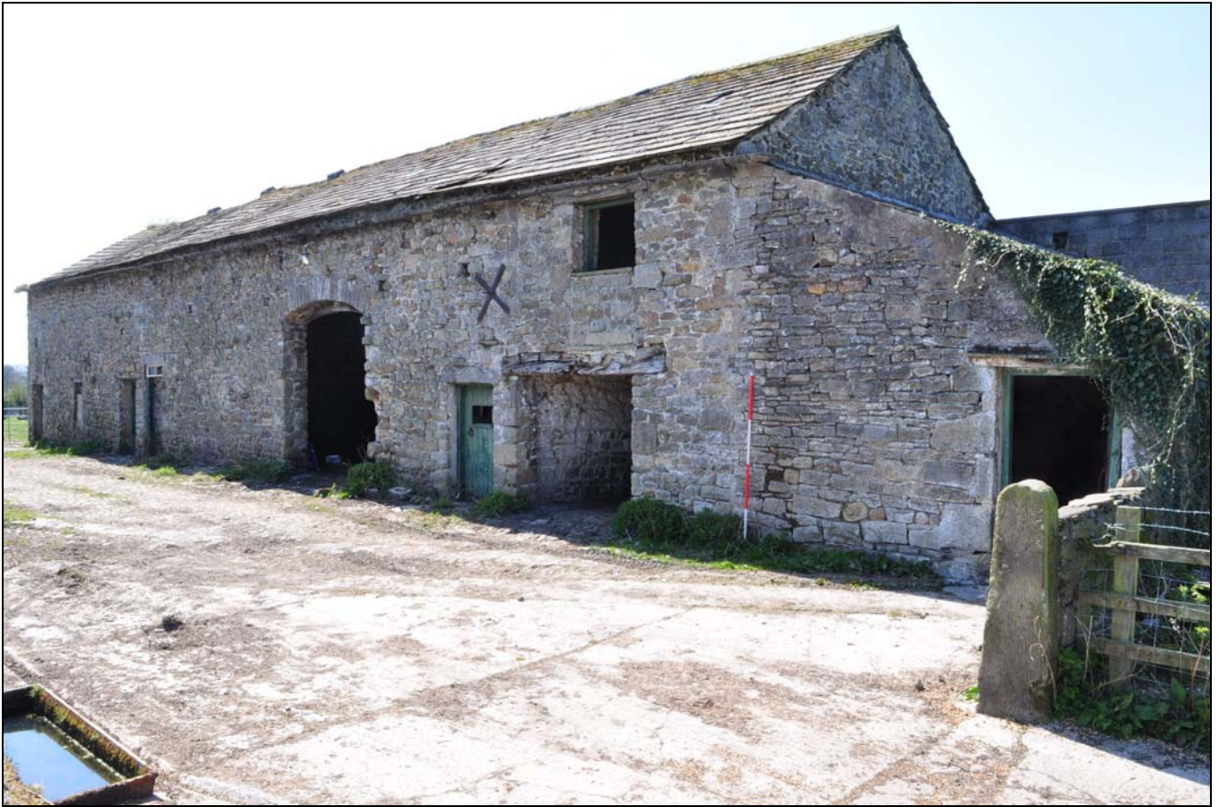
Photo 1: Front of the barn range, looking south-west
