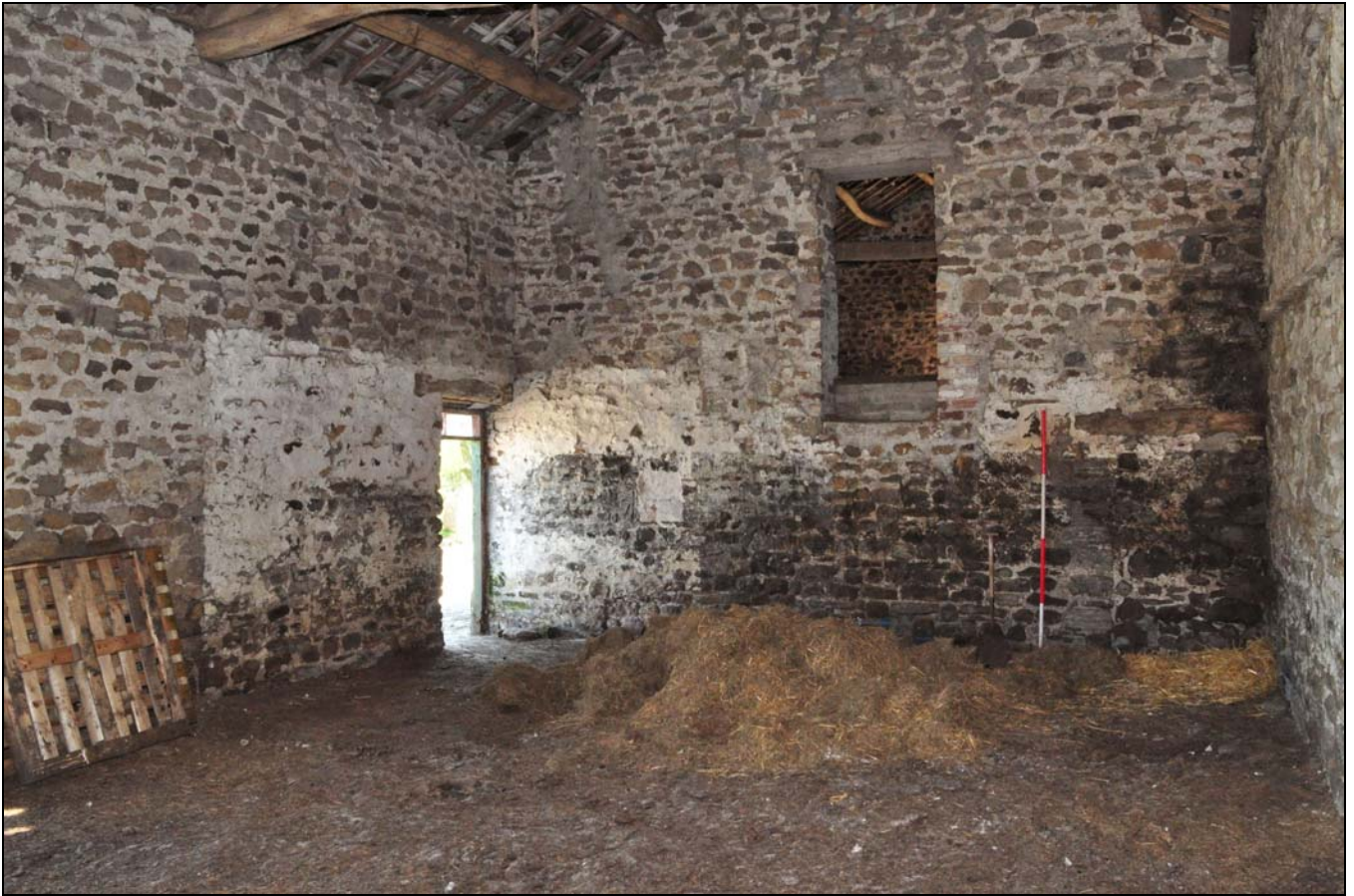
Photo 7: Interior of original part of barn, looking south-east
