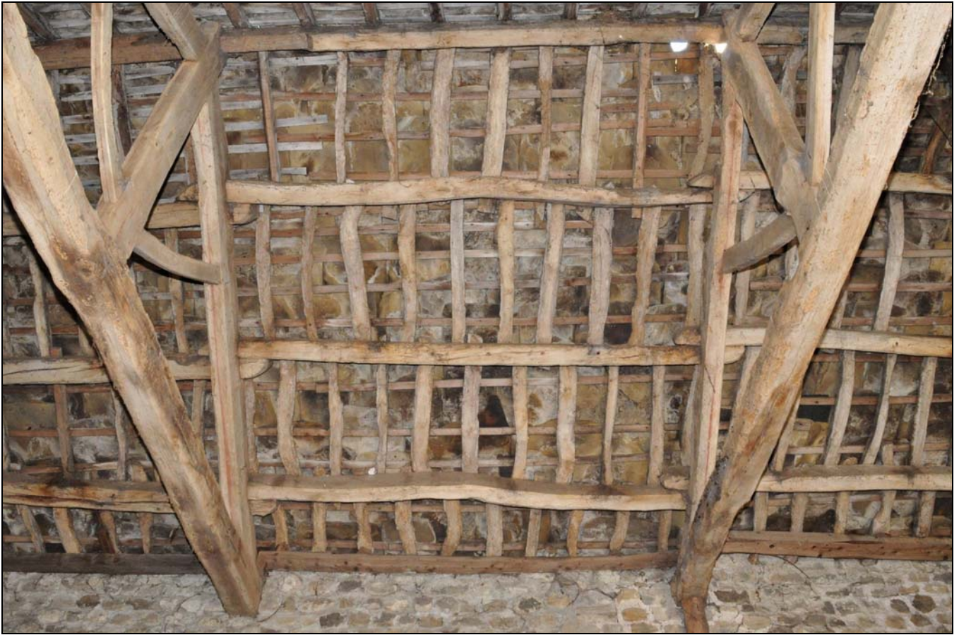
Photo 25: Underside of west roof pitch in original barn
