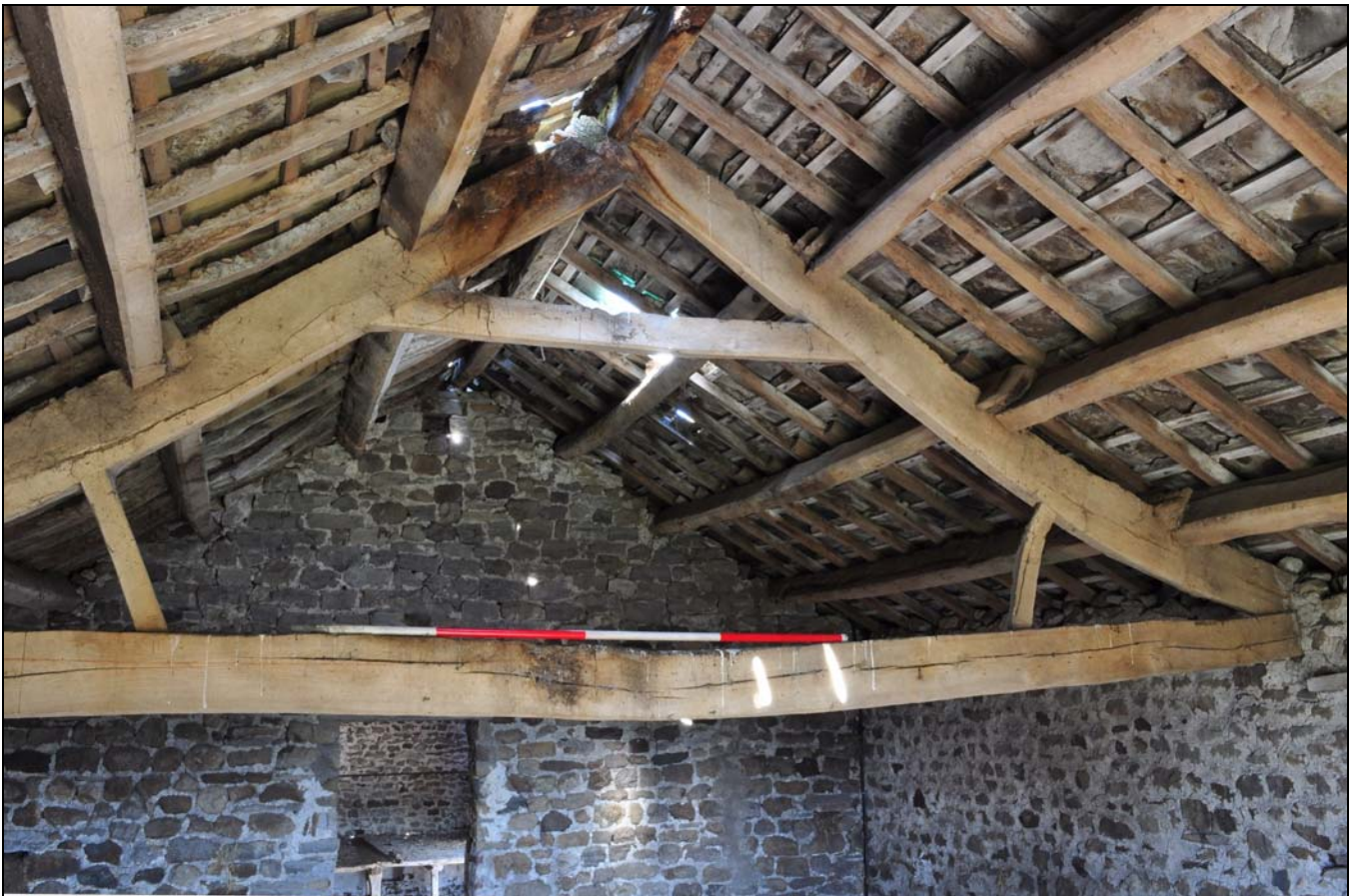
Photo 36: Added shippon to south of barn: roof truss, looking north-east
