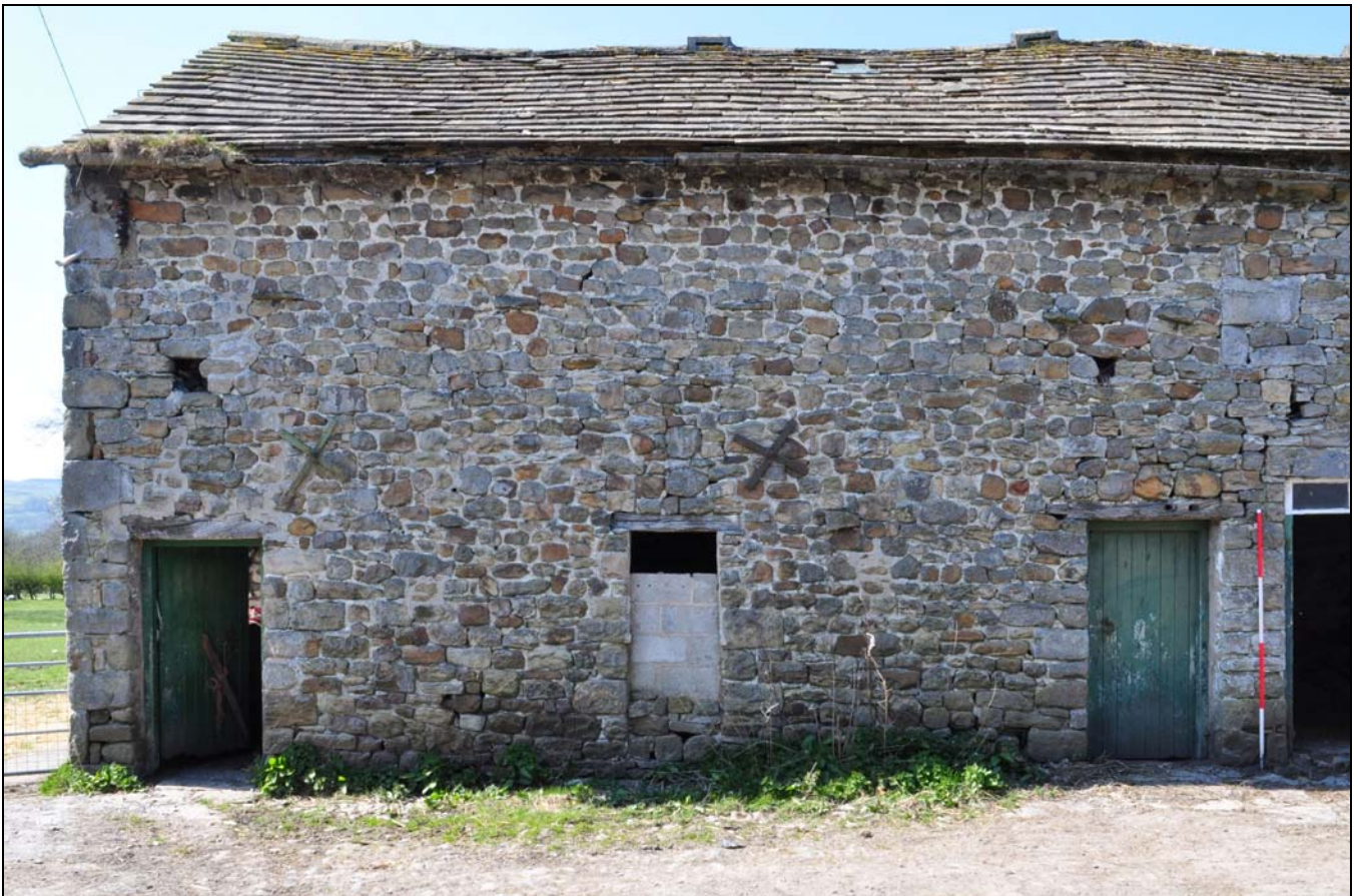
Photo 28: Front of added shippon to south of barn
