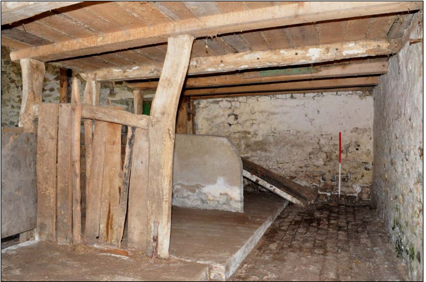
Photo 17: Stalls in shippon, looking west
