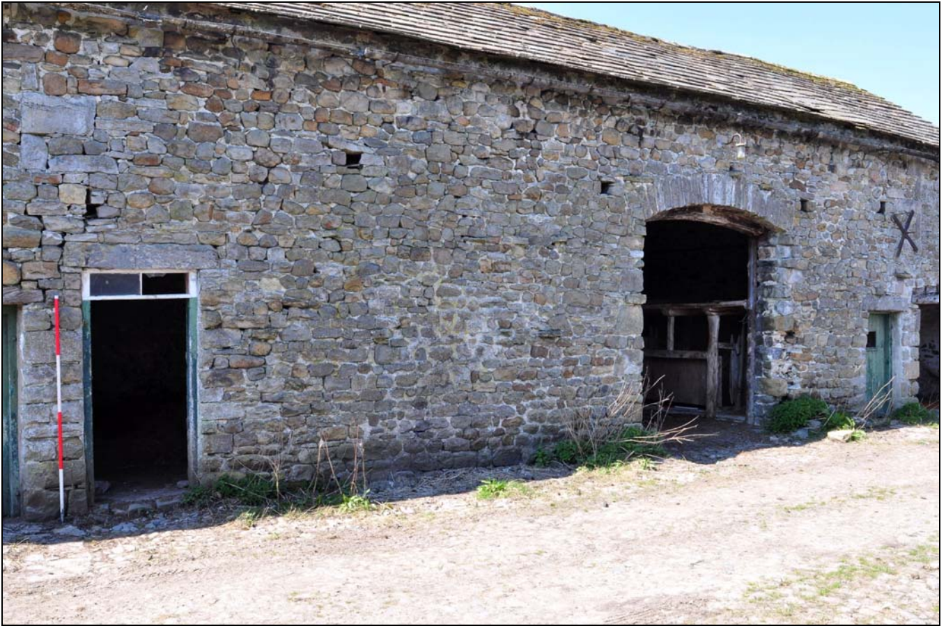
Photo 3: Original part of barn range
