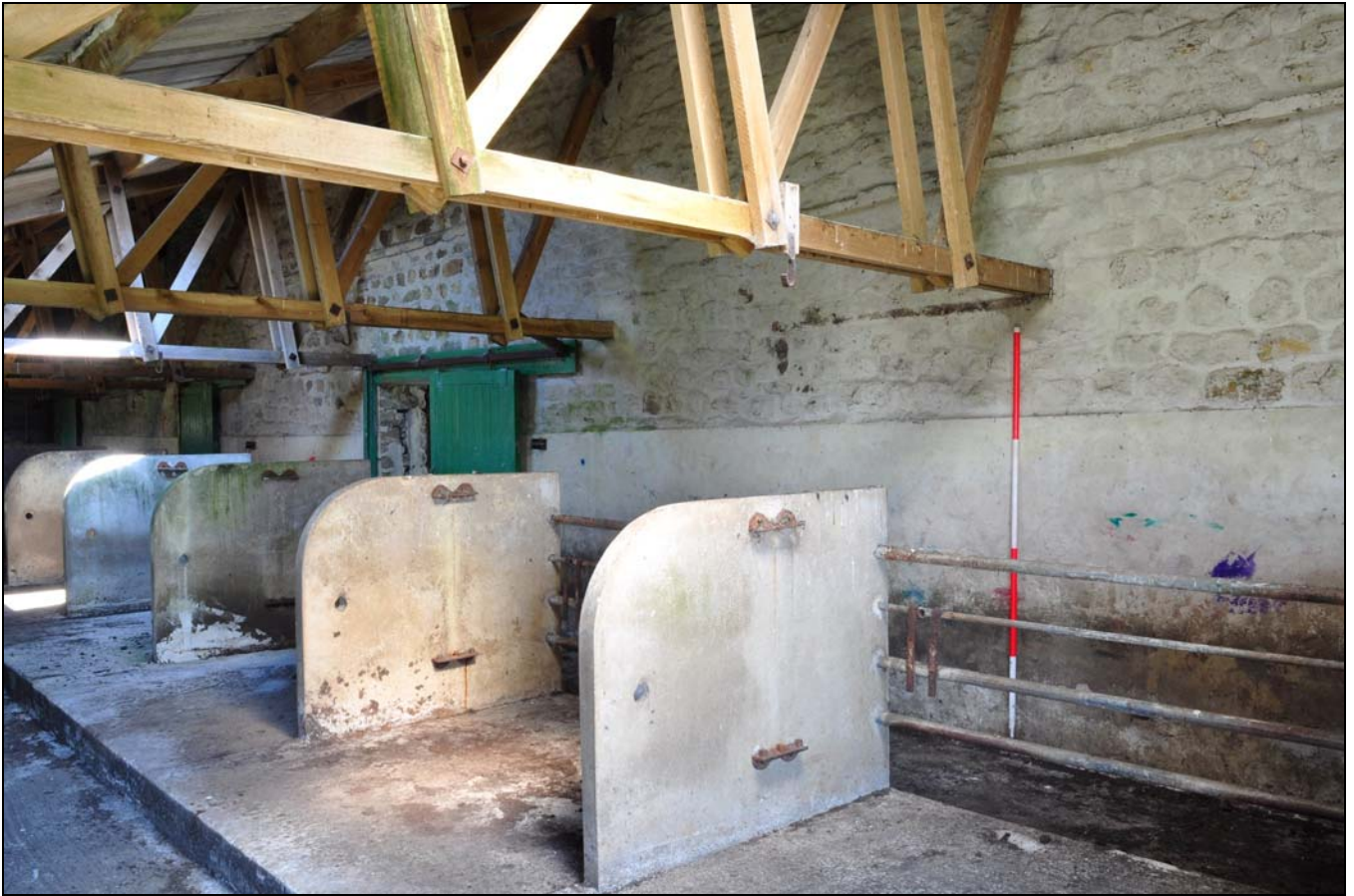
Photo 5: Rear of original barn, in modern lean-to, with areas of rebuilding
