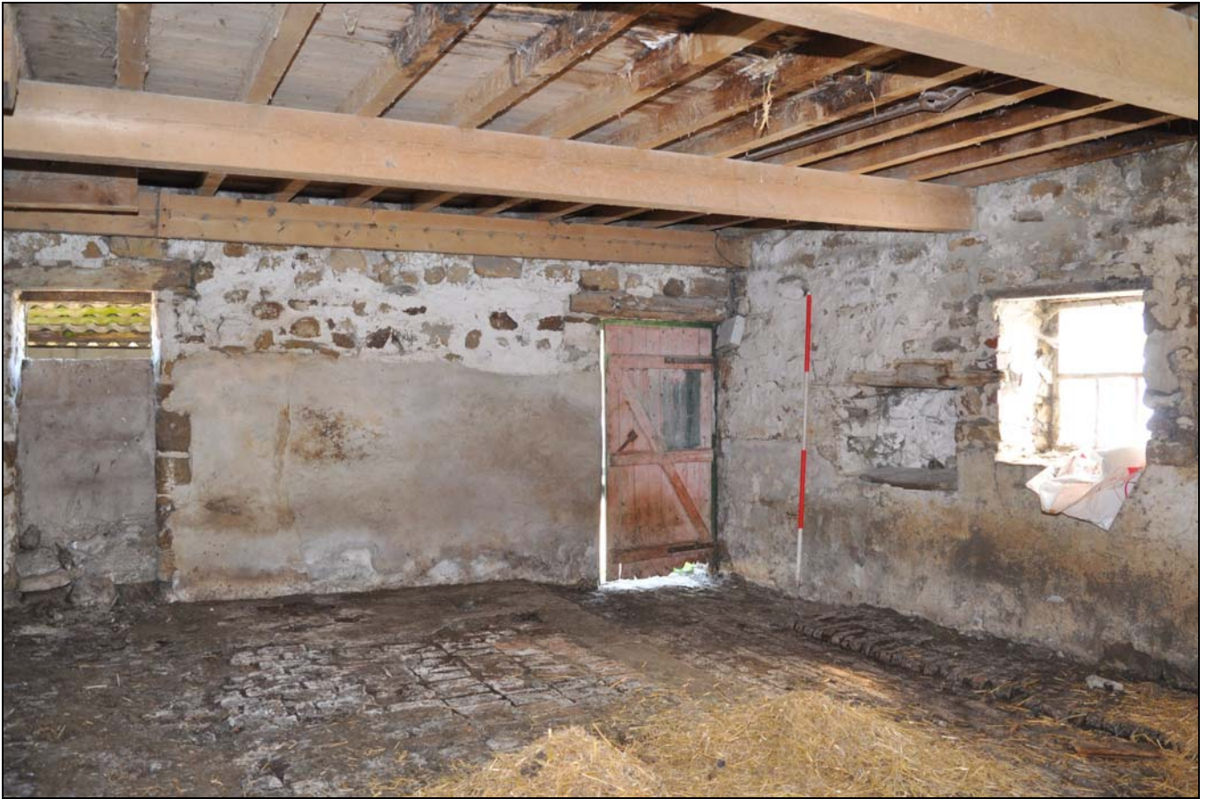
Photo 34: Added shippon to south of barn: ground floor, looking south-east
