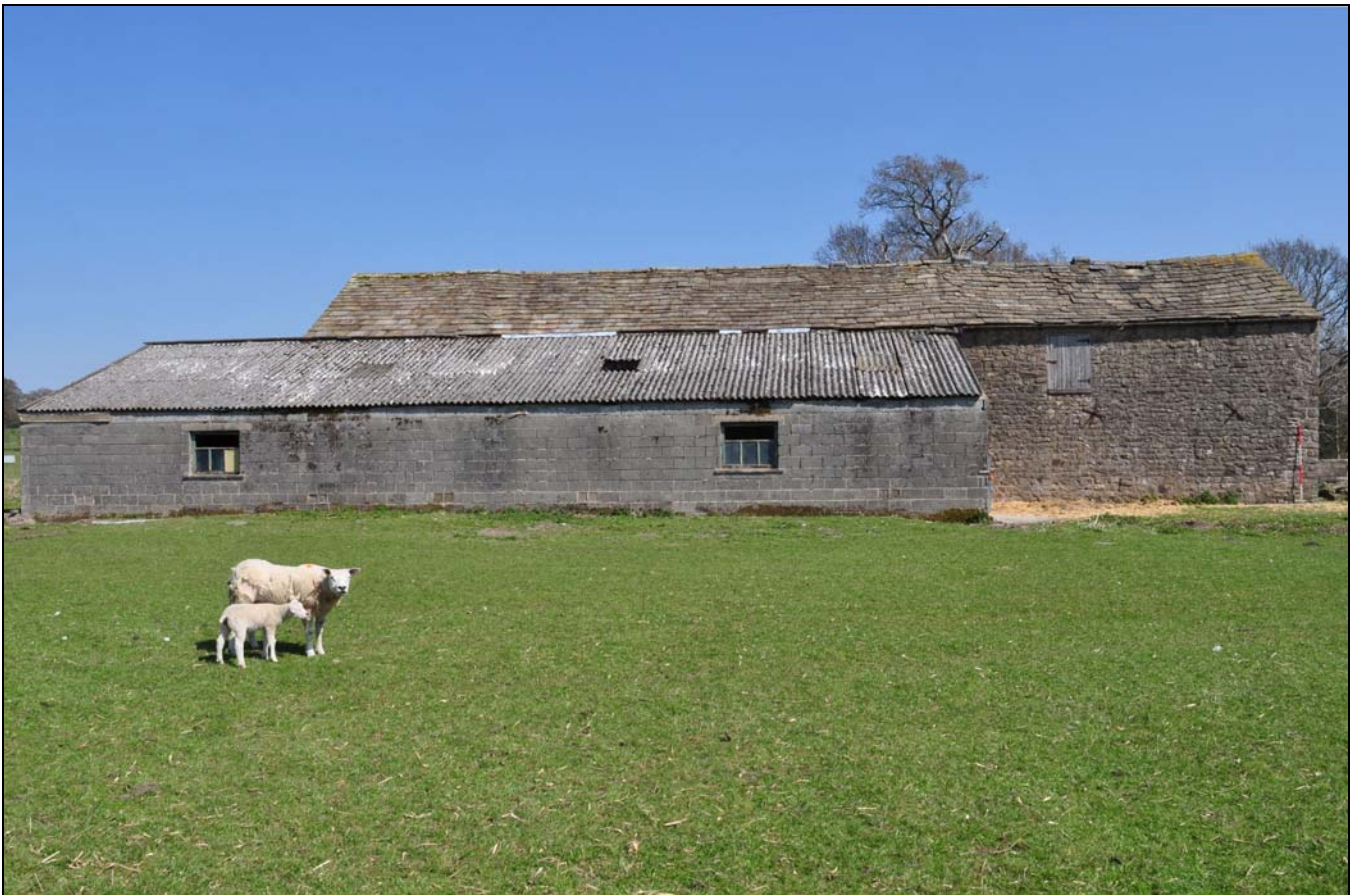
Photo 2: Rear of the barn range, looking east
