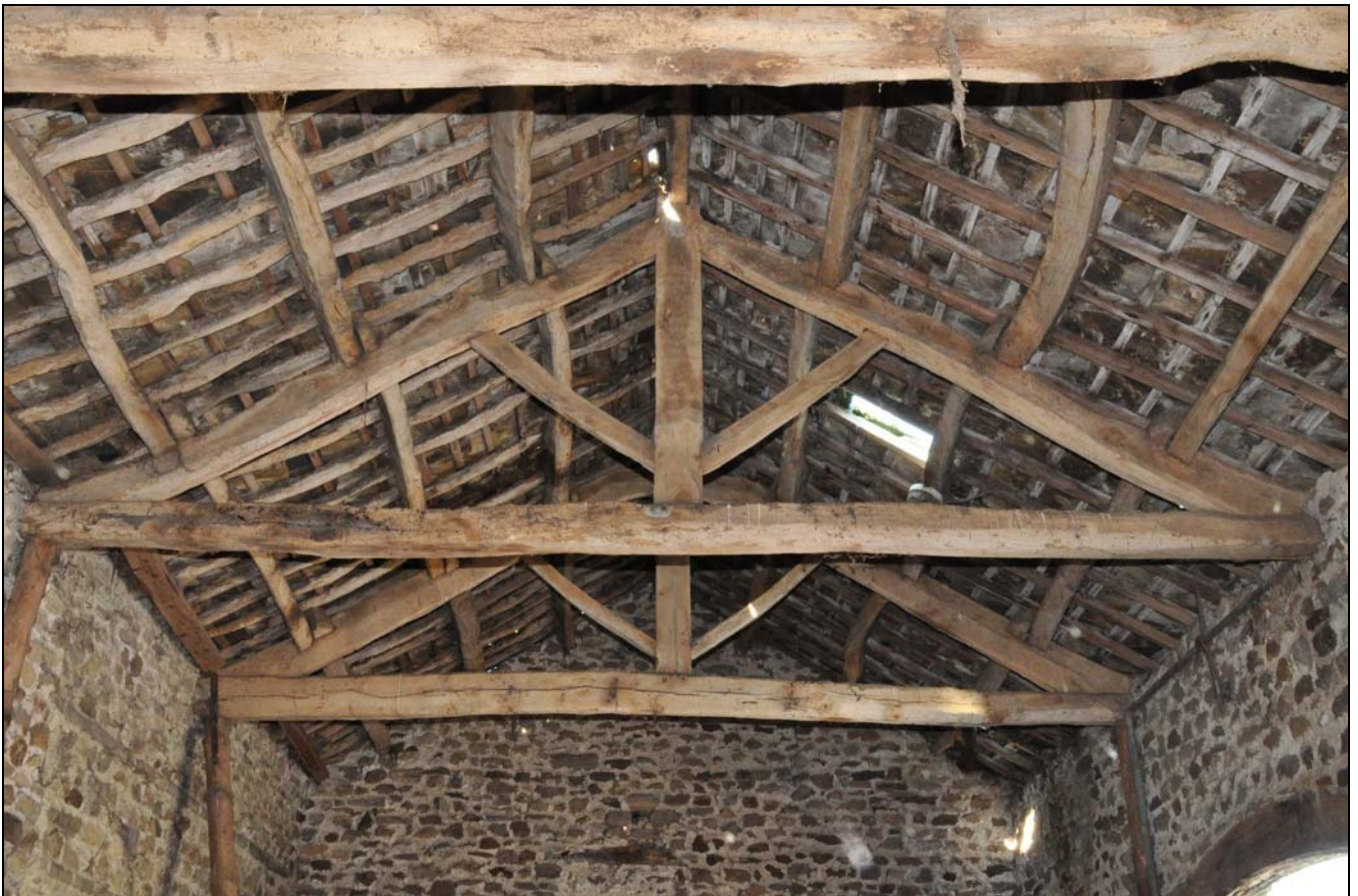
Photo 23: Central roof truss in original barn, looking north
