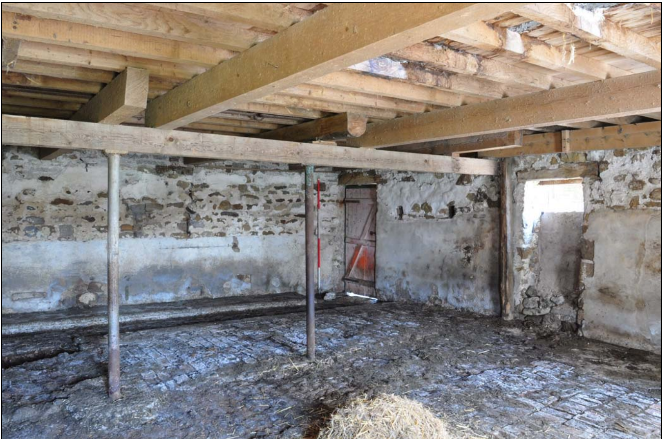
Photo 32: Added shippon to south of barn: ground floor, looking north-east
