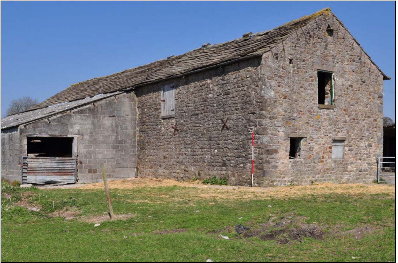
Photo 30: Added shippon to south of barn, looking north-east
