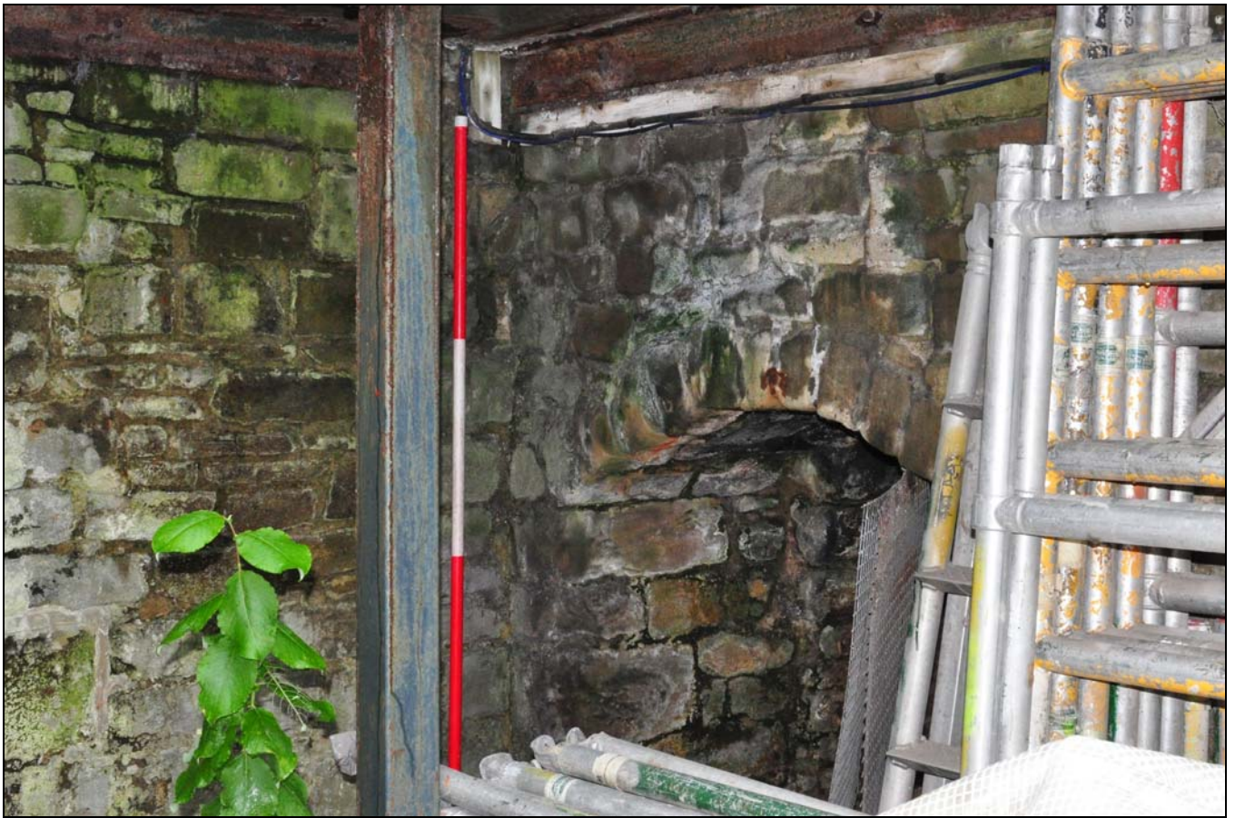
Photo 17: Flue to south-west of boiler house, beneath modern gantry
