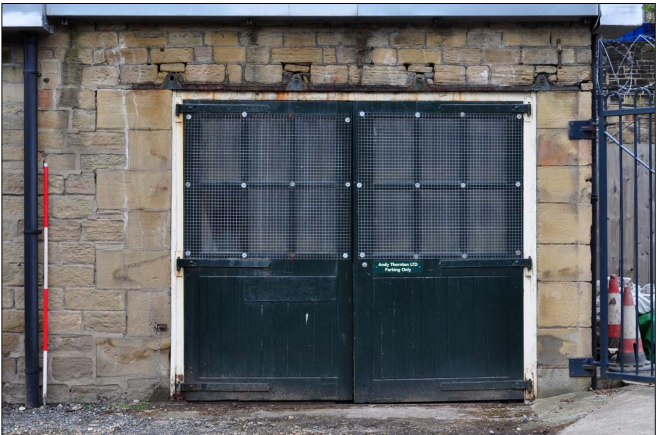
Photo 6: Detail of entrance to boiler house
