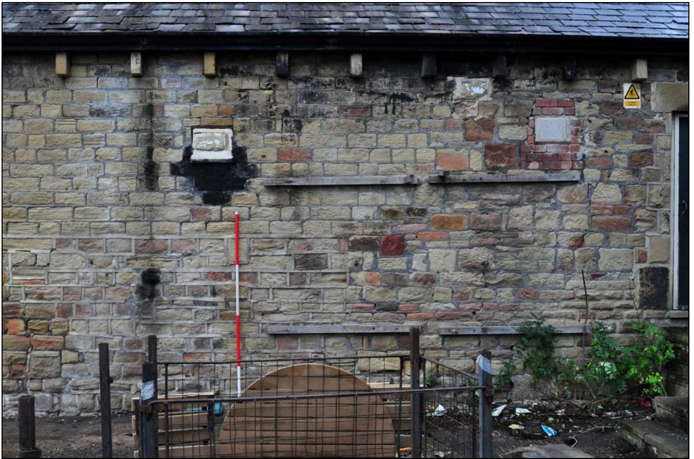
Photo 13: South-west side of boiler house: central part, with two bearing boxes
