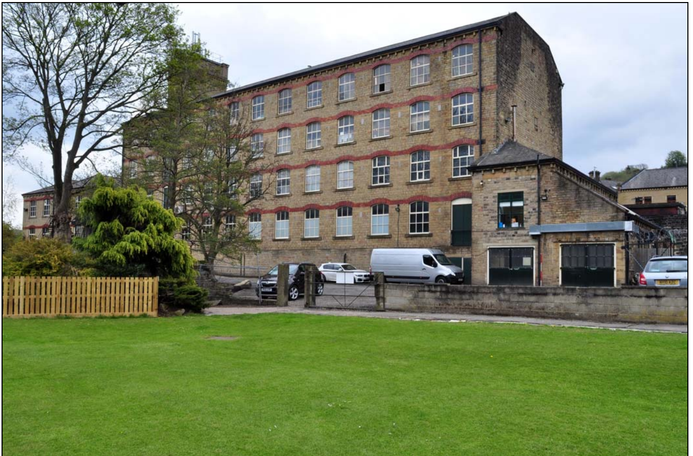
Photo 2: General view of the mill, from the west
