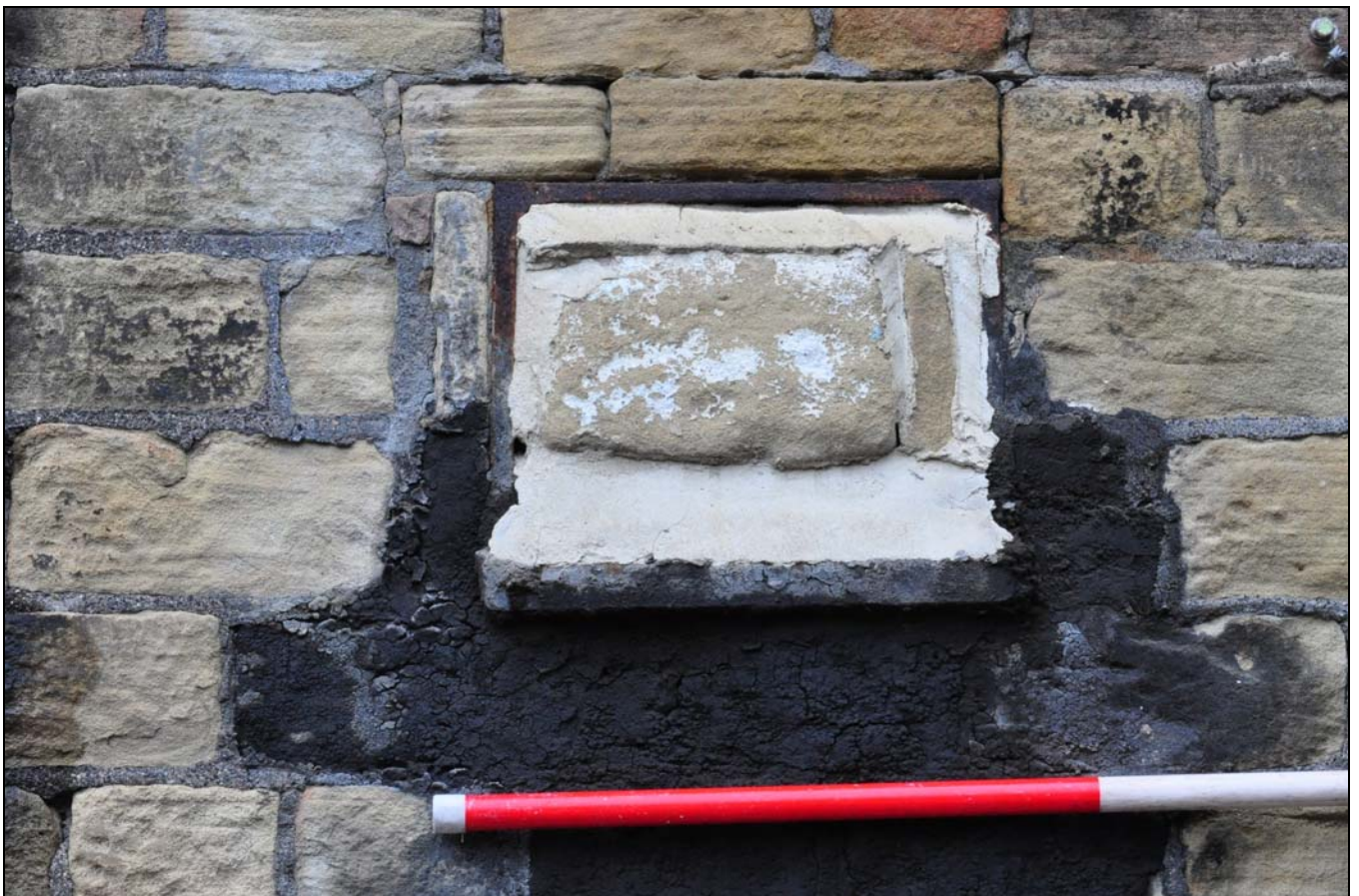
Photo 14: South-west side of boiler house: detail of bearing box
