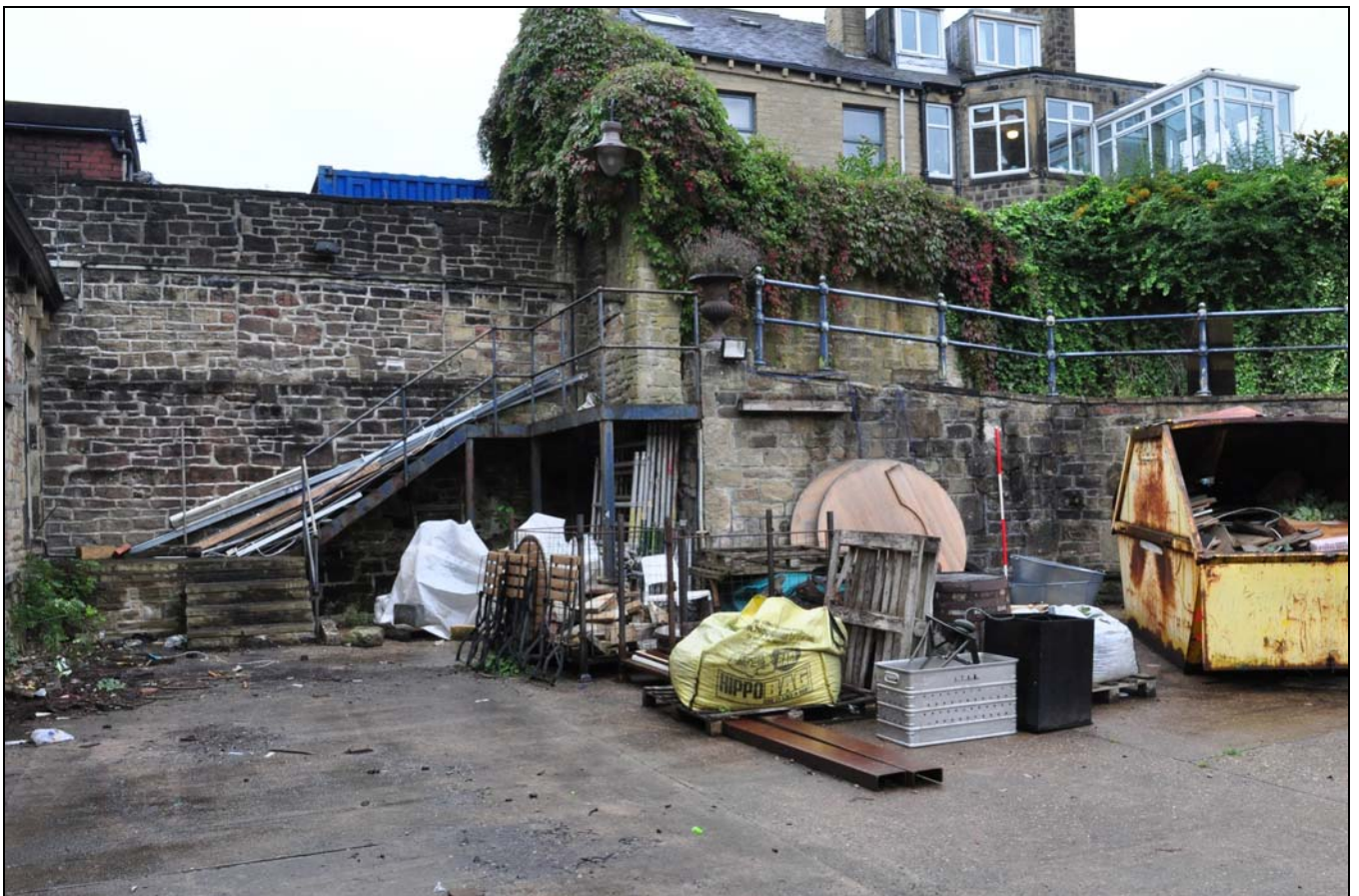
Photo 18: Yard to south-west of boiler house, where flue runs to former chimney
