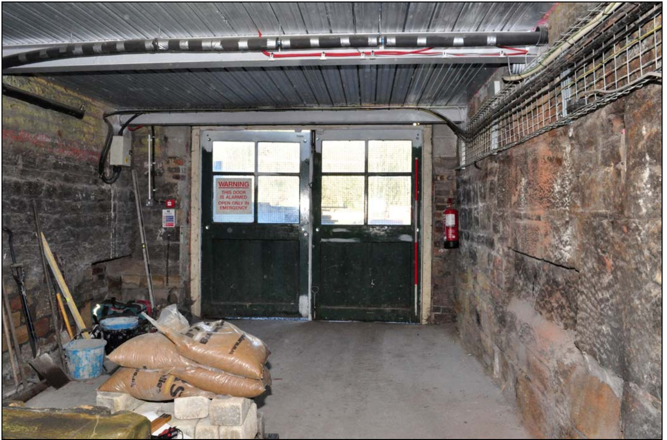
Photo 45: Ground floor of engine house, from the south-east
