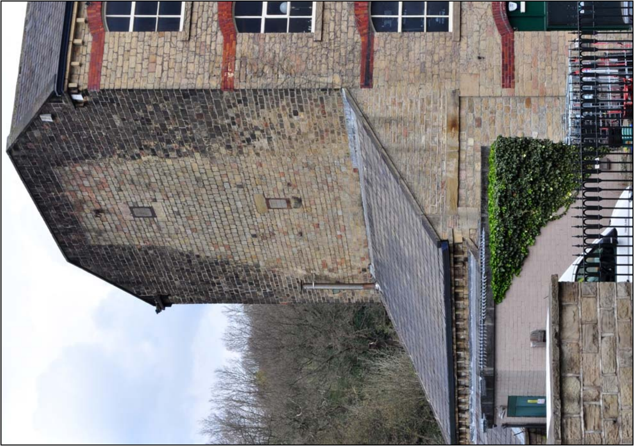
Photo 21: Engine house with end wall of mill behind, with outline of former rope race, from the south
