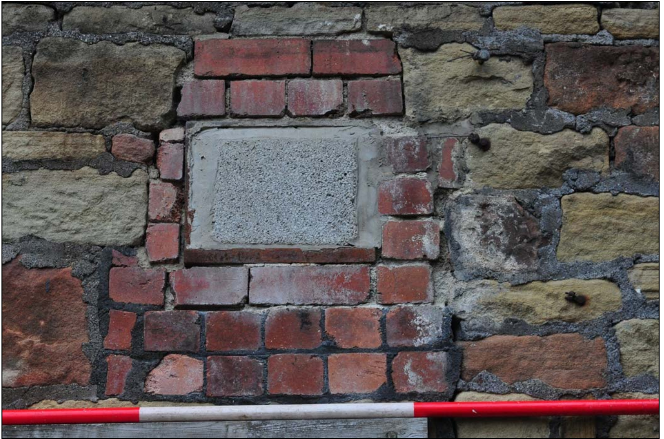
Photo 15: South-west side of boiler house: detail of bearing box
