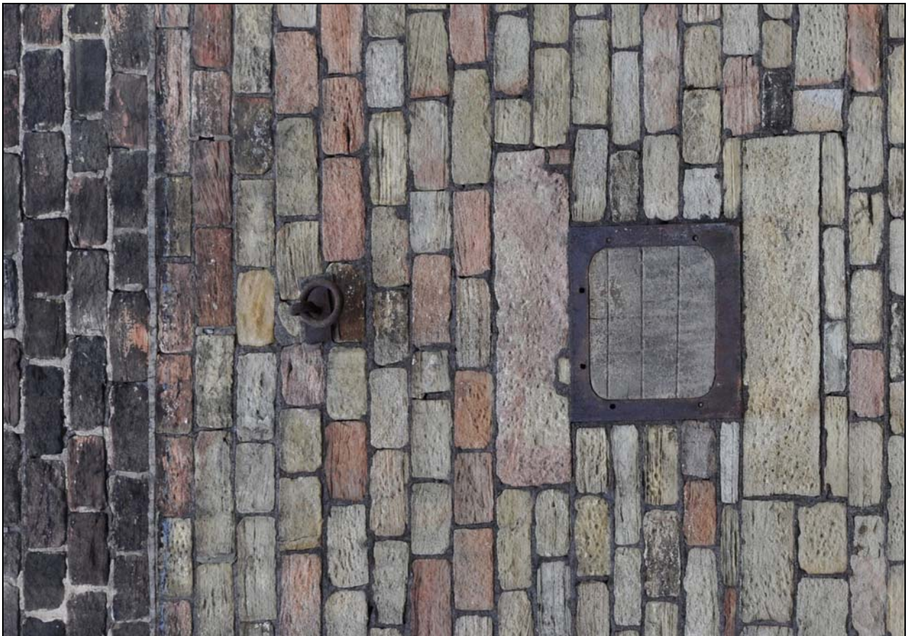
Photo 24: Upper bearing for shafts from rope race, and ring, in end wall of mill, from the south-west
