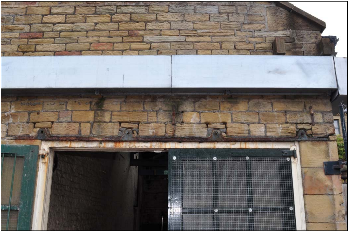
Photo 7: Detail of lintel over entrance to boiler house
