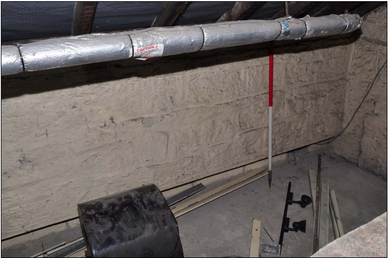
Photo 63: Window lintel in north-west side of engine house roof space, from the south
