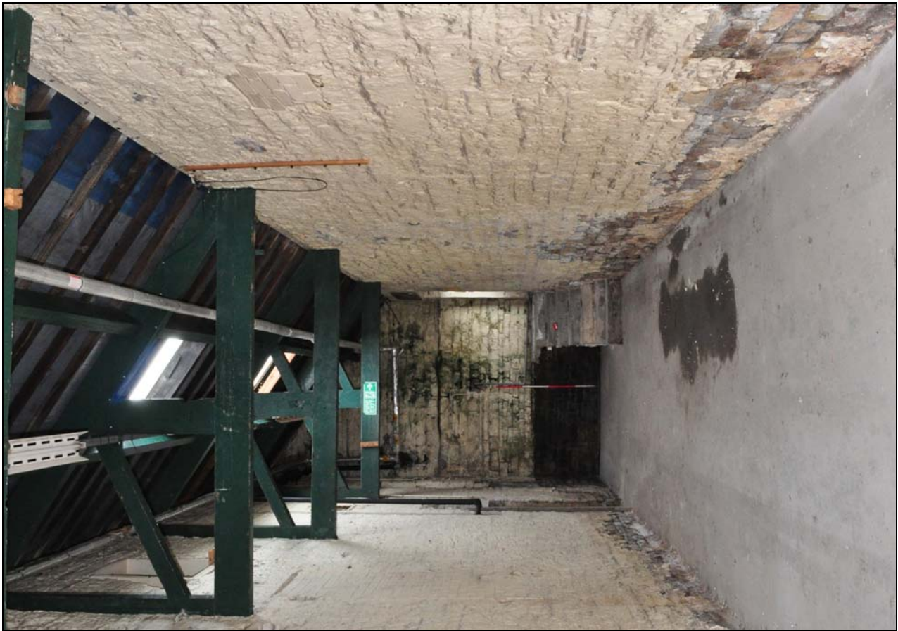
Photo 27: Interior of boiler house, from the north-west
