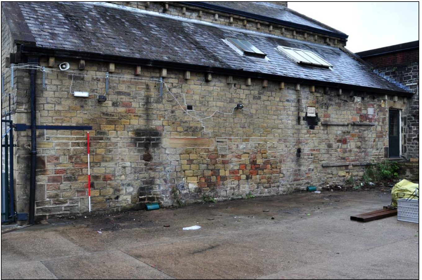
Photo 11: South-west side of boiler house
