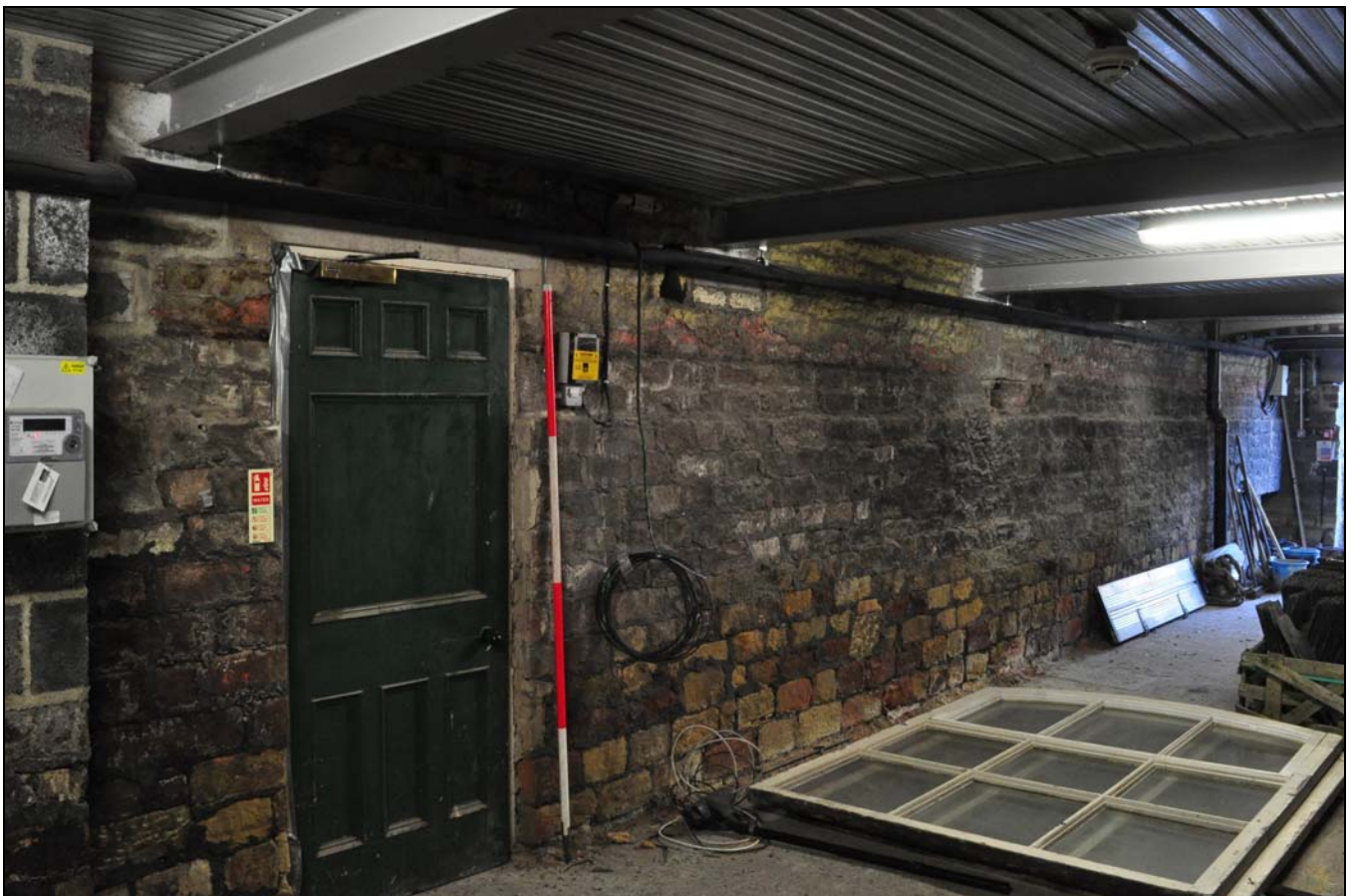
Photo 60: Ground floor of engine house, south-west side, from the east
