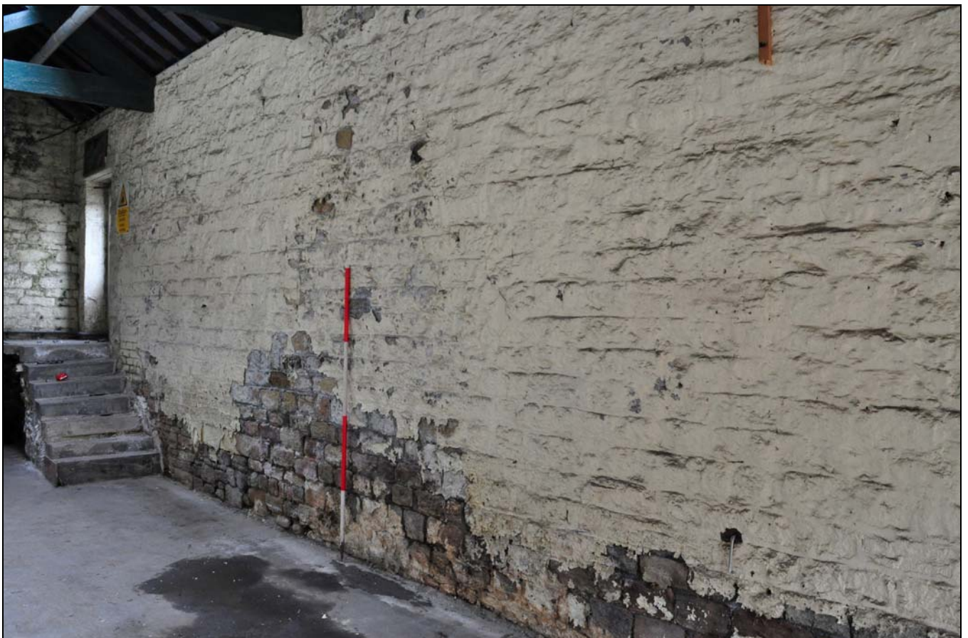
Photo 32: Interior of boiler house: south-west side, from the north
