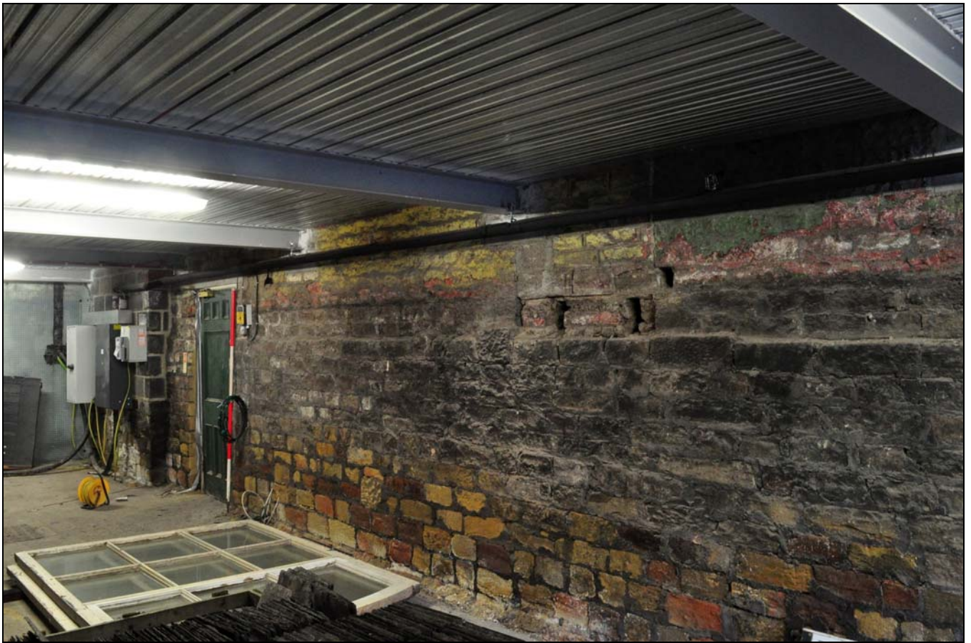
Photo 59: Ground floor of engine house, south-west side, from the north
