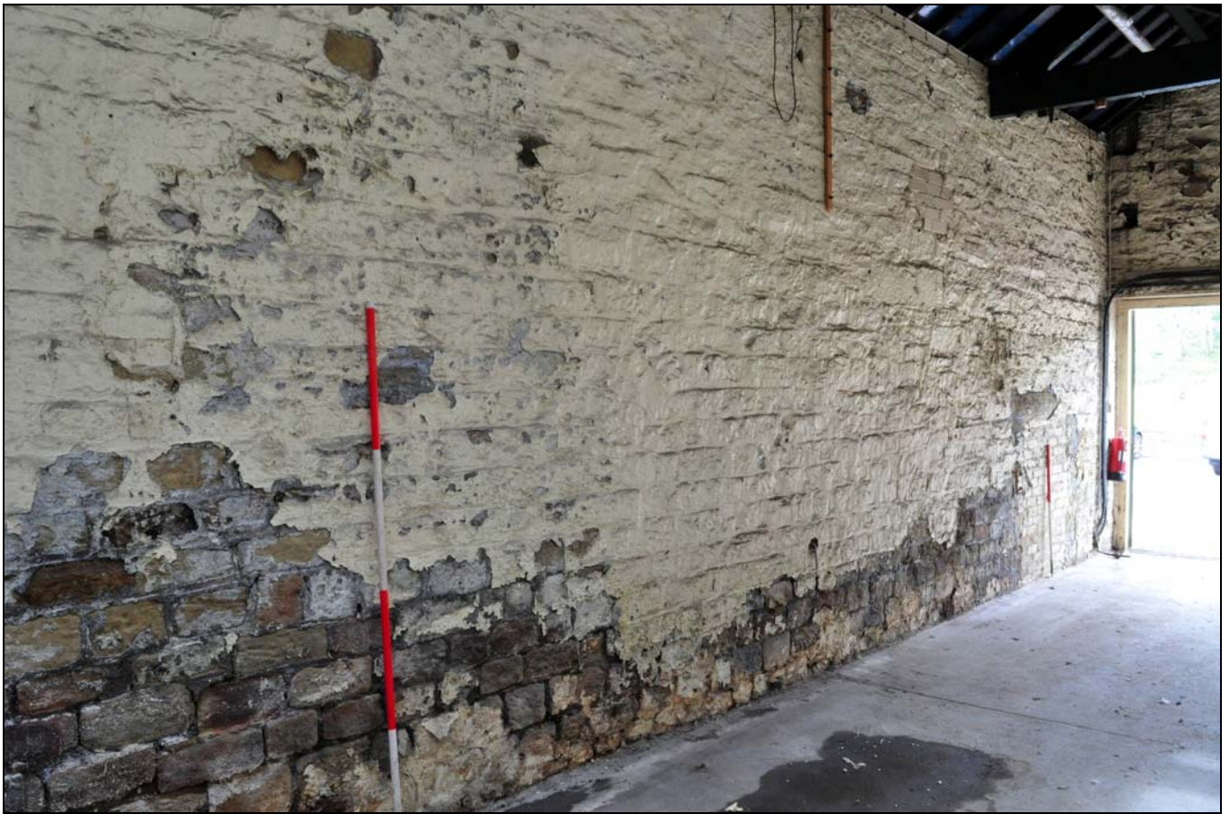
Photo 33: Interior of boiler house: south-west side, from the east
