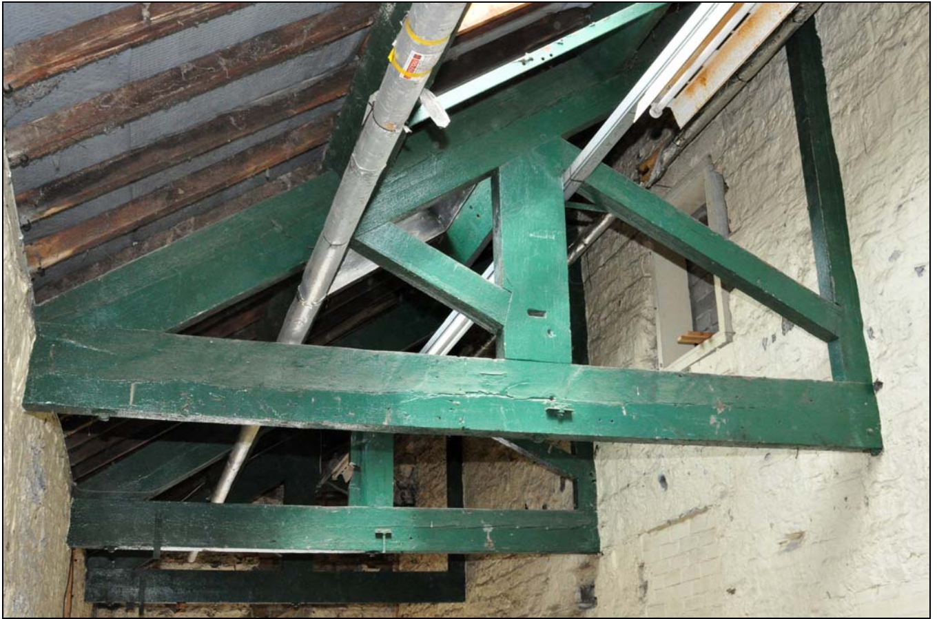
Photo 43: Roof trusses over boiler house, from the south-east
