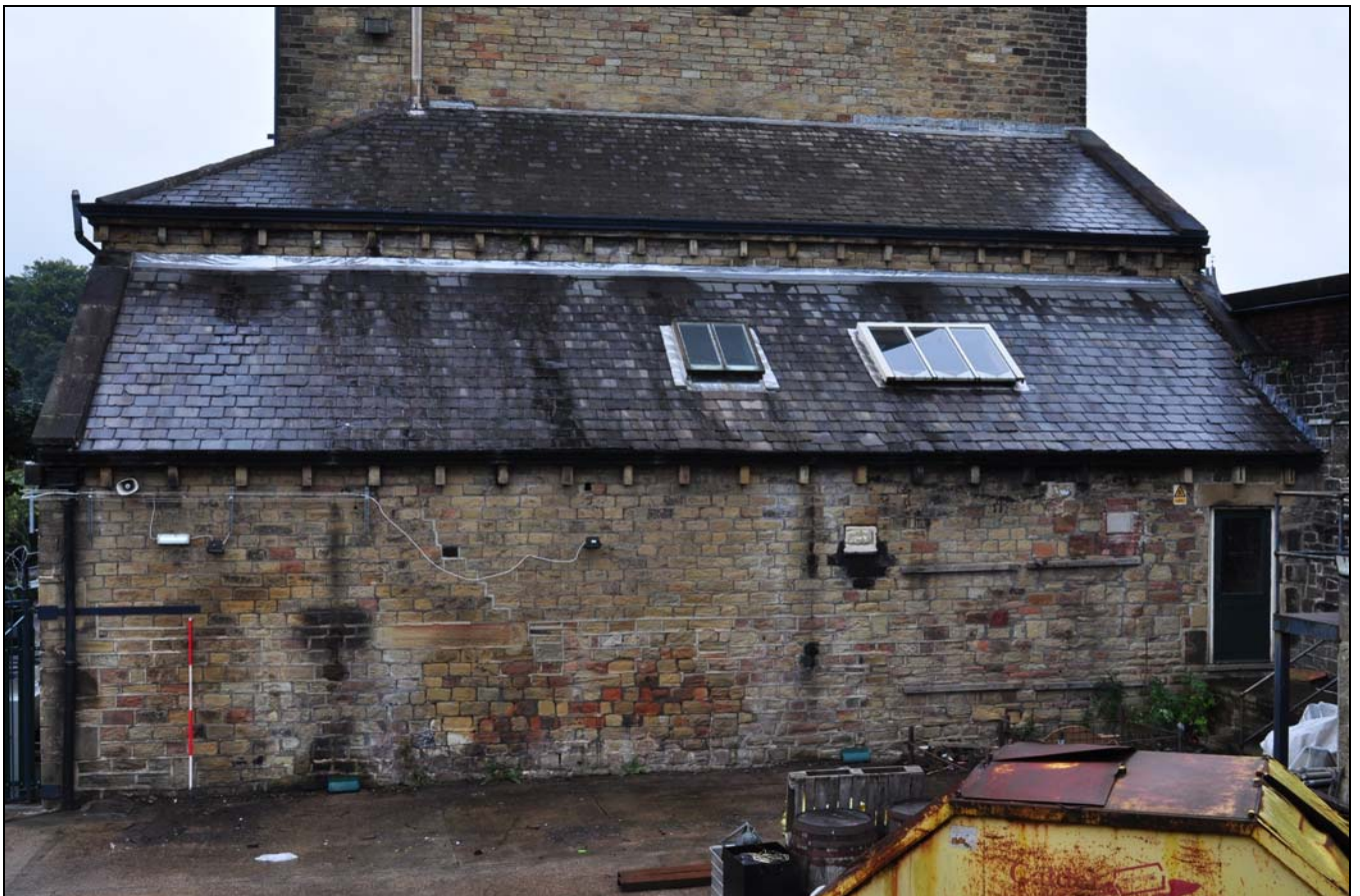
Photo 10: South-west side of boiler house with engine house and mill behind
