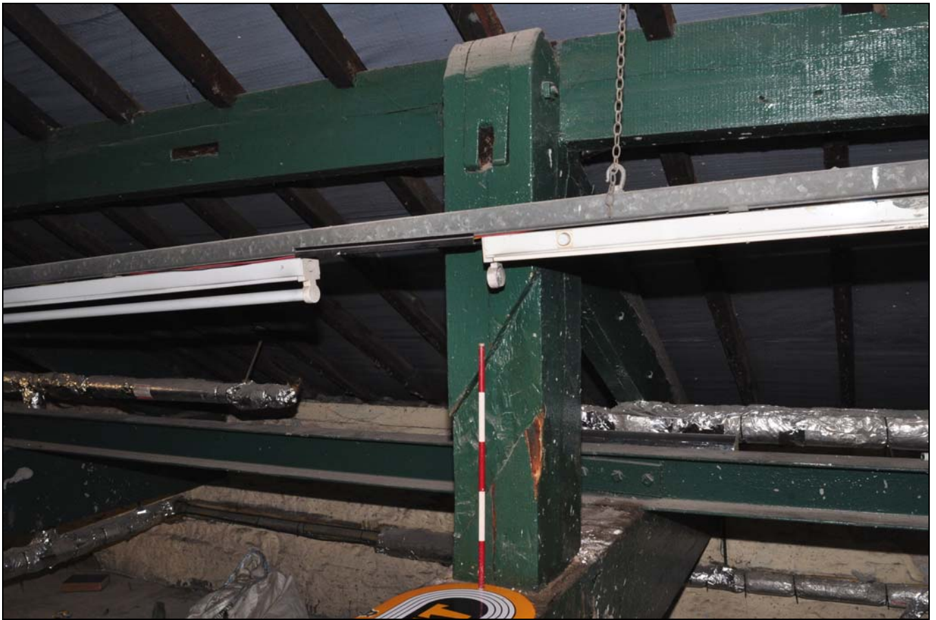
Photo 67: Large post on tie beam over engine house (part of rope race enclosure?), from the north
