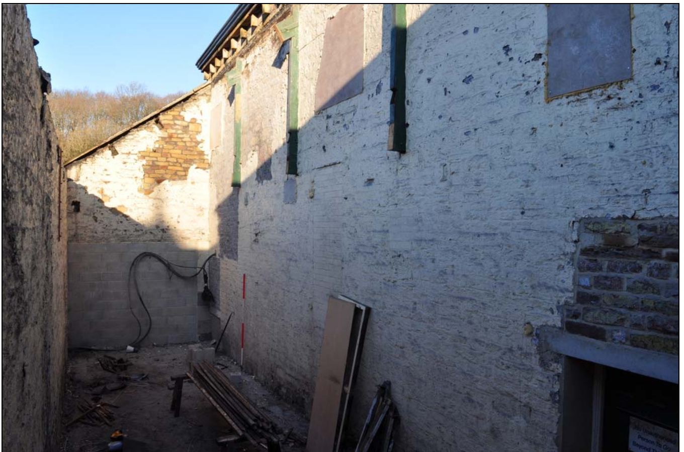
Photo 36: Interior of boiler house: north-east side, from the south (during demolition)
