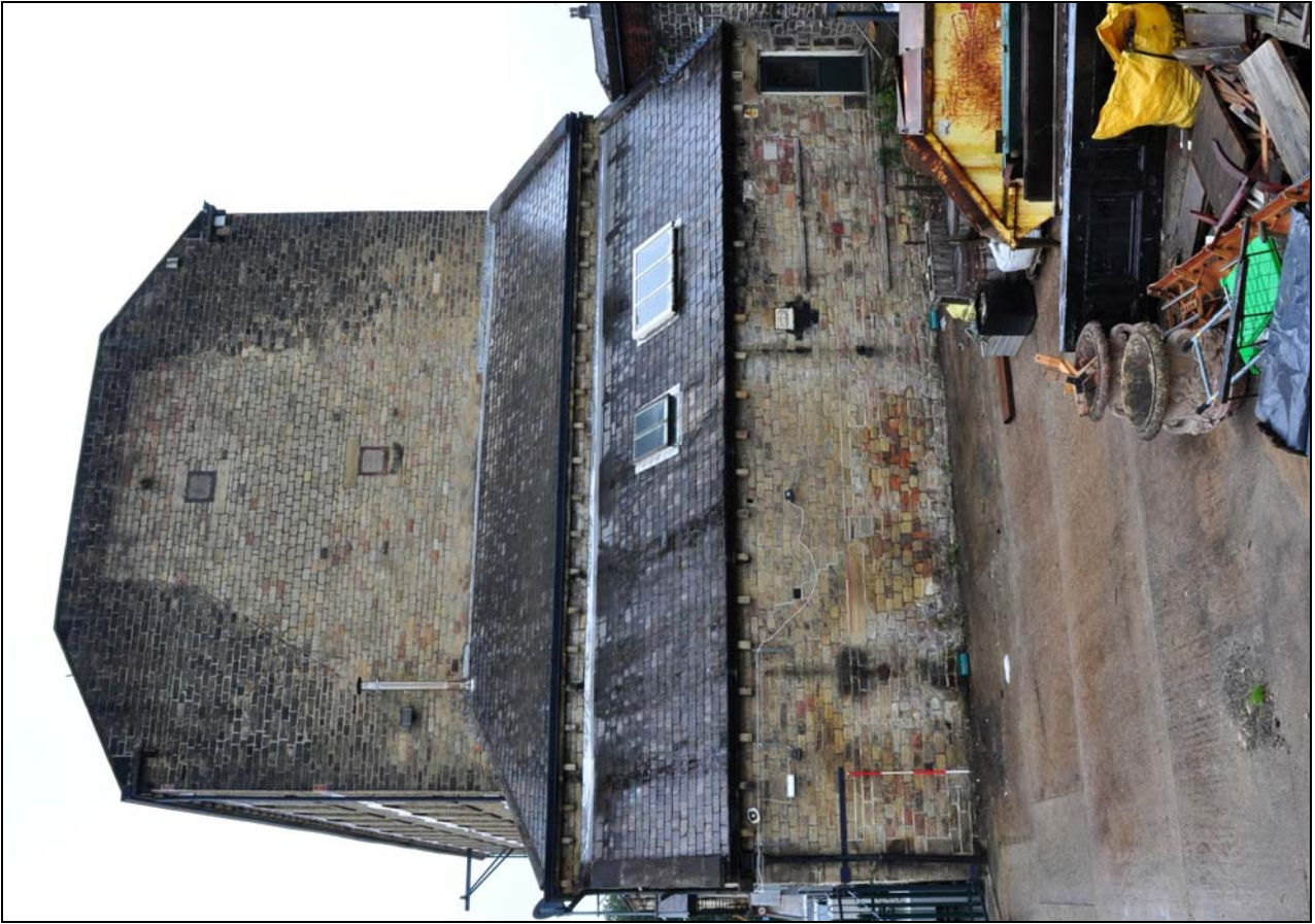
Photo 19: Engine and boiler houses with end of mill behind, with outline of former rope race, from the south-west
