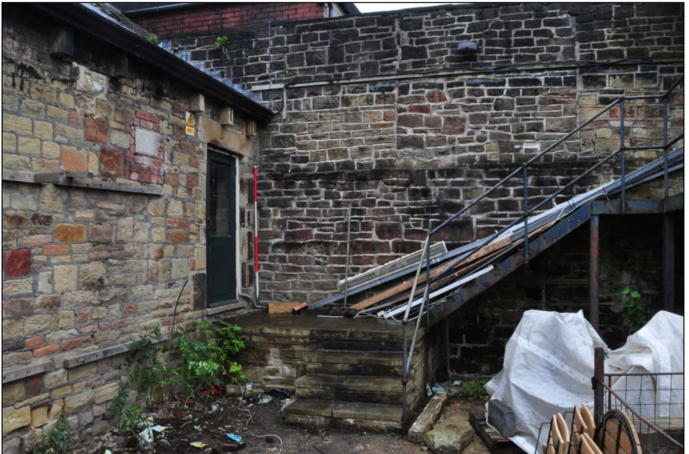
Photo 16: South-west side of boiler house, at junction with retaining wall
