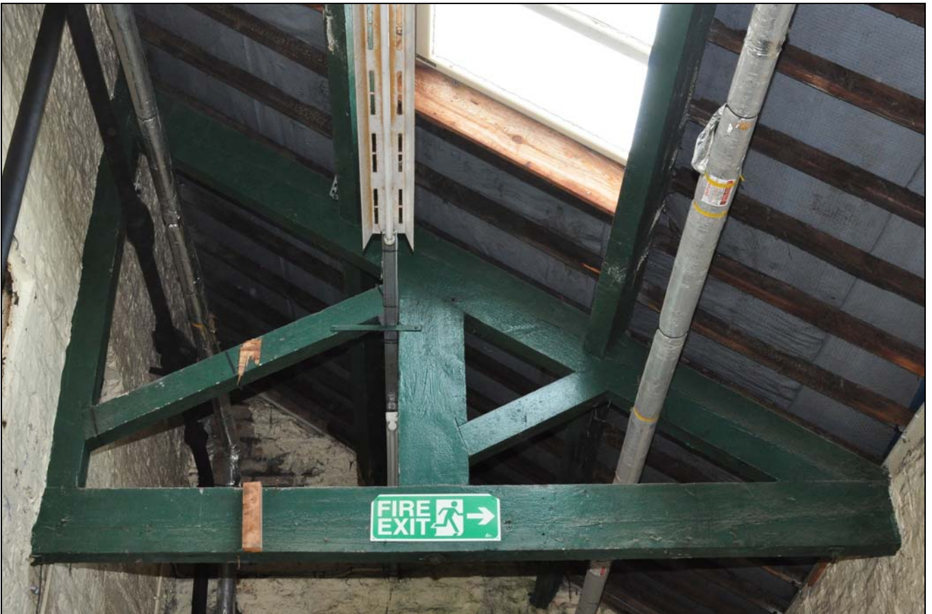
Photo 42: Roof truss over boiler house, from the north-west
