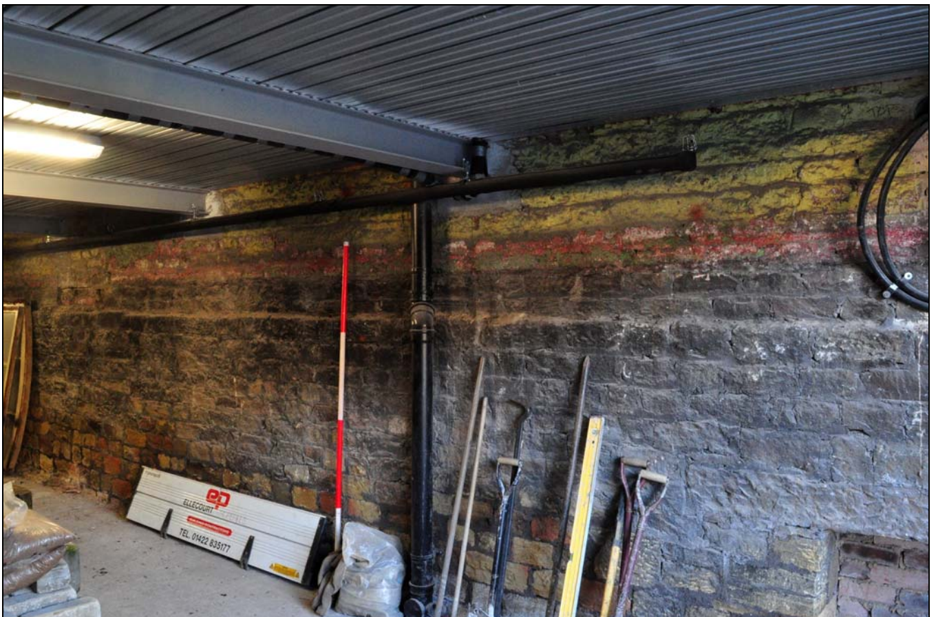
Photo 58: Ground floor of engine house, south-west side, from the north
