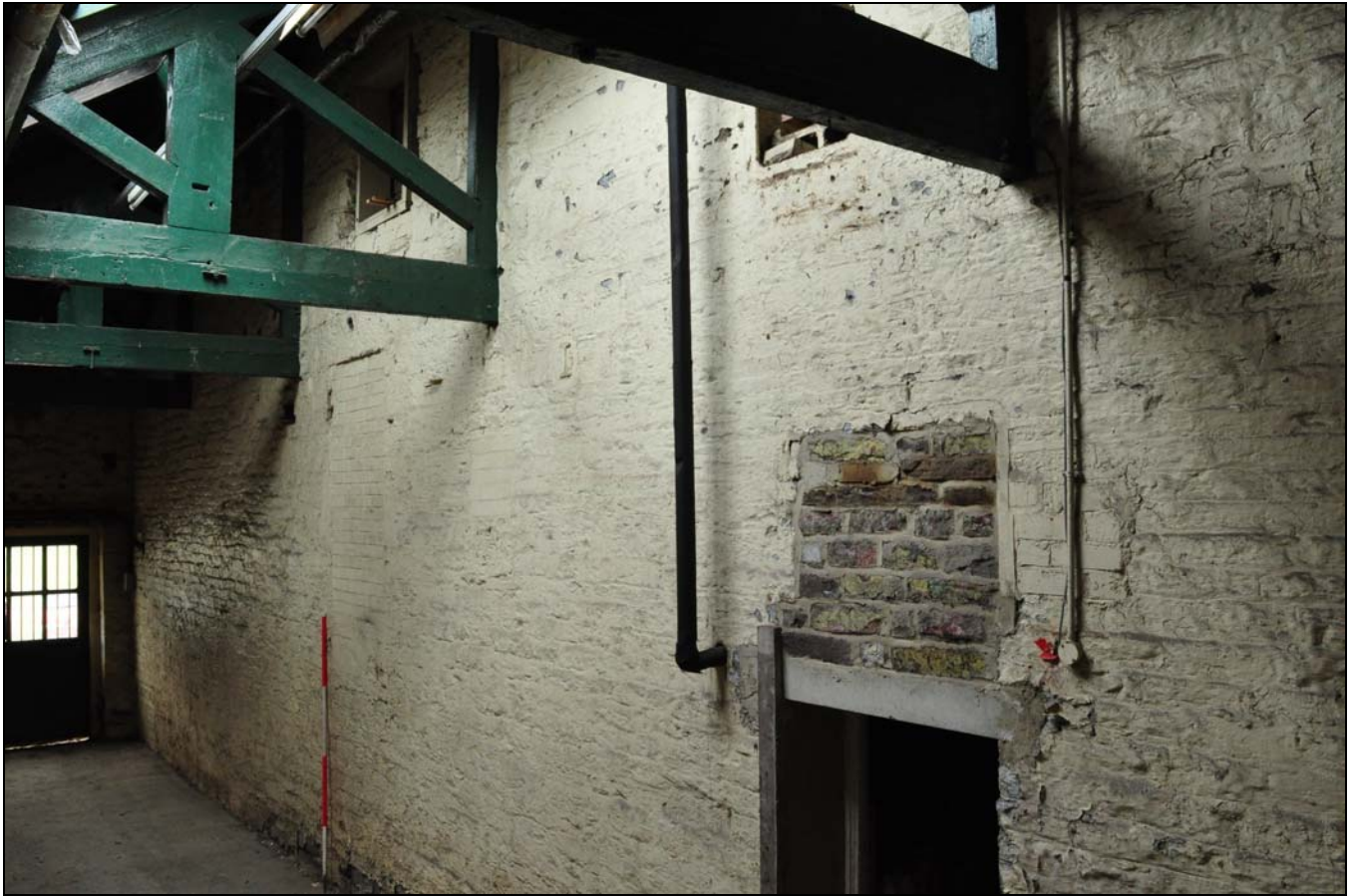
Photo 35: Interior of boiler house: north-east side, from the south
