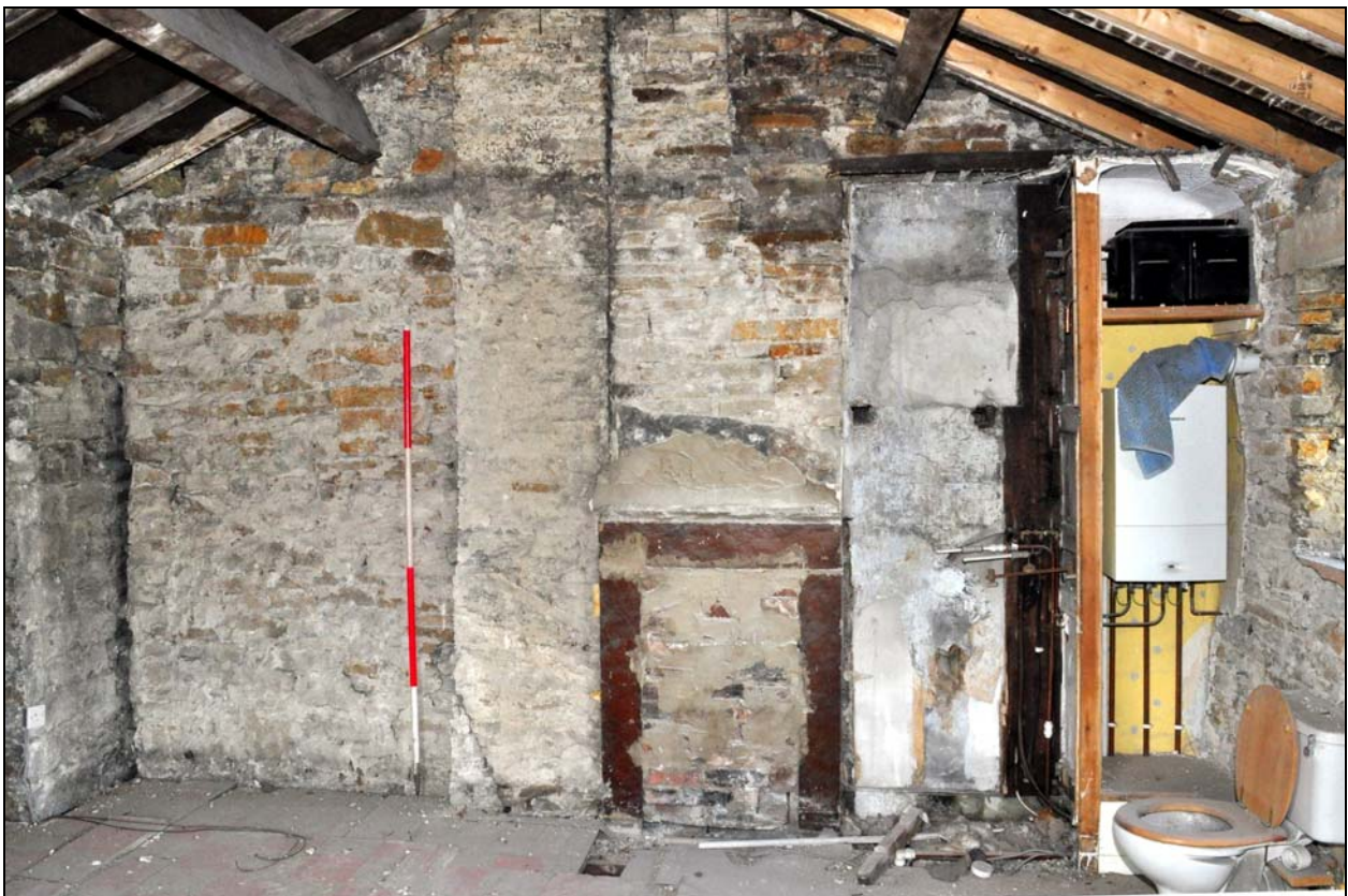
Photo 28: First floor of nineteenth century extension, looking south-west
