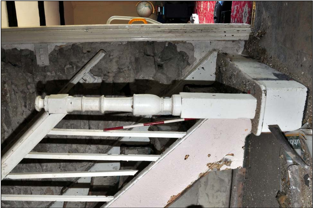
Photo 19: Ground floor room in front part of cottage: detail of stairs
