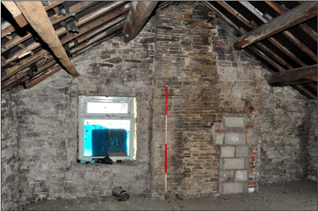
Photo 25: First floor room in front part of cottage, looking north-east towards widened chimney-breast
