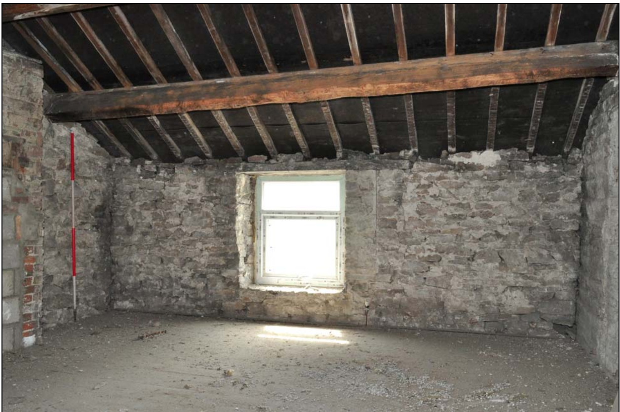
Photo 24: First floor room in front part of cottage, looking south-east
