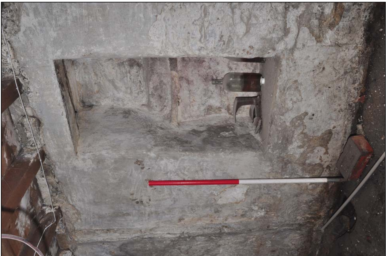
Photo 21: Cellar: recesses and scar of cross-wall, in south-east side
