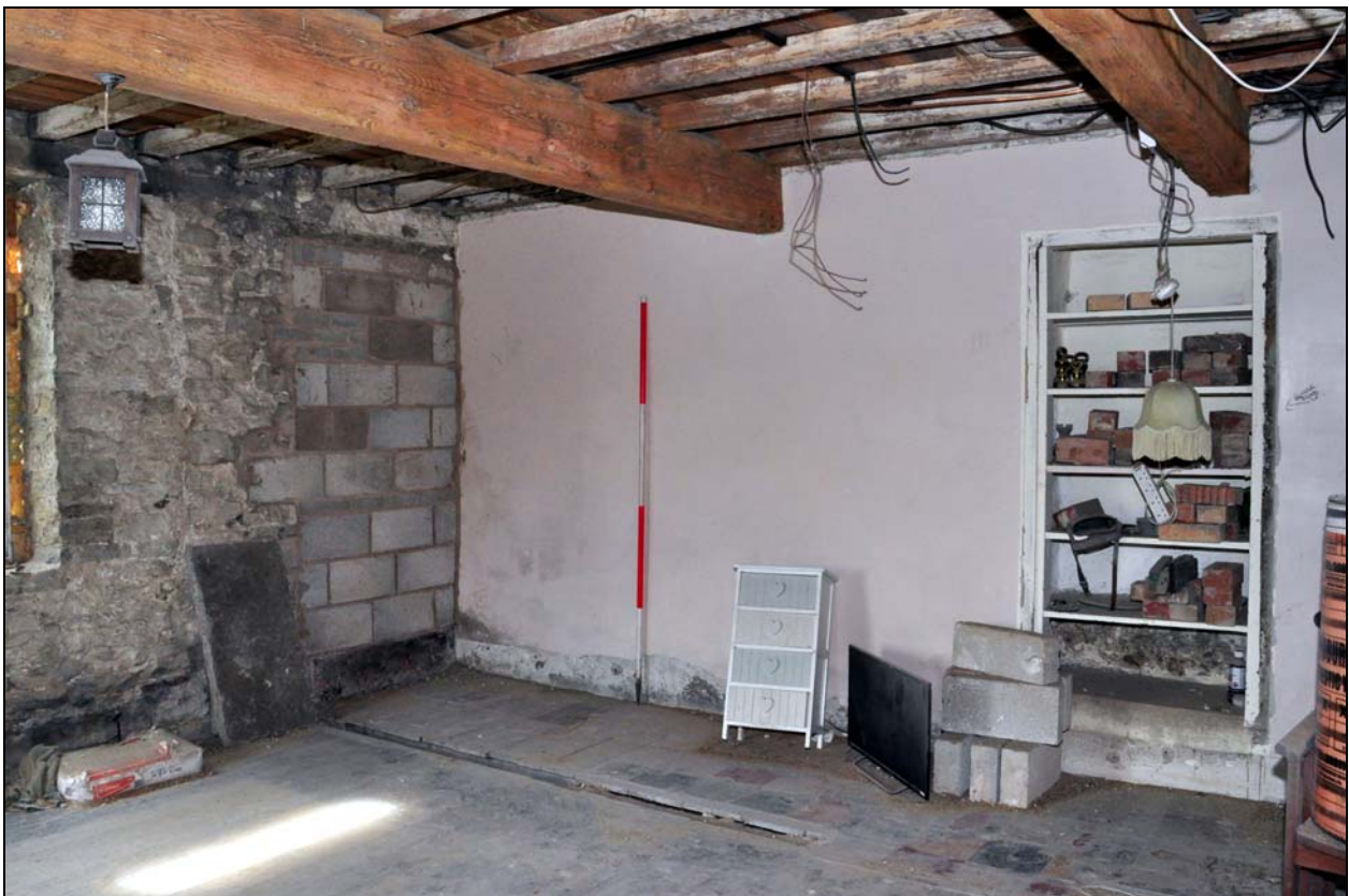
Photo 16: Ground floor room in front part of cottage, looking south
