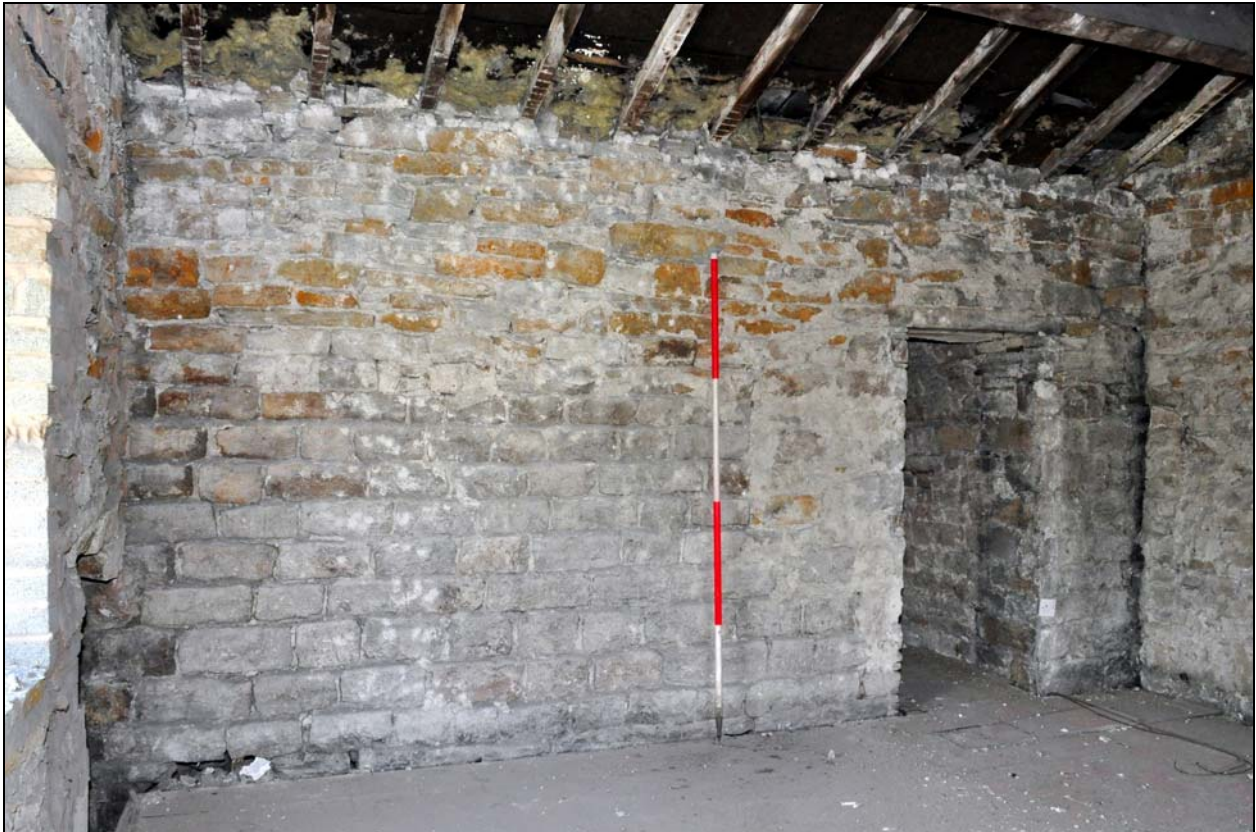
Photo 29: First floor of nineteenth century extension, looking south-east
