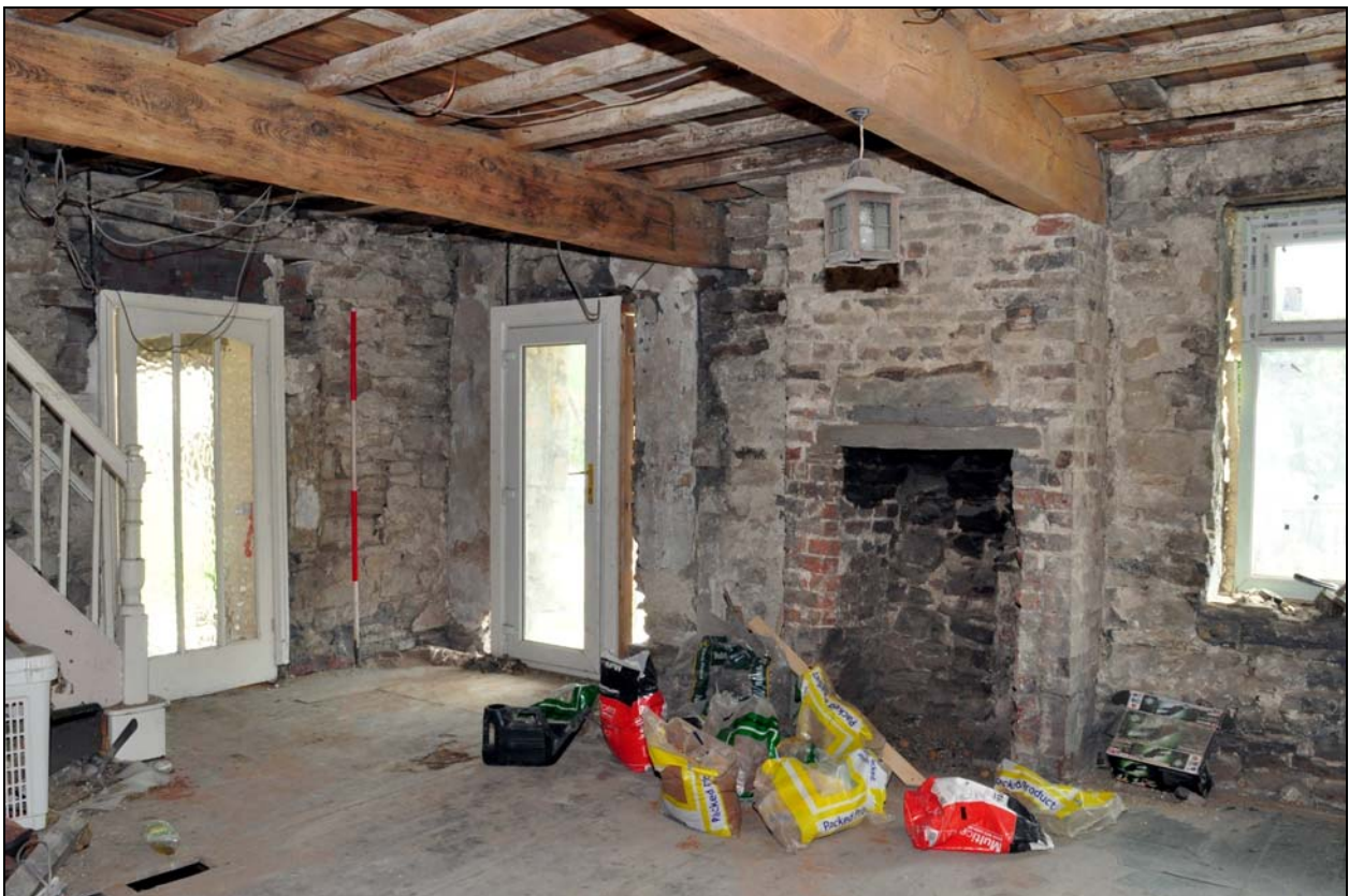
Photo 14: Ground floor room in front part of cottage, looking north
