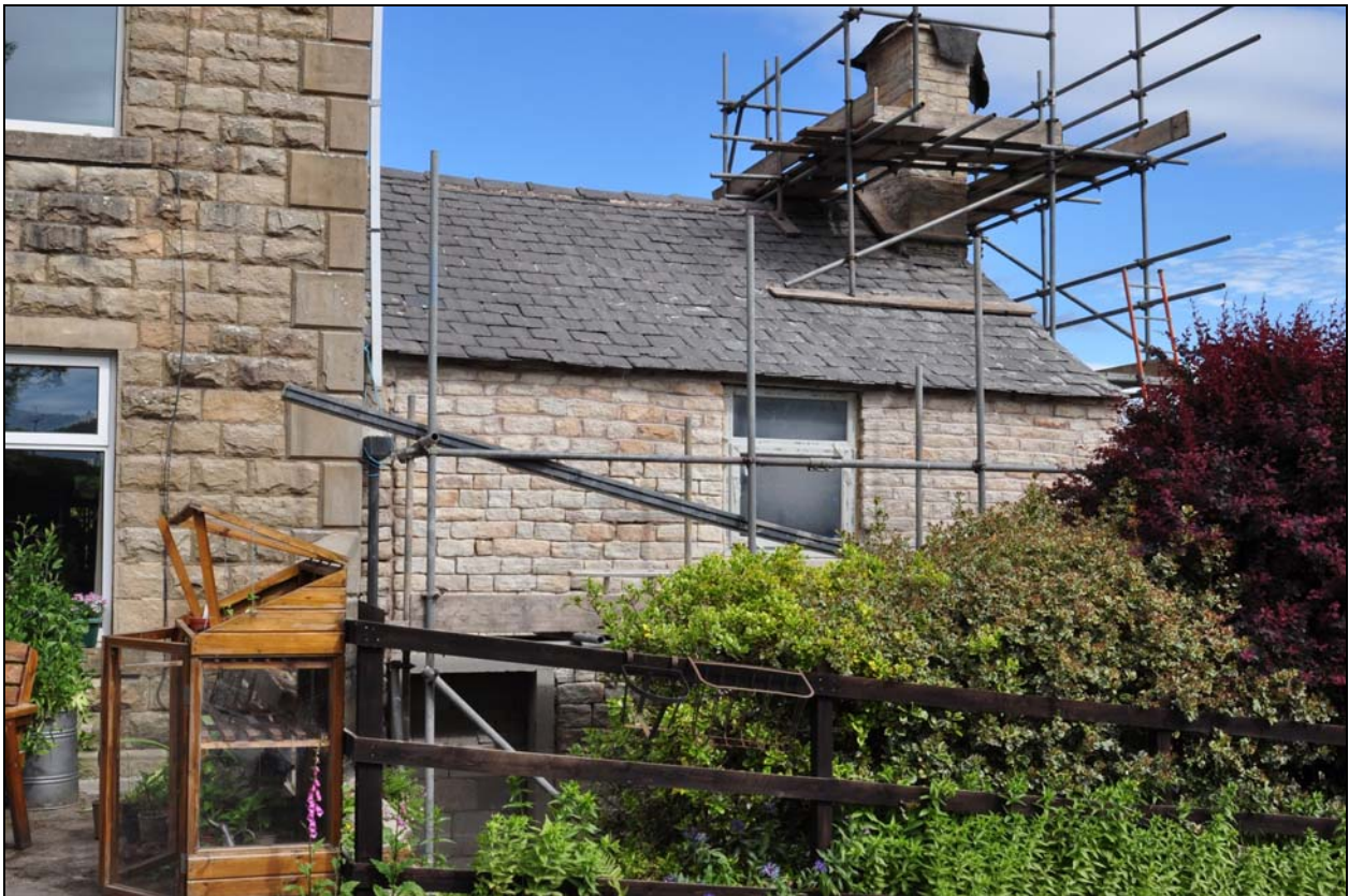
Photo 2: Front elevation of cottage
