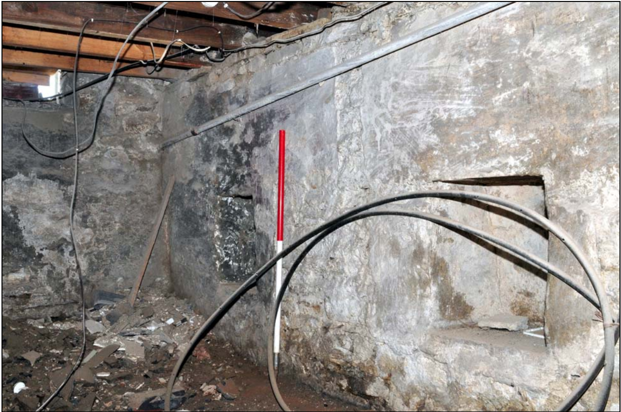
Photo 21: Cellar: recesses and scar of cross-wall, in south-east side
