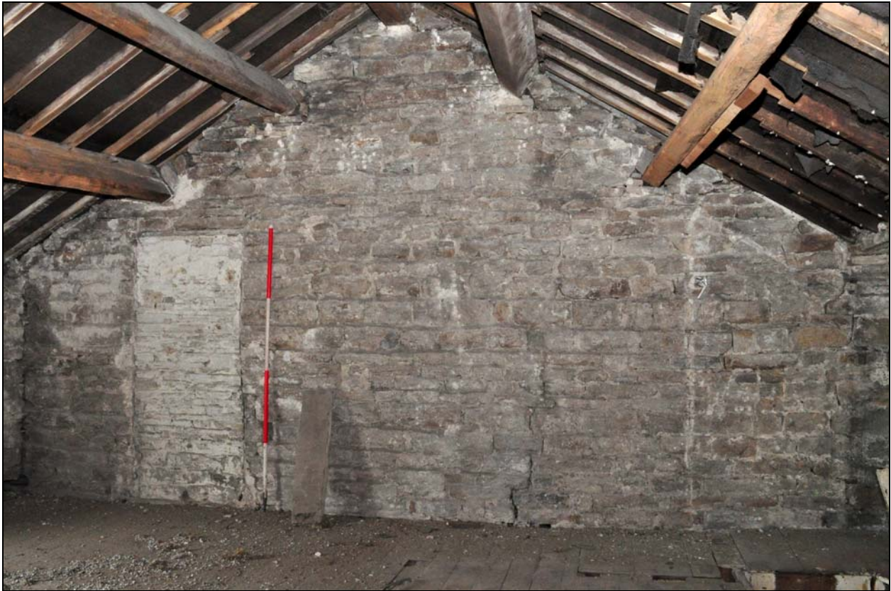
Photo 23: First floor room in front part of cottage: south-west side (former external wall face)
