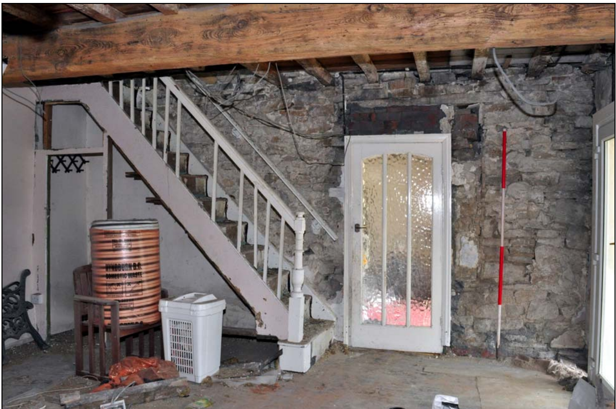
Photo 18: Ground floor room in front part of cottage, looking north-west
