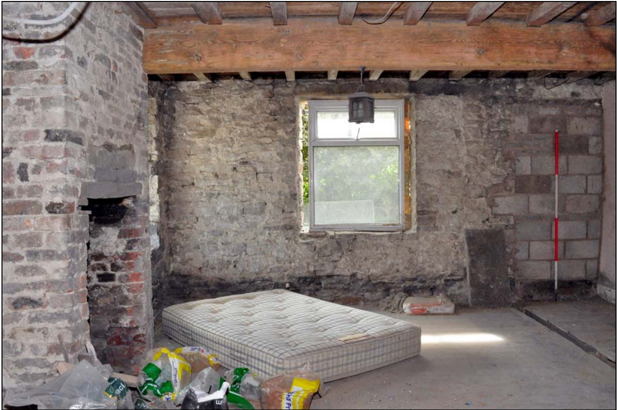
Photo 13: Ground floor room in front part of cottage, looking south-east
