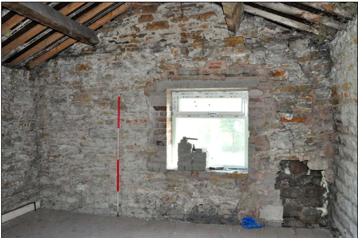
Photo 30: First floor of nineteenth century extension, looking north-east
