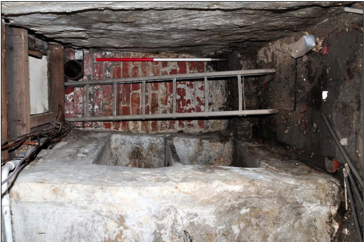
Photo 20: Cellar: looking south-west towards blocked doorway in wall with Farmhouse
