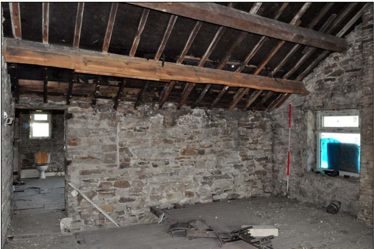
Photo 26: First floor room in front part of cottage, looking north
