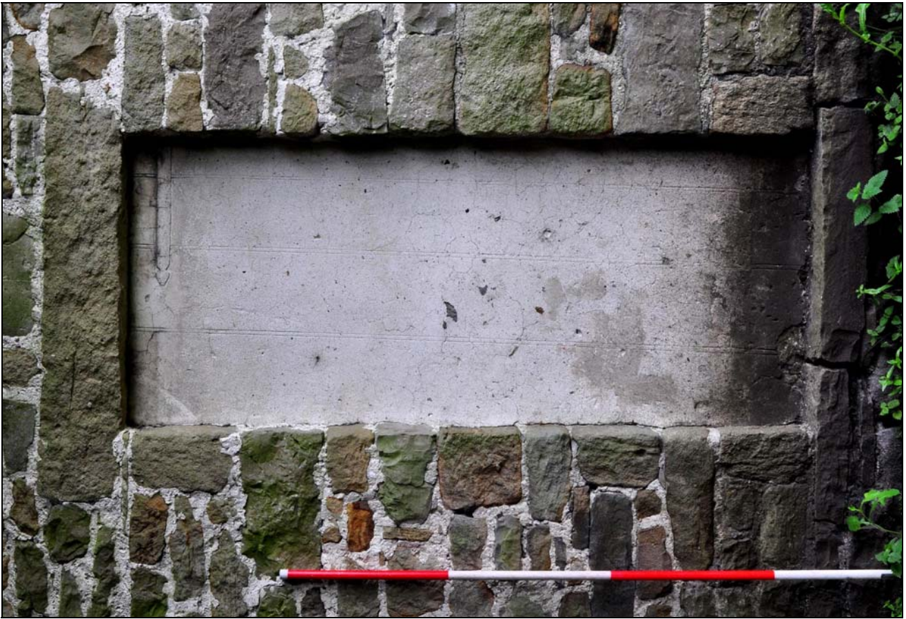
Photo 7: Detail of false doorway in front elevation (north)
