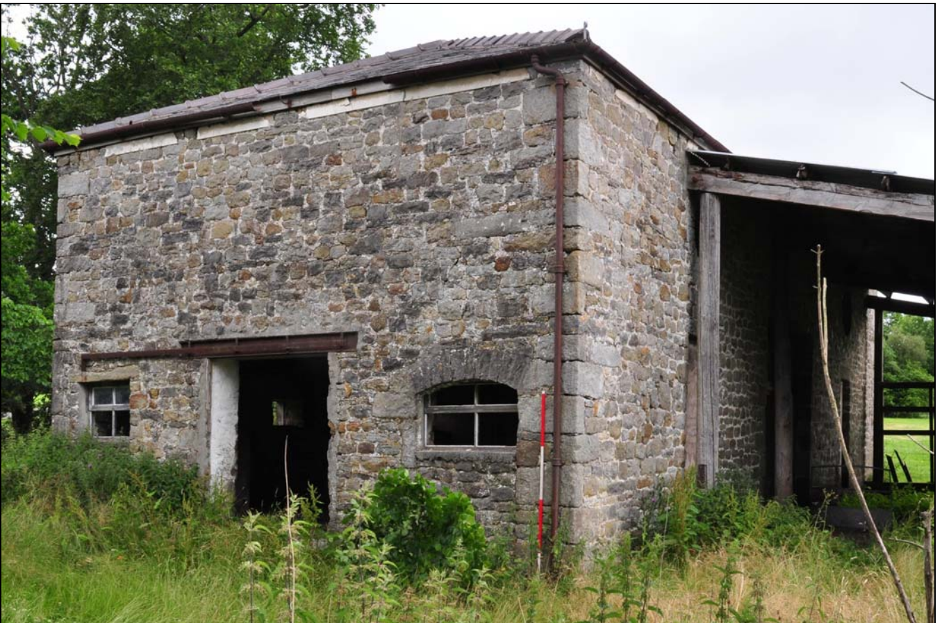
Photo 10: General view, from the south-east
