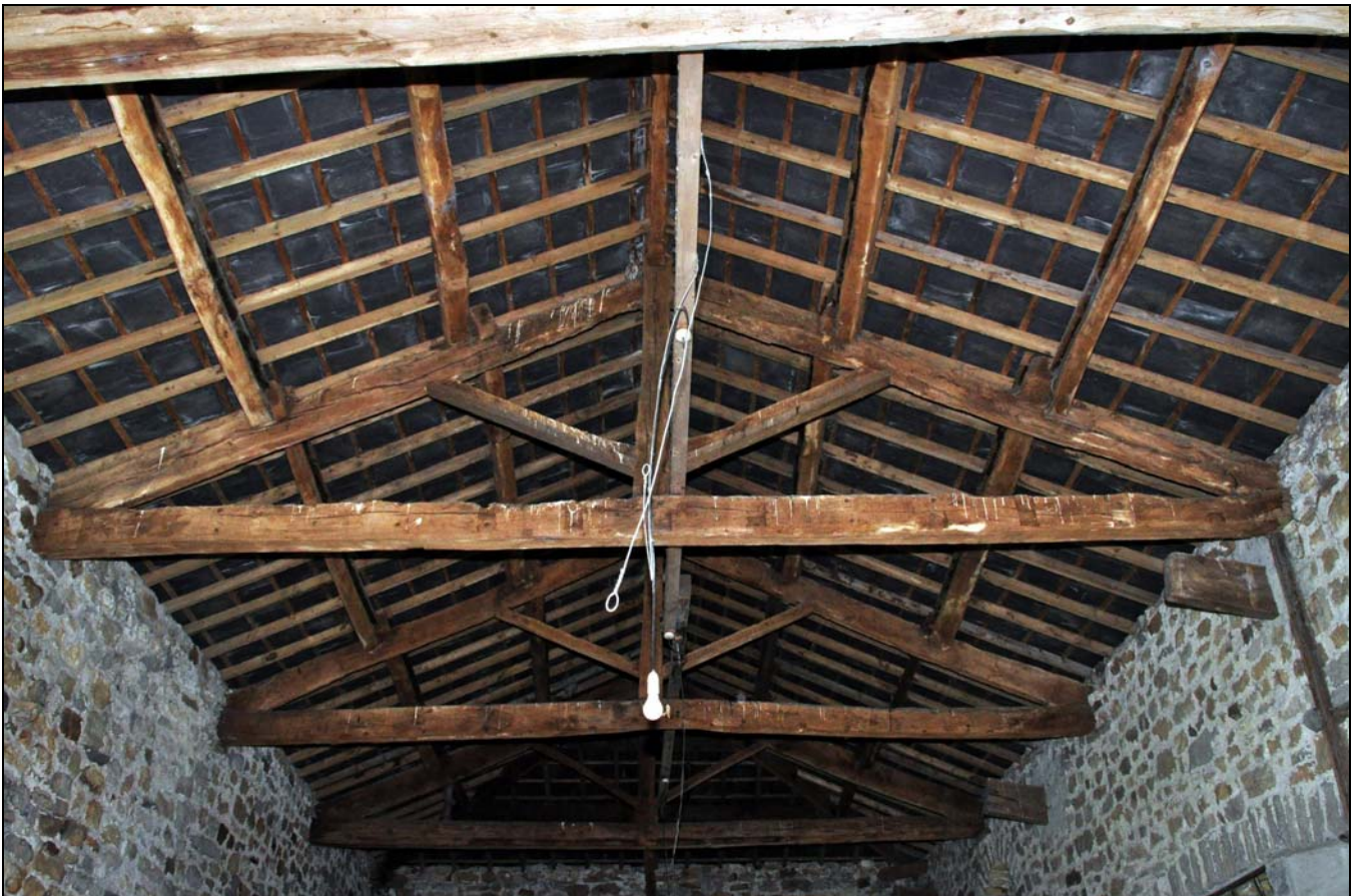
Photo 25: Interior: roof trusses, from the south
