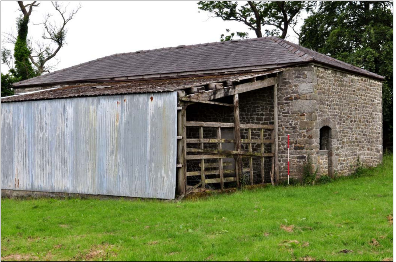
Photo 1: General view, from the north-east
