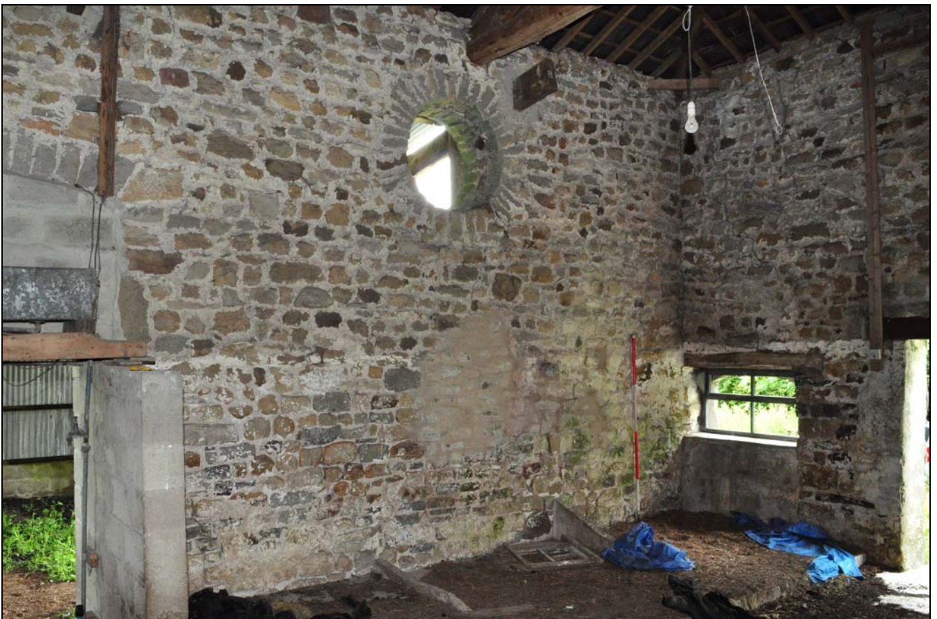
Photo 22: Interior: south-east corner
