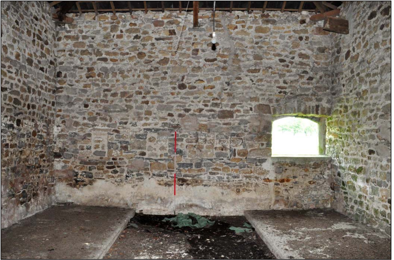
Photo 23: Interior: north end
