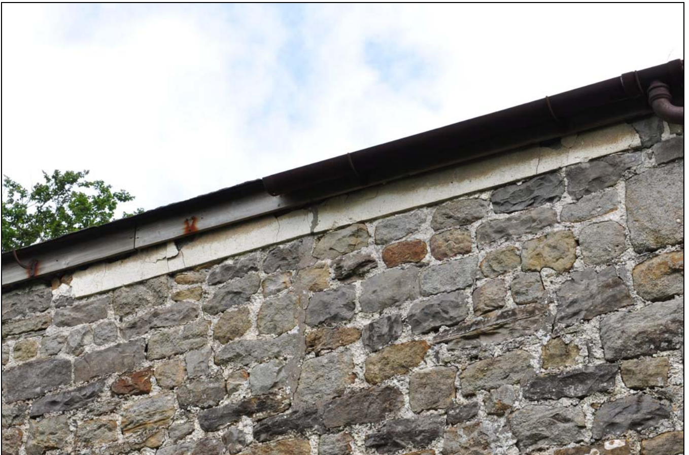
Photo 2: Detail of lime mortar strip at eaves
