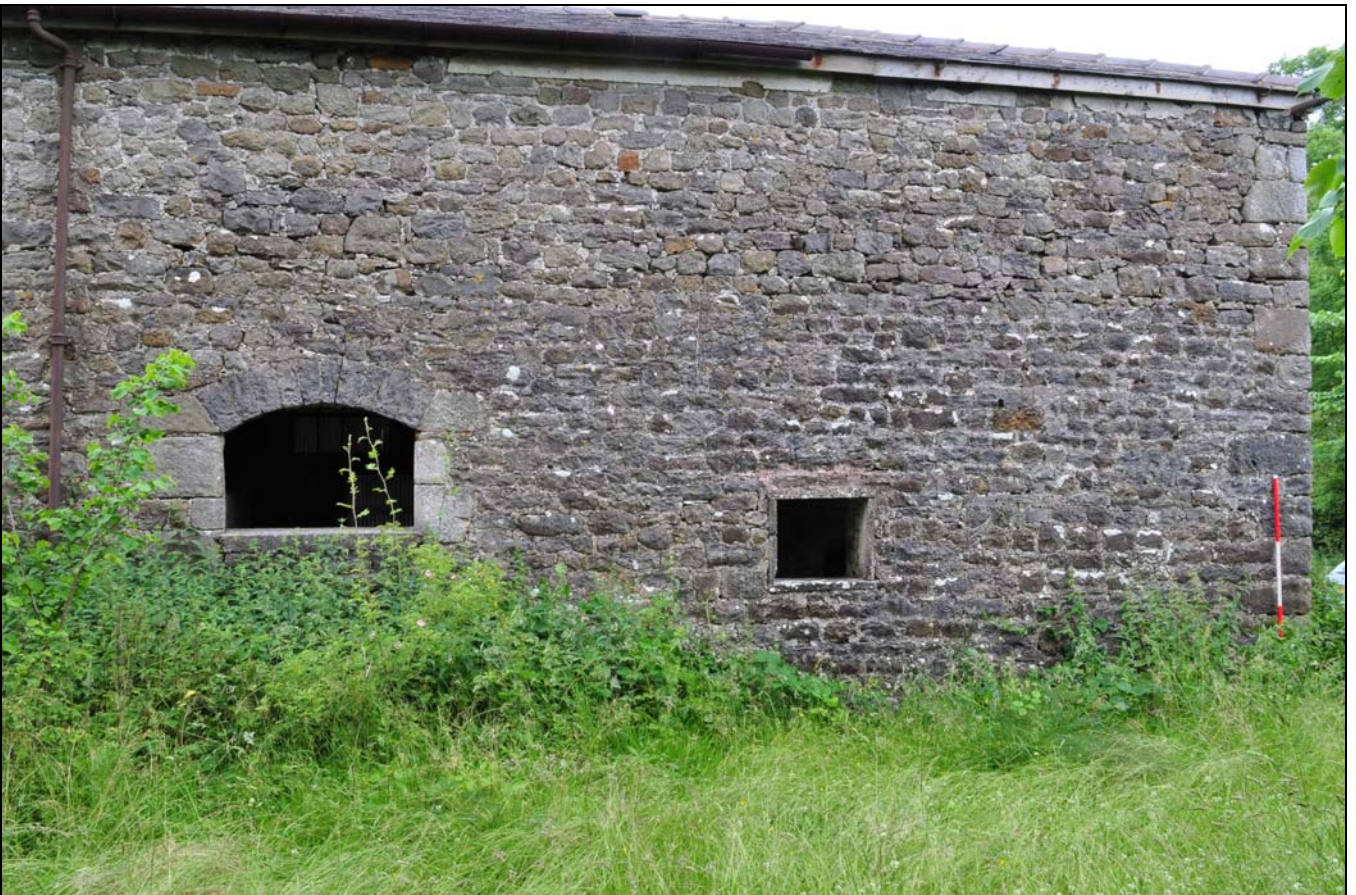
Photo 15: Winnowing doorway and smaller opening, rear elevation
