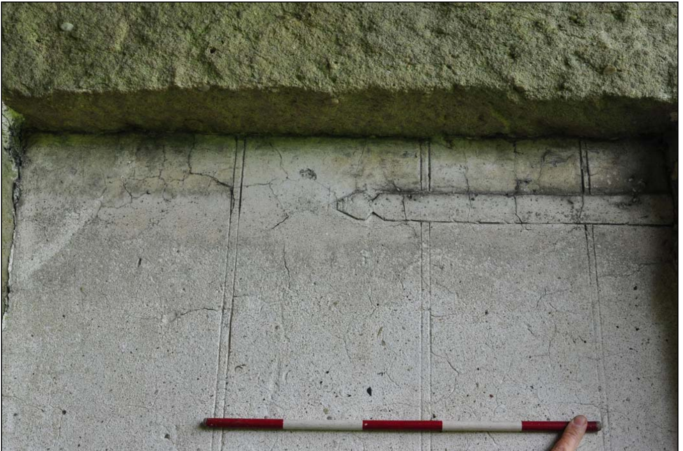
Photo 8: Detail of false doorway in front elevation (north)
