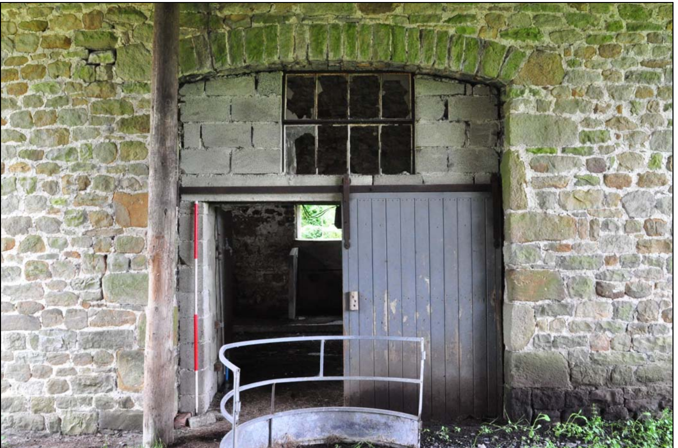
Photo 5: Detail of cart entrance in front elevation
