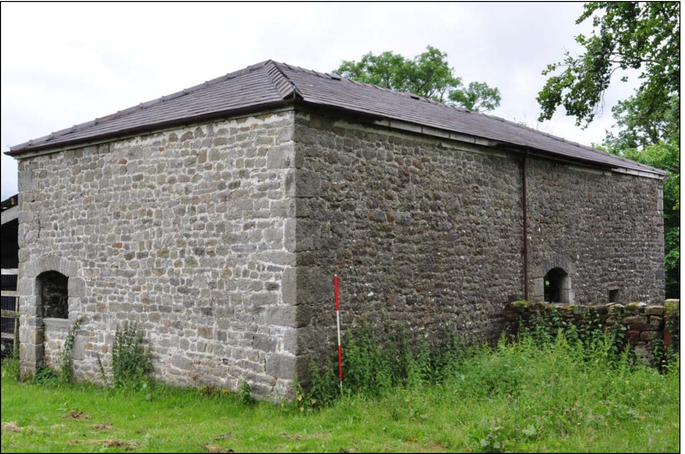
Photo 14: Rear elevation, from the north-west
