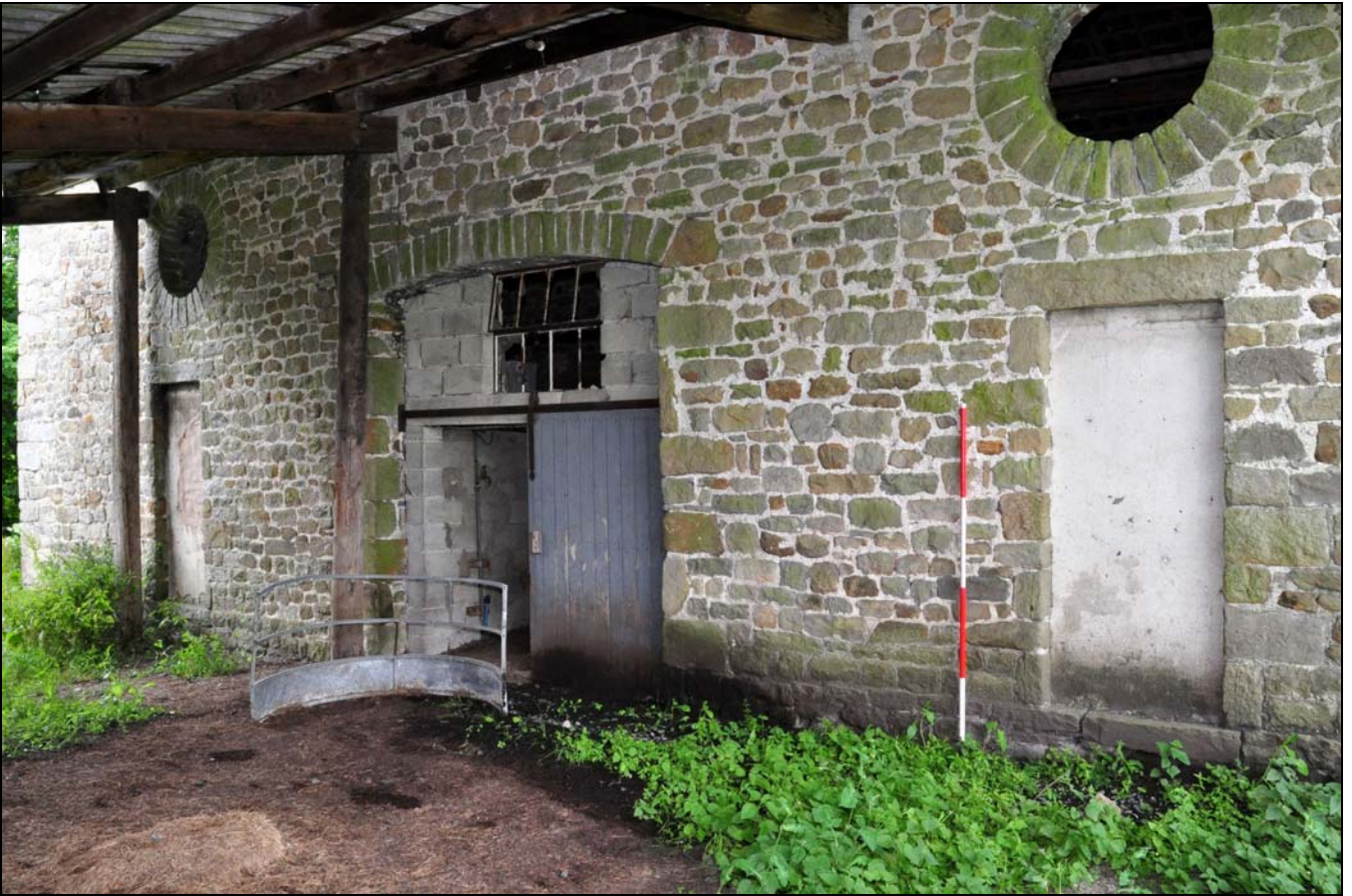
Photo 4: Front elevation, from the north-east
