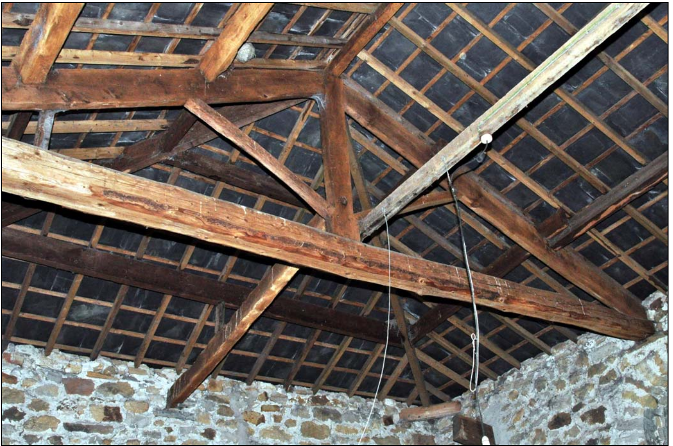
Photo 27: Interior: north roof truss
