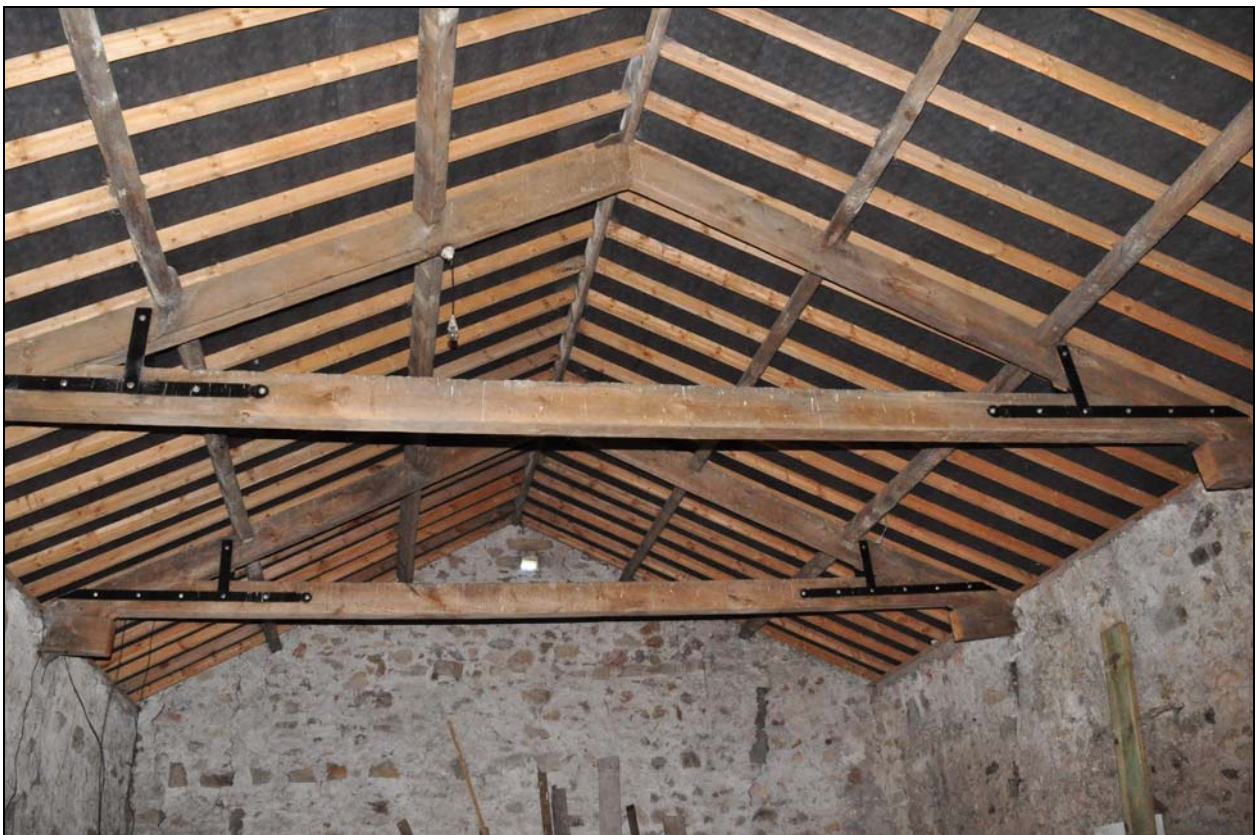
Photo 38: Roof over hayloft, looking east
