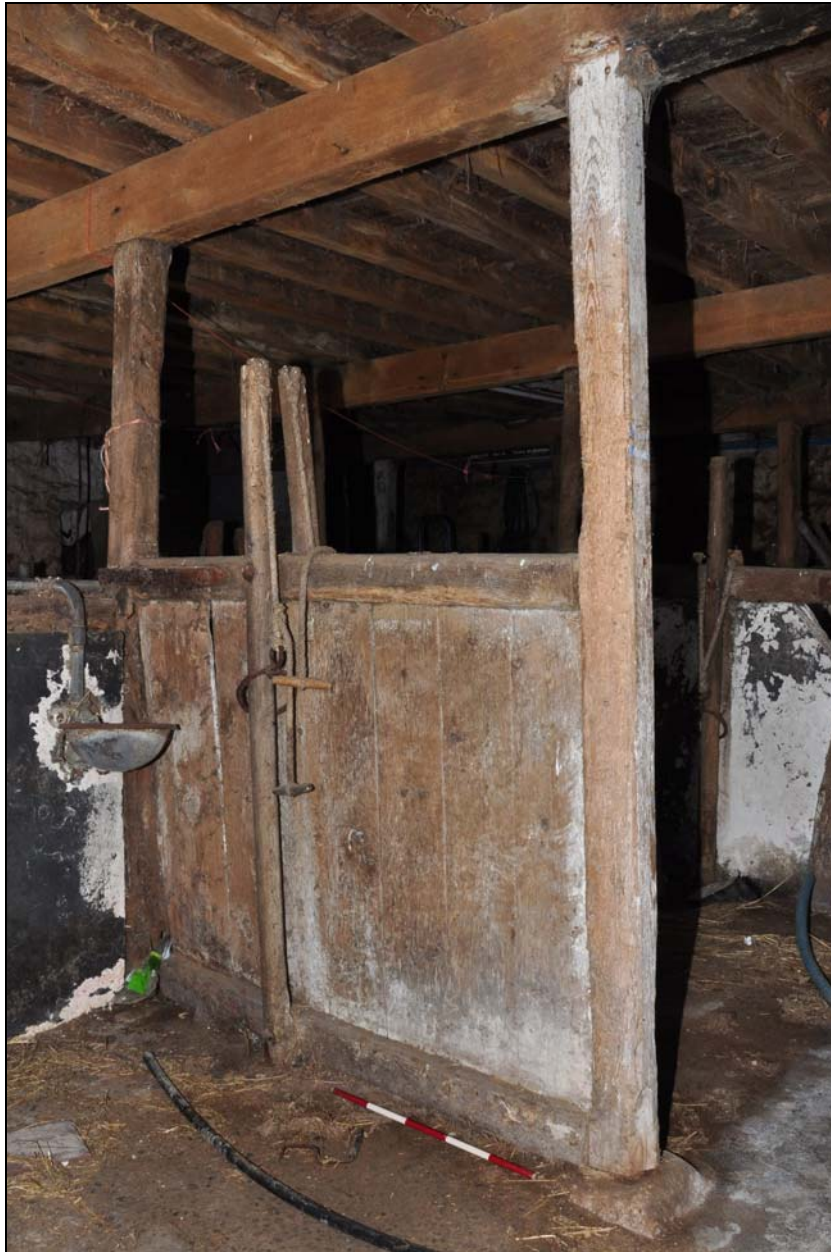
Photo 21: Shippon: stalls in east side, looking north-west
