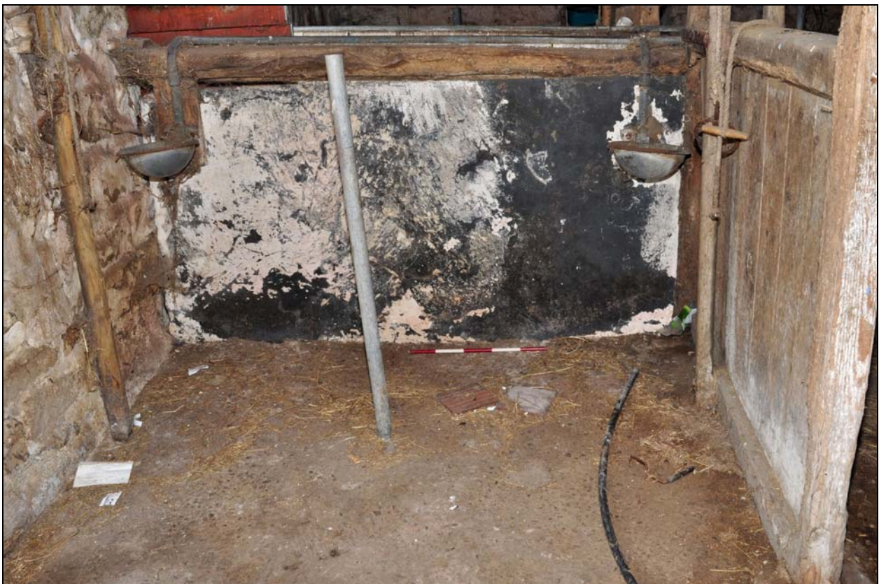
Photo 20: Shippon: stalls in east side, looking west
