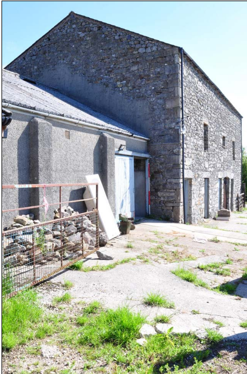
Photo 9: General view of the barn, from the south-west
