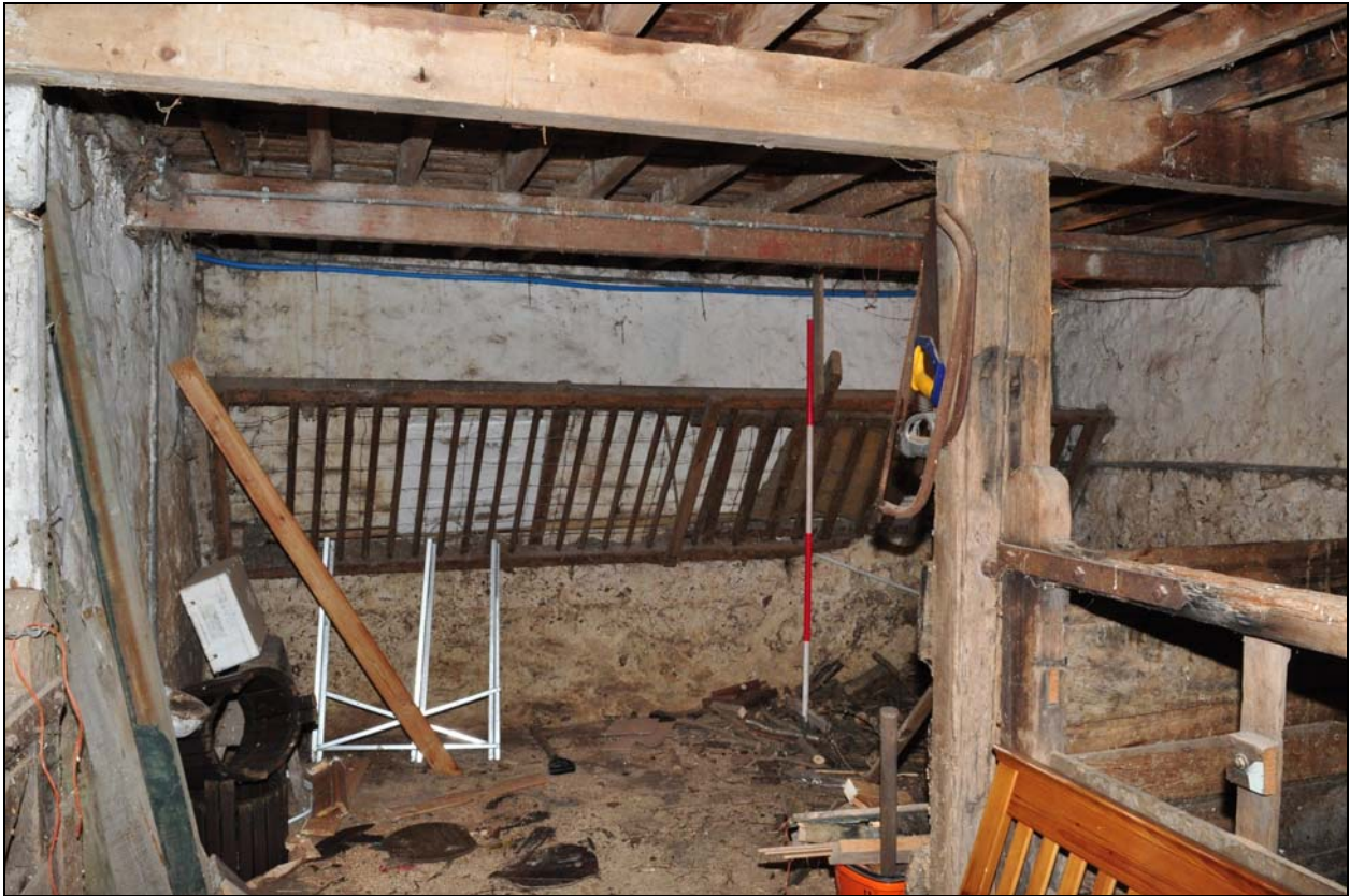
Photo 31: Former stable, looking north
