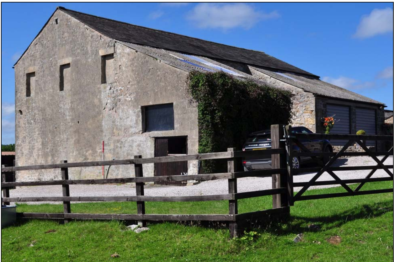
Photo 8: General view of the barn, from the north-east
