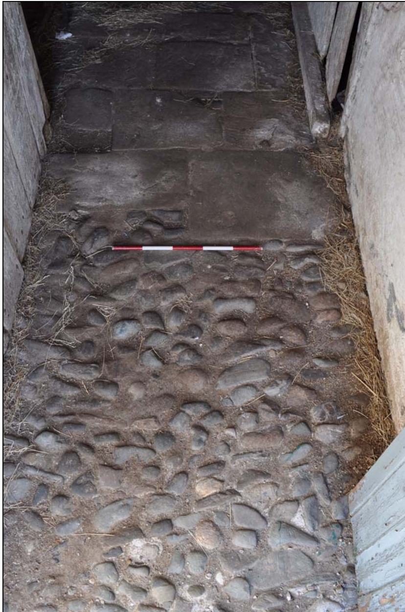
Photo 17: Shippon: cobbles and flagstones to feeding passage
