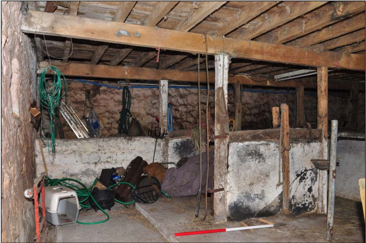
Photo 23: Shippon: stalls in west side, looking north-east
