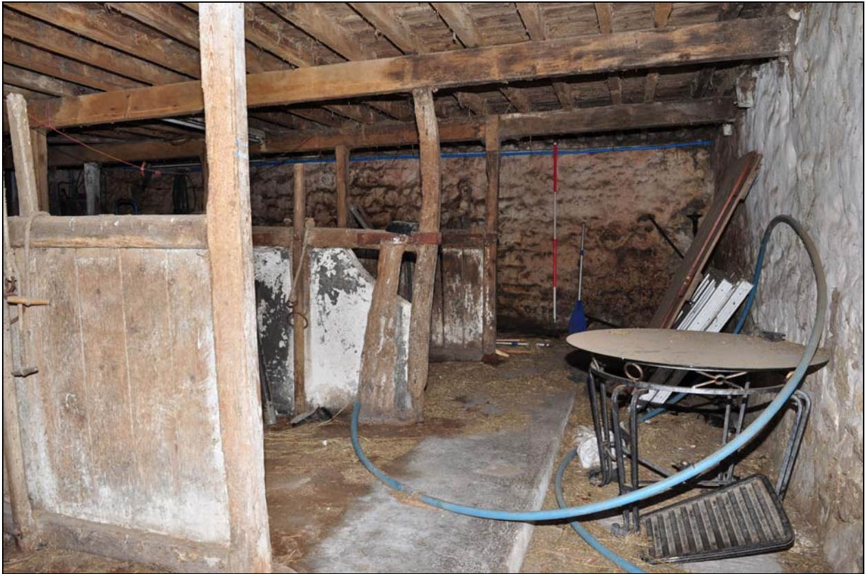
Photo 19: Shippon: stalls in east side, looking north-west
