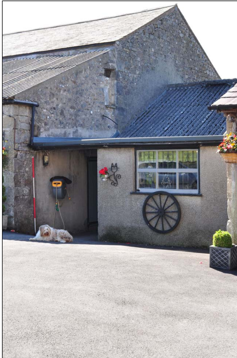
Photo 10: General view of the barn, from the north-west
