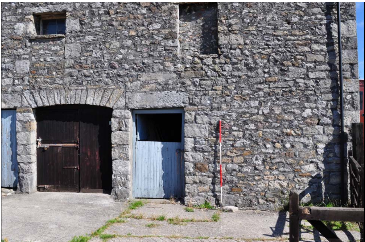
Photo 6: South elevation: doorways to cart bay and stable
