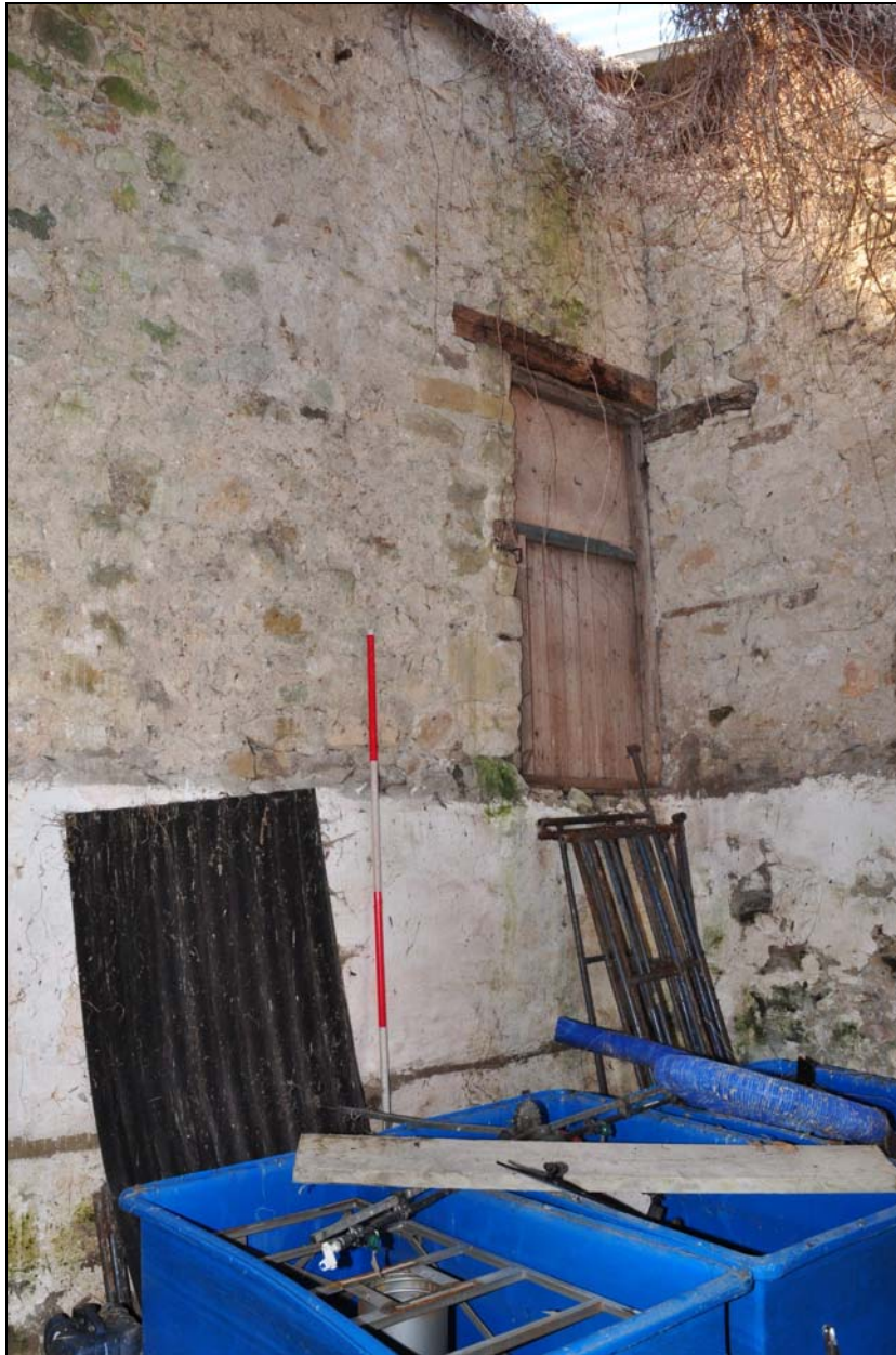
Photo 15: Interior of north-east outshut: inserted hayloft doorway
