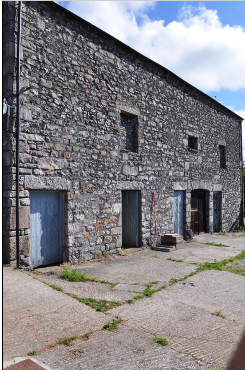
Photo 2: South elevation, from the south-west
