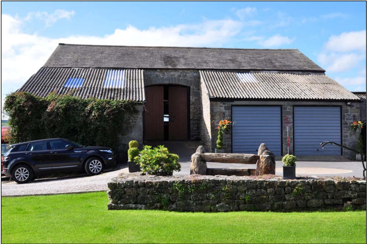
Photo 13: General view of the barn, from the north
