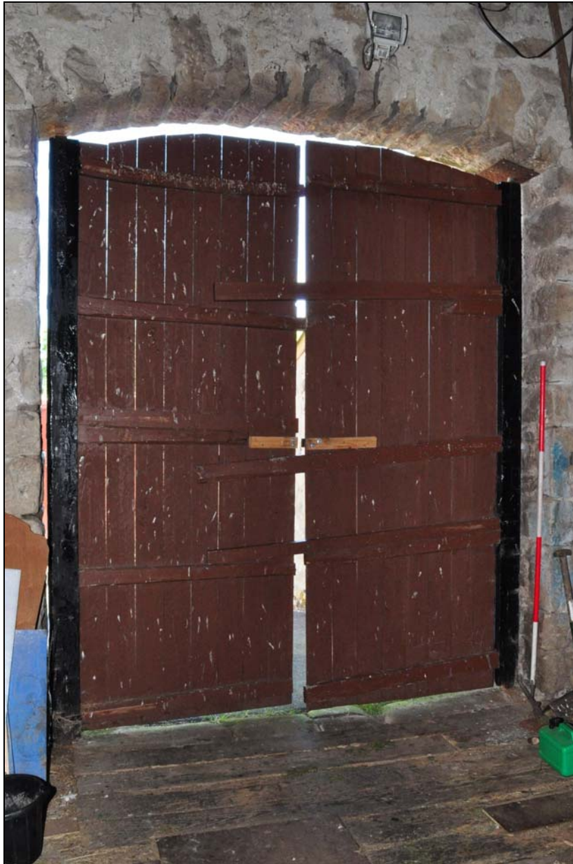
Photo 32: Hayloft: cart entry, looking north-east
