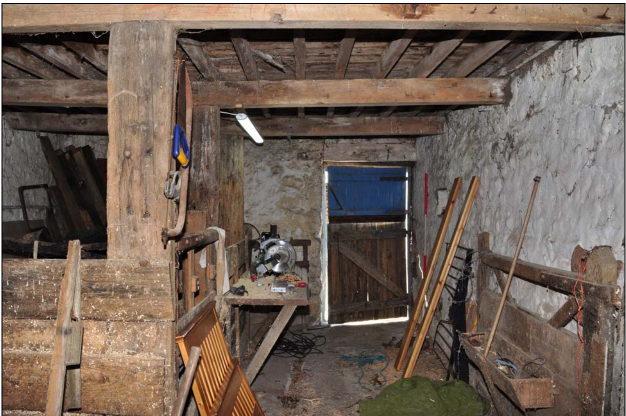
Photo 30: Former stable, looking south
