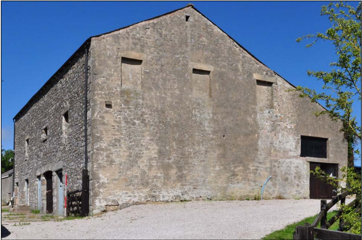
Photo 7: General view of the barn, from the south-east
