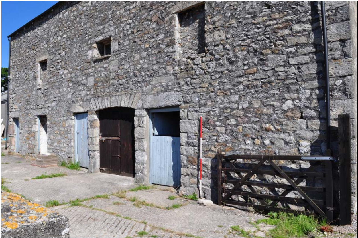
Photo 3: South elevation, from the south-east
