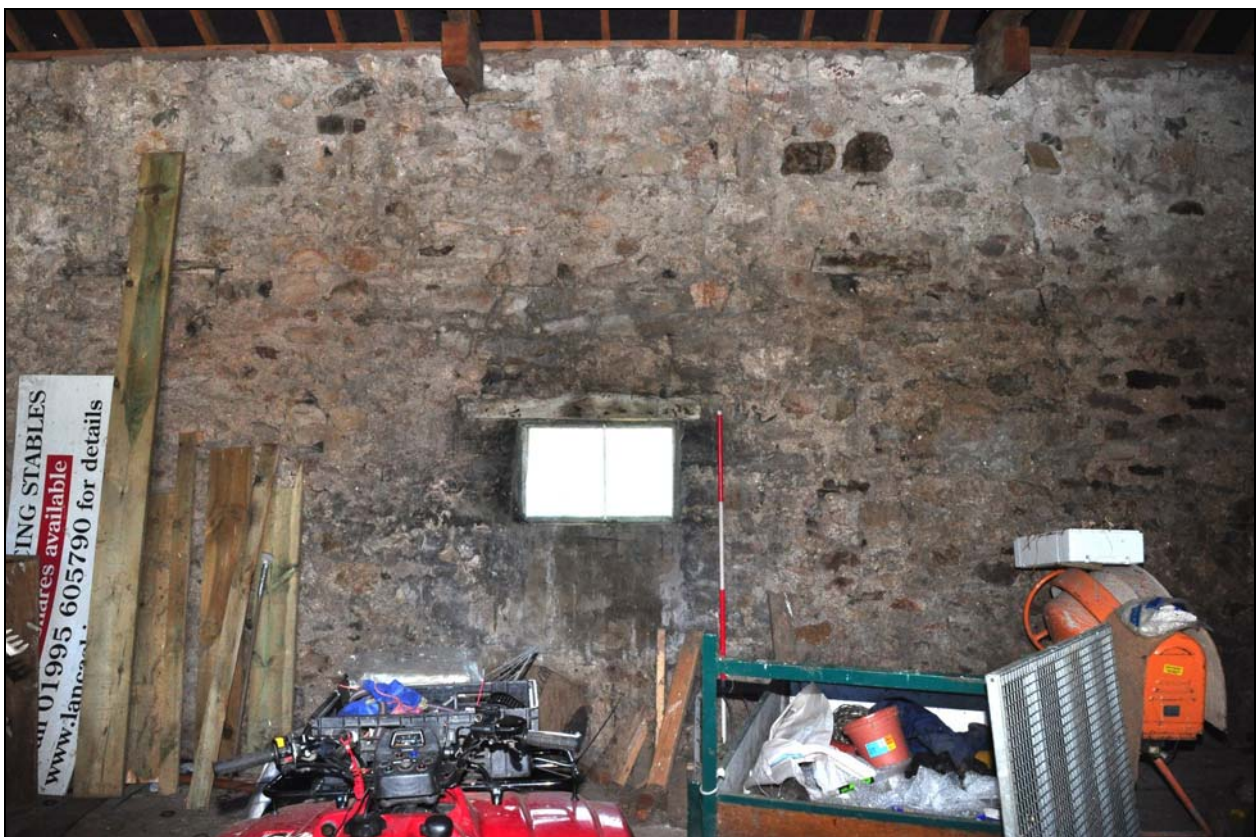
Photo 36: Hayloft, looking south towards former winnowing doorway
