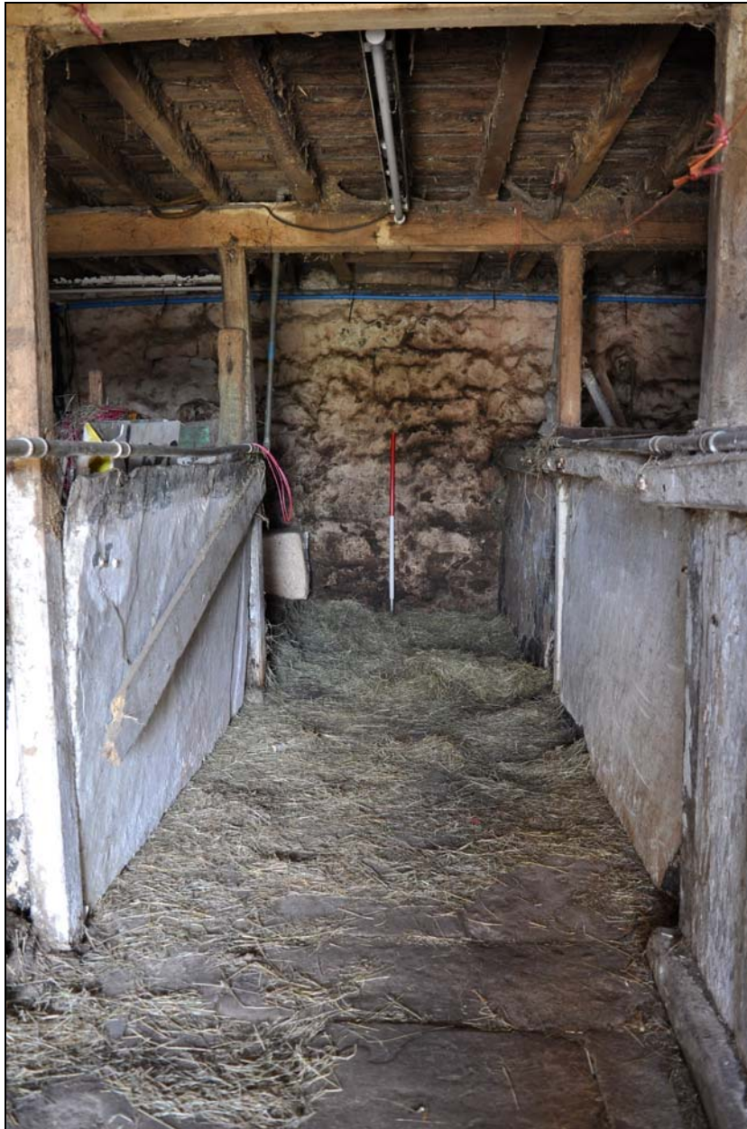
Photo 18: Shippon: feeding passage, looking north
