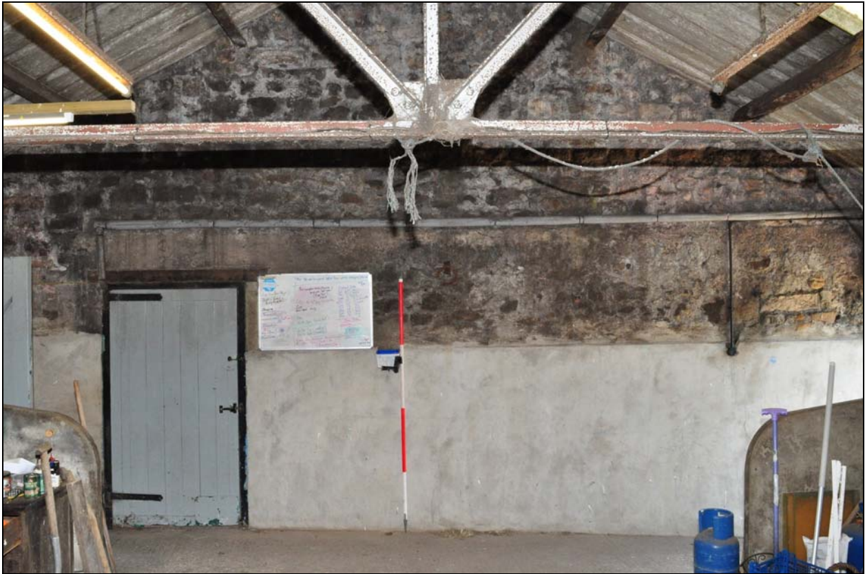
Photo 11: Inserted doorway in west gable, inside modern shippon
