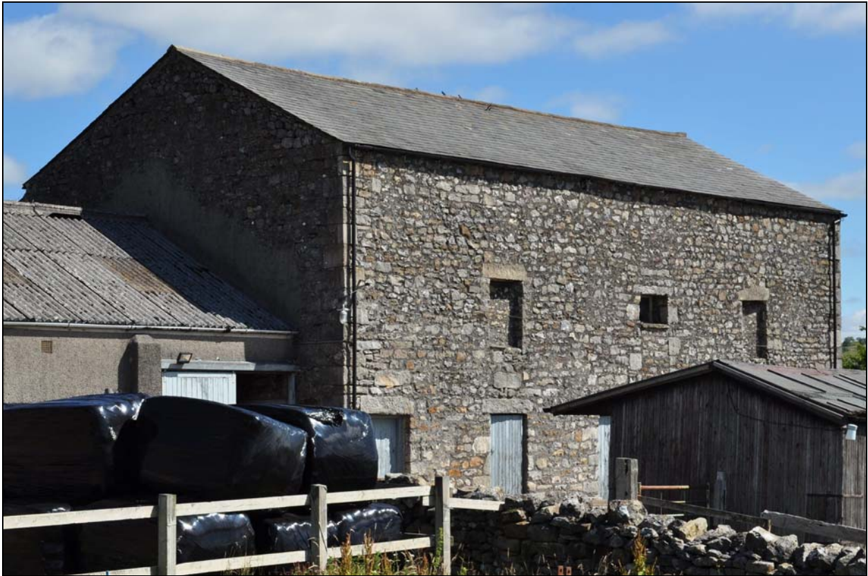
Photo 1: General view of the barn, from the south-west
