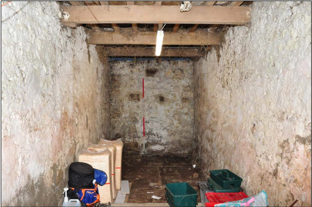
Photo 29: Cart bay, looking north
