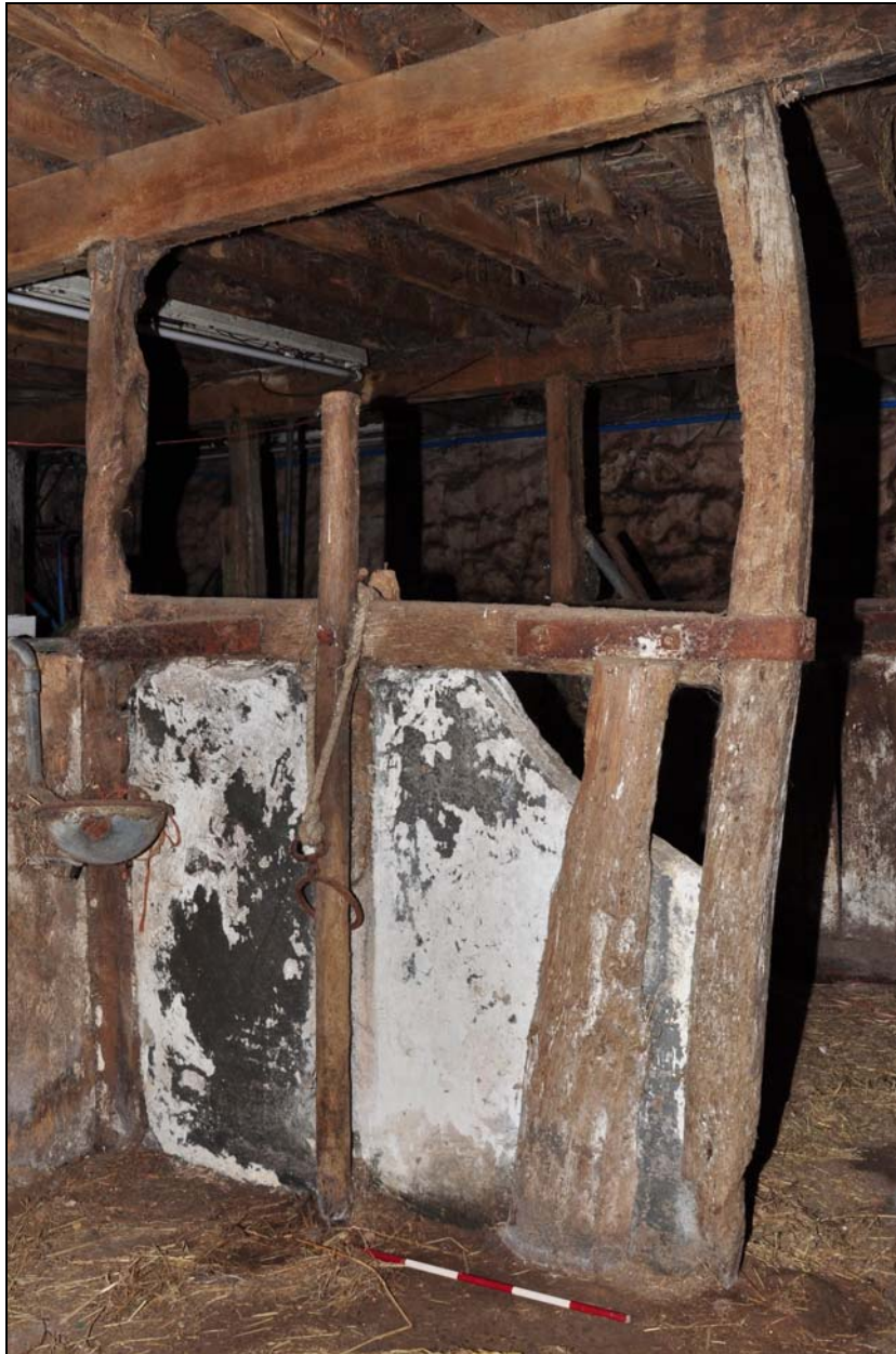
Photo 22: Shippon: stalls in east side, looking north-west
