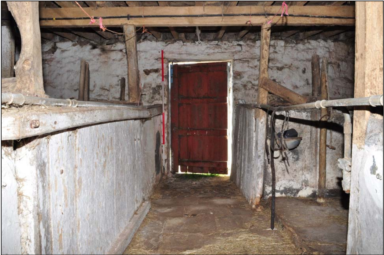
Photo 16: Shippon: feeding passage, looking south
