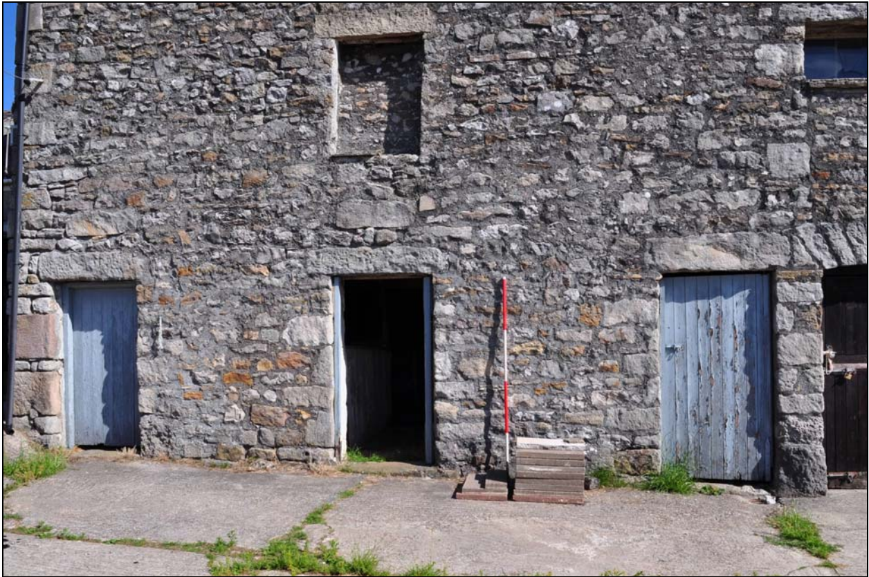
Photo 5: South elevation: three doorways to shippon
