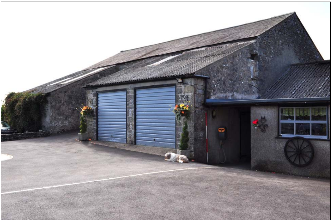
Photo 12: General view of the barn, from the north-west
