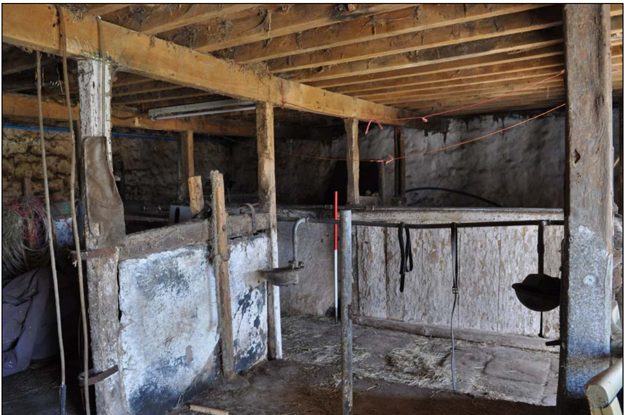
Photo 24: Shippon: stalls in west side, looking north-east
