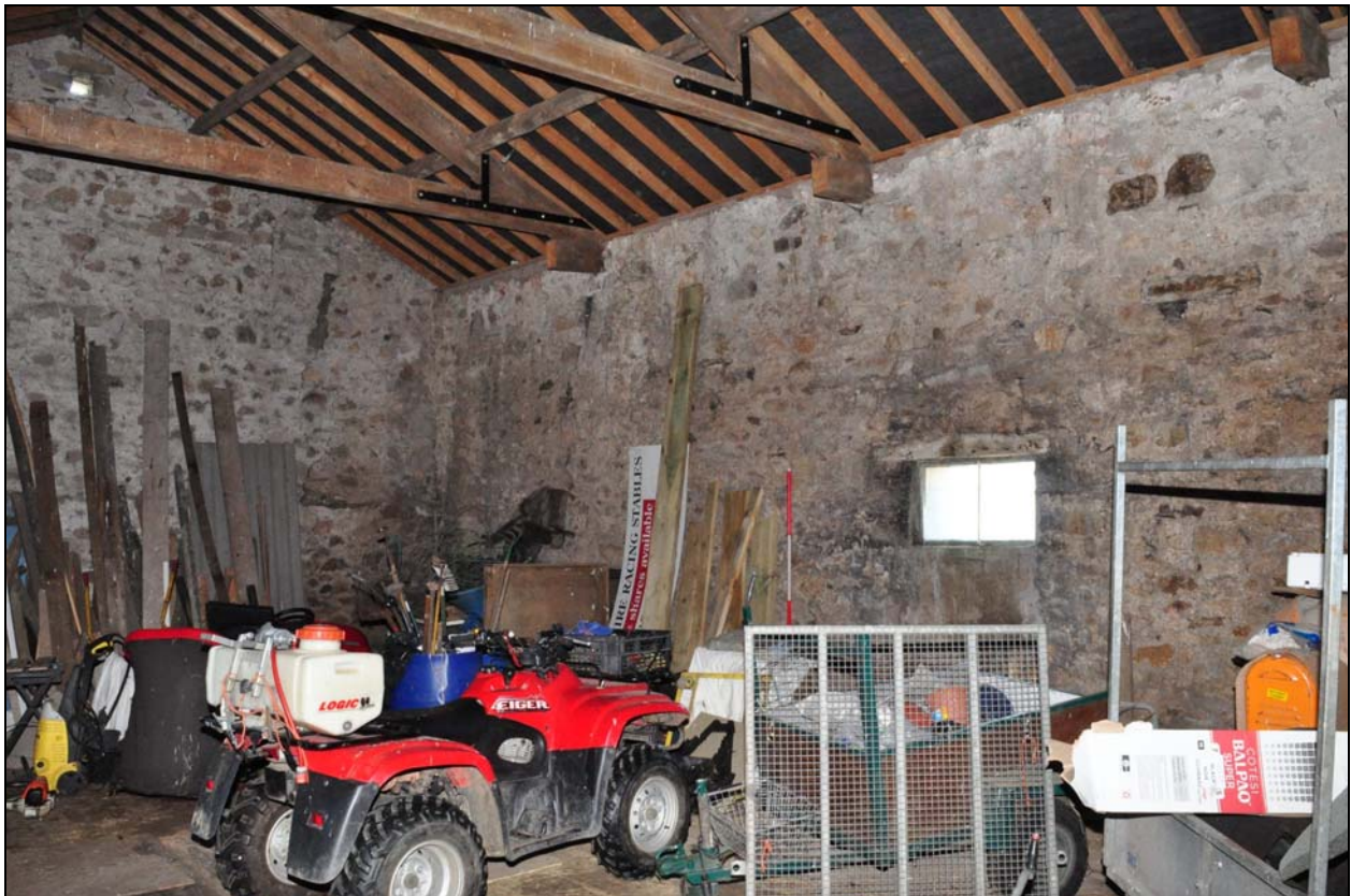
Photo 35: Hayloft, looking south-east
