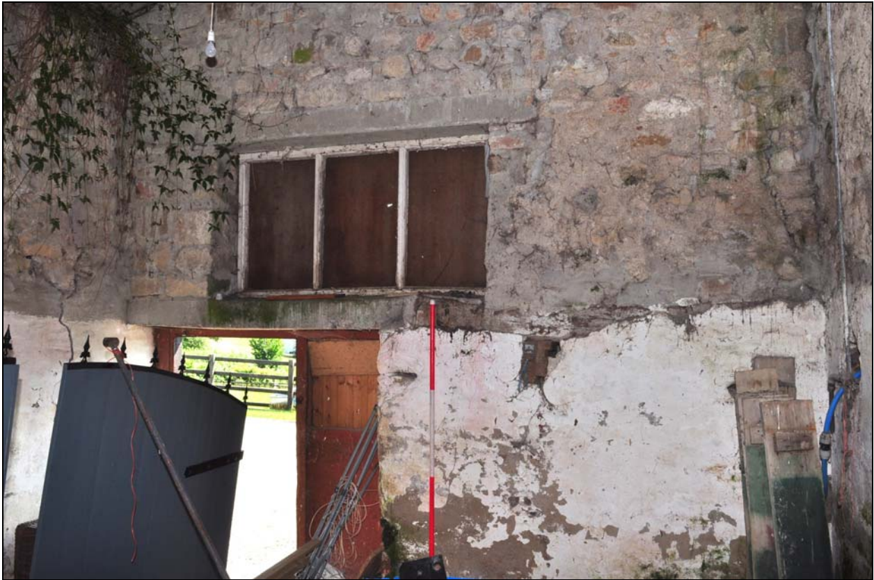
Photo 39: North-east outshut, looking north-east
