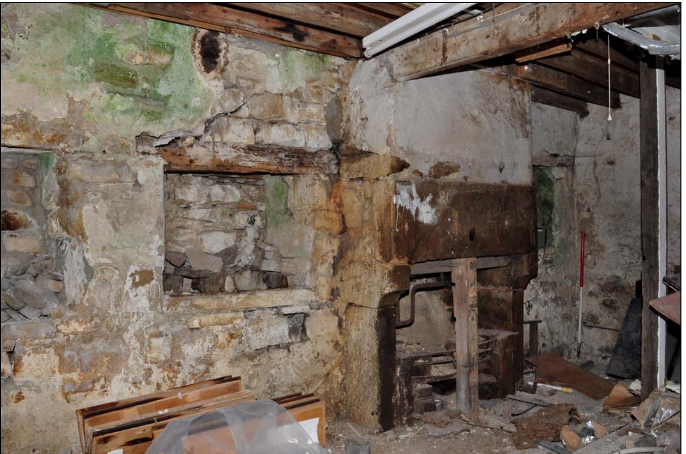
Photo 31: Ground floor room, south-west end of house, looking west
