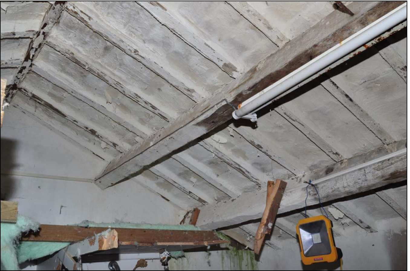
Photo 44: First floor room, south-west end of house: purlins, looking east
