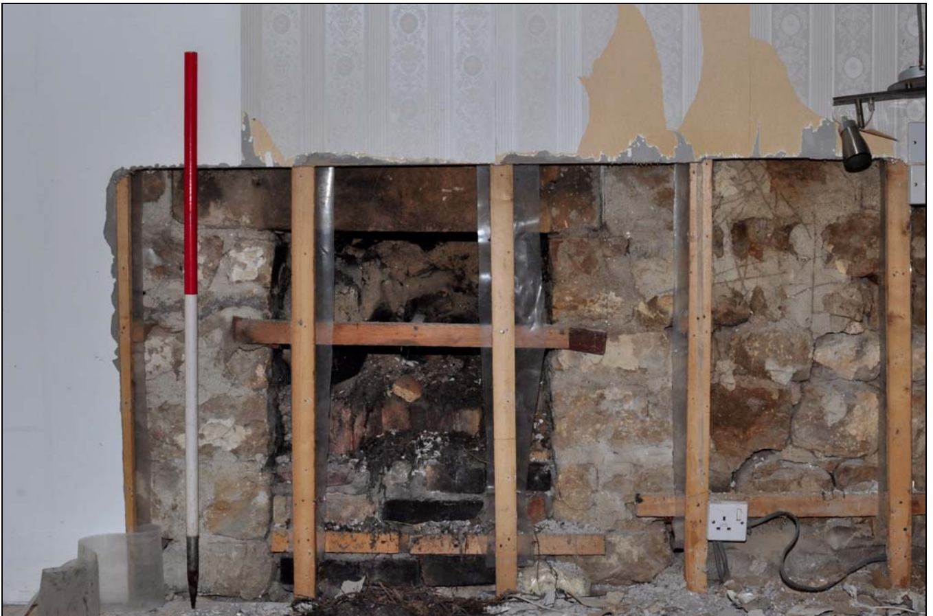
Photo 22: First floor: gable fireplace opening, north-east bedroom
