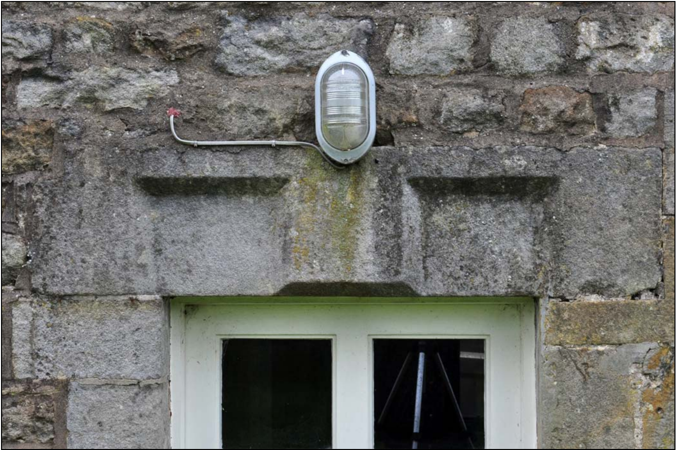
Photo 6: Lintel over front doorway, north-west elevation
