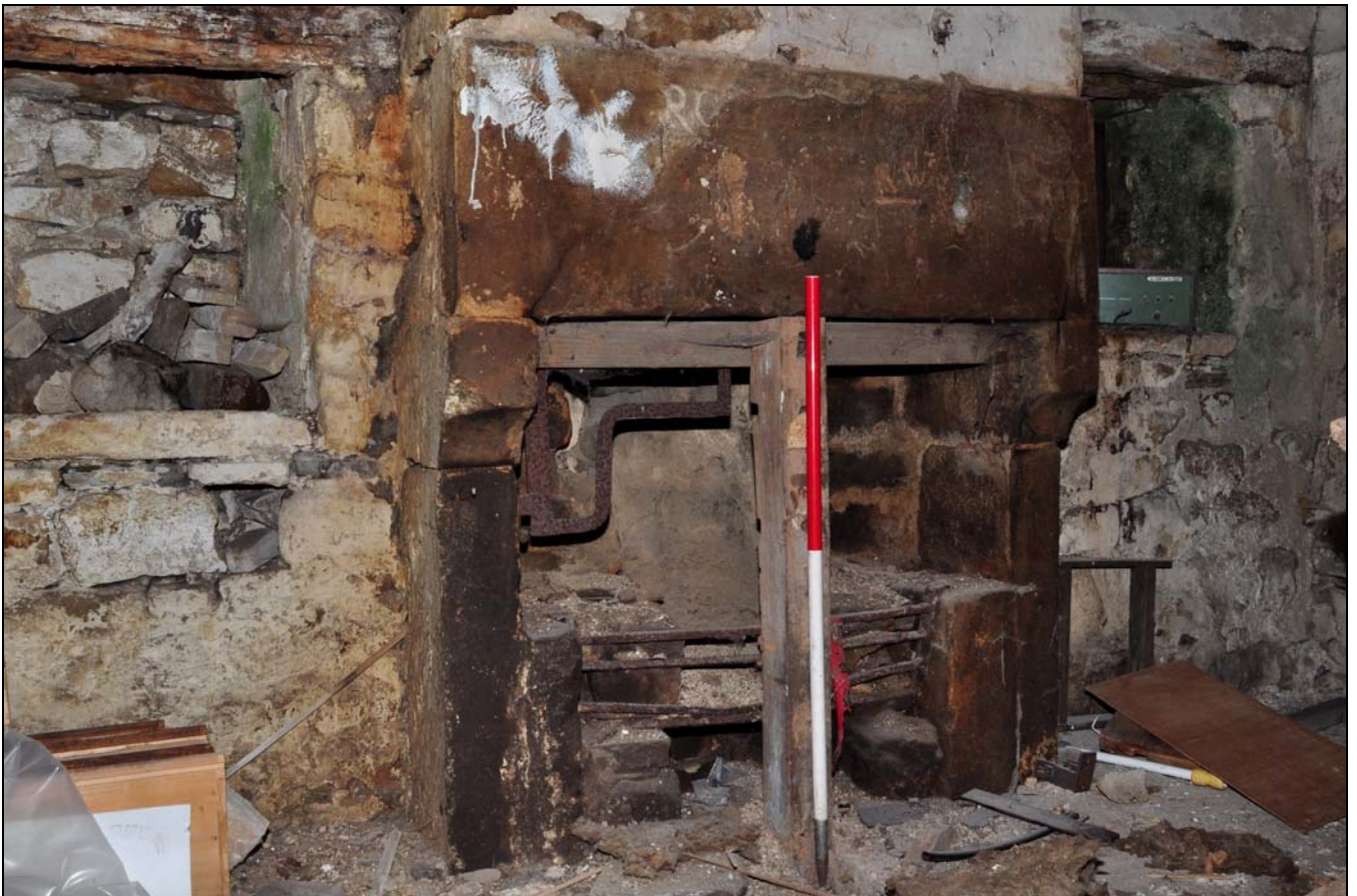
Photo 34: Ground floor room, south-west end of house: fireplace
