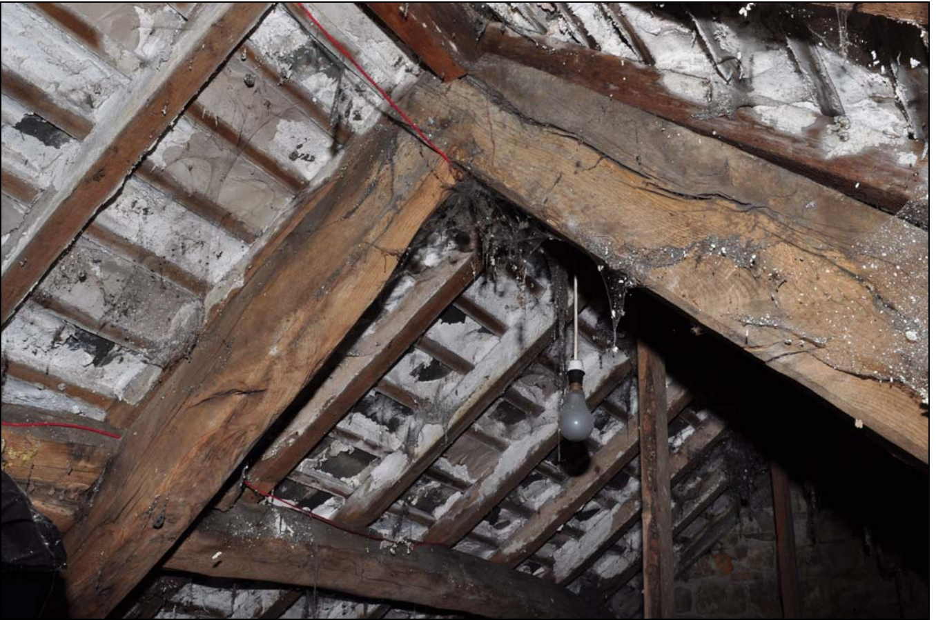
Photo 29: Roof truss over main part of house, looking north
