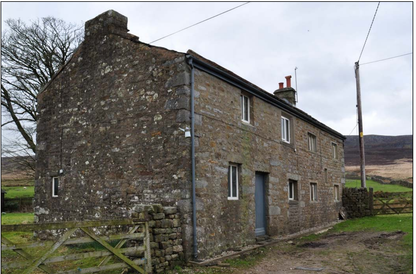
Photo 5: The house, looking north
