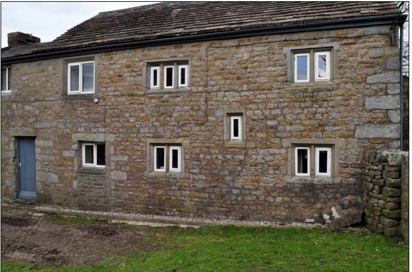
Photo 8: South-east (rear) elevation of main part of house
