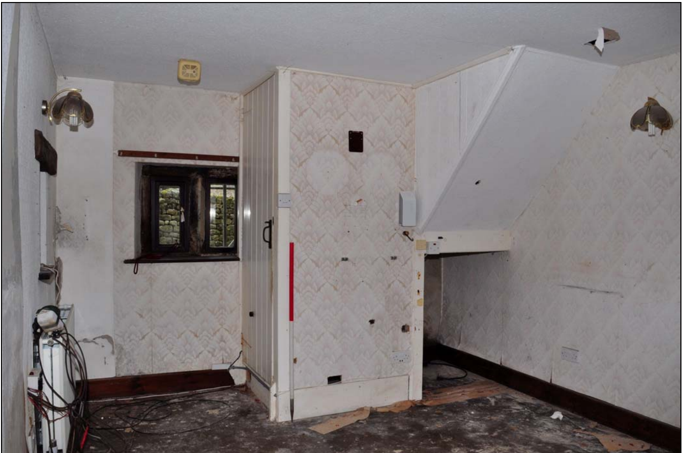
Photo 15: Ground floor: present living room, looking south-east
