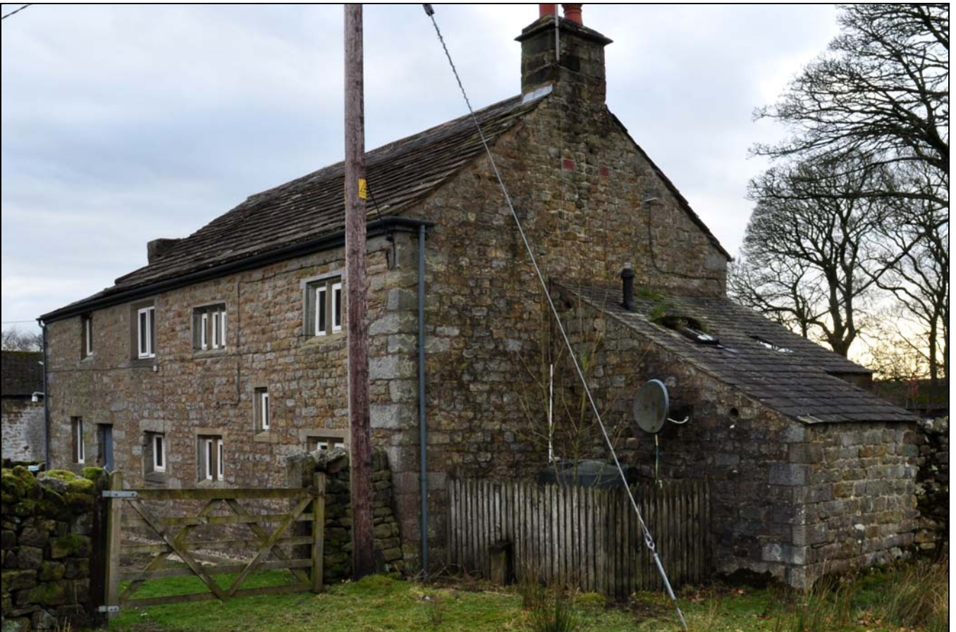
Photo 46: Lean-tos at north-east end of house, looking west
