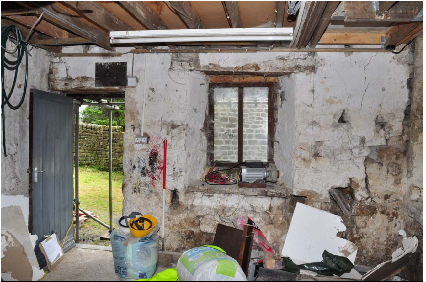
Photo 32: Ground floor room, south-west end of house, looking south-east
