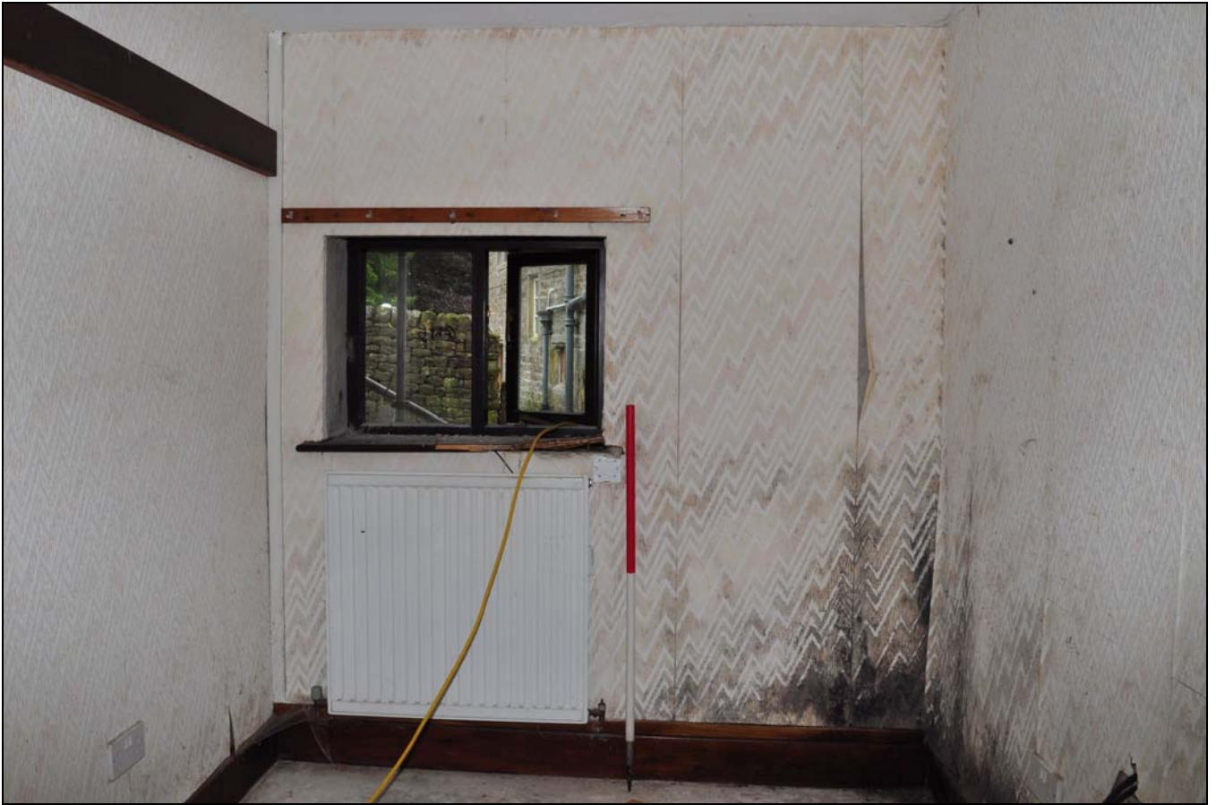
Photo 20: Ground floor: present bathroom, looking south-east
