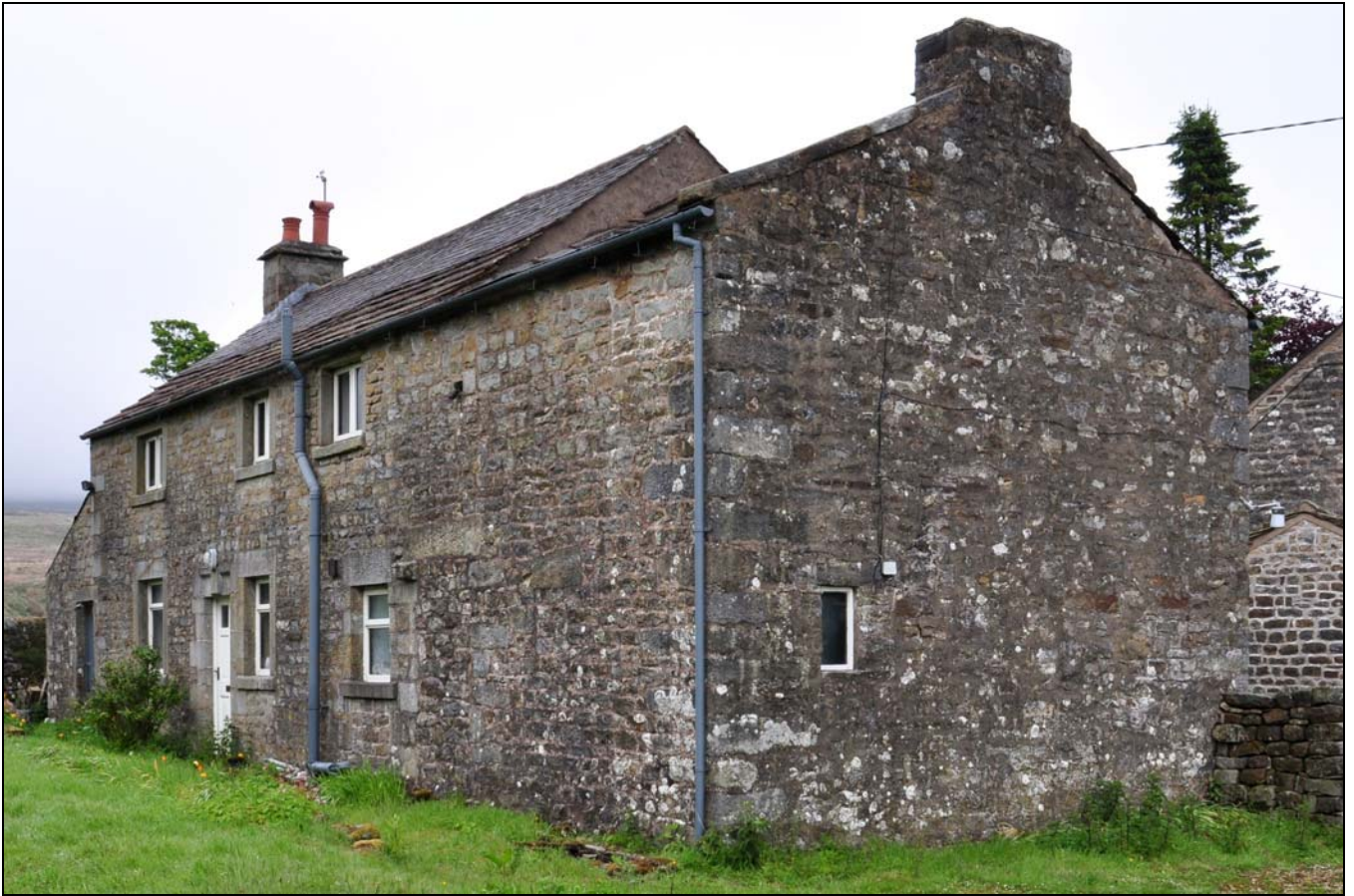
Photo 3: The house, looking east
