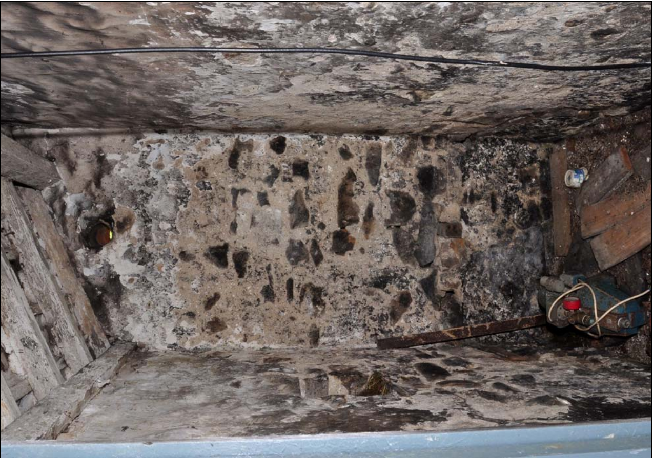
Photo 50: Interior of smaller lean-to (earth closet), looking south-east
