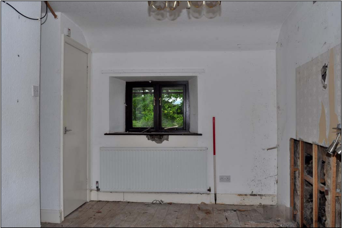
Photo 24: First floor: north-east bedroom, looking north-west
