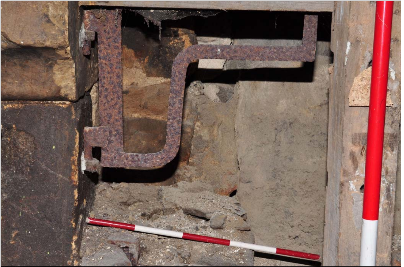
Photo 37: Ground floor room, south-west end of house: fireplace crane
