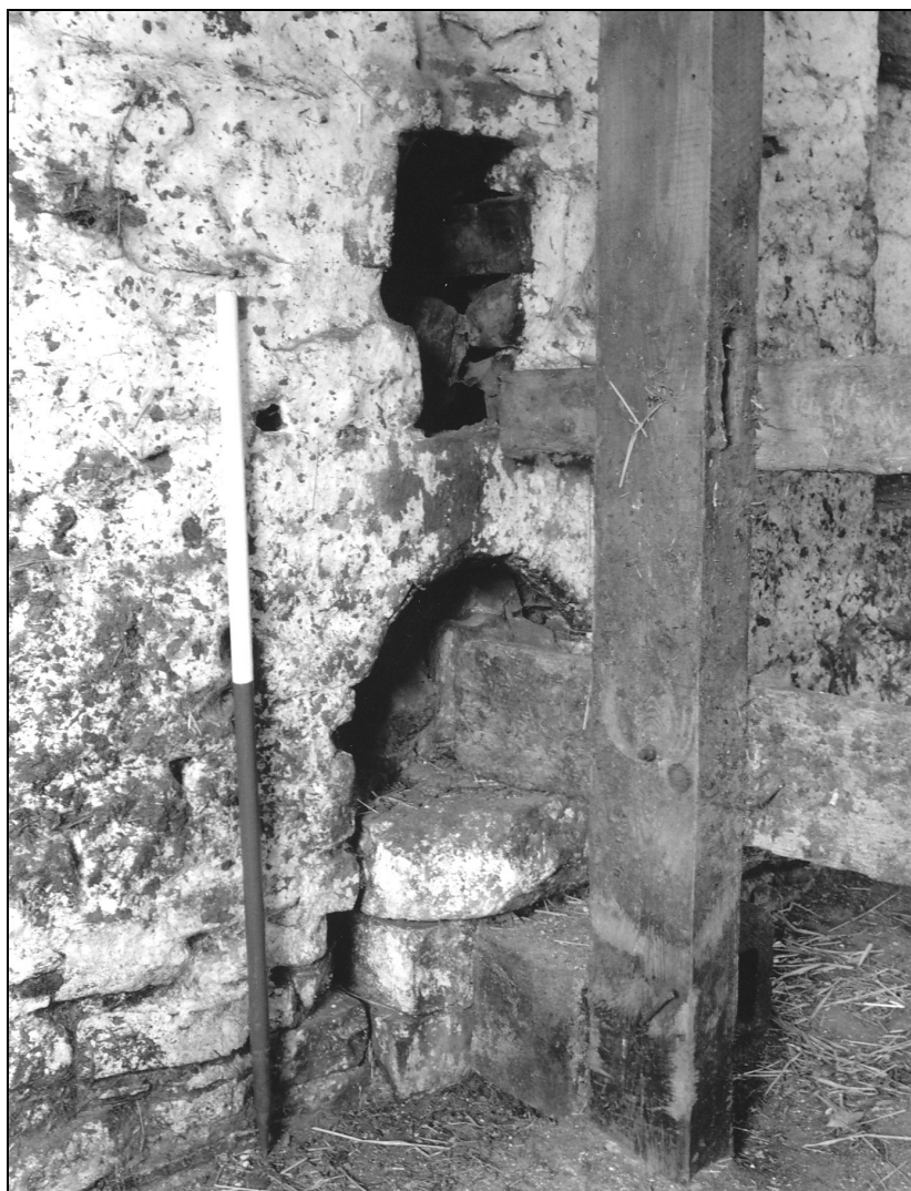
Photo 56: Bobbin Mill: fireplace/stove recess in south-west side of ground floor
