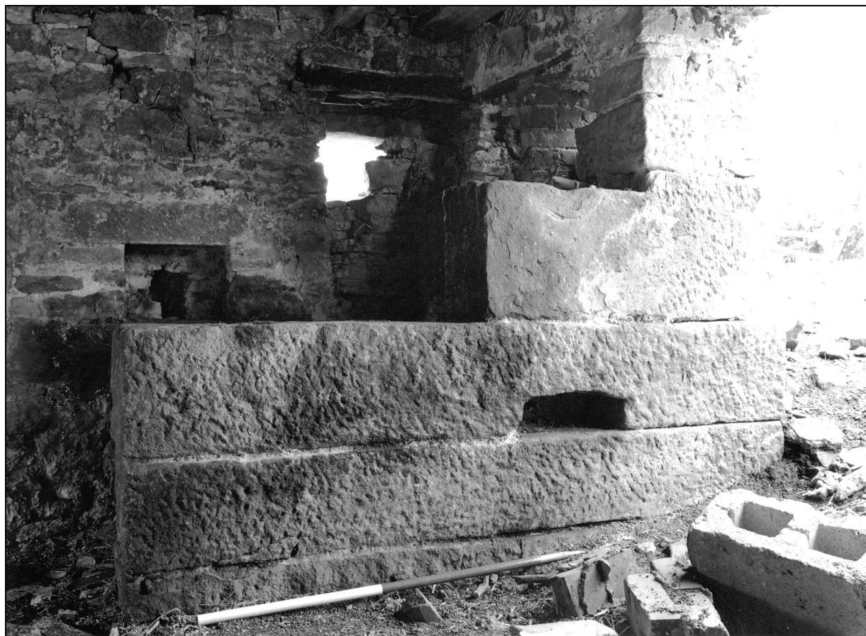
Photo 33: Power House: stone blocks to side of wheelpit, carrying two bearings
