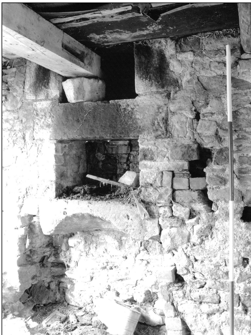
Photo 37: Power House: inserted recesses in south corner of wheelhouse, perhaps for stoking furnace in now demolished building beyond
