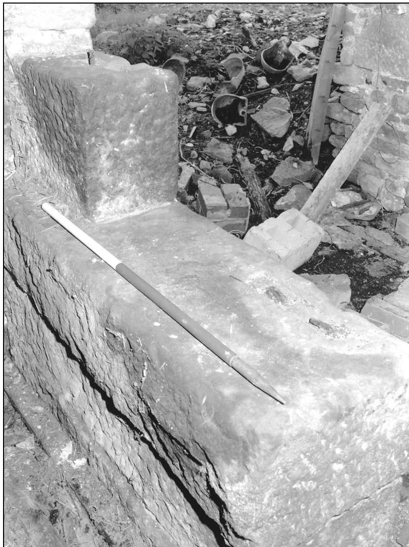
Photo 35: Power House: stone blocks to side of wheelpit, carrying two bearings with cotter bolts
