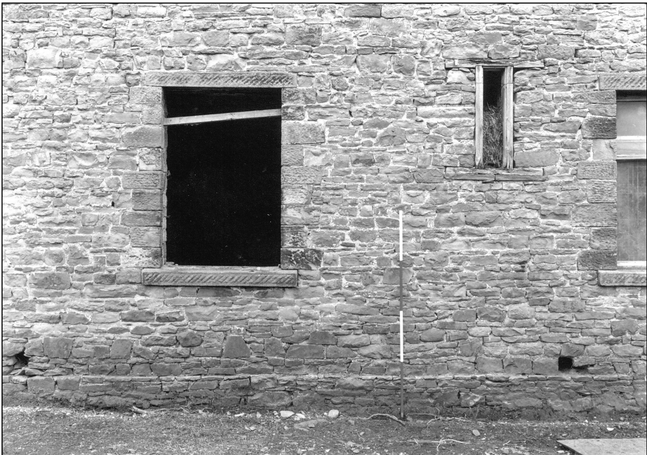
Photo 45: Bobbin Mill: detail of window and slot for belt drive in south-east elevation
