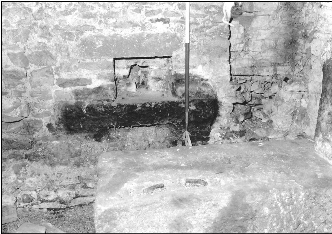
Photo 34: Power House: opposing bearings with cotter bolts, on either side of wheelpit, from the north-east
