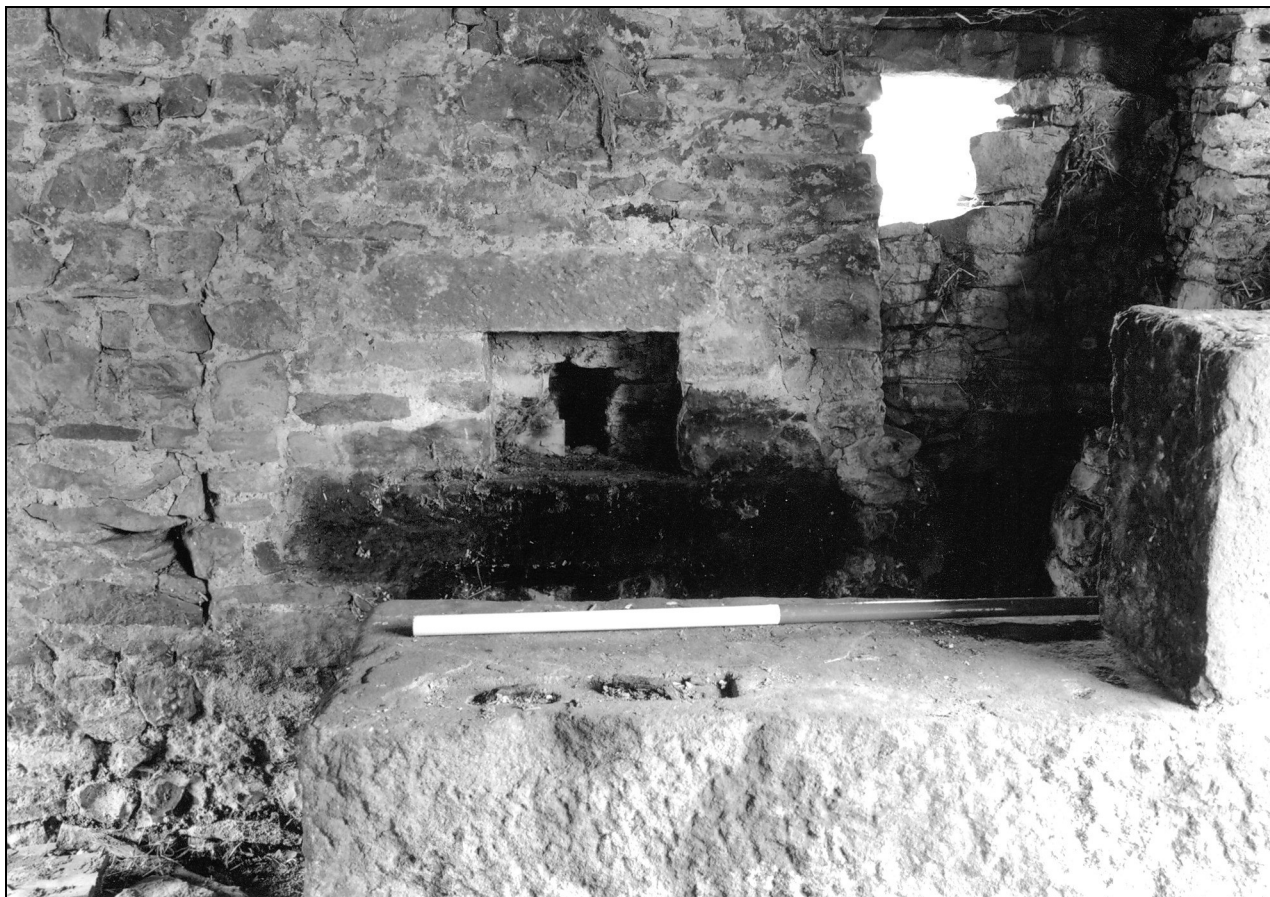
Photo 32: Power House: opposing bearings across wheelpit, from the north-east, probably for waterwheel axle
