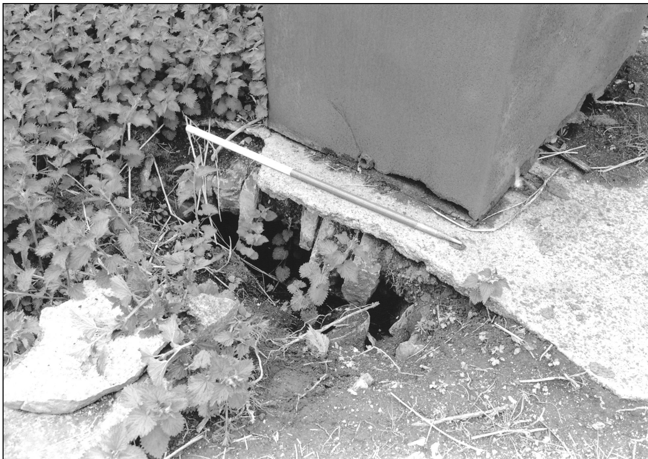
Photo 12: Arch of tail race culvert visible through concrete floor to east of Power House, from the east
