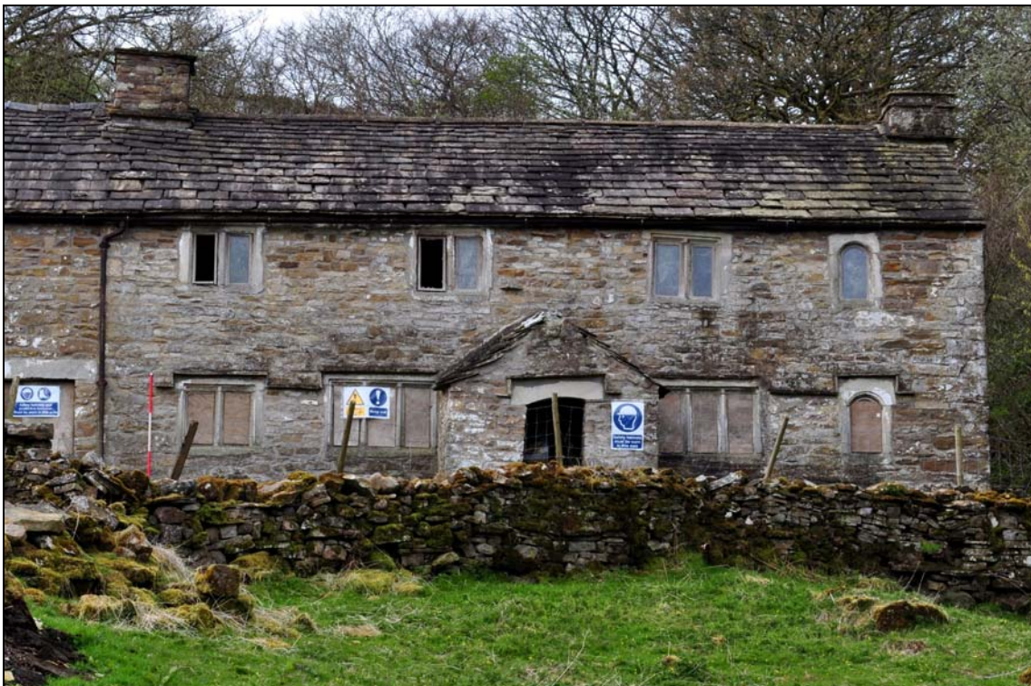
Photo 2: West part of farmhouse, front elevation
