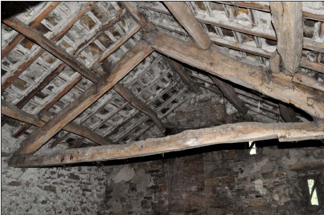
Photo 75: East part, interior: east roof truss, looking north-east
