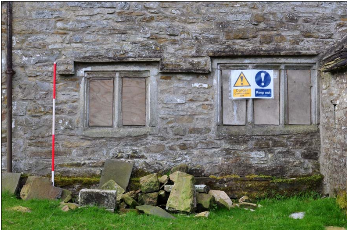
Photo 9: Housebody windows in front elevation
