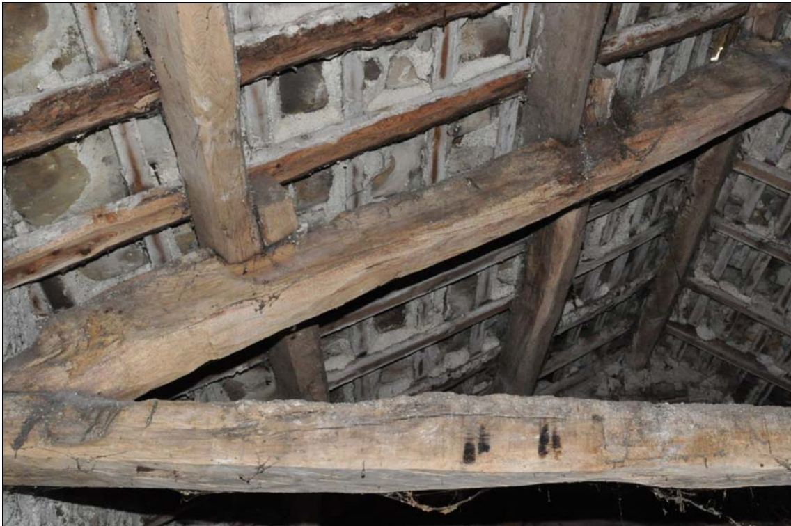
Photo 78: East part, interior: candle marks on east tie-beam, looking east
