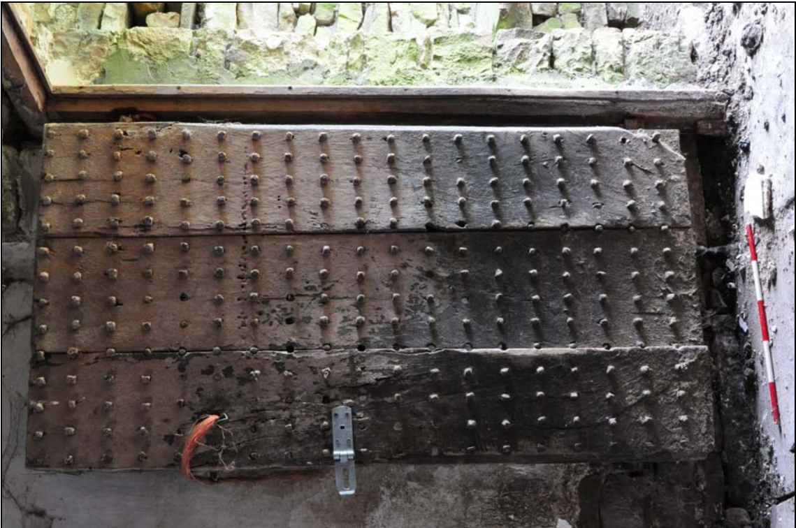
Photo 7: Detail of front door to farmhouse (outer face)
