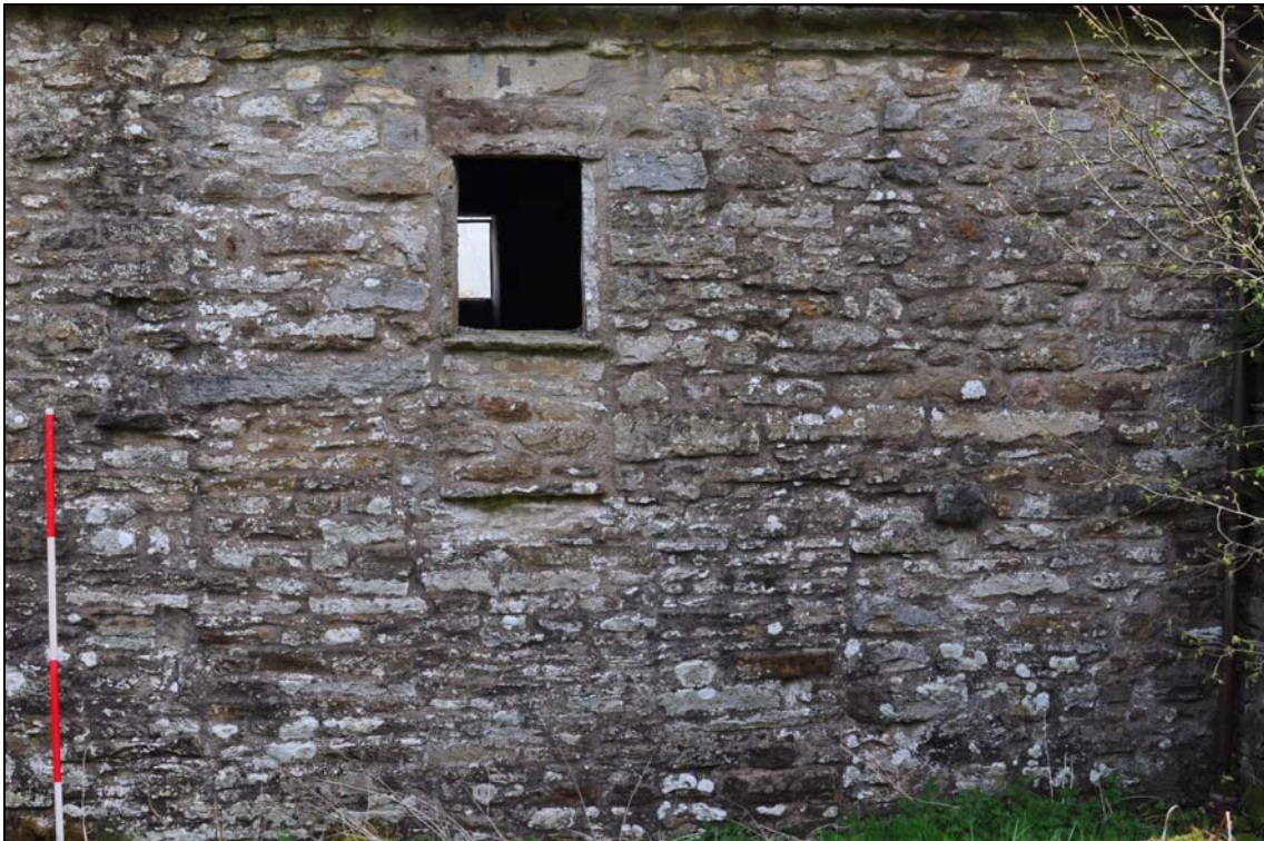
Photo 23: Rear of farmhouse: site of demolished stairs outshut
