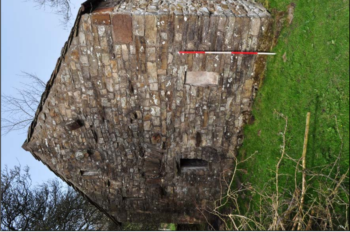
Photo 53: Farmhouse range: east gable
