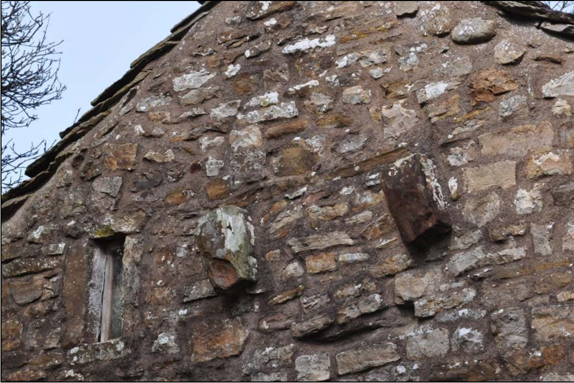
Photo 55: Detail of corbels for former chimney, east gable
