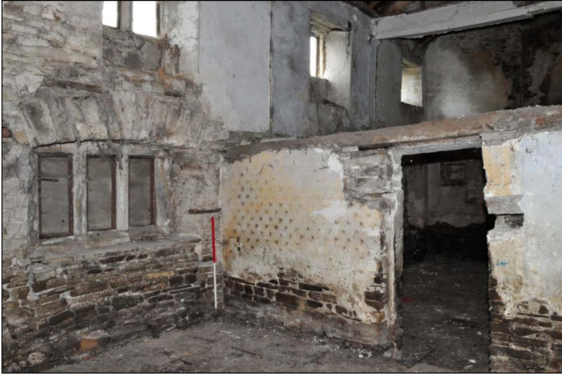
Photo 39: Farmhouse interior: parlour, looking north-east
