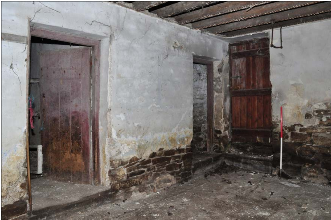
Photo 59: East part, interior: back kitchen, looking south-east
