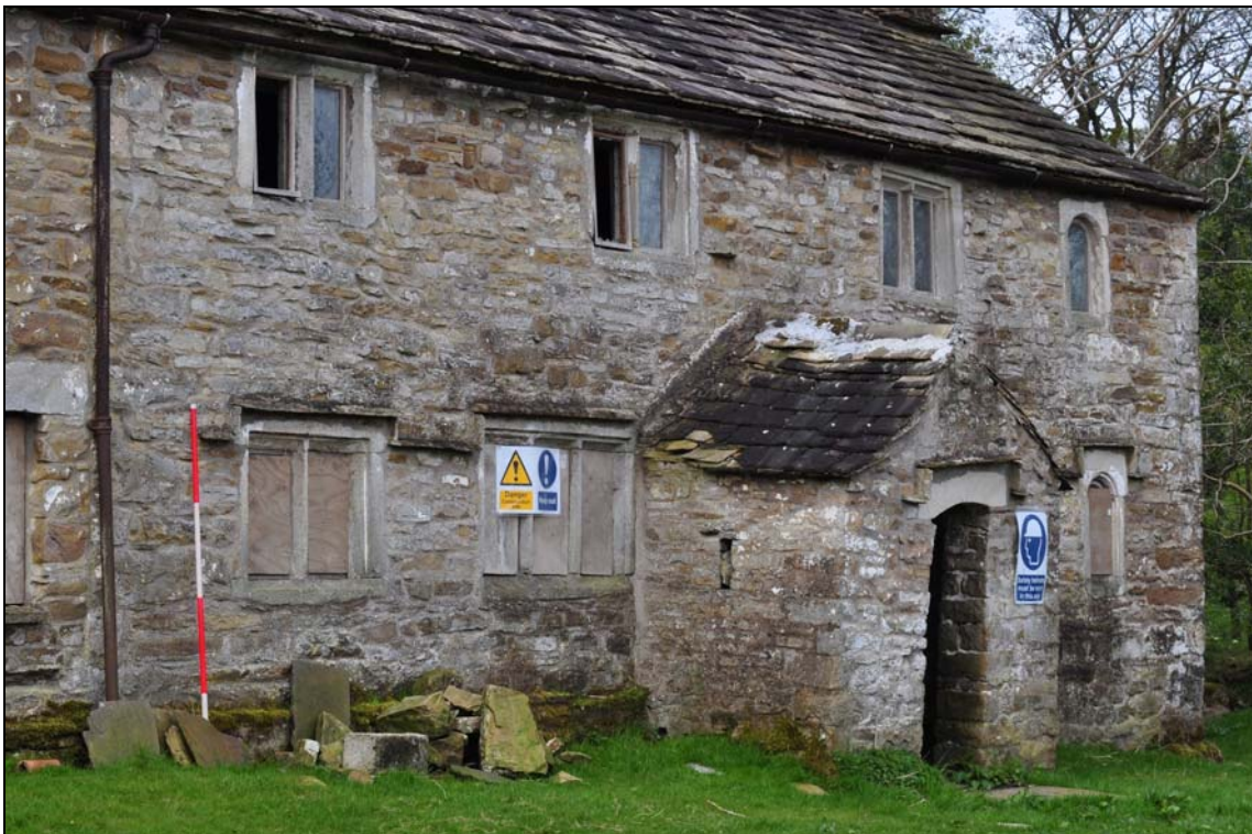
Photo 4: West part of farmhouse, front elevation, looking south-west
