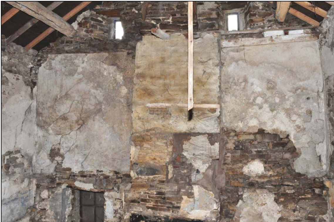
Photo 44: Farmhouse interior: first floor over parlour, looking west
