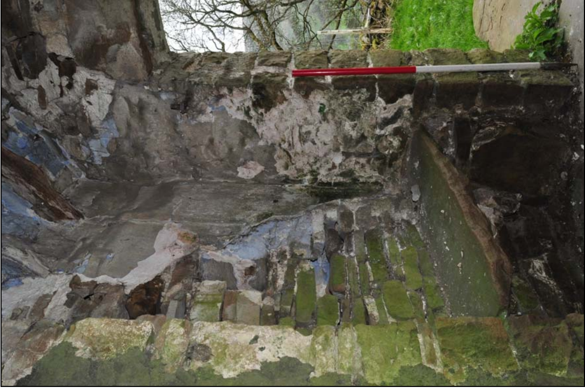
Photo 6: Interior of porch, looking north-west
