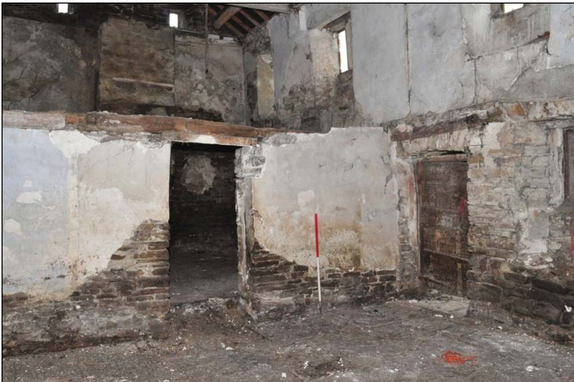
Photo 25: Farmhouse interior: housebody, looking north-west
