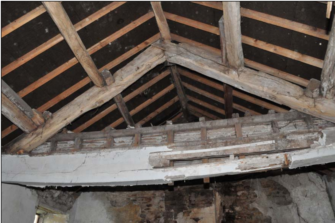
Photo 51: Farmhouse roof: east truss, looking east
