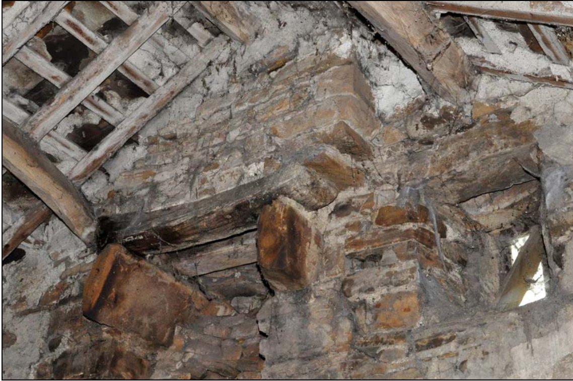
Photo 72: East part, interior: detail of corbelling to former chimney, east gable
