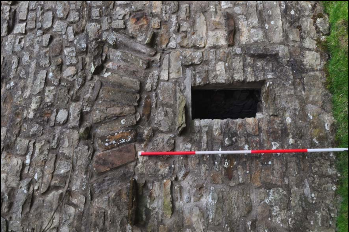
Photo 54: Detail of former doorway in east gable
