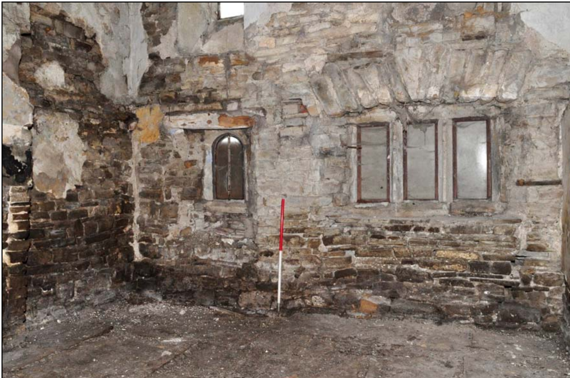
Photo 34: Farmhouse interior: parlour, looking north-west
