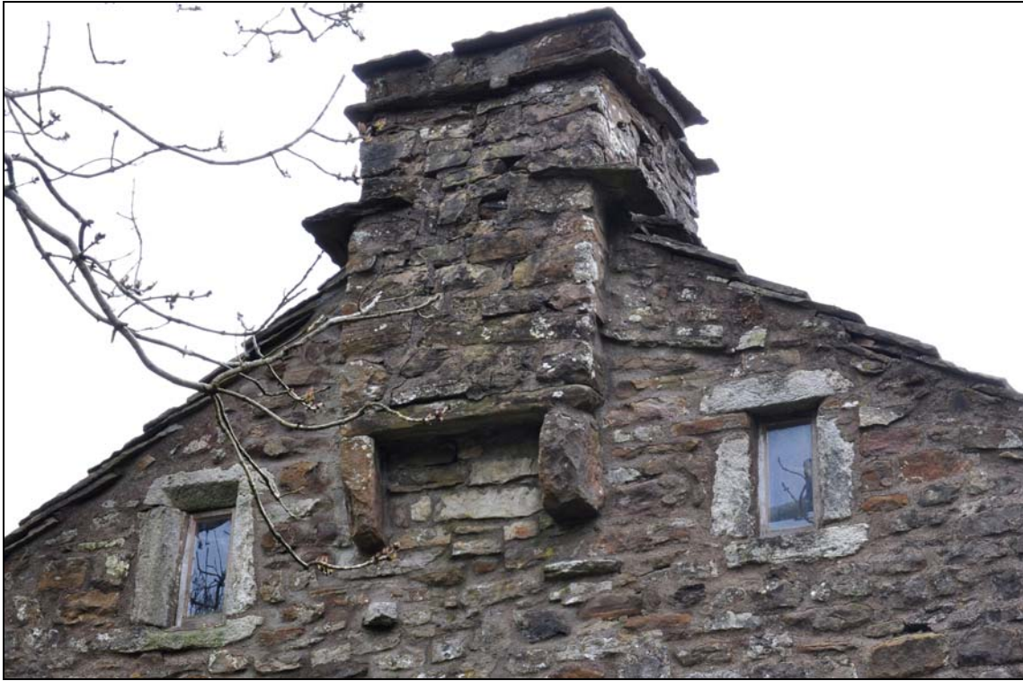
Photo 16: West gable: detail of attic windows and corbelled chimney
