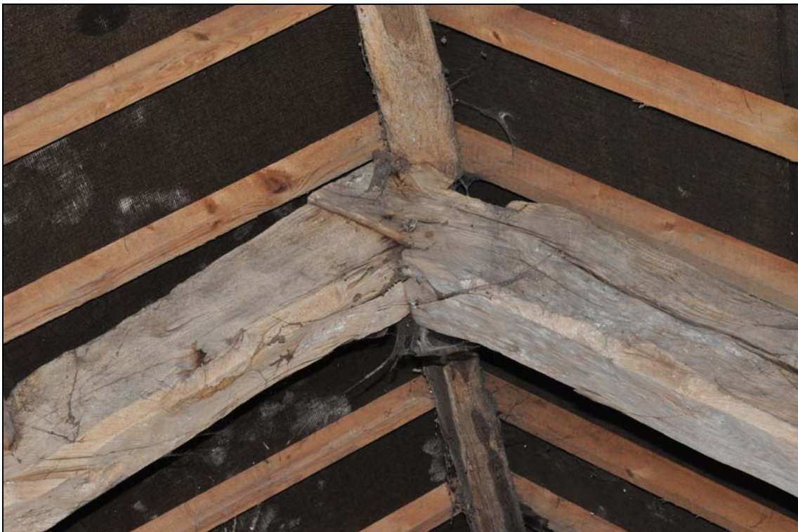
Photo 52: Farmhouse roof: detail at top of east truss, looking east
