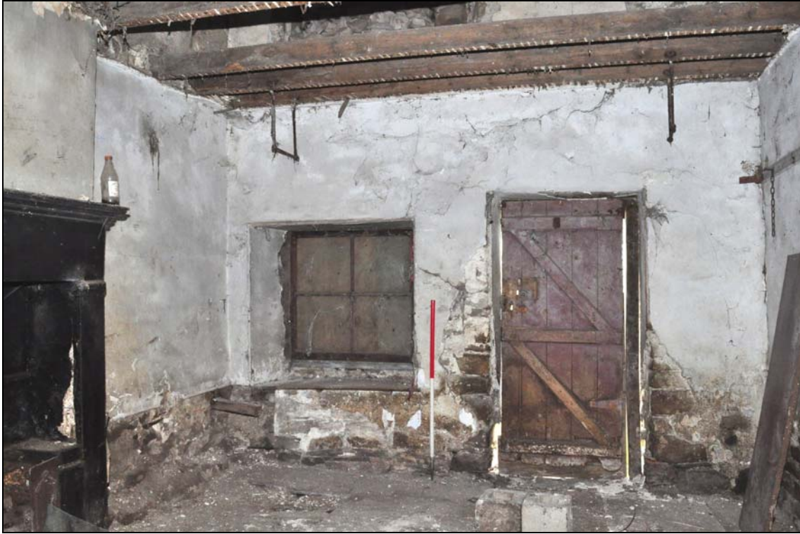
Photo 58: East part, interior: back kitchen, looking north
