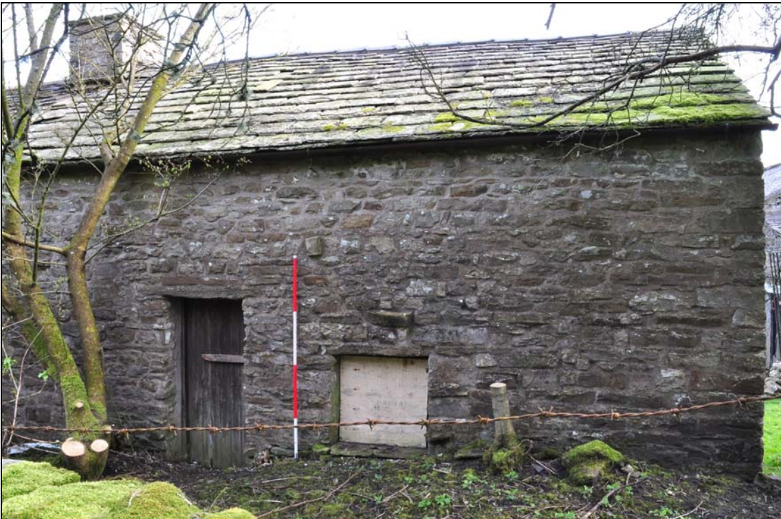
Photo 57: South elevation of east part of farmhouse
