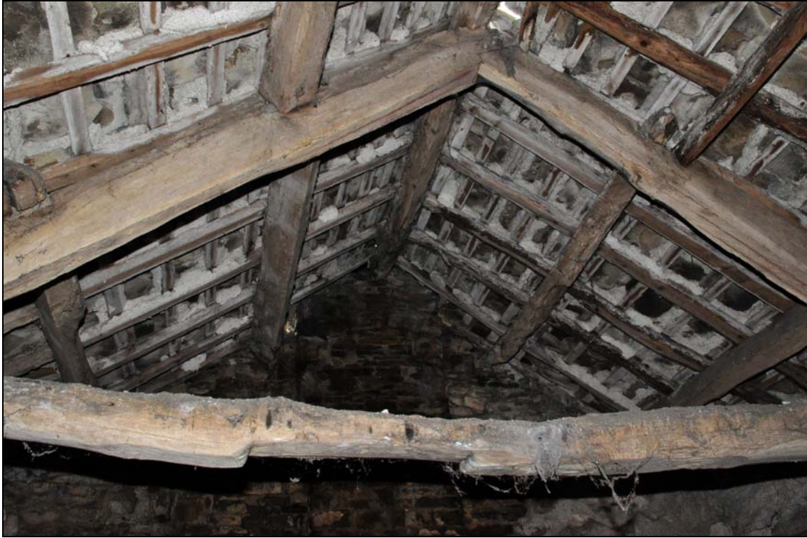
Photo 77: East part, interior: west roof truss, looking west
