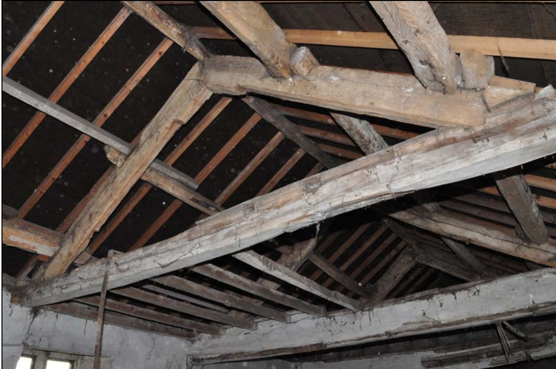
Photo 47: Farmhouse roof: west truss, looking north-east
