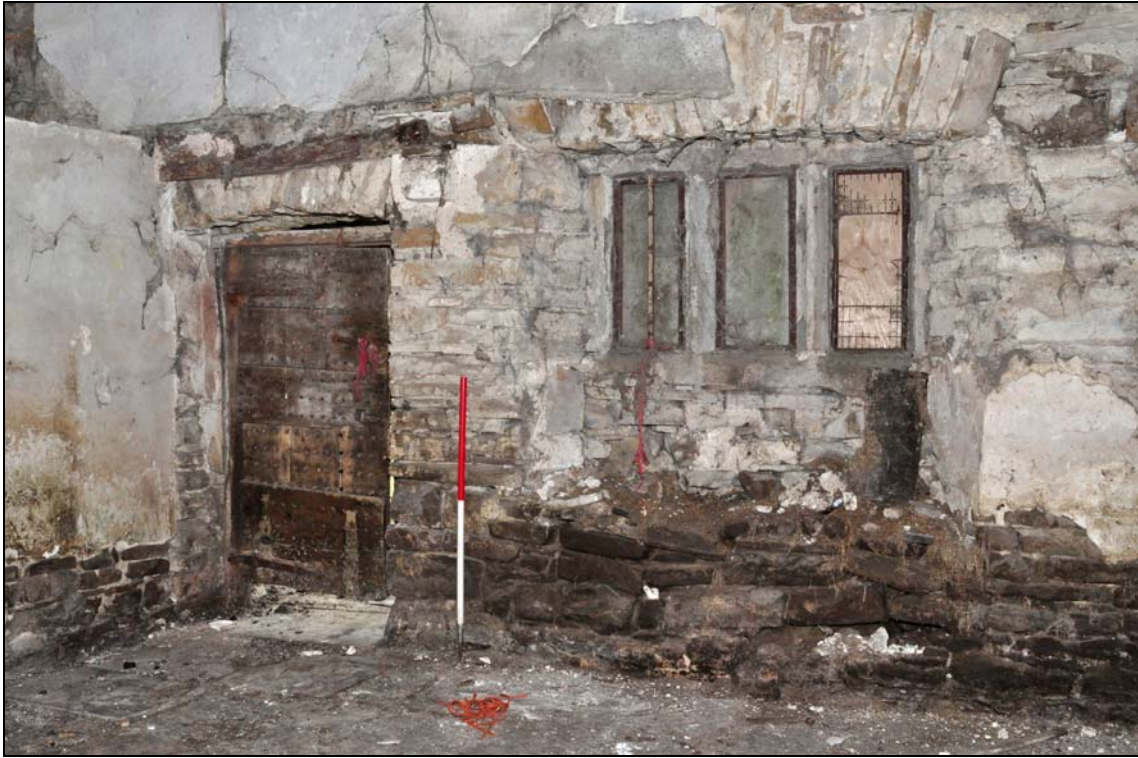
Photo 24: Farmhouse interior: housebody, looking north-west
