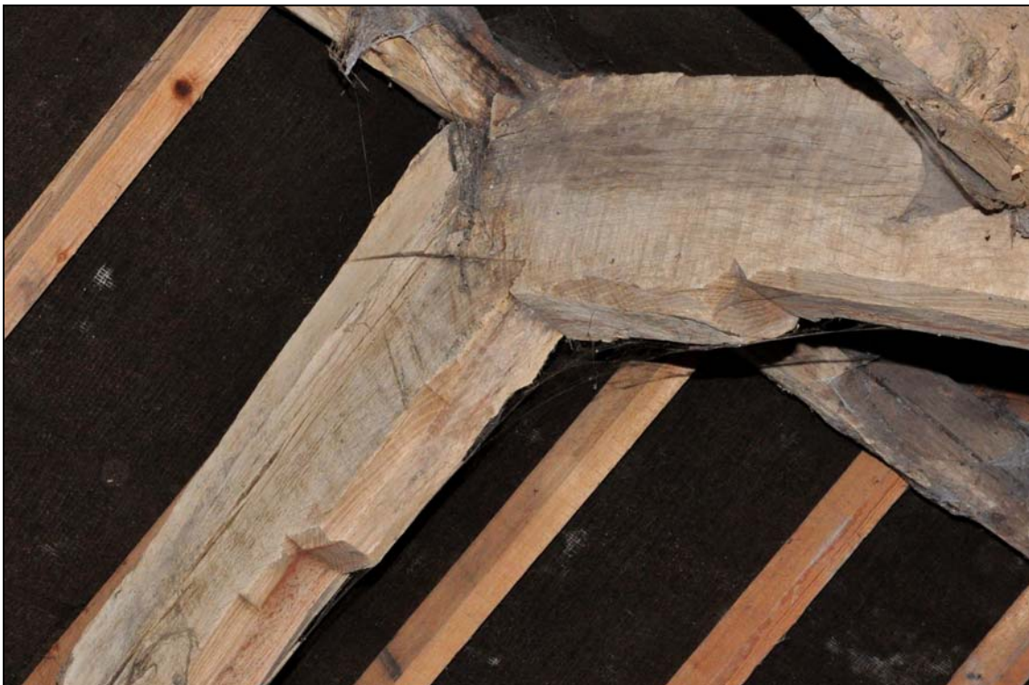
Photo 49: Farmhouse roof: detail at top of west truss, looking north-east
