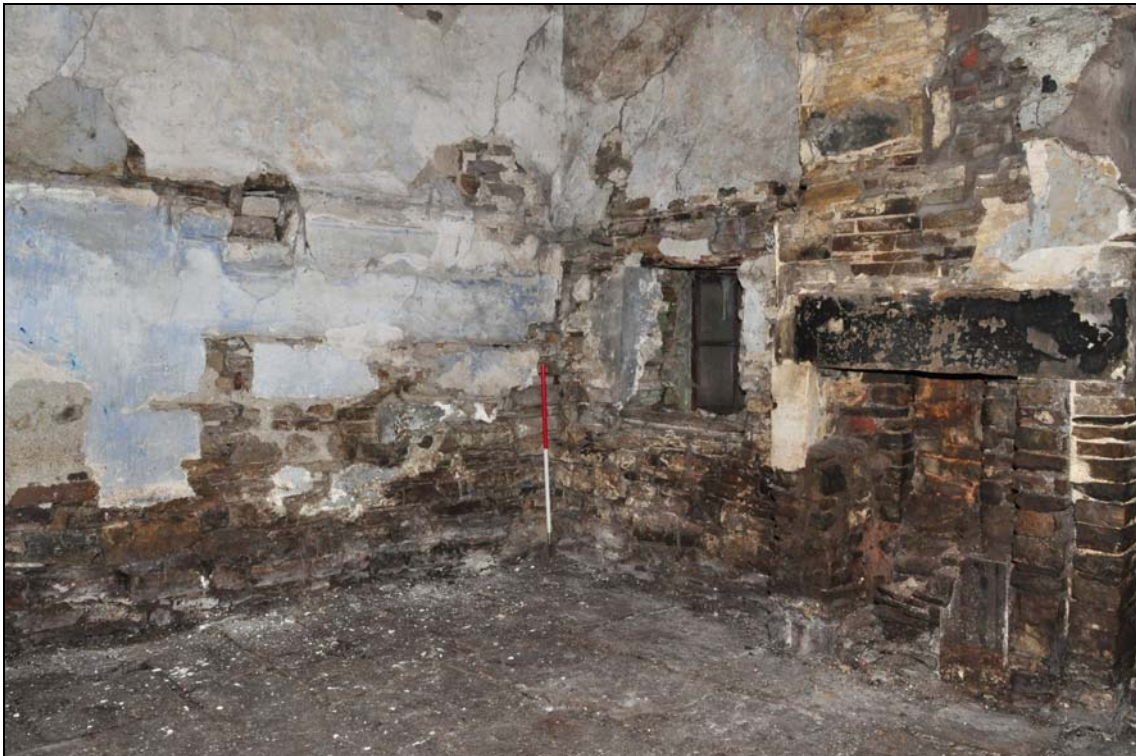
Photo 38: Farmhouse interior: parlour, looking south-west
