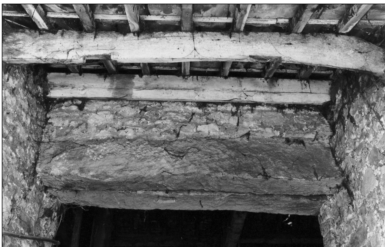
Photo 22: Stone lintels of barn entrance and purlins of porch roof
