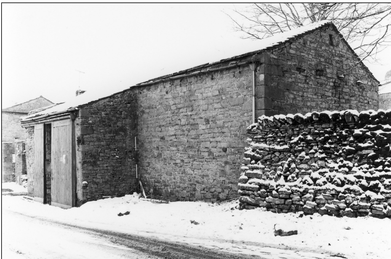
Photo 2: The barn, from the south-east
