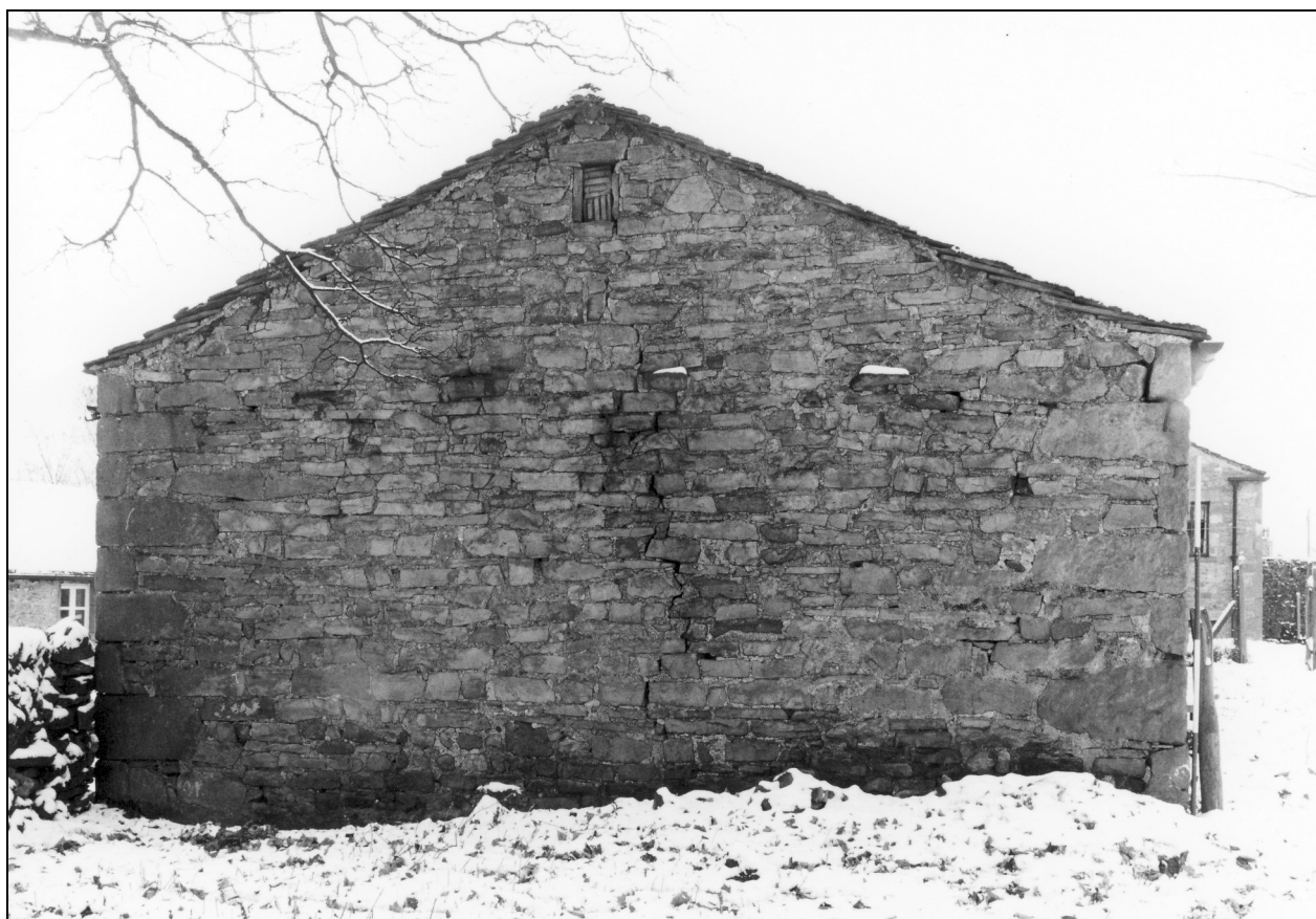
Photo 16: The east gable
