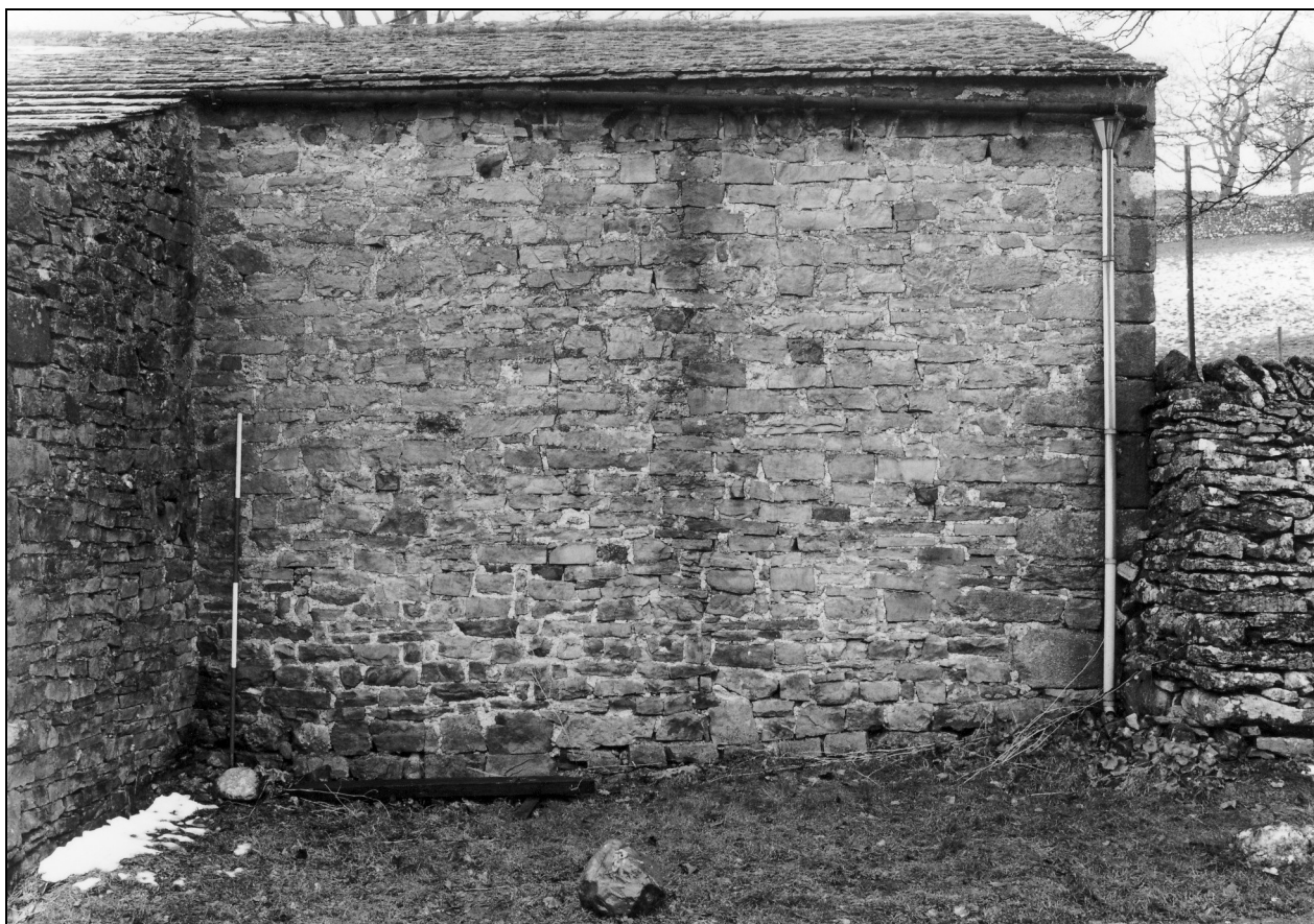
Photo 14: South side of barn to east of porch, showing row of blocked breathers
