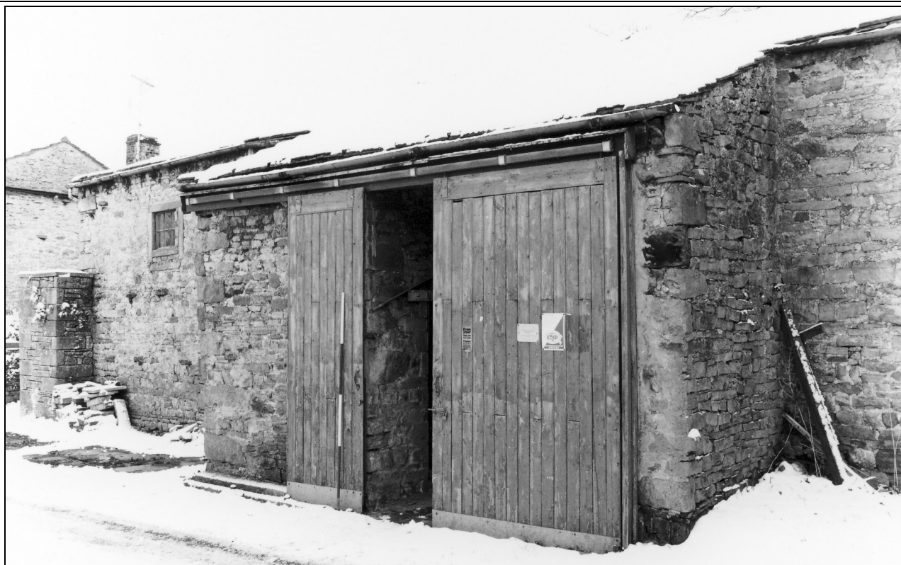
Photo 11: Barn porch, from the south-east
