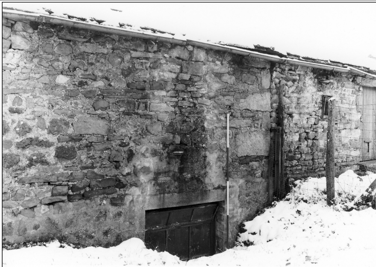
Photo 19: Window in north elevation of barn
