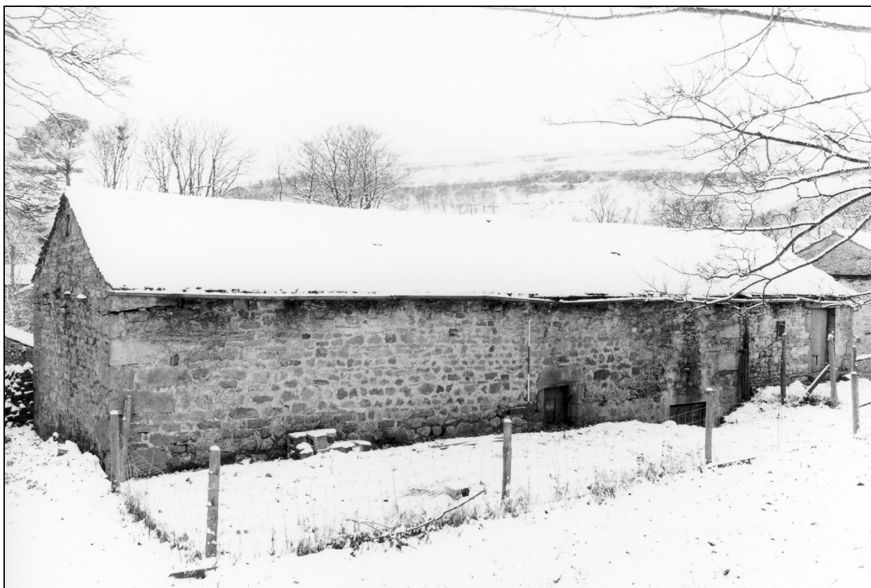
Photo 17: The barn, from the north-east
