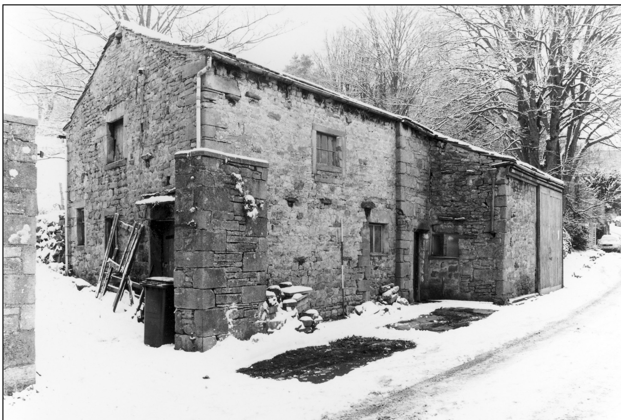
Photo 4: The barn, from the south-west
