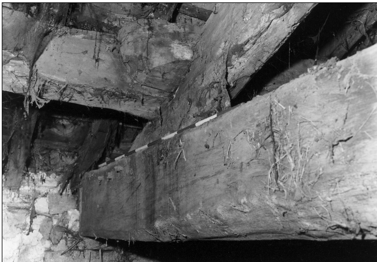
Photo 39: South end of west roof truss, from the north-east
