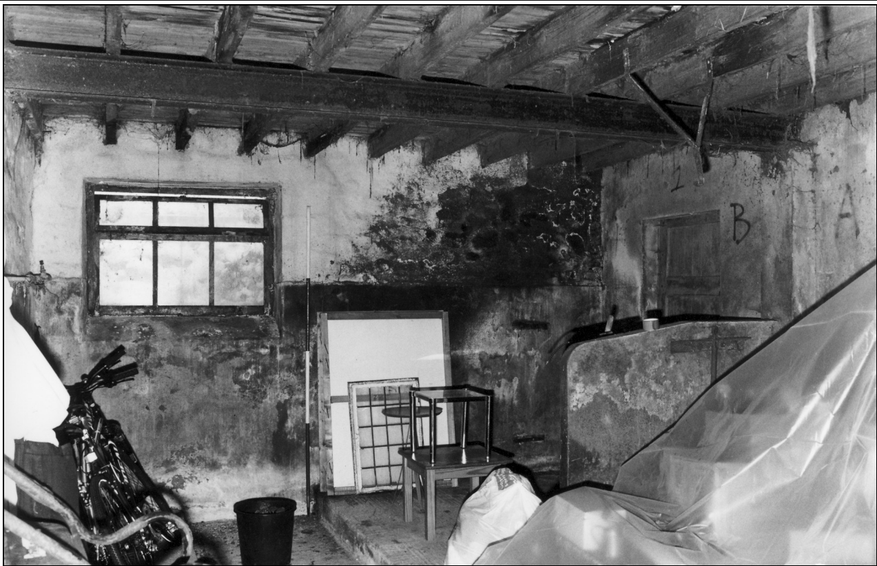
Photo 32: Interior of shippon, from the south (refitted in 20th century)
