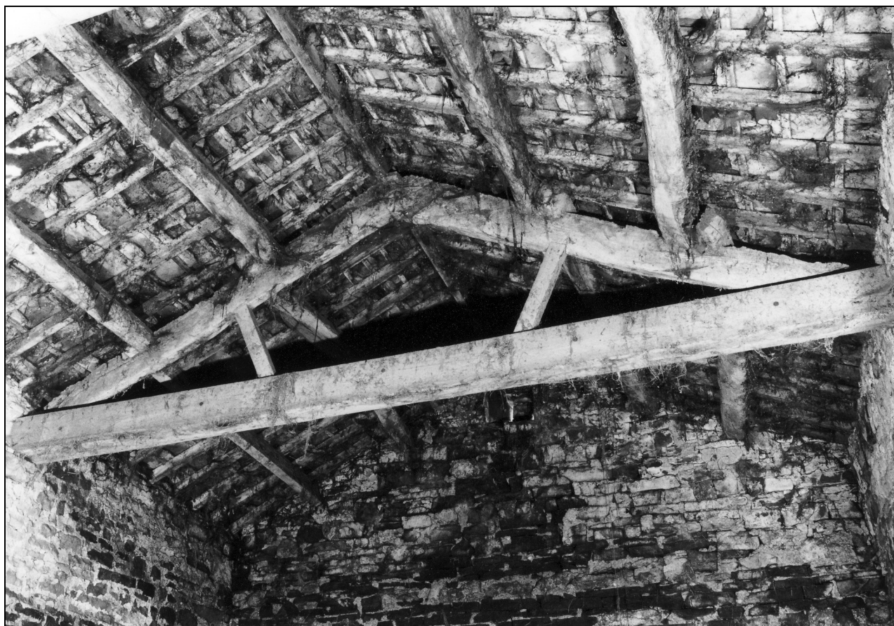
Photo 37: East roof truss, from the west
