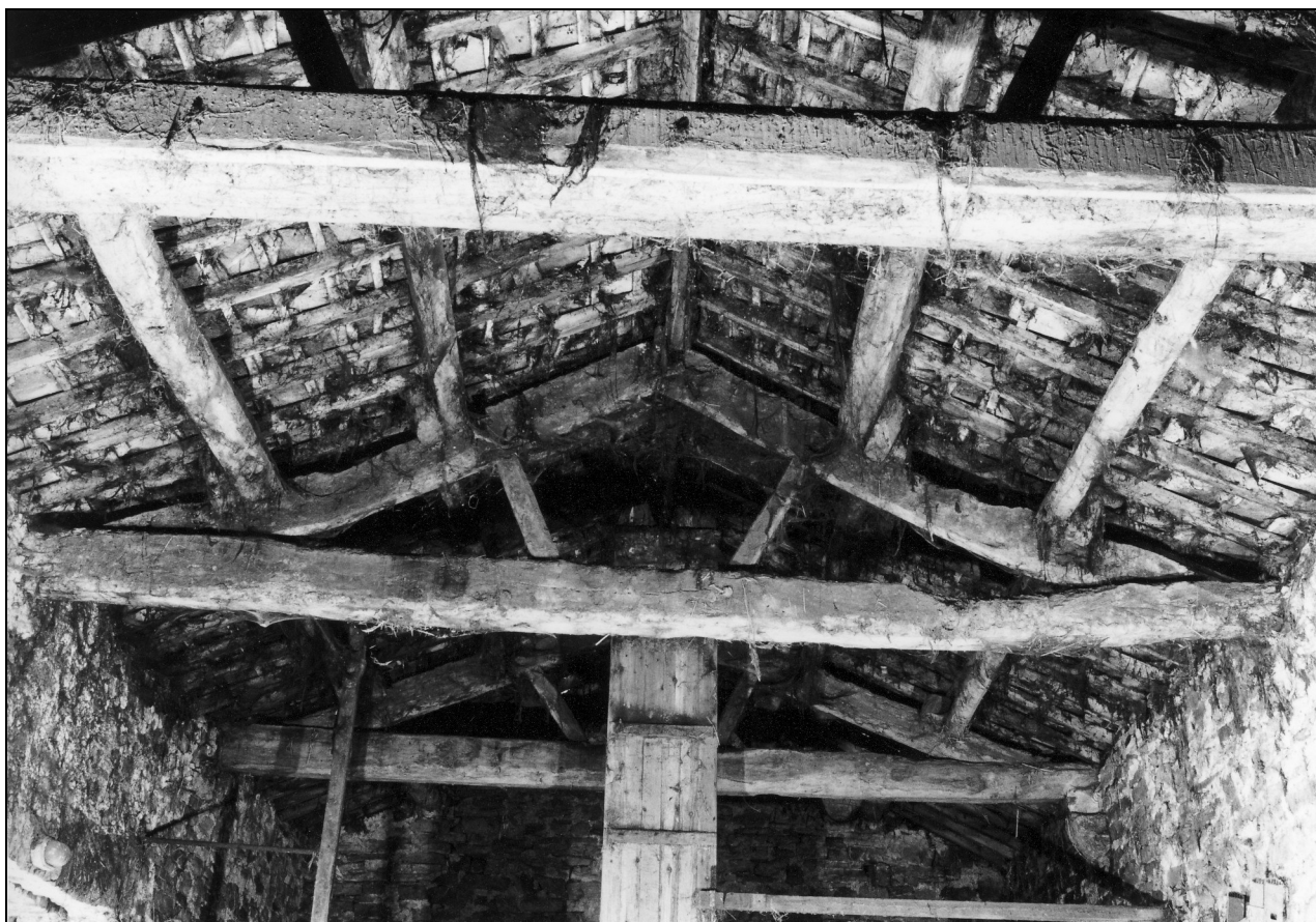
Photo 35: Central roof truss, from the east
