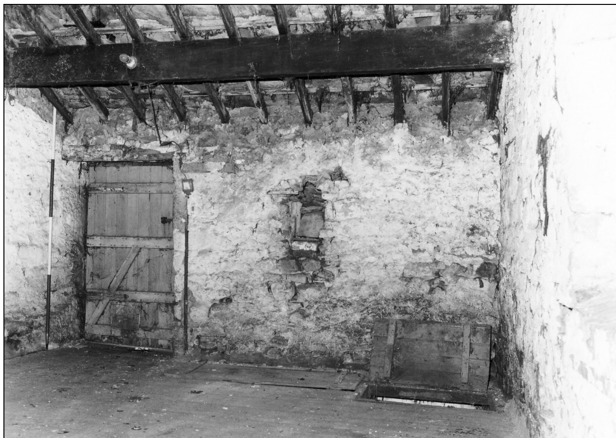
Photo 53: Hay loft over stable, from the south-east
