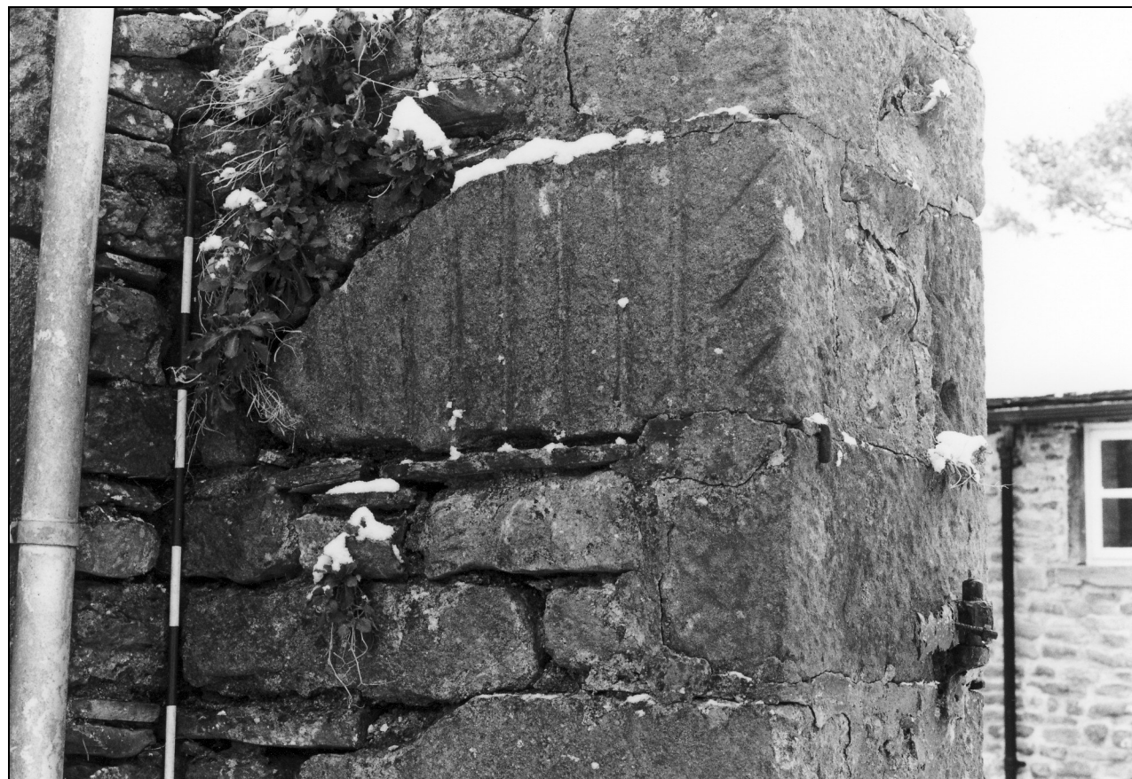
Photo 56: Detail of millstone fragment in east gate pier
