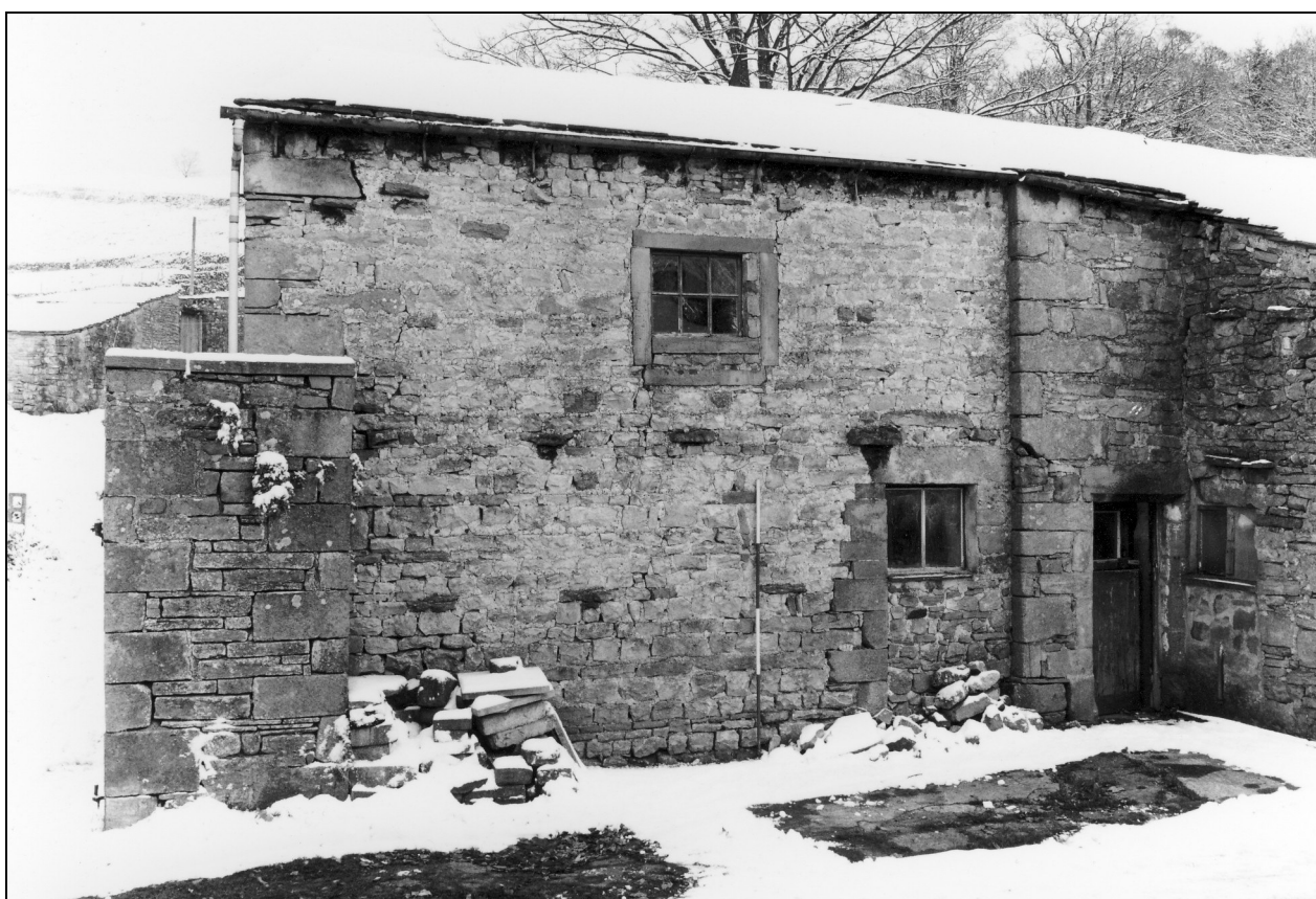
Photo 43: South side of stable
