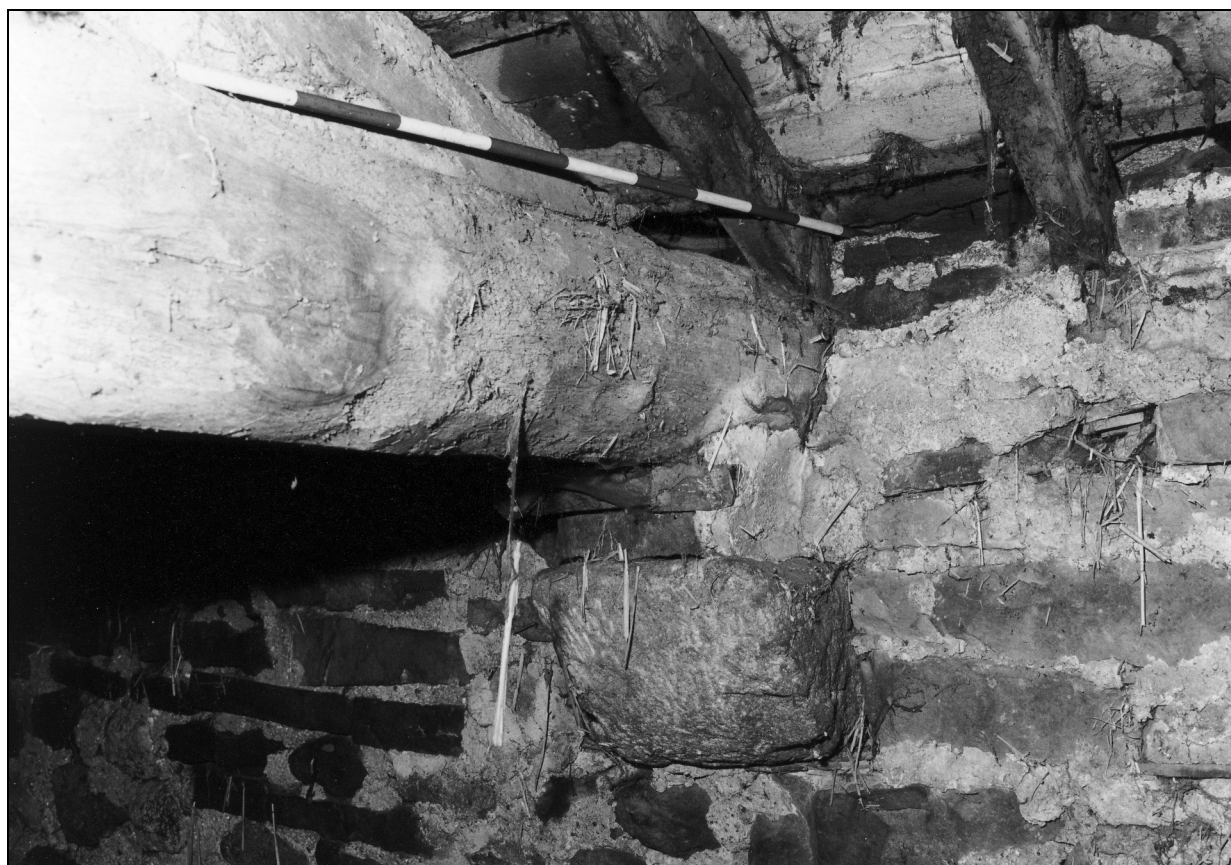
Photo 41: North end of west roof truss, with corbel, from the south-east
