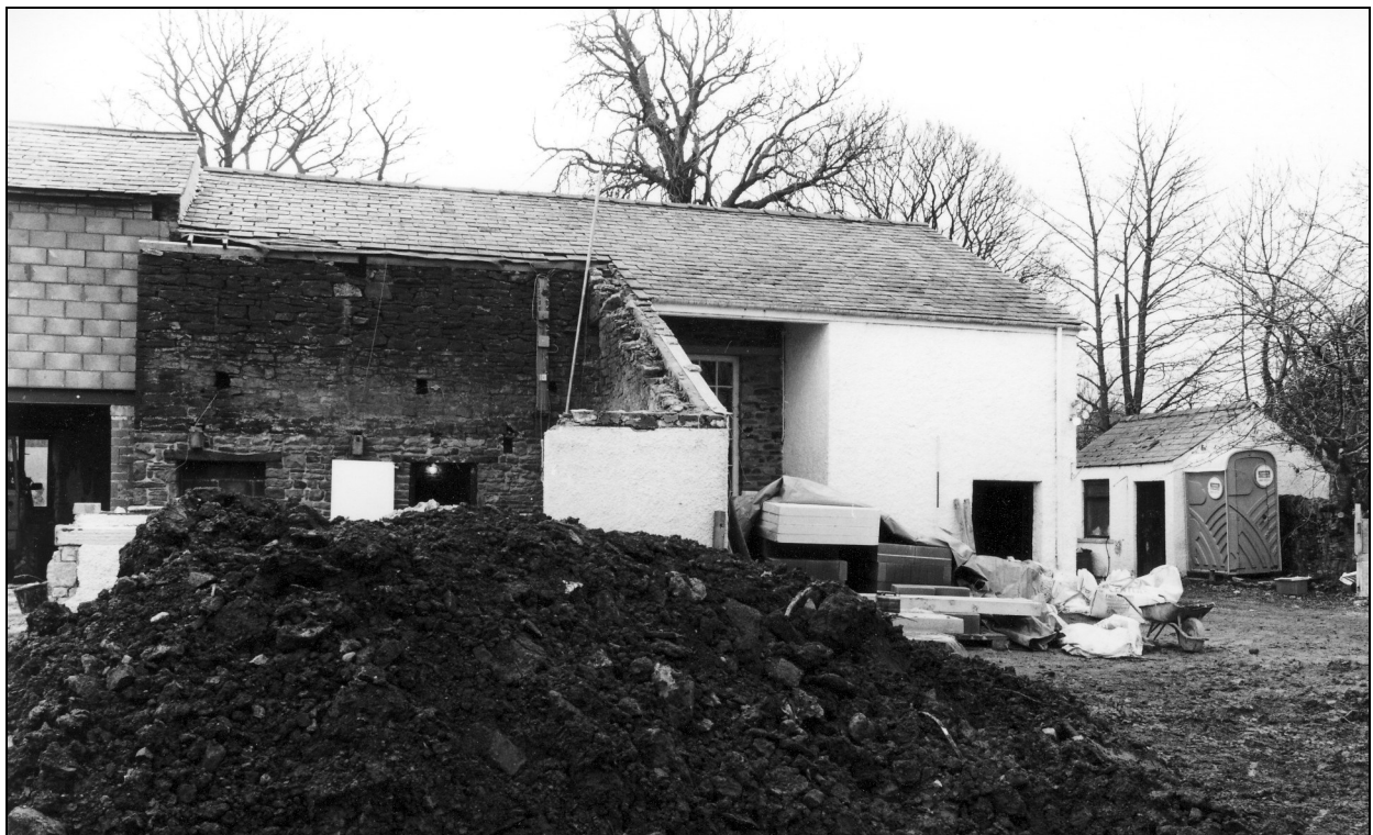
Photo 3: Barn and added shippon, from the north
