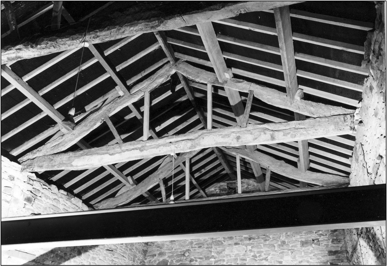
Photo 13: Central truss in barn, from the west
