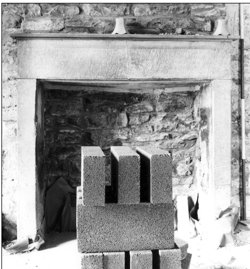
Photo 33: Ground floor fireplace in rear part of house (room 4)
