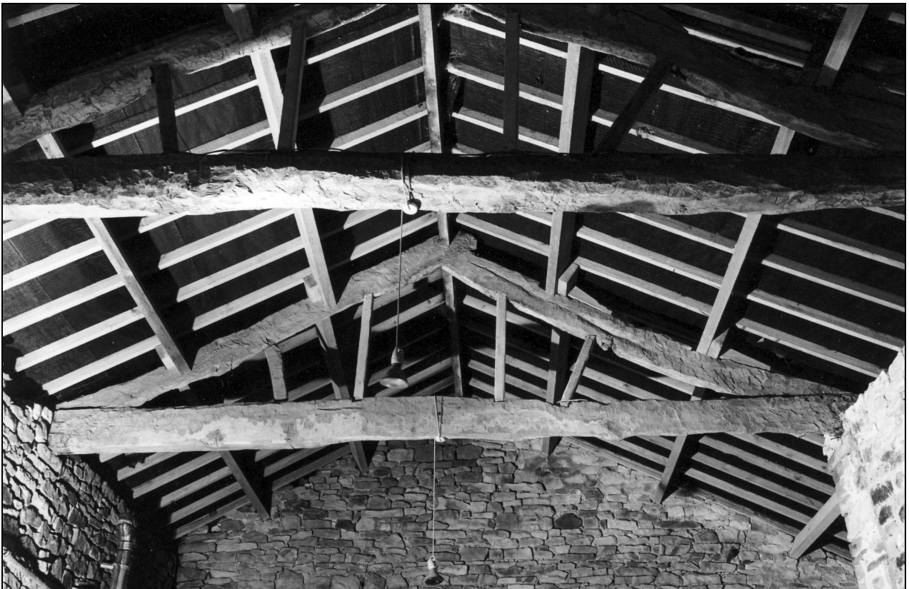
Photo 14: West truss in barn, from the east
