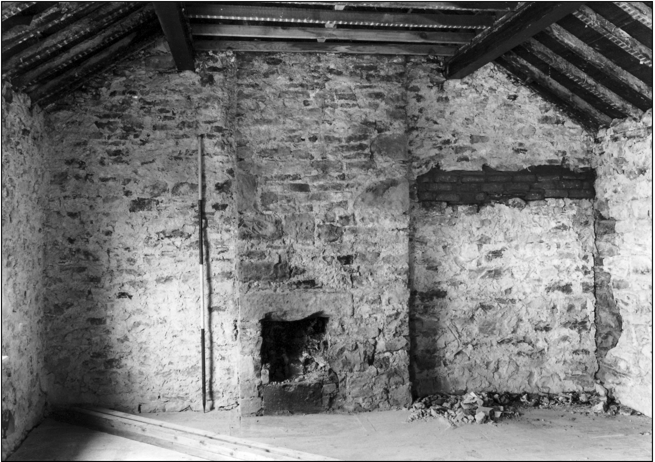
Photo 34: First floor room 9, from the west
