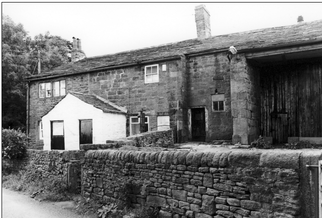
Photo 4: Front elevation of the house and barn, from the south-east
