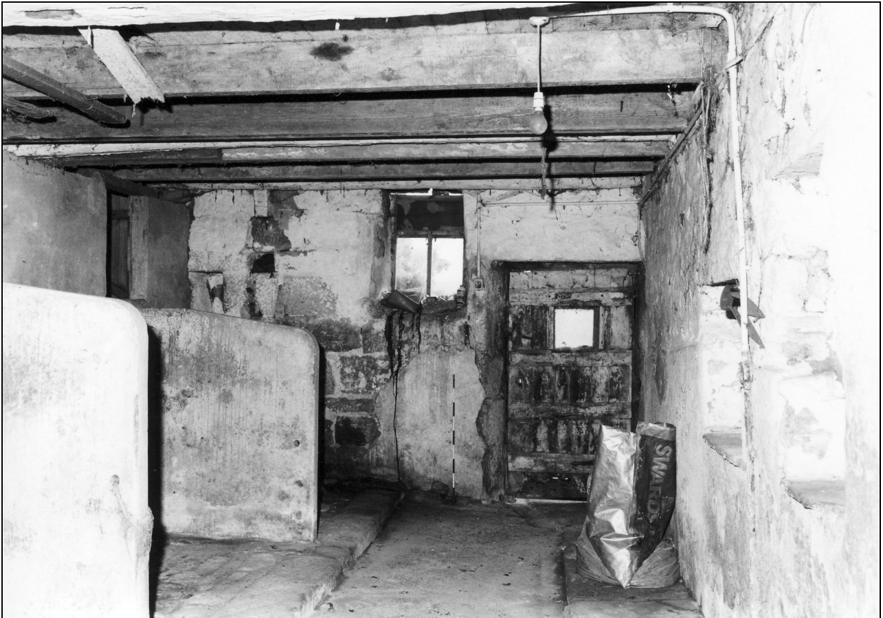
Photo 23: Interior of shippon in west end of barn, from the north
