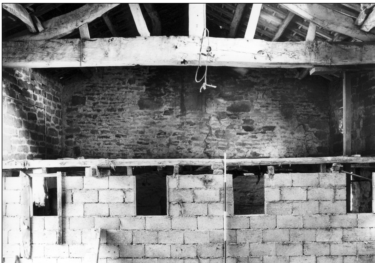
Photo 22: West end of the barn interior, showing rubble wall to house
