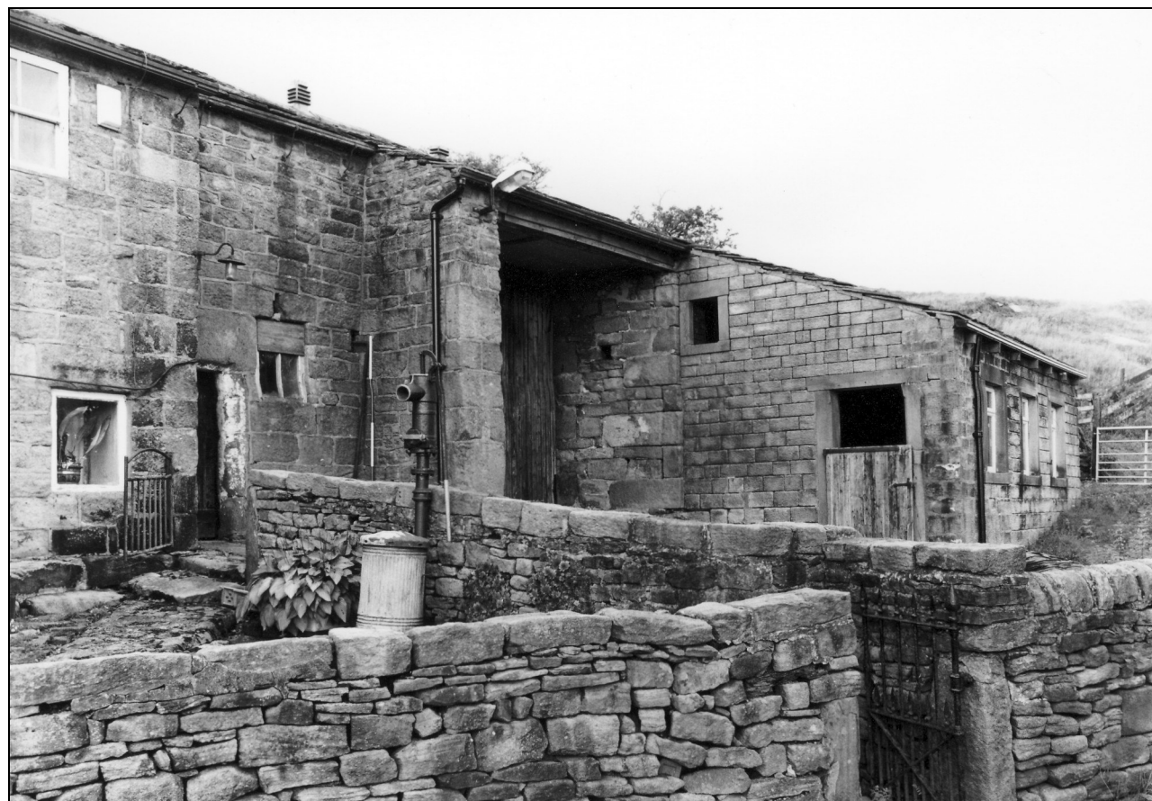
Photo 7: Front elevation of the barn, and later stable, from the south-west
