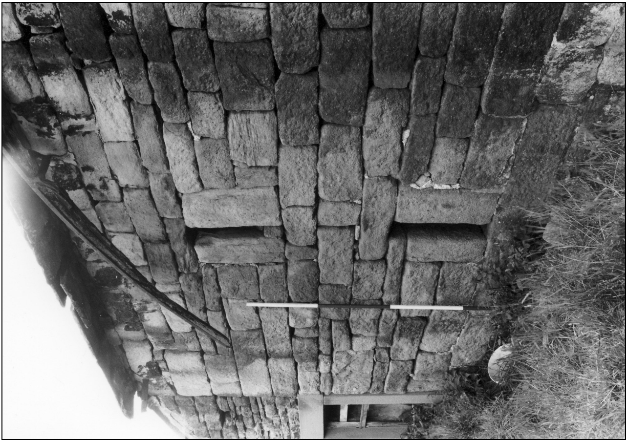
Photo 20: Detail of breathers in rear elevation of the barn
