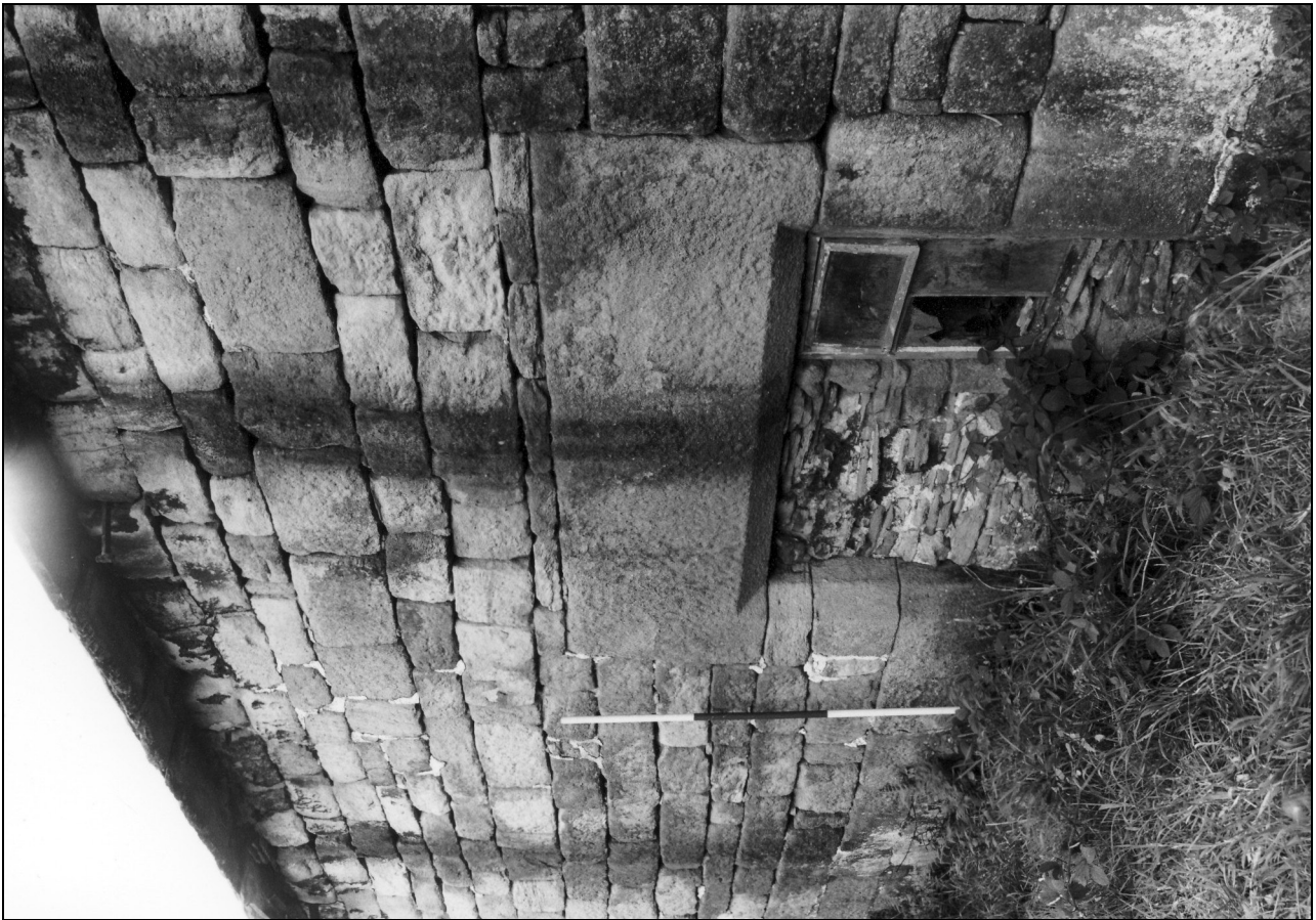
Photo 18: Detail of former doorway in rear elevation of the barn
