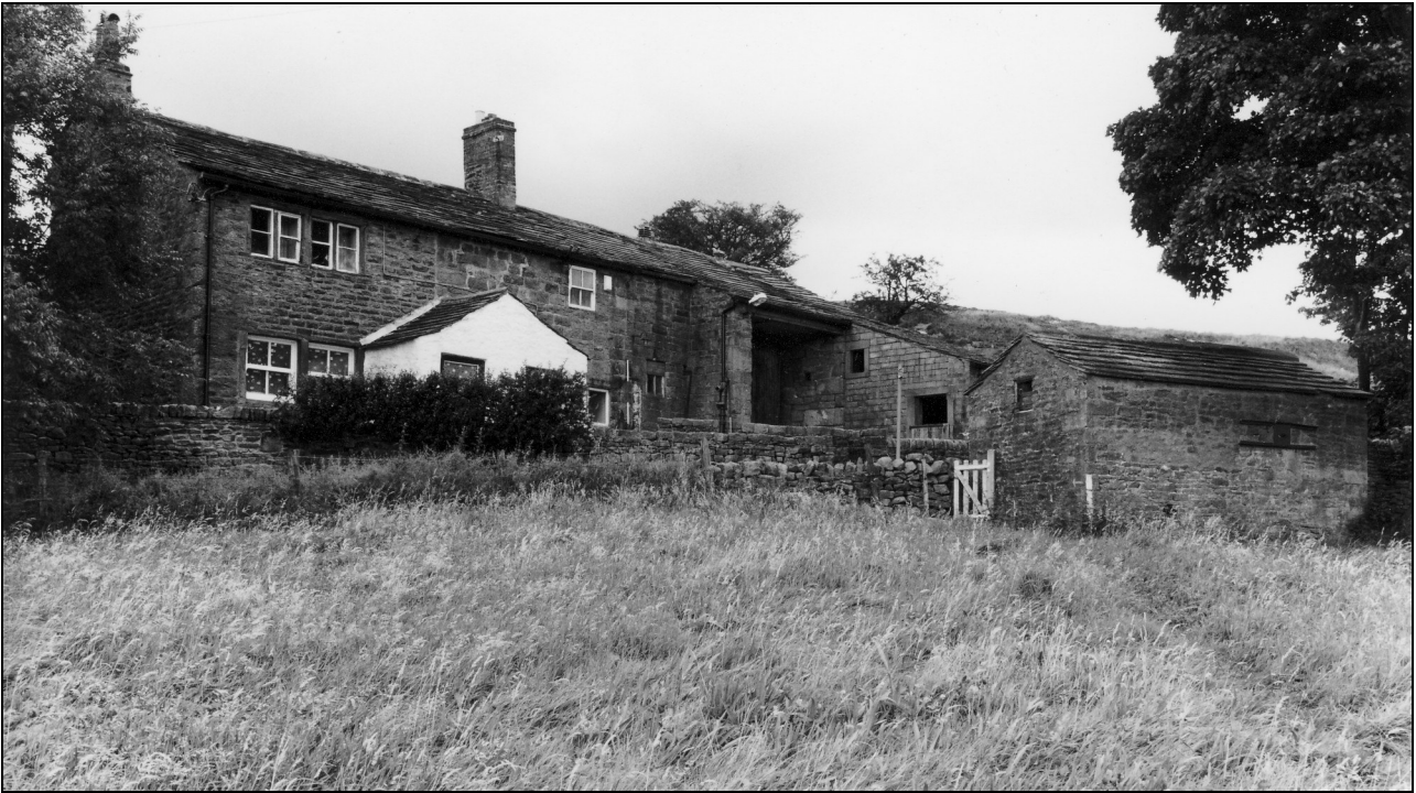
Photo 1: General view, from the south-west
