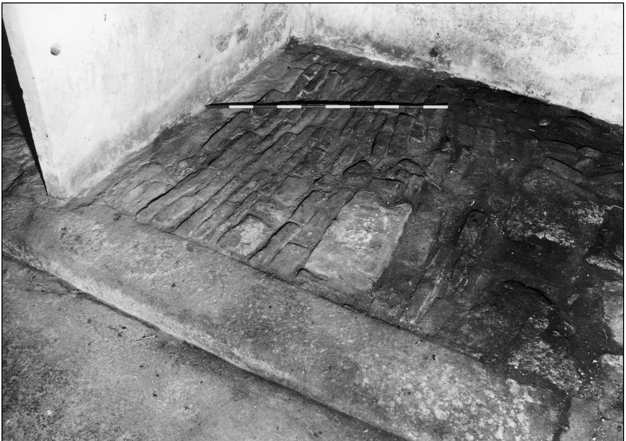
Photo 26: Detail of pitched stones to stalls in shippon
