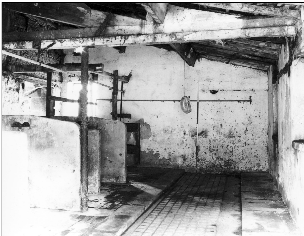
Photo 60: Interior of lean-to shippon at east end
