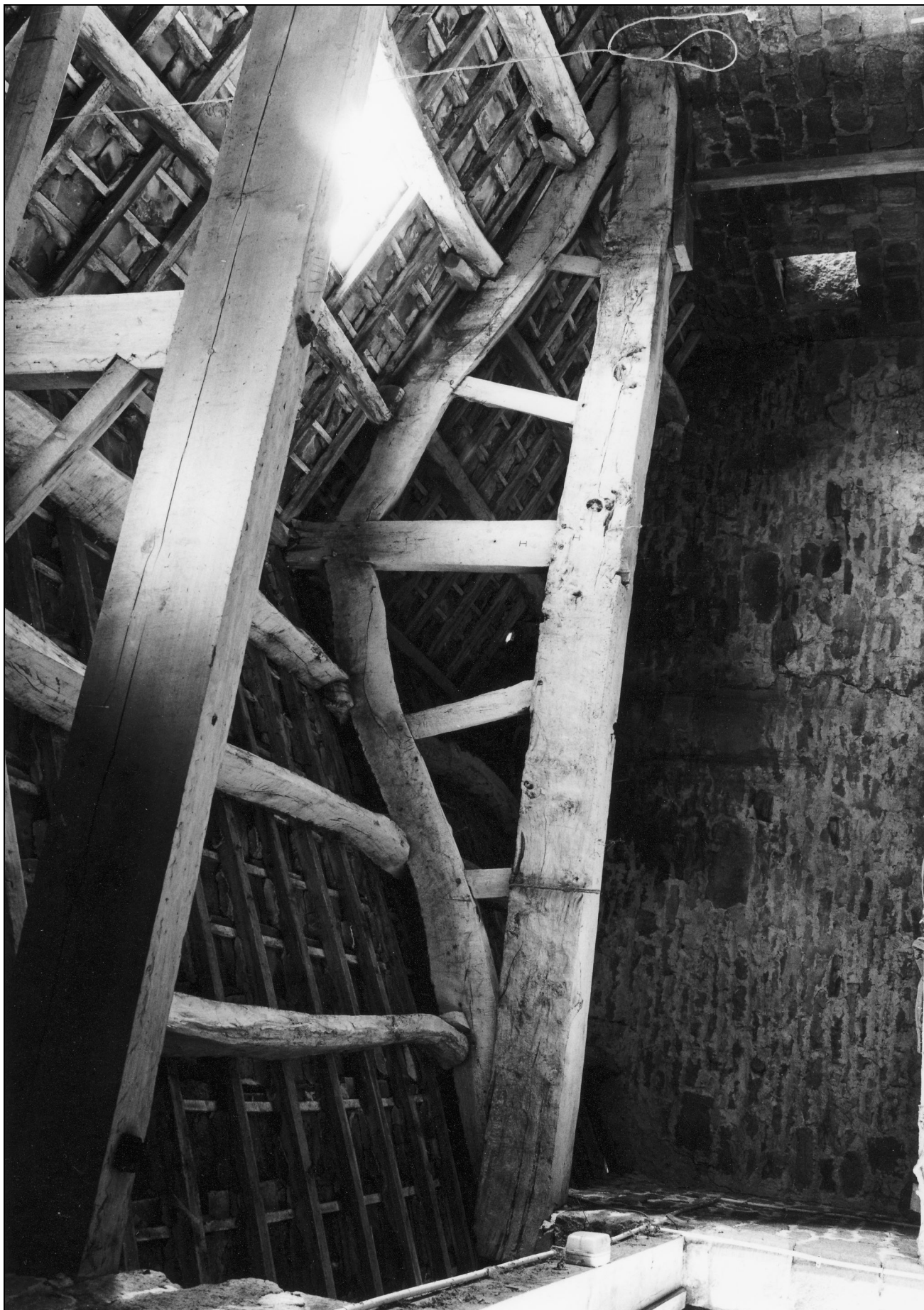
Photo 38: Original roof truss in the barn, from the east
