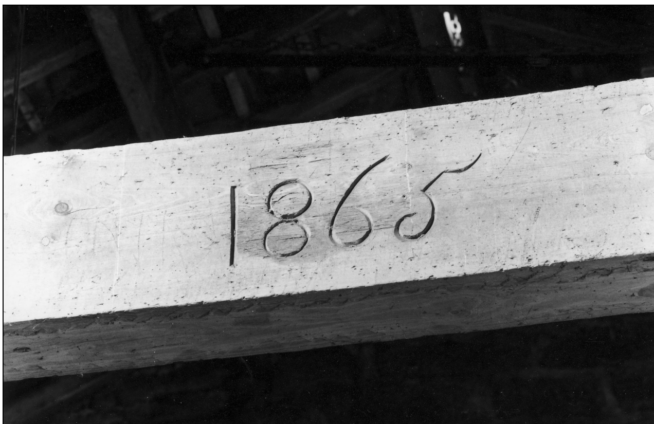
Photo 48: Date carved tie-beam of later truss in barn (west side)
