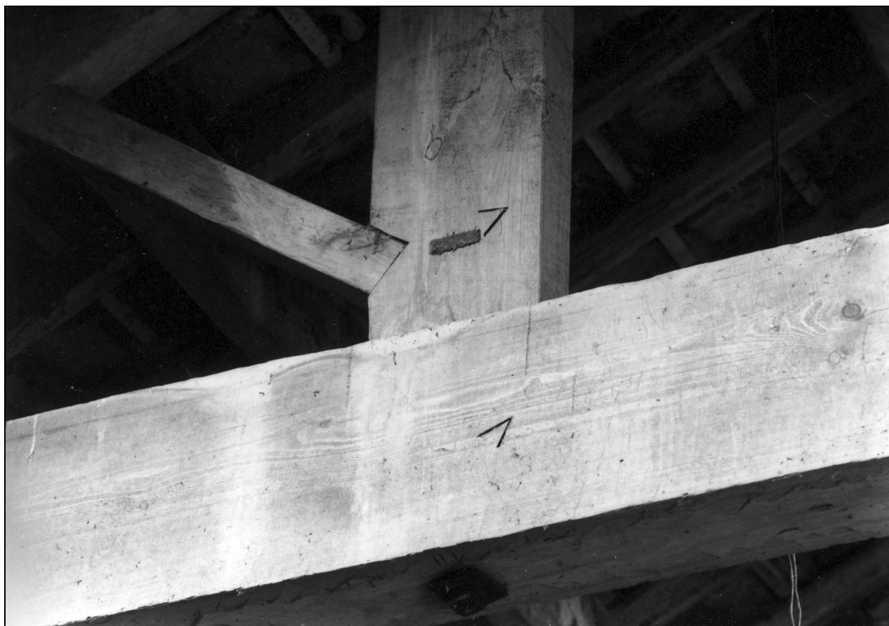
Photo 49: Assembly numbers carved in later truss in barn (west side)
