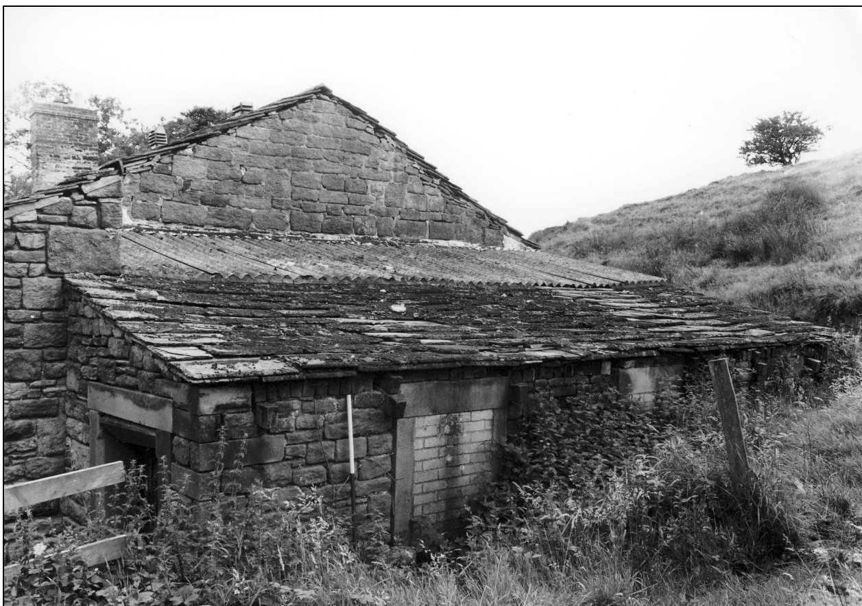
Photo 59: Lean-to shippon against east gable of barn, from the south-east
