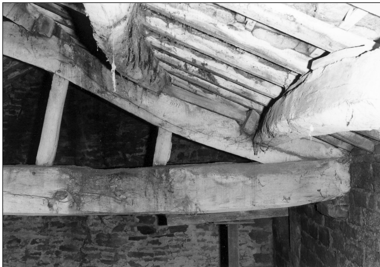
Photo 41: Upper face of west truss in barn: north end
