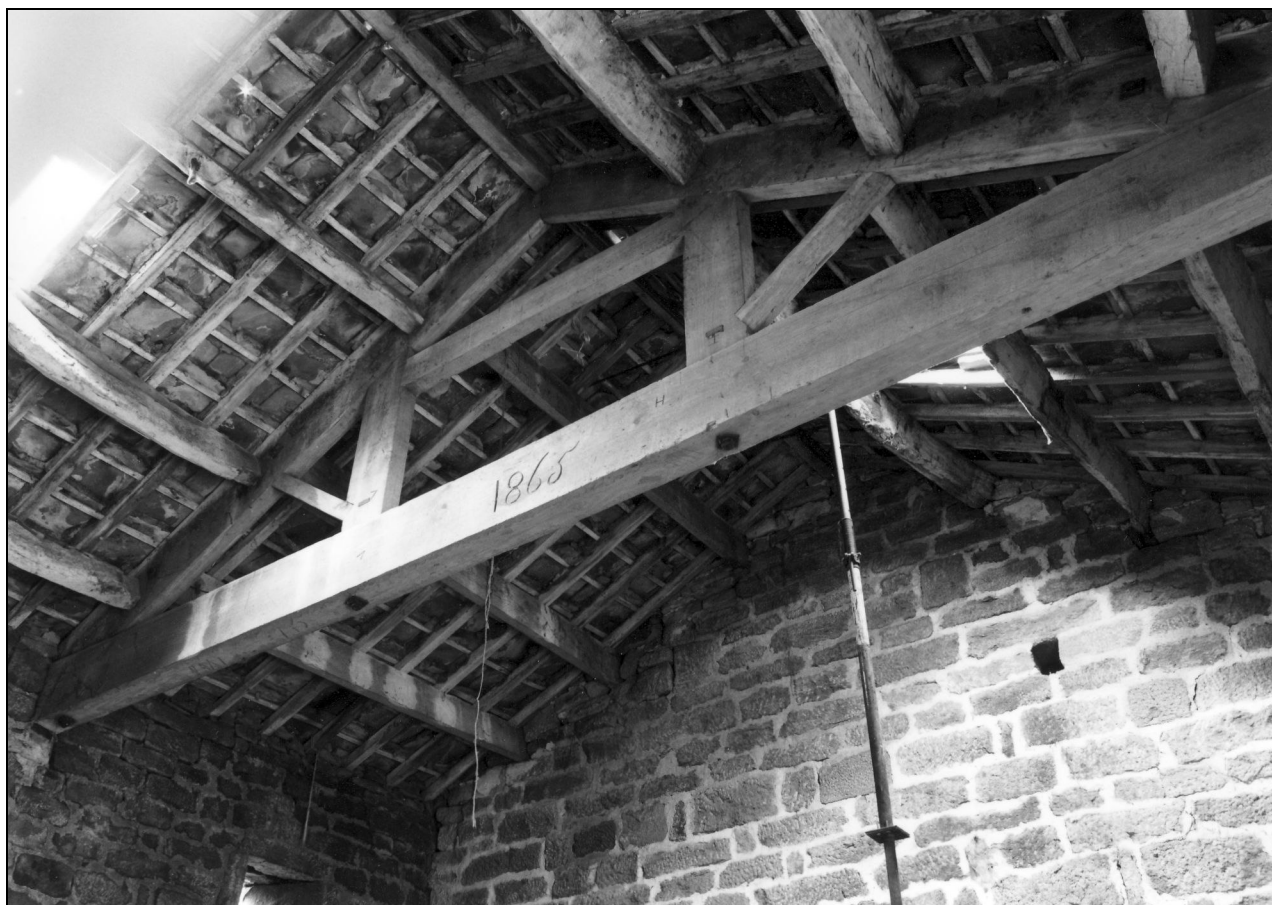
Photo 47: East truss in barn, from the south-west (dated 1865)
