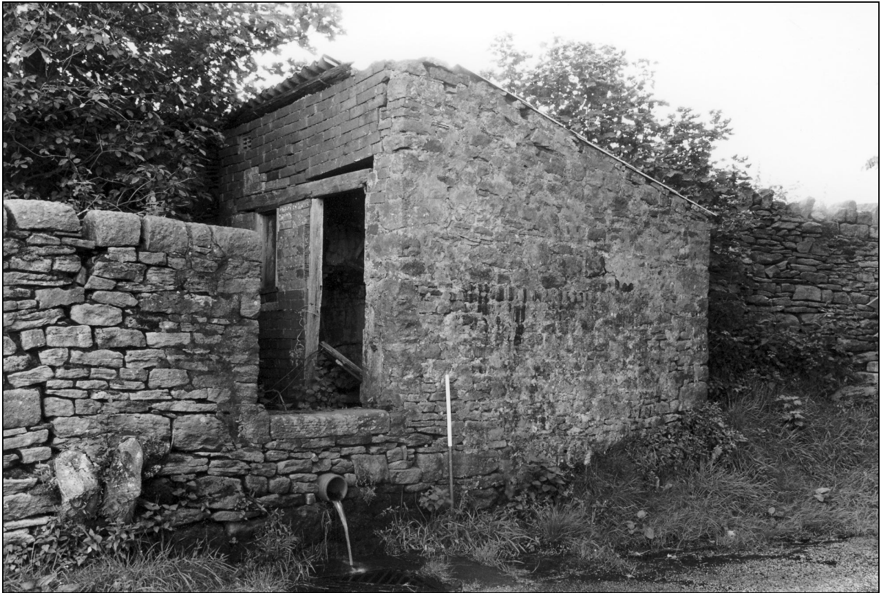
Photo 65: Outbuilding on north side of road, from the south-west
