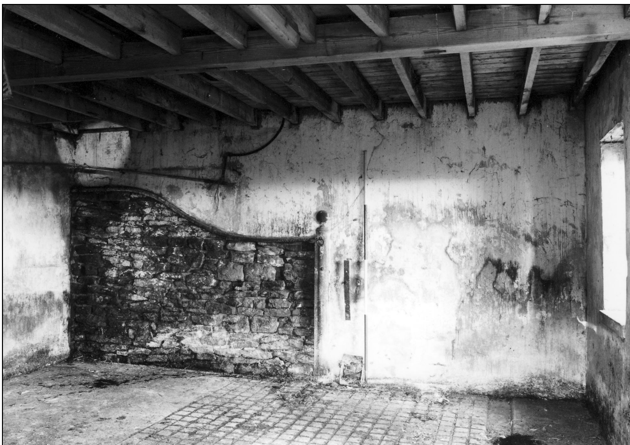
Photo 54: Interior of added stable, from the west
