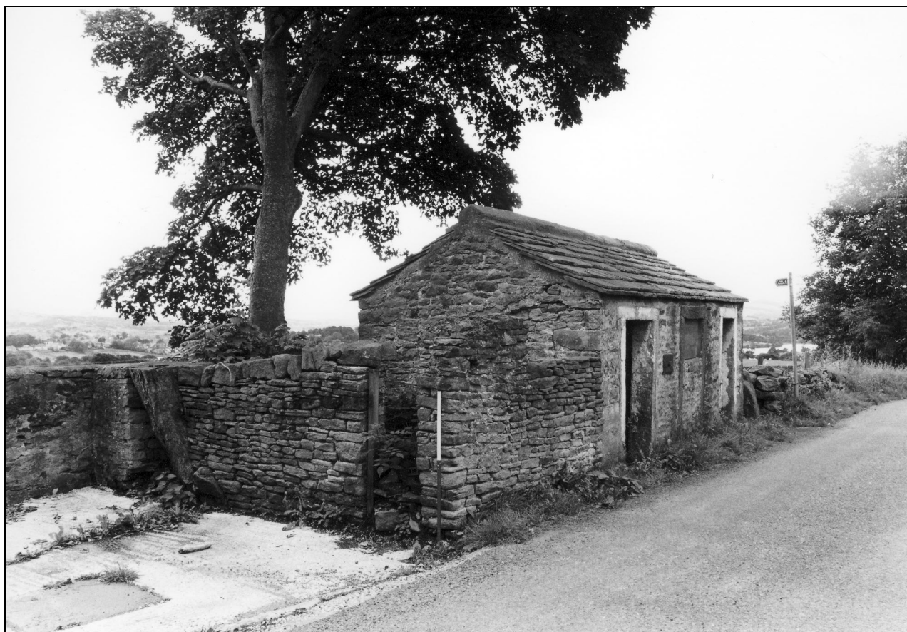
Photo 63: Outbuilding on south side of road, from the north-east
