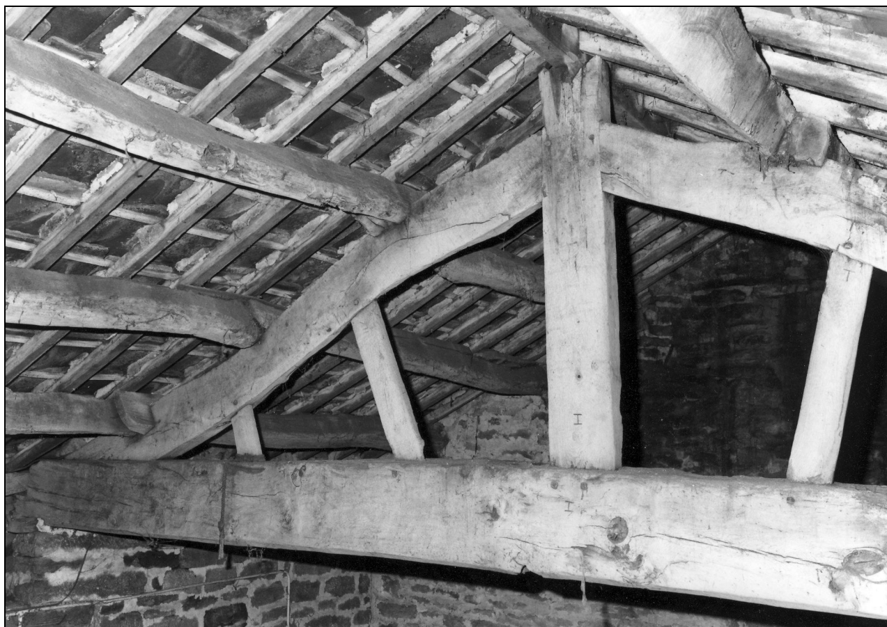
Photo 39: Upper face of west truss in barn, from the north-east
