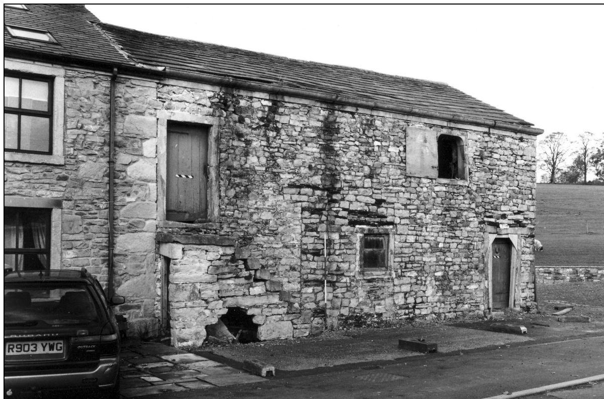
Photo 3: Front elevation, from the south-west
