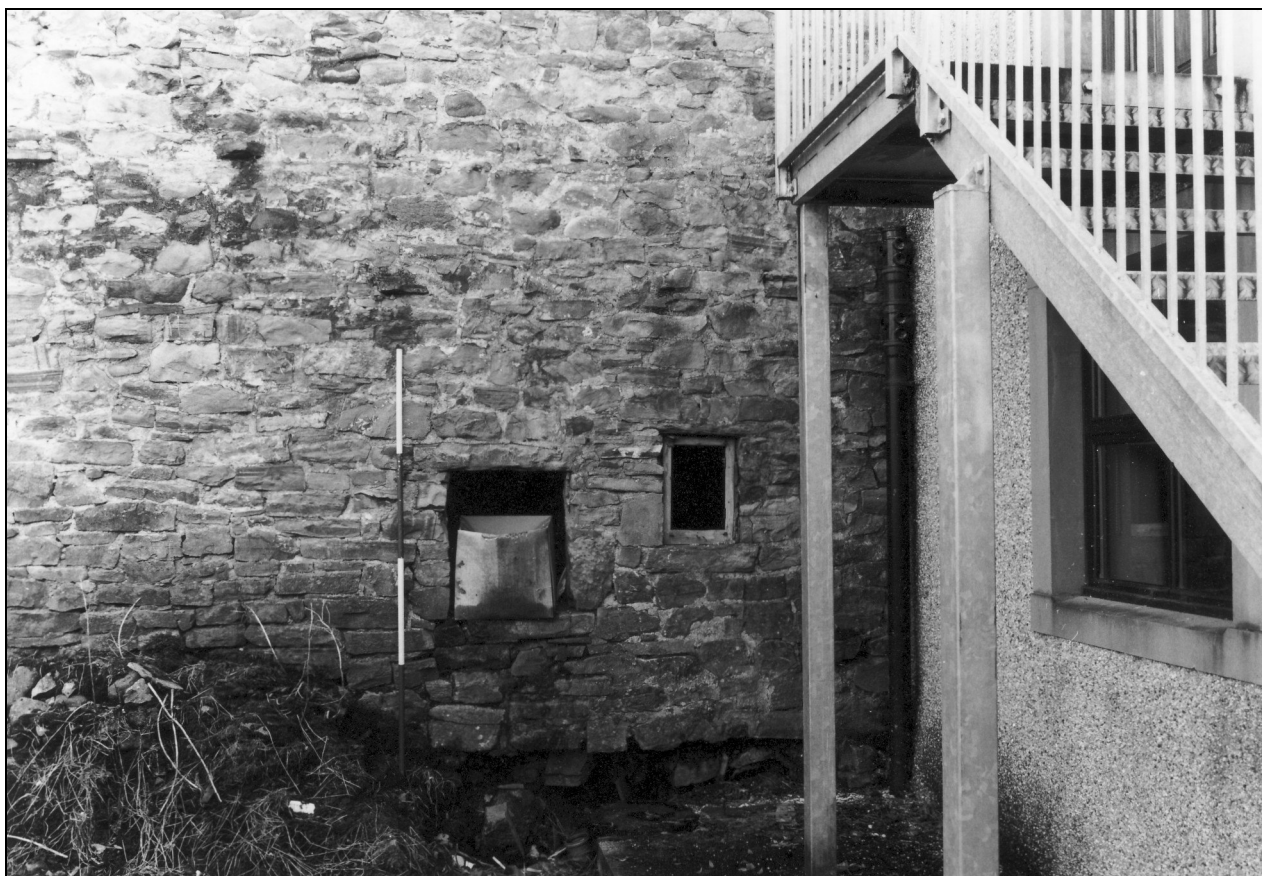
Photo 15: Ground floor openings in rear elevation
