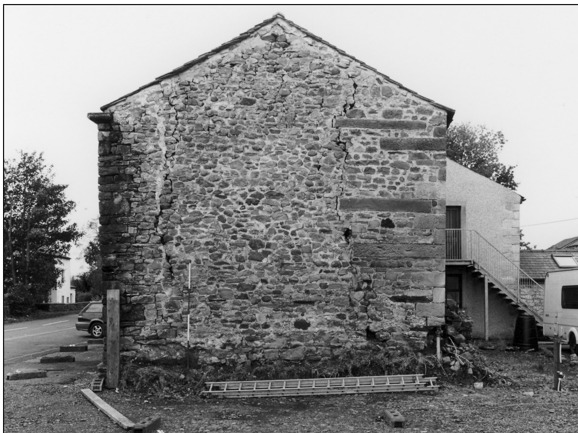
Photo 10: East gable of the stable
