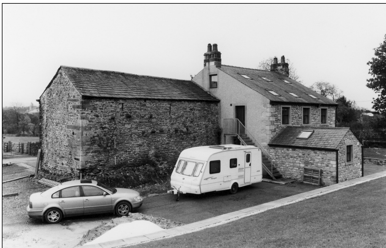
Photo 12: Stable and house, from the north-east
