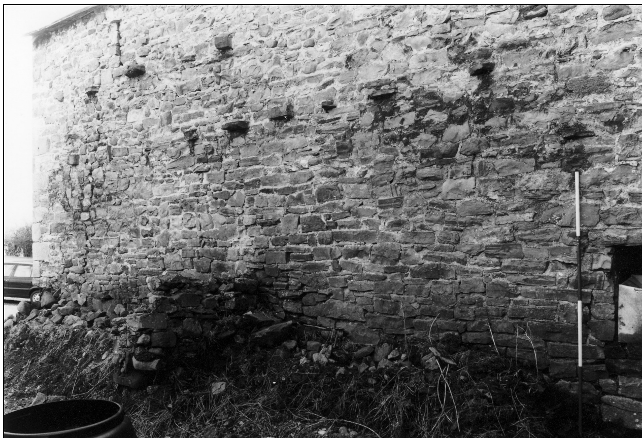
Photo 14: Rear elevation, from the north-west
