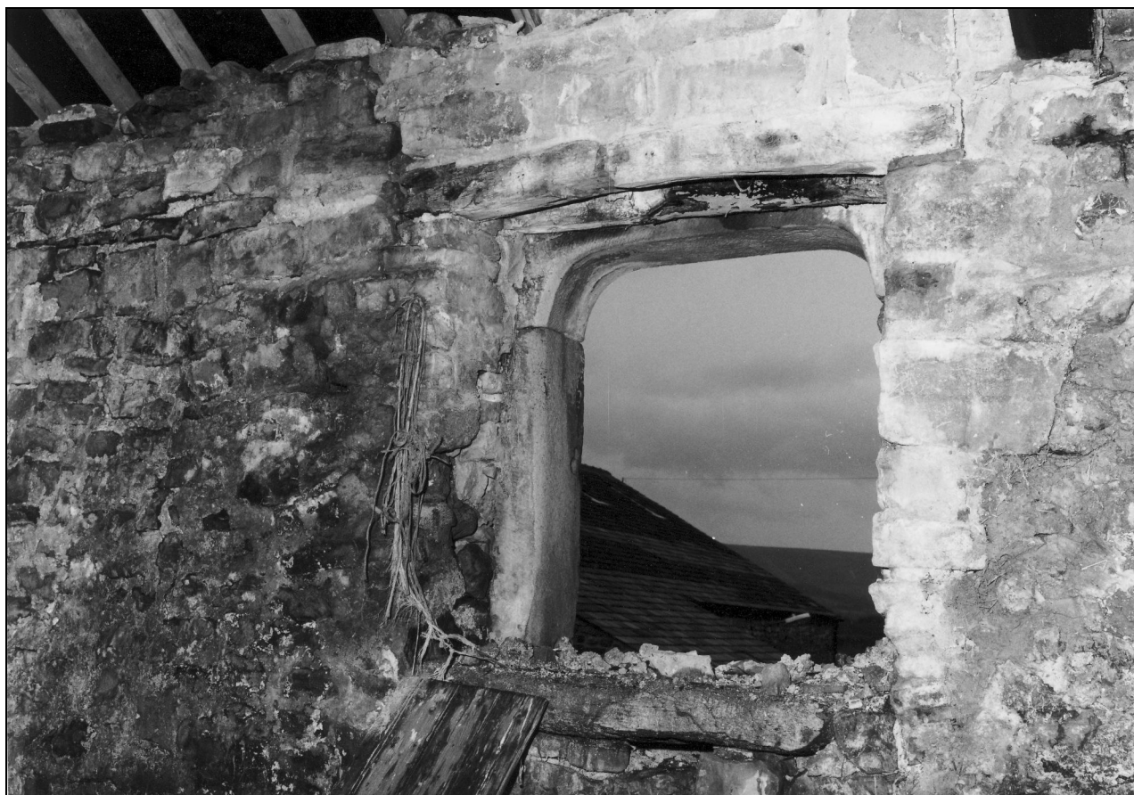
Photo 26: Internal view of forking hole in front elevation
