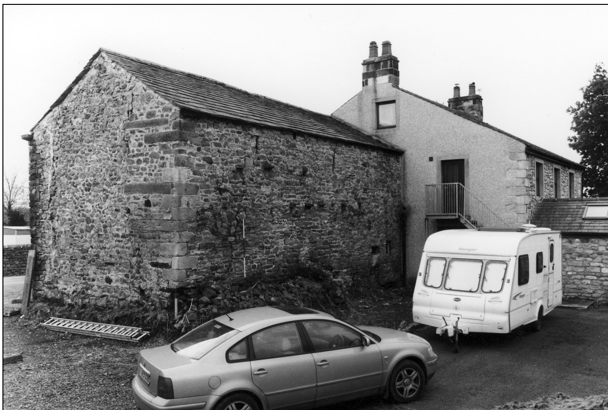
Photo 13: Stable and house, from the north-east
