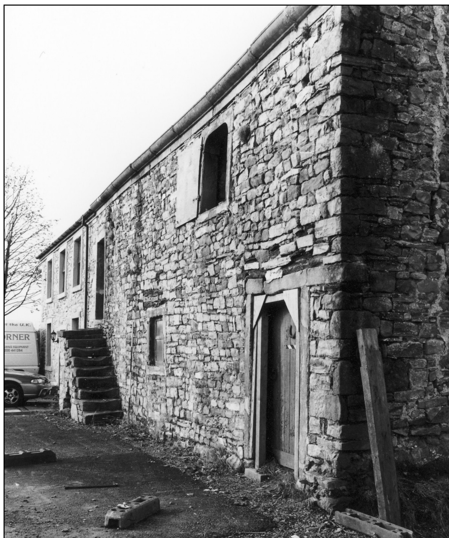
Photo 4: Front elevation, from the east
