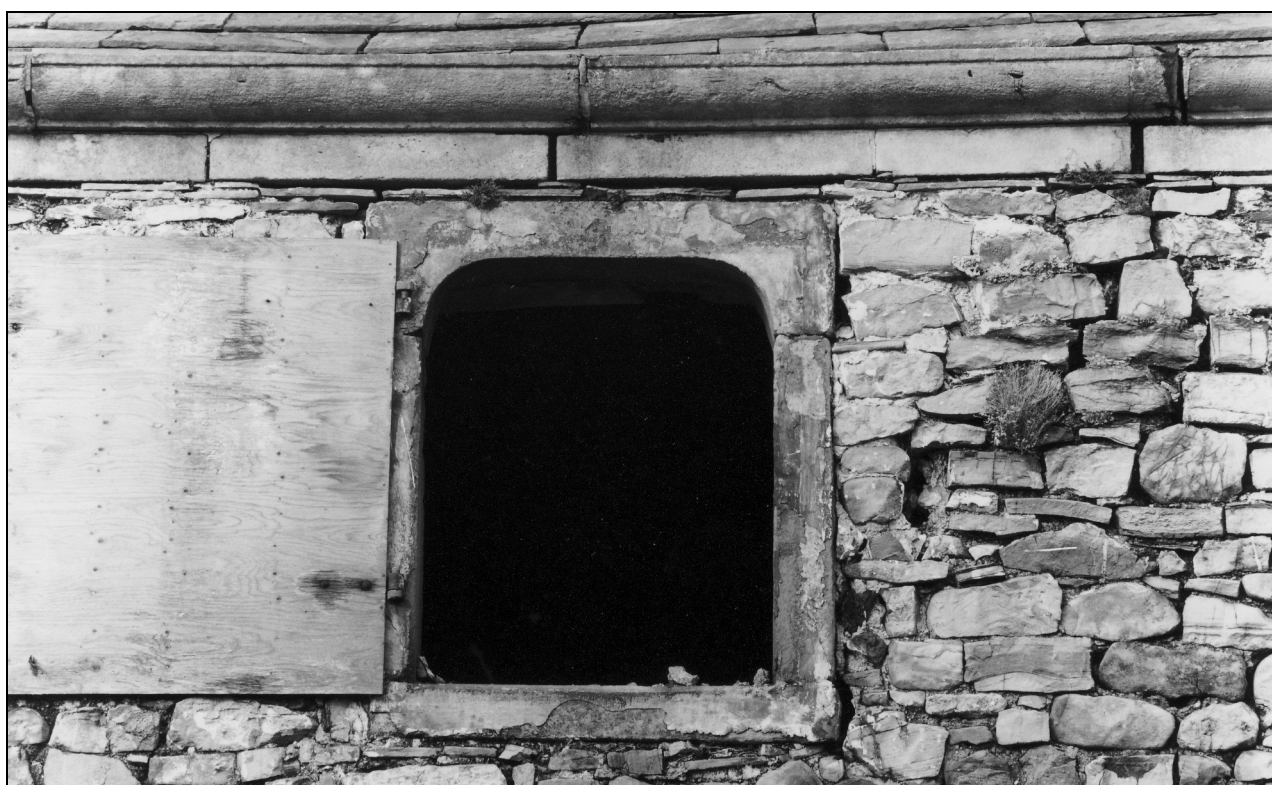
Photo 8: Detail of forking hole and gutter in front elevation
