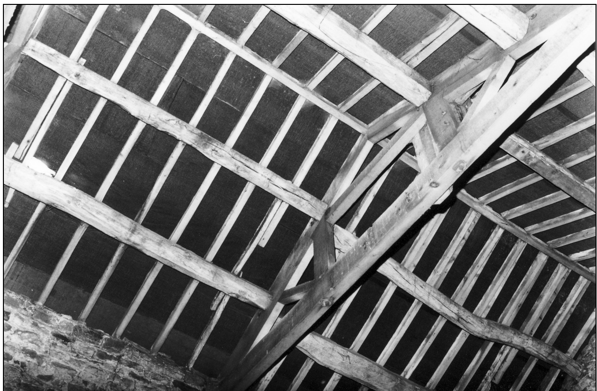
Photo 18: View of underside of barn roof, from the west
