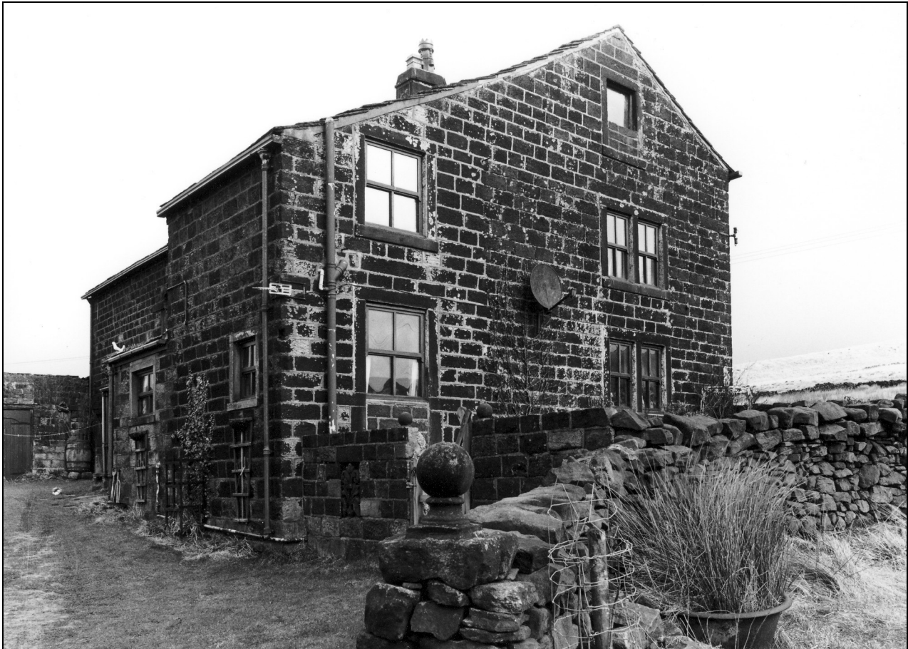
Photo 3: The house, from the south
