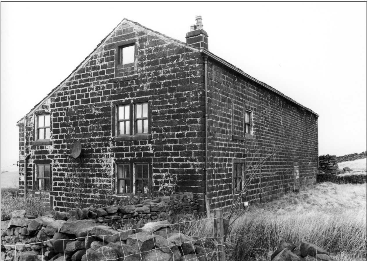
Photo 6: House and barn, from the south-east
