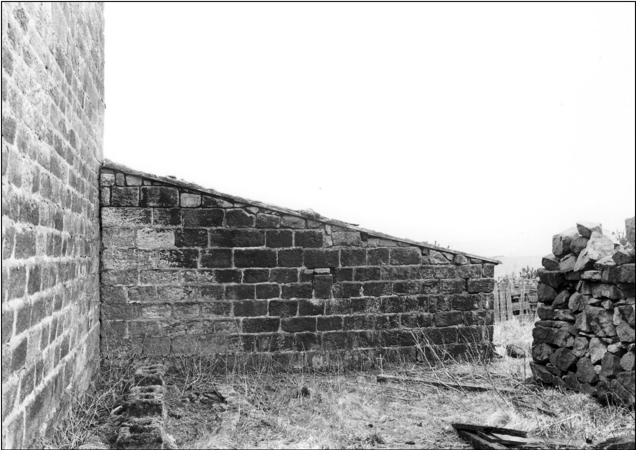
Photo 21: East side of north-west addition
