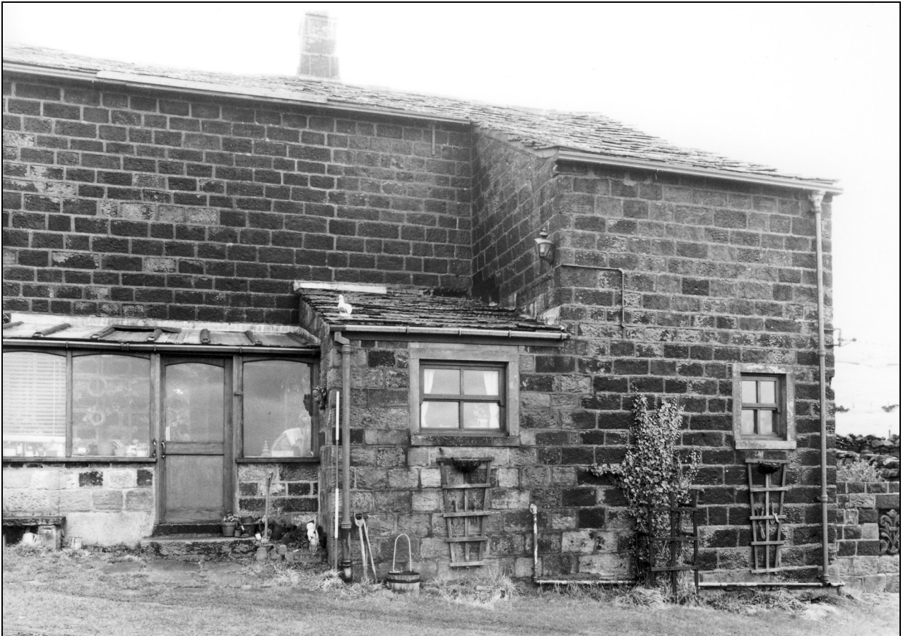
Photo 5: House and south end of barn, from the west
