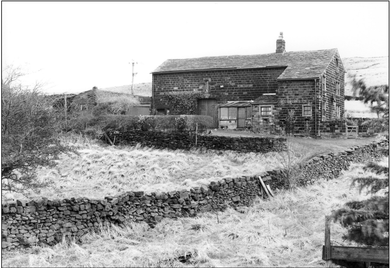
Photo 1: General view of the house and barn, from the south-west
