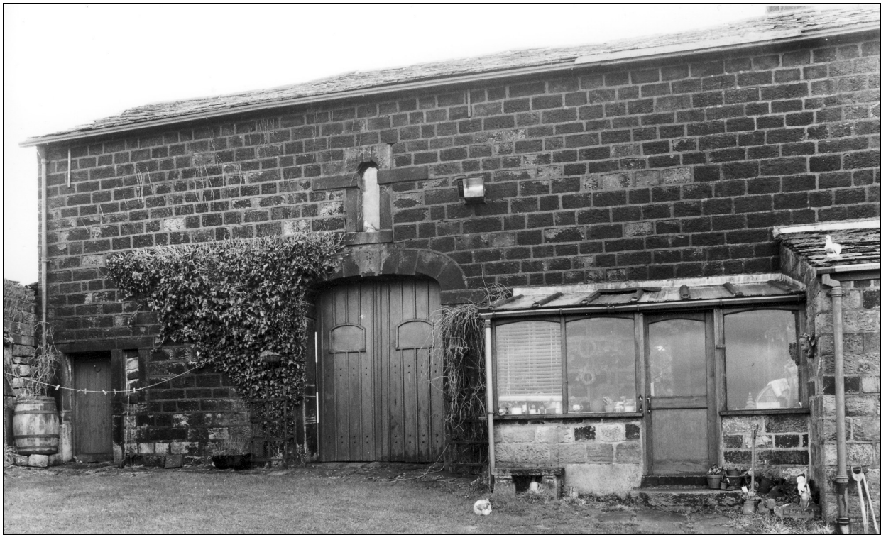
Photo 9: The barn, from the south-west
