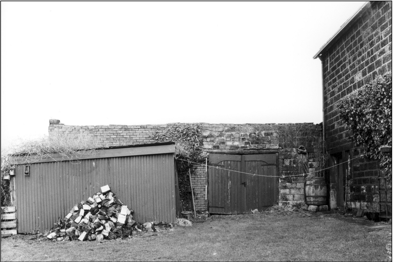
Photo 19: North-west addition, from the south
