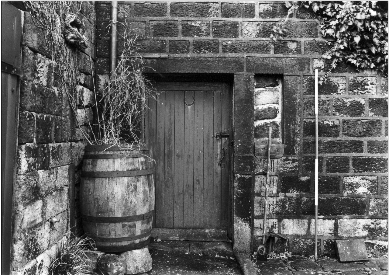
Photo 13: Detail of doorway at north end of barn
