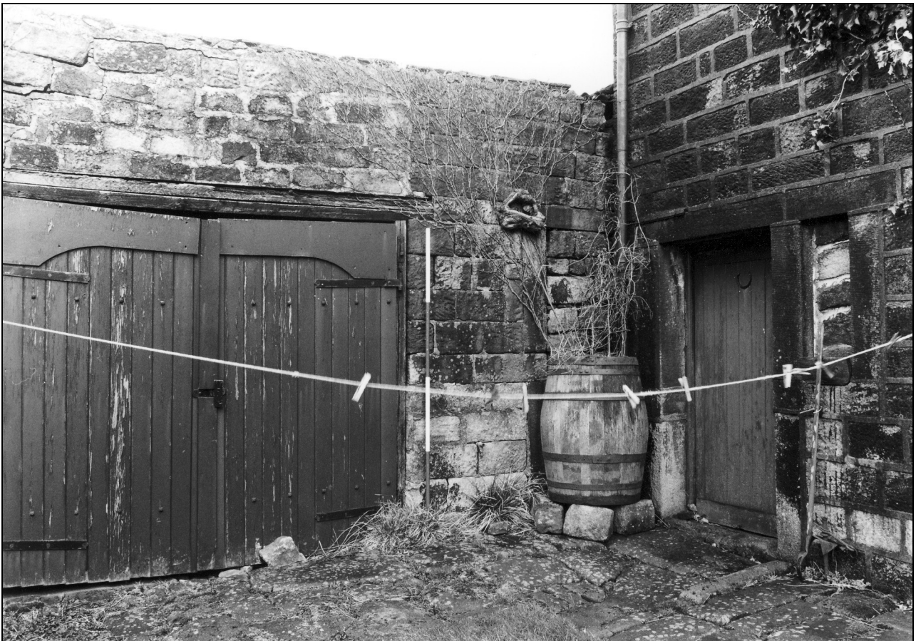
Photo 20: Detail of blocked doorway into addition, from the south-west
