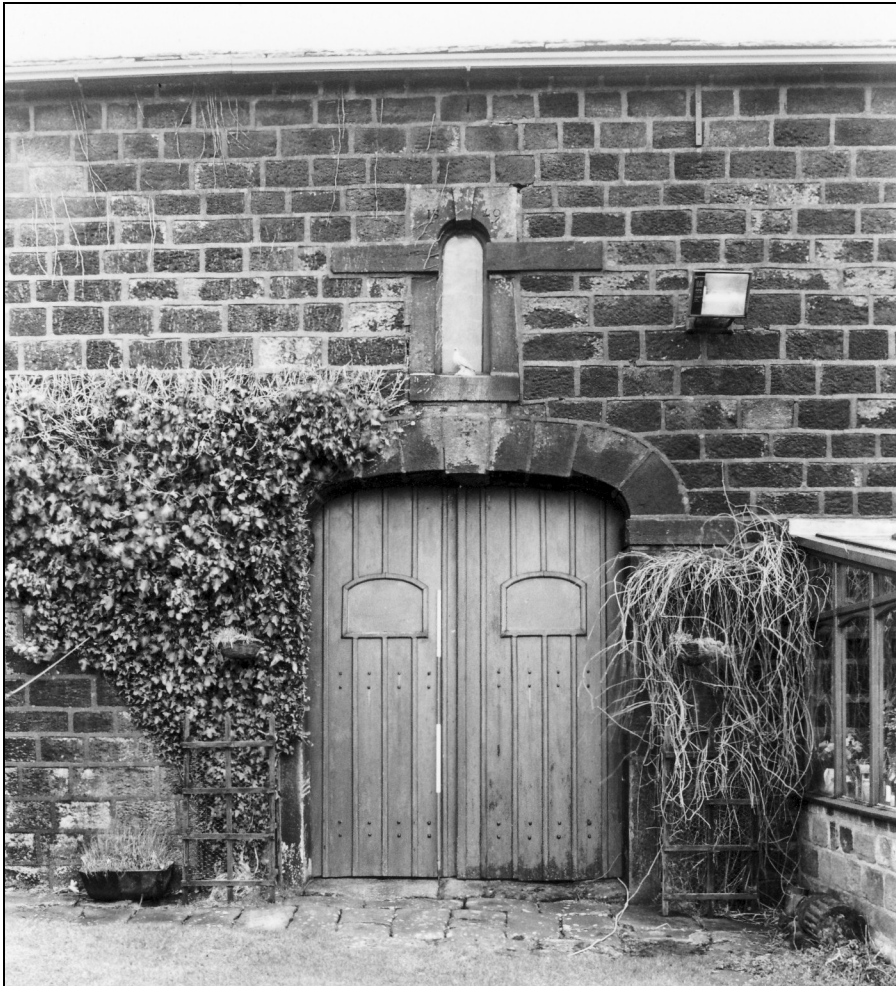
Photo 11: Detail of cart entrance to barn, and window over
