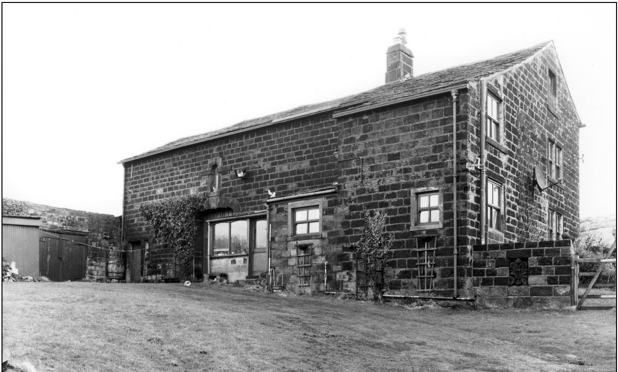
Photo 2: House and barn, from the south-west
