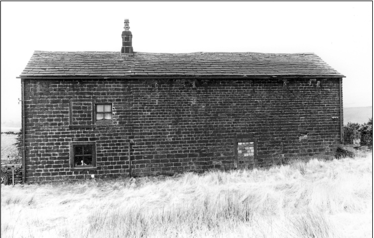
Photo 7: Rear elevation of house and barn
