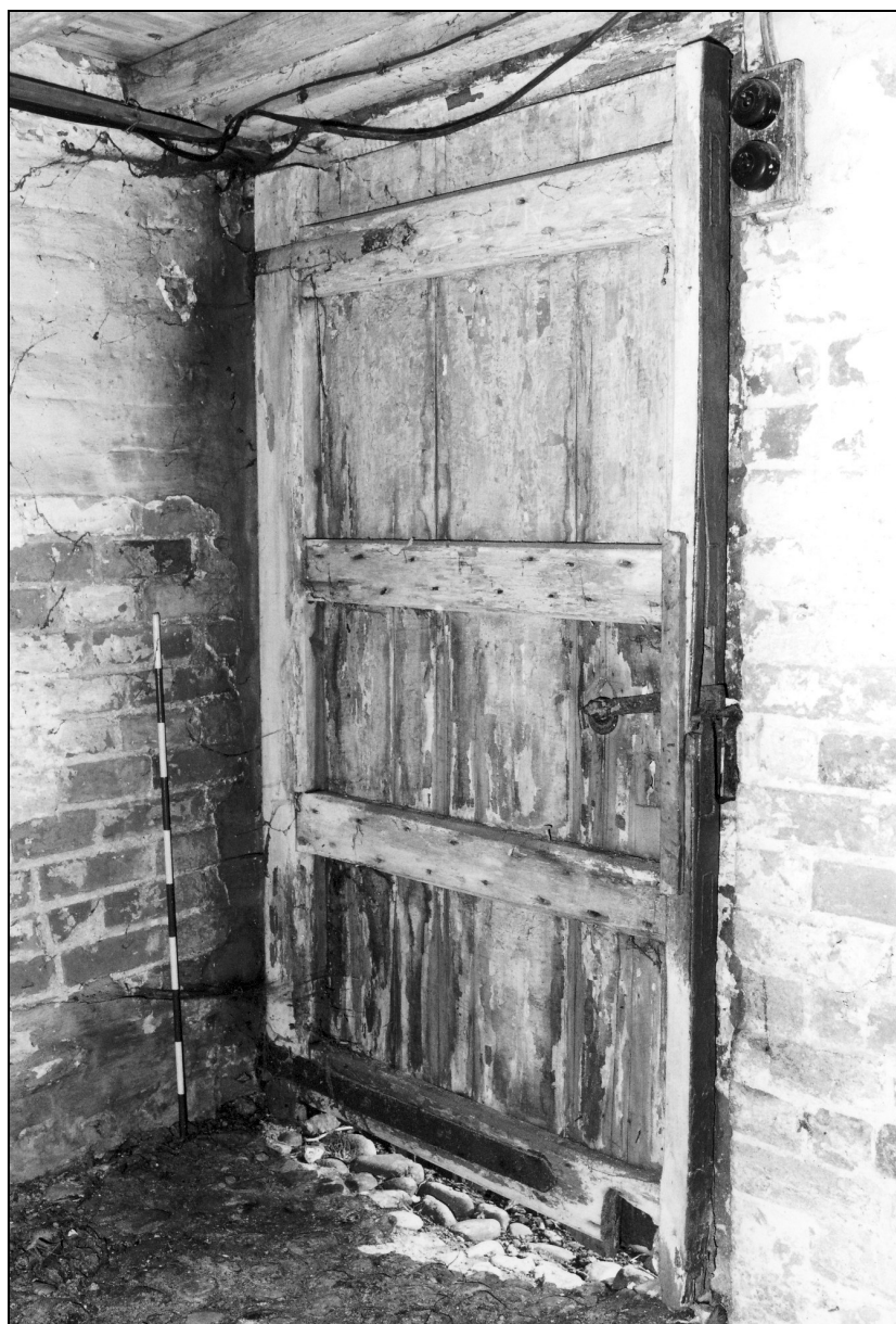
Photo 9: Detail of south door (internal face)
