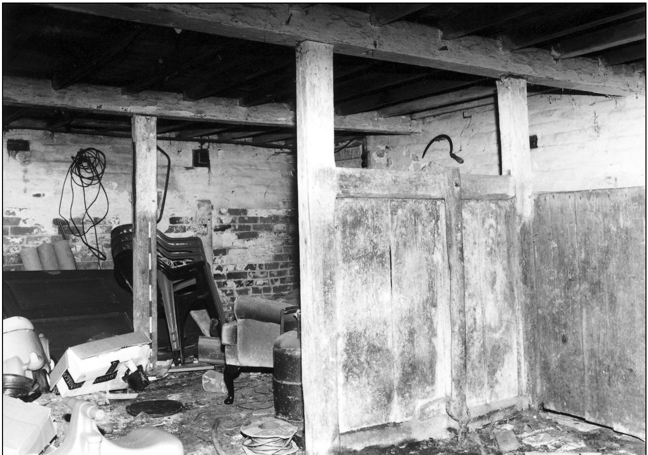
Photo 15: Remains of stalls, from the north-west
