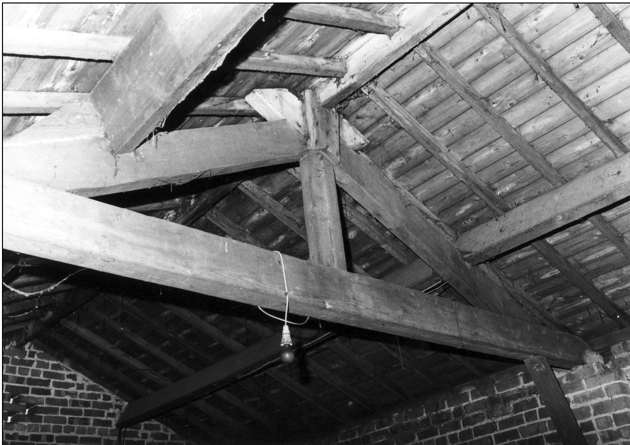
Photo 25: Roof truss, from the north-west
