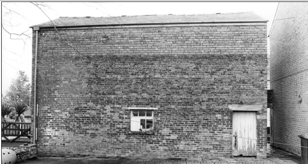
Photo 7: Rear elevation of the shippon
