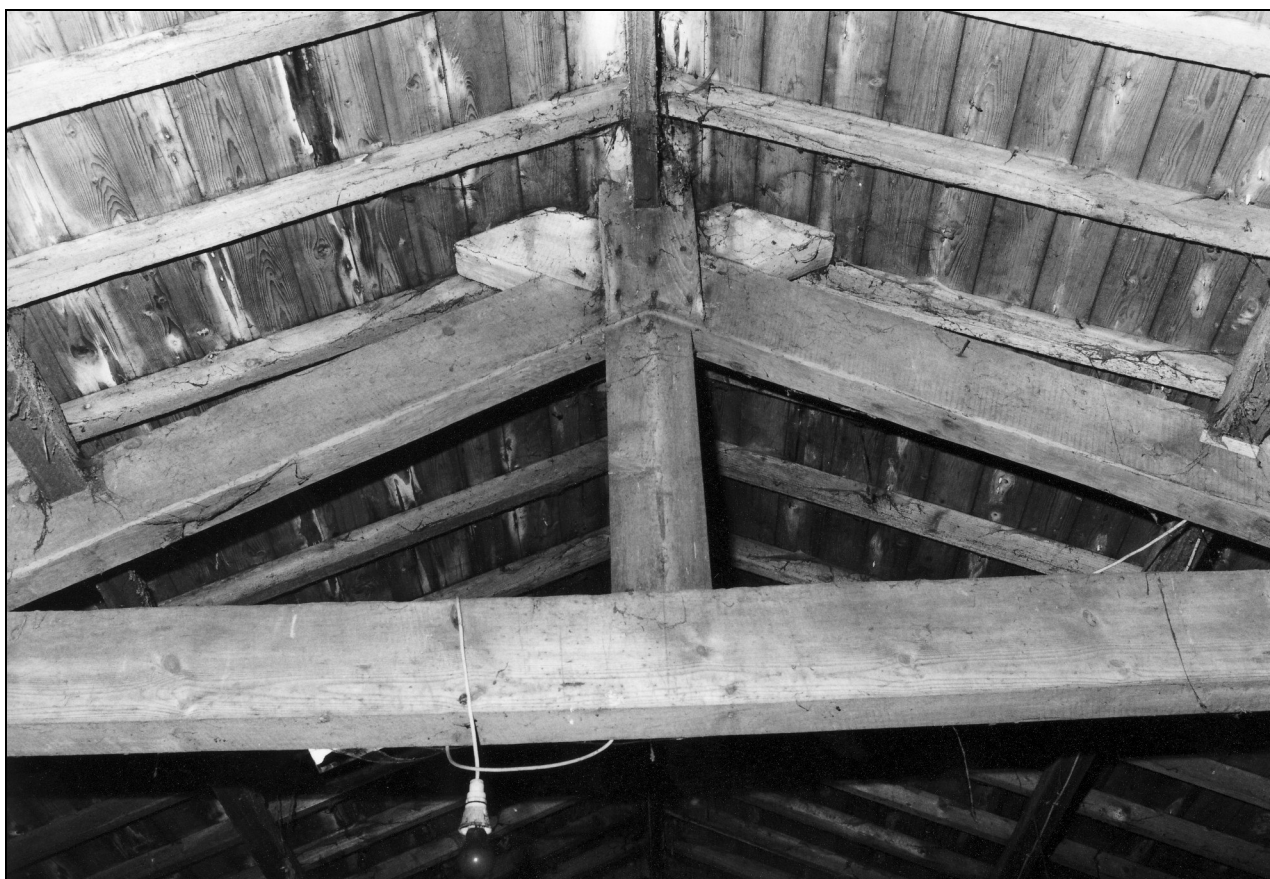
Photo 26: Roof truss, from the west
