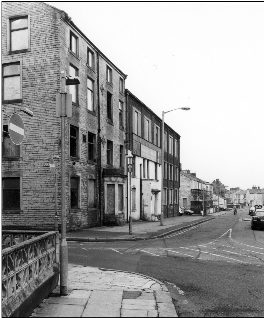
Photo 2: View of the building from the north-east (Every Street elevation)
