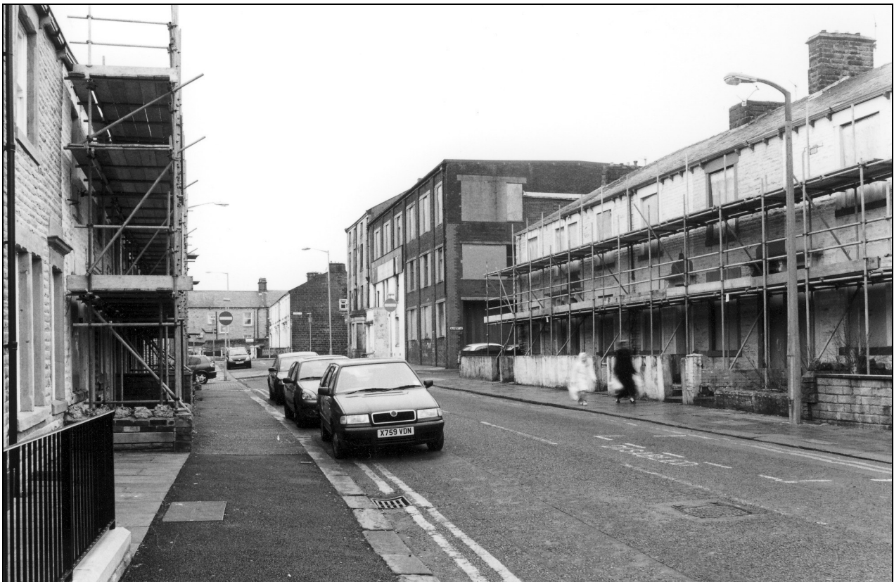
Photo 3: Distant view of the building from the south-west, along Every Street
