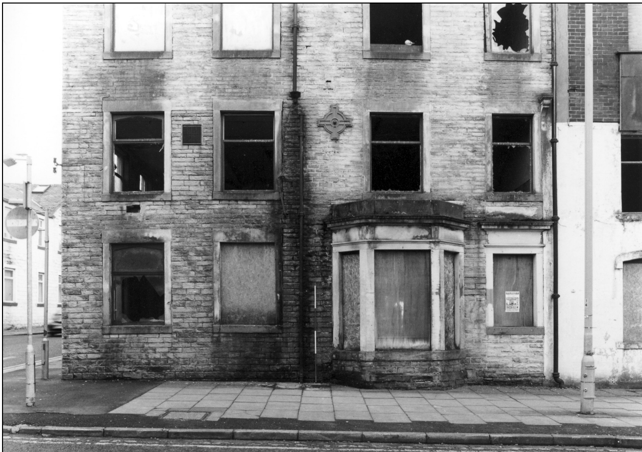
Photo 5: Lower part of Every Street elevation, of no. 109
