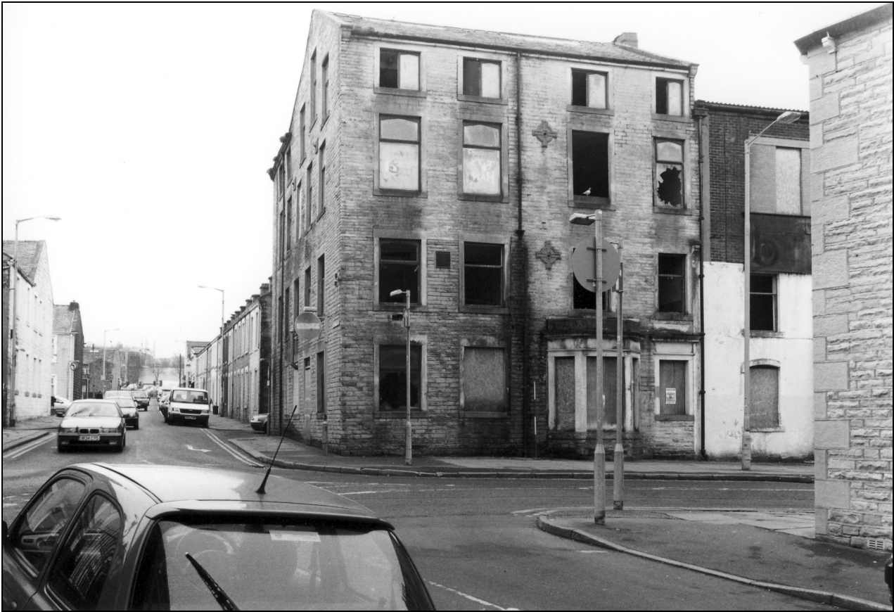
Photo 4: View of the building from the north (Every Street elevation)
