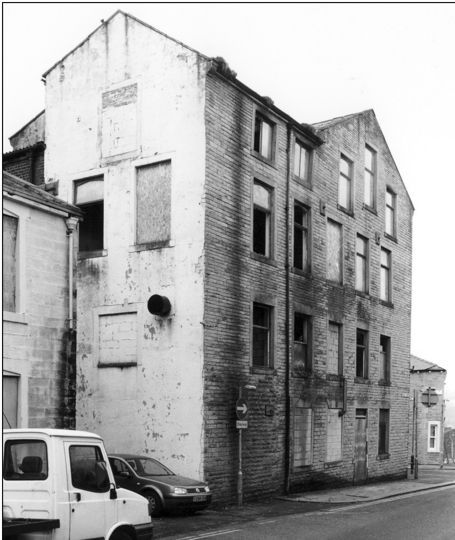
Photo 7: View of the building from the east (Stanley Street elevation)
