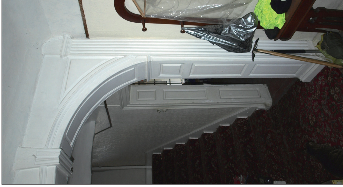
Photo 4: Moulded timber arch between entrance hall and stairs
