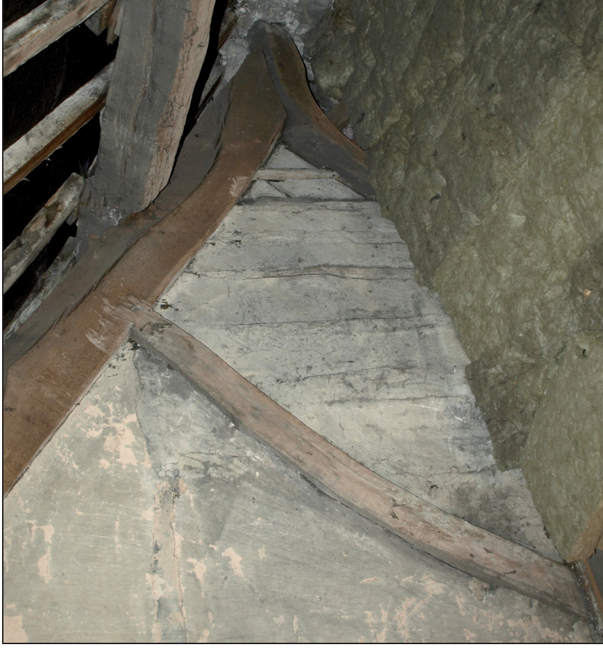
Photo 15: Lower part of roof truss in attic, west side of house
