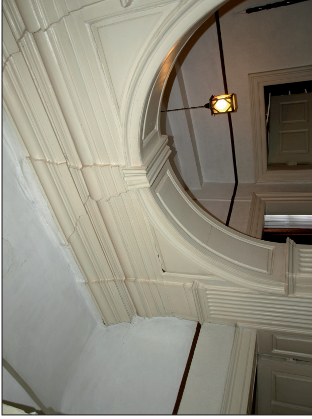
Photo 12: Arch on first floor
