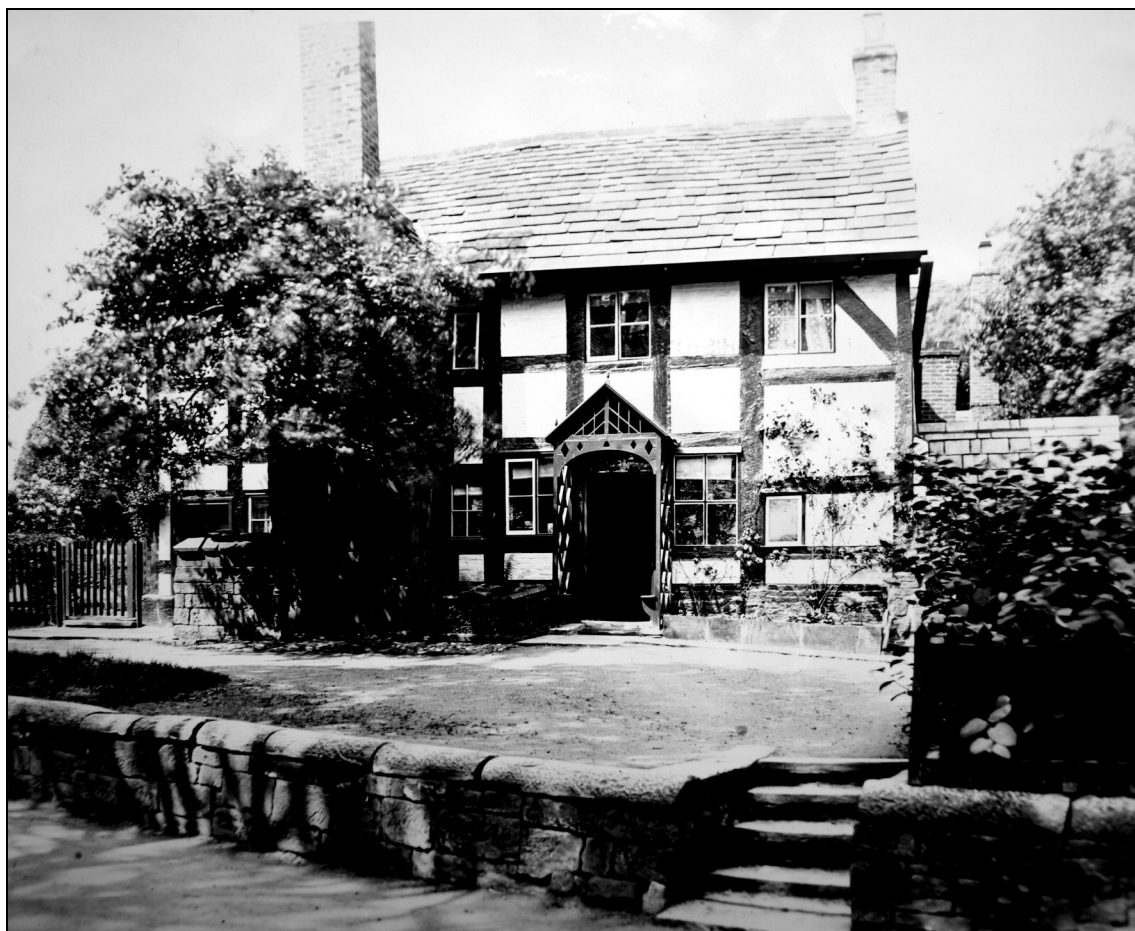
Figure 15: Photograph of the east wing (no.246), from the east; mid 20th century (Salford Local Studies Library)
