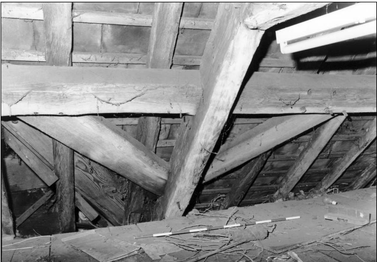
Photo 20: Wind braces on east side of middle truss
