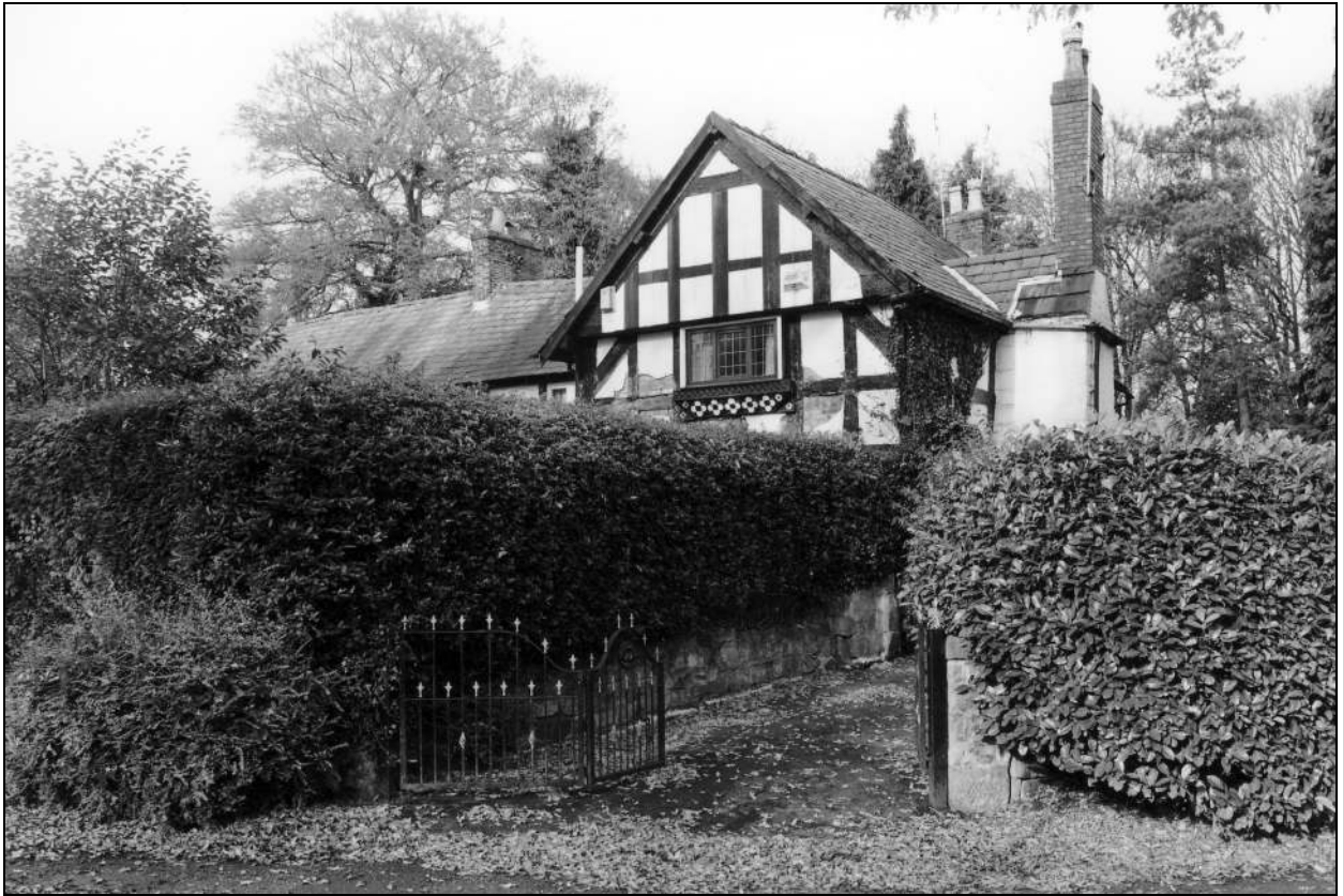
Photo 3: The east wing, from the south-east
