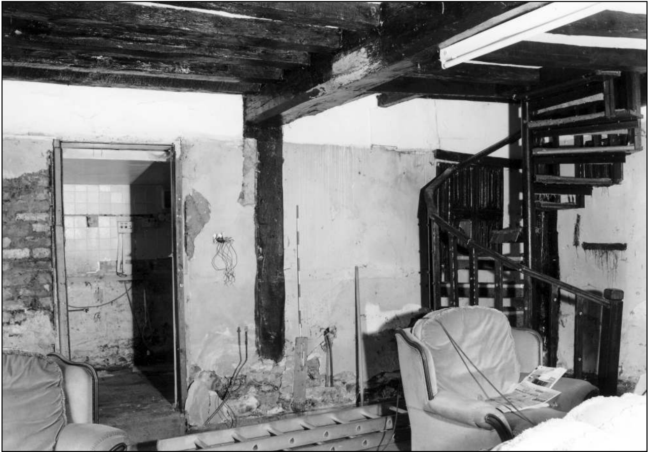
Photo 17: Ground floor room of no 247, from the south-east
