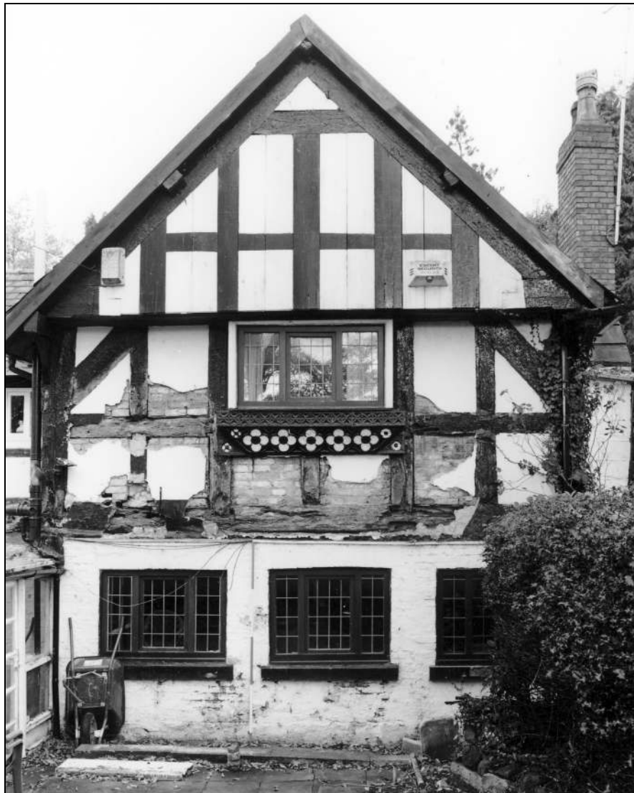
Photo 8: South elevation of the east wing
