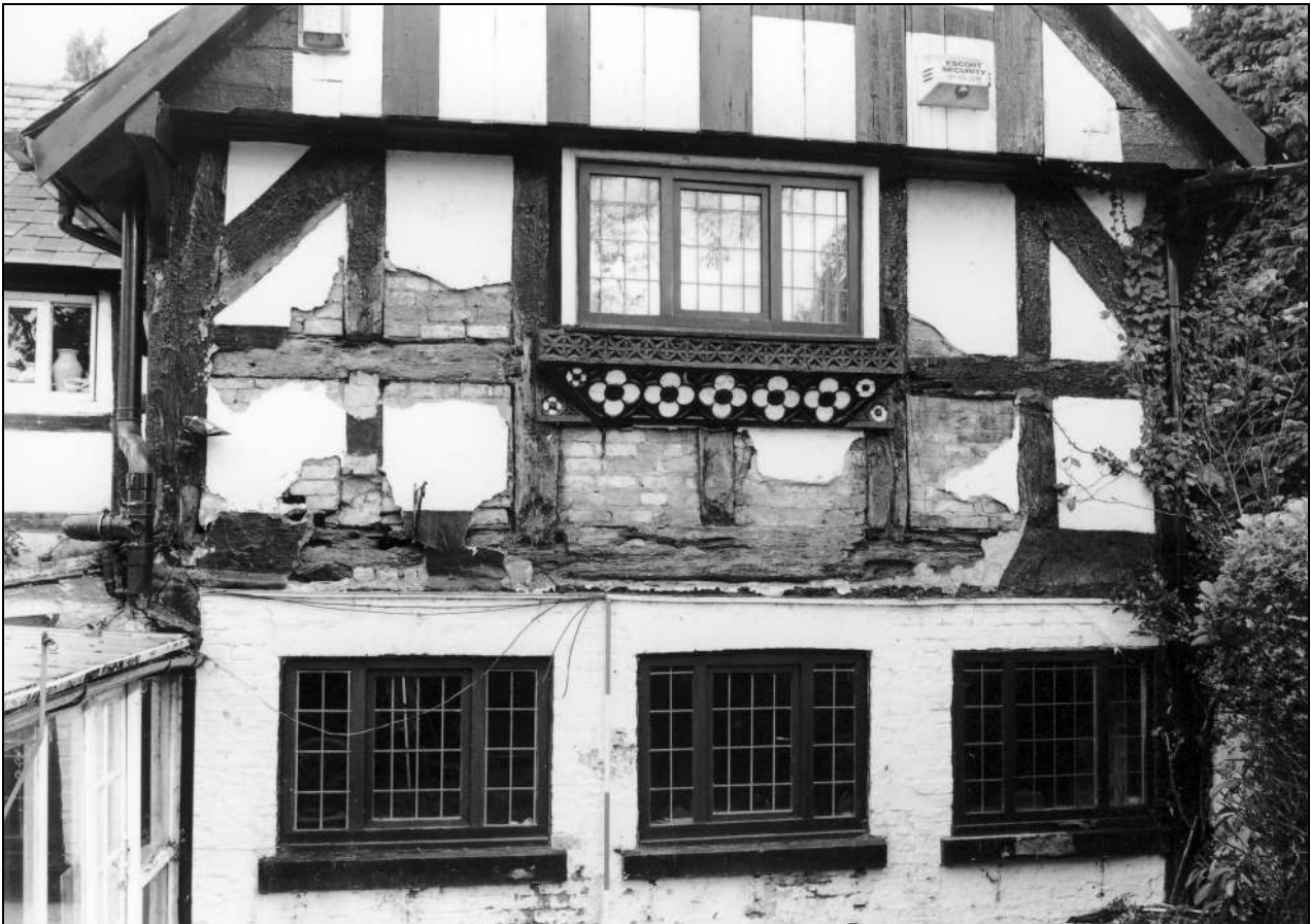
Photo 10: East wing: middle part of front elevation
