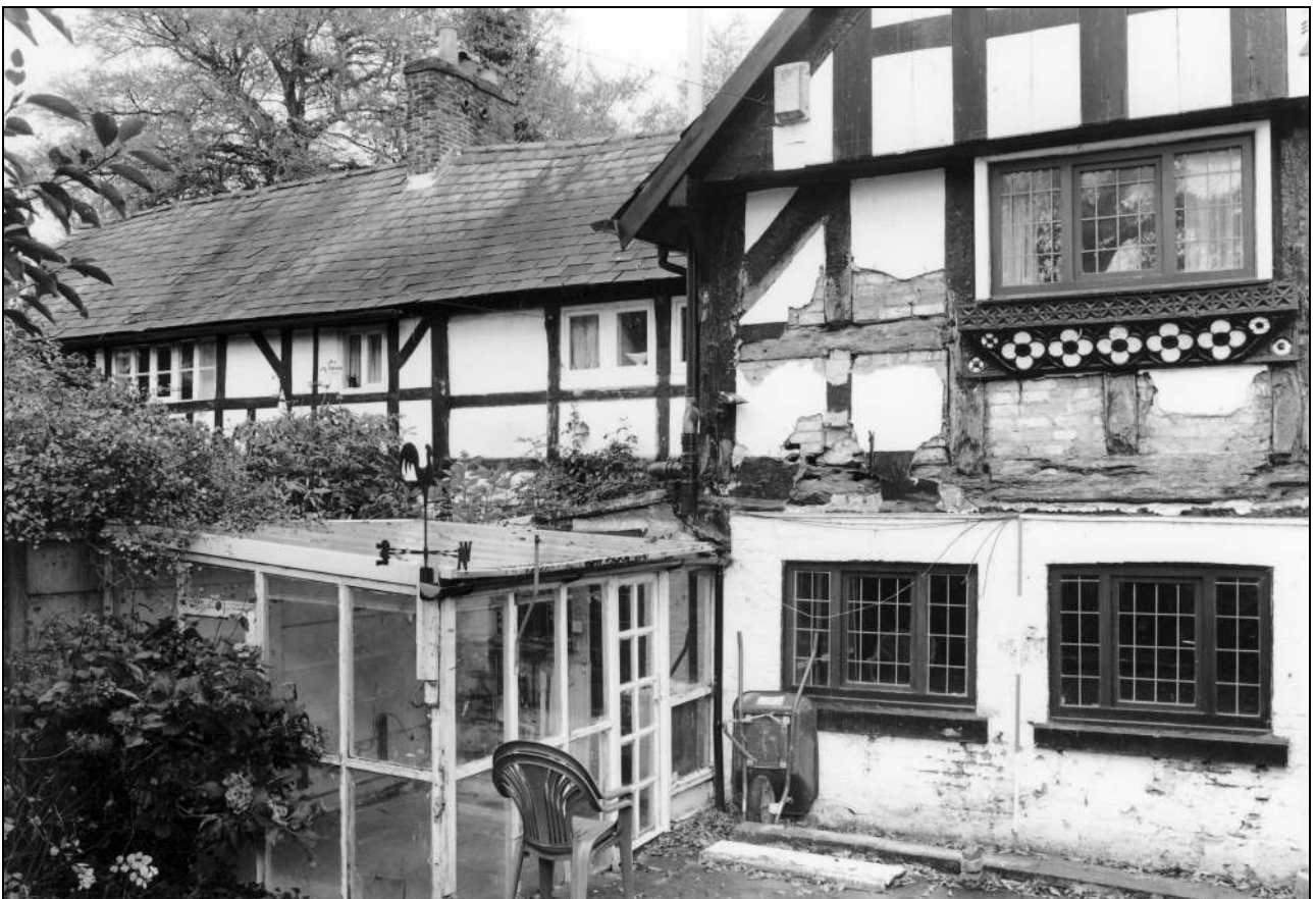
Photo 4: The east wing and main range, from the south
