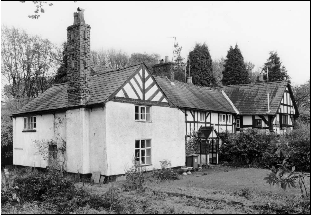
Photo 1: General view of the Hall, from the south-west
