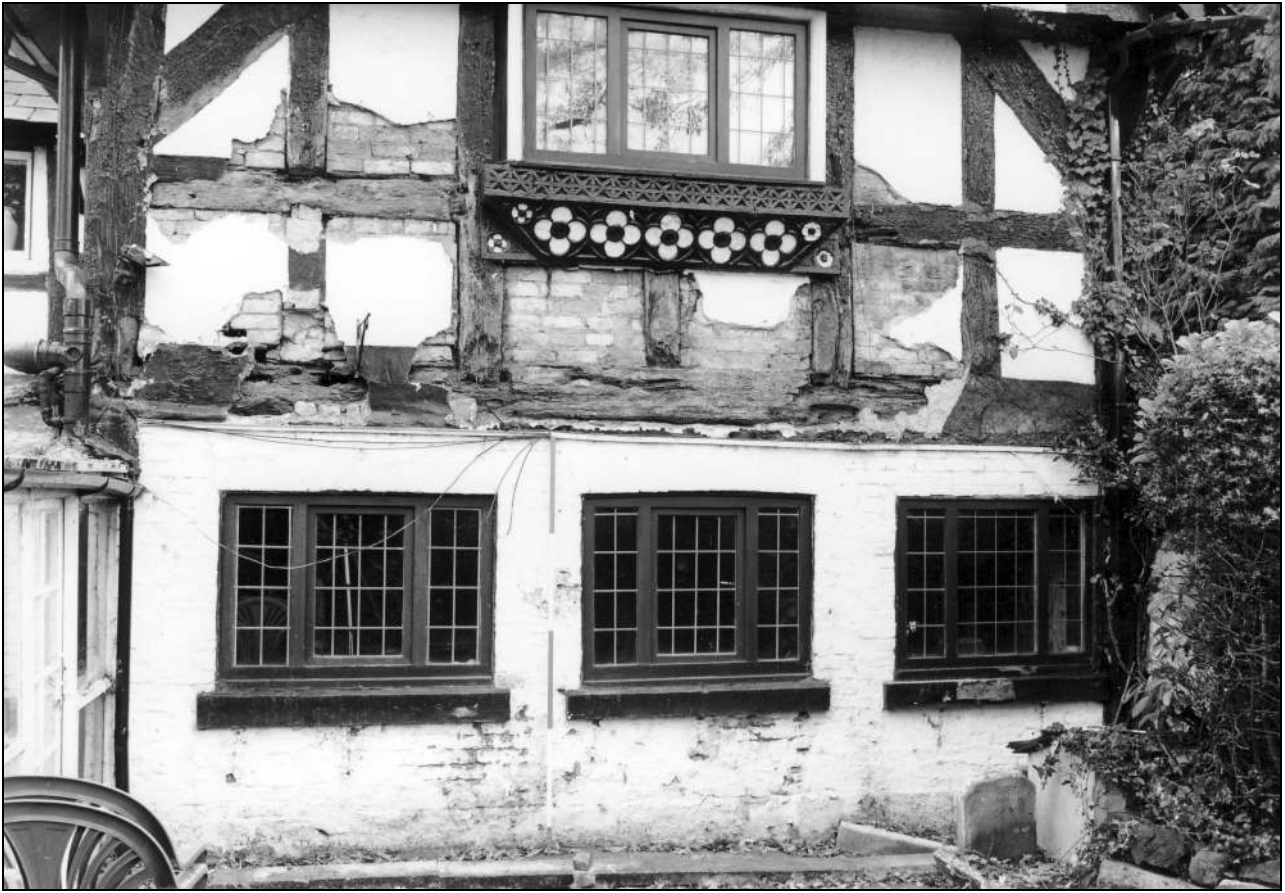
Photo 9: East wing: lower part of front elevation
