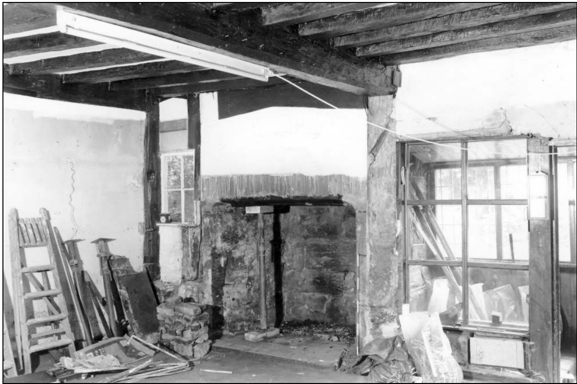
Photo 33: Ground floor room of no 247, from the south-west
