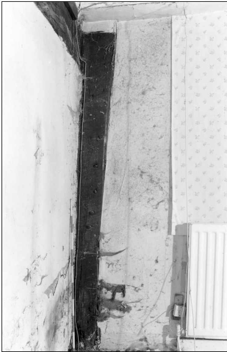
Photo 37: First floor: internal view of south-east wall post
