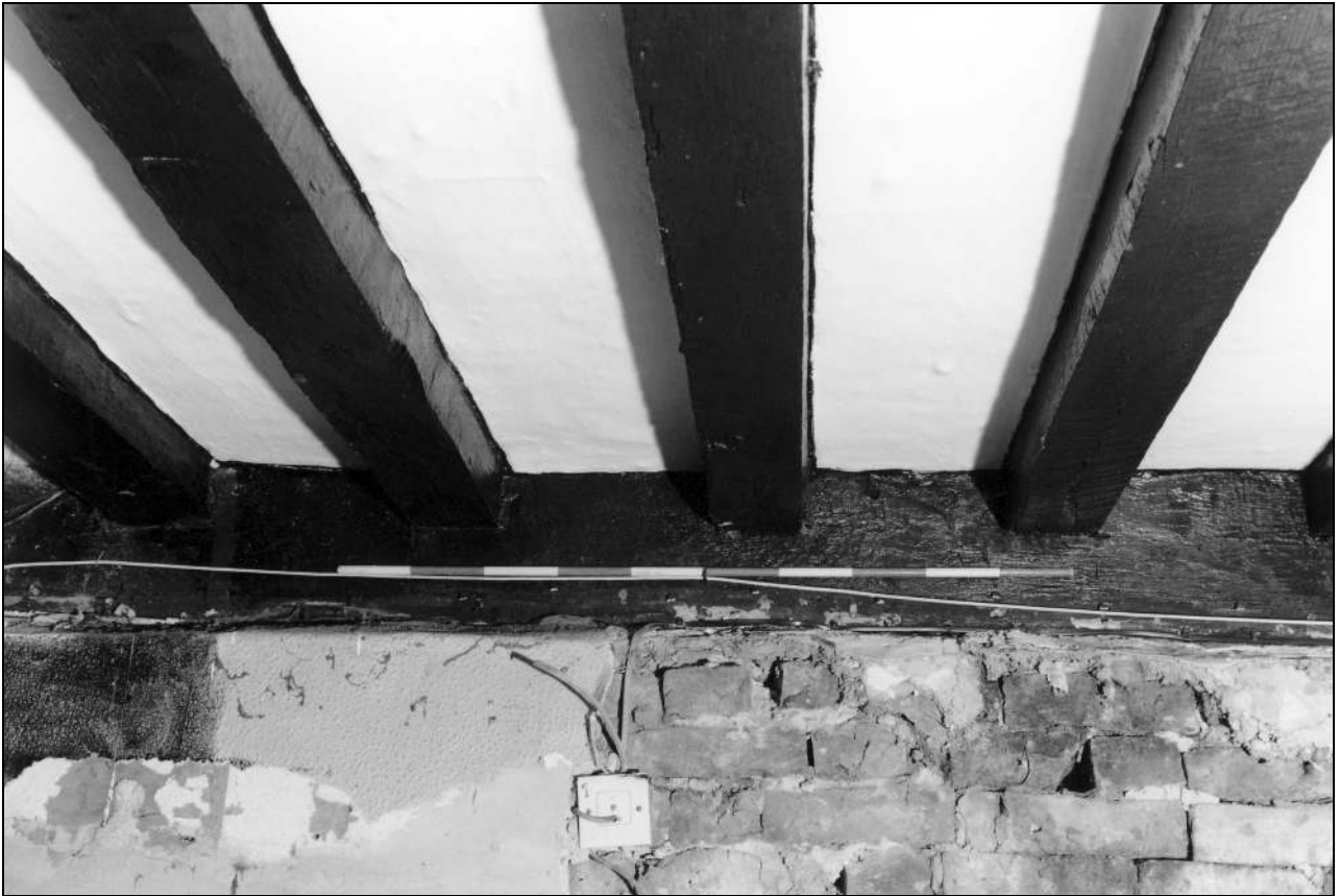
Photo 45: Detail of joists over ground floor room
