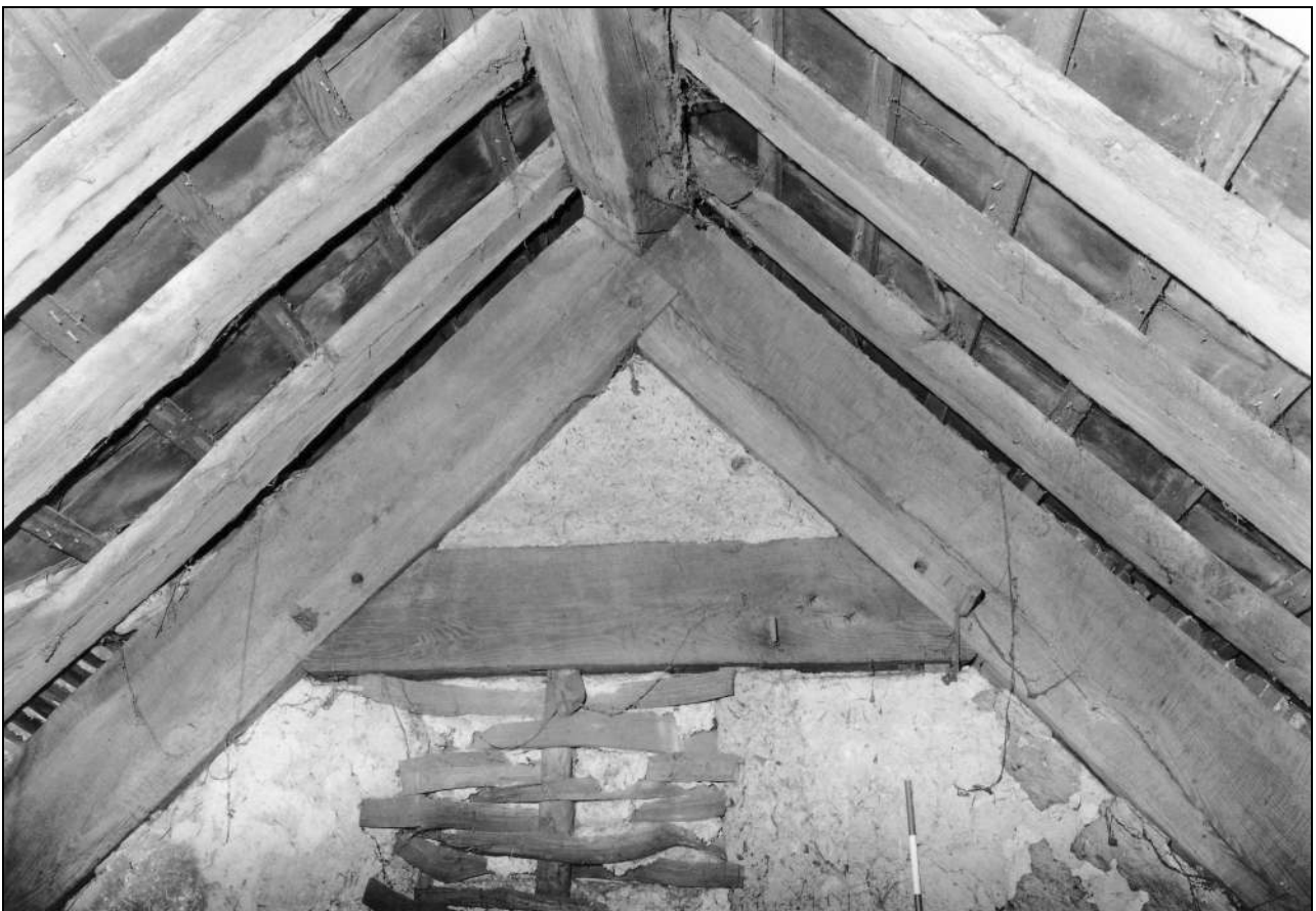
Photo 28: Collar and ridge of truss forming north side of no.247
