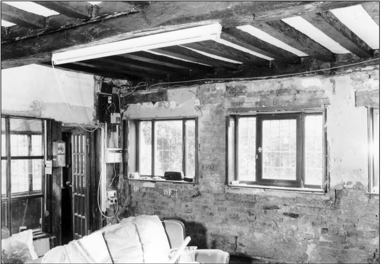
Photo 41: Ground floor room of no 247, from the north-west
