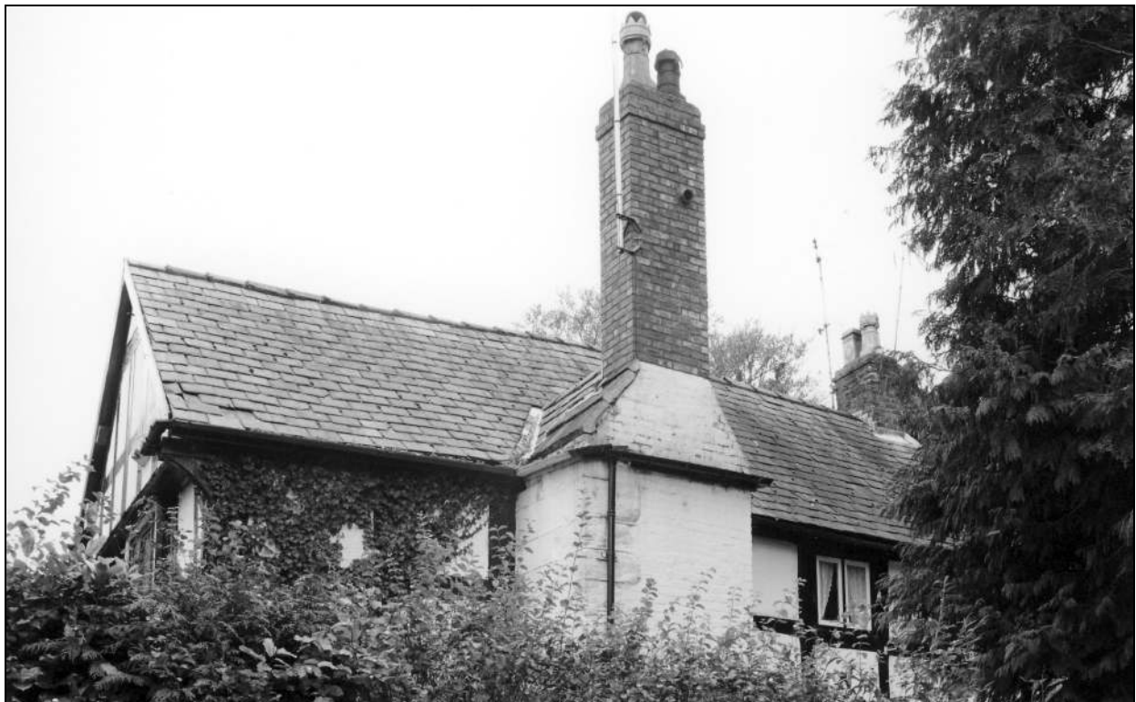
Photo 30: Chimney and roof of east wing, from the east
