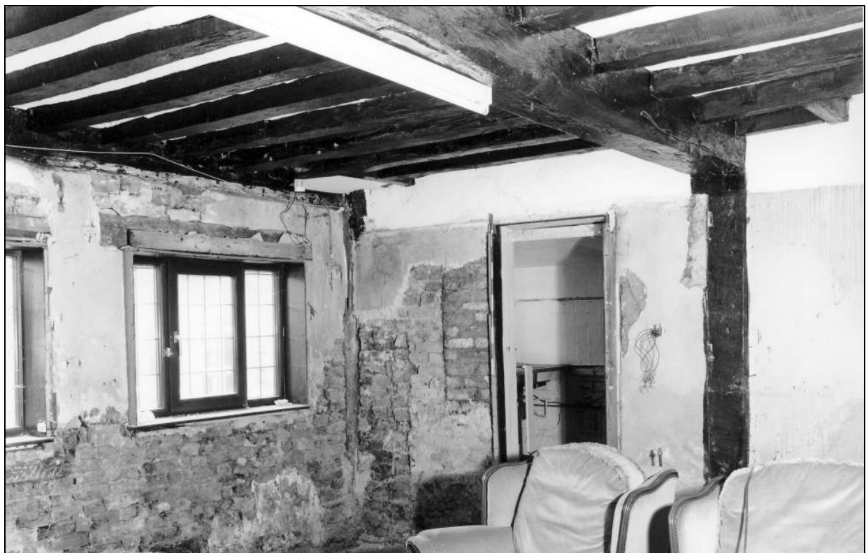
Photo 38: Ground floor room of no 247, from the north-east
