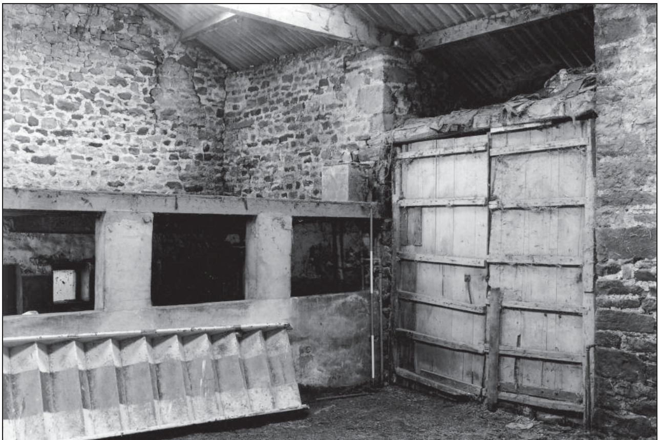
Photo 21: Interior of the barn, from the north-west, showing main entrance and modern shippon
