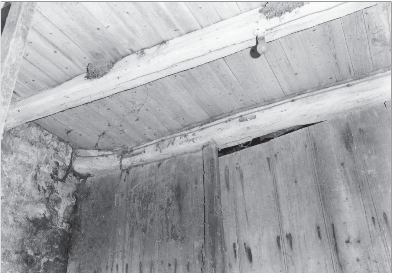
Photo 15: Re-used timber (elbowed principal rafter), over main doors
