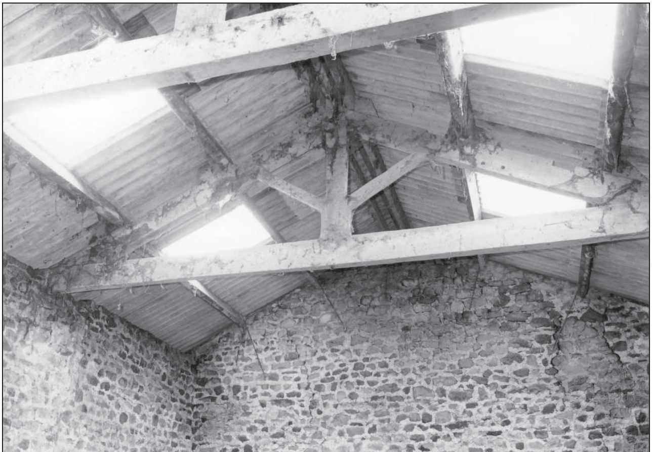
Photo 27: The east roof truss, from the west
