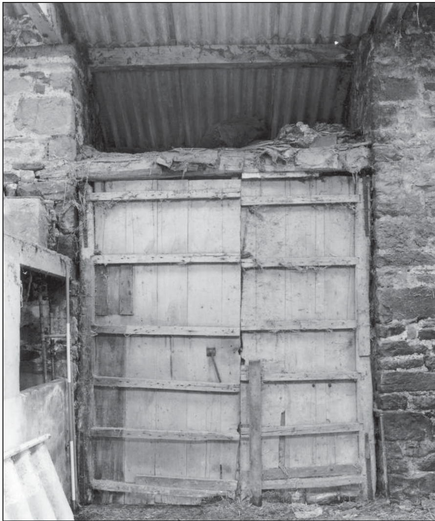
Photo 18: Interior view of main doors, from the north
