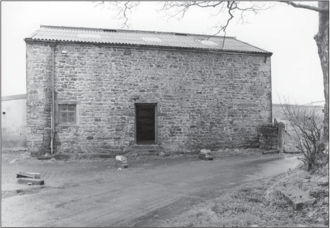
Photo 12: North elevation of the barn
