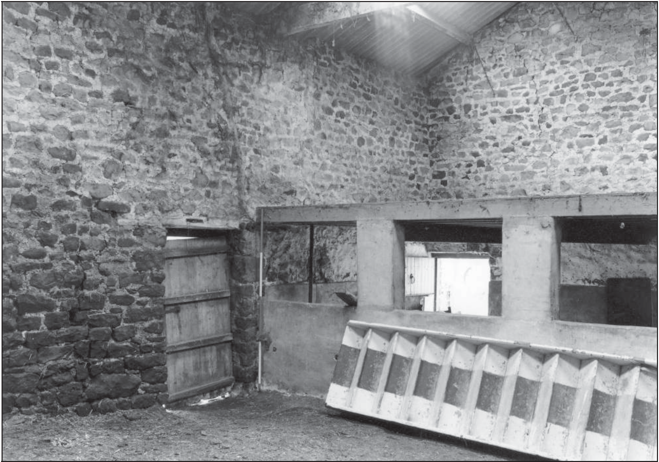
Photo 22: Interior of the barn, from the south-west
