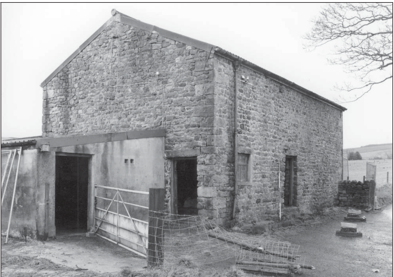
Photo 9: The barn, from the north-east
