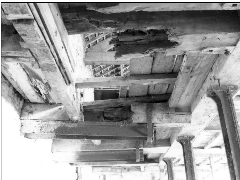
Photo 32: Underside of the hurst, from the north-west
