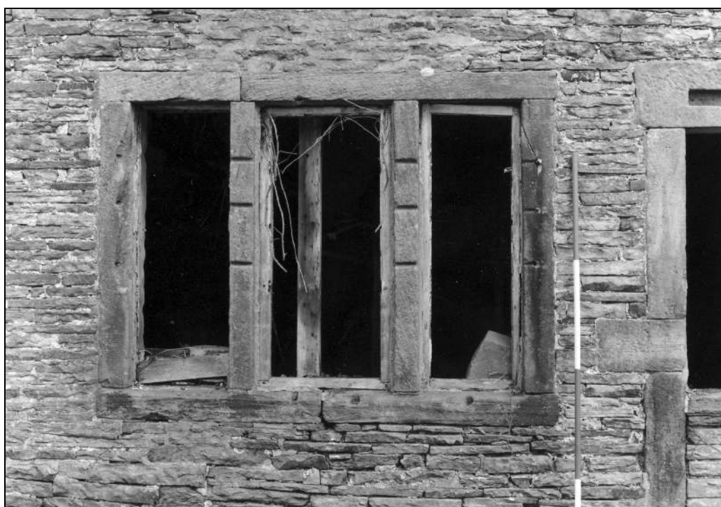
Photo 5: Detail of three-light window in front elevation
