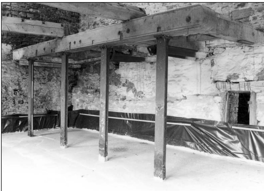
Photo 24: The hurst, after the removal of the shippon fixtures
