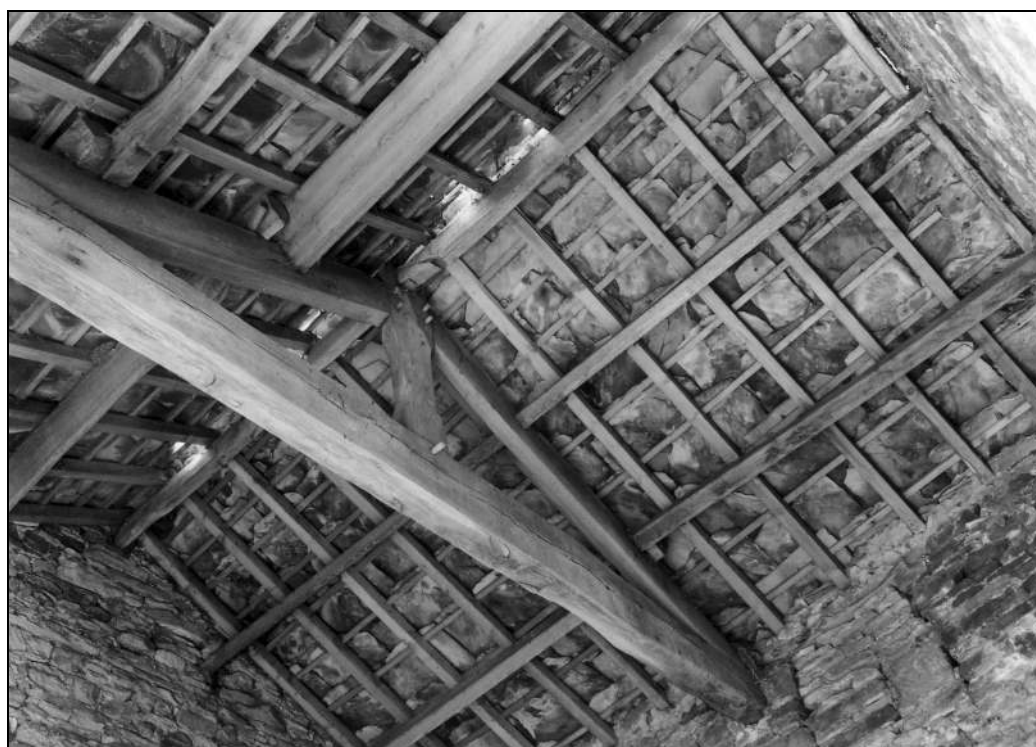
Photo 70: Added store: roof truss
