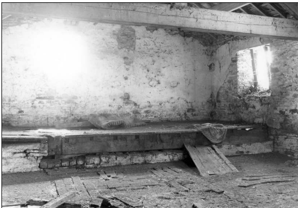
Photo 38: First floor of mill: the south-east bay
