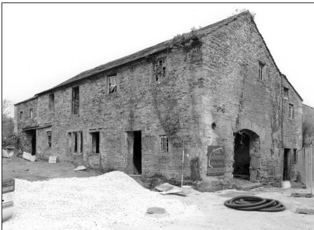
Photo 1: General view of the mill, from the south
