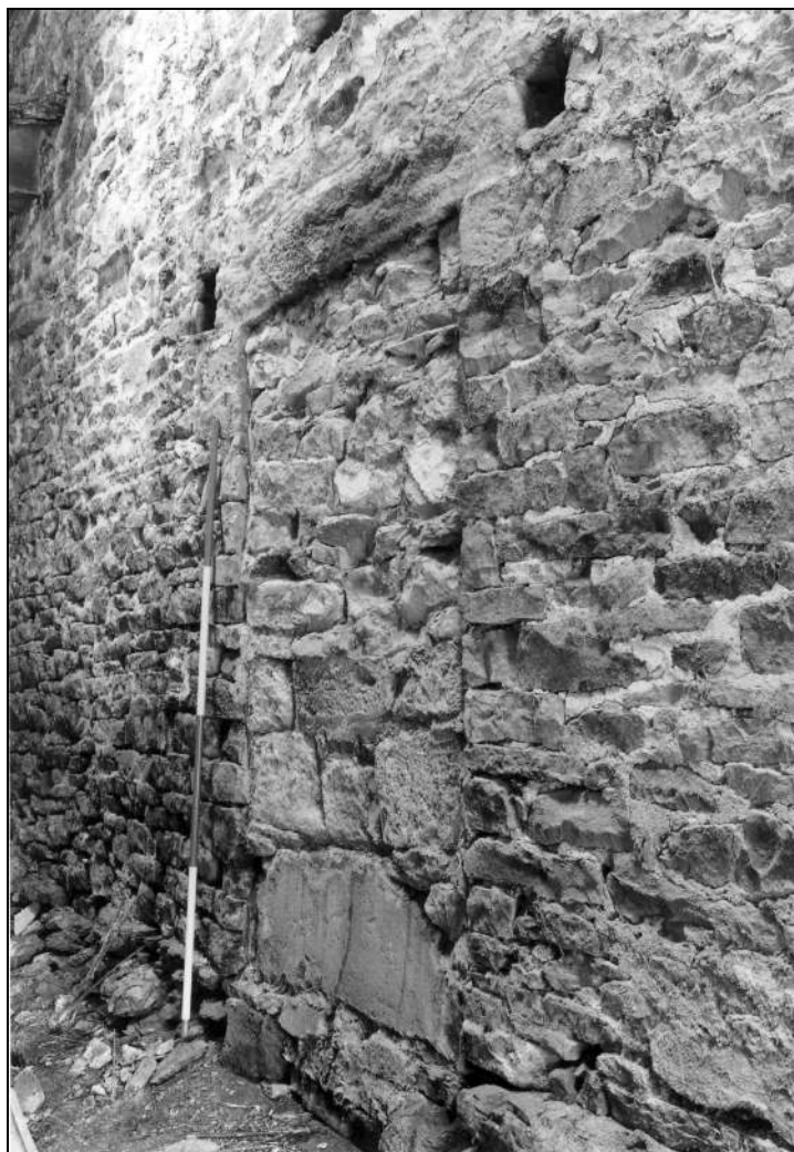
Photo 46: Blocked door in north-east side of wheel-house, from the south
