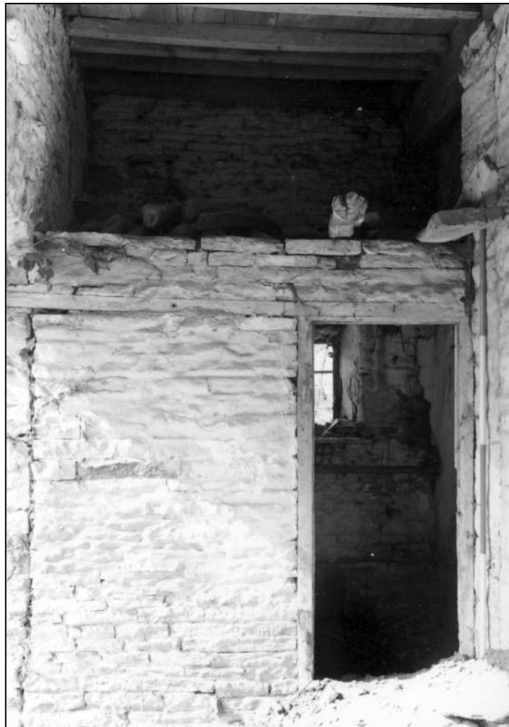
Photo 16: Office in mill, from the north-east
