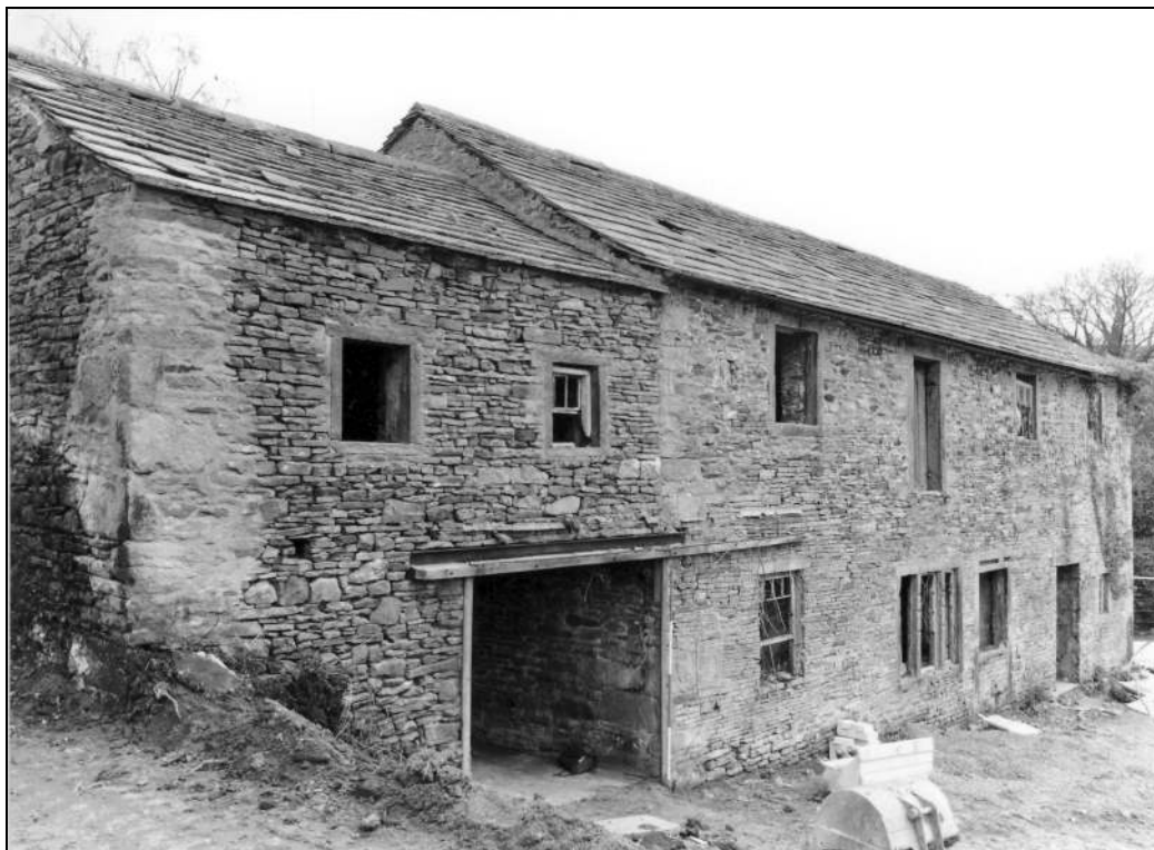
Photo 64: Added store at north-west end of range
