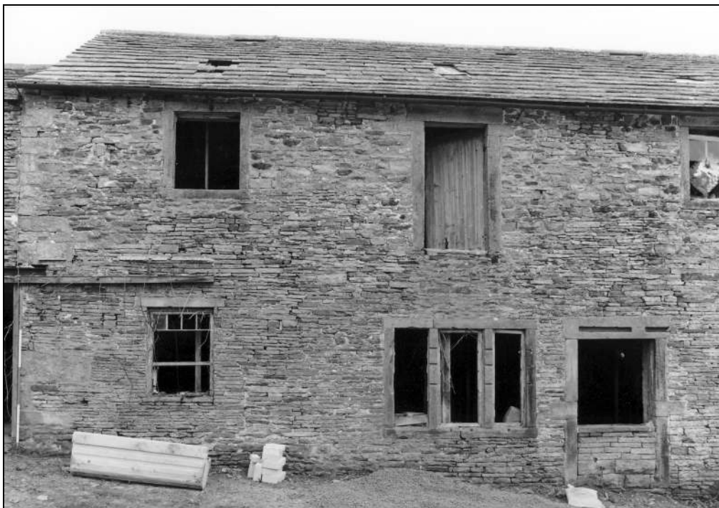
Photo 6: Front elevation (north-west end)
