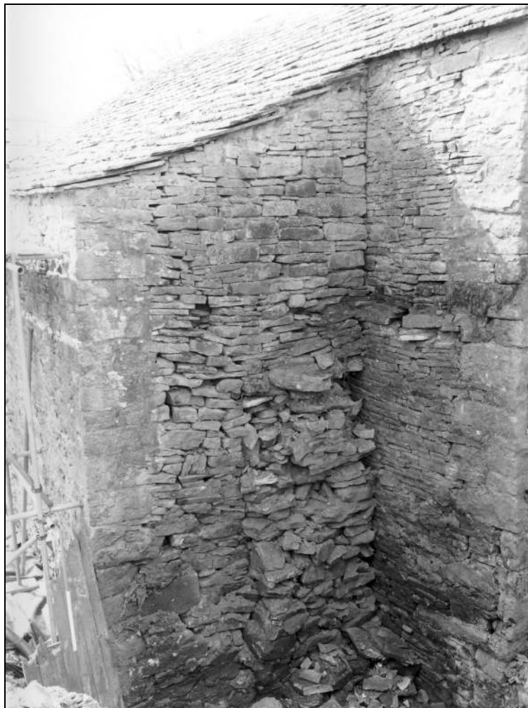
Photo 55: North-west end of wheel-house after excavation, showing buttress or laundry support
