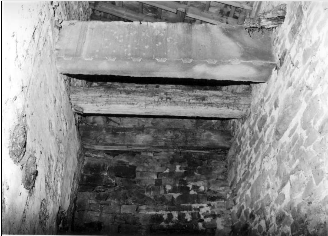
Photo 53: Stone block and timbers above north-west end of wheel-pit
