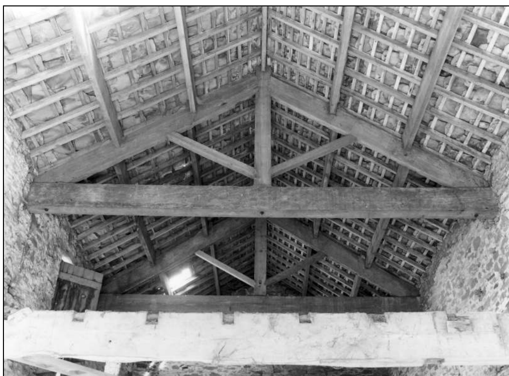
Photo 41: Roof trusses in mill, from the south-east
