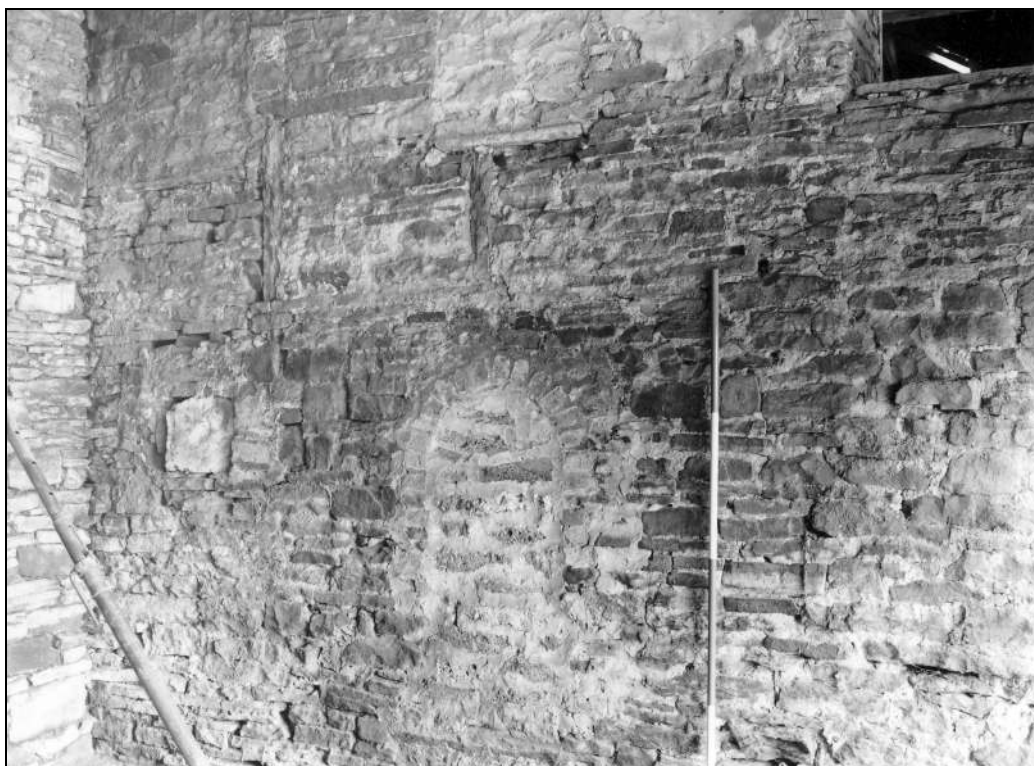
Photo 10: North-west gable of main building, within later store (ground floor)
