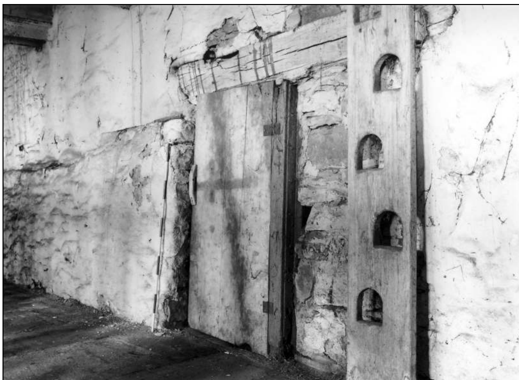
Photo 33: Doorway at former waterwheel bearing, and Jacob's ladder
