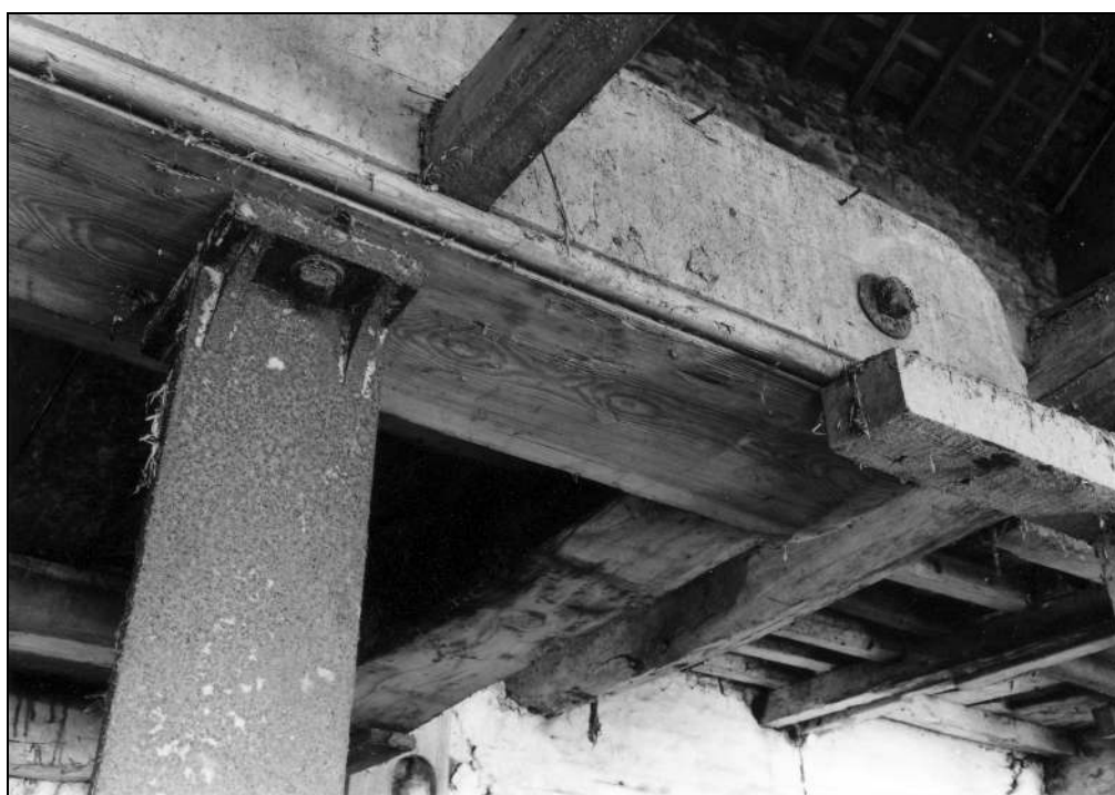
Photo 28: The beam forming the south-west side of the hurst
