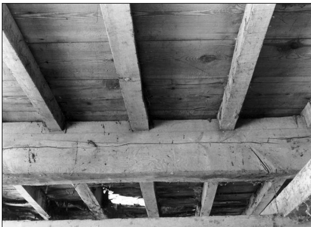
Photo 37: Underside of the first floor in mill, from the south-east
