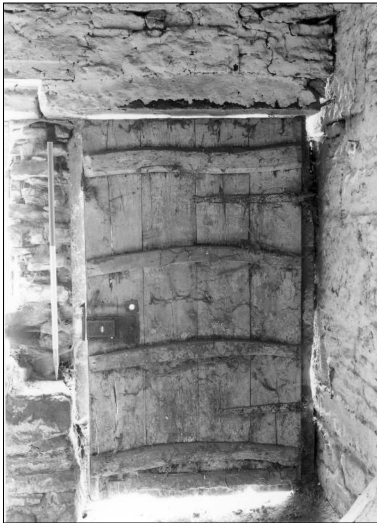
Photo 62: Door to added store (inner face)
