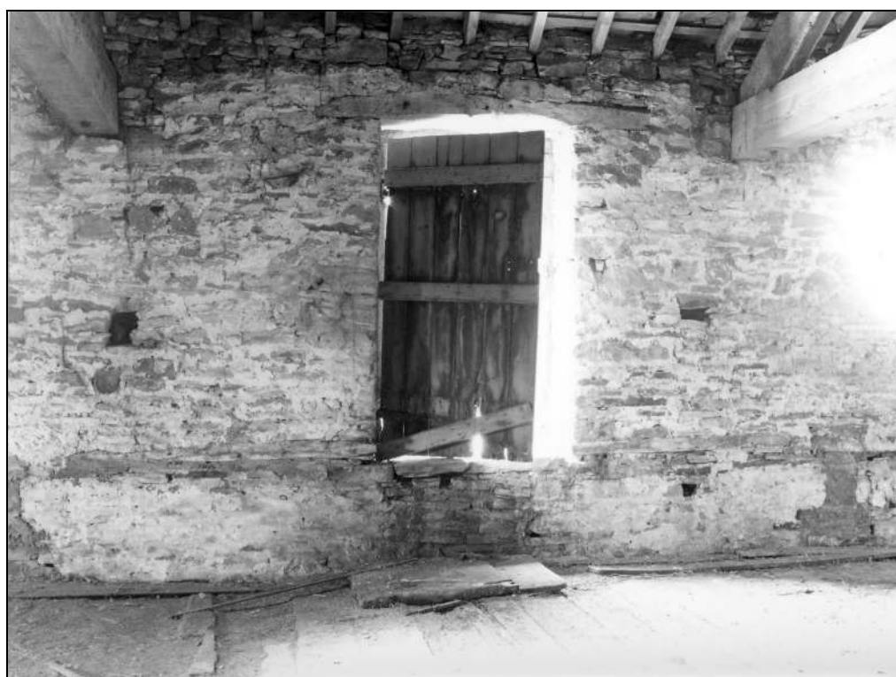
Photo 39: First floor of mill: taking-in door in south-west side, showing former floor level
