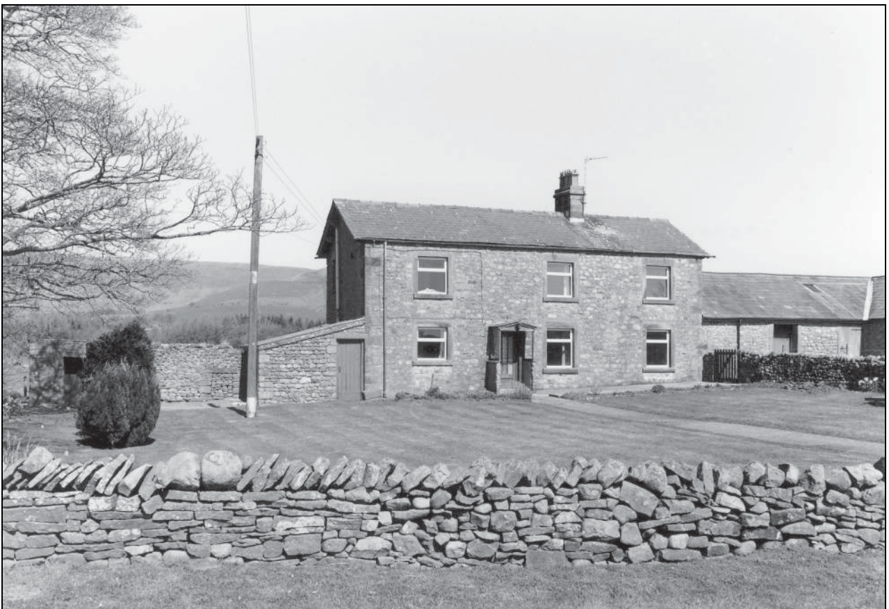
Photo 3: General view of the farmhouse etc, from the south-west
