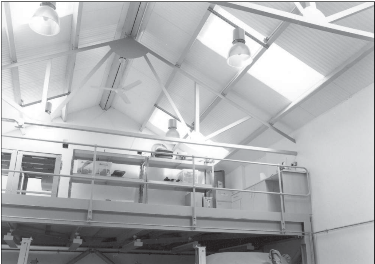
Photo 36: Interior of barn (now workshop), from the south
