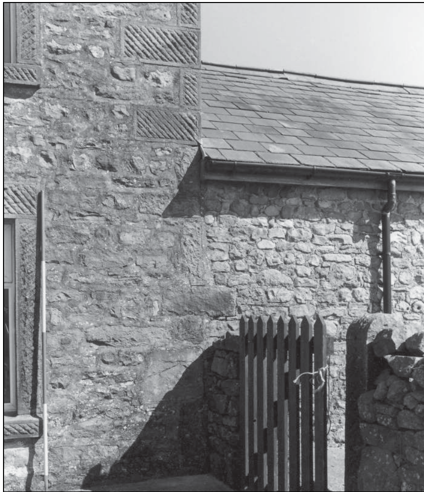
Photo 7: The farmhouse: south-east corner, where earlier quoins survive
