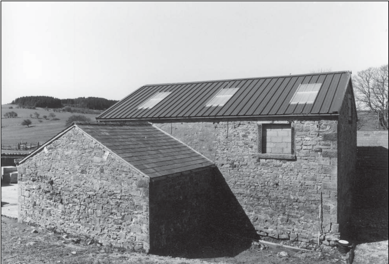
Photo 34: Barn and cart-shed, from the east
