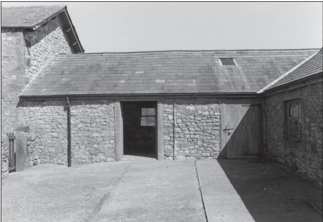
Photo 20: Loose boxes to east of farmhouse, from the south
