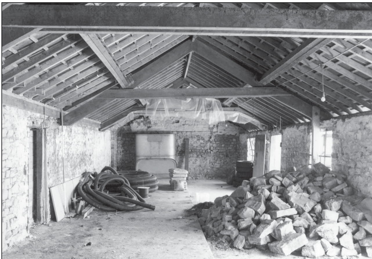
Photo 30: Interior of shippon, from the north
