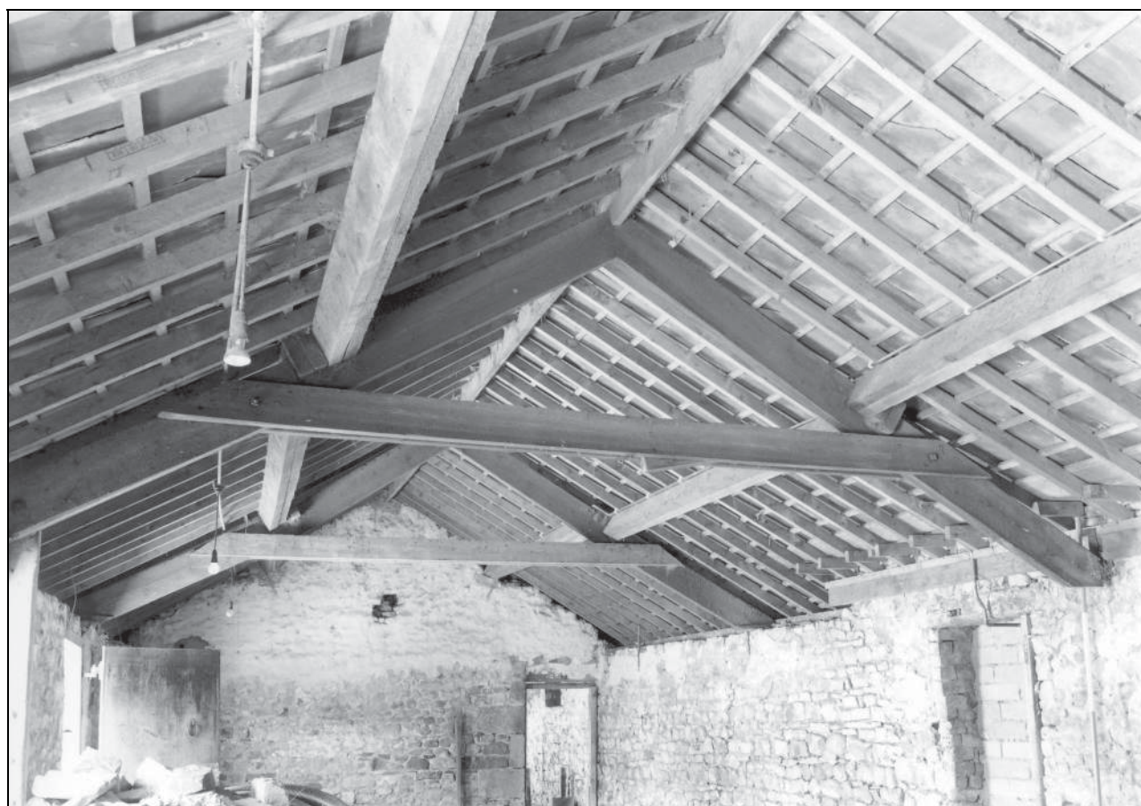
Photo 31: Roof trusses in shippon, from the south
