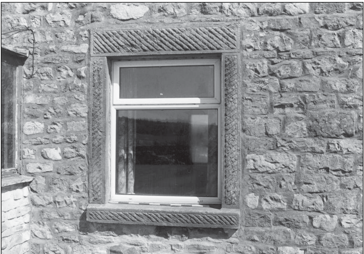
Photo 6: The farmhouse: detail of ground floor window with distinctive dressings
