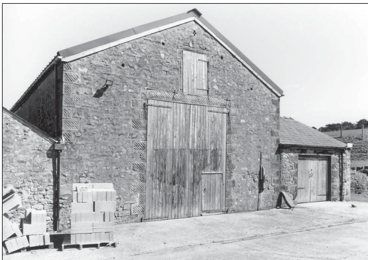
Photo 33: Barn and cart-shed, from the south-west
