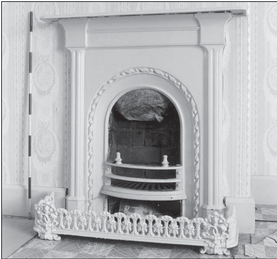
Photo 13: The farmhouse: 19th century bedroom fire-grate
