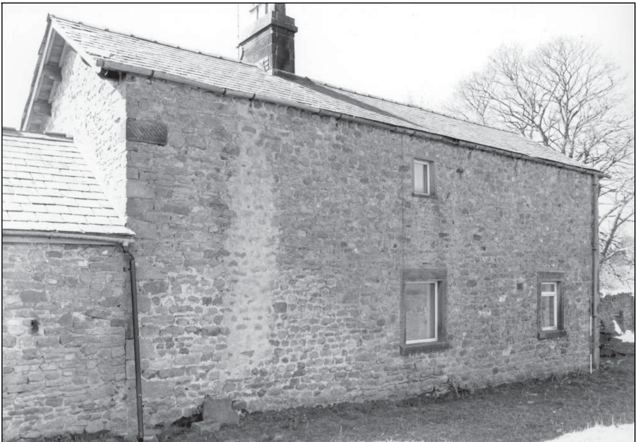
Photo 8: The farmhouse: rear elevation
