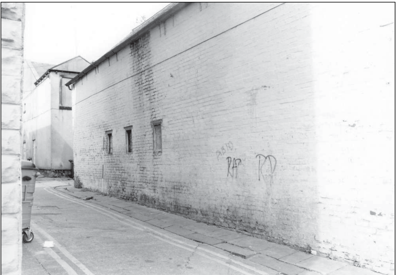
Photo 8: The south-east elevation
