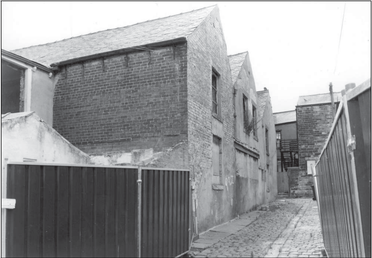
Photo 11: The rear of the building, from the north-west
