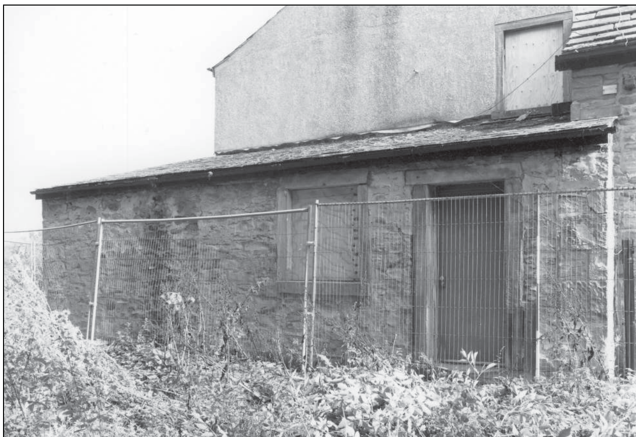
Photo 43: The 19th century house: lean-to at north-west corner
