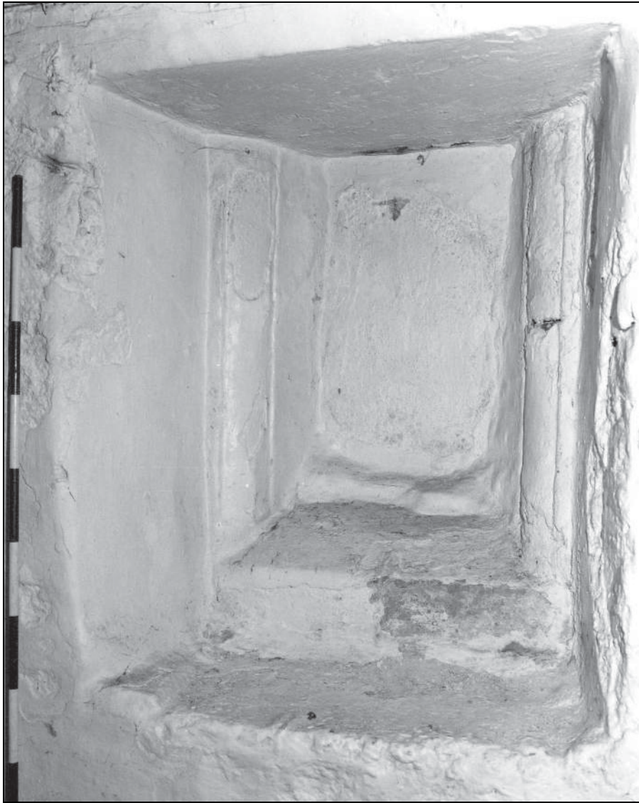
Photo 27: The 17th century house: blocked cellar window with ovolo moulding
