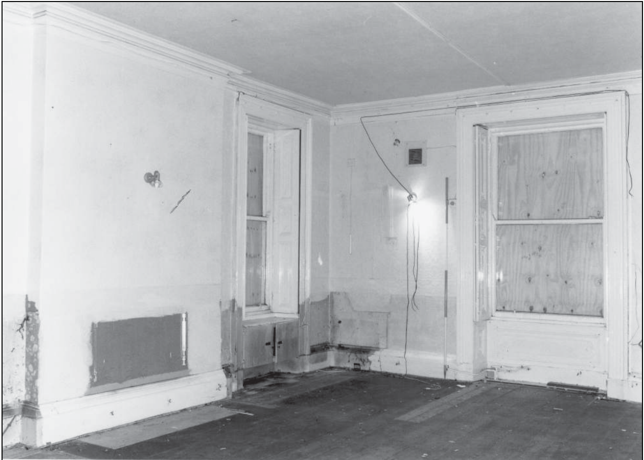
Photo 57: The 19th century house: north-east ground floor room, from the south-west
