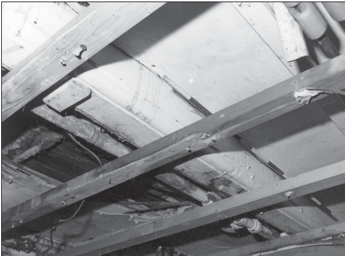
Photo 71: The 19th century house: ovolo moulded beam in main cellar
