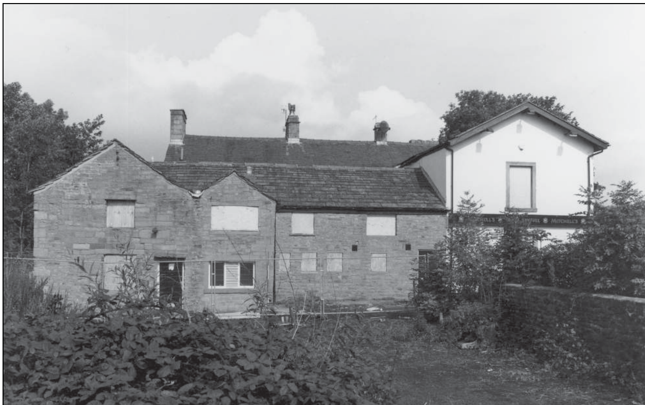
Photo 1: General view of the building, from the south
