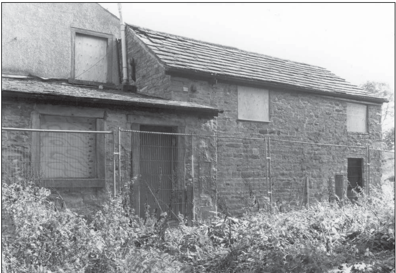
Photo 7: The 17th century house: south-west wing, from the north-west
