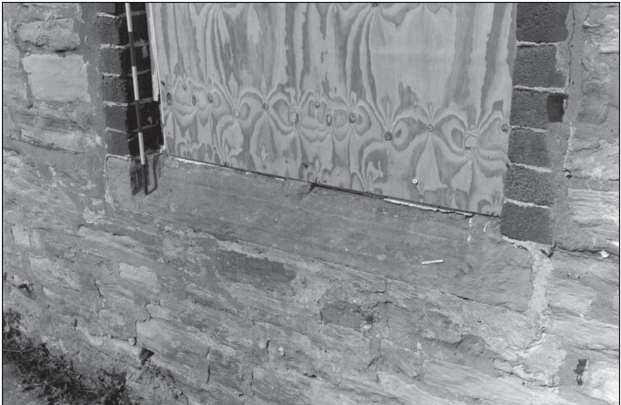
Photo 5: The 17th century house: ground floor window sill, south-west wing
