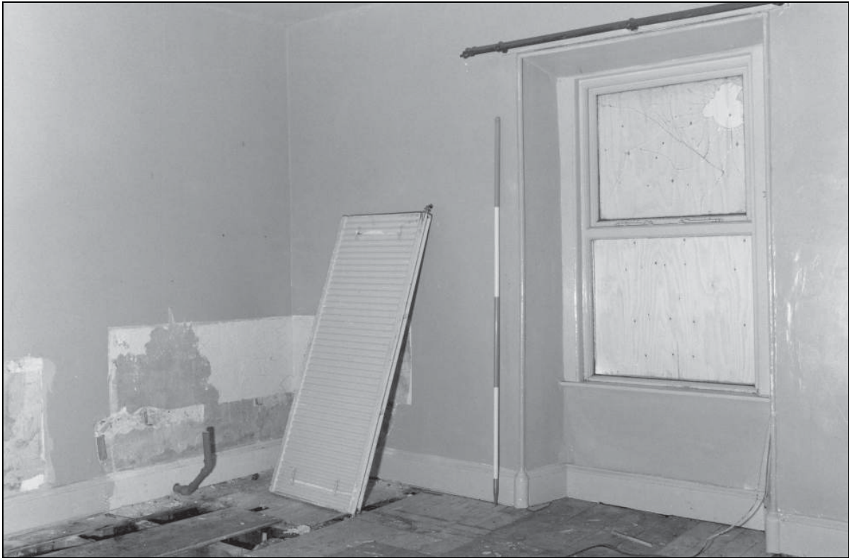
Photo 76: The 19th century house: north-east first floor room, from the south-west
