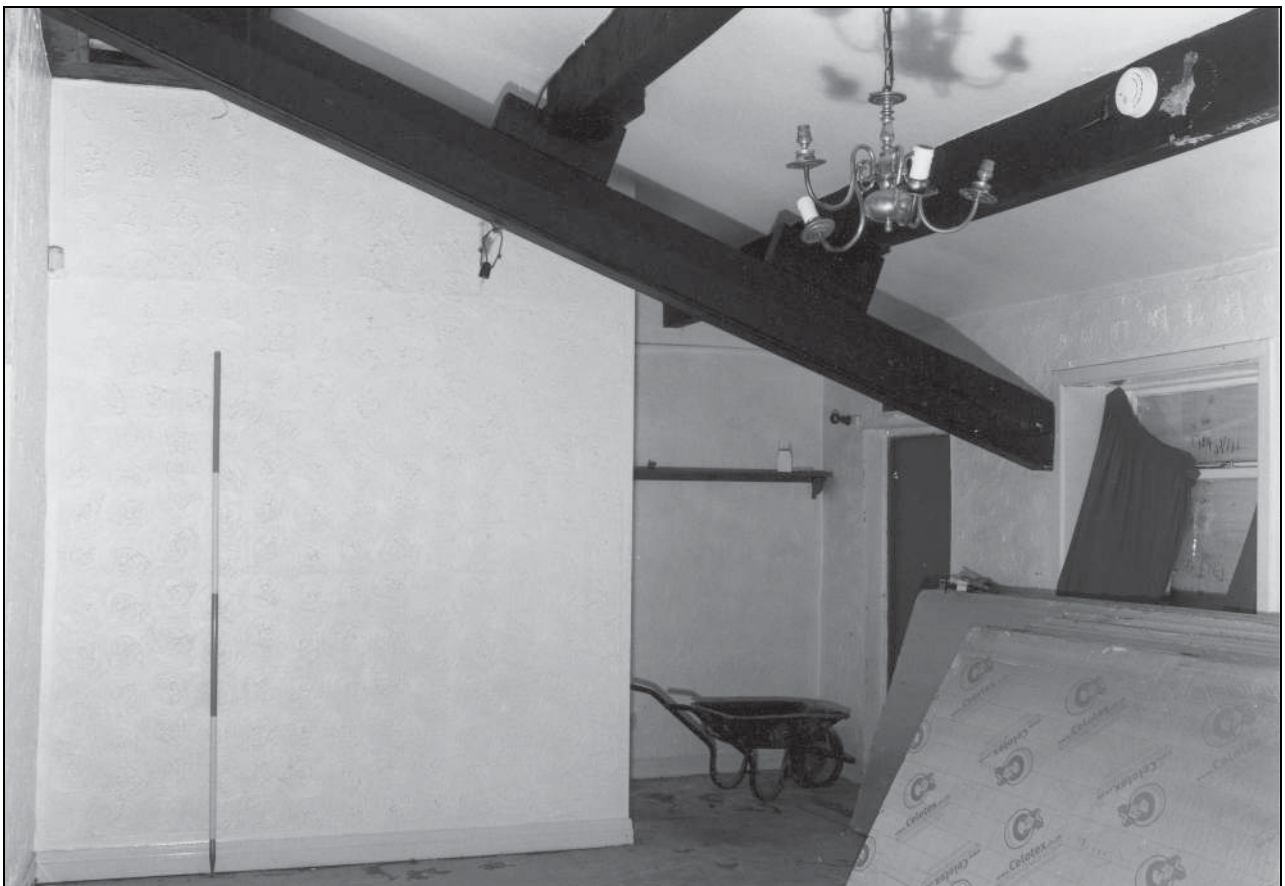
Photo 69: The 19th century house: interior of north-west lean-to
