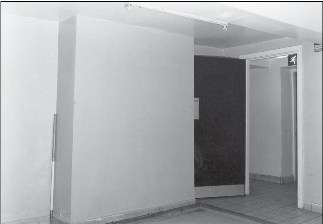
Photo 12: The 17th century house: chimney breast at east end of former housebody
