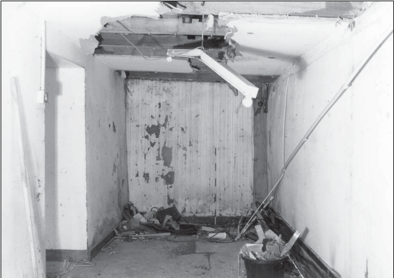
Photo 10: The 17th century house: possible former through passage
