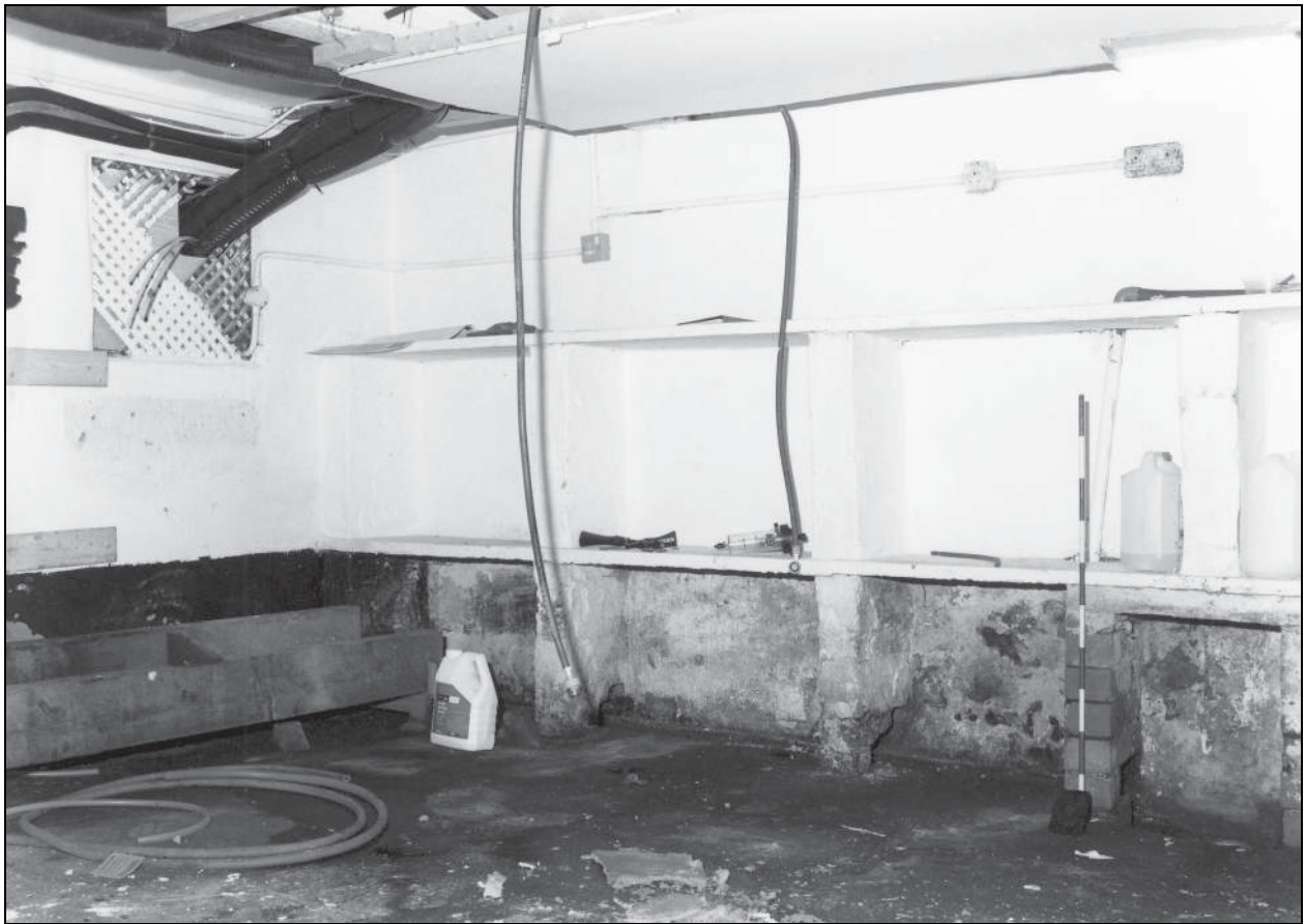
Photo 70: The 19th century house: the main cellar, from the north-east
