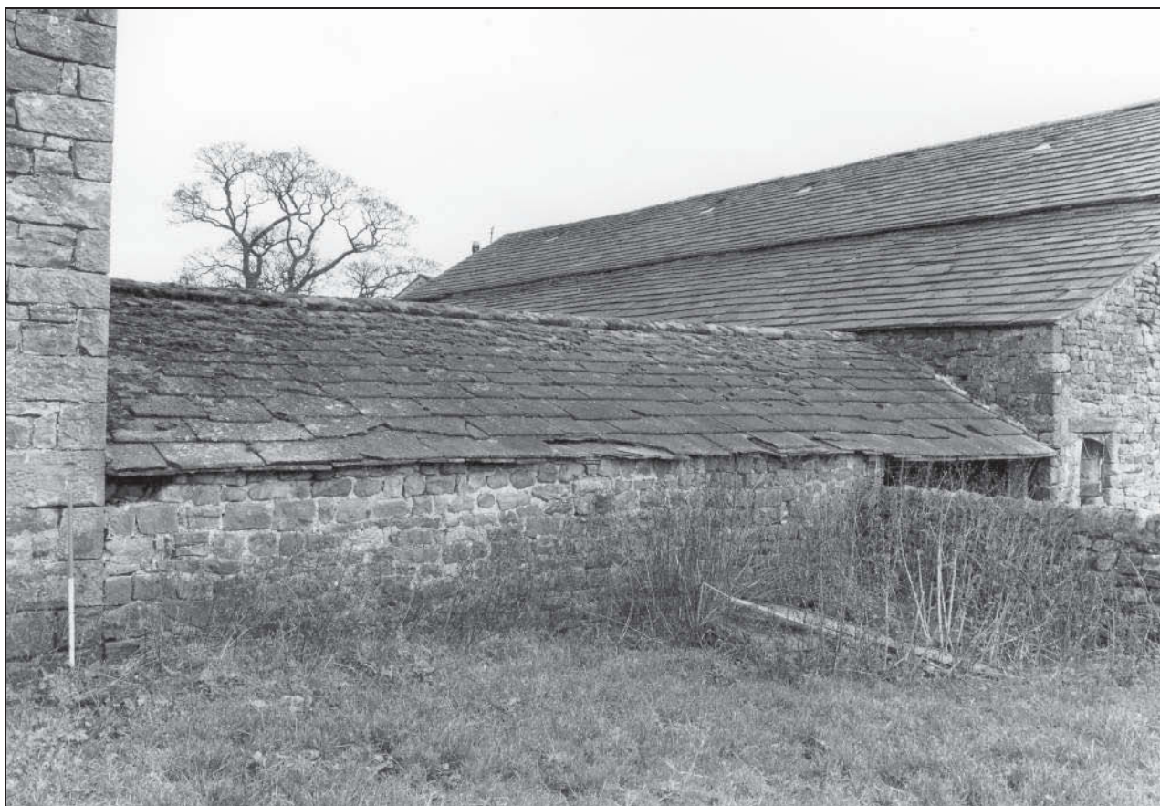
Photo 26: The cart shed: rear elevation, from the south-west
