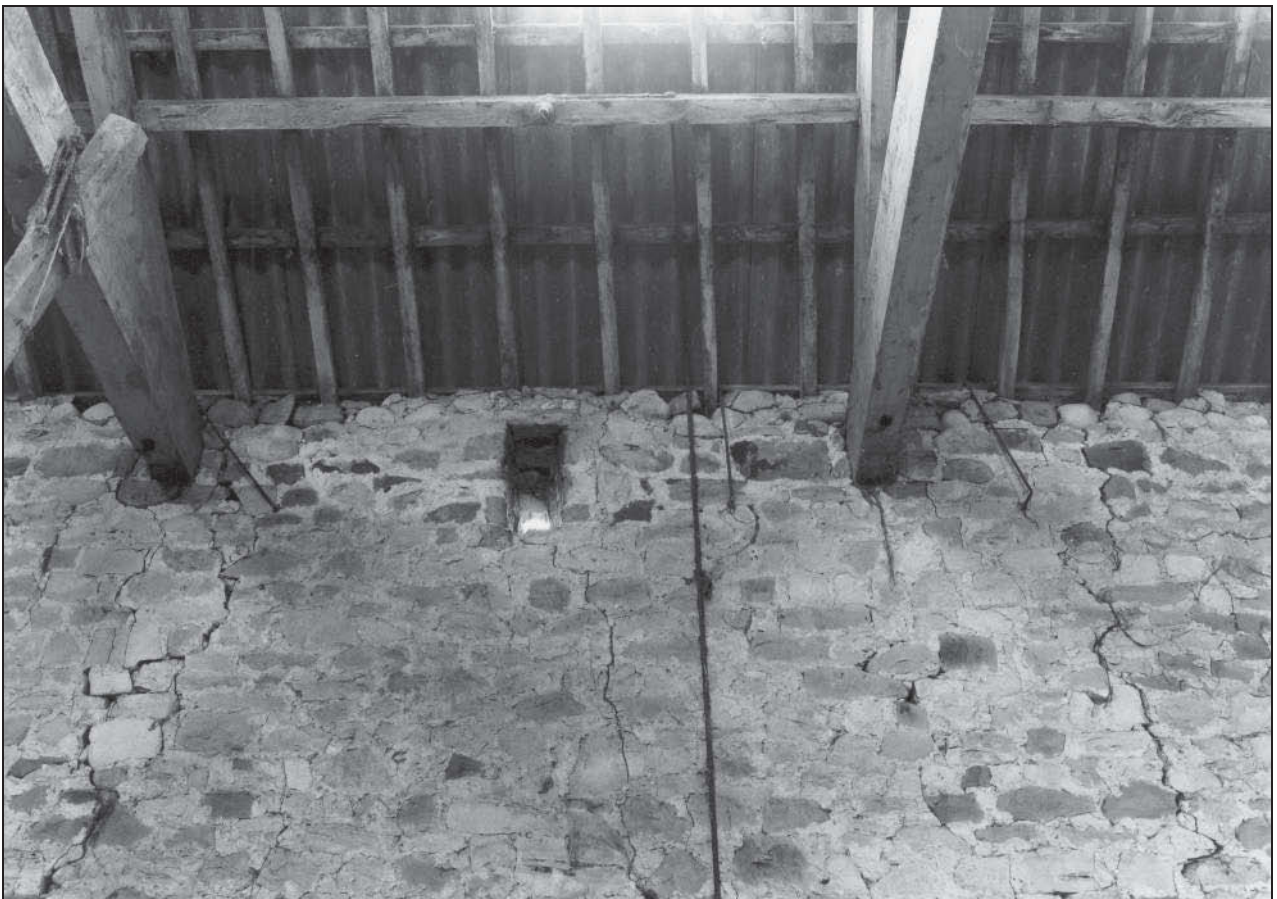
Photo 21: Bank barn: high level breather, in north wall
