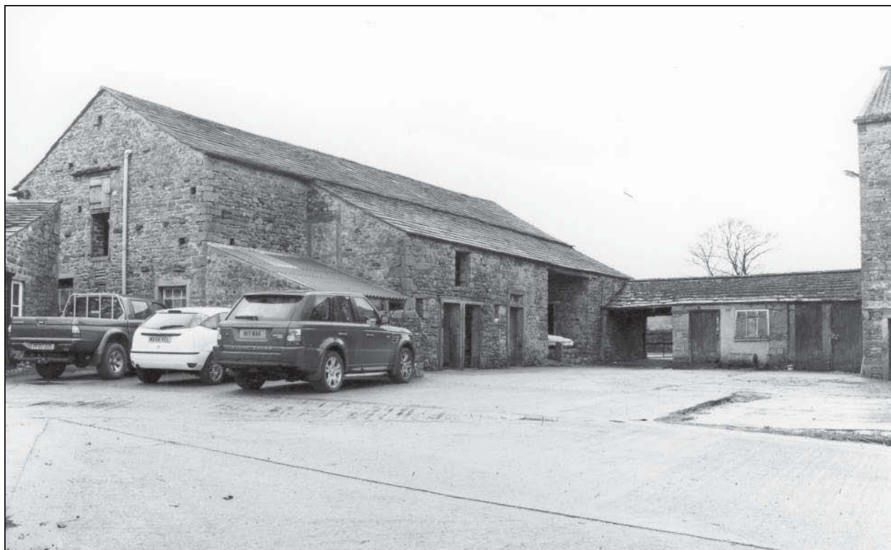
Photo 24: Cart shed (to right) and earlier barn (to left), from the north-west
