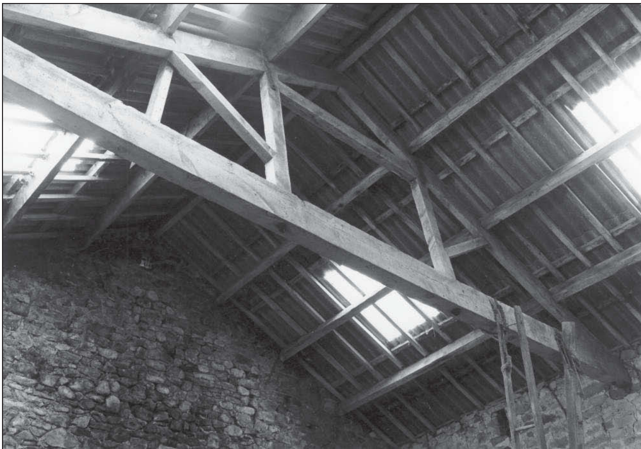
Photo 23: Bank barn: west roof truss, from the south-east
