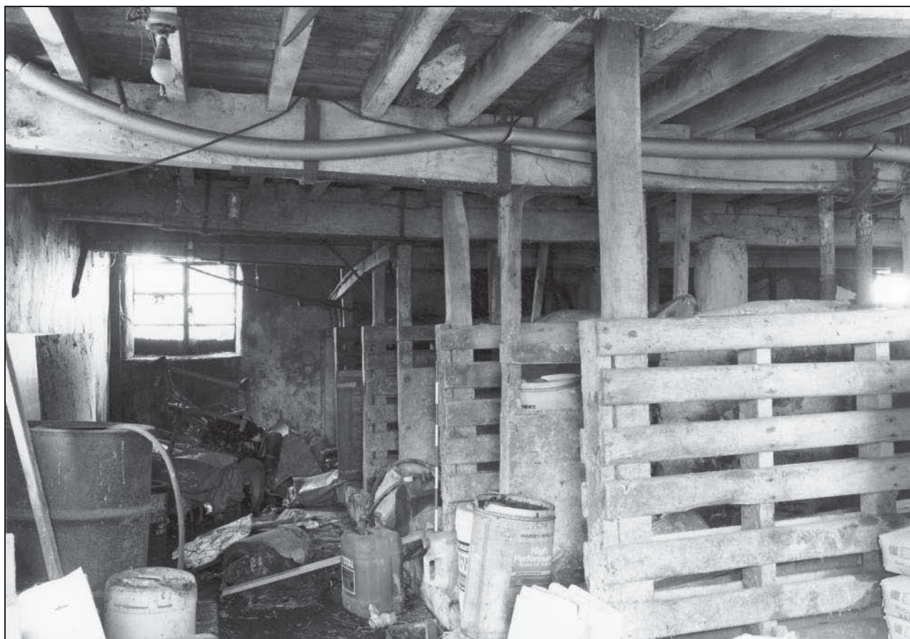
Photo 10: Bank barn: the shippon in the east end, from the north
