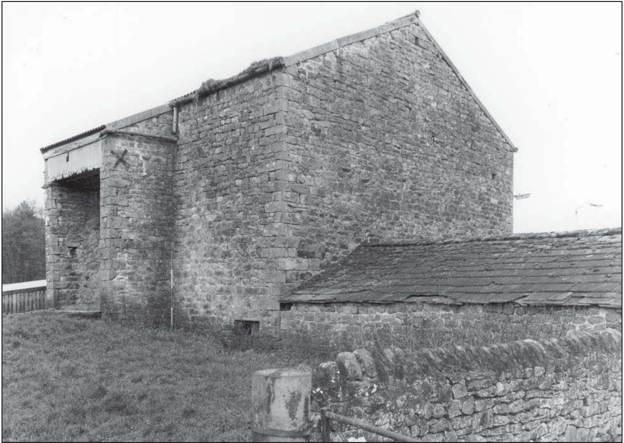
Photo 15: The bank barn, from the south-east
