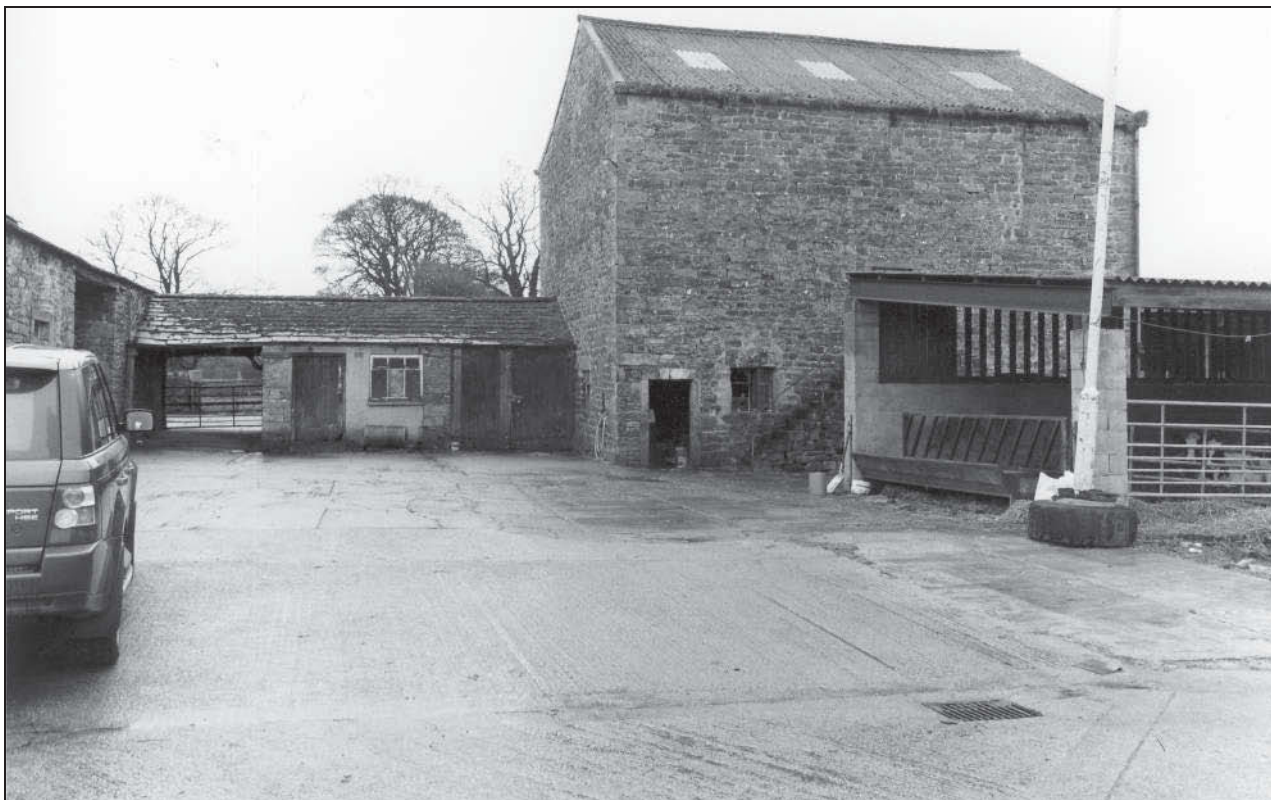
Photo 4: Cart shed (to left) and bank barn (to right), from the north
