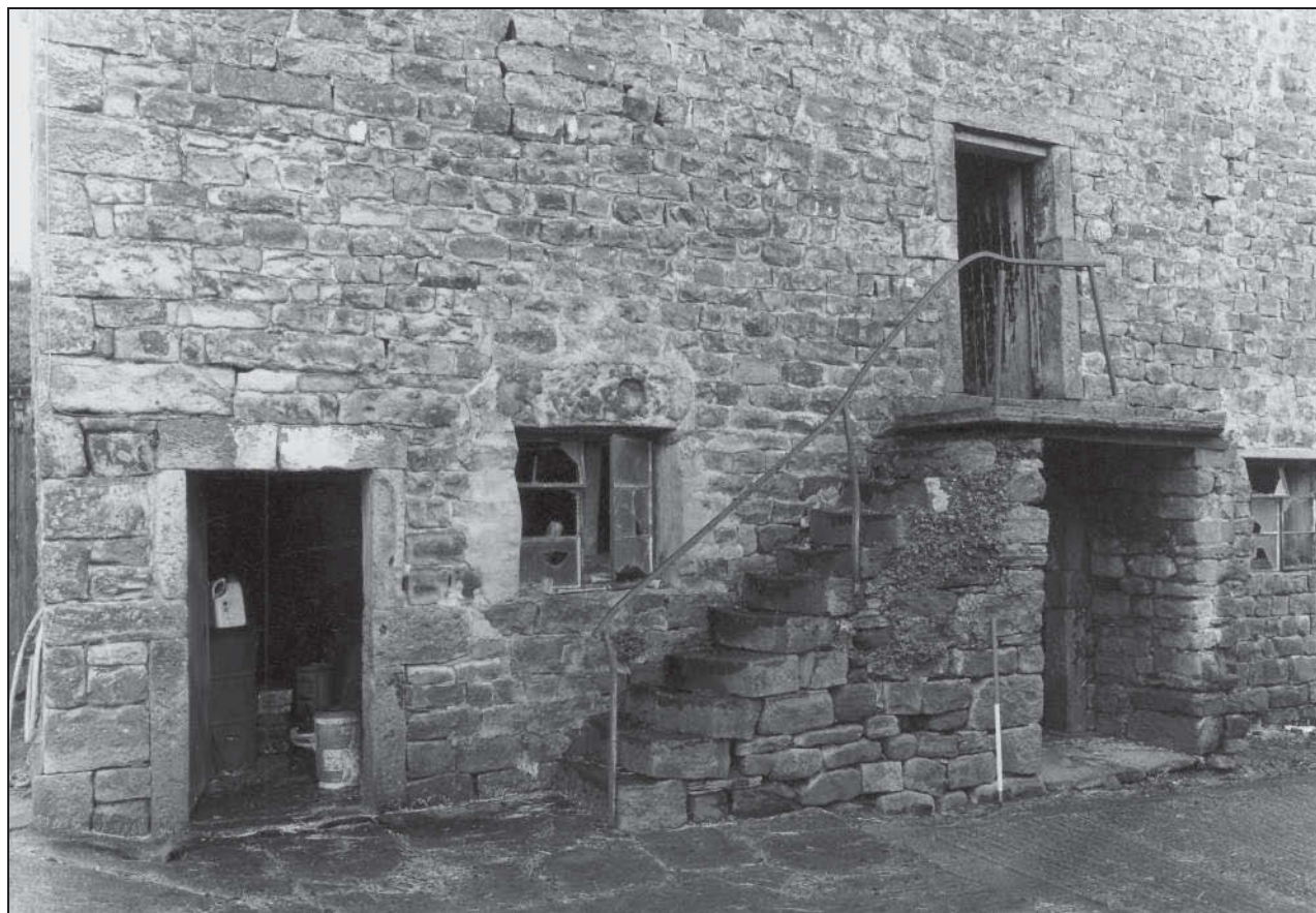
Photo 7: The bank barn: details of rear elevation, from the north-east
