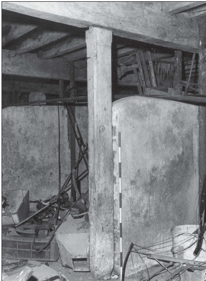
Photo 12: Bank barn: surviving oak heel post on ground floor
