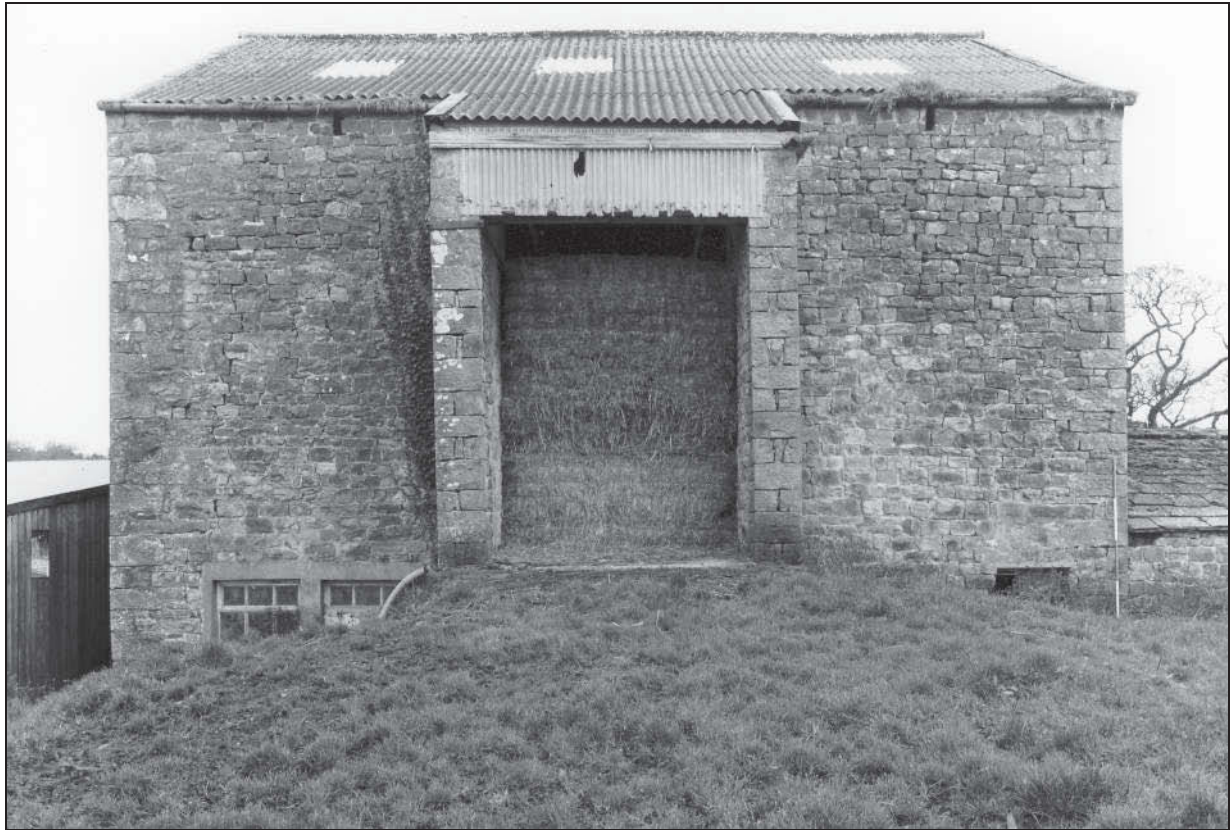
Photo 17: The bank barn: south elevation
