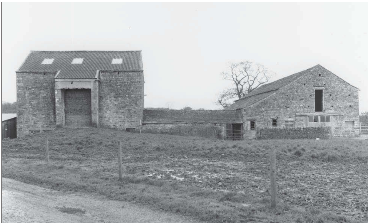
Photo 1: General view of the barn, cart shed, and earlier barn, from the south-east
