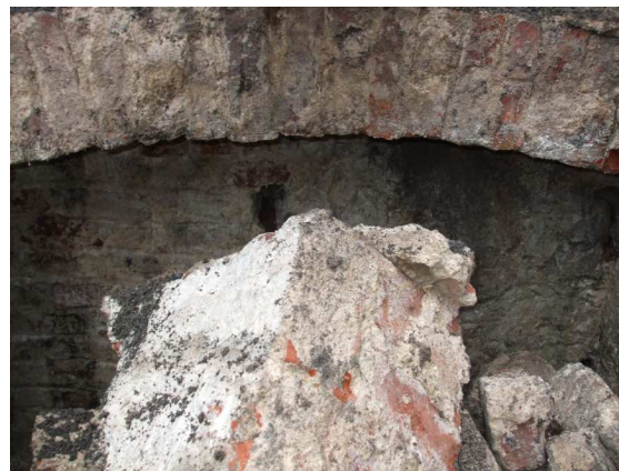
Plate 2: Brick alcove in Feature 1 facing south-west
