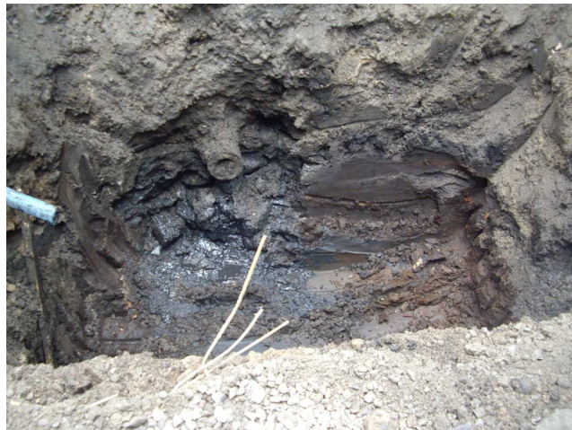
Plate 19: Organic material at base of trench (right), facing south-west
