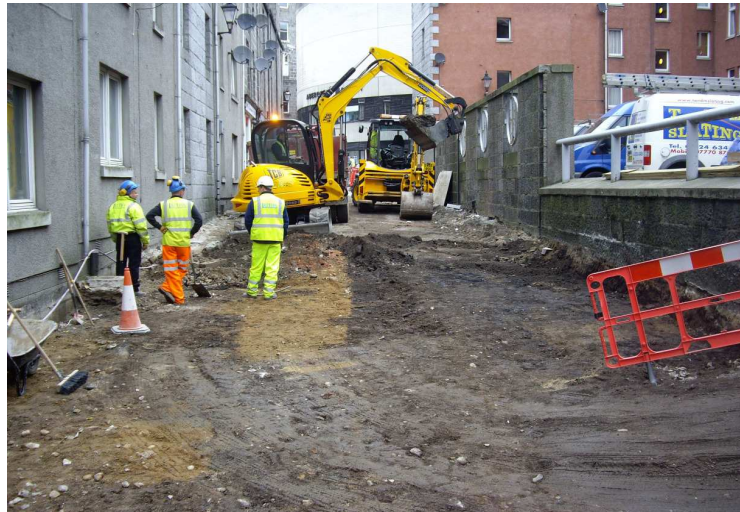
Plate 10: Excavations on Carmelite Street facing north
