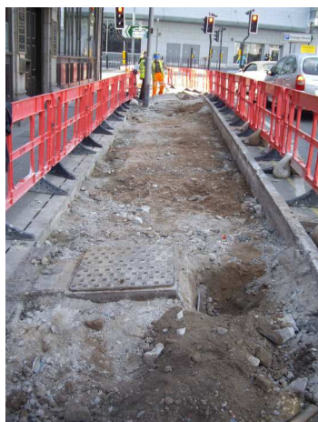
Plate 19: Excavations in the pavement on Wapping Street, facing south-west
