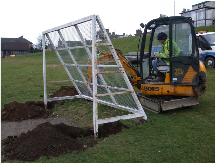
Illus 4 The small trenches for the removal of the goalposts
