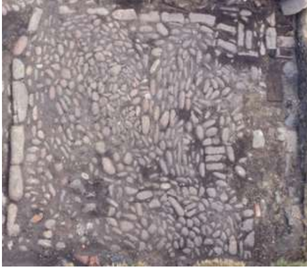
Illus 38 Building 3: Cobbled surface BF showing circular patterns made during laying
