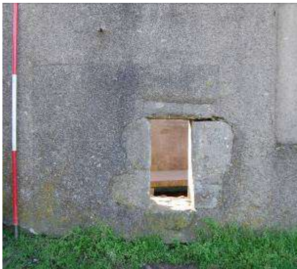
Illus 53 North wall: W4 (centre) with scar of W6, left and infilled window W3, right
