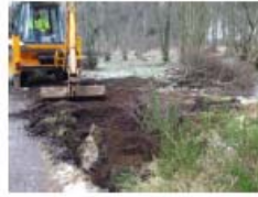
Tr 5 being backfilled
