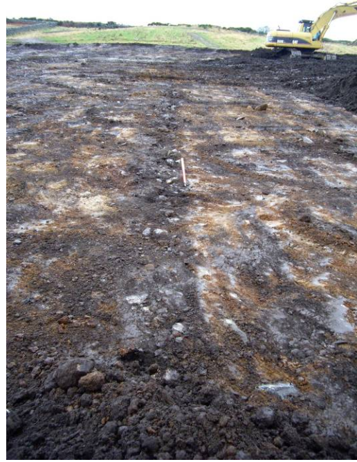
III 6 Central field drain facing west
