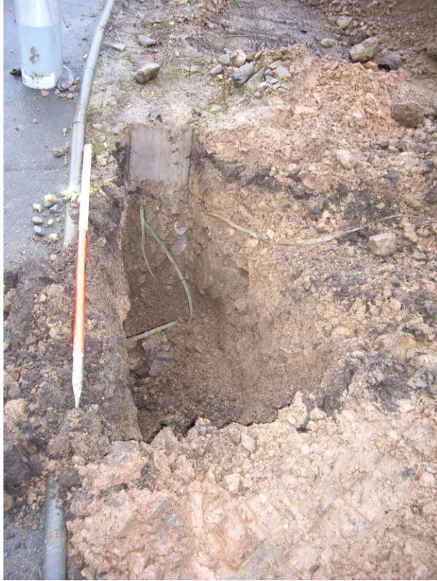
III 4 Pit excavated for fence posts, facing east
