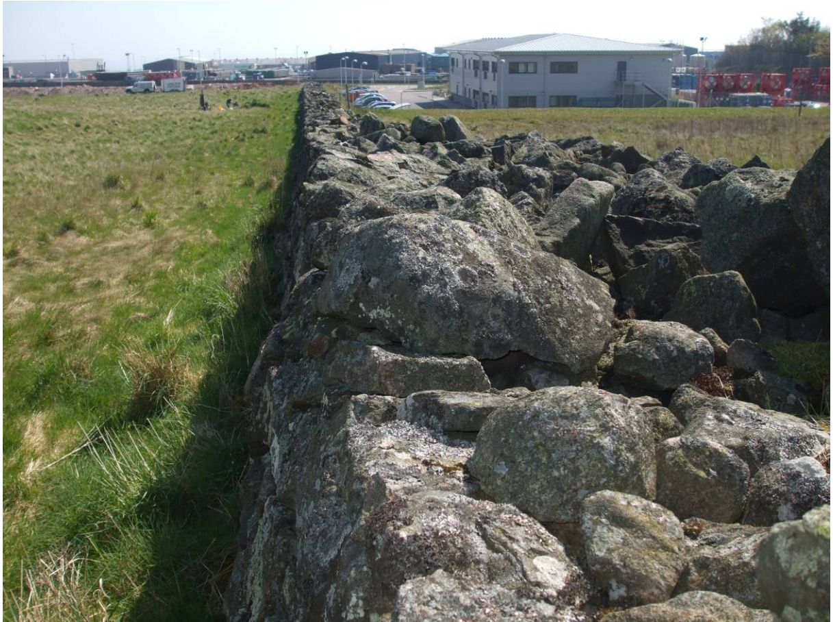
Ill 1 Consumption dyke NJ90SE 0027 facing south). The site is on the left.
